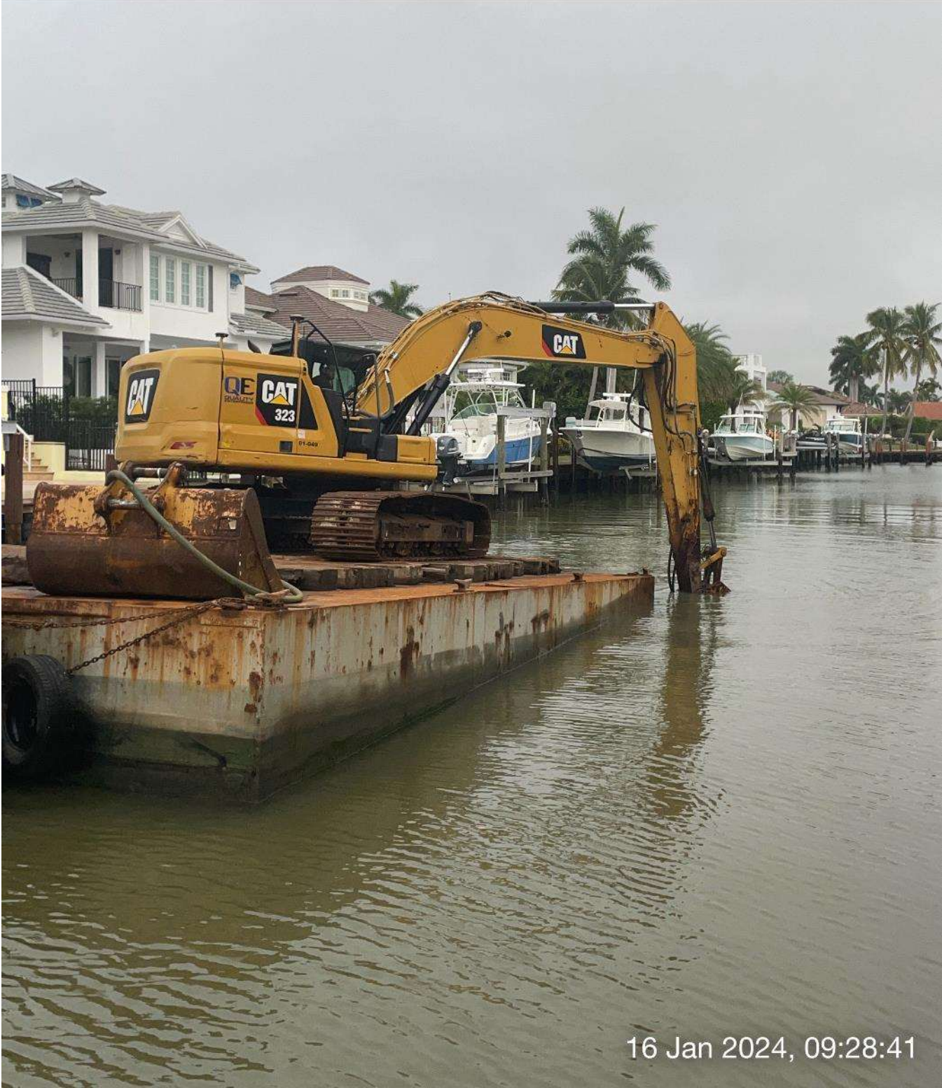
323 excavator grinding rock at station 7+75 in Canal A-A.
