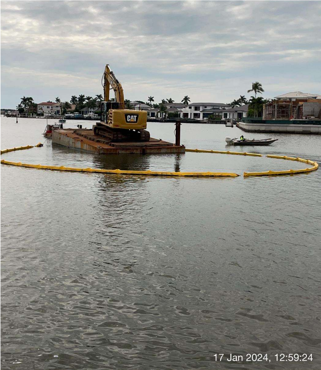
Turbidity curtain in place around the barge.
