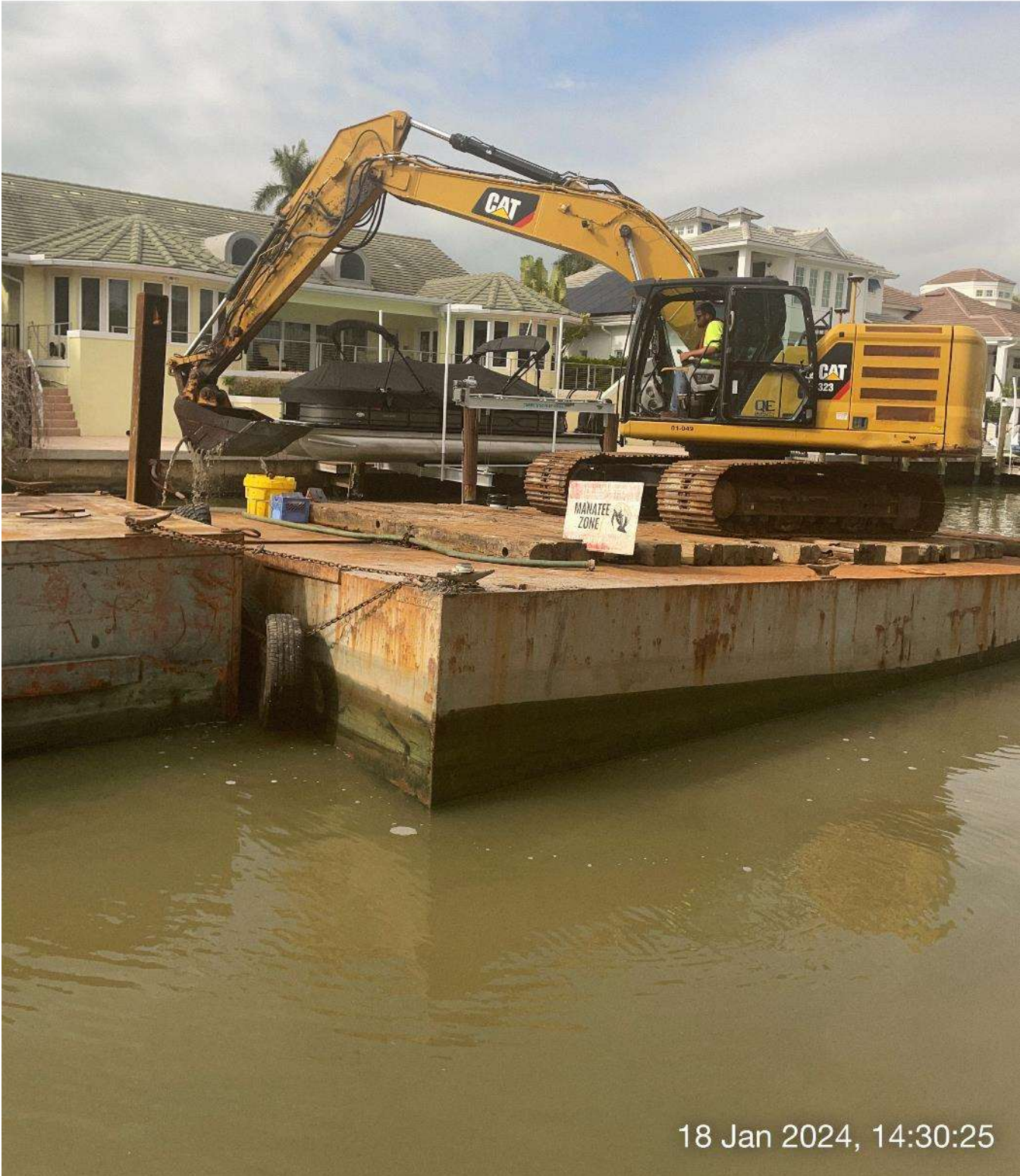
323 excavator removing sediment at station 8+00 in Canal A-A.
