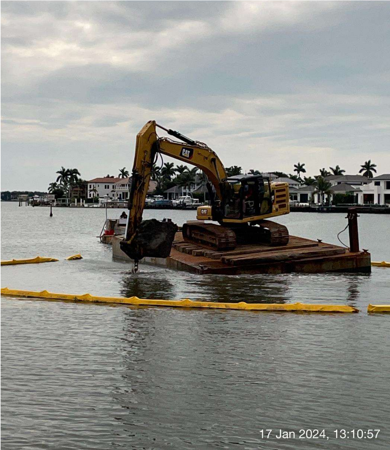
323 excavator removing sediment at station 2+50 in Canal Main B.
