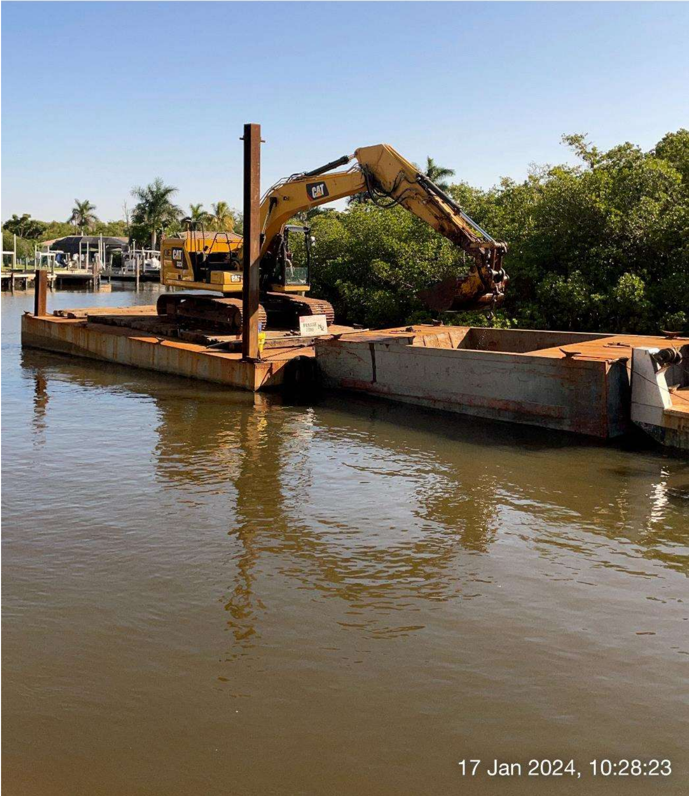
323 excavator removing sediment at station 8+00 in Canal Main B.
