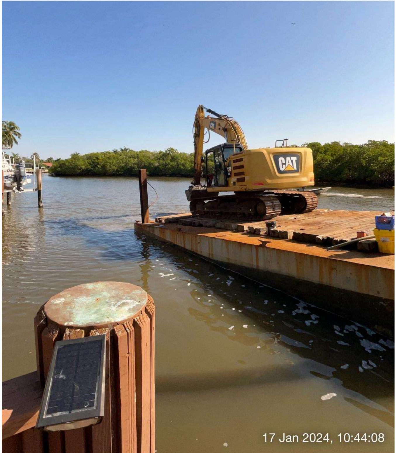
323 excavator removing sediment at station 3+25 in Canal Main B.
