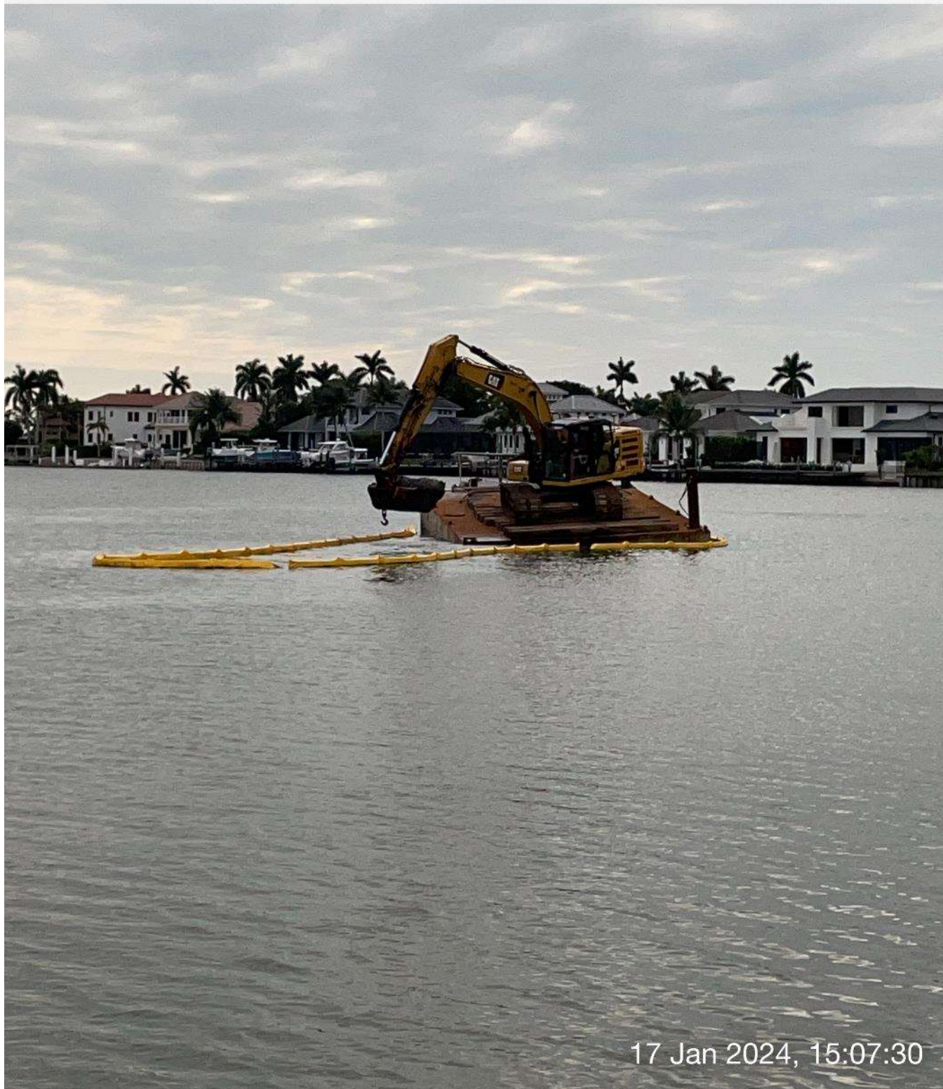
323 excavator removing sediment at station 2+00 in Canal Main B.
