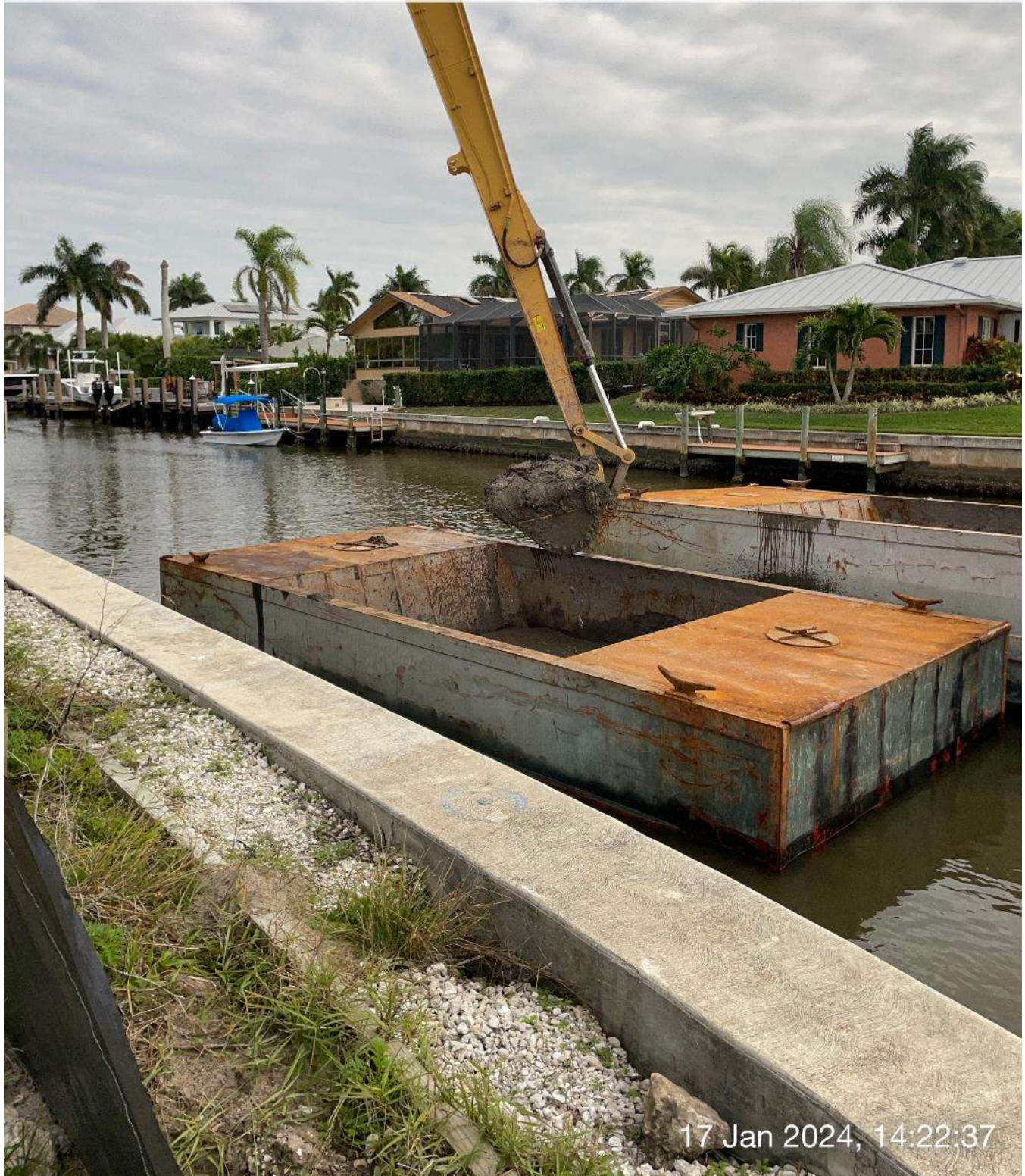
Long reach excavator removing sediment from hopper.
