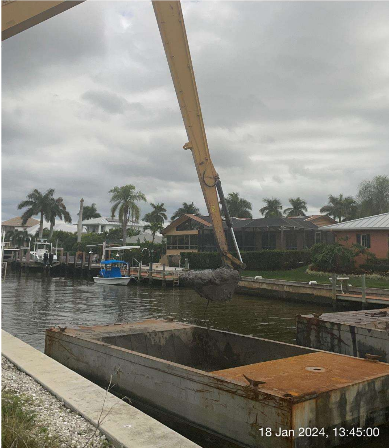
Long reach excavator removing sediment from hopper.
