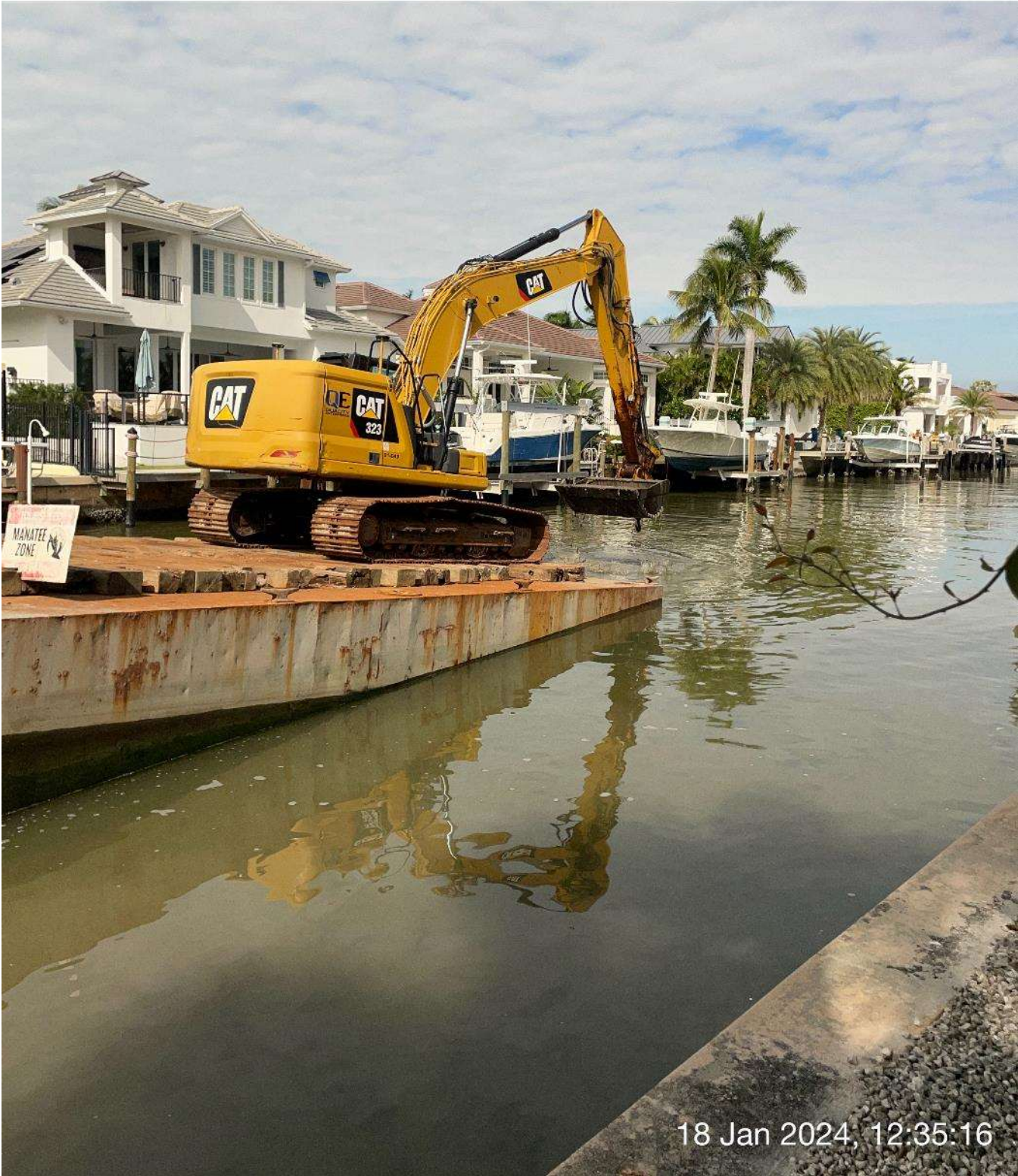
323 excavator removing sediment at station 8+50 in Canal A-A.
