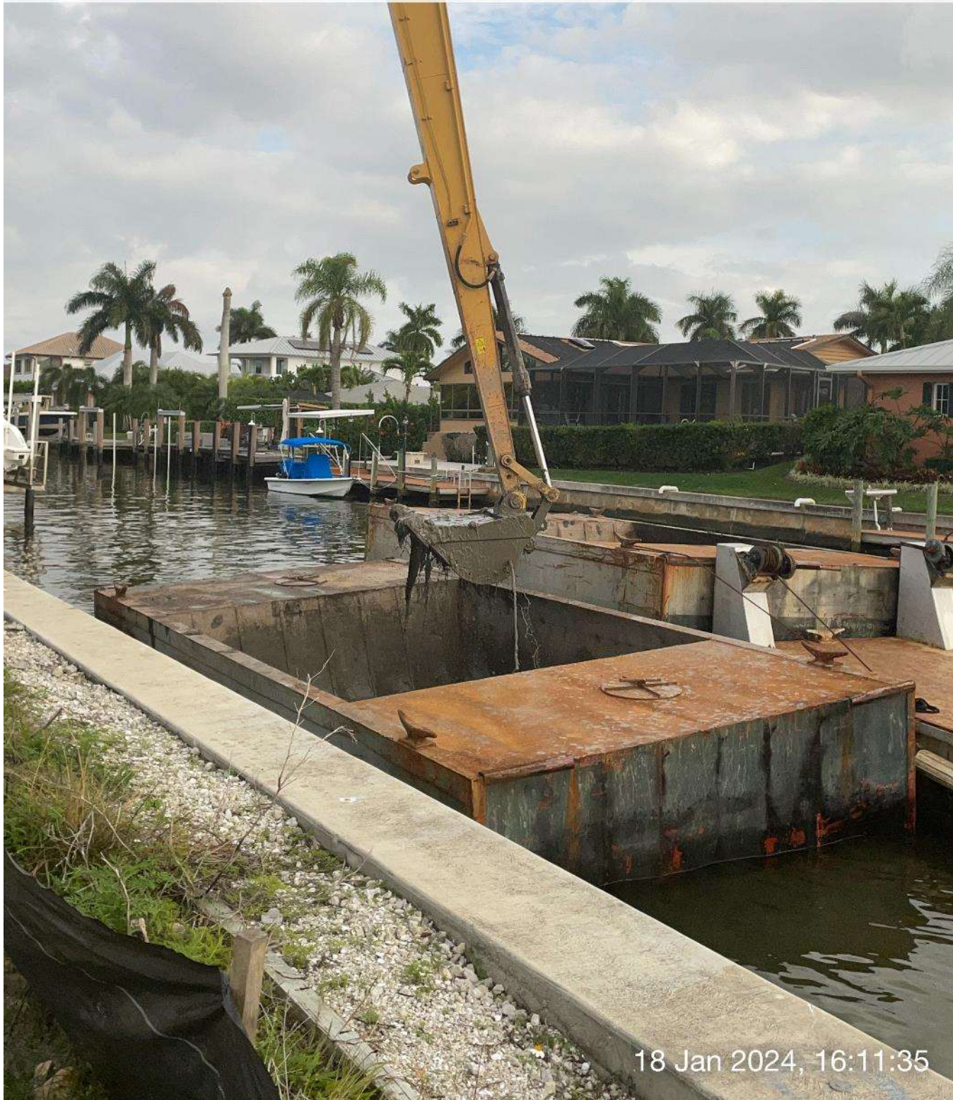
Long reach excavator removing sediment from hopper.
