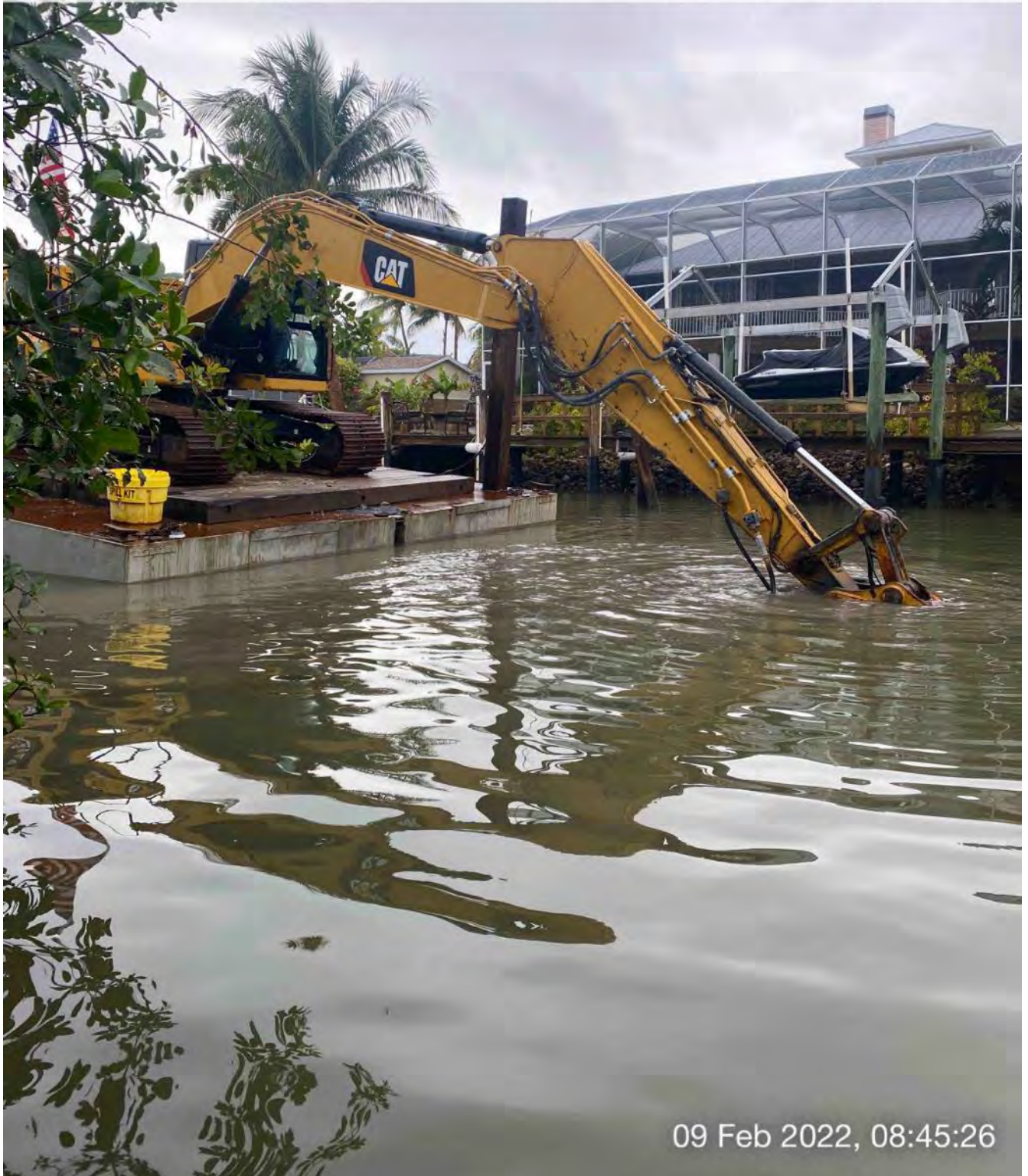
323 excavator grinding rock at station 9+50
