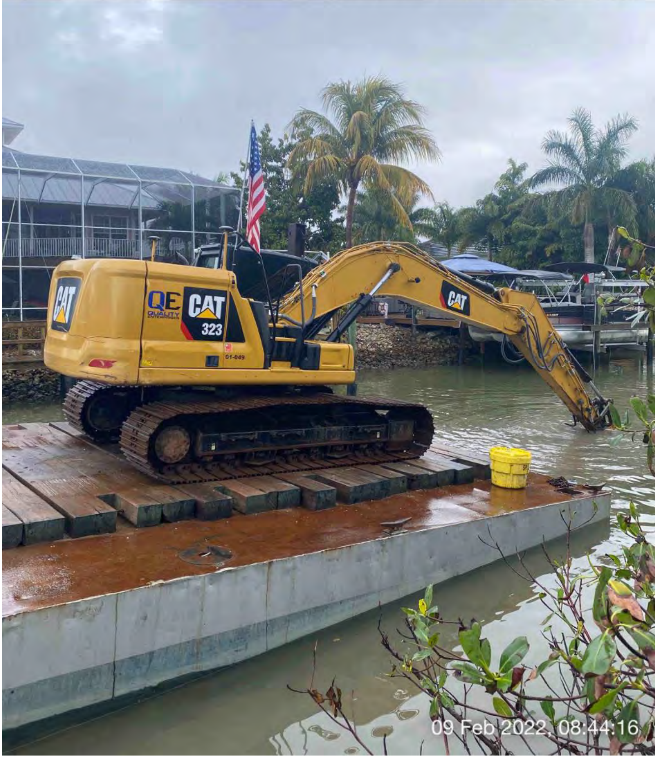
323 excavator grinding rock at station 9+50
