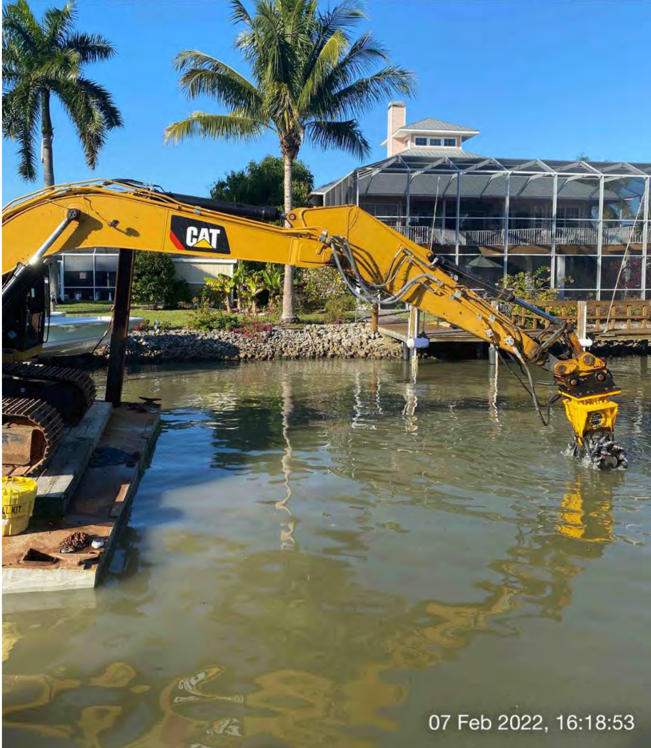
323 excavator grinding rock at station 9+00
