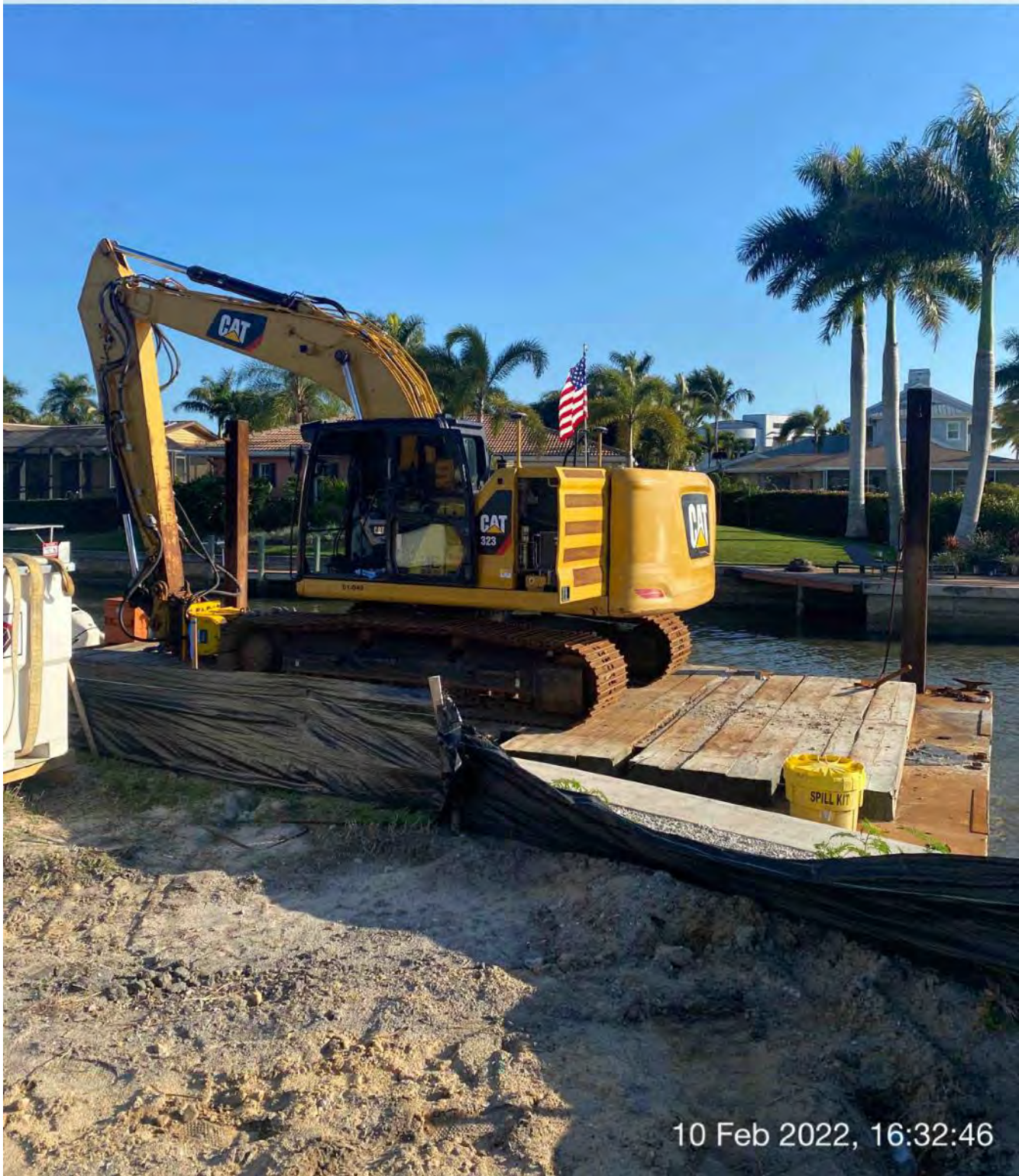
323 excavator and barge stationed in Canal CC-CC at station 1+50
