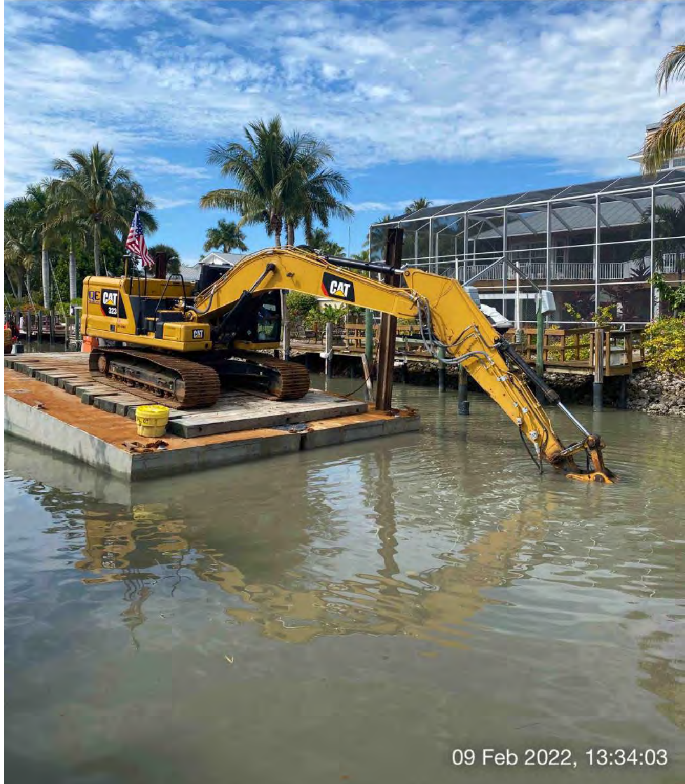
323 excavator grinding rock at station 9+75
