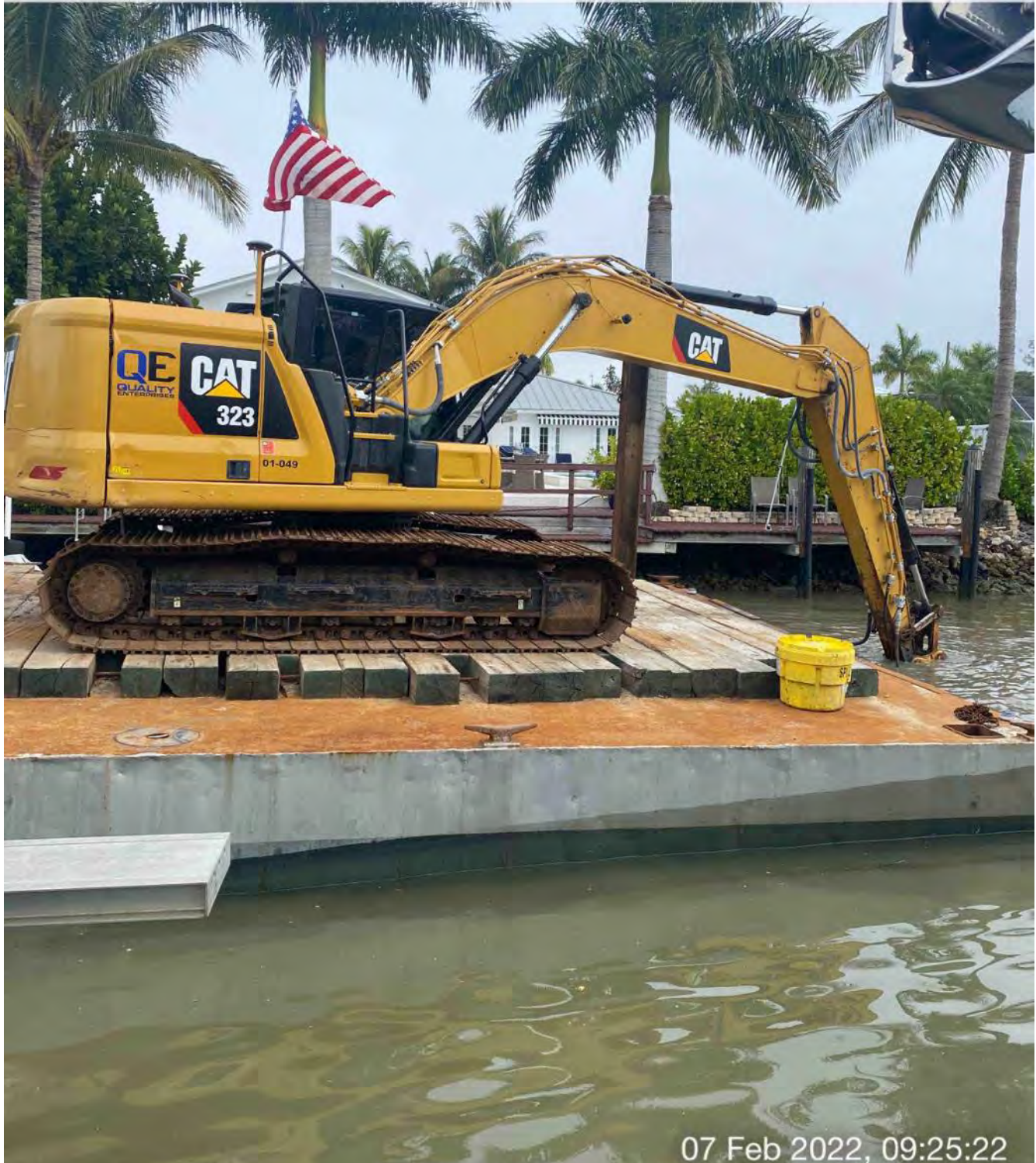
323 excavator grinding rock at station 8+25
