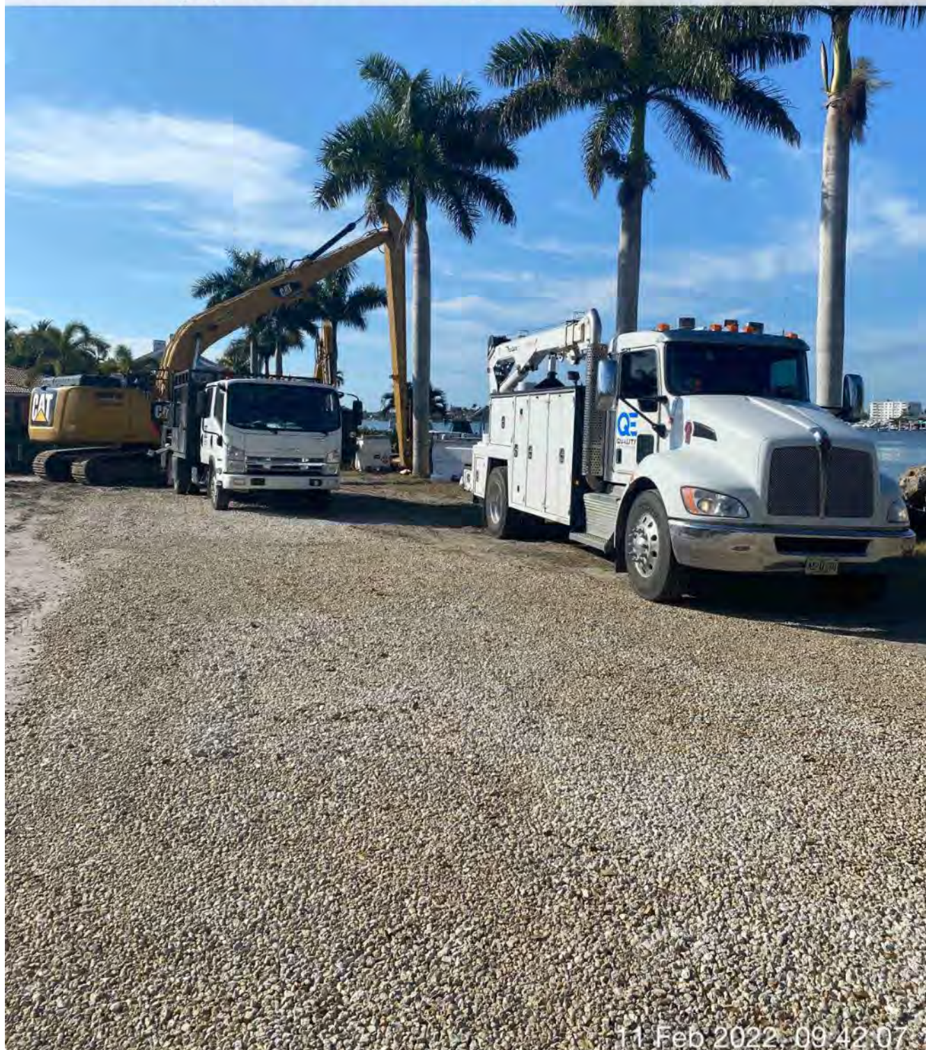
Mechanic trucks on site at 1300 Curlew Avenue
