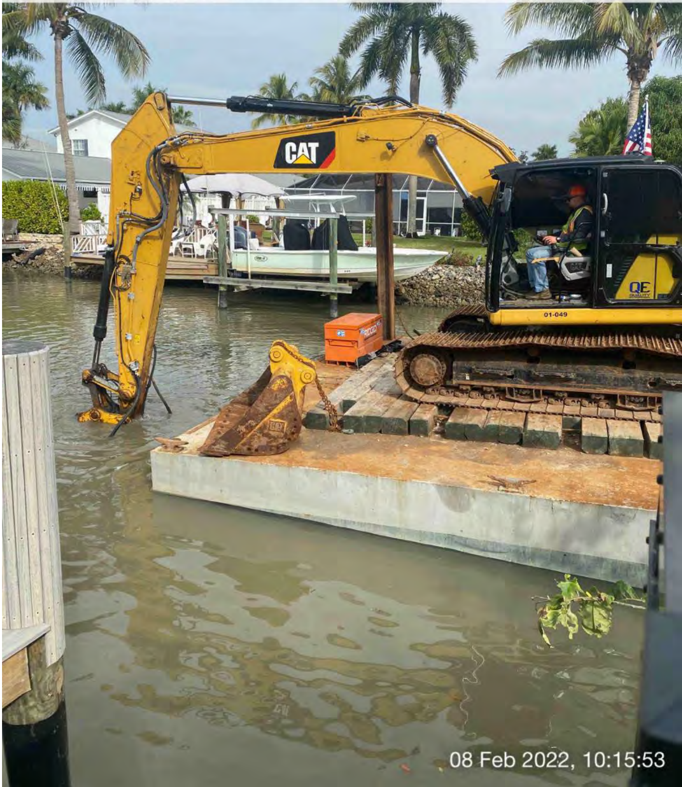
323 excavator grinding rock at station 8+75
