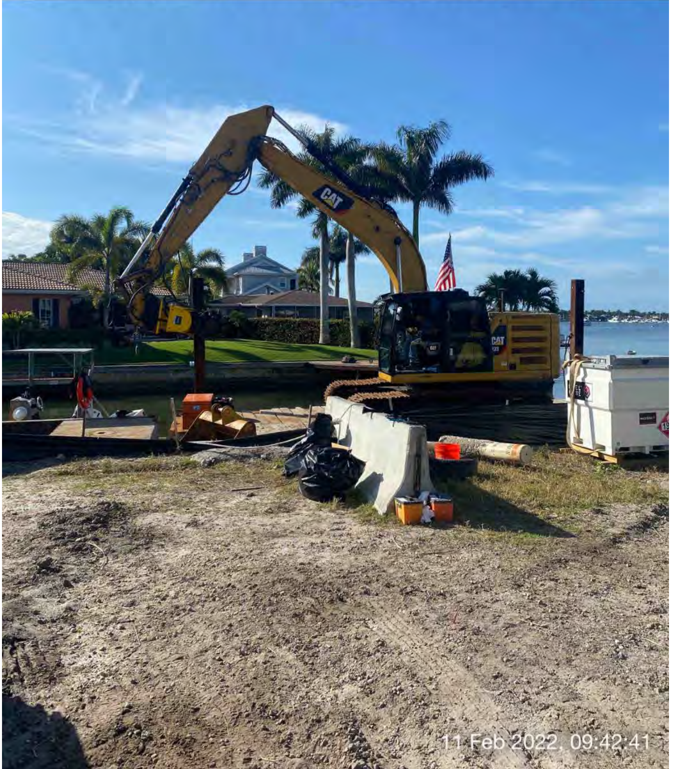
Mechanic checking operation of 323 excavator
