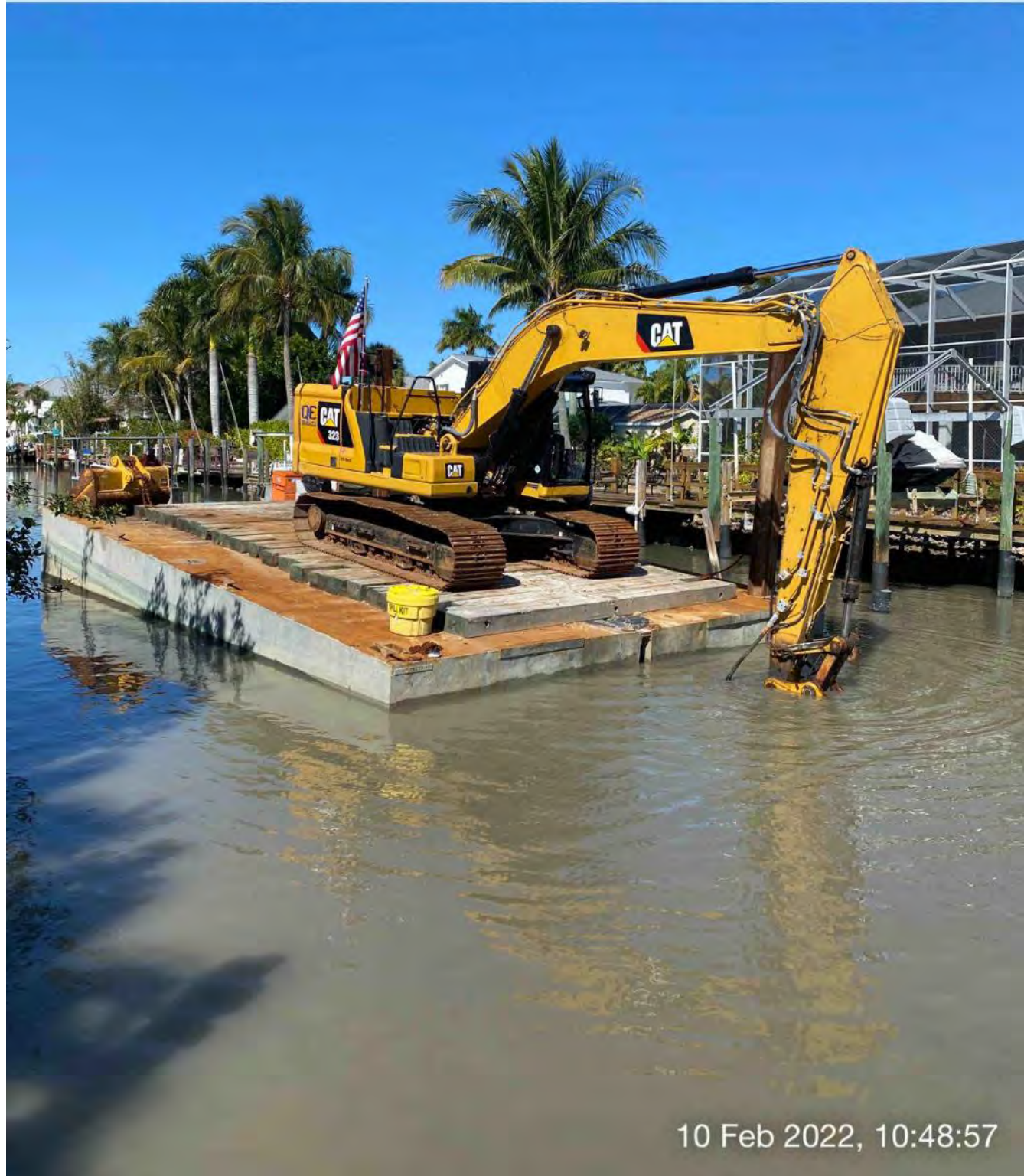
323 excavator grinding rock at station 9+50
