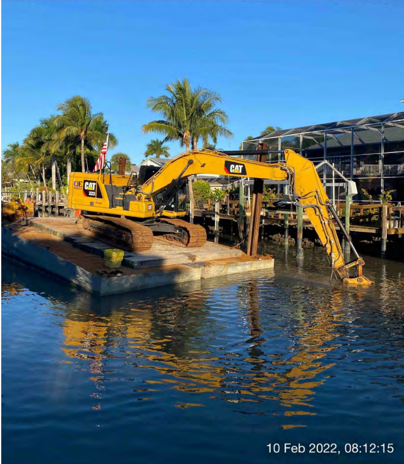
323 excavator grinding rock at station 9+50
