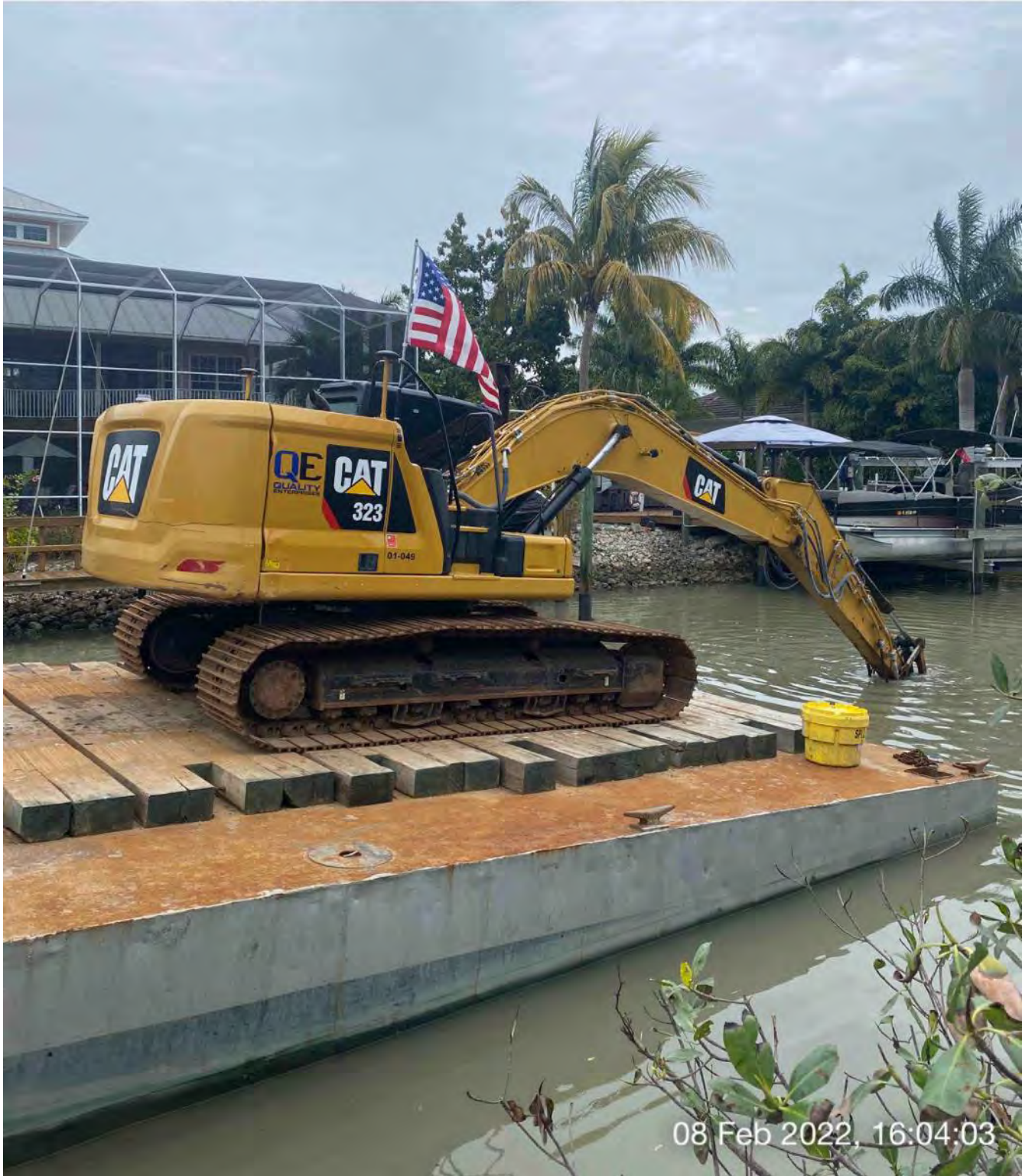
323 excavator grinding rock at station 9+50
