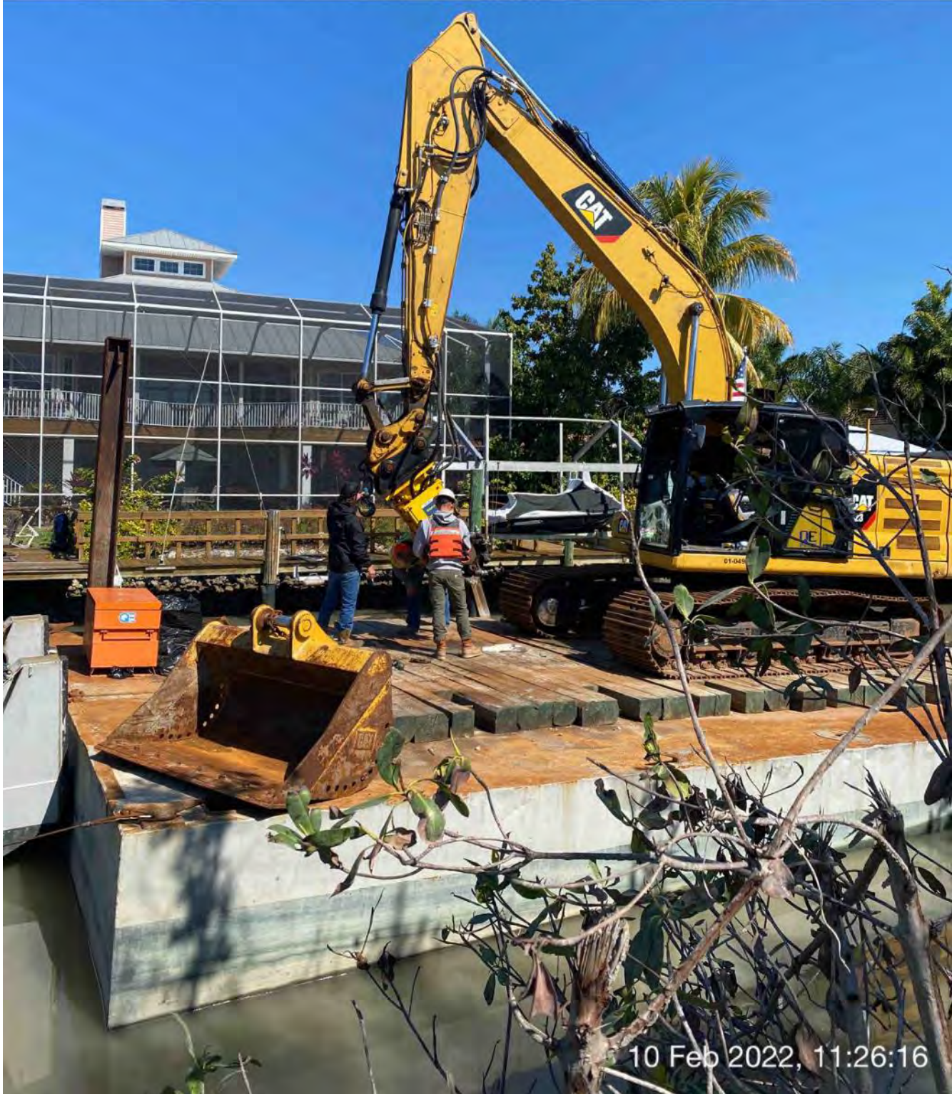
Contractor changing teeth on the Epiroc grinder
