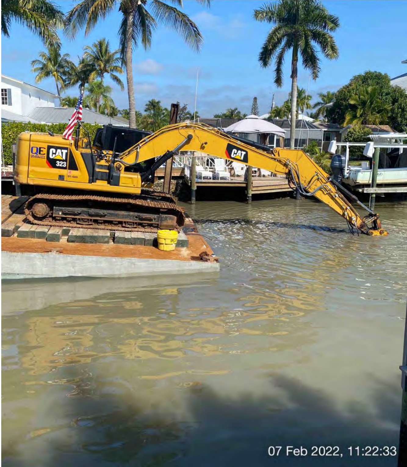
323 excavator grinding rock at station 8+50
