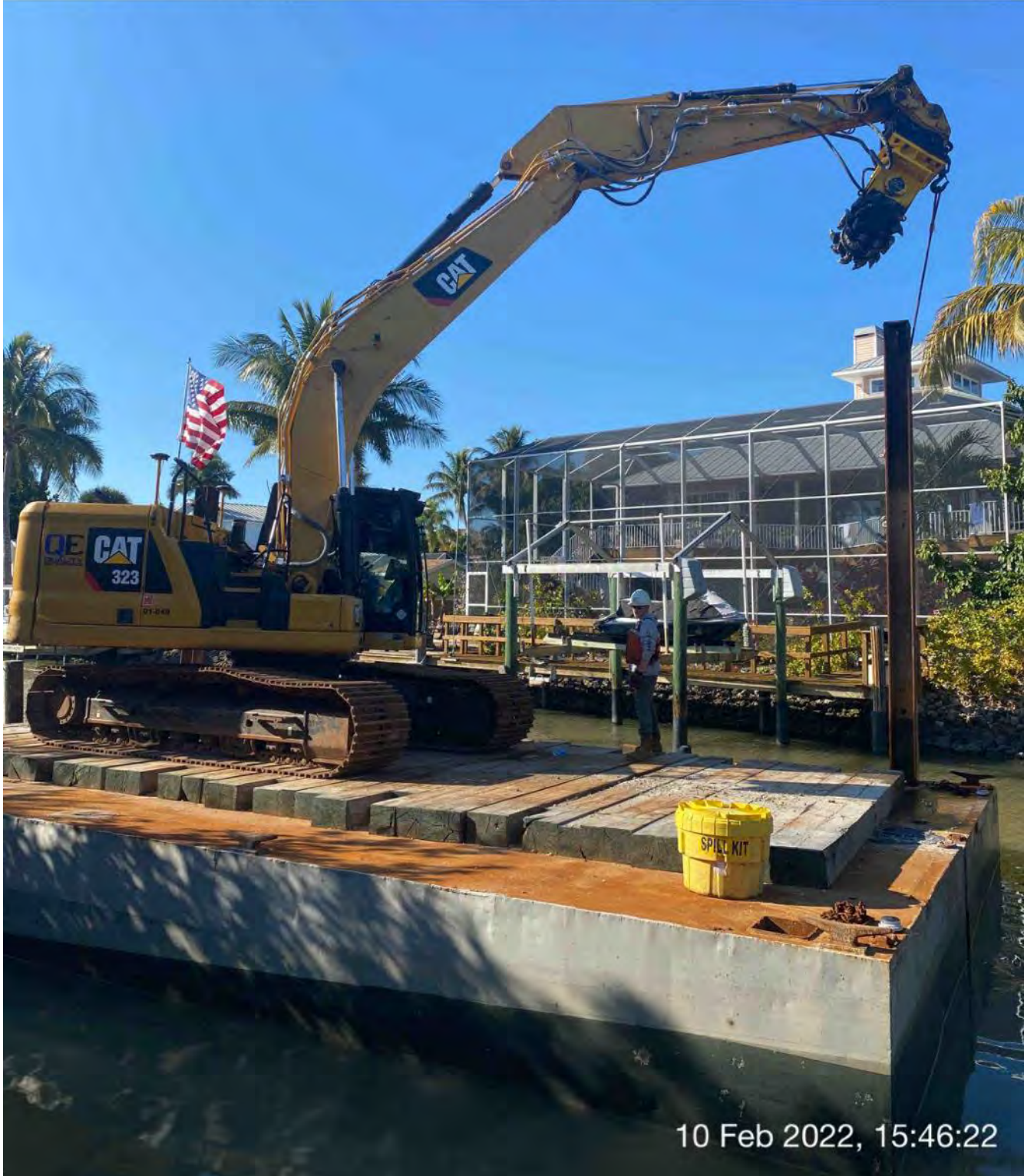
323 excavator lifting spud to allow push boat to mobilize barge at station 9+50
