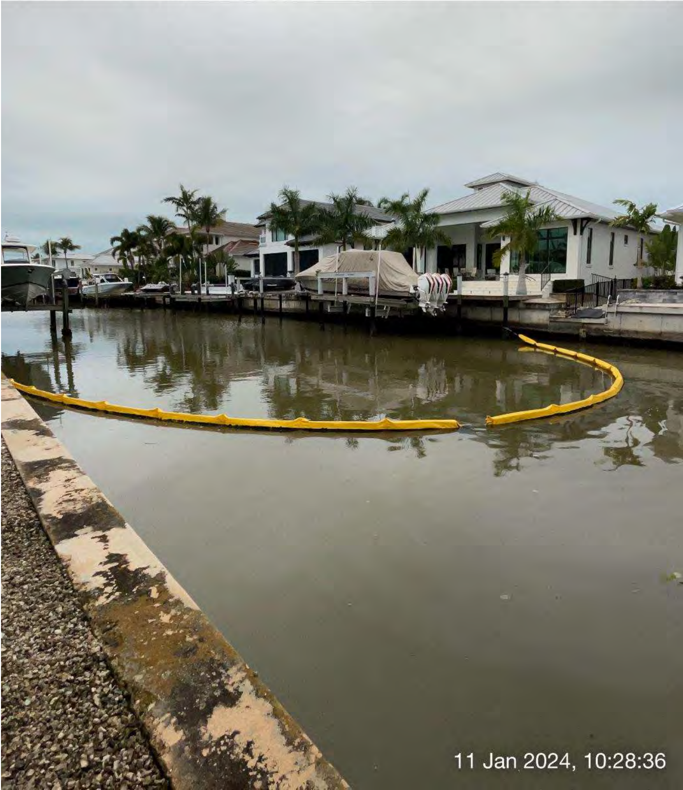
Turbidity curtain in place at station 5+50 in Canal A-A.
