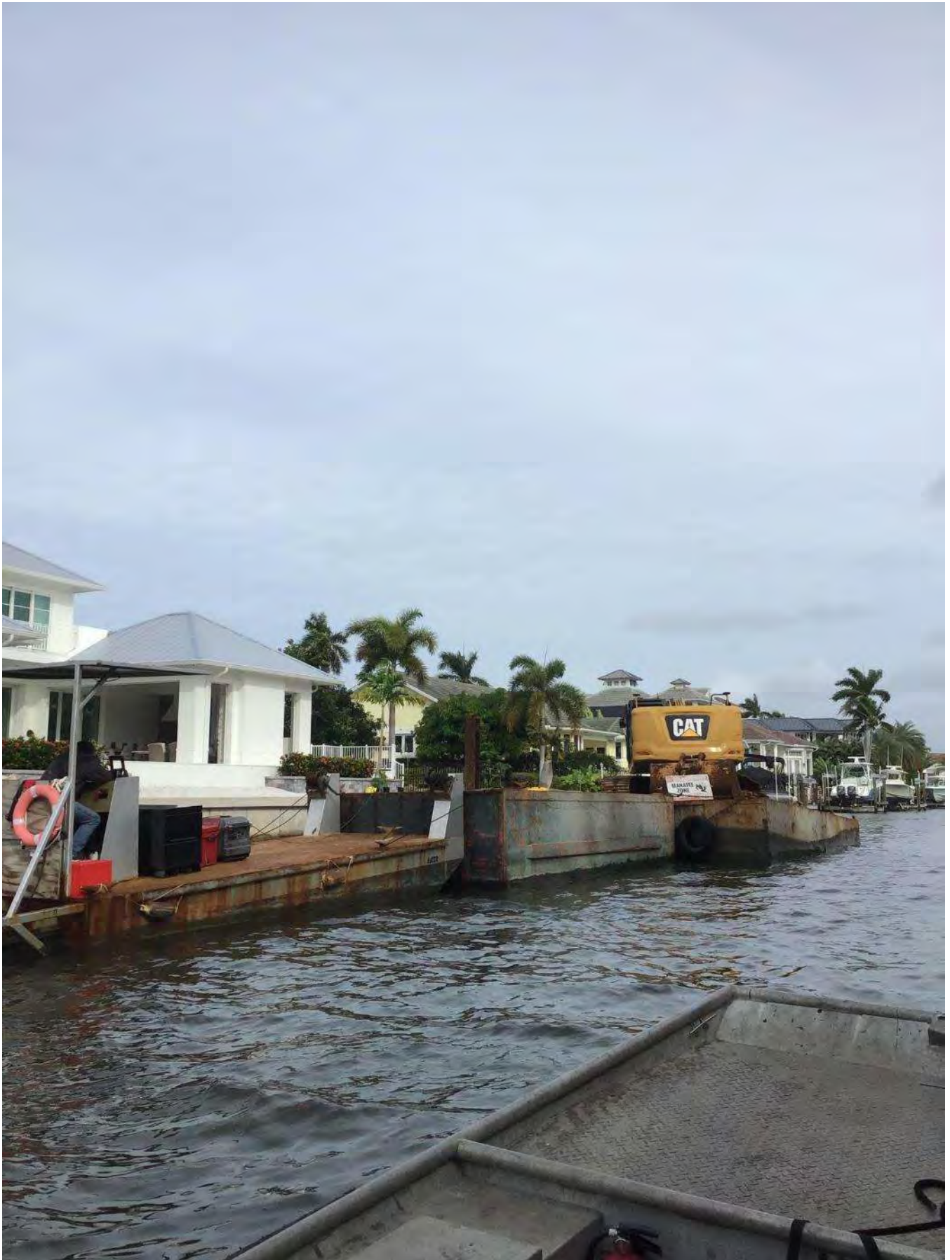
323 excavator grinding rock at station 6+00 in Canal A-A.
