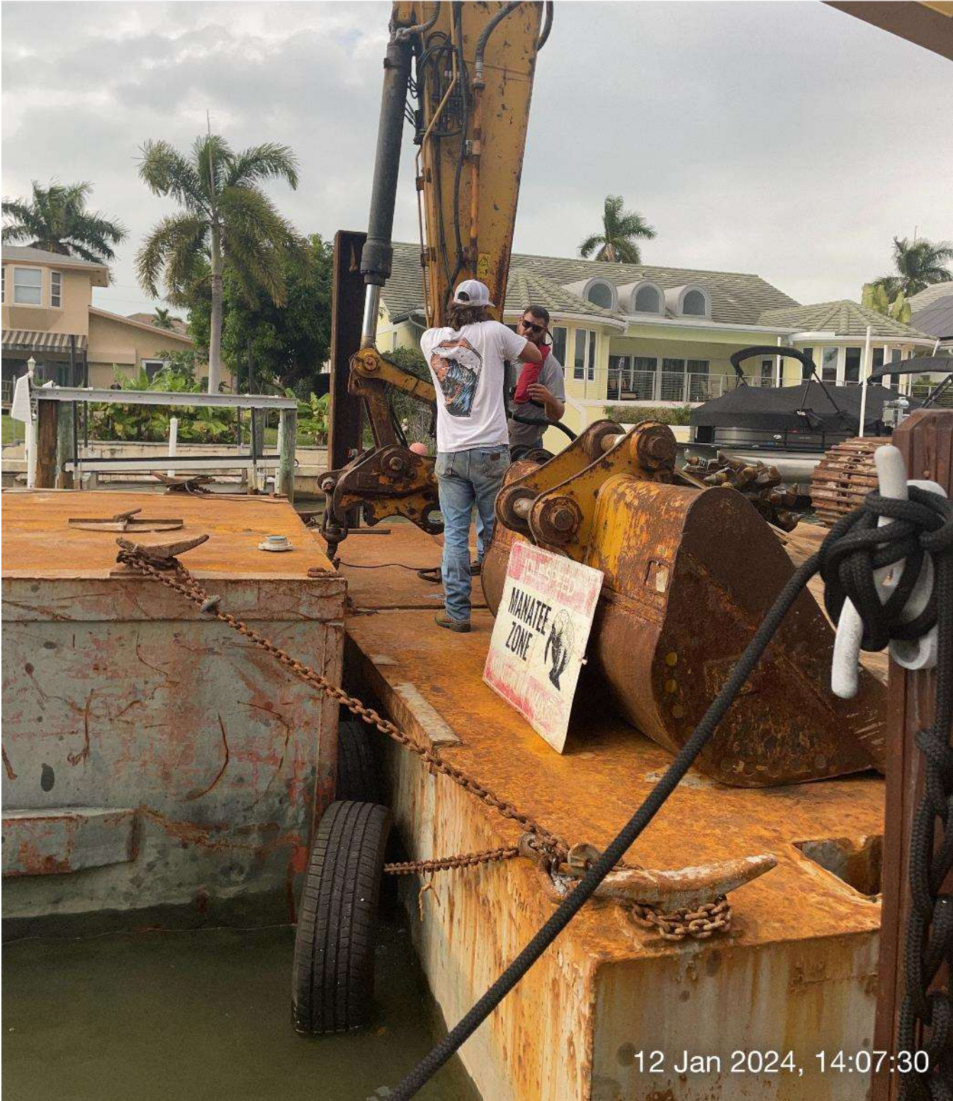
Contractor removing Epiroc grinder from 323 excavator.
