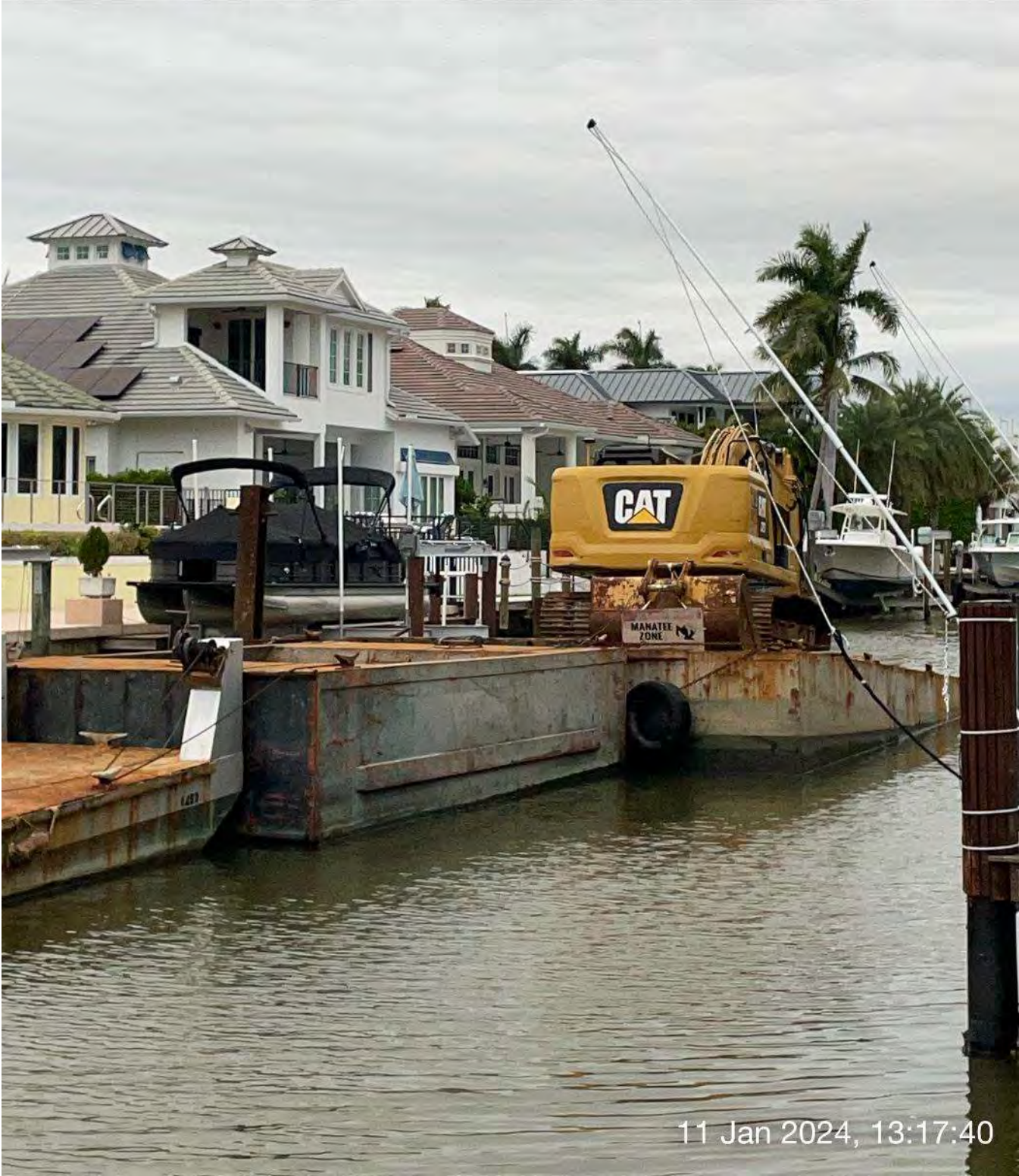
323 excavator grinding rock at station 7+50 in Canal A-A.
