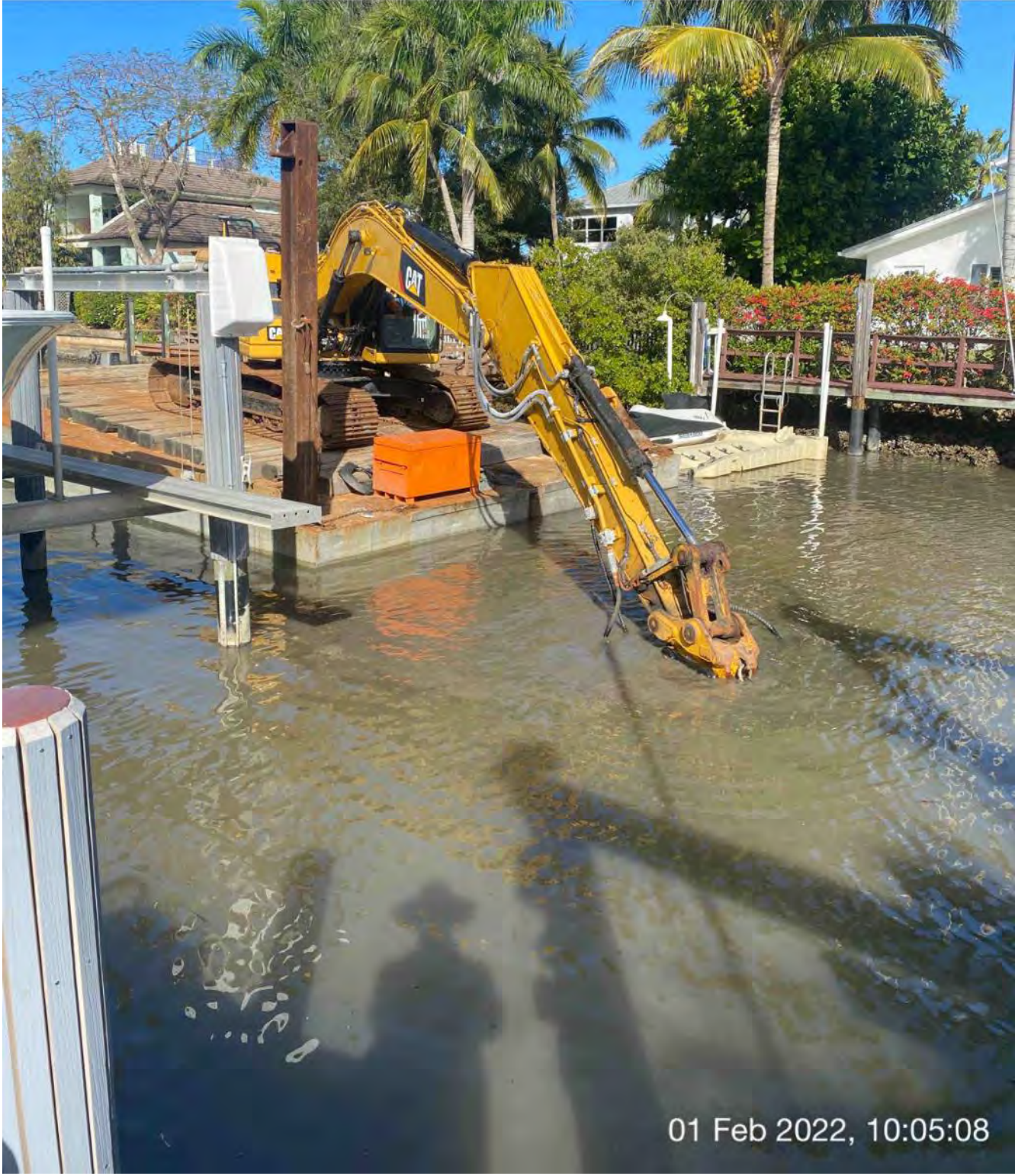
323 excavator grinding rock at station 7+50
