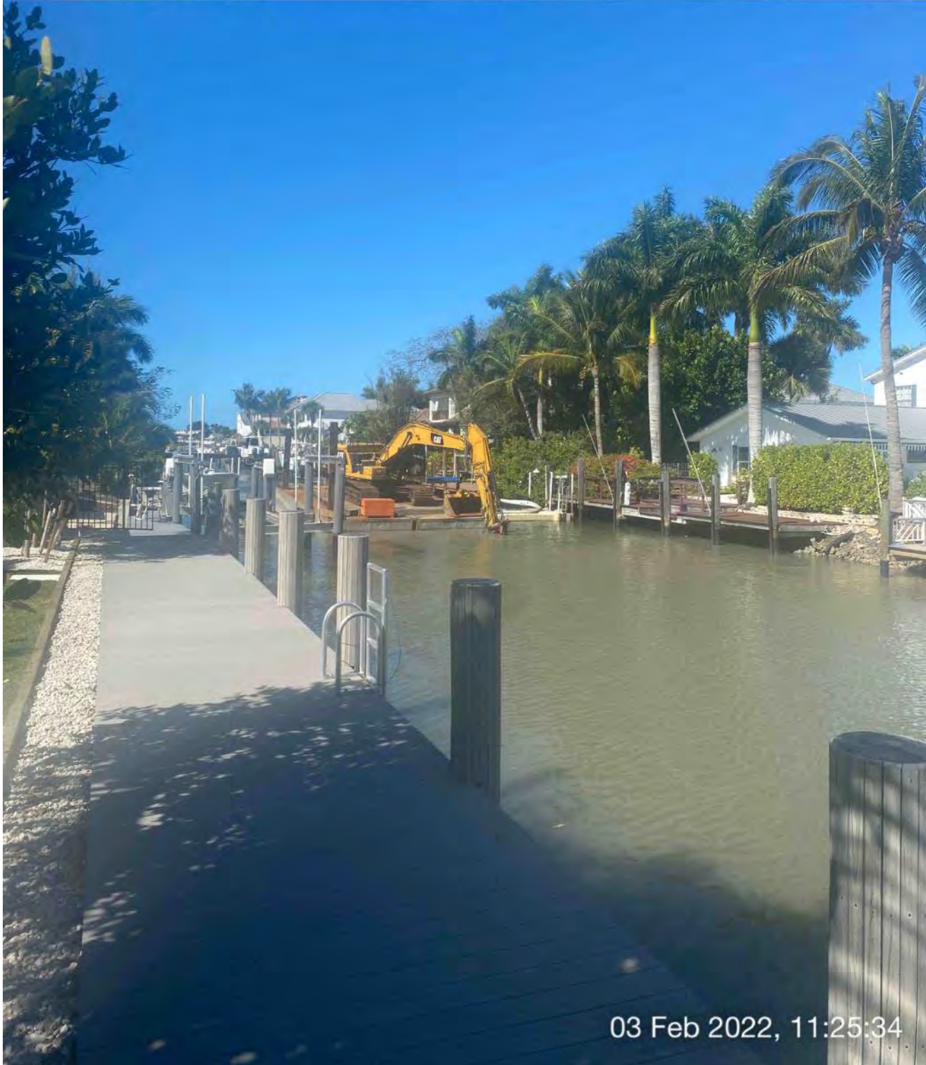
323 excavator grinding rock at station 7+75
