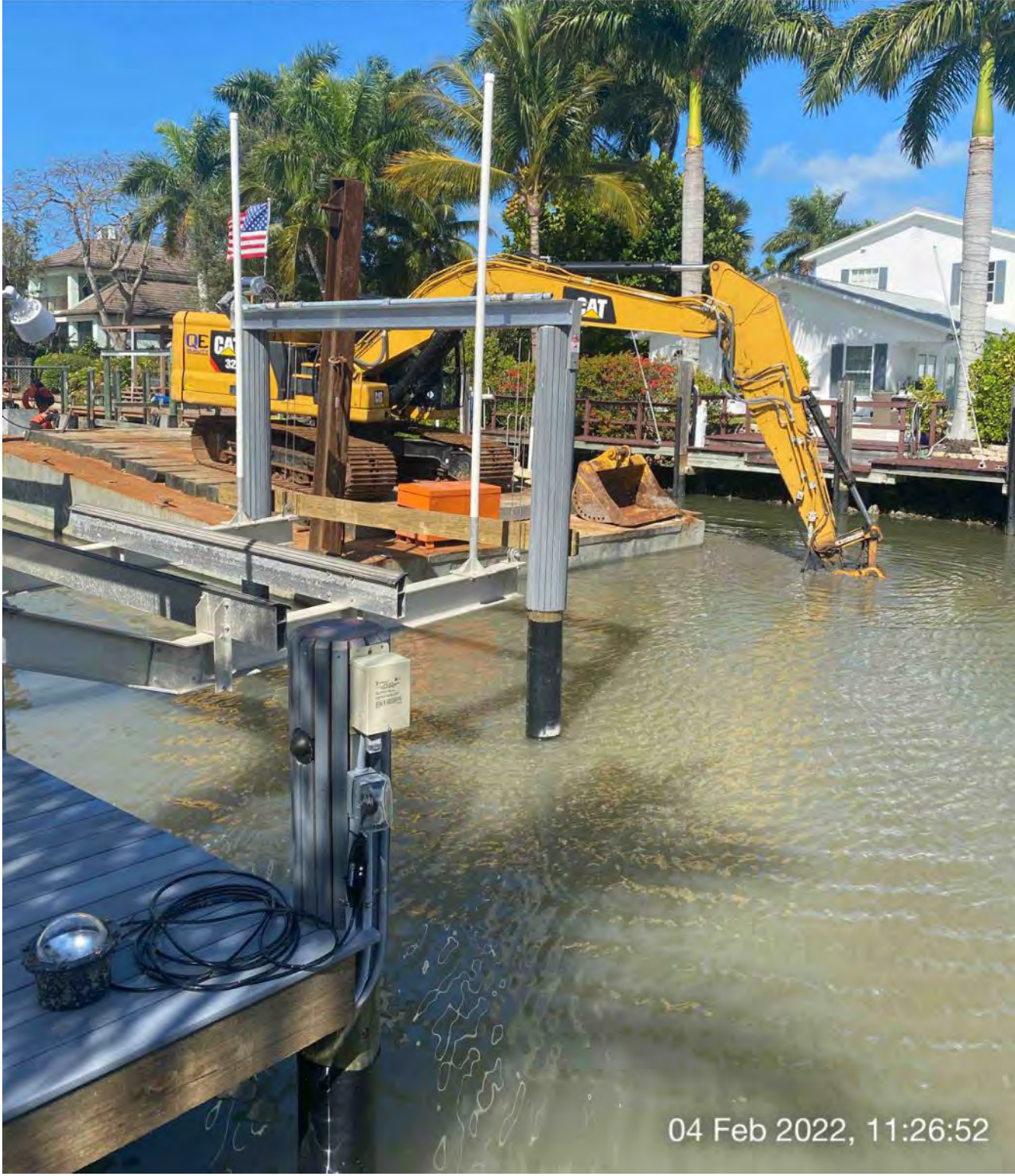
323 excavator grinding rock at station 8+00
