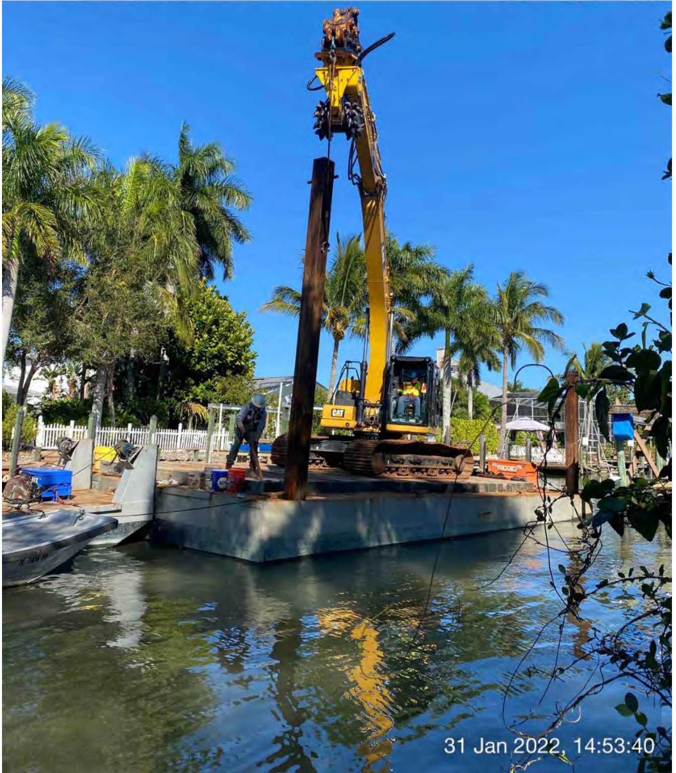
323 excavator lifting spud to allow push boat to mobilize barge at station 7+25
