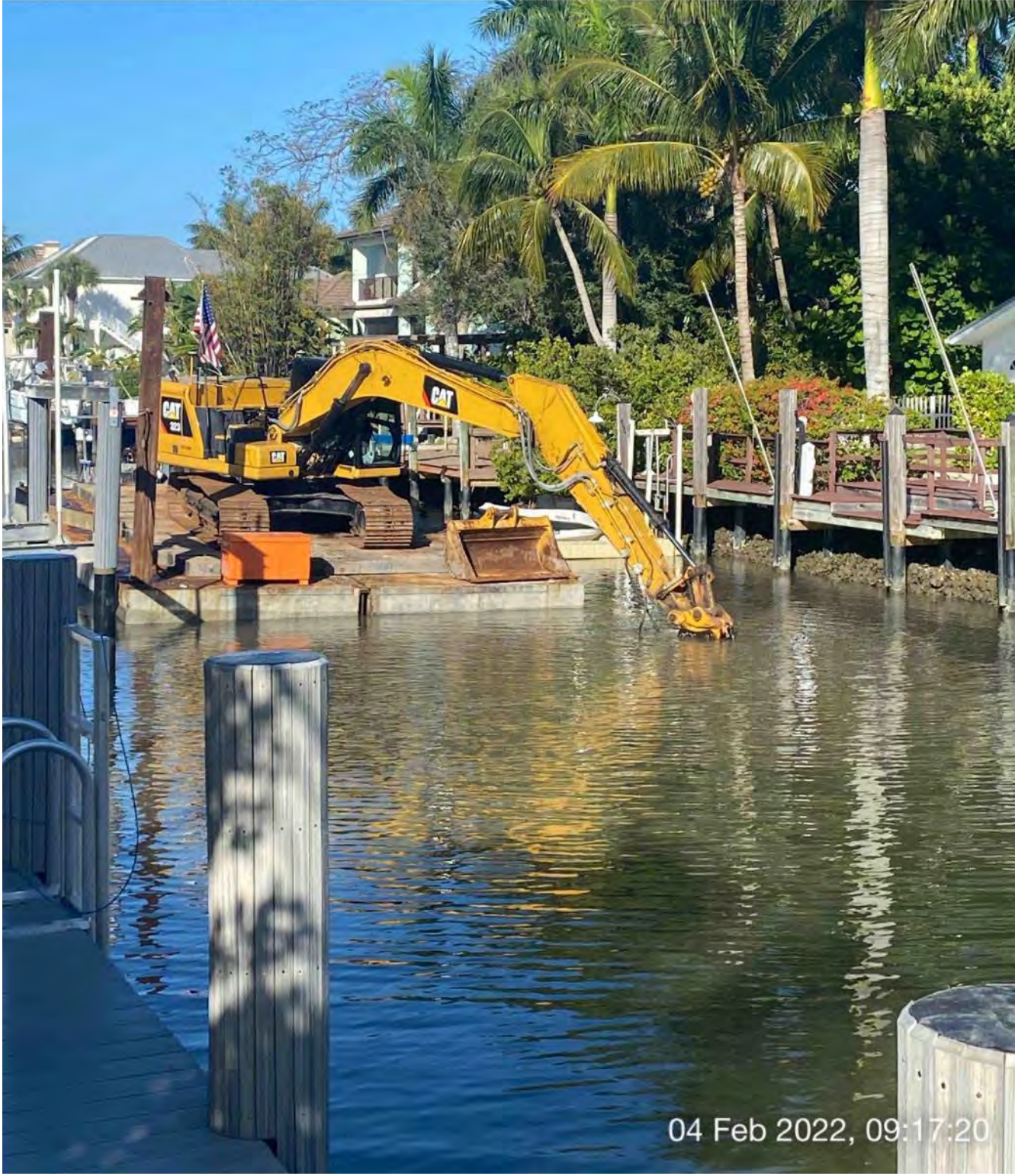
323 excavator grinding rock at station 8+00
