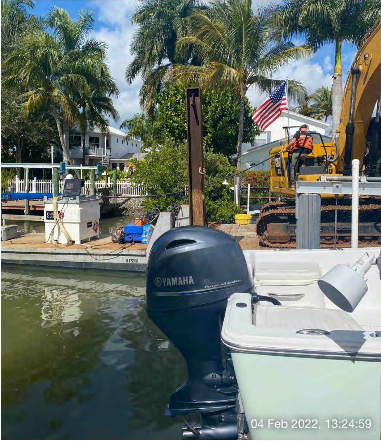
Refueling 323 excavator with small fuel cube
