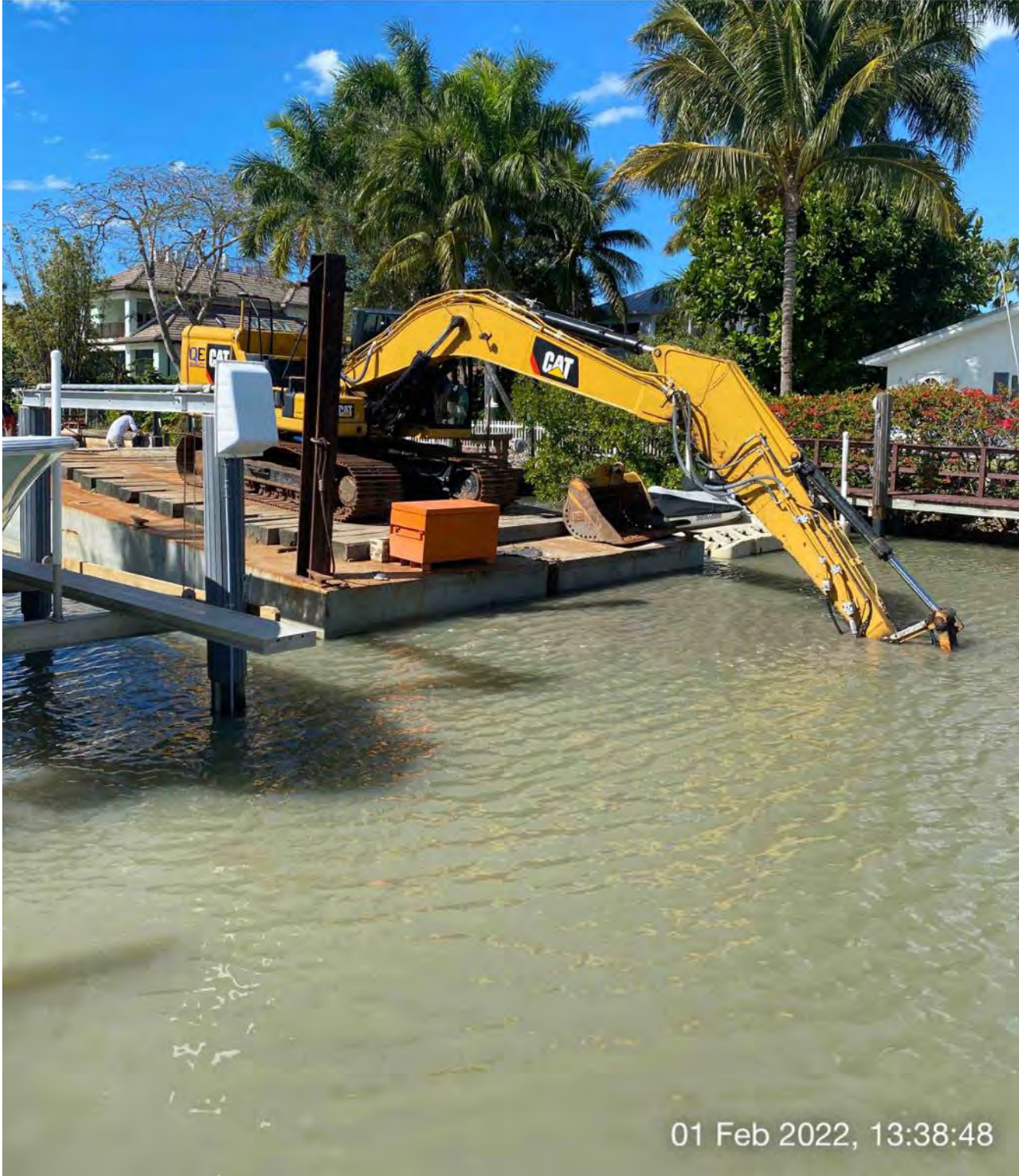
323 excavator grinding rock at station 7+50
