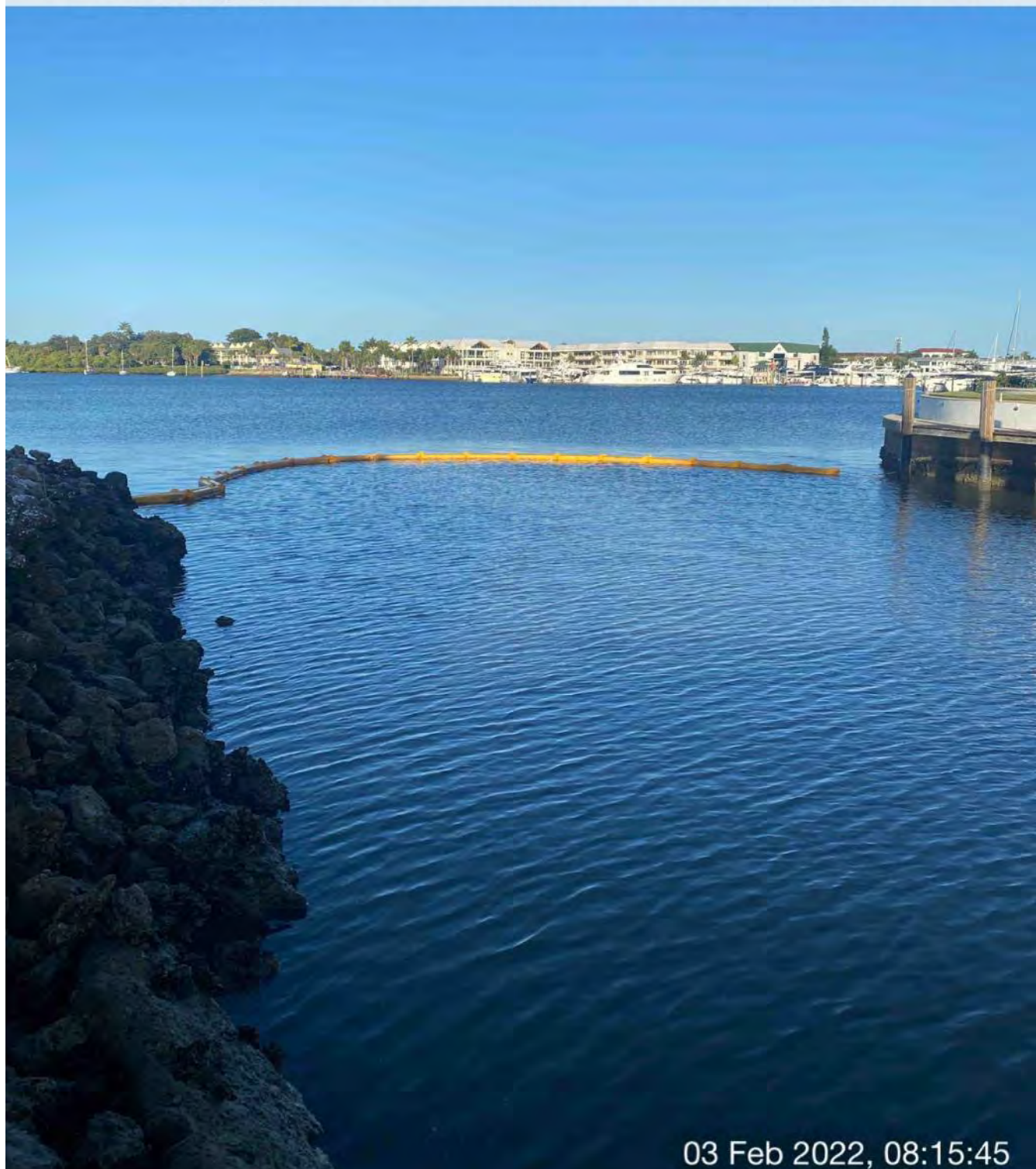
Turbidity curtain across the mouth of Canal BB-BB
