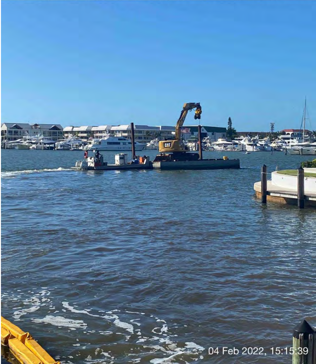
Push boat transporting barge and 323 excavator from Canal BB-BB to Canal CC-CC
