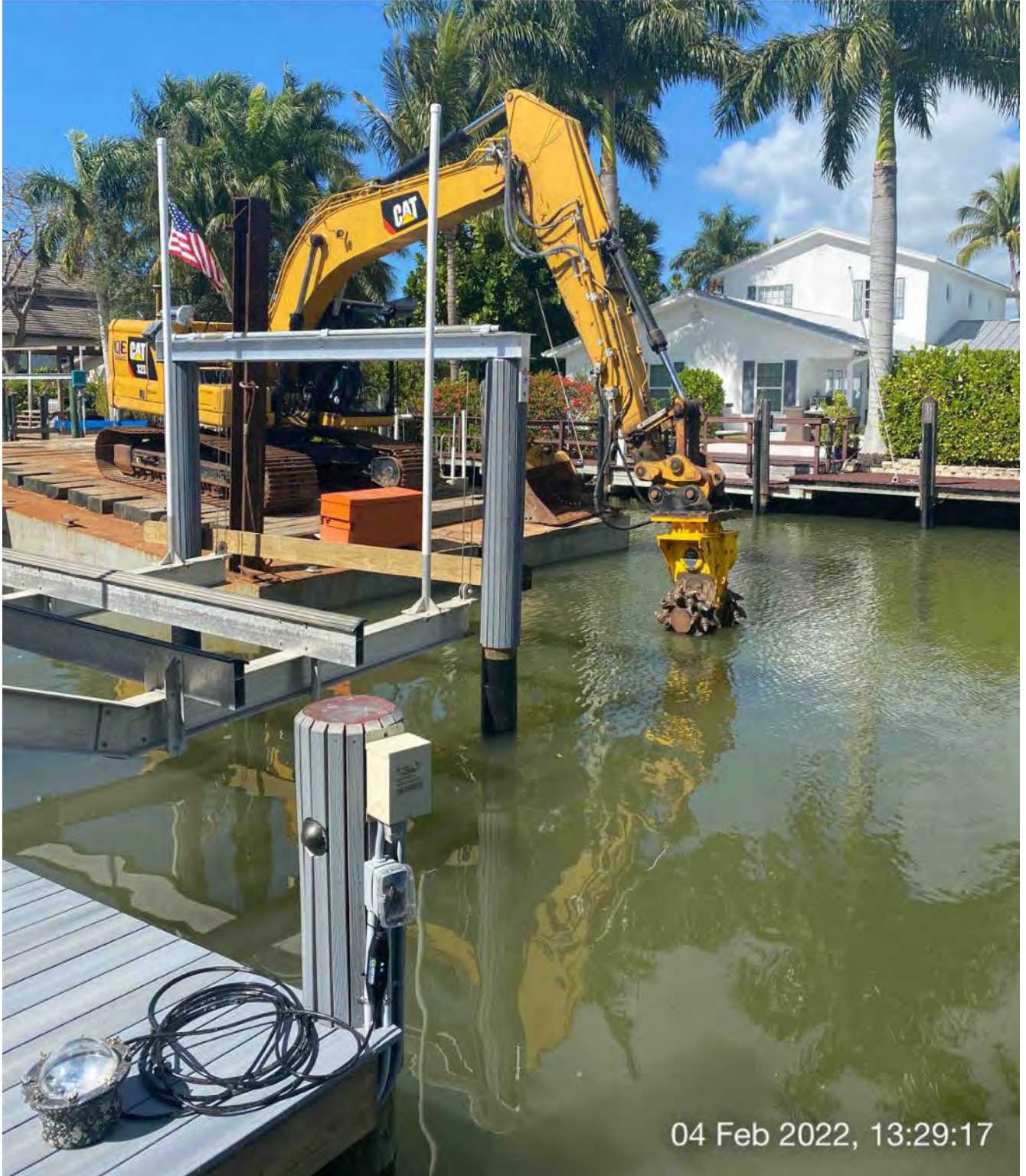
323 excavator grinding rock at station 8+00
