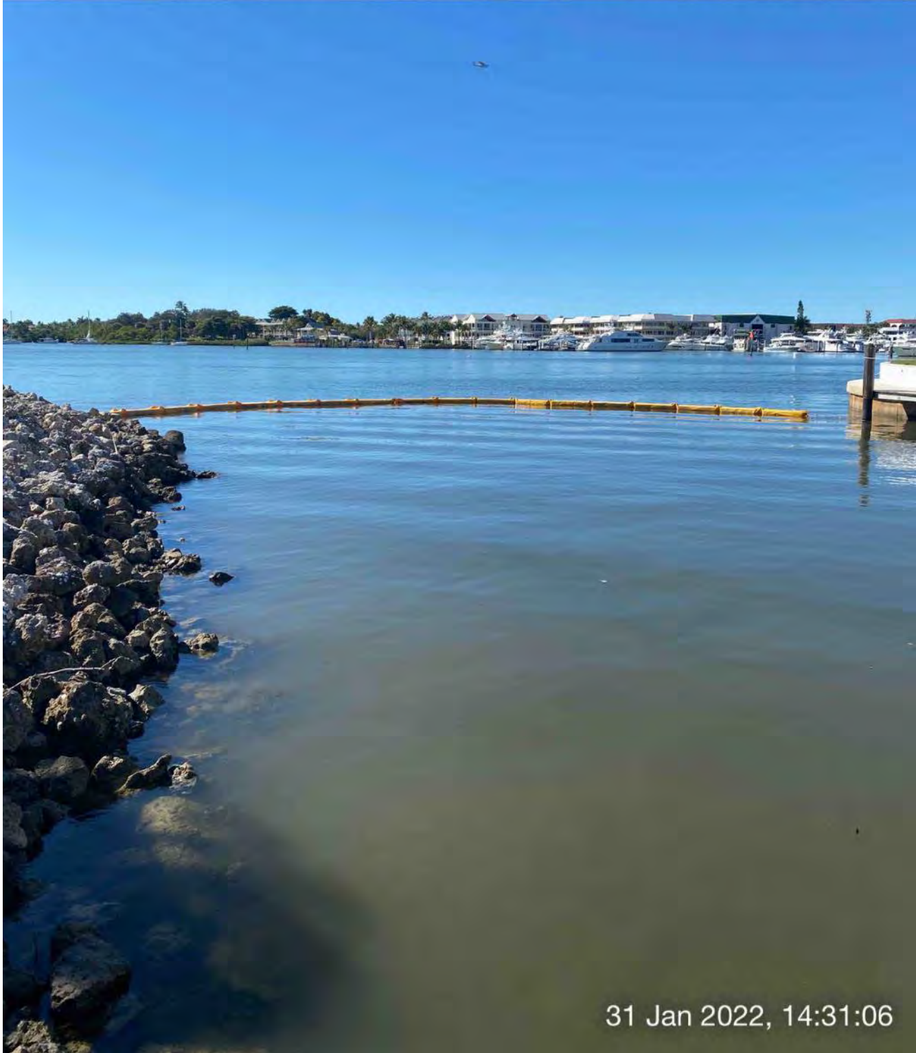
Turbidity curtain across the mouth of Canal BB-BB
