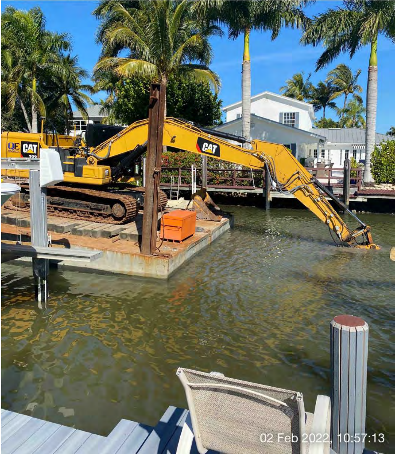
323 excavator grinding rock at station 7+75
