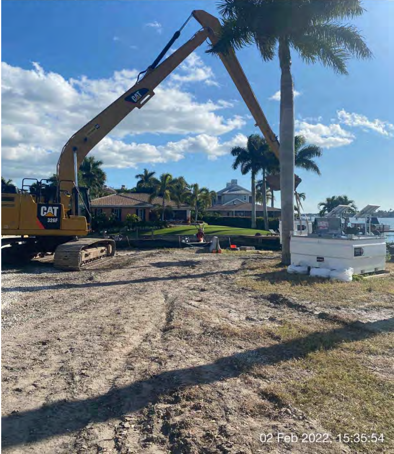
326 excavator lifting small fuel cube at 1300 Curlew Avenue
