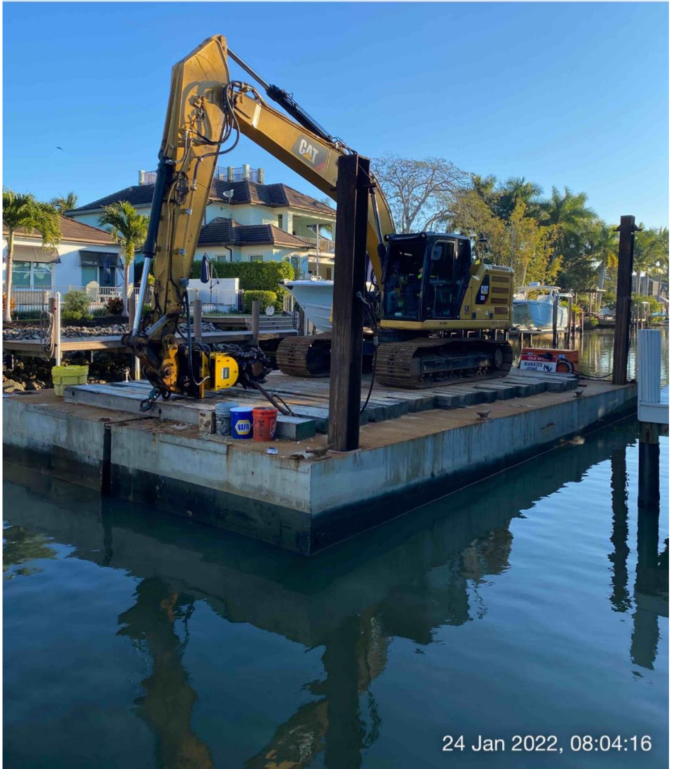
323 excavator on barge at station 4+75
