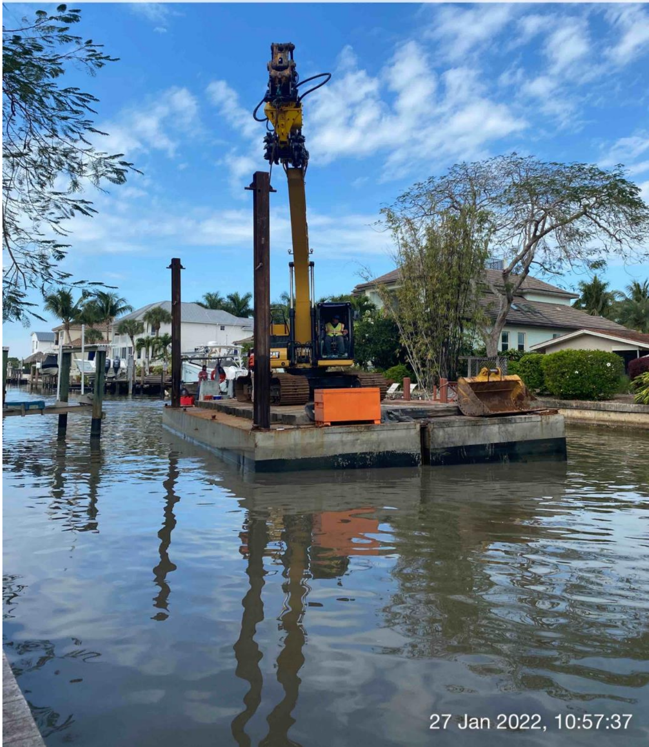
323 excavator lifting spud to allow push boat to move the barge at station 6+50
