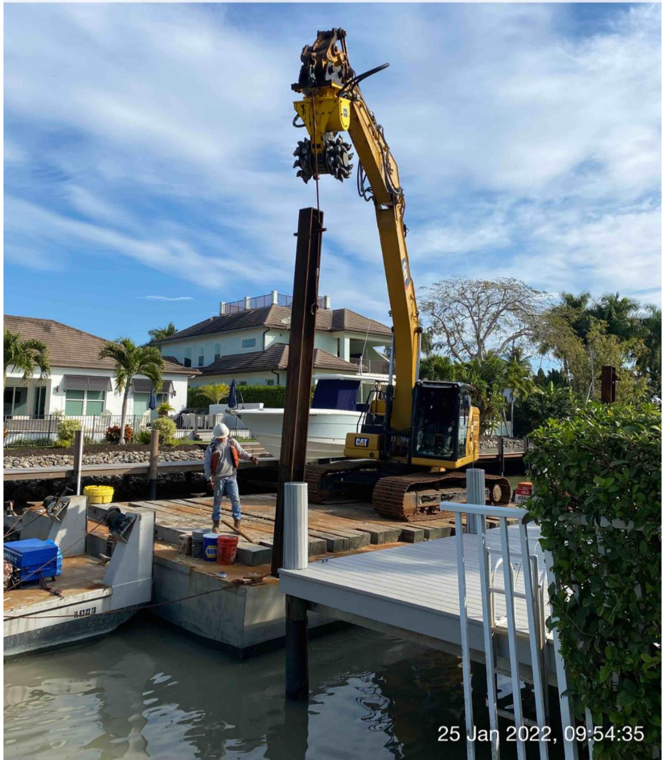
323 excavator lifting spud to allow push boat to move barge at station 5+00
