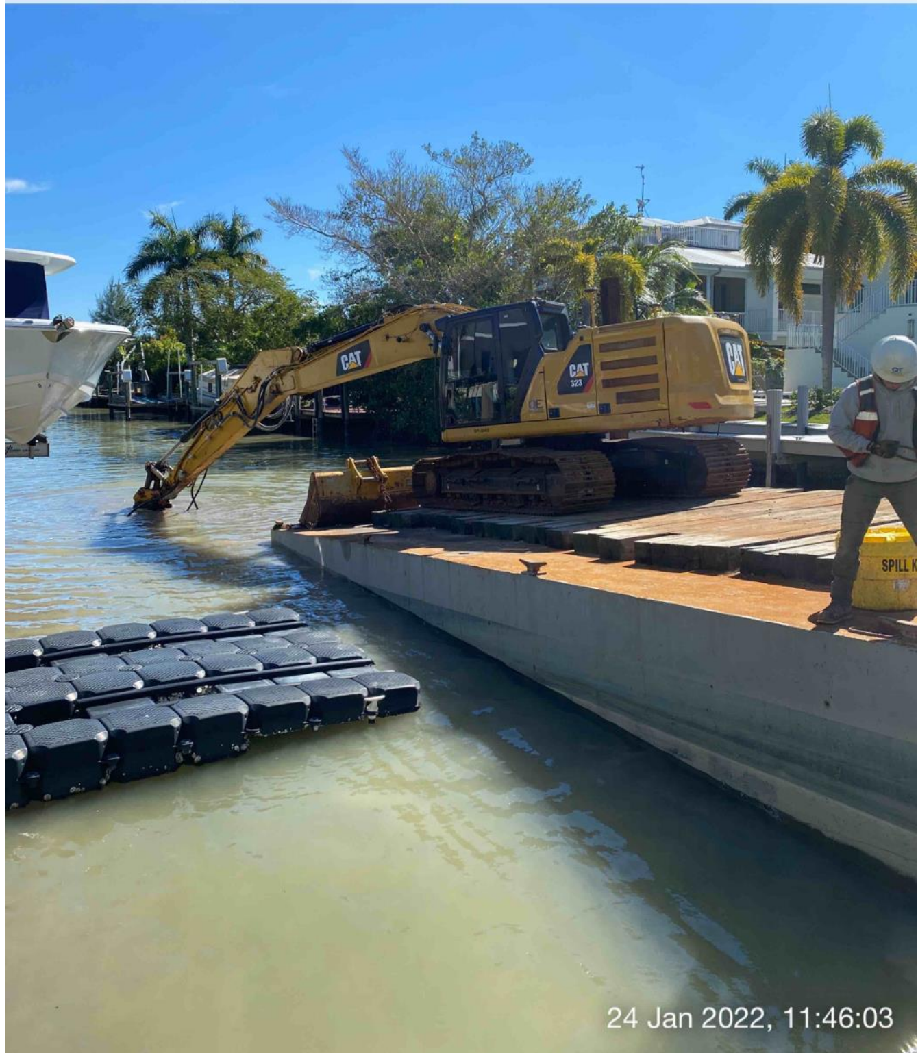
323 excavator grinding rock at station 5+00
