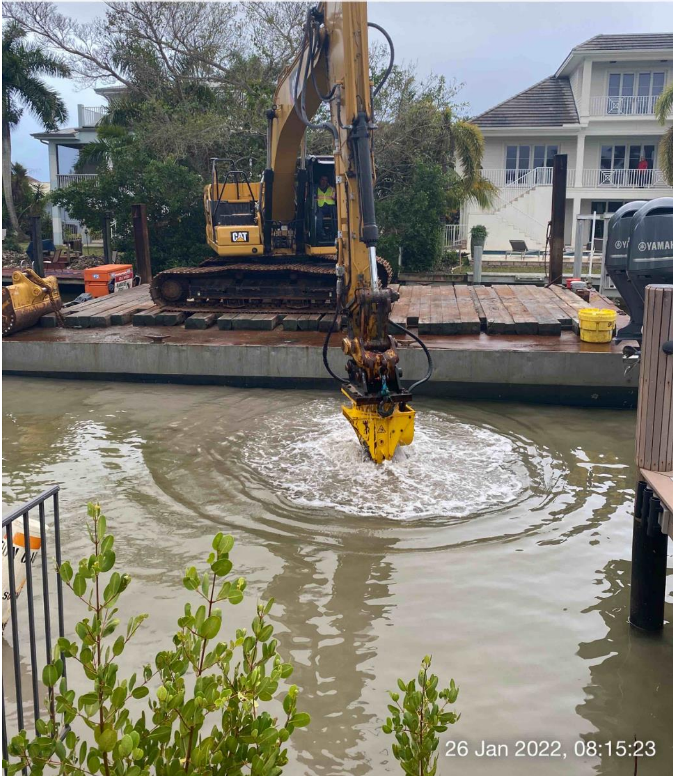
323 excavator grinding rock at station 5+50
