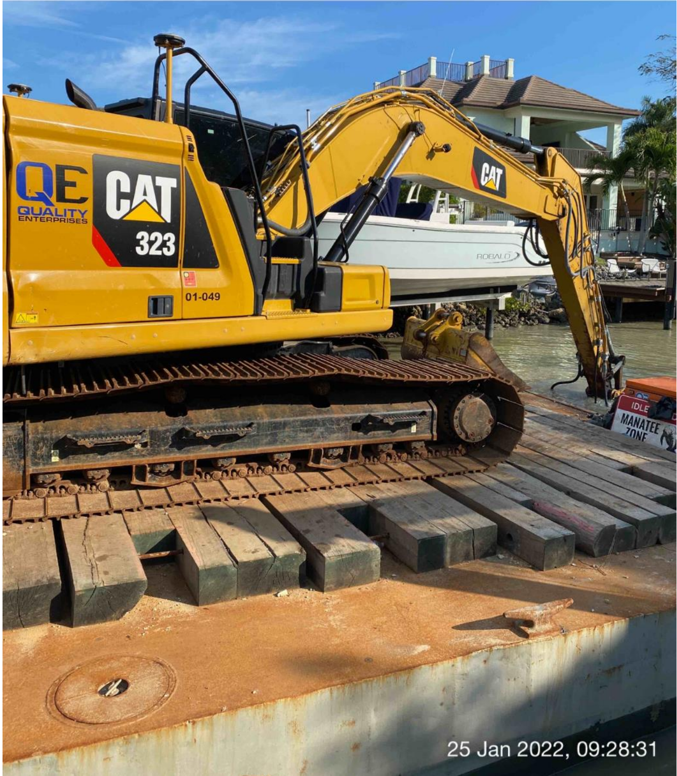
323 excavator grinding rock at station 5+00
