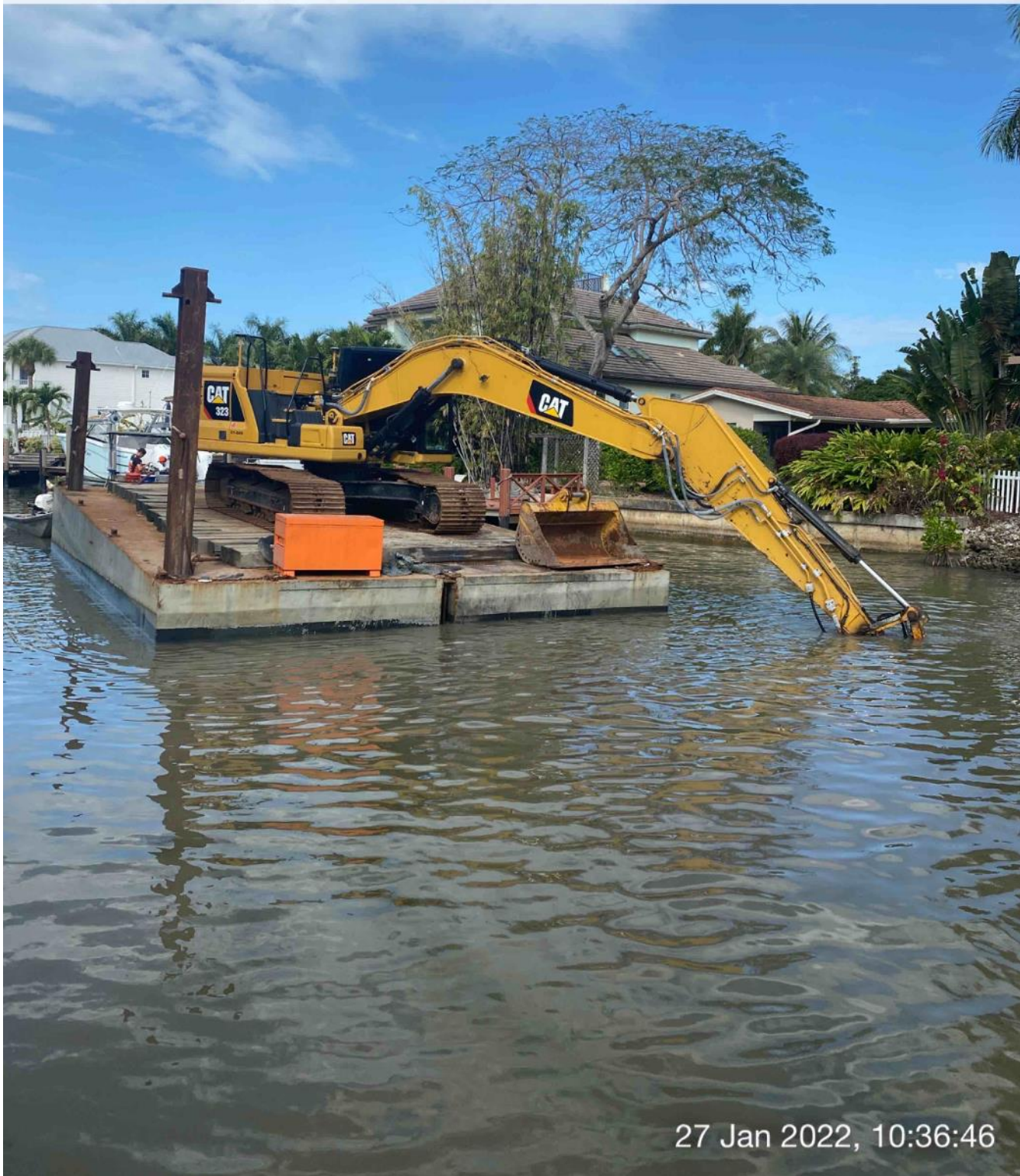
323 excavator grinding rock at station 6+50
