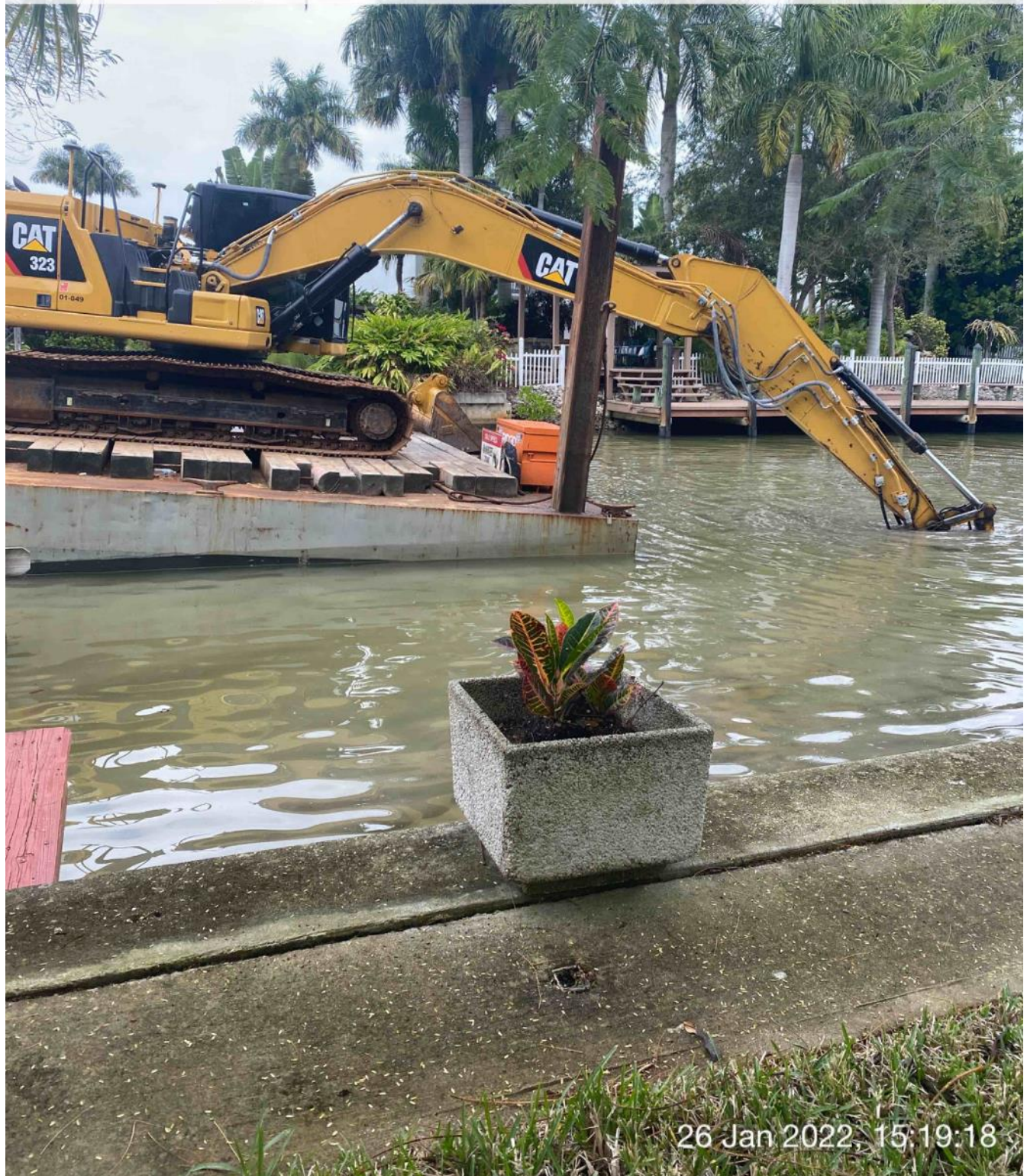
323 excavator grinding rock at station 6+50
