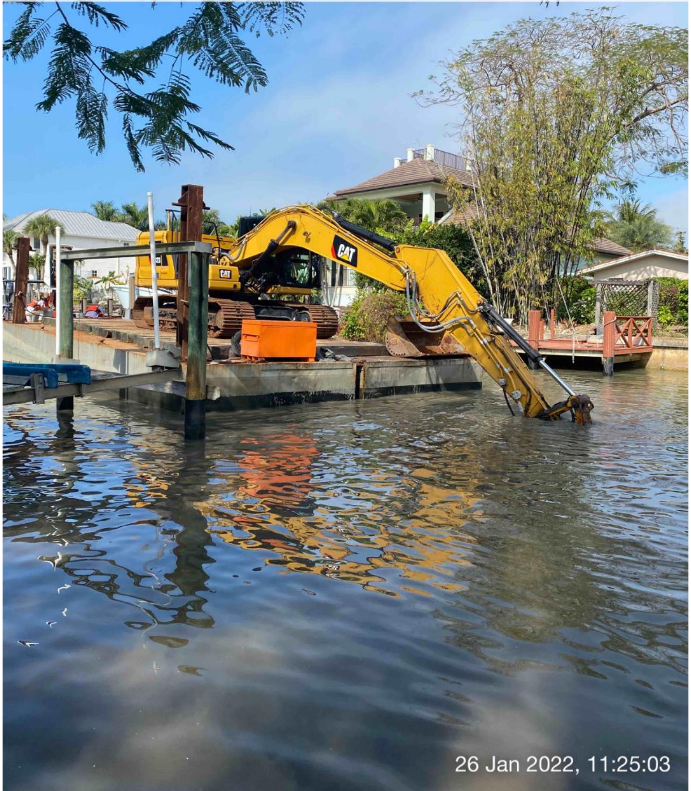
323 excavator grinding rock at station 6+00
