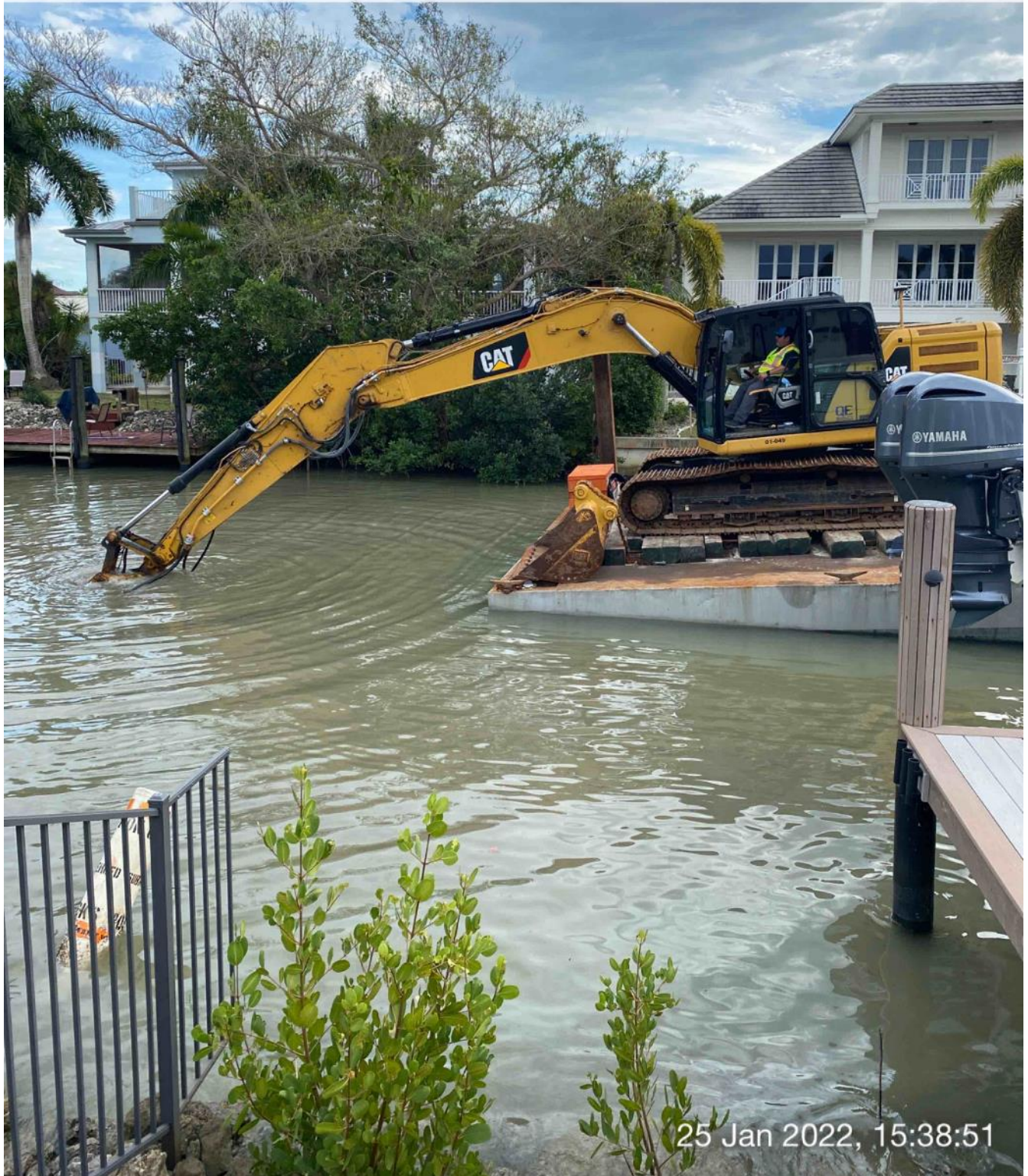
323 excavator grinding rock at station 5+25
