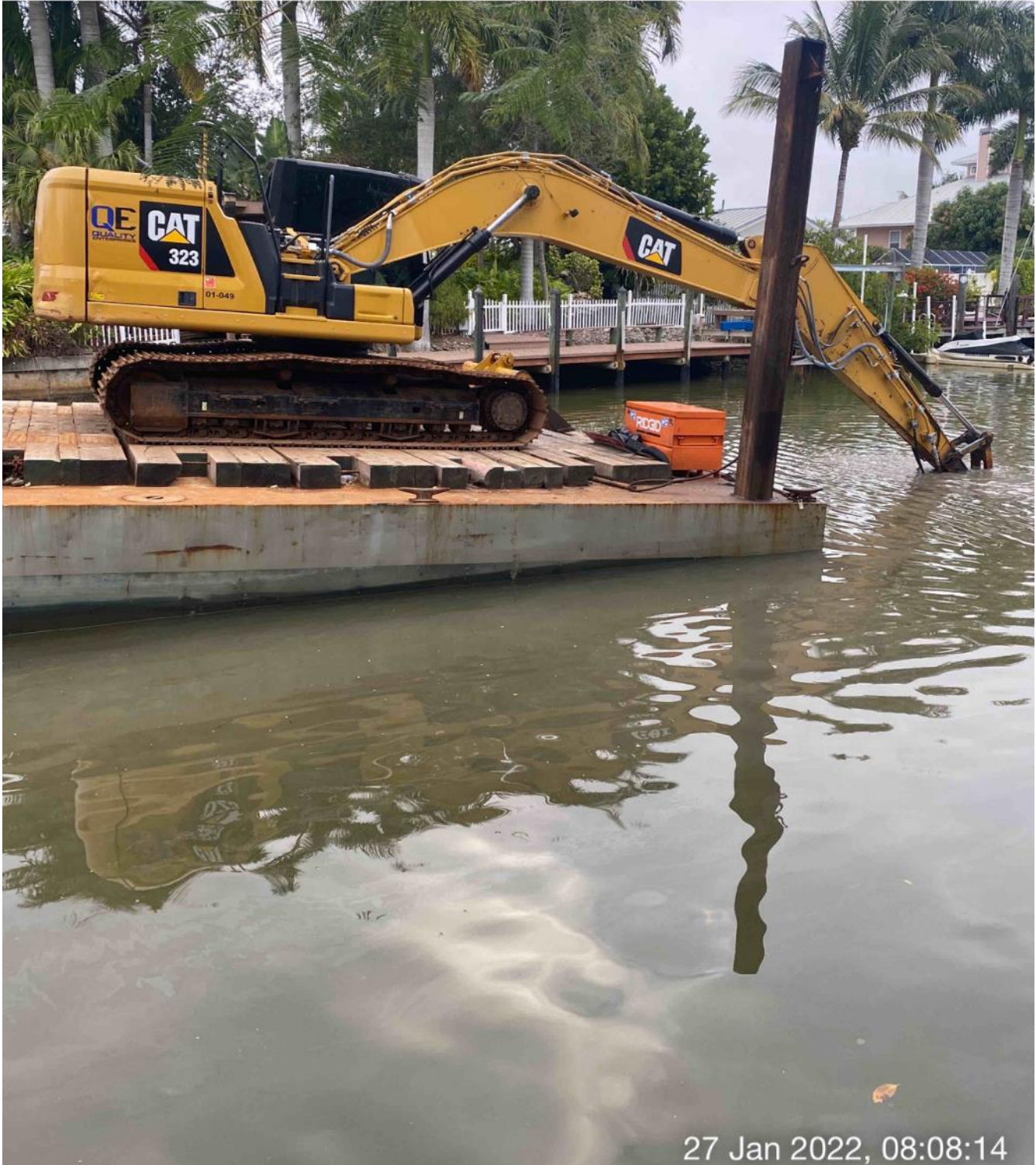
323 excavator grinding rock at station 6+50
