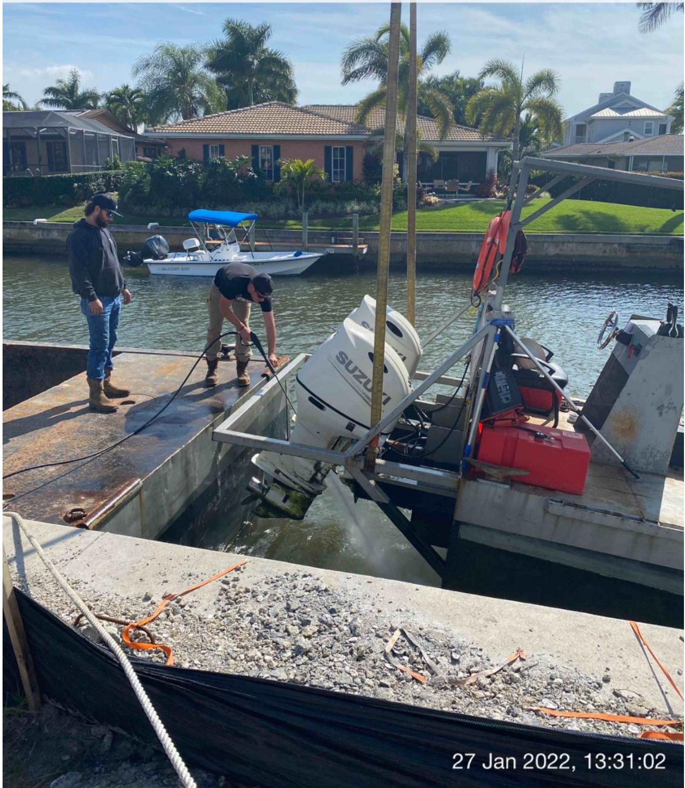
Contractor using water tank to pressure wash boat engines
