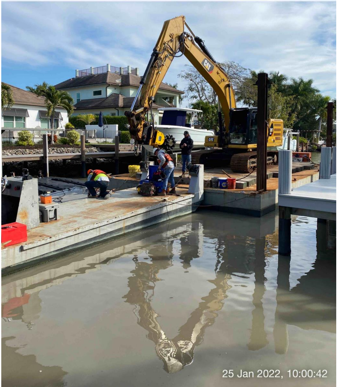
Contractor replacing teeth on Epiroc grinder at station 5+00
