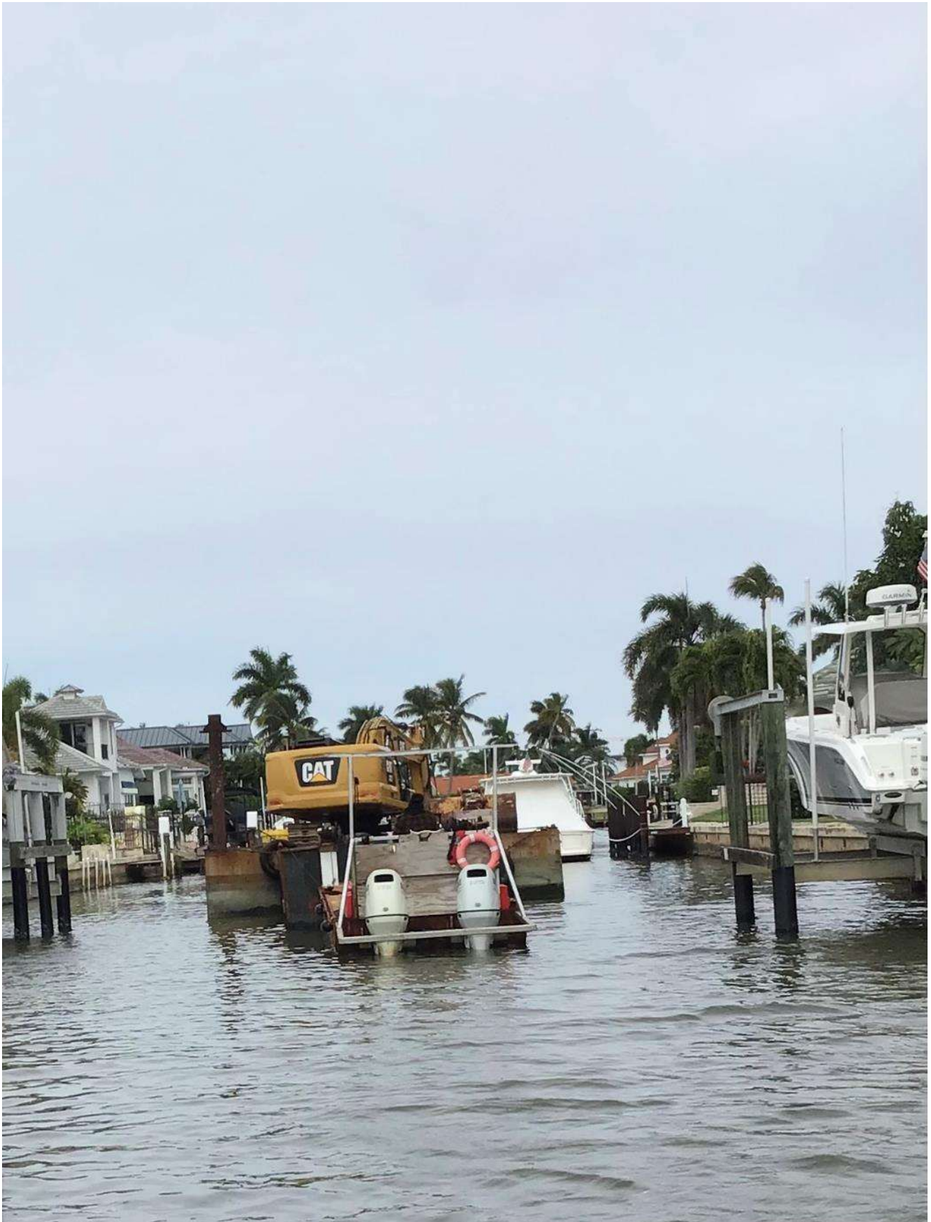
323 excavator grinding rock at station 5+50 in Canal A-A.
