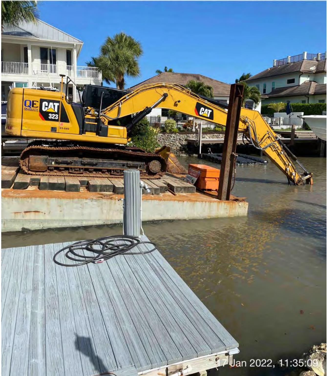
323 excavator grinding rock at station 4+50
