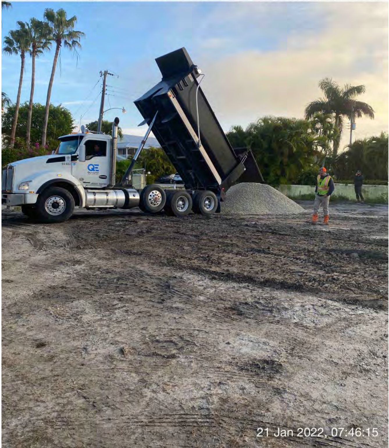
Dump truck dumping pebbles on site at 1300 Curlew Avenue
