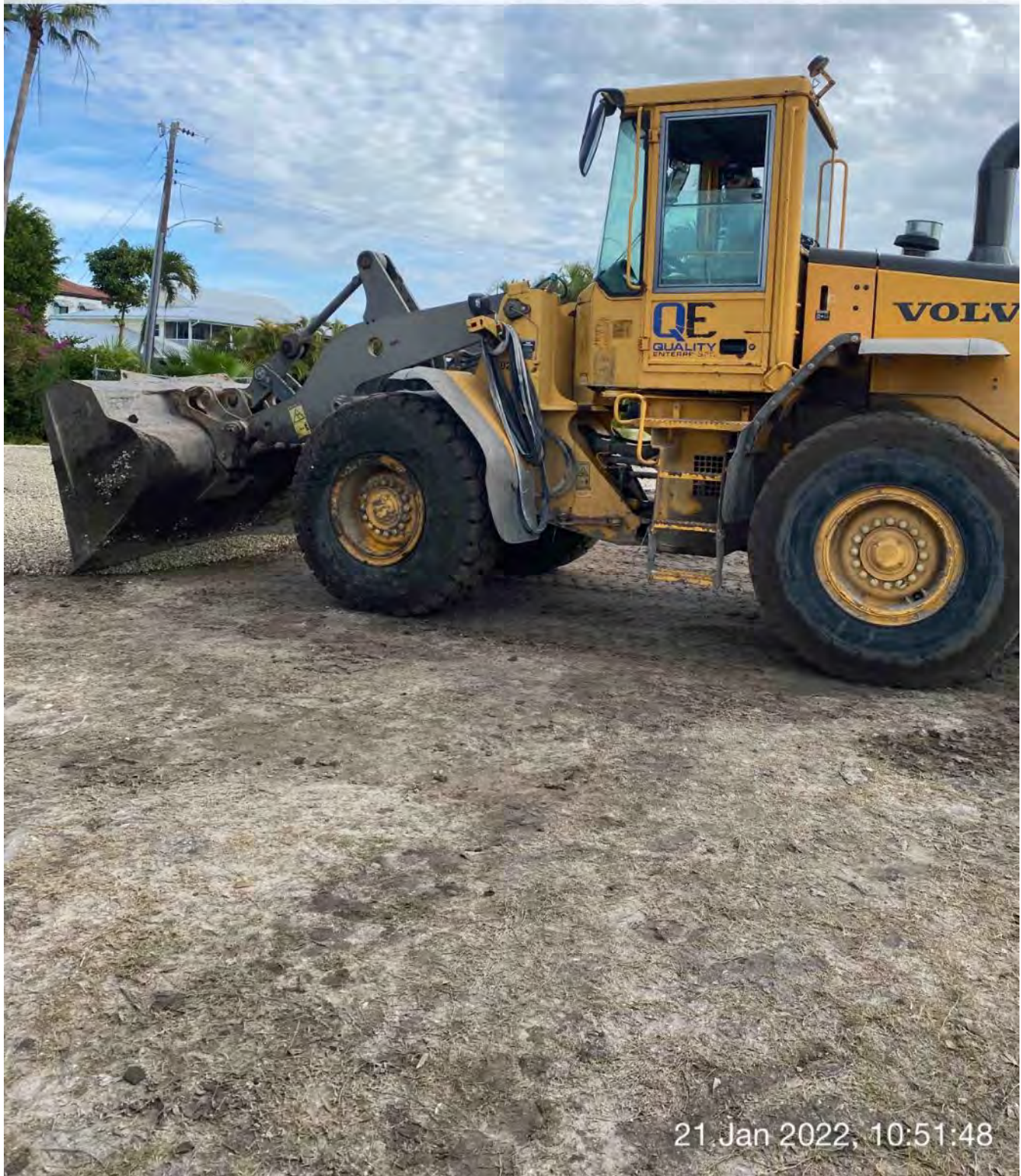
Front end loader spreading pebbles on site at 1300 Curlew Avenue
