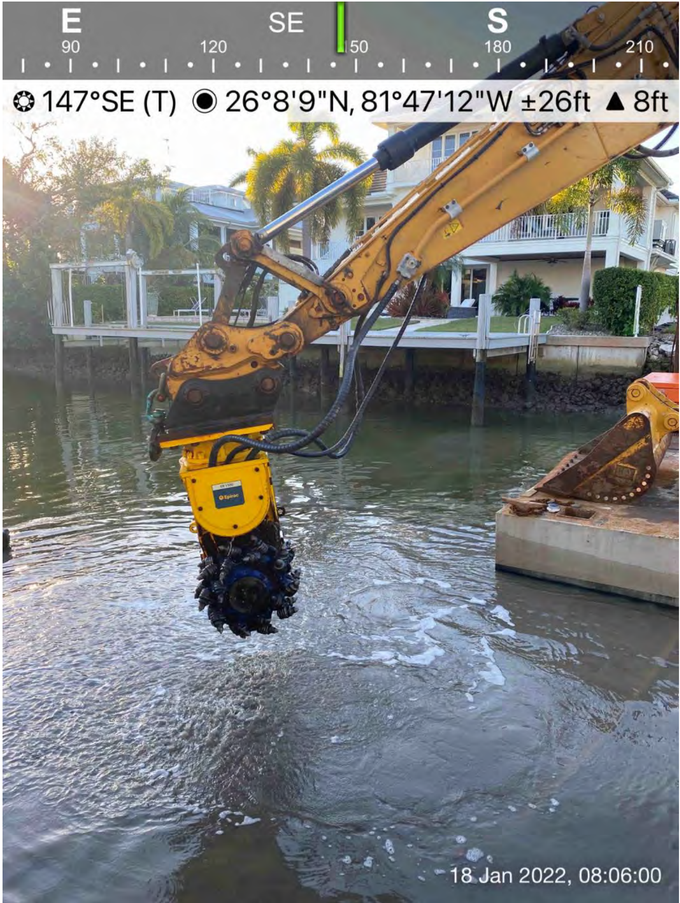
323 excavator grinding rock at station 4+50
