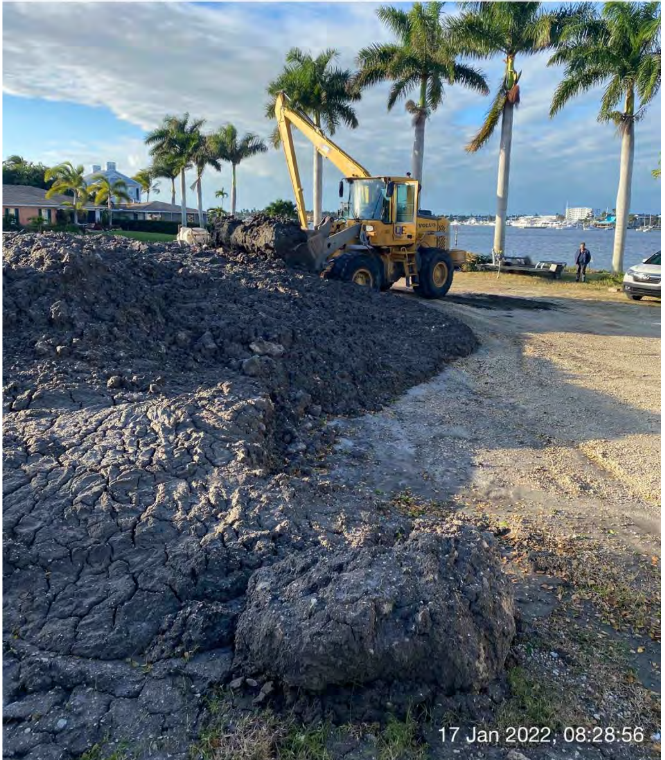
Front end loader transferring material from dewatering site to dump truck at 1300 Curlew Avenue
