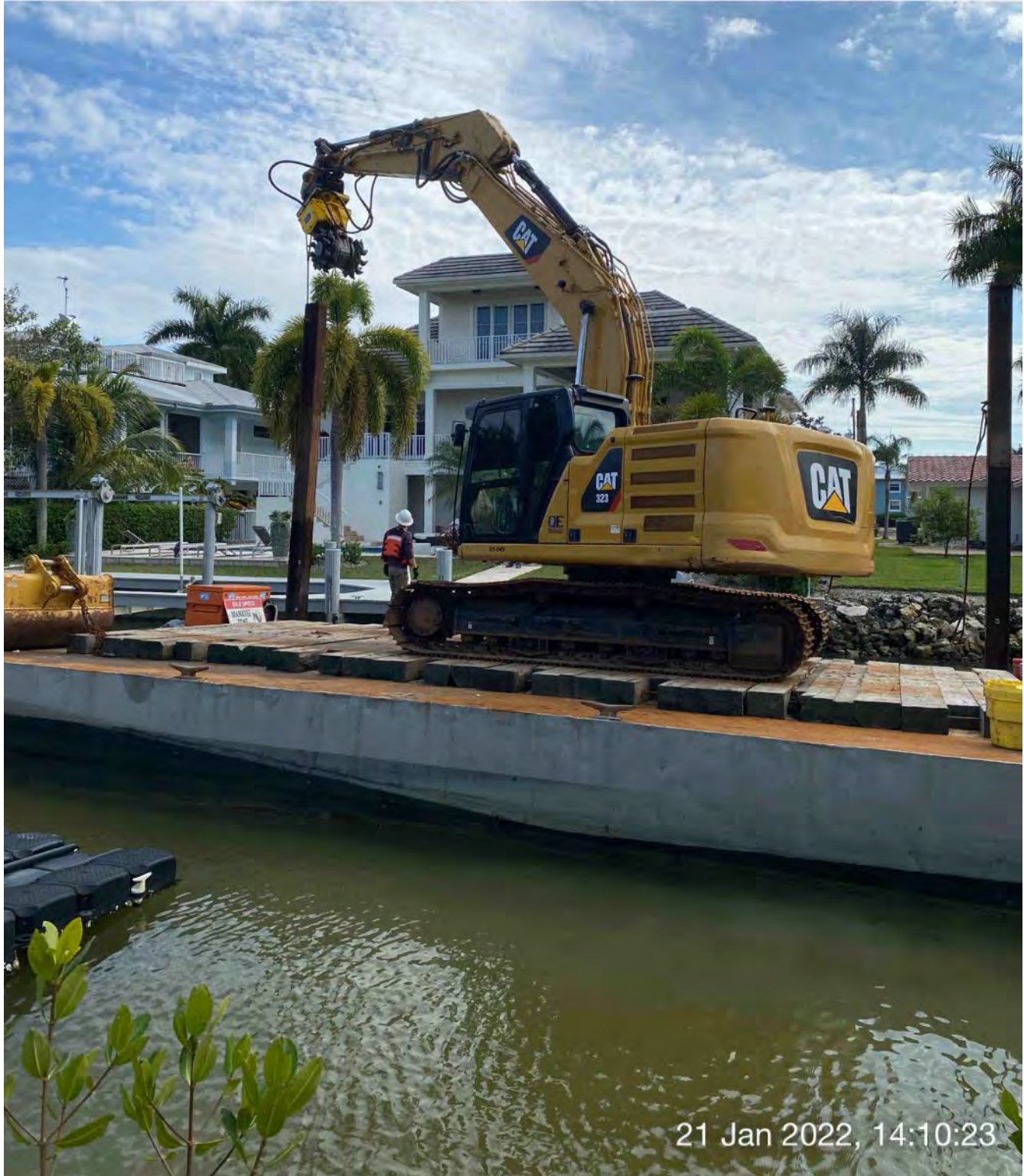
323 excavator lifting spud to allow push boat to move barge at station 4+75
