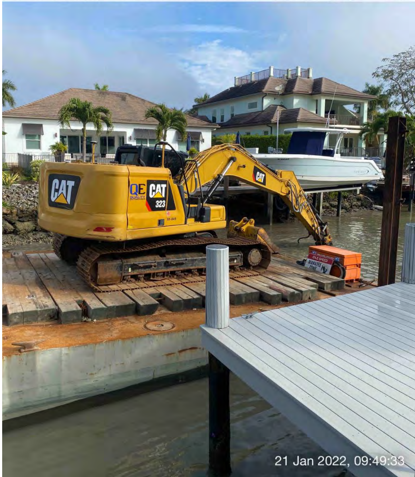
323 excavator grinding rock at station 5+00
