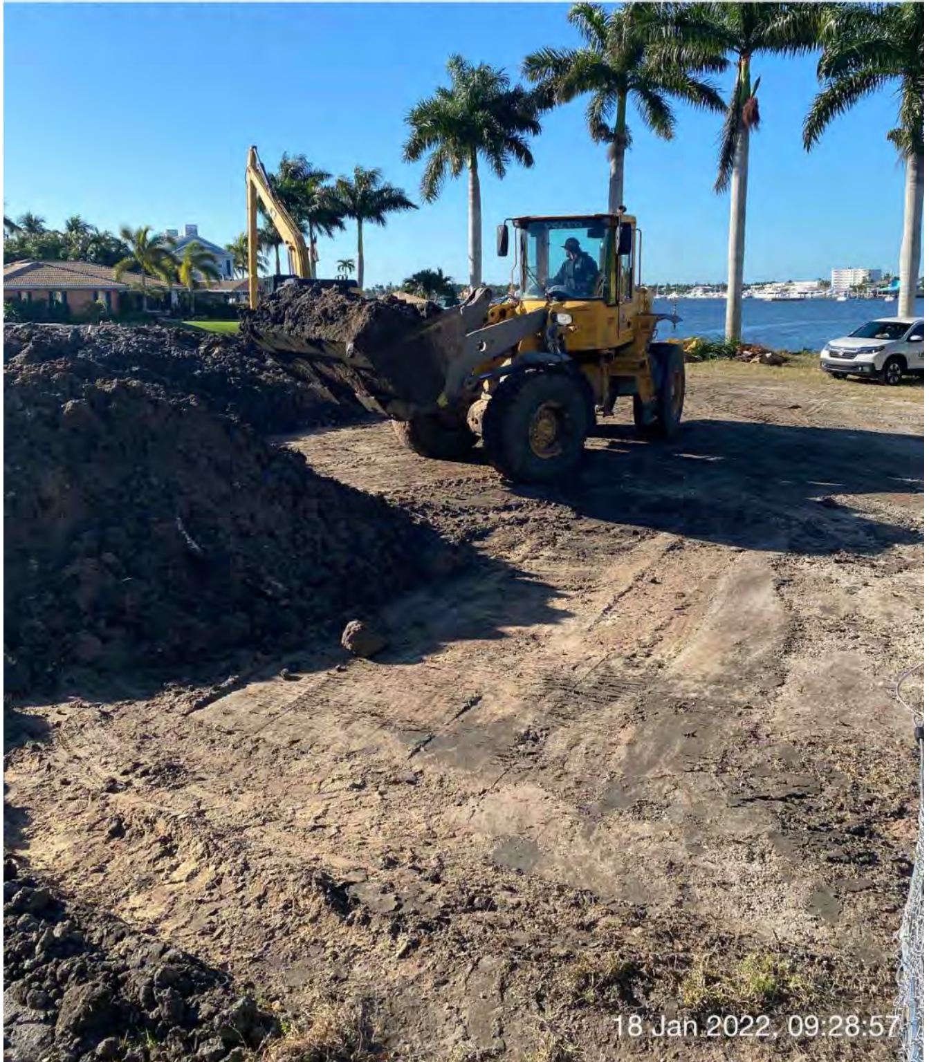
Front end loader transferring material from dewatering site to dump truck at 1300 Curlew Avenue
