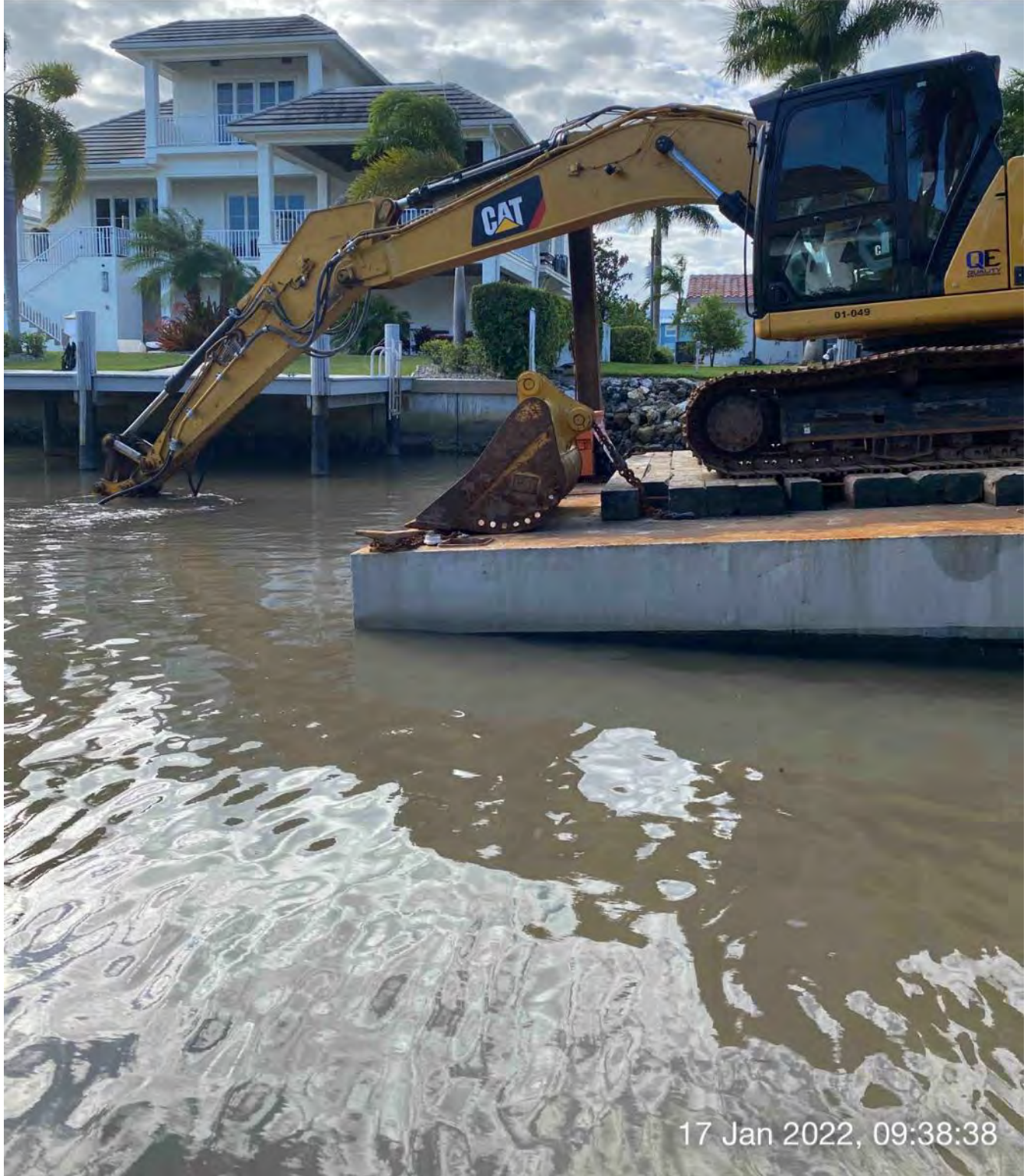
323 excavator grinding rock at station 4+25
