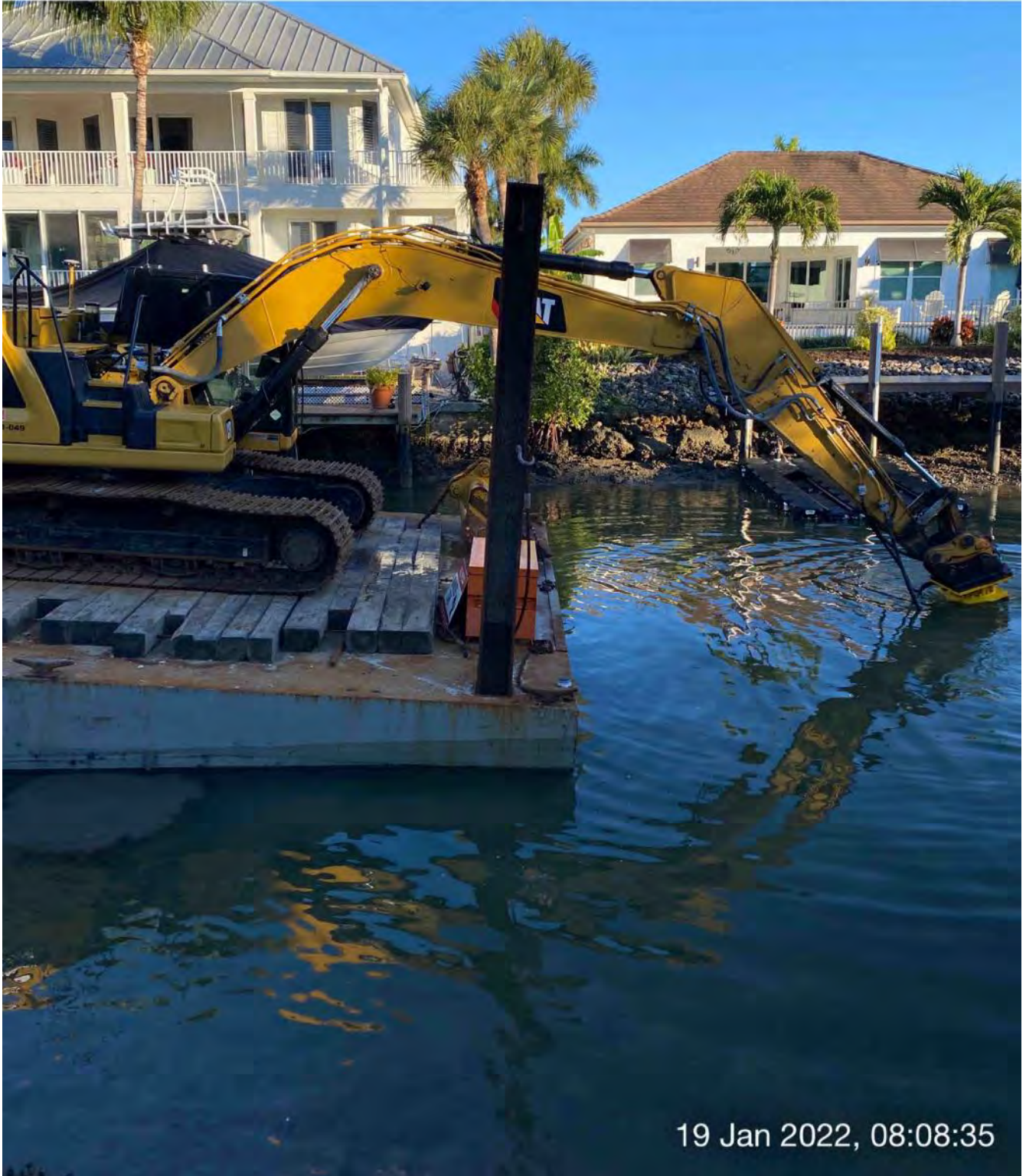
323 excavator grinding rock at station 4+50
