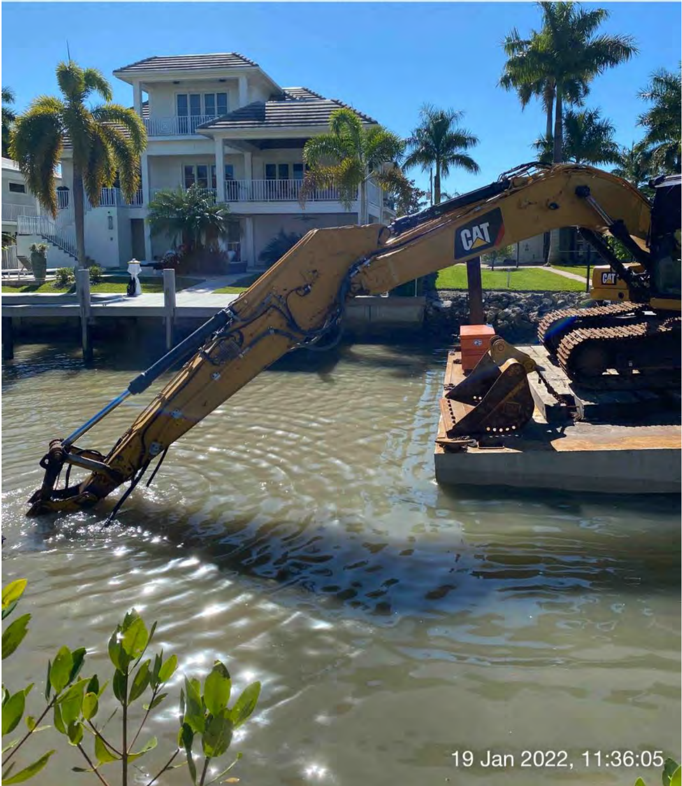
323 excavator grinding rock at station 4+50
