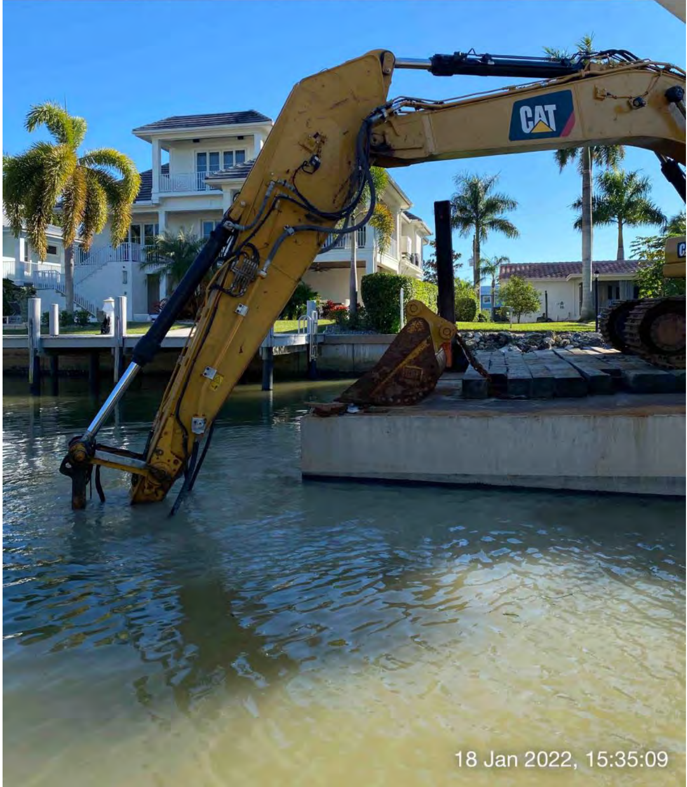
323 excavator grinding rock at station 4+50
