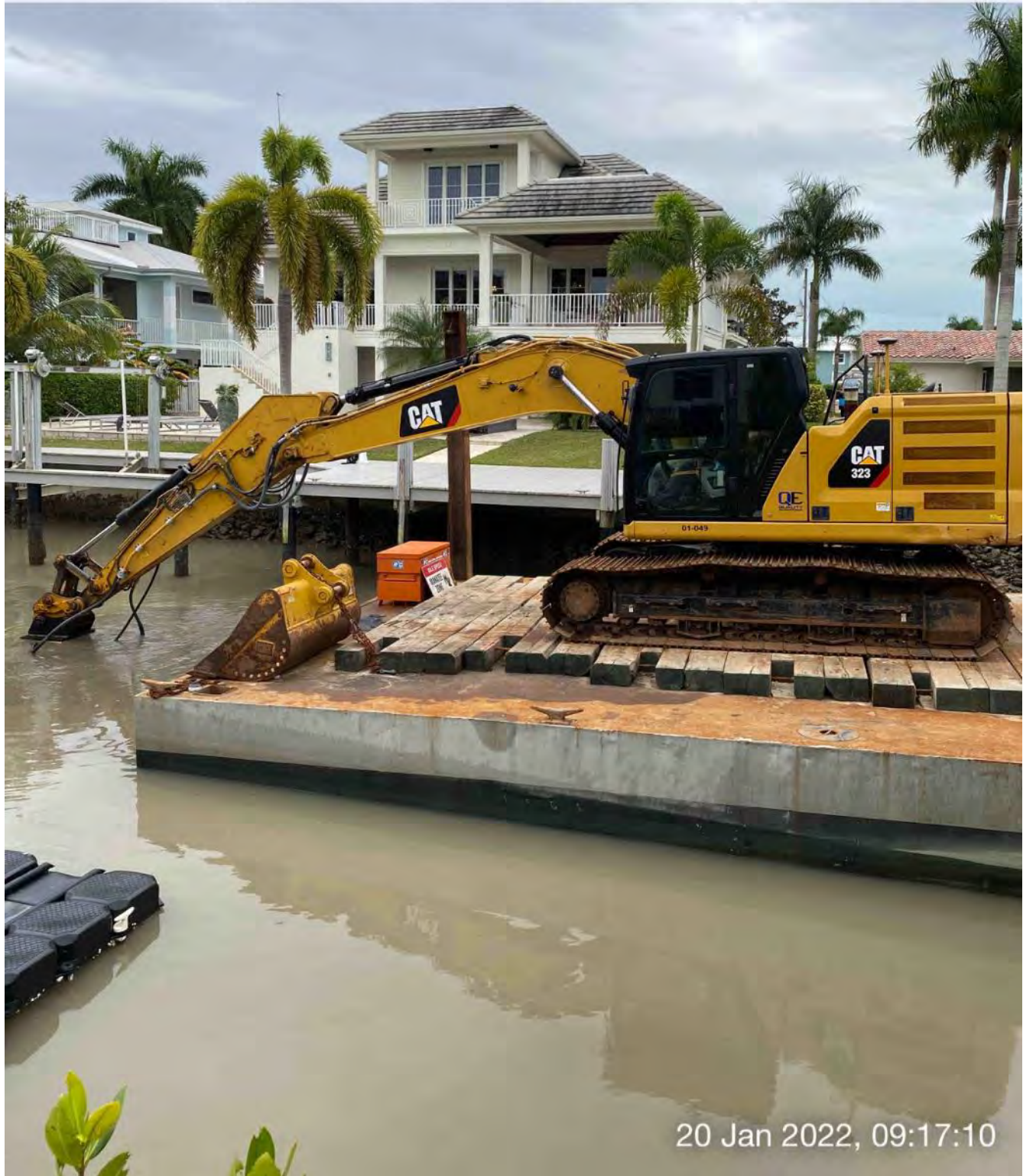
323 excavator grinding rock at station 4+50
