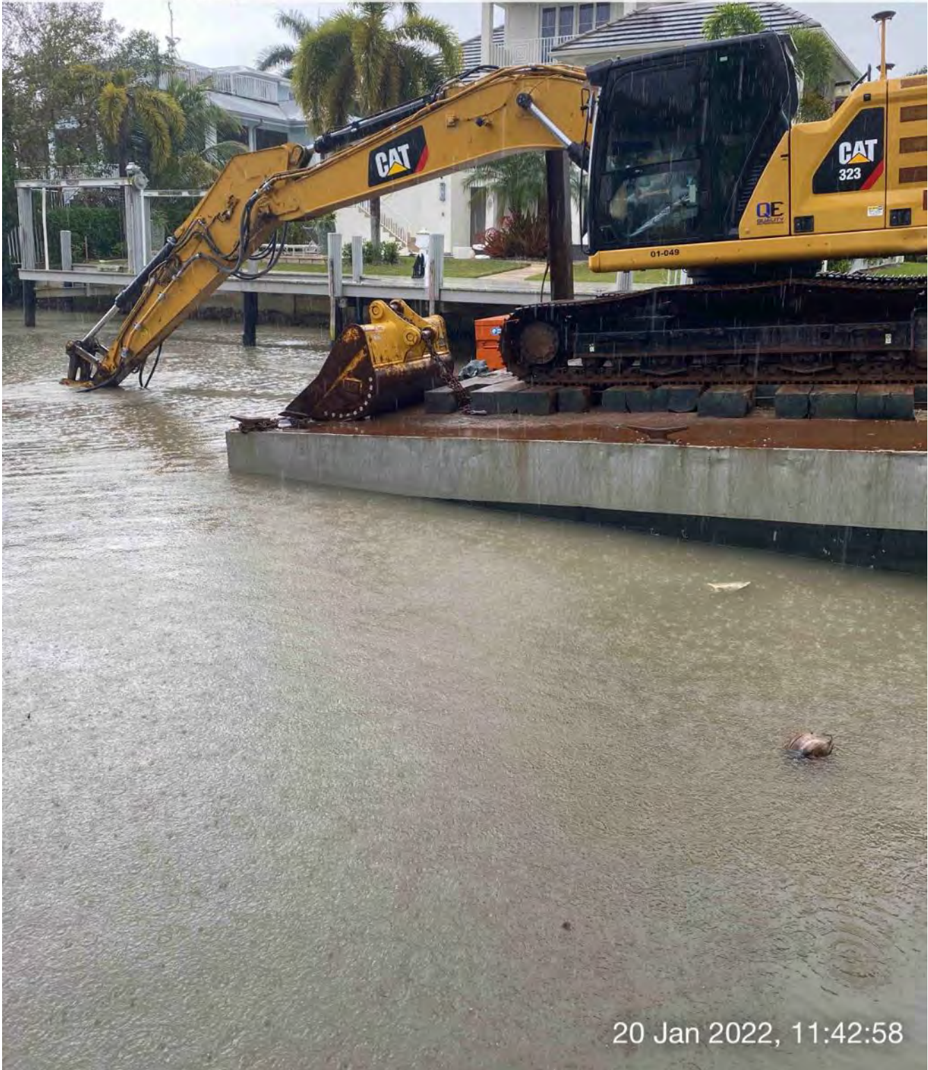
323 excavator grinding rock at station 4+50
