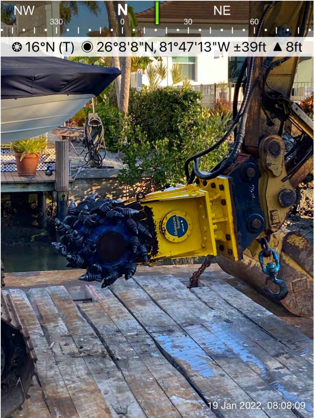
Epiroc grinder attached to 323 excavator on barge at station 4+25
