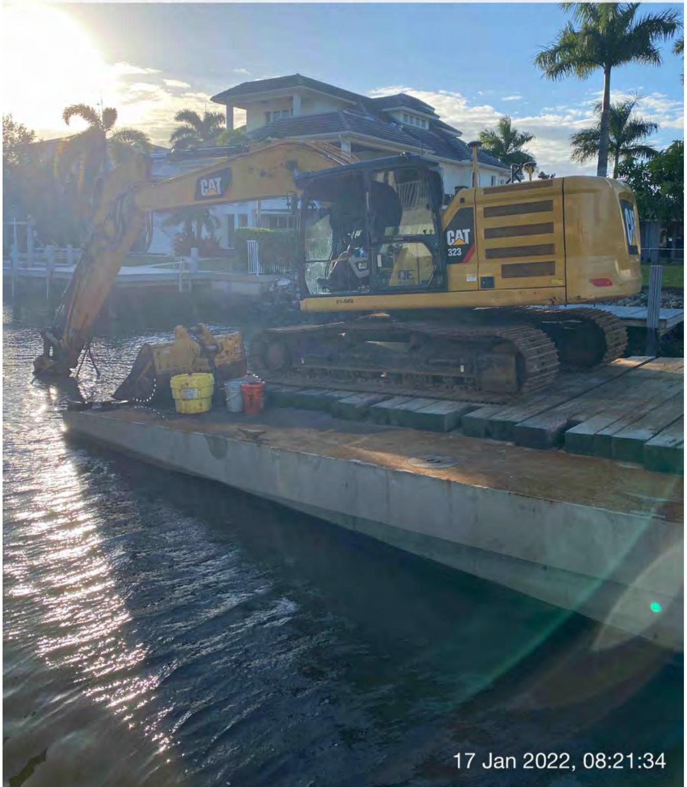
323 excavator grinding rock at station 4+25
