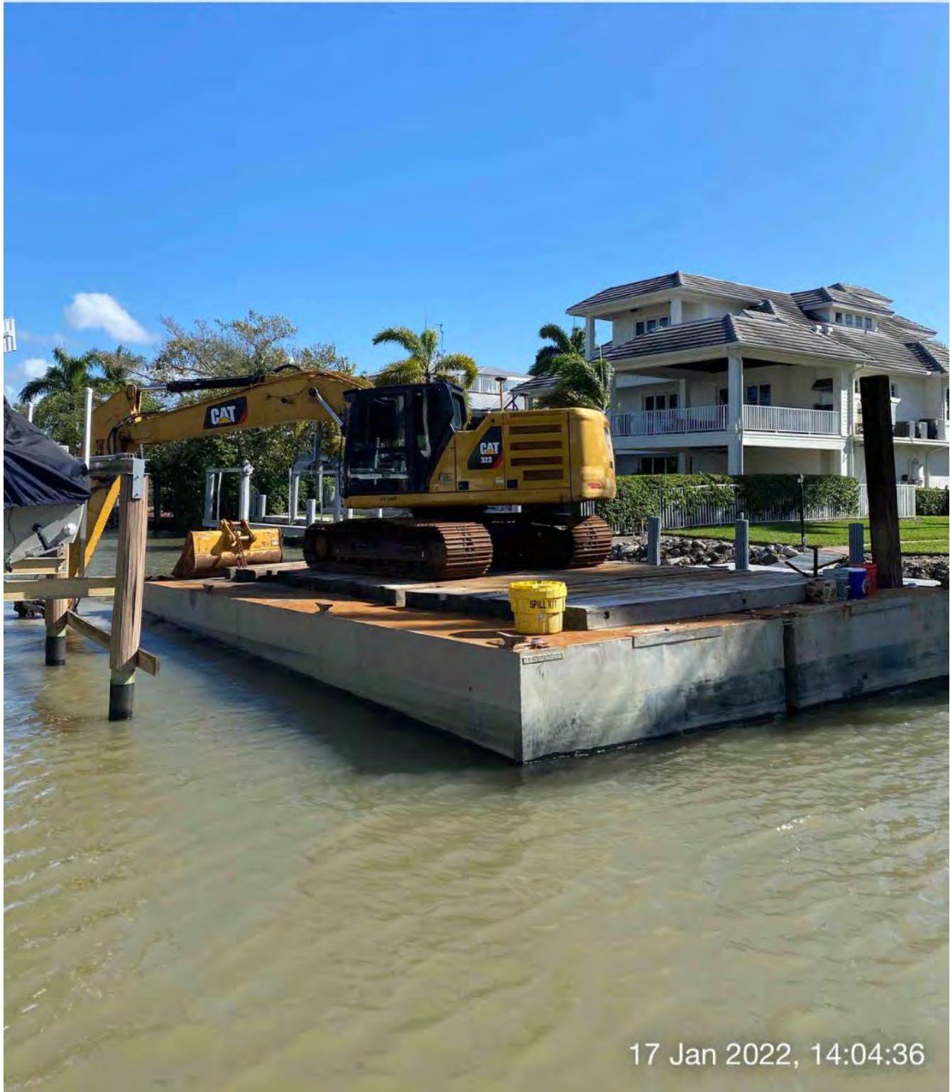
323 excavator grinding rock at station 4+50
