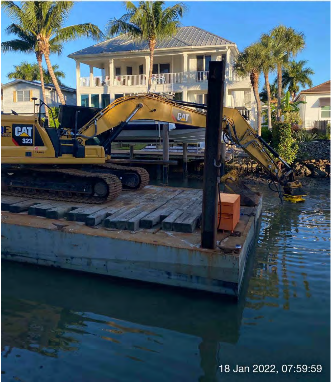
323 excavator grinding rock at station 4+50
