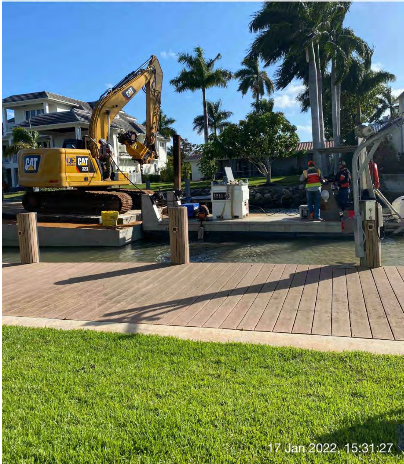
Refueling 323 excavator with small fuel cube
