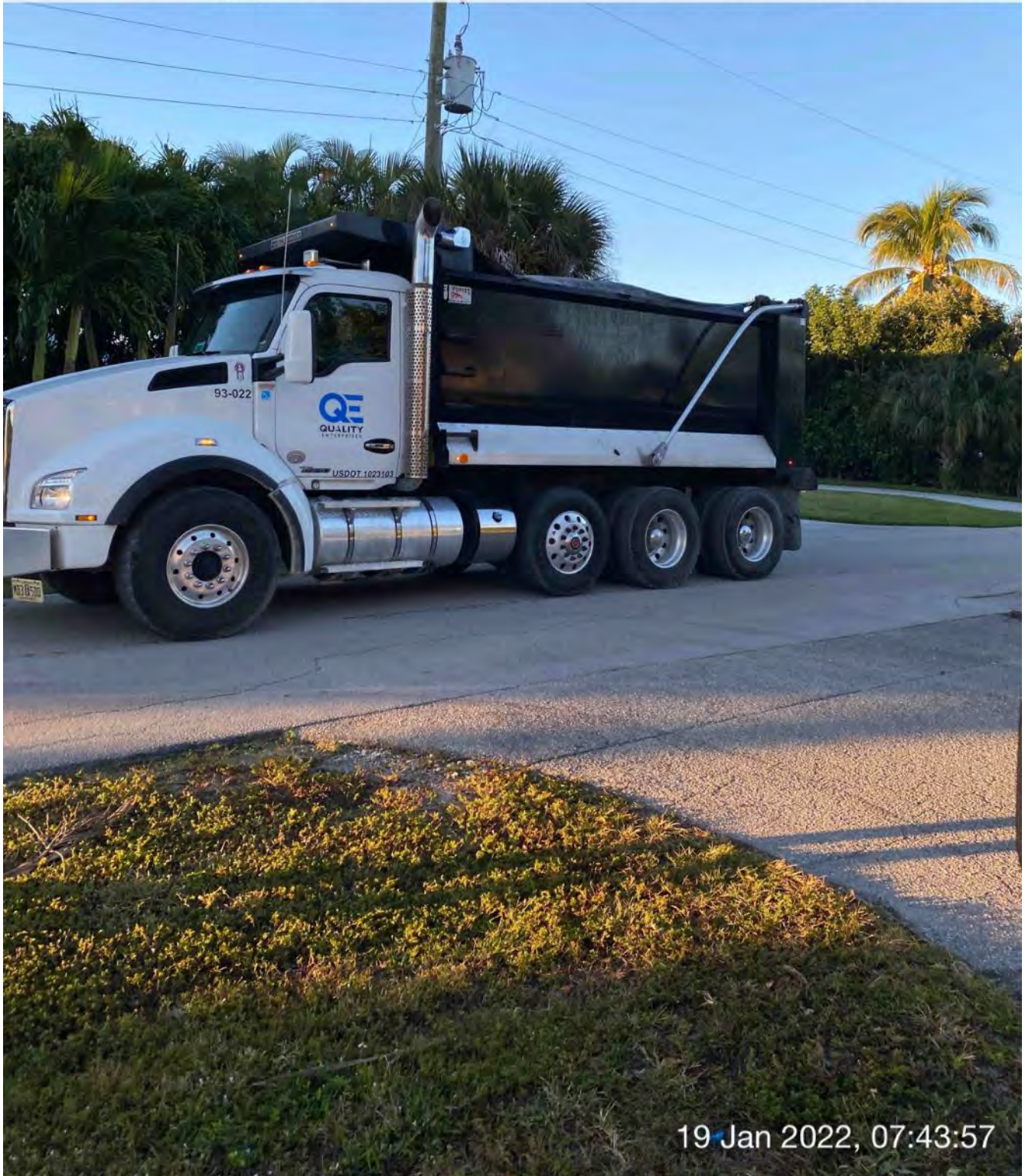
Full dump truck taking material away from the site at 1300 Curlew Avenue
