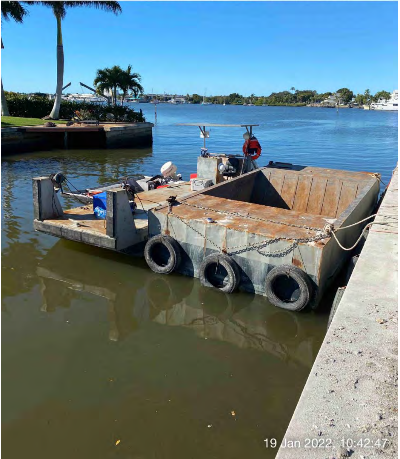
Hopper, push boat, and support boat at station 1+50 in Canal CC-CC
