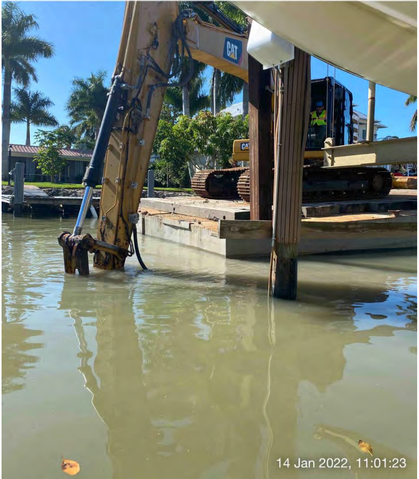
323 excavator grinding rock at station 4+25
