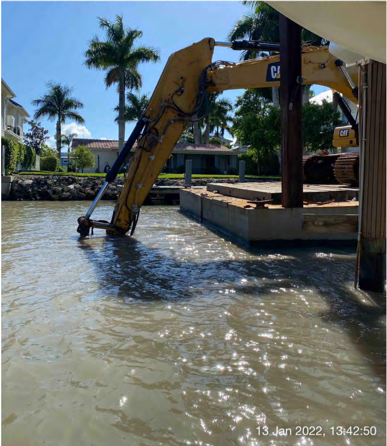
323 excavator grinding rock at station 4+25
