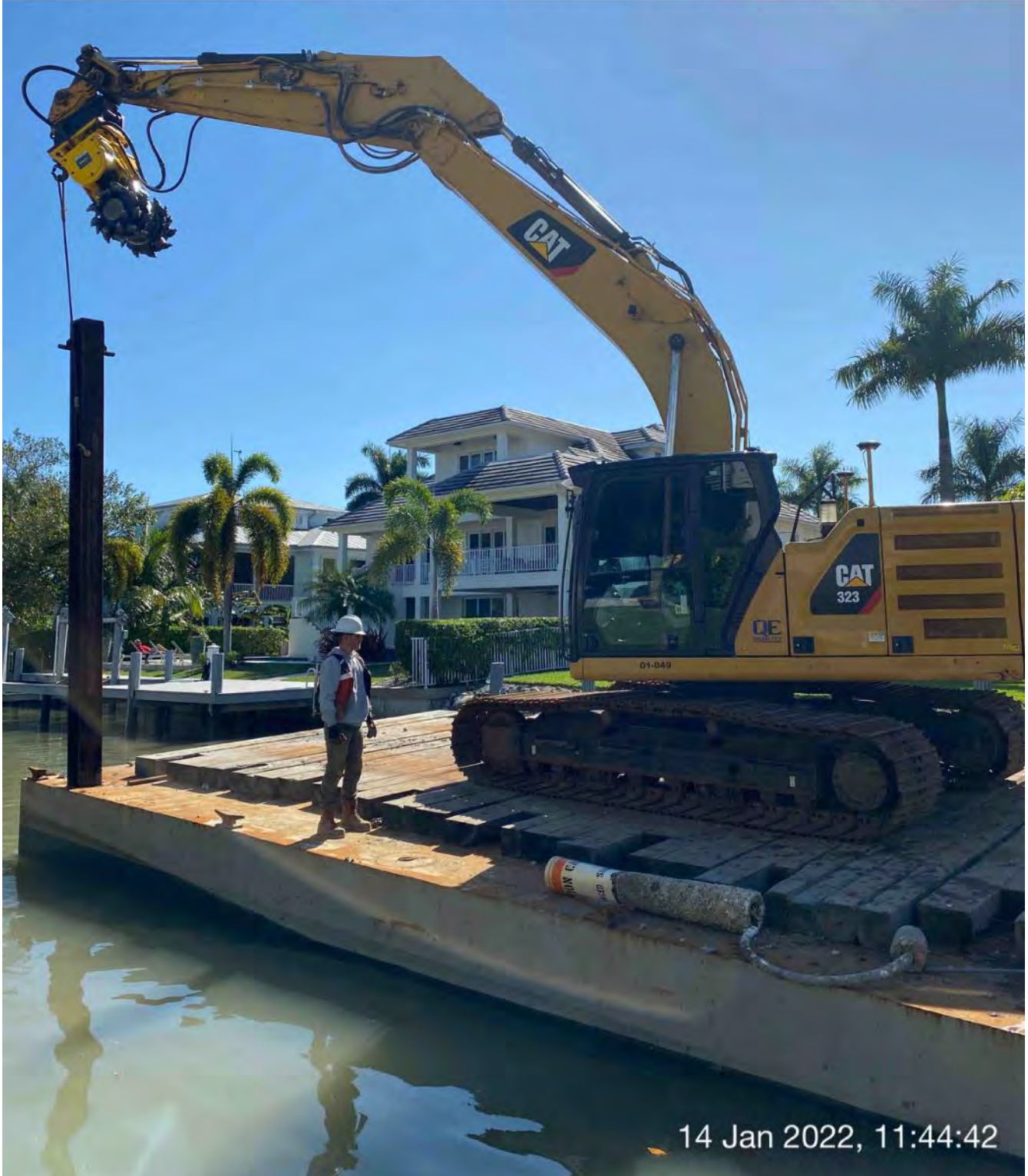
323 excavator lifting spud to allow push boat to move barge at station 4+25
