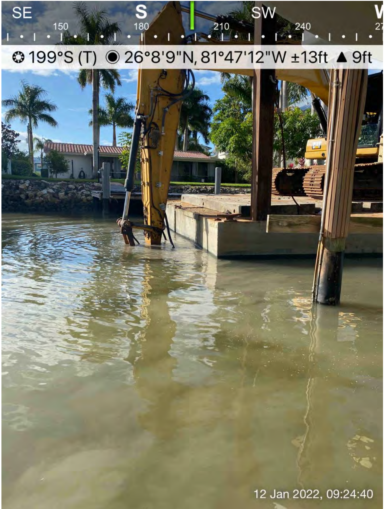
323 excavator grinding rock at station 4+25
