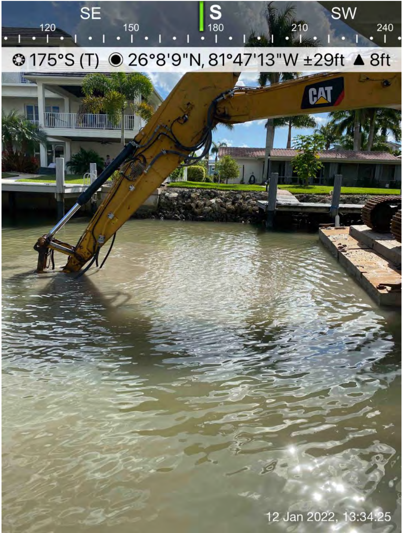
323 excavator grinding rock at station 4+25
