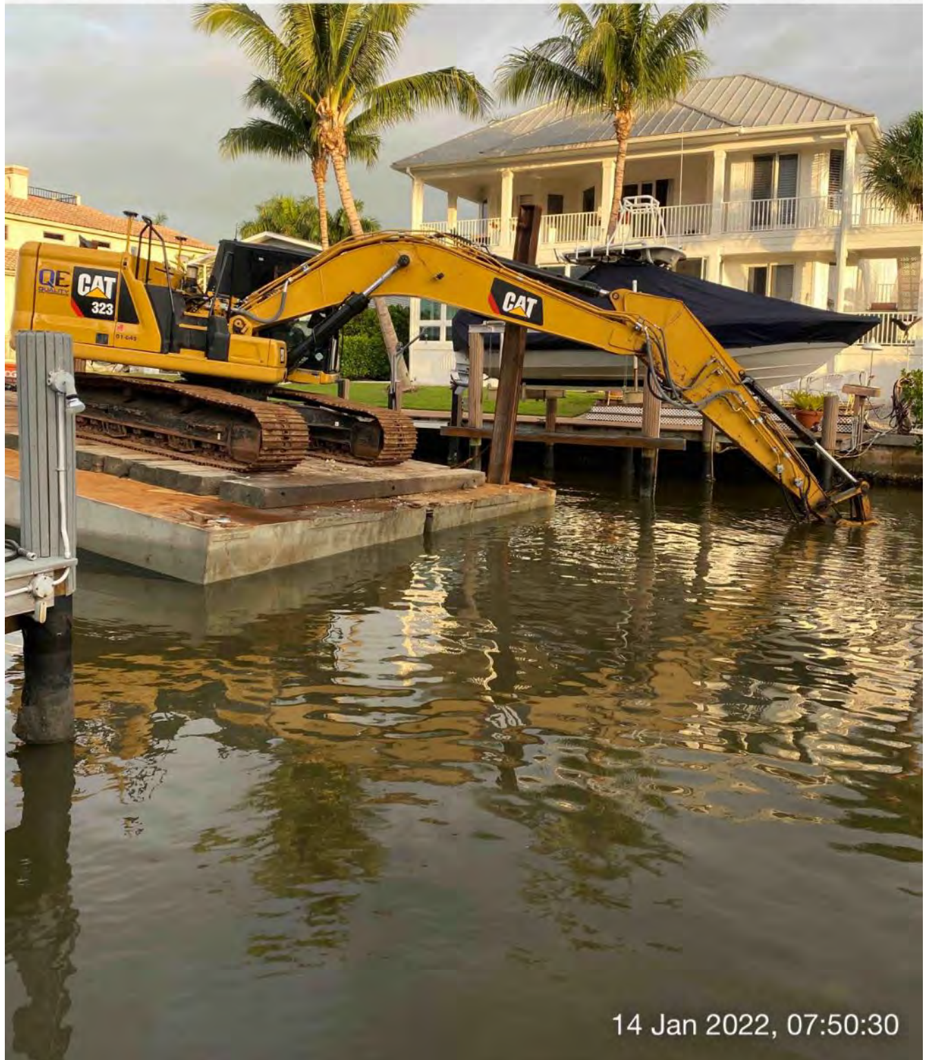
323 excavator grinding rock at station 4+25
