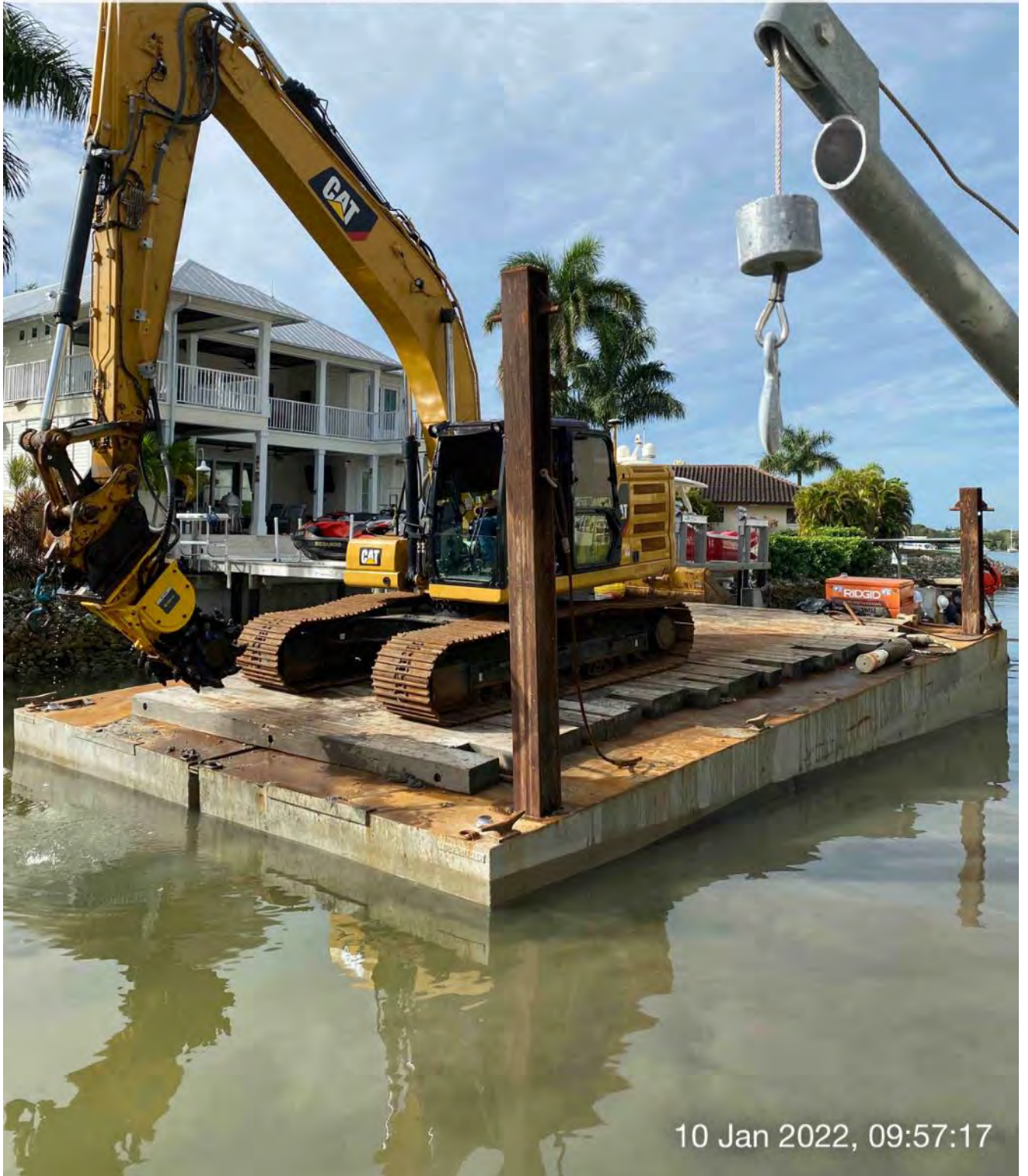
323 excavator with Epiroc grinder on barge at station 4+00
