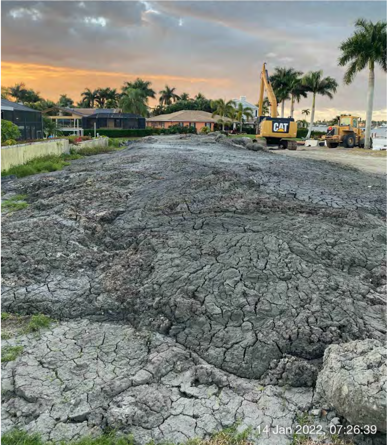
Removed material from Canal CC-CC at dewatering site at 1300 Curlew Avenue
