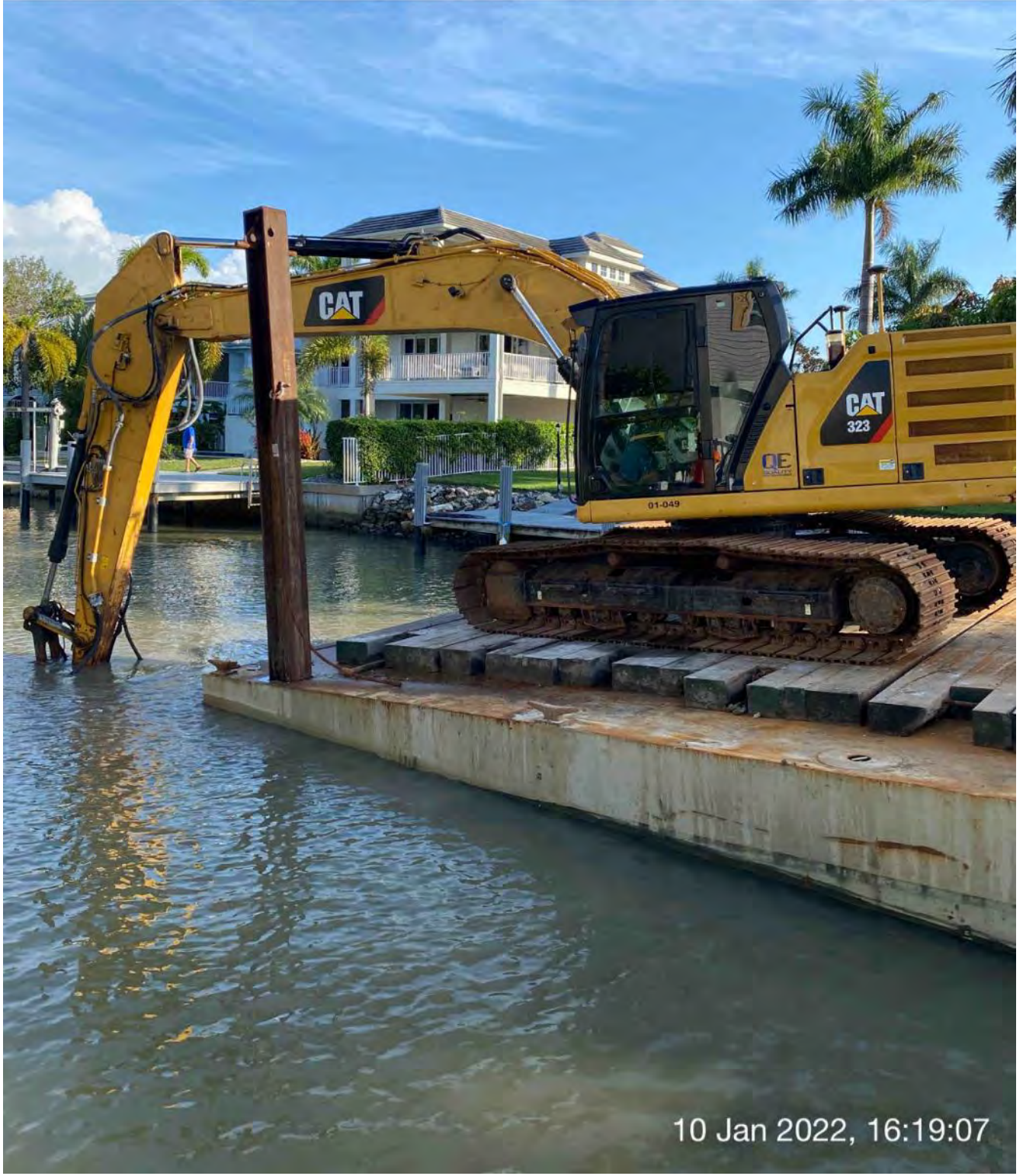
323 excavator grinding rock at station 4+25
