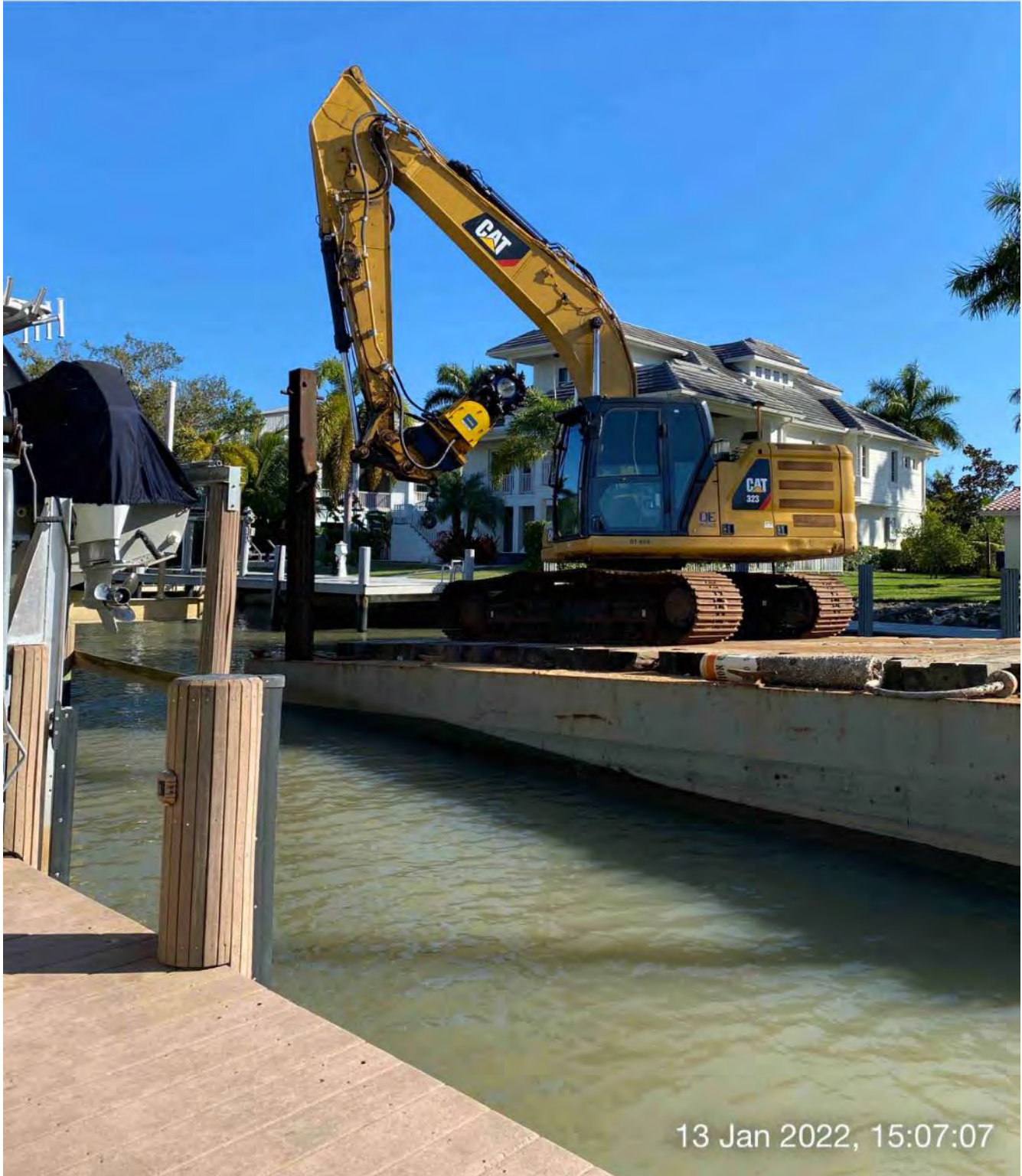
323 excavator with Epiroc grinder on barge at station 4+25
