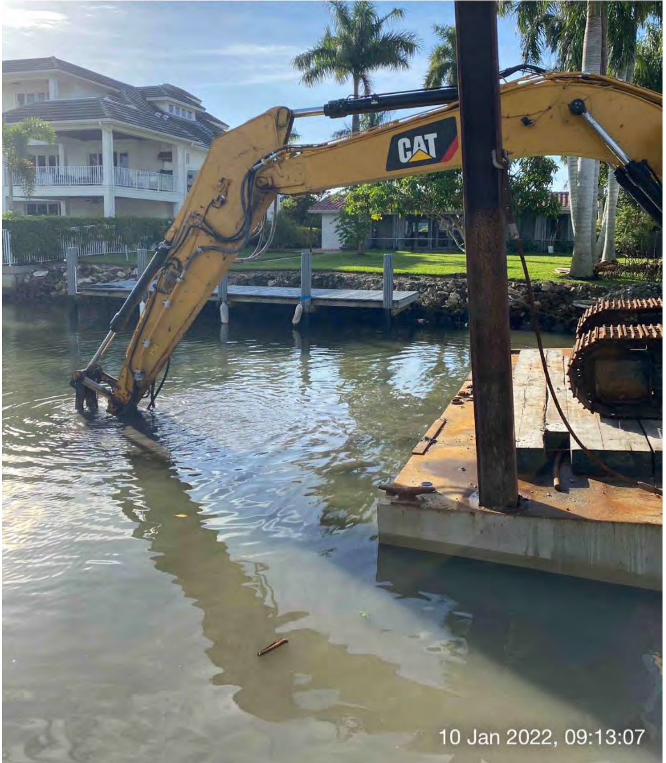
323 excavator grinding rock at station 4+00
