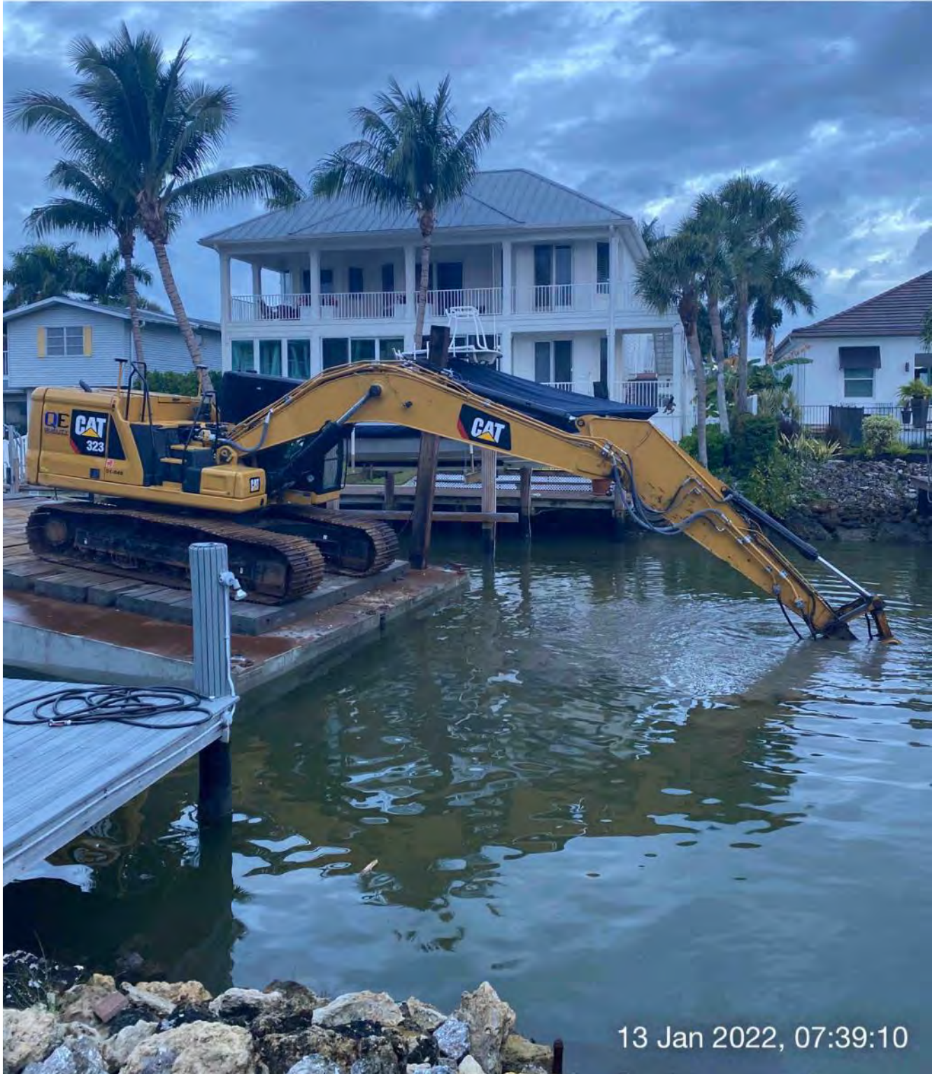
323 excavator grinding rock at station 4+25
