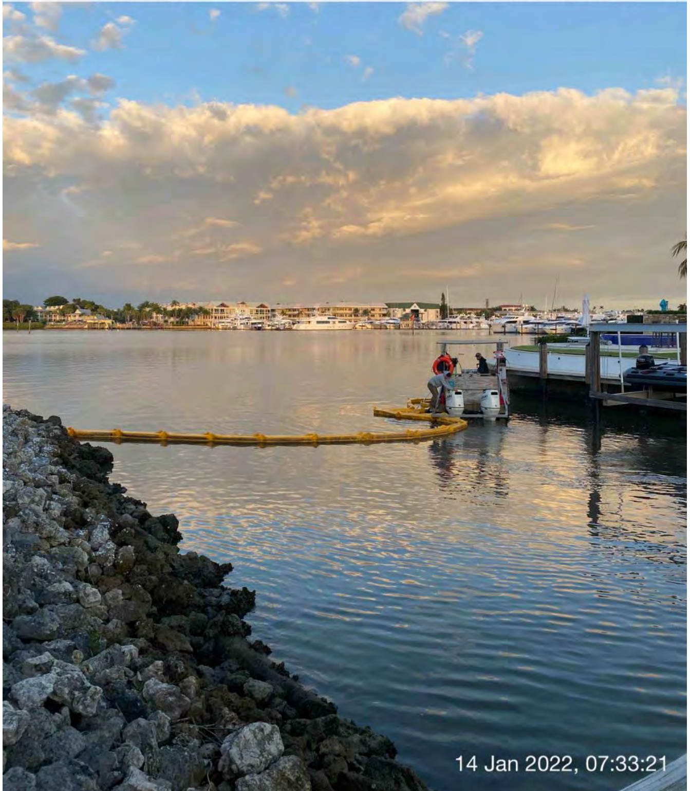
Installing turbidity curtain across the mouth of Canal BB-BB with push boat
