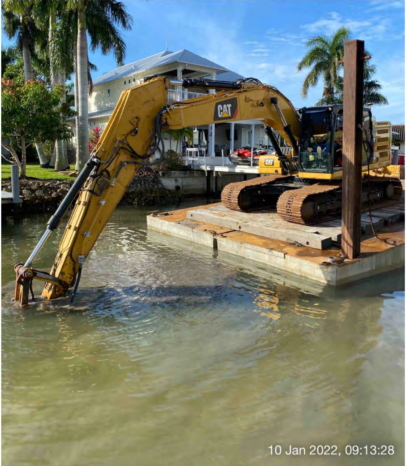
323 excavator grinding rock at station 4+00
