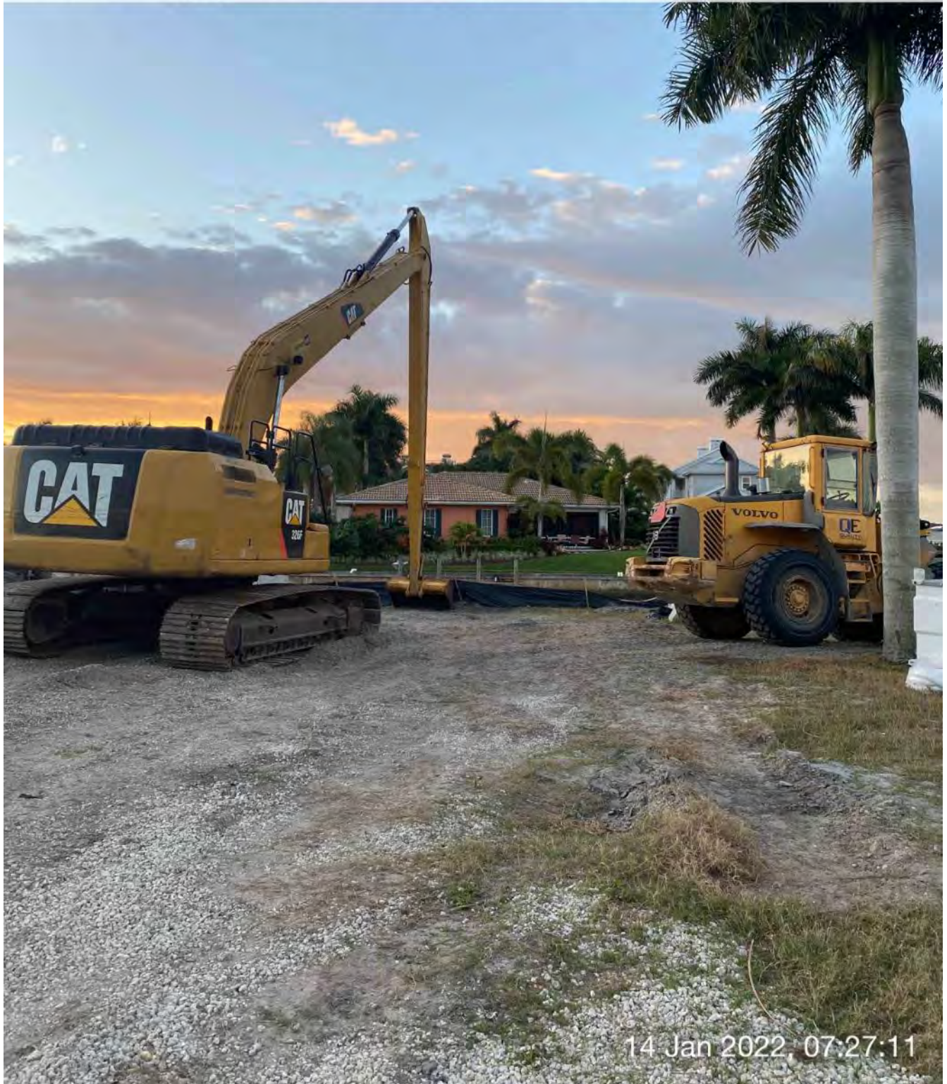
326 excavator and front end loader on south end of 1300 Curlew Avenue
