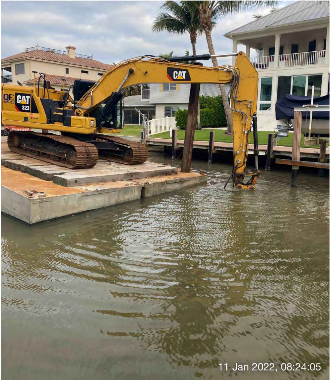
323 excavator grinding rock at station 4+00
