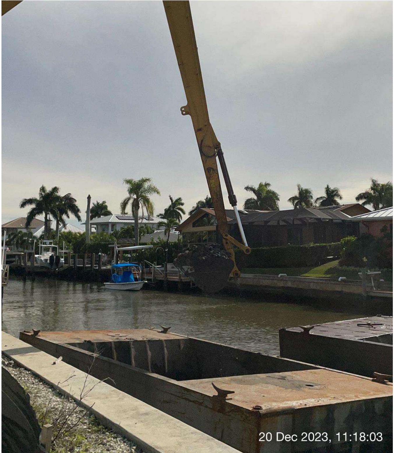
Long reach excavator removing sediment from hopper.
