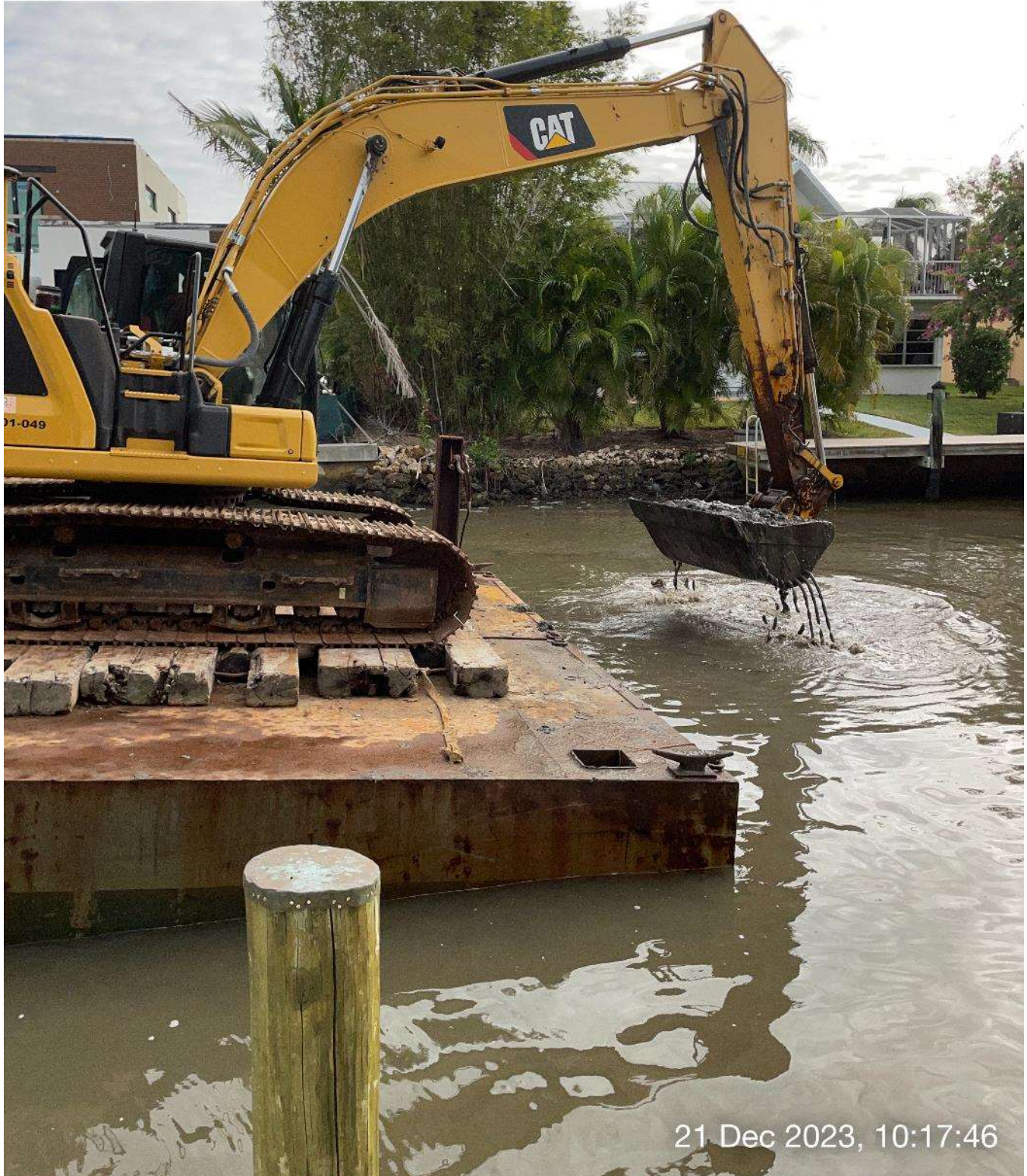
323 excavator removing sediment at station 1+25 in Canal AA-AA.
