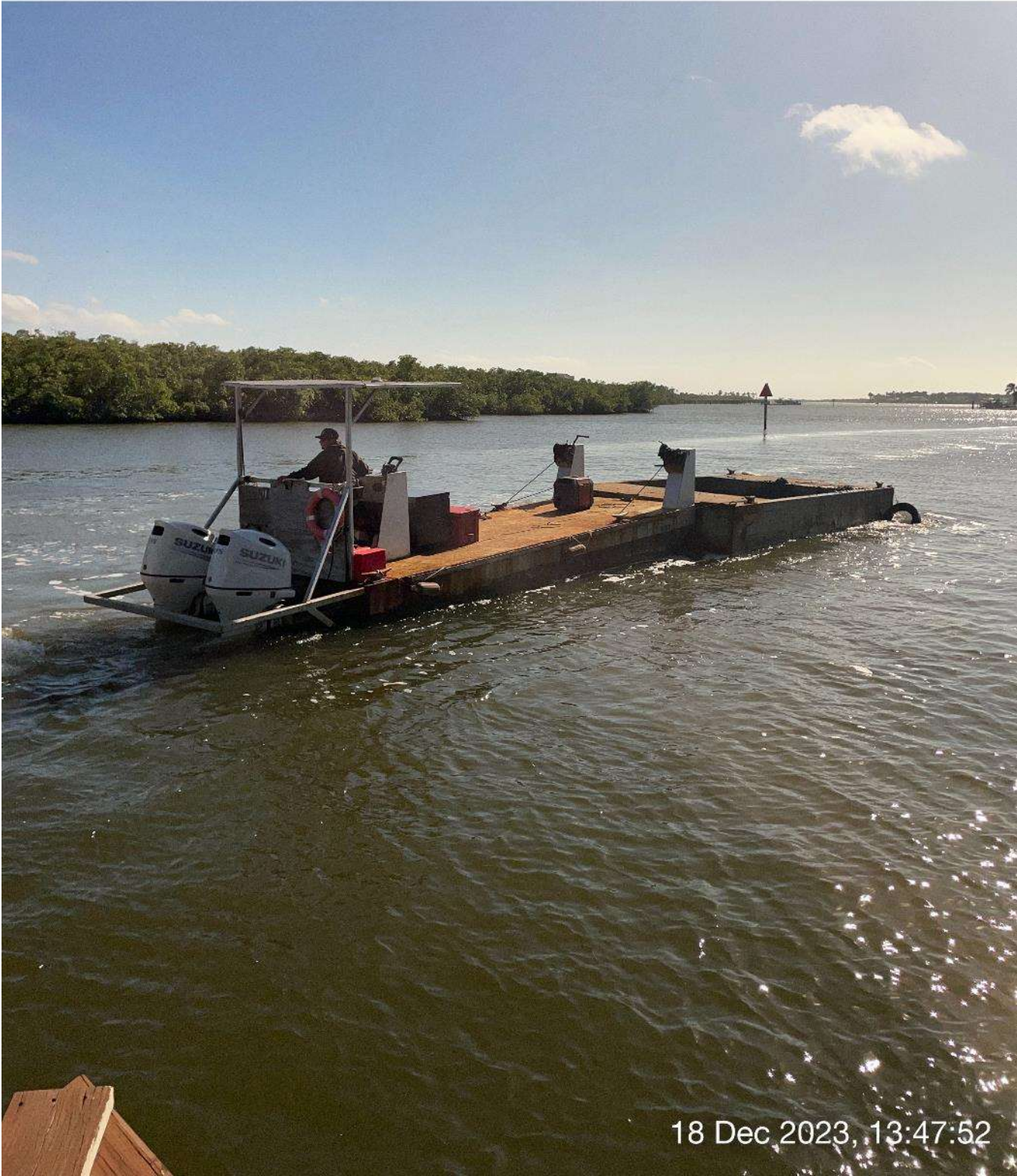
Push boat taking hopper to staging area.
