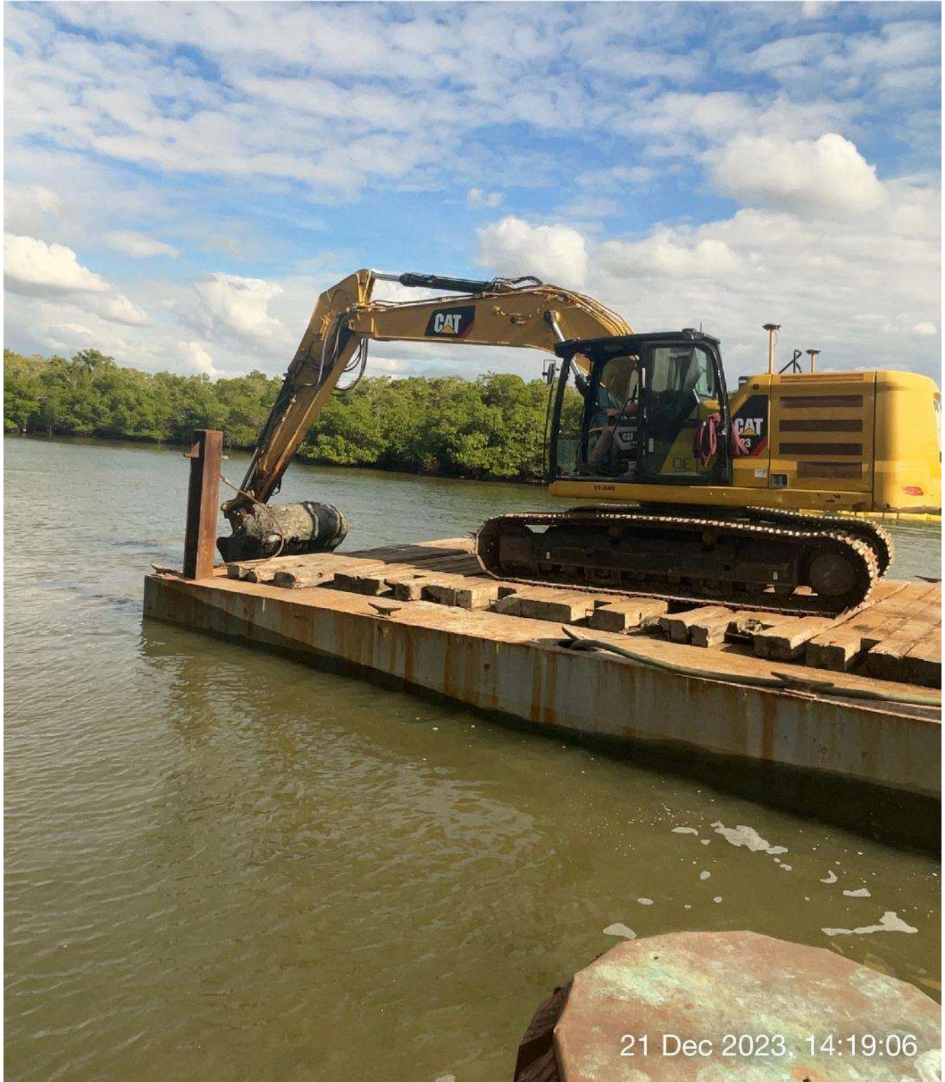
323 excavator removing sediment at station 3+50 in Canal Main B.
