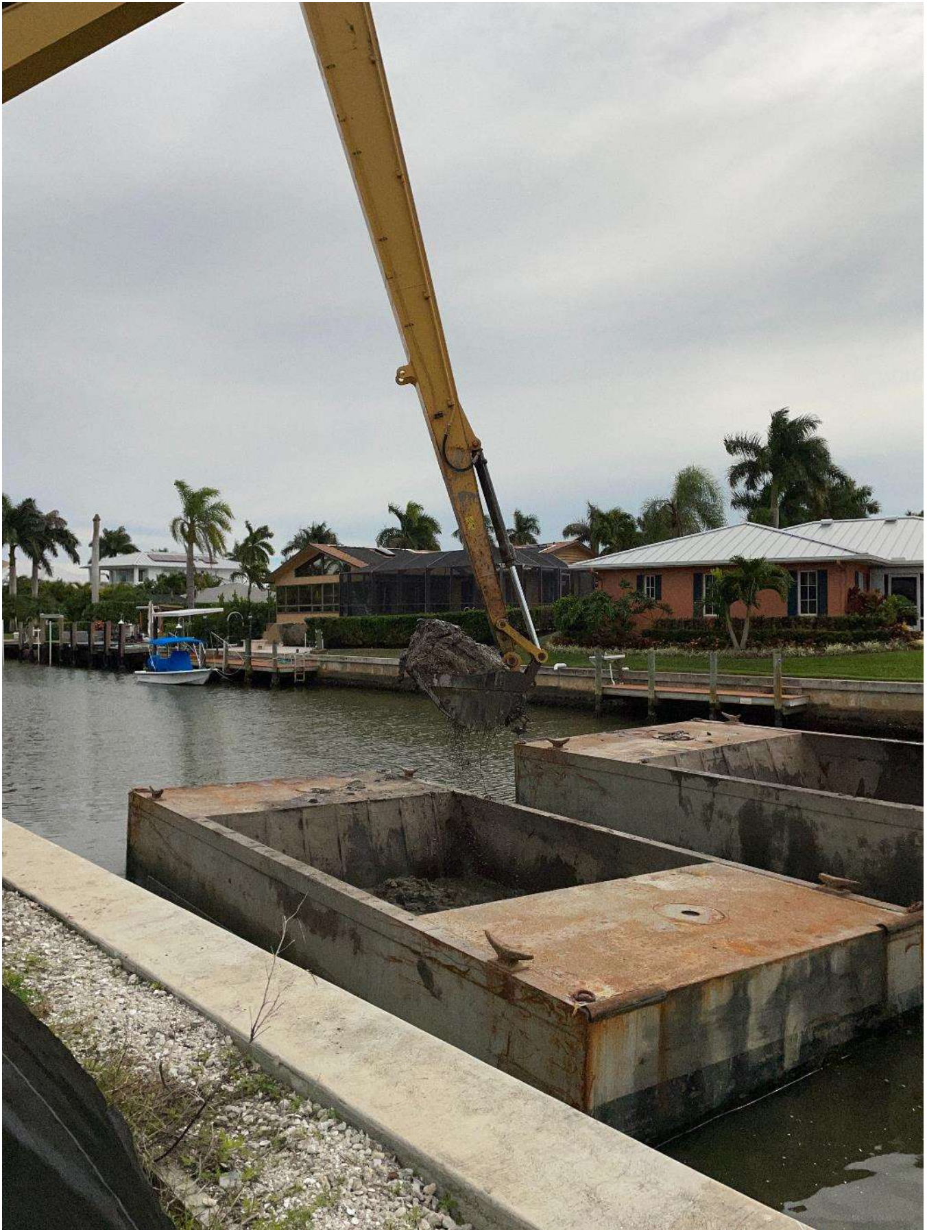
Long reach excavator removing sediment from hopper.
