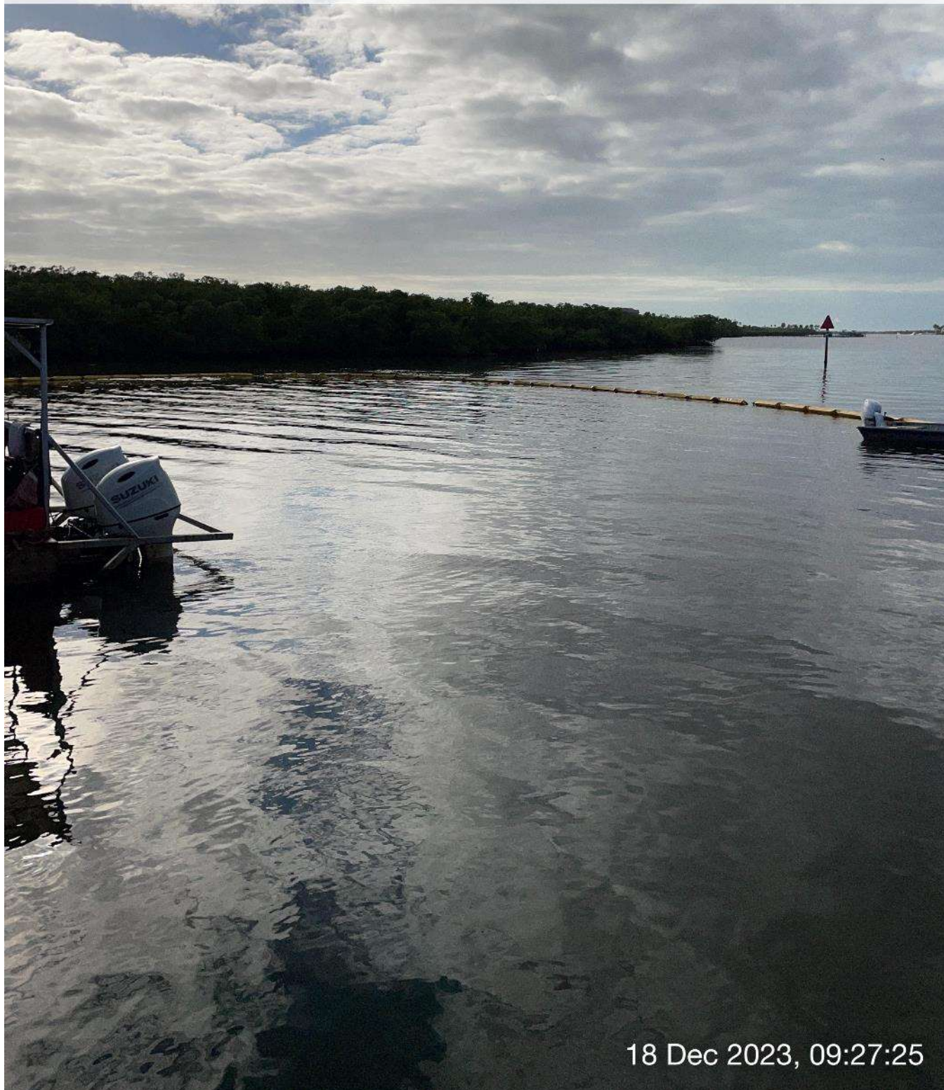
Turbidity curtain in place at station 3+50 in Canal Main B.
