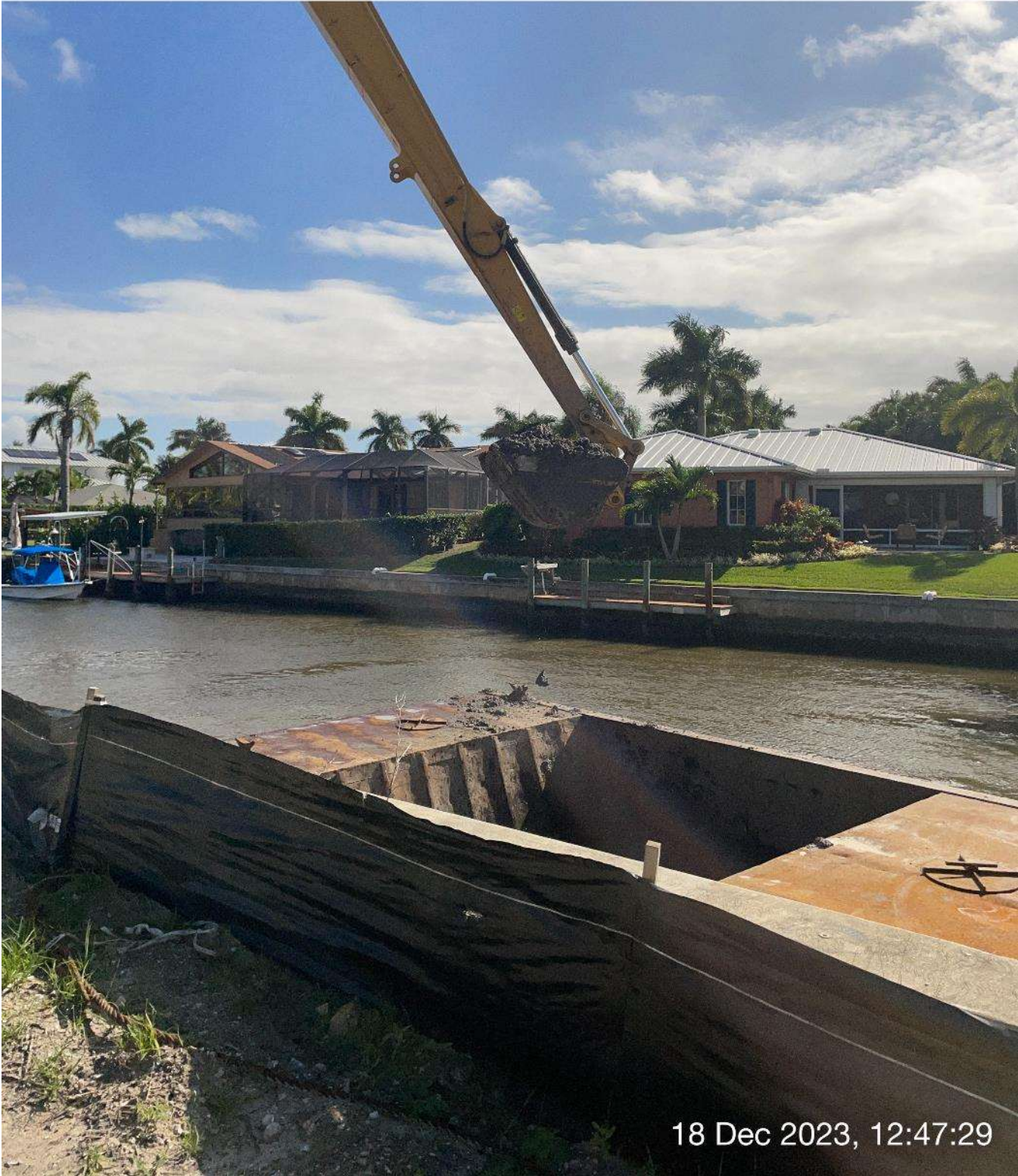
Long reach excavator removing sediment from hopper.
