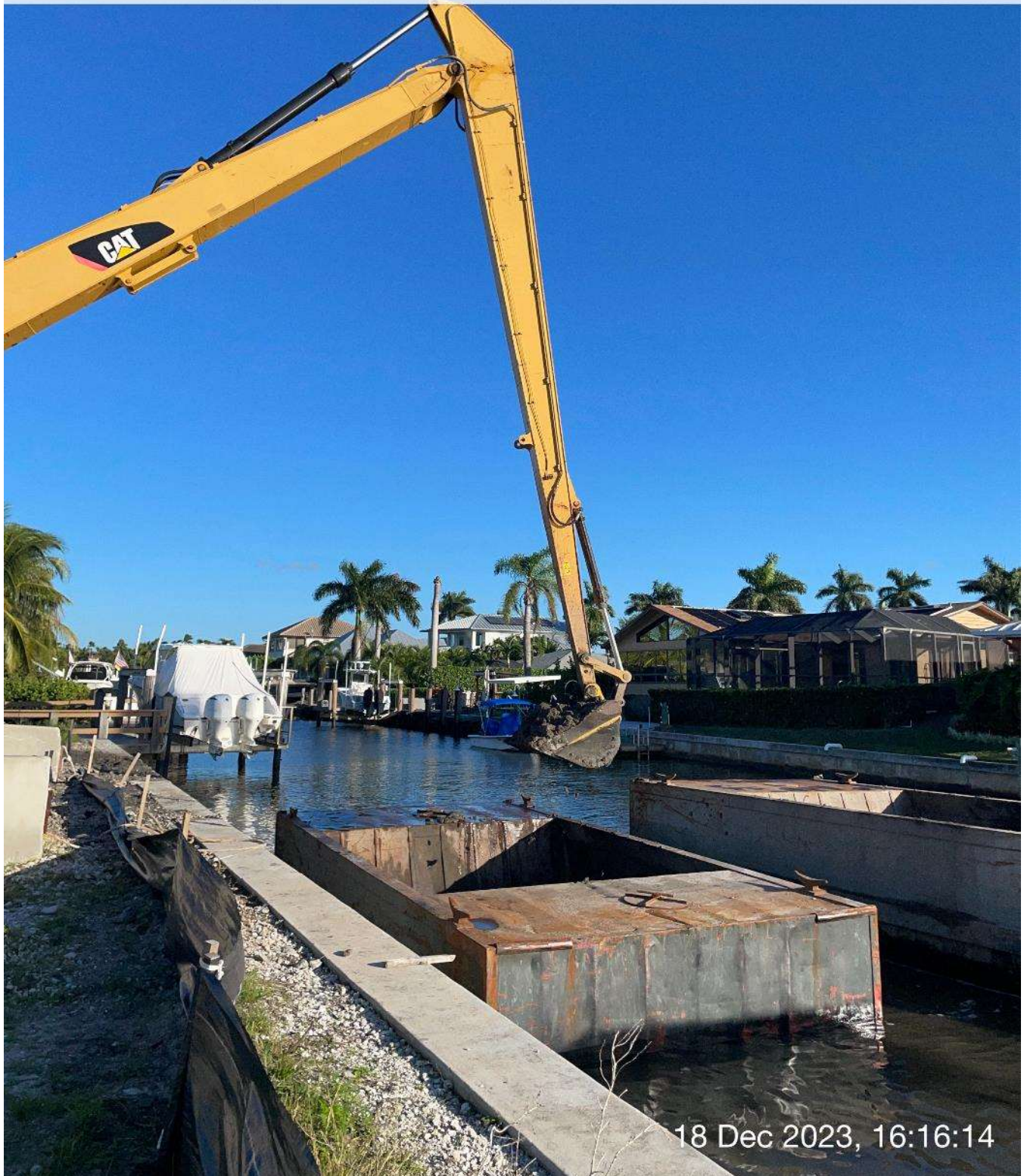
Long reach excavator removing sediment from hopper.
