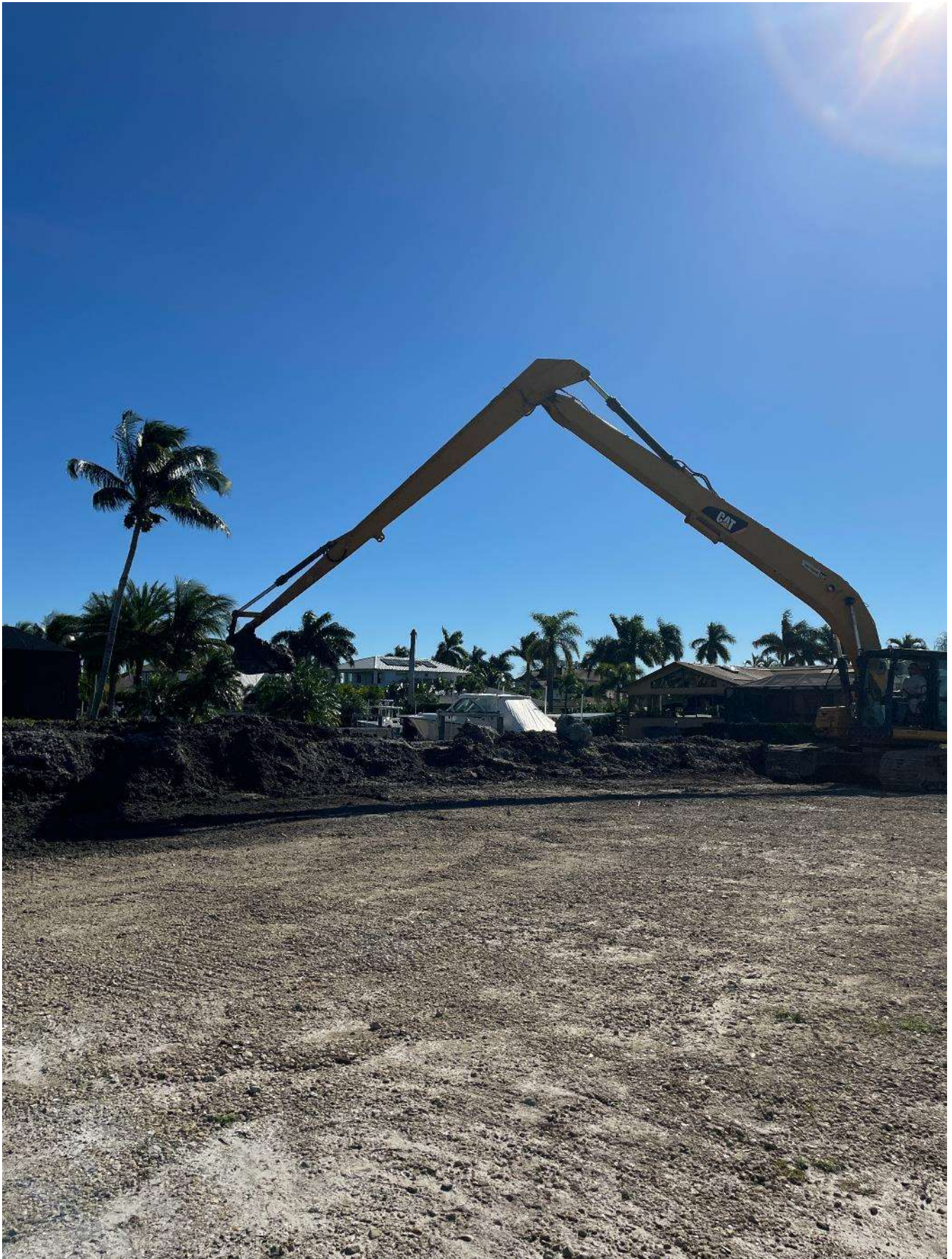
Long reach excavator spreading sediment onto staging area.
