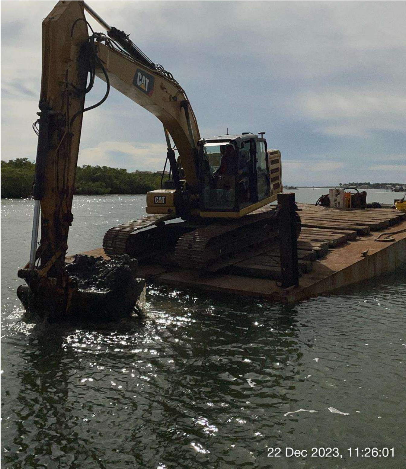
323 excavator removing sediment at station 3+00 in Canal Main B.
