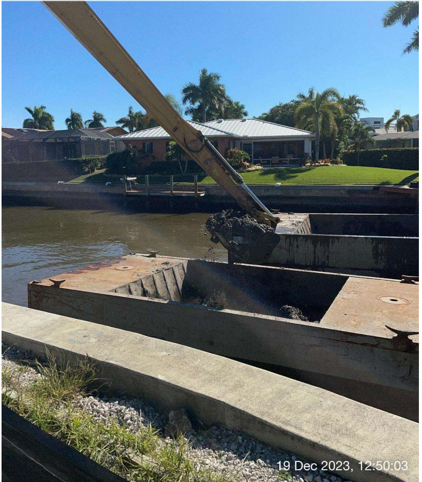
Long reach excavator removing sediment from hopper.
