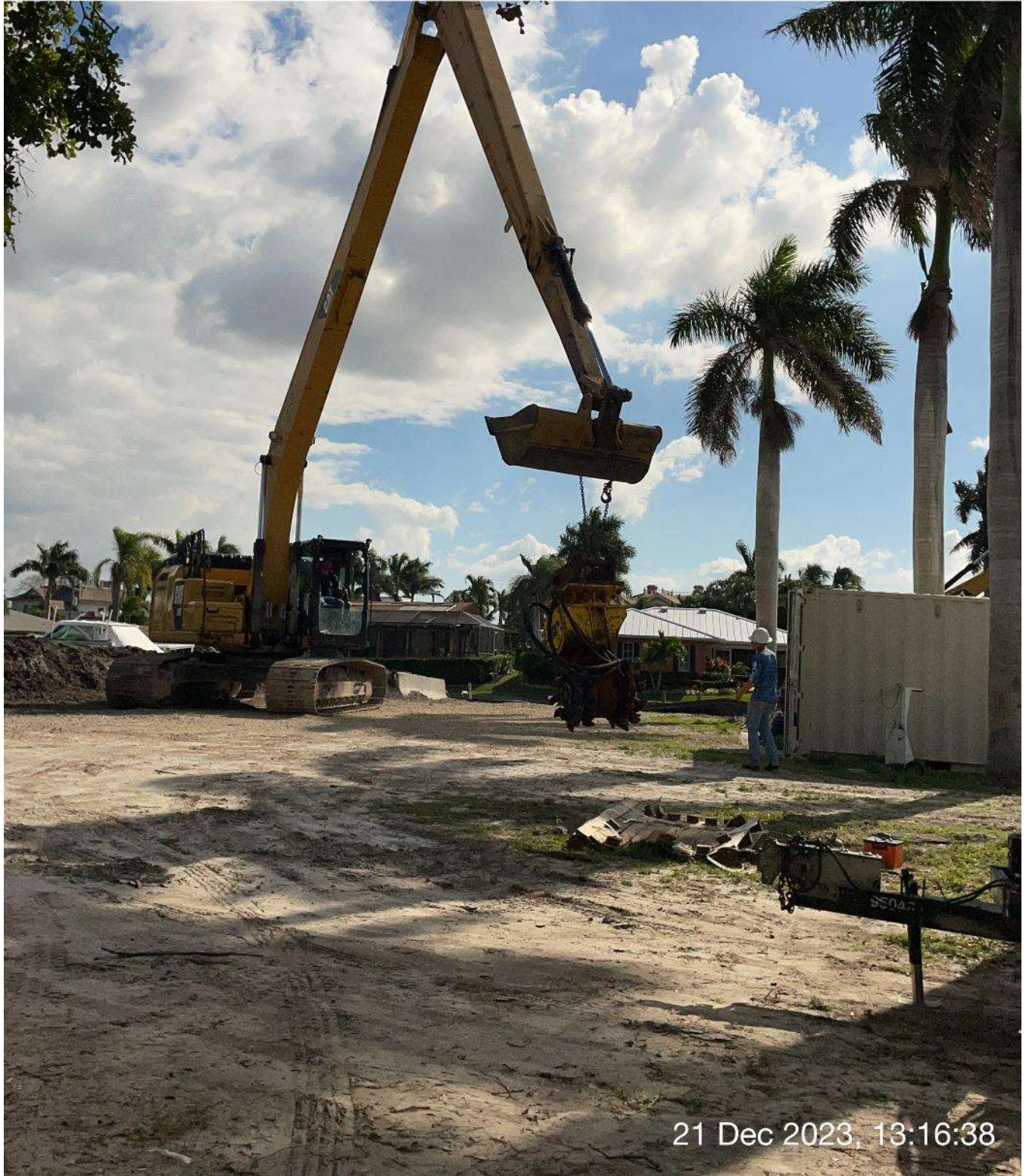
Long reach excavator loading Epiroc grinder onto the barge.
