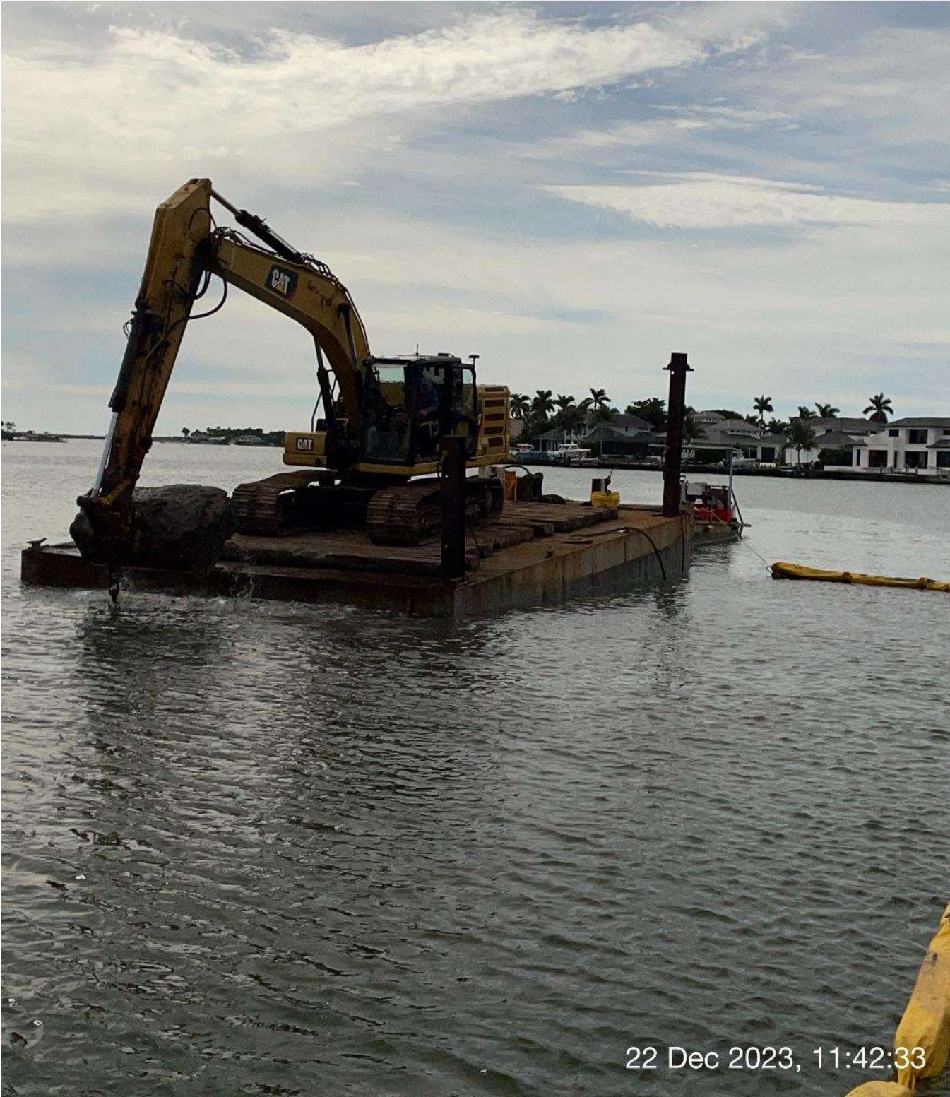
323 excavator removing sediment at station 2+75 in Canal Main B.
