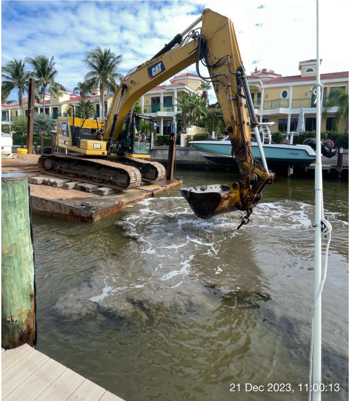
323 excavator removing sediment at station 2+75 in Canal Y-Y.
