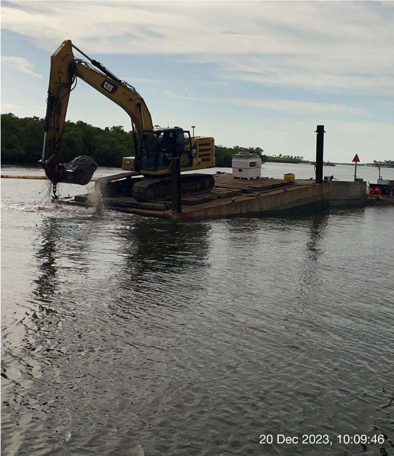
323 excavator removing sediment at station 3+75 in Canal Main B.
