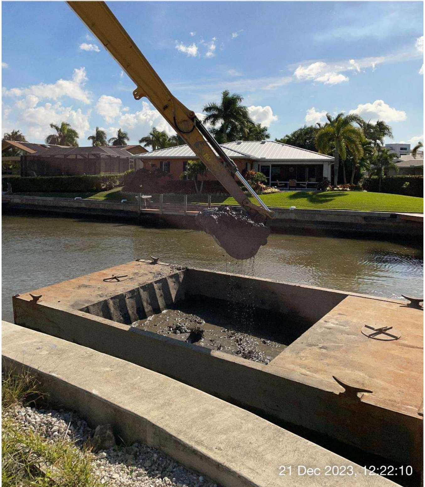
Long reach excavator removing sediment from hopper.
