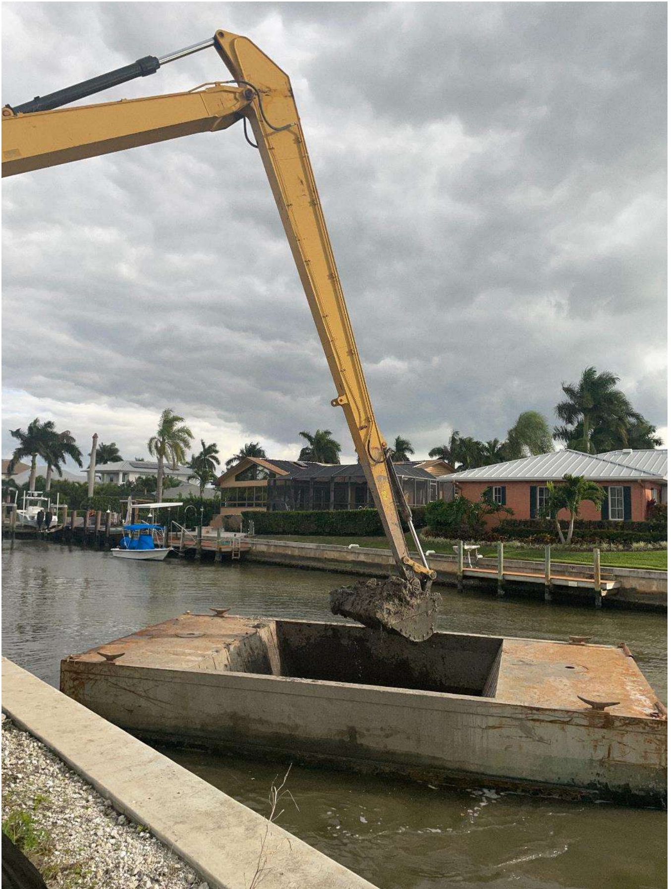
Long reach excavator removing sediment from hopper.
