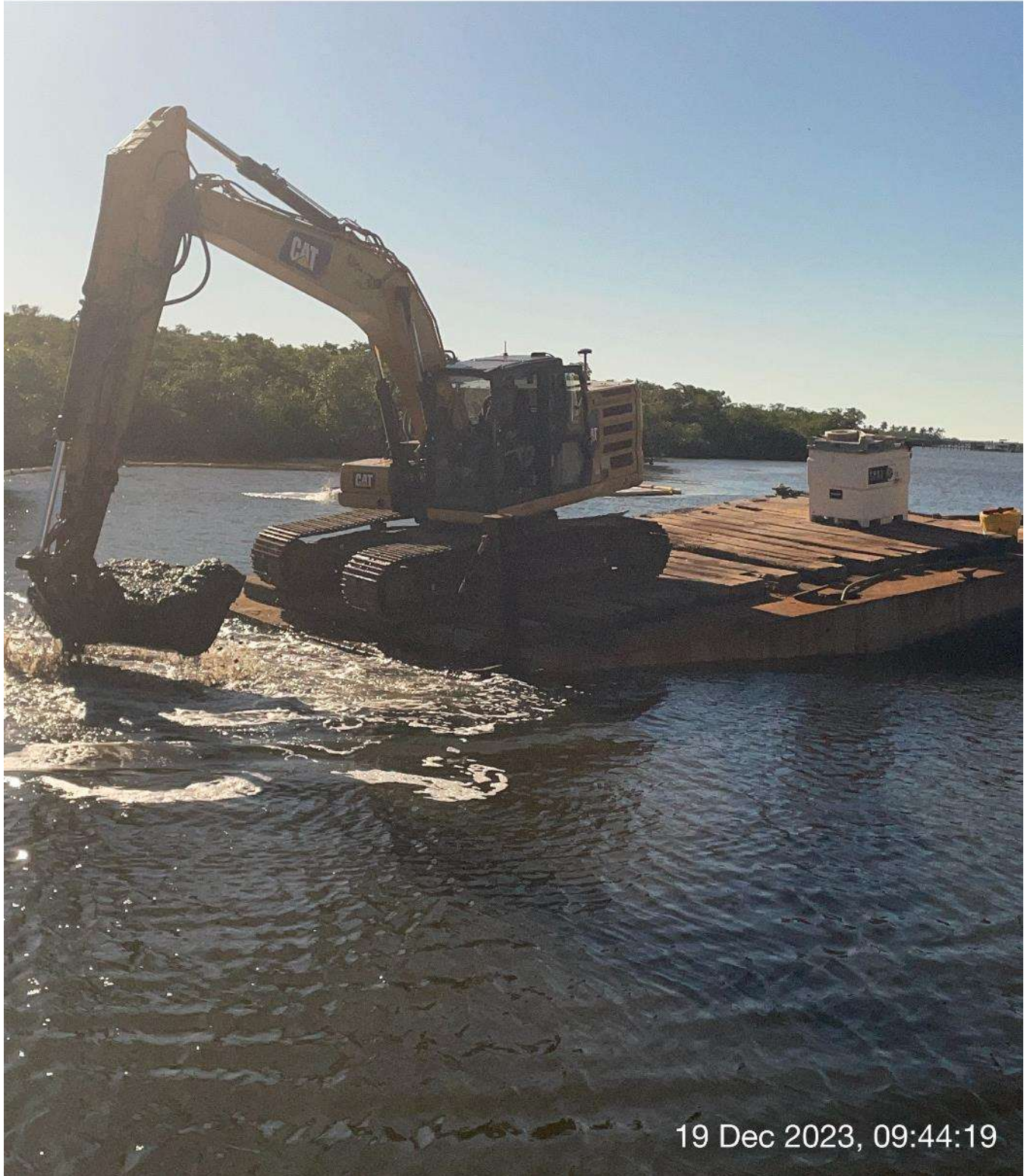
323 excavator removing sediment at station 4+25 in Canal Main B.
