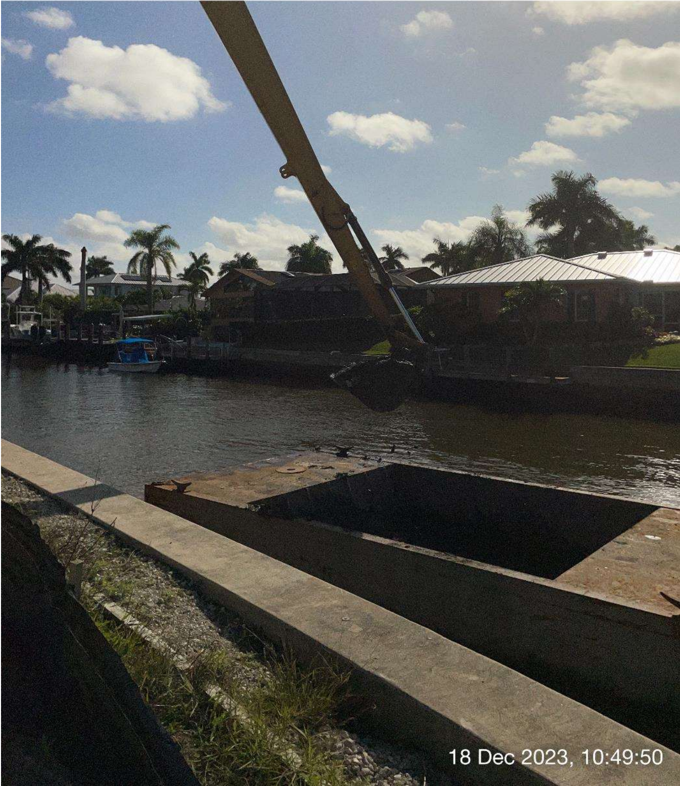
Long reach excavator removing sediment from hopper.
