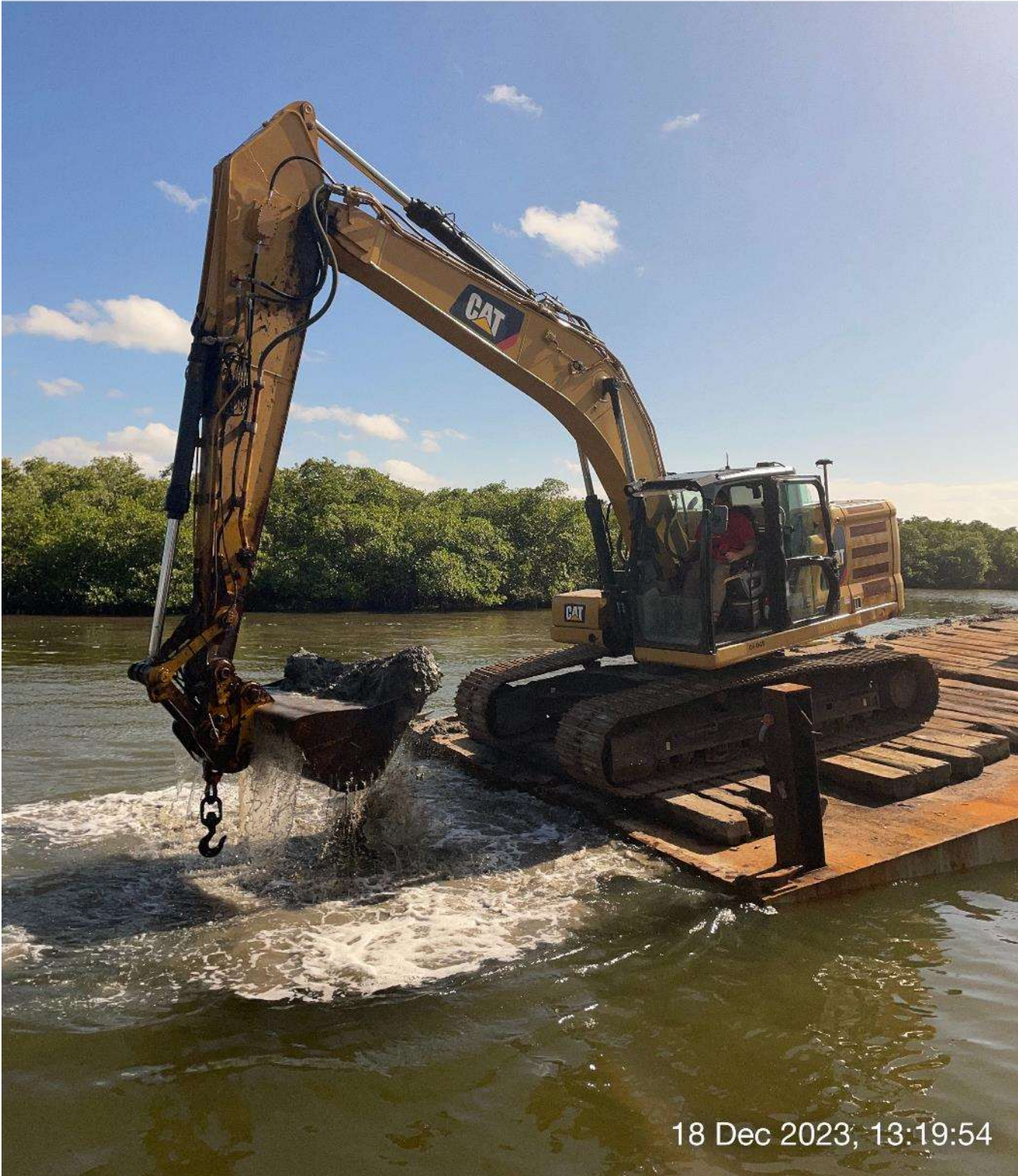
323 excavator removing sediment at station 4+50 in Canal Main B.
