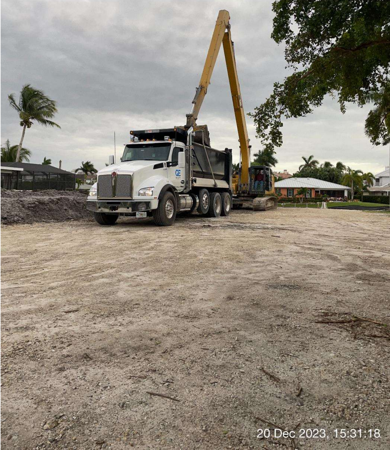
Long reach excavator loading material into dump truck.
