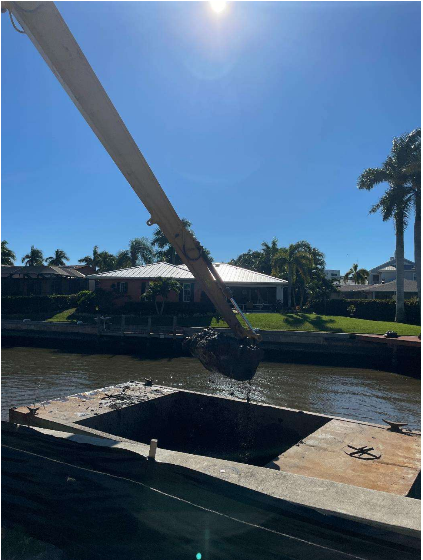
Long reach excavator removing sediment from hopper.
