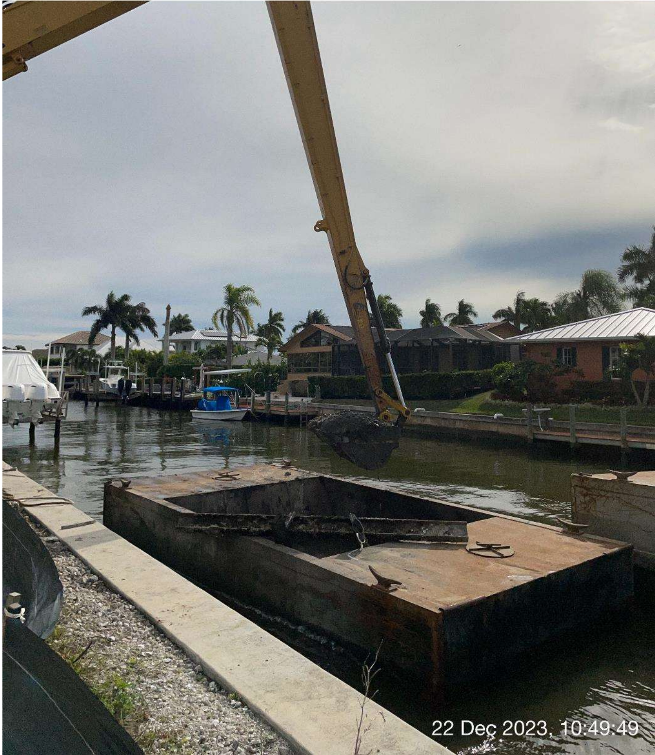
Long reach excavator removing sediment from hopper.
