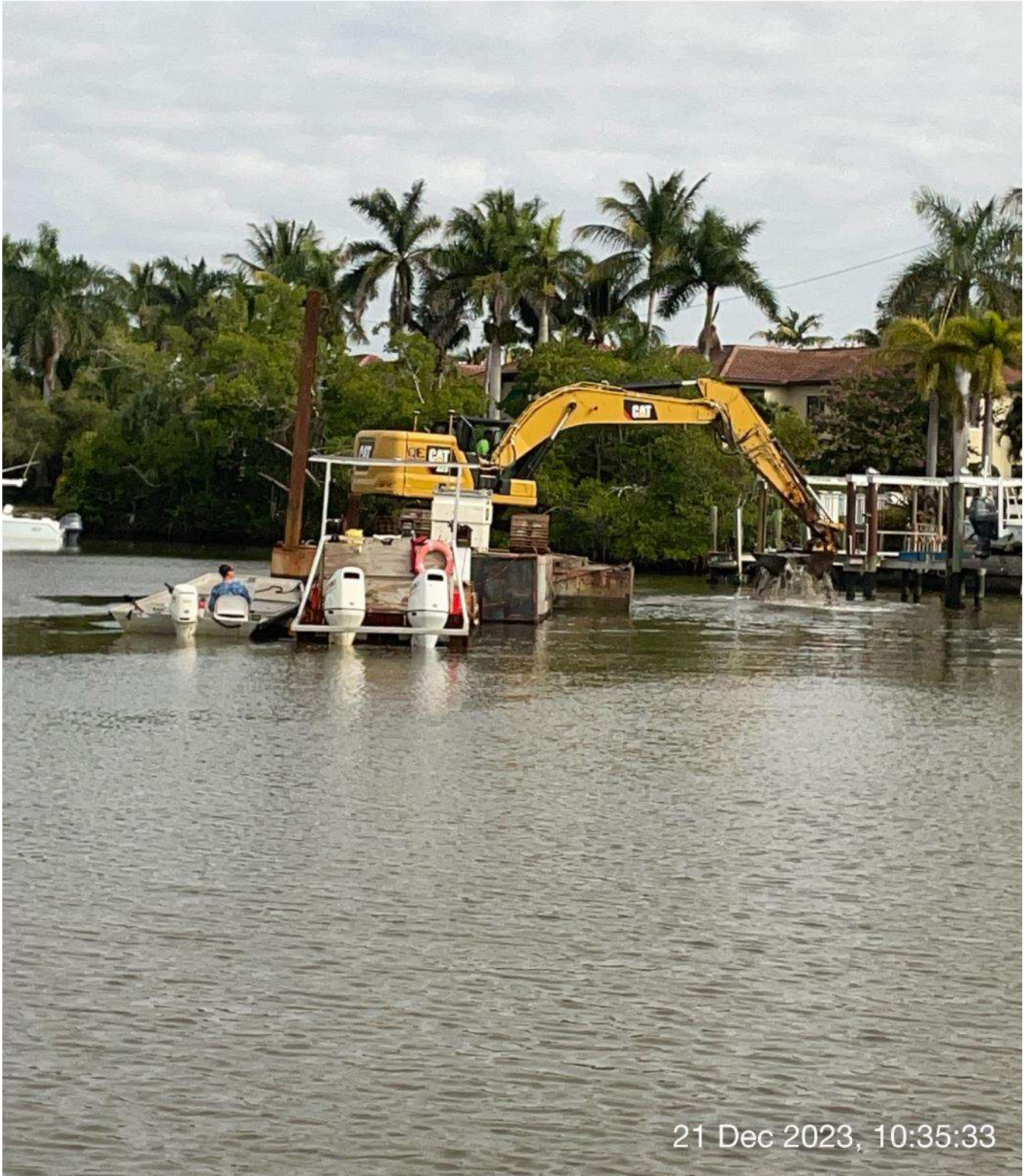
323 excavator removing sediment at station 14+65 in Canal X-X.
