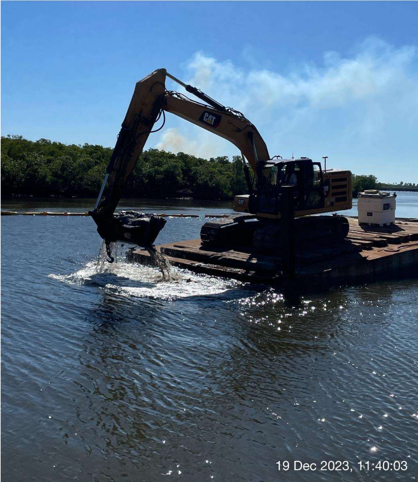
323 excavator removing sediment at station 4+00 in Canal Main B.
