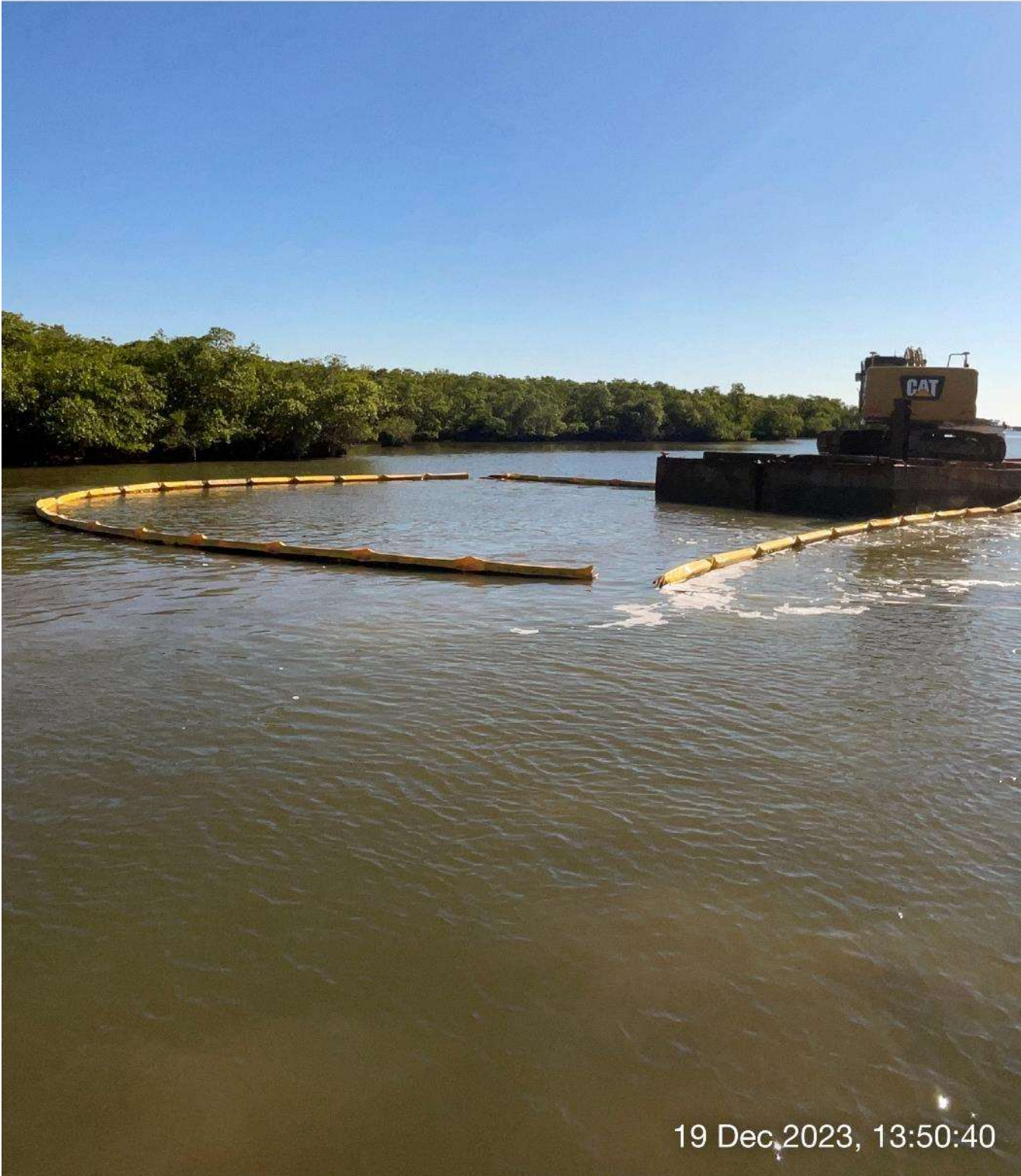
Turbidity curtain in place around barge.
