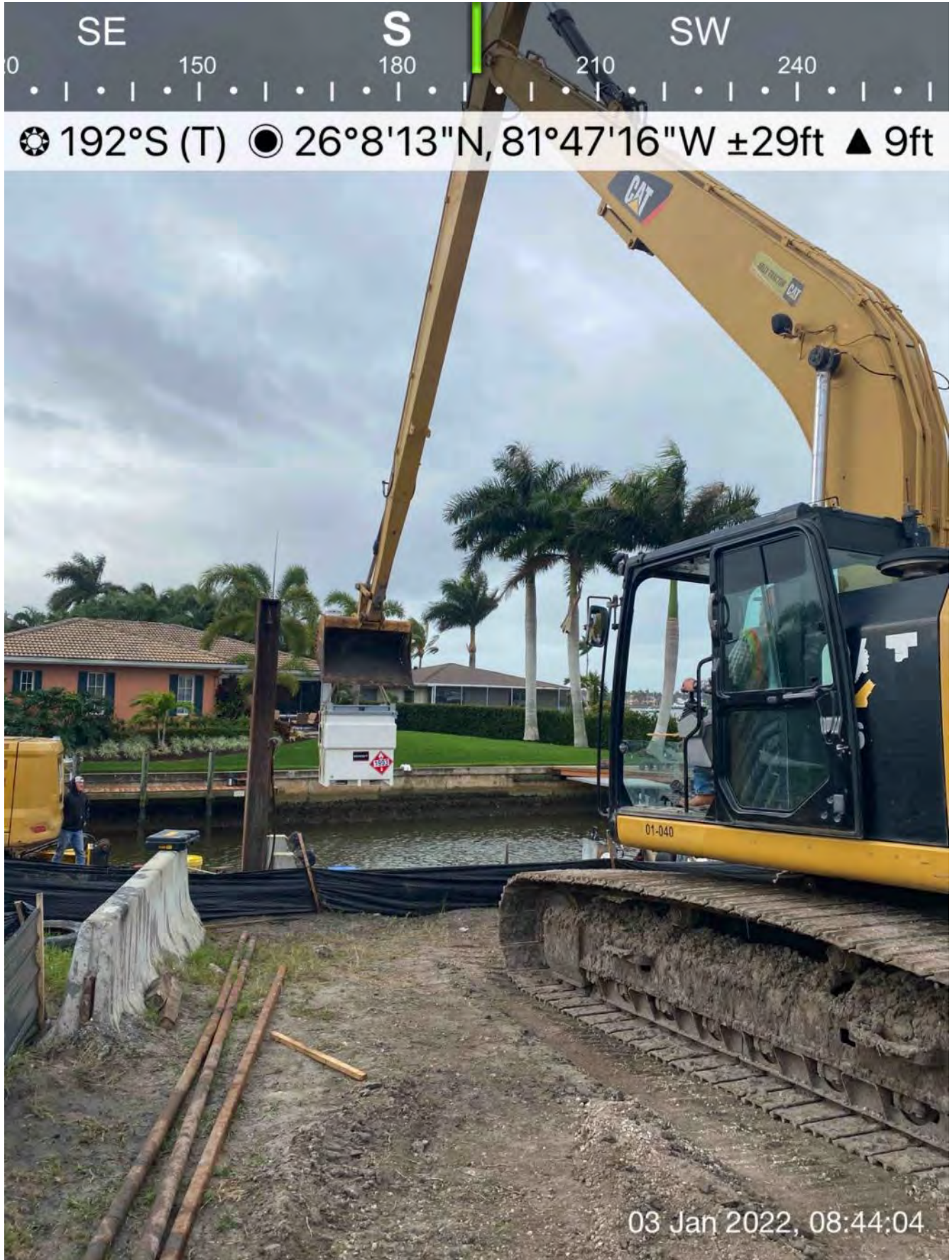
326 excavator lifting fuel cube to the barge to refuel 323 excavator
