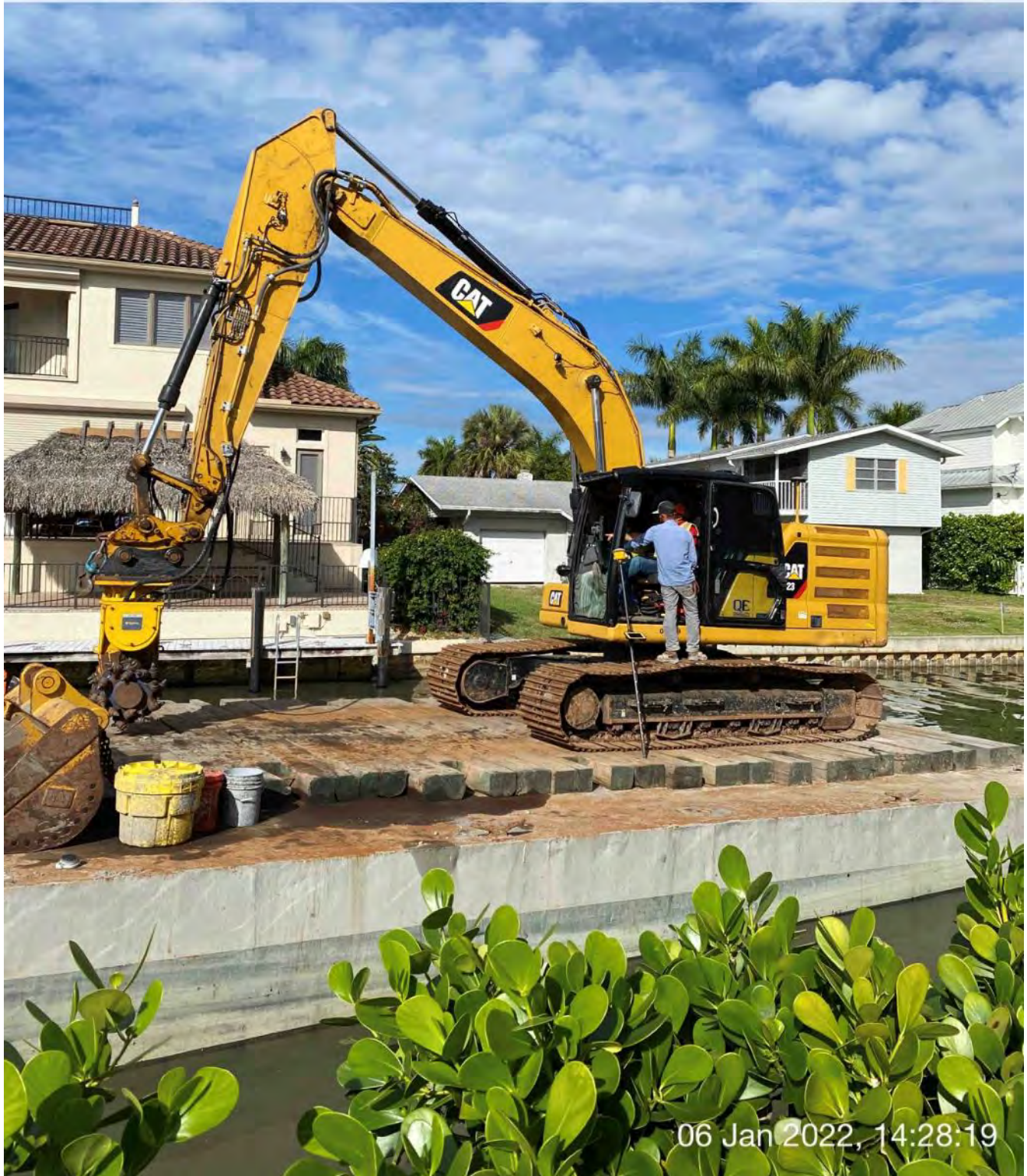
Checking 323 excavator elevation readings
