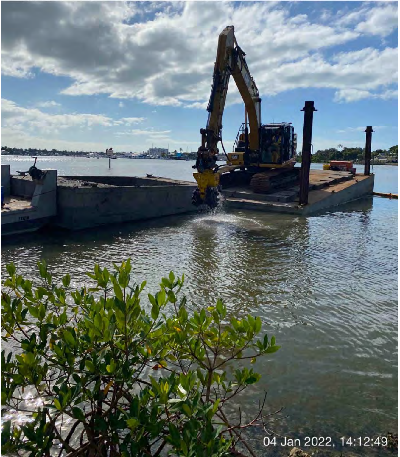
323 excavator grinding rock at station 0+50
