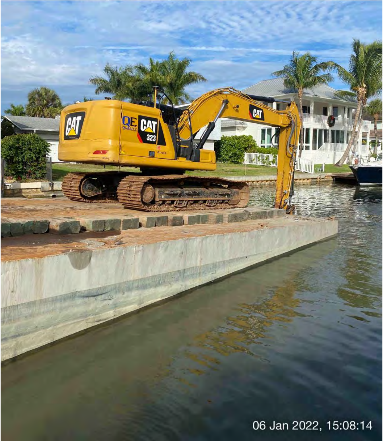
323 excavator checking bottom elevations and grinding material at station 3+00 in Canal BB-BB
