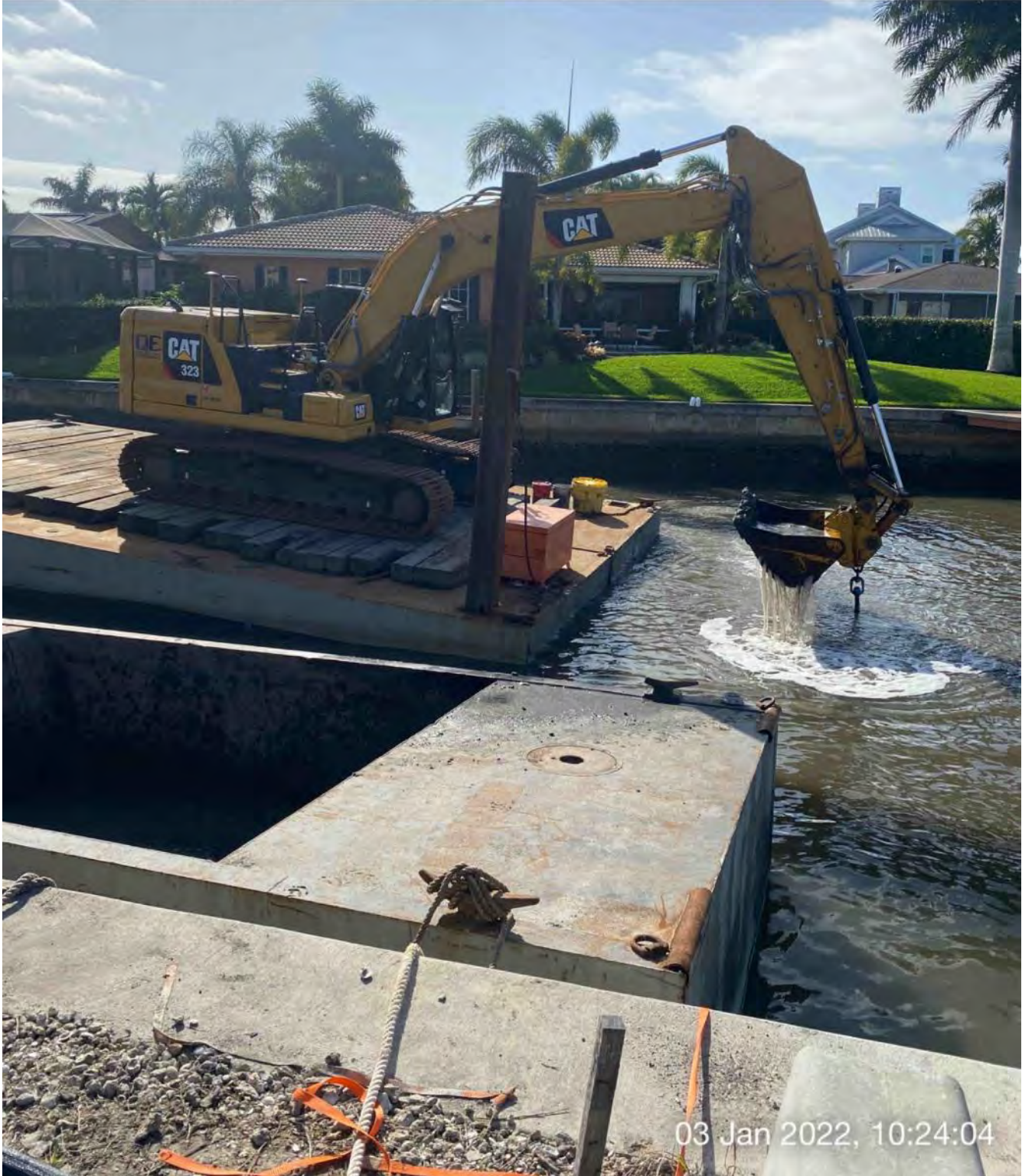
323 excavator removing material and transferring to hopper at station 1+50
