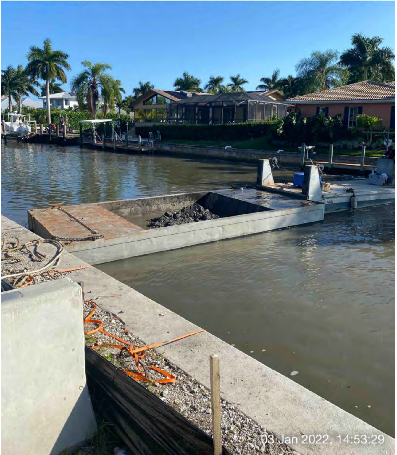
Full hopper of material at station 1+50
