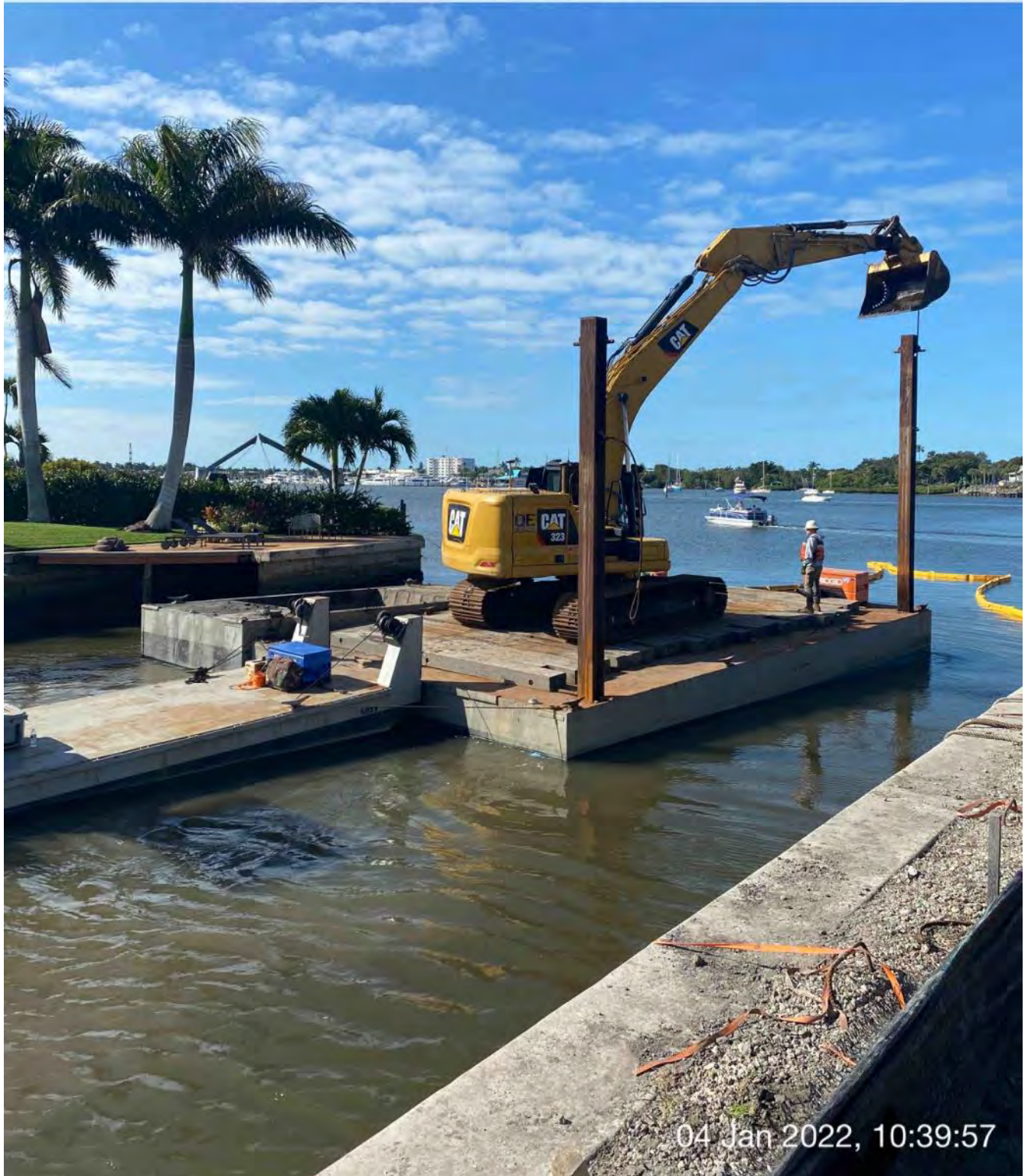
323 excavator lifting spud to allow push boat to move barge at station 1+00
