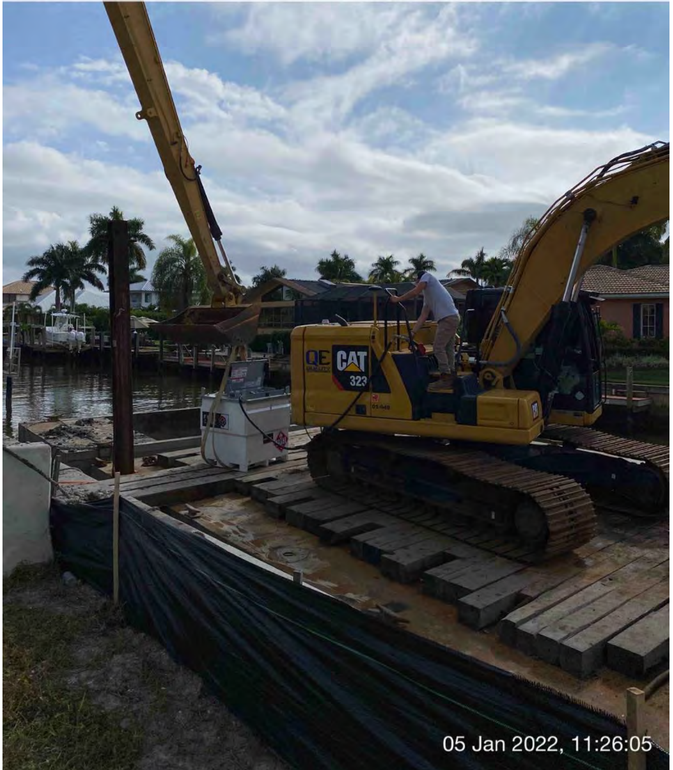
Small fuel cube on the barge being used to refuel 323 excavator
