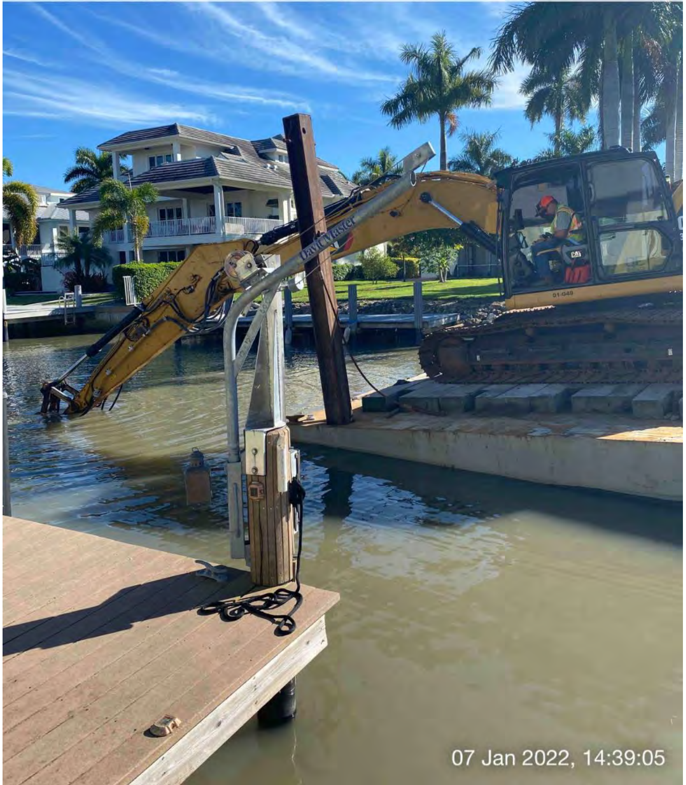
323 excavator grinding rock at station 4+00 in Canal BB-BB
