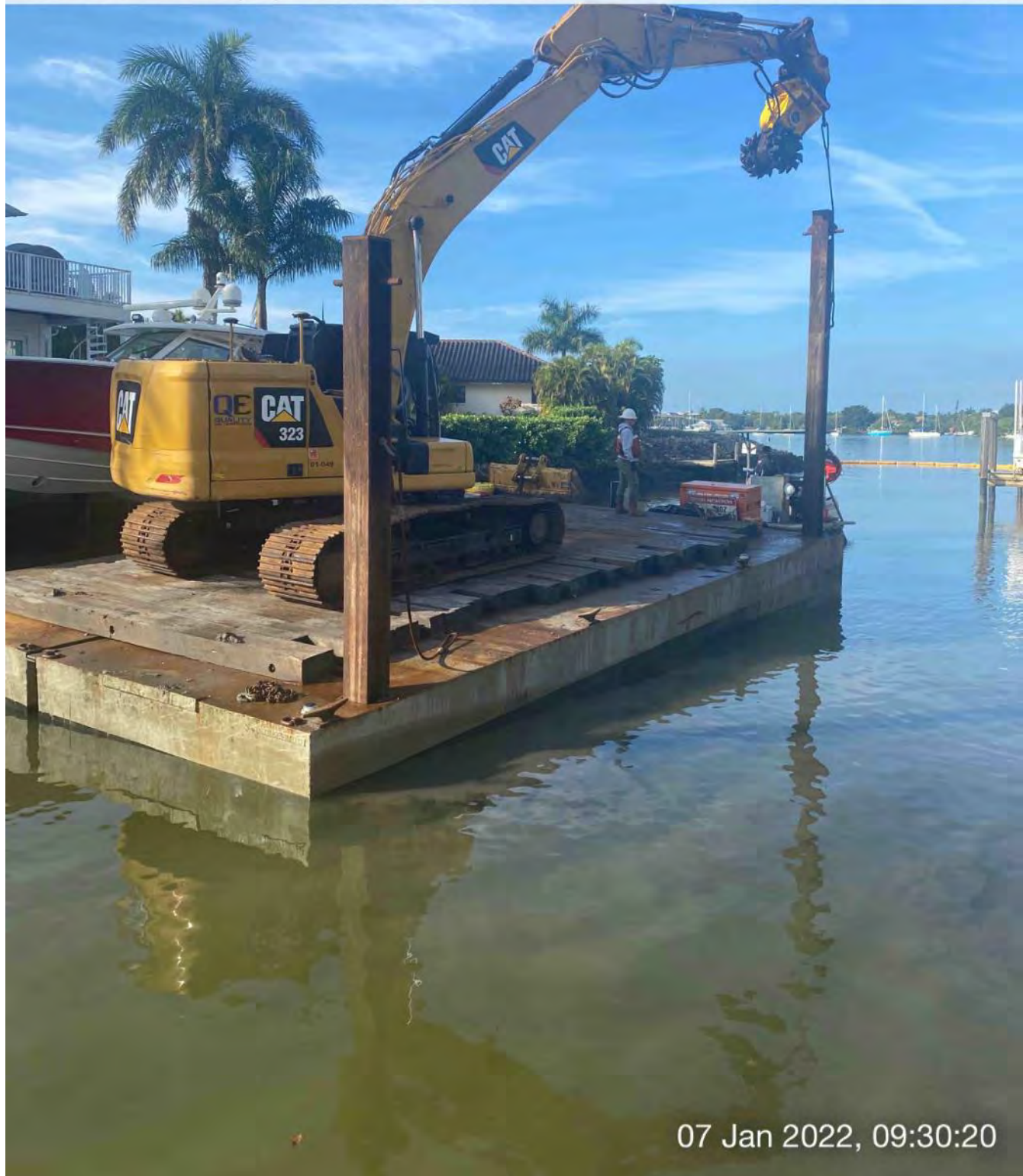
323 excavator lifting spud to allow push boat to move barge at station 3+50 in Canal BB-BB
