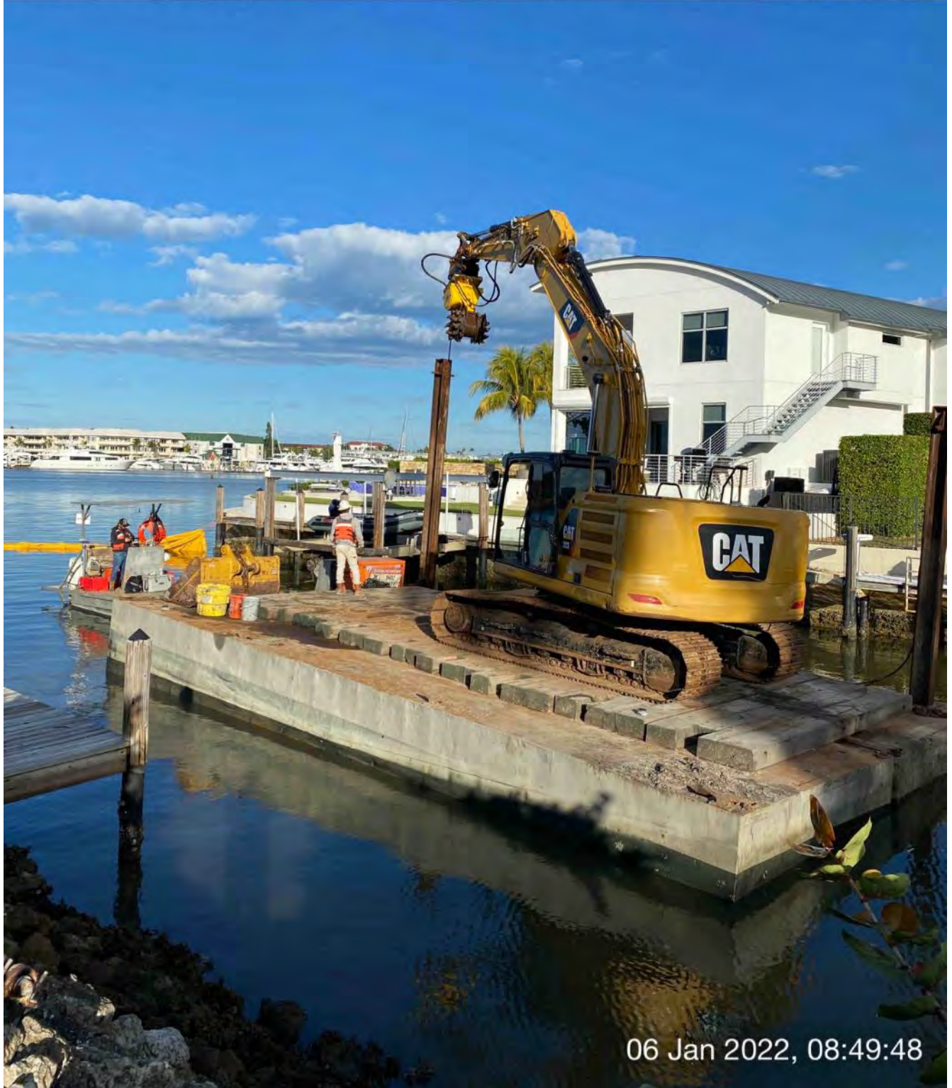
323 excavator lifting spud to allow push boat to move barge at station 2+00 in Canal BB-BB
