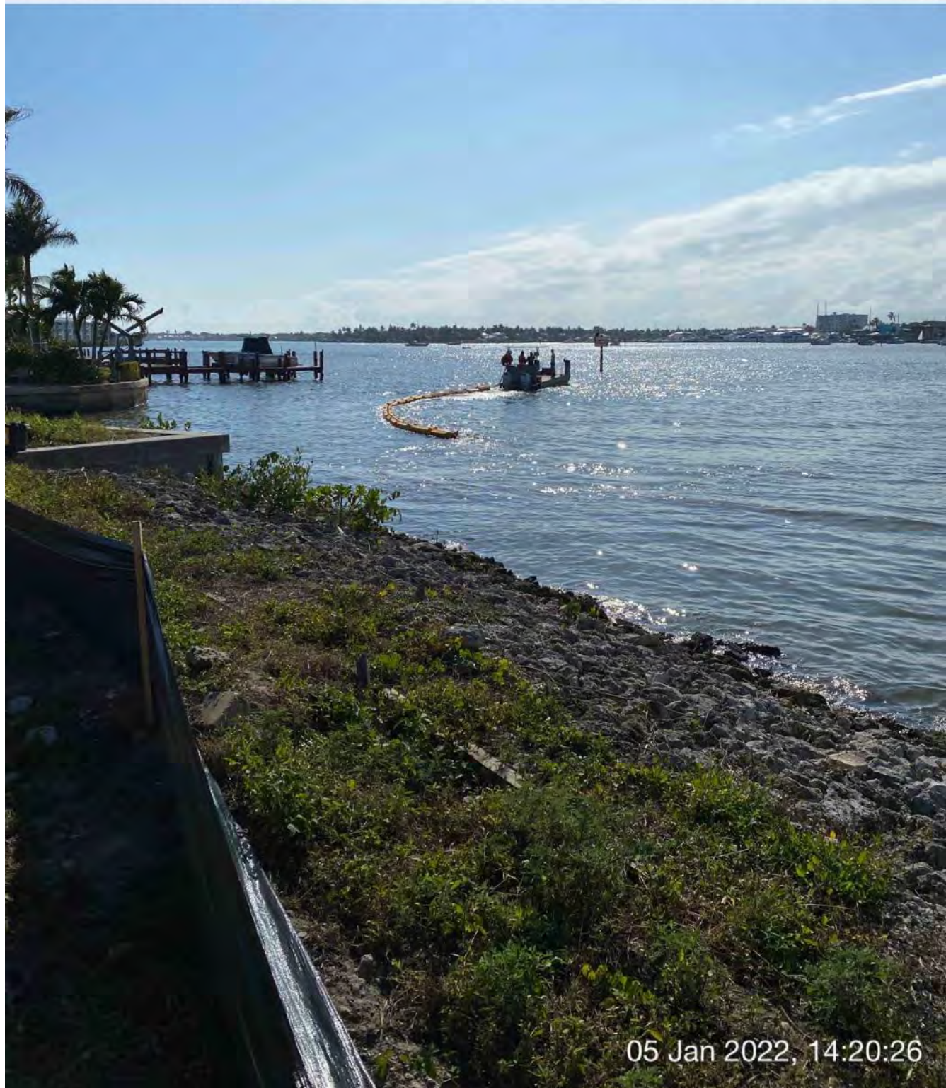
Push boat transporting turbidity curtain from Canal CC-CC to Canal BB-BB
