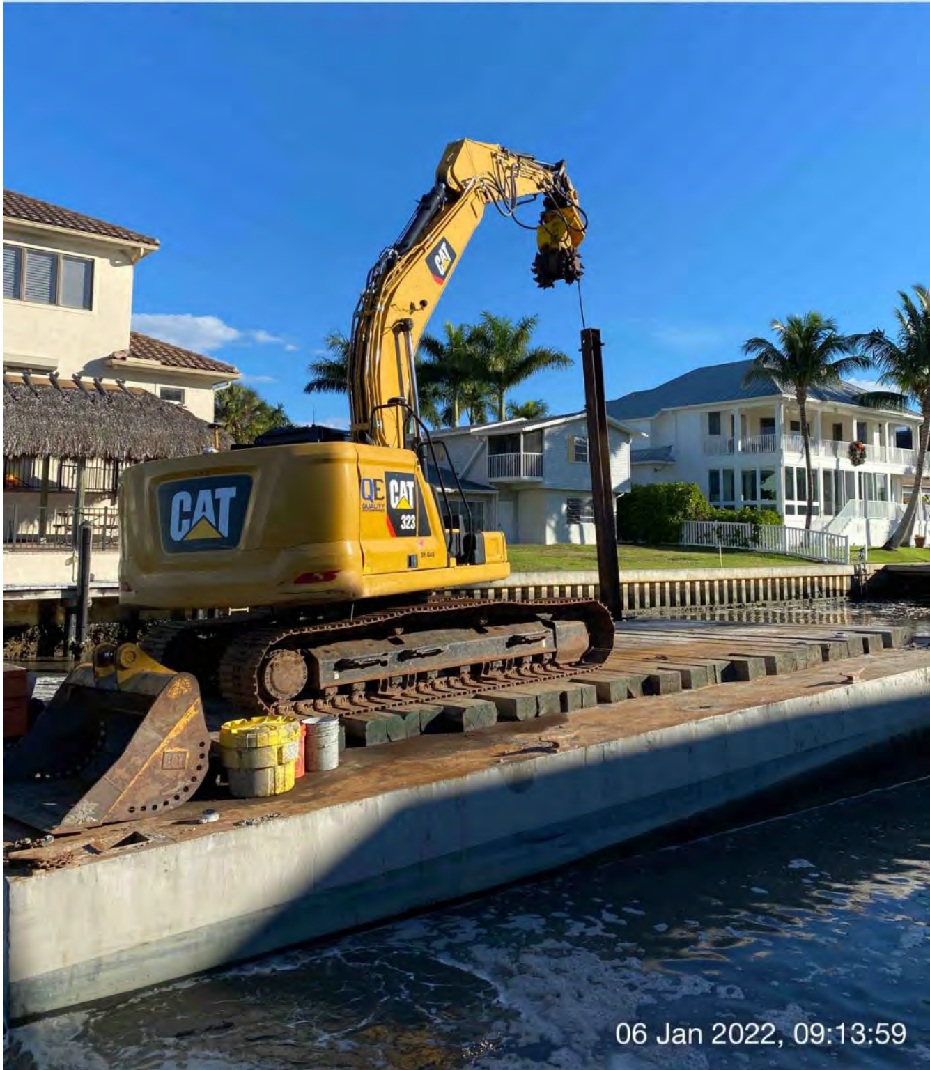
323 excavator lifting spud to allow push boat to move barge at station 2+50 in Canal BB-BB
