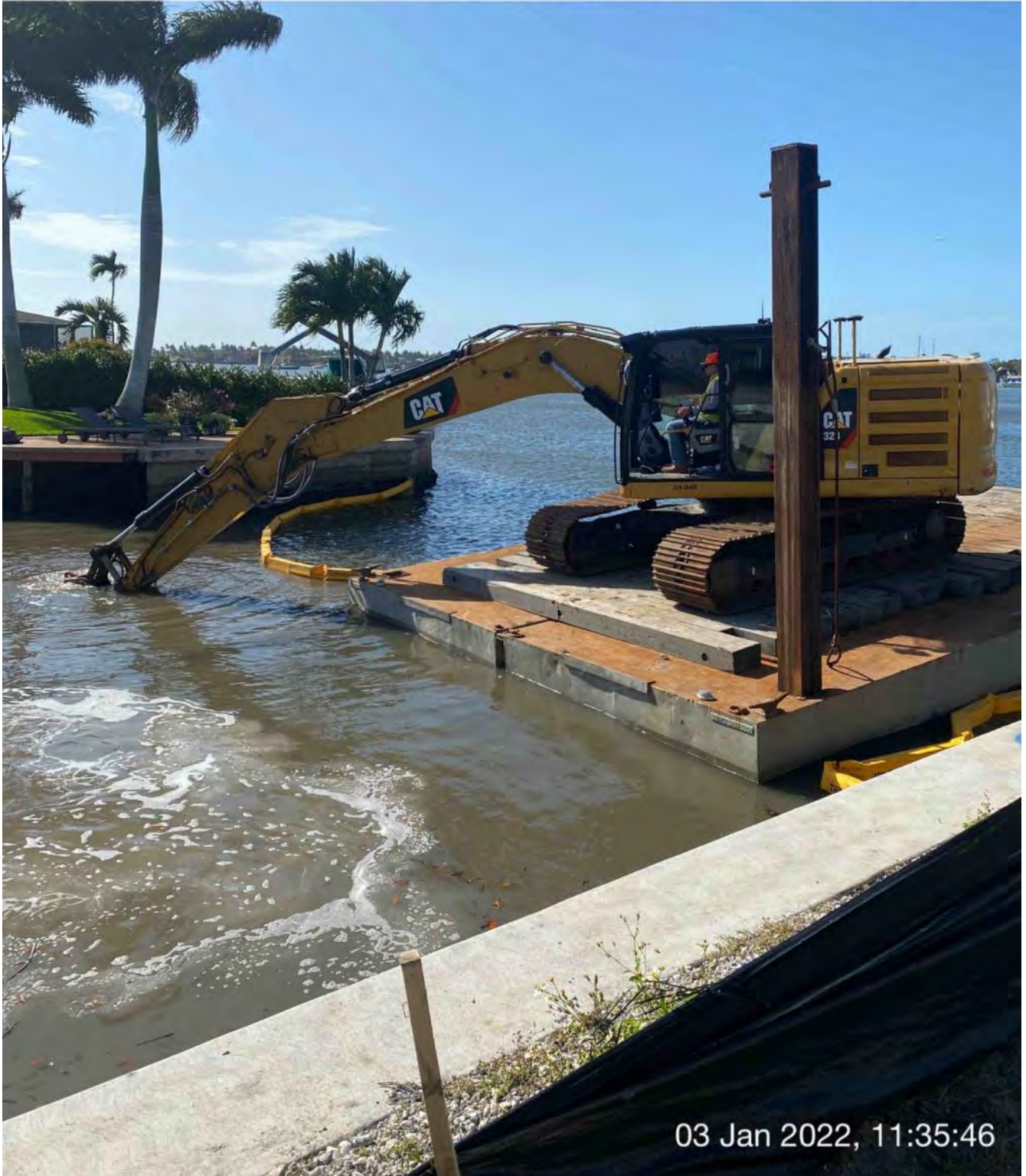
323 excavator checking bottom elevations at station 1+00
