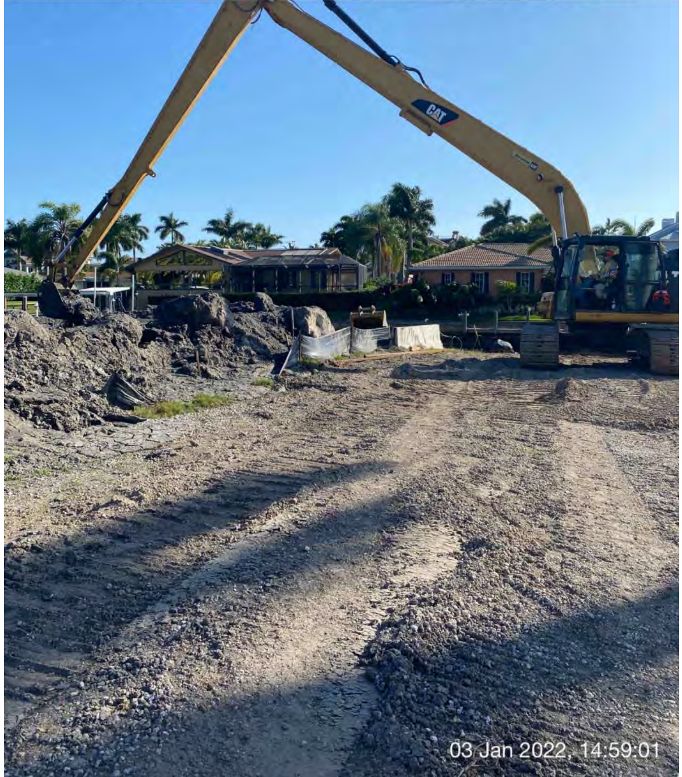
326 excavator transferring 1 hopper of material to dewatering site at 1300 Curlew Avenue
