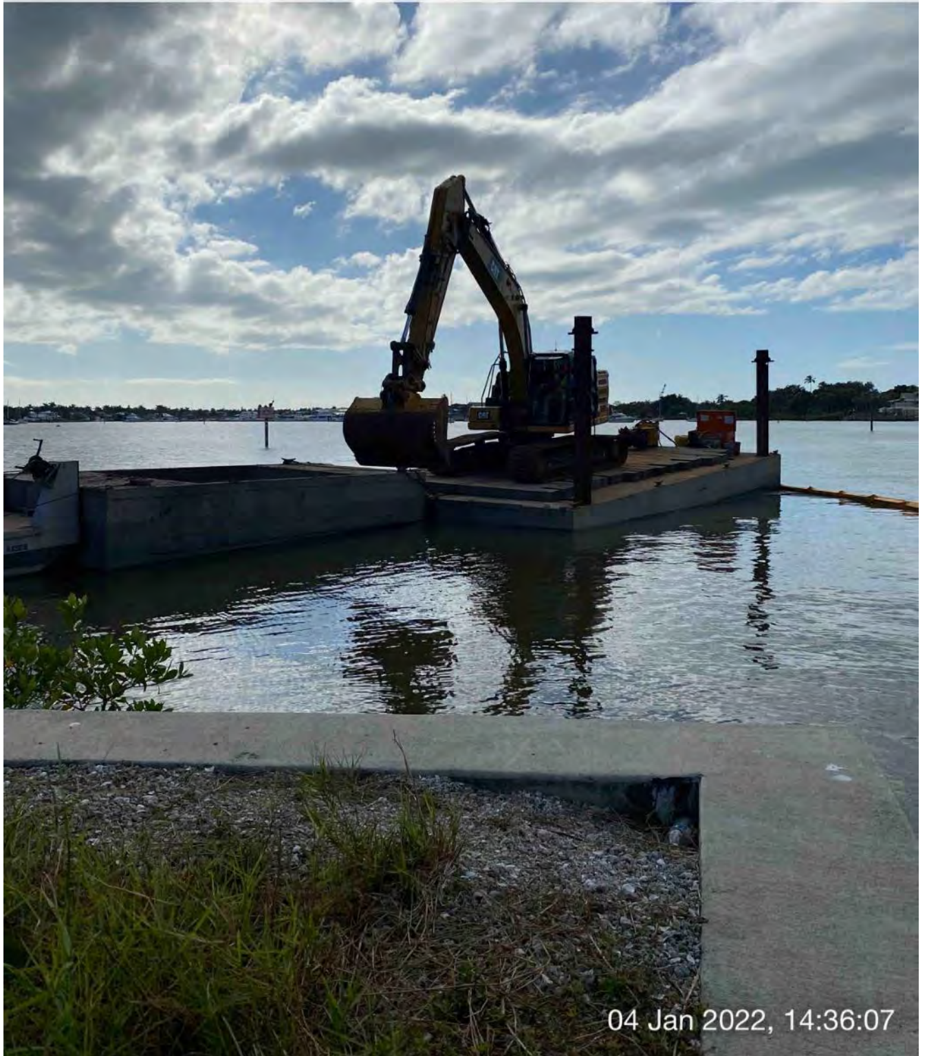
323 excavator removing material and transferring to hopper at station 0+50
