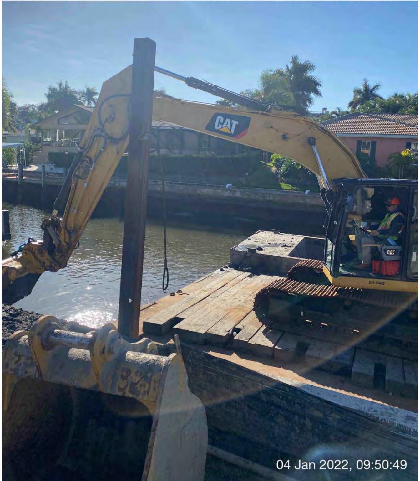
323 excavator removing material and transferring to hopper at station 2+00
