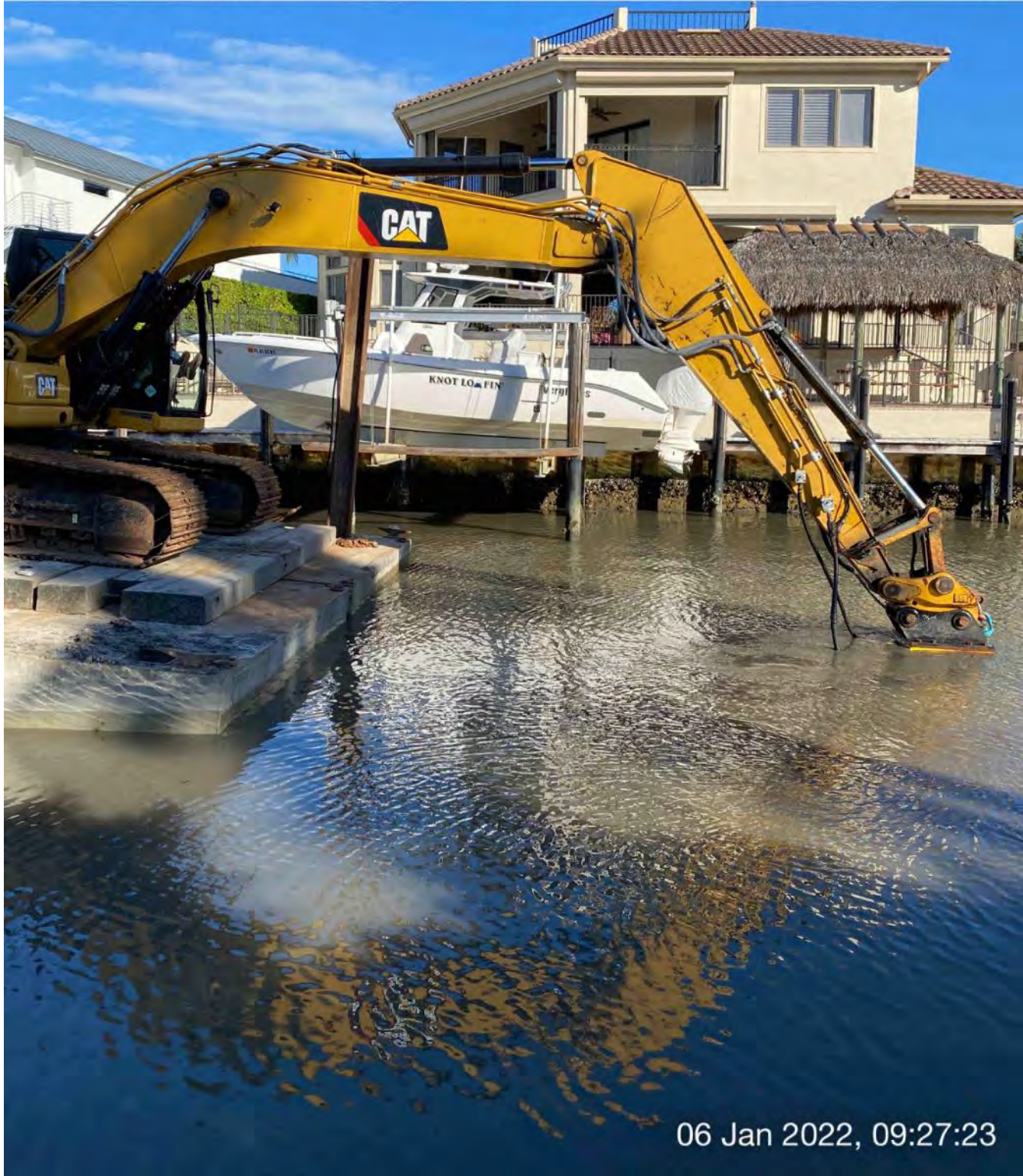
323 excavator checking bottom elevations and grinding material at station 2+50 in Canal BB-BB
