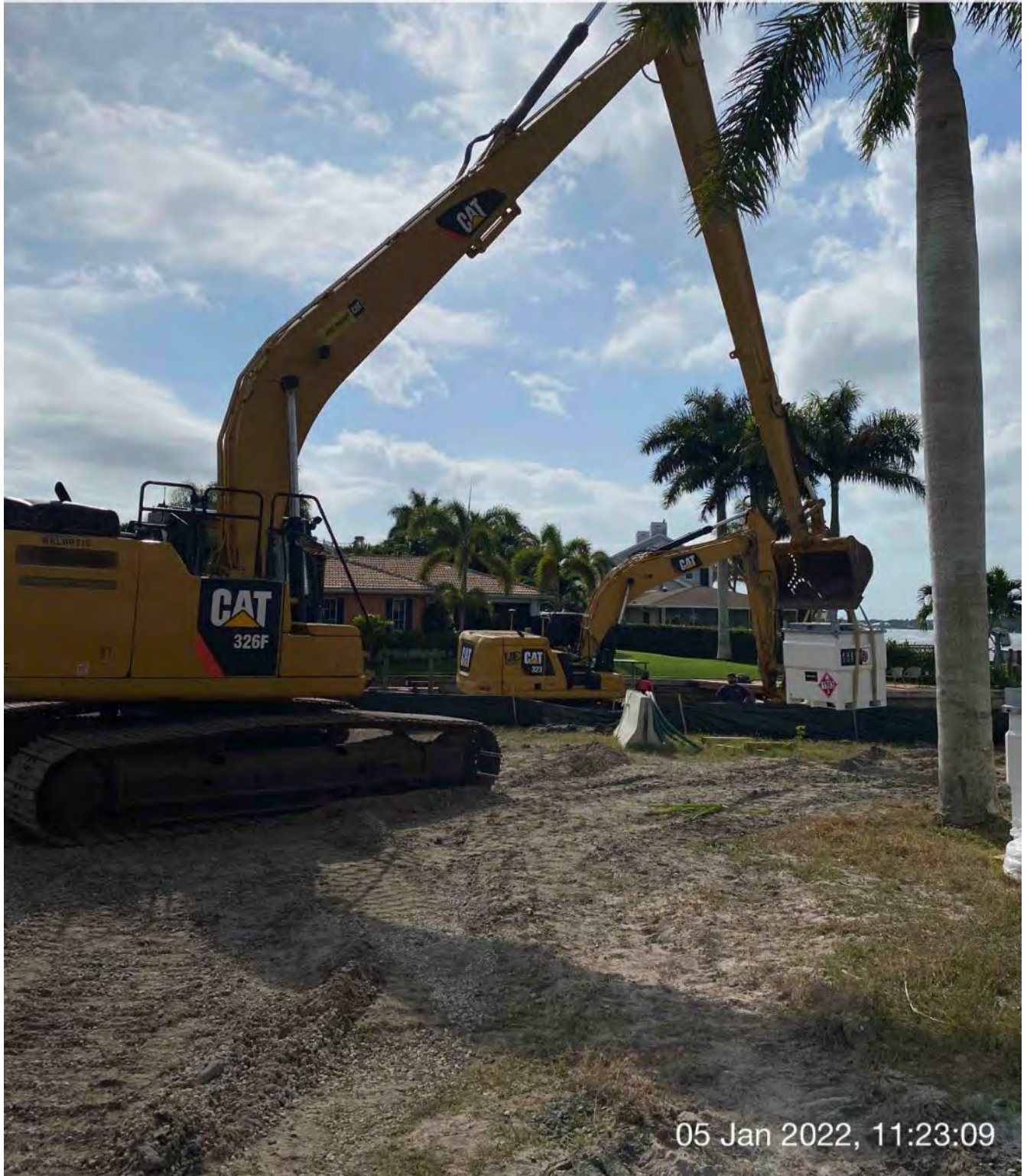
326 excavator lifting small cube and transporting it to barge
