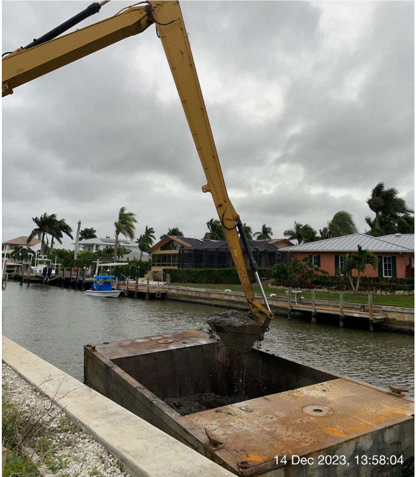
Long reach excavator removing sediment from hopper.
