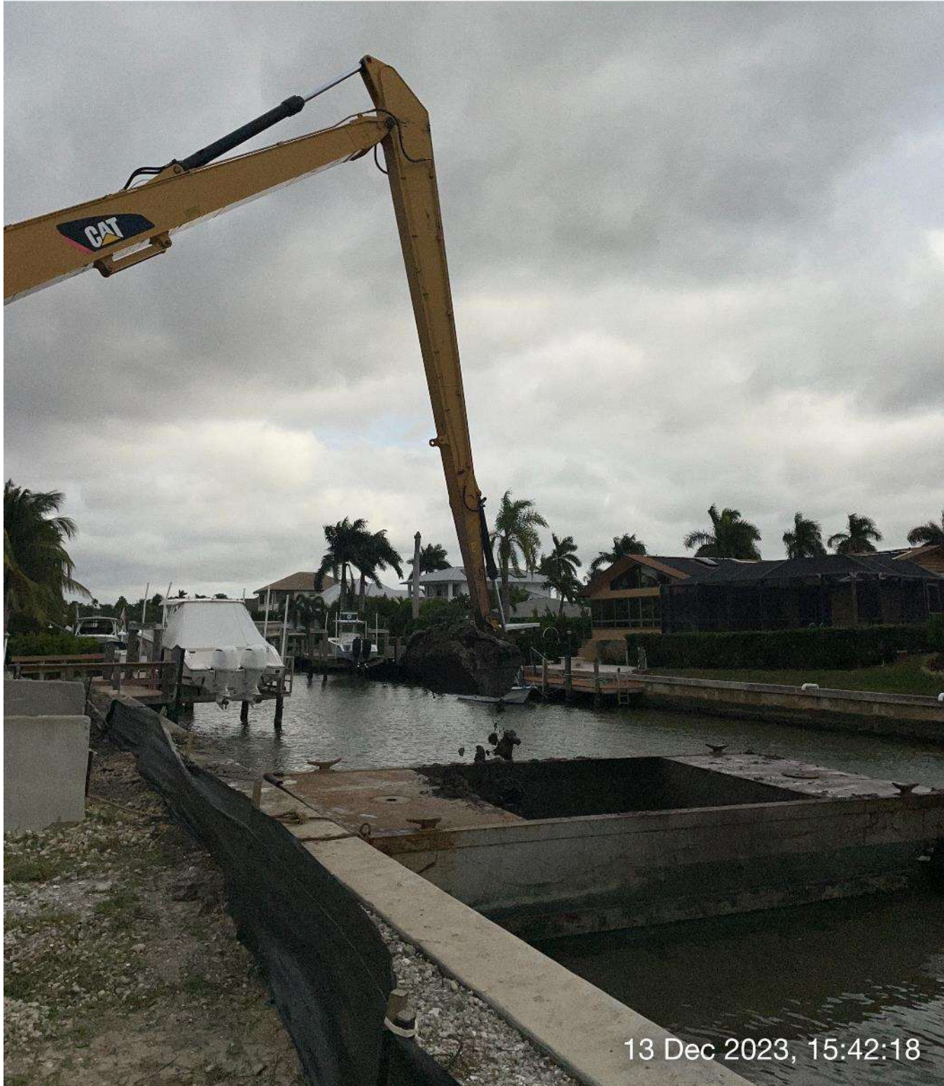
Long reach excavator removing sediment from hopper.
