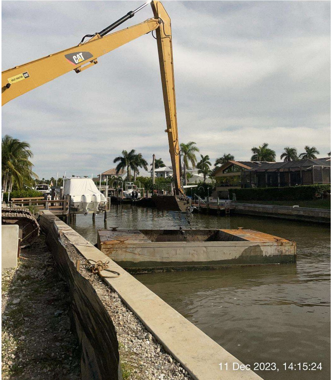
Long reach excavator removing sediment from hopper.
