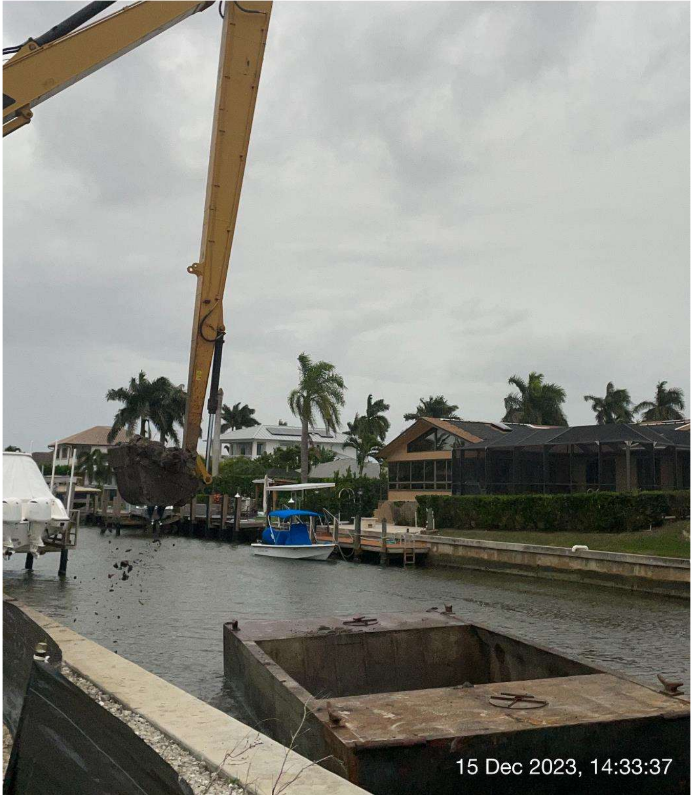
Long reach excavator removing sediment from hopper.
