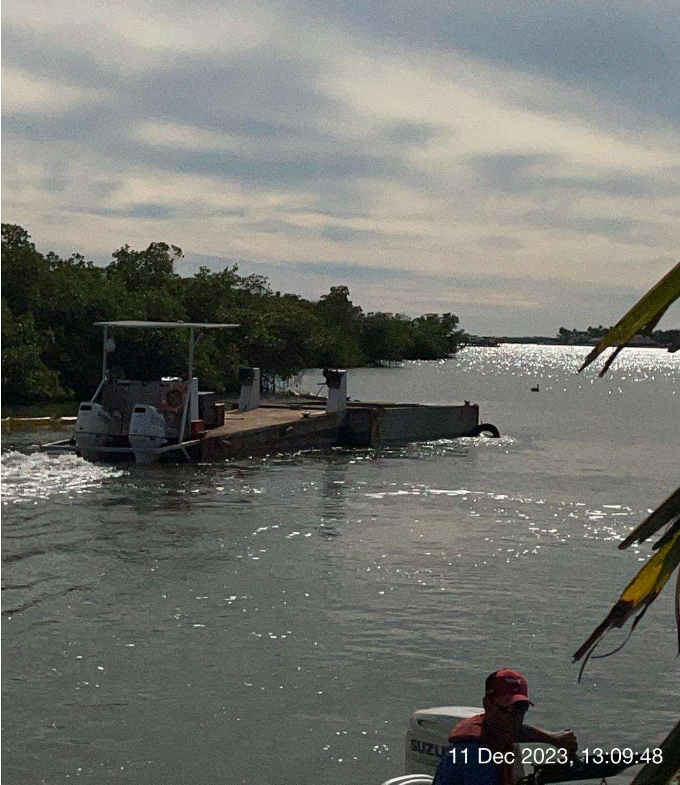
Push boat taking hopper to staging area.
