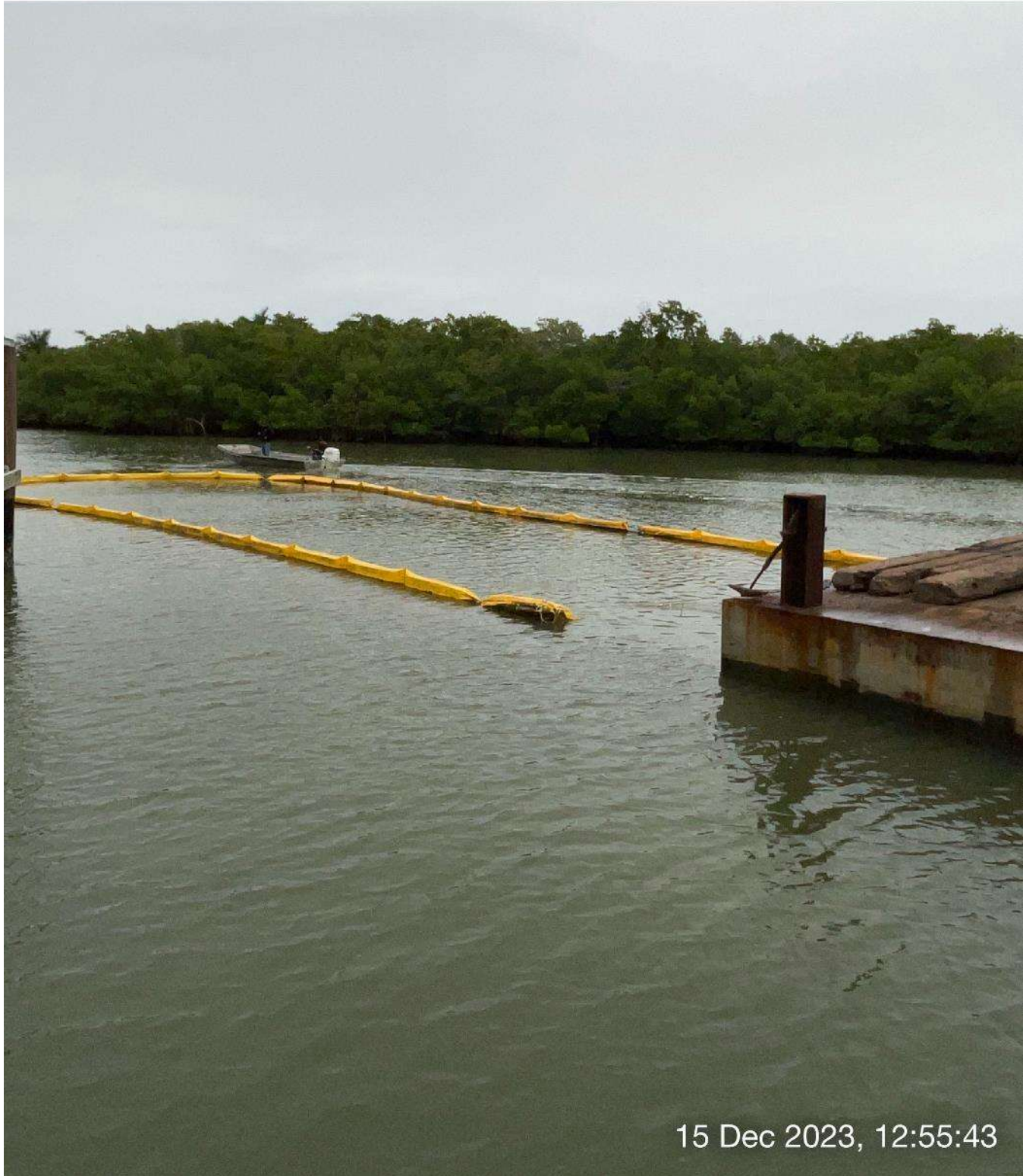
Turbidity curtain in place around barge.
