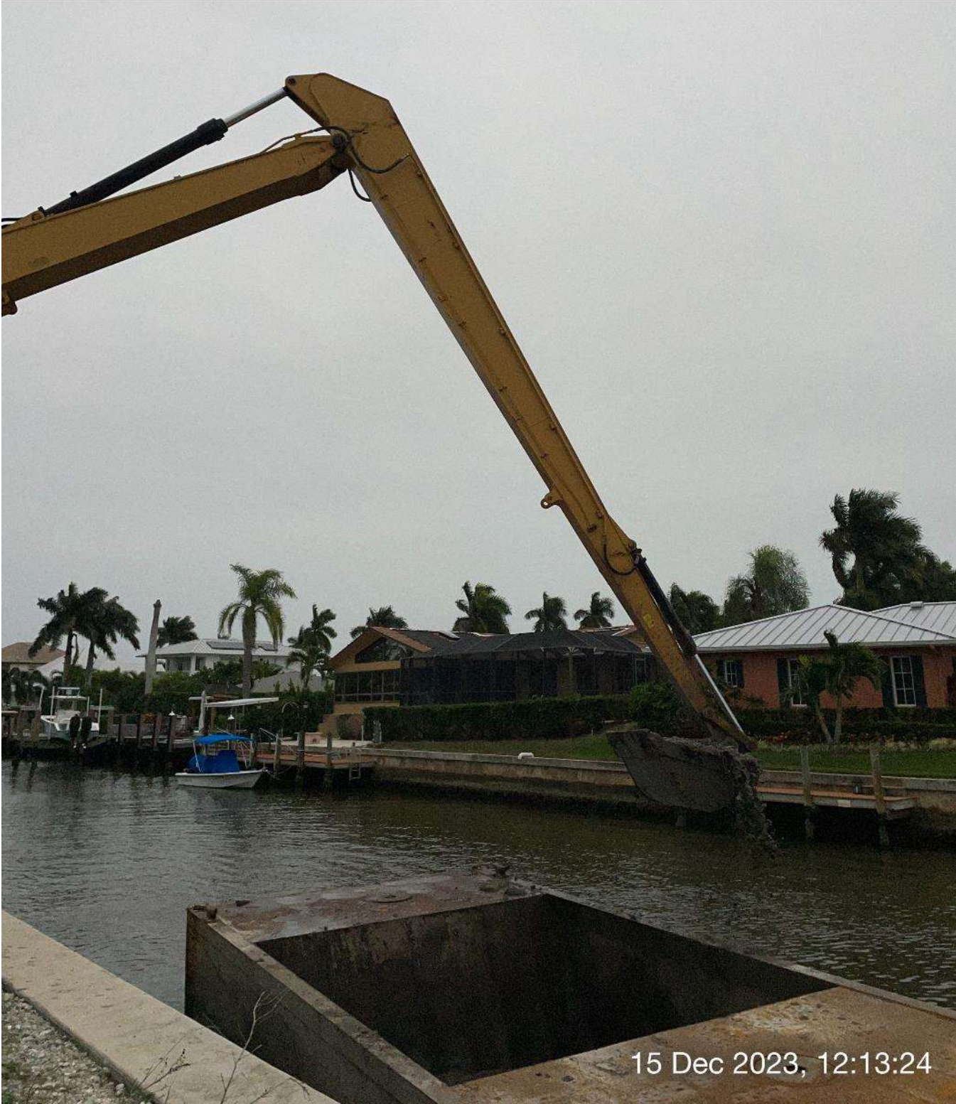
Long reach excavator removing sediment from hopper.
