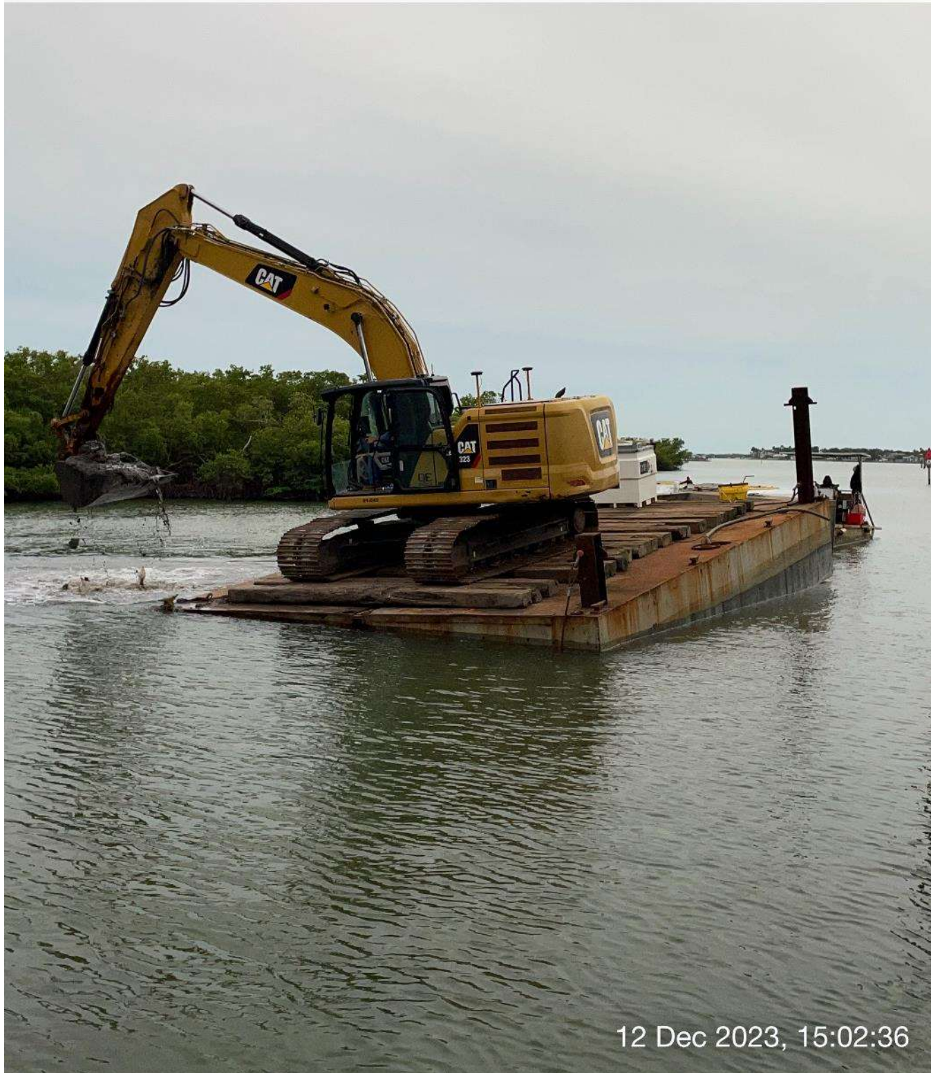
323 excavator removing sediment at station 5+50.
