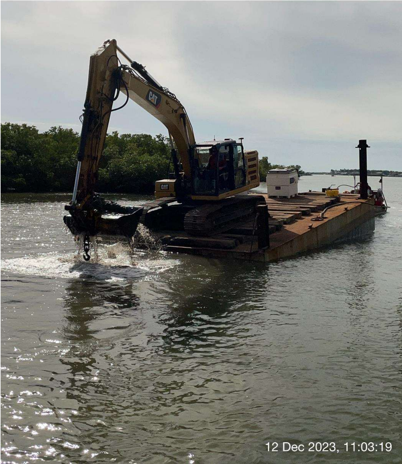
323 excavator removing sediment at station 5+75.
