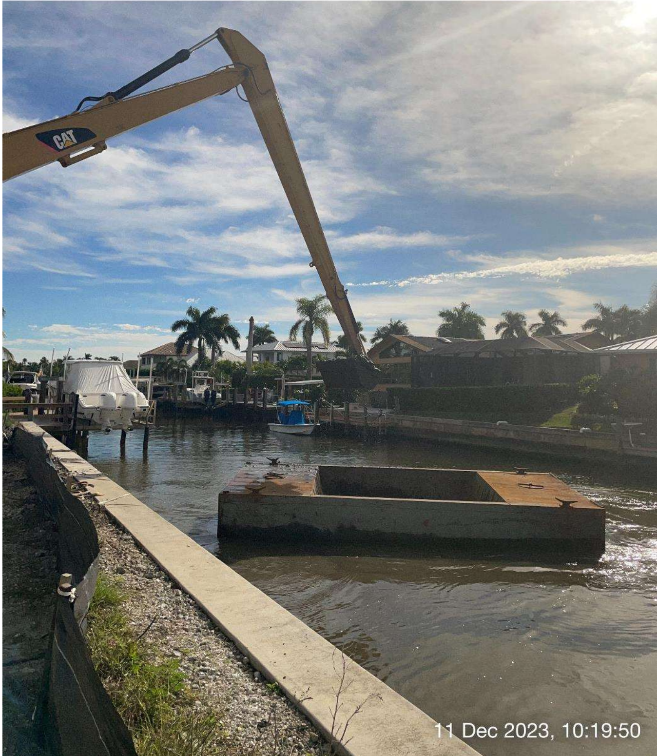
Long reach excavator removing sediment from hopper.
