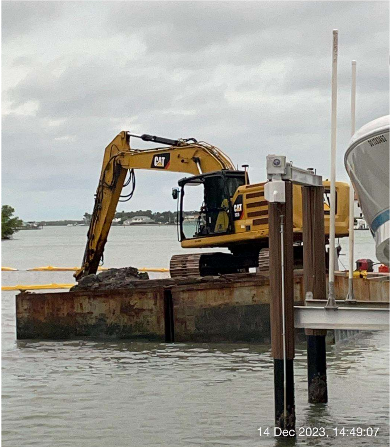
323 excavator removing sediment at station 5+25.
