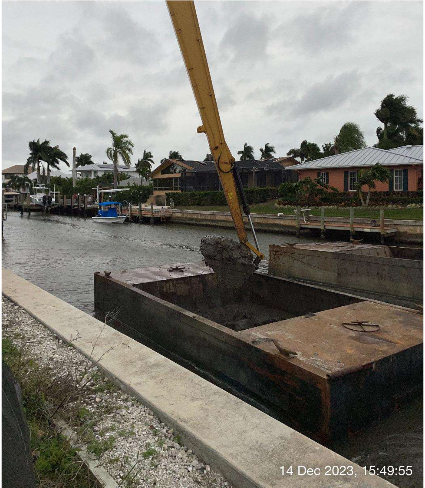
Long reach excavator removing sediment from hopper.
