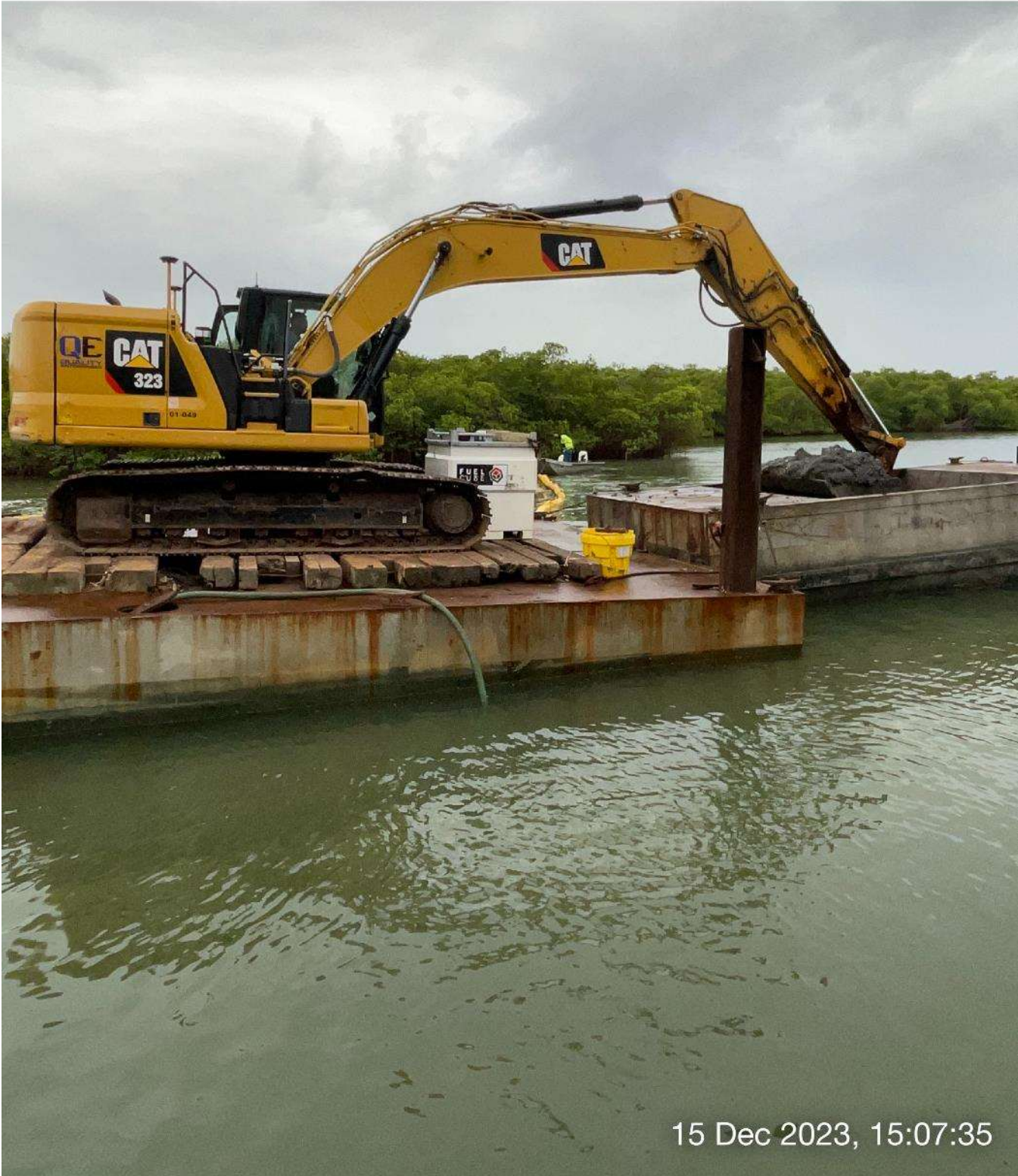
323 excavator removing sediment at station 5+00 in Canal Main B.
