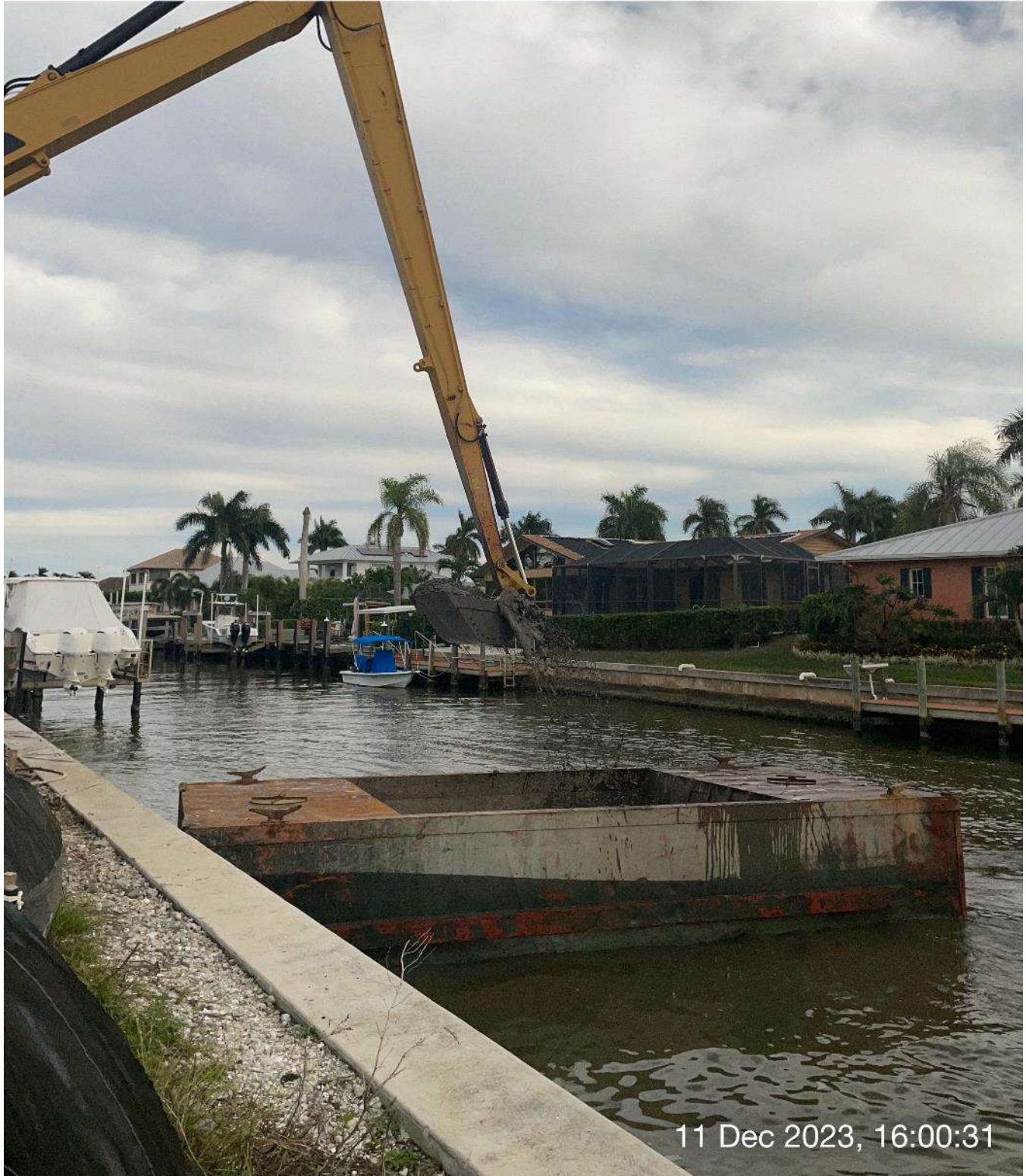
Long reach excavator removing sediment from hopper.
