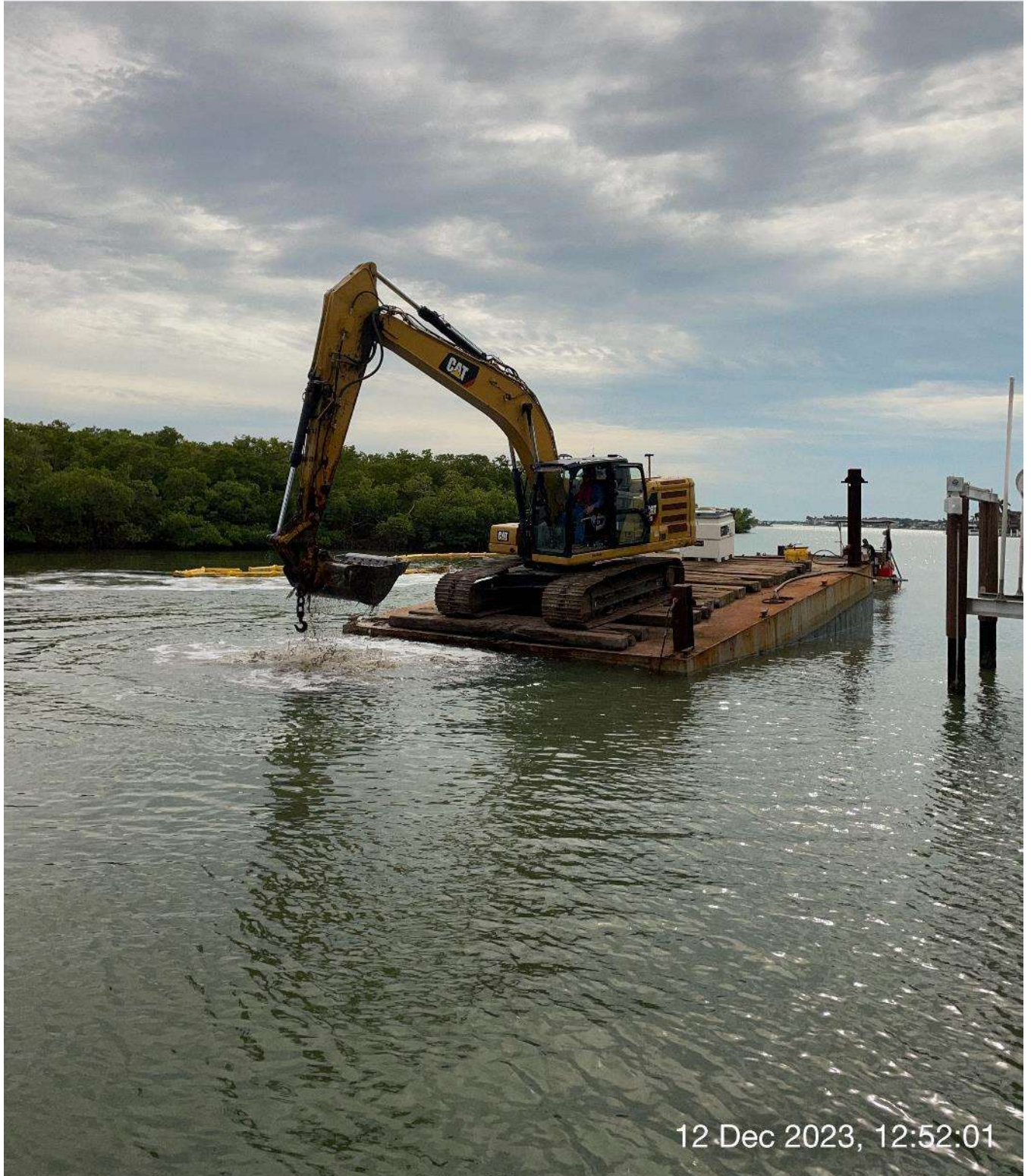
323 excavator removing sediment at station 5+75.
