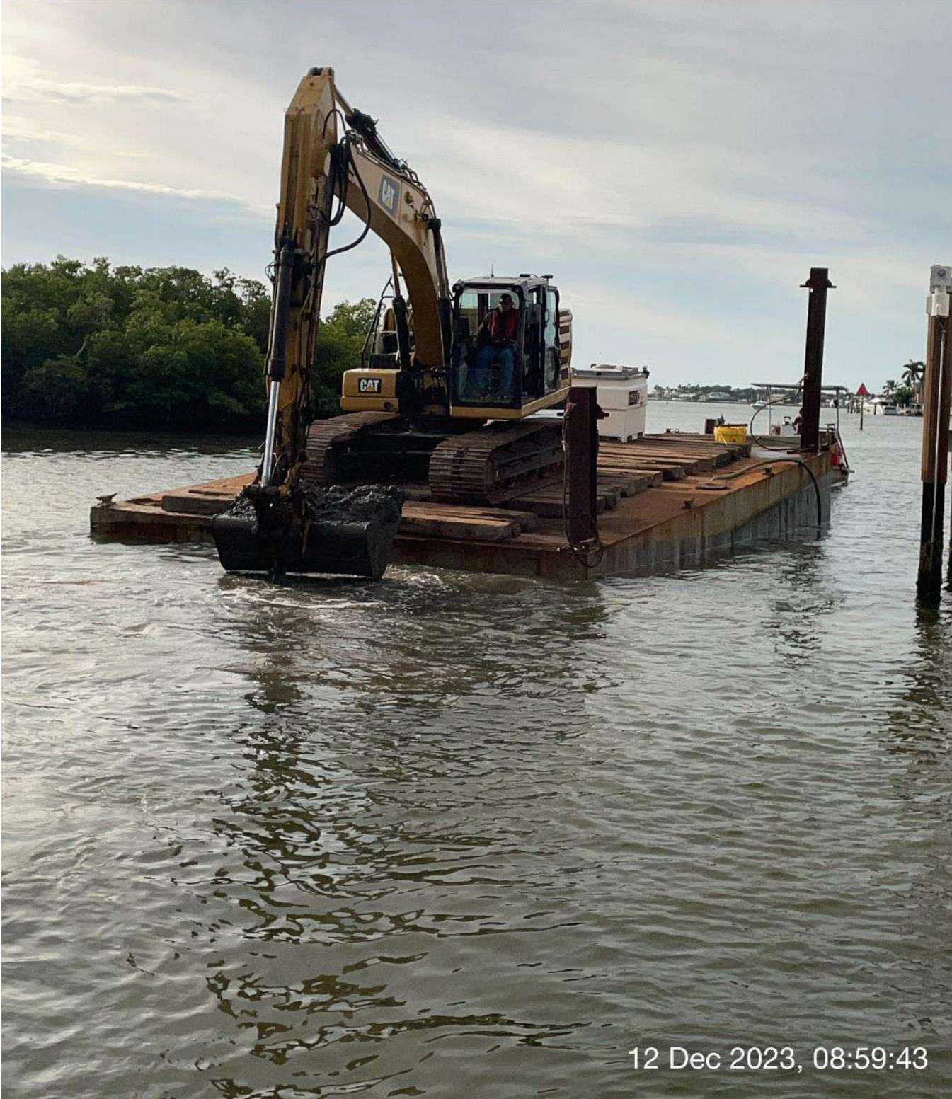
323 excavator removing sediment at station 5+75.
