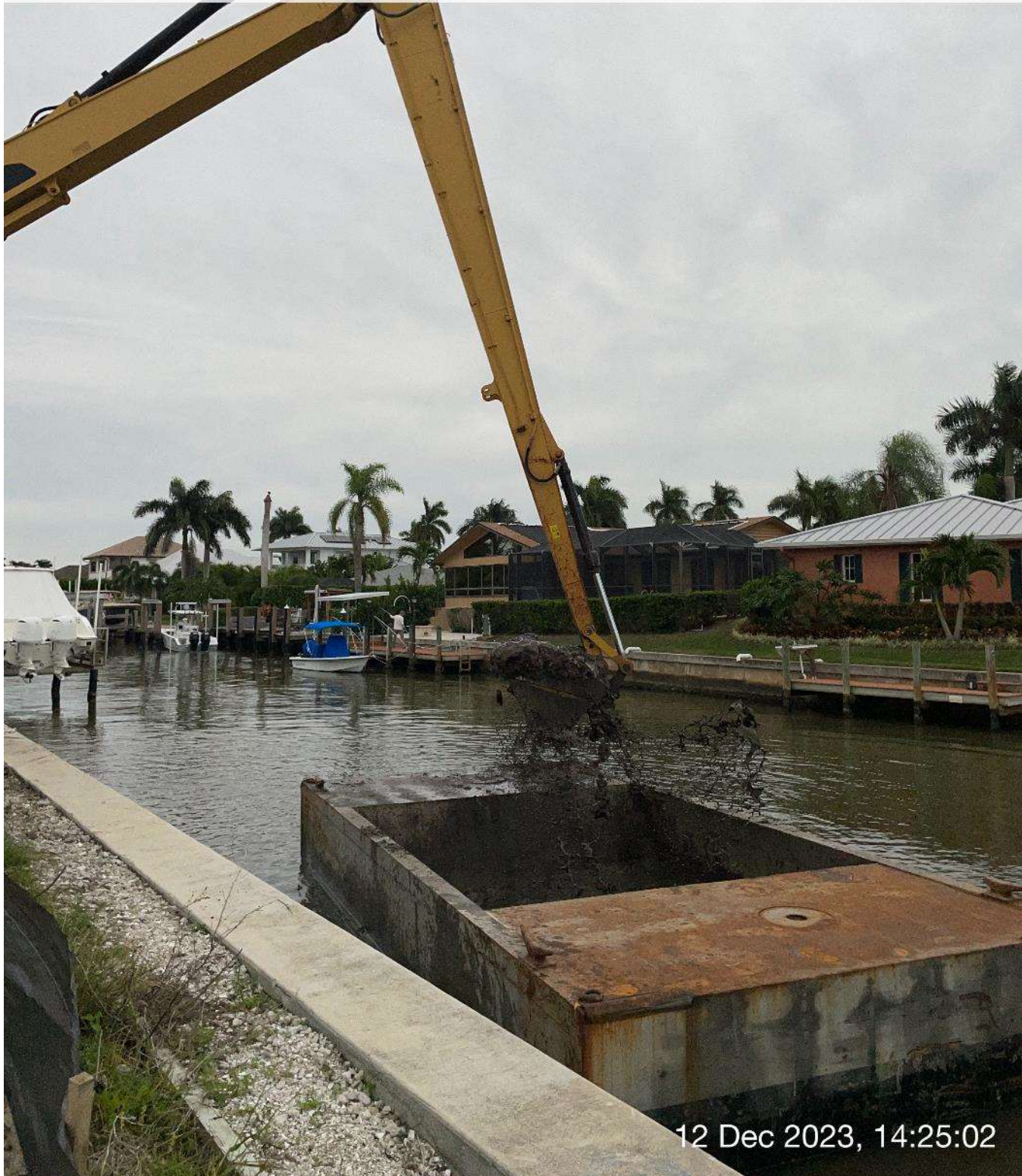
Long reach excavator removing sediment from hopper.
