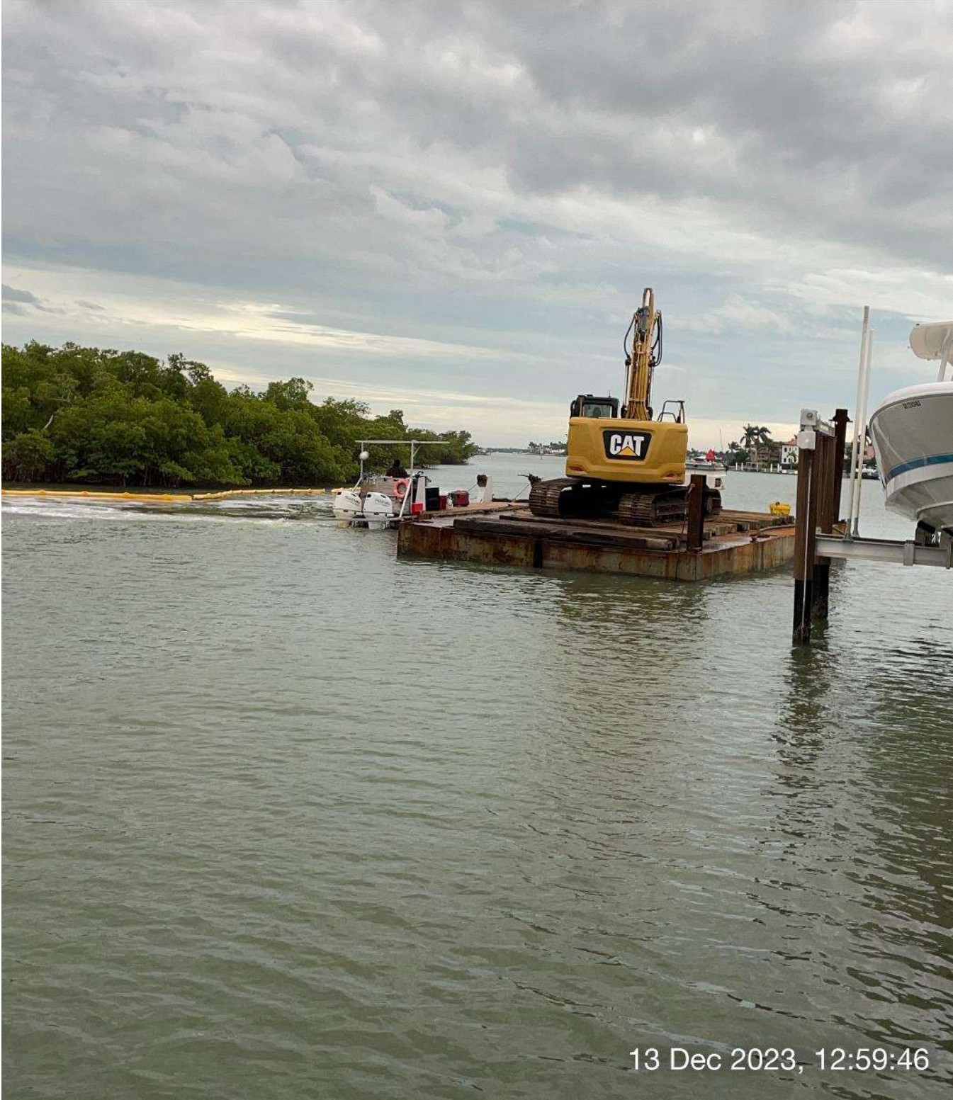
Push boat taking hopper to staging area.
