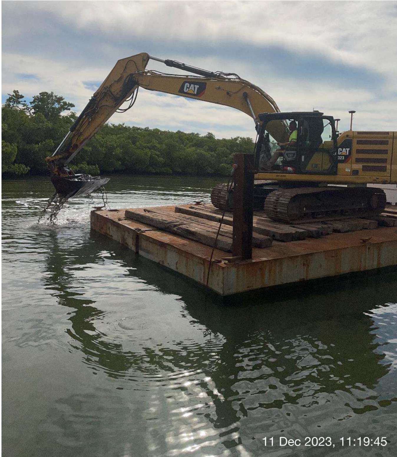
323 excavator removing sediment at station 6+25 in Canal Main B.
