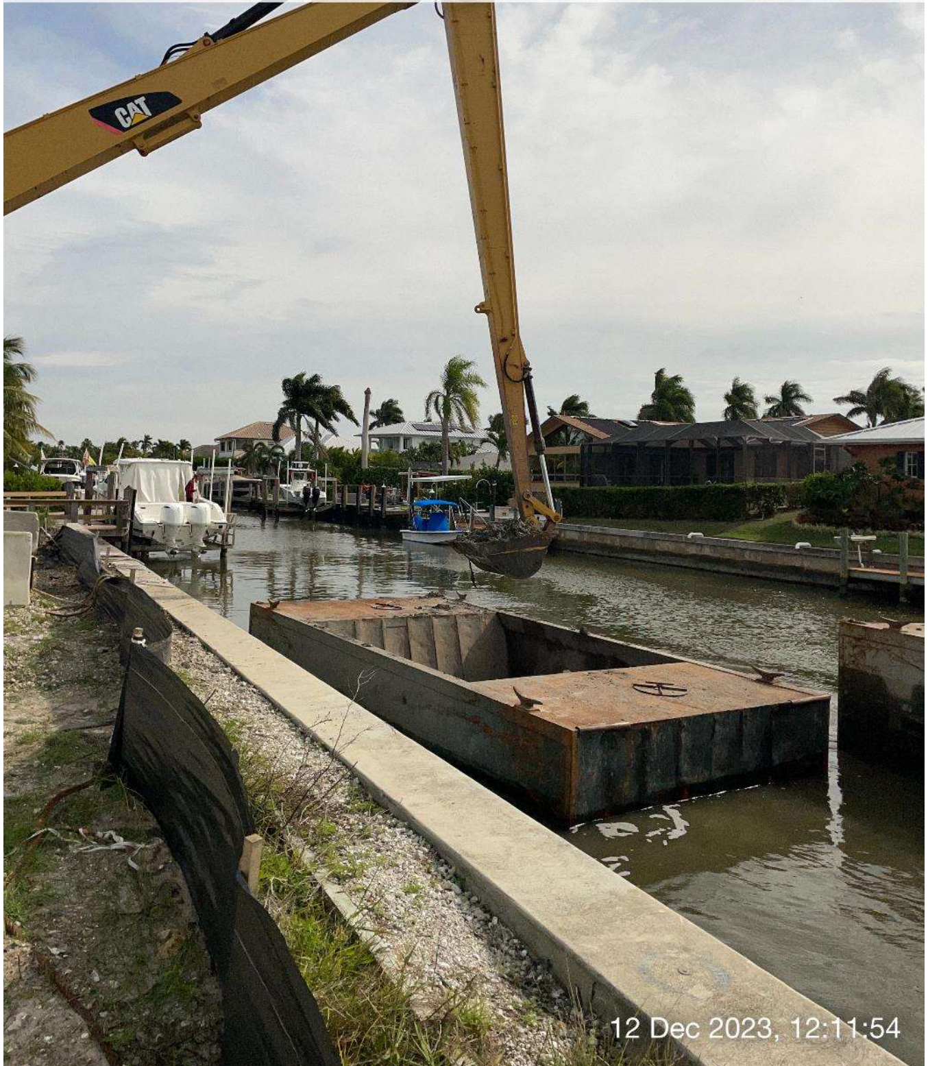
Long reach excavator removing sediment from hopper.
