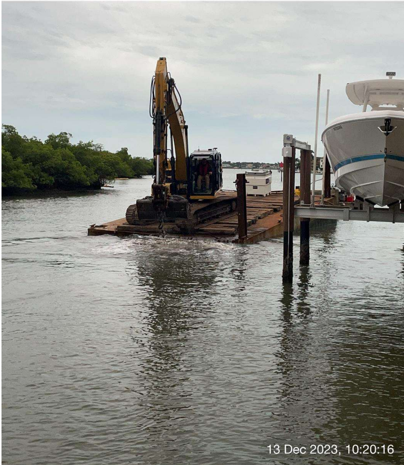
323 excavator removing sediment at station 5+50 in Canal Main B.
