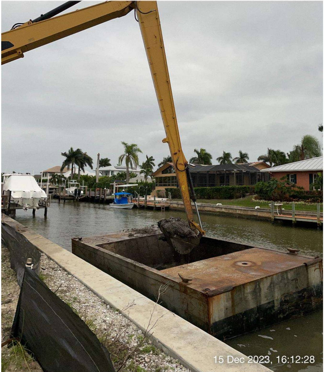
Long reach excavator removing sediment from hopper.
