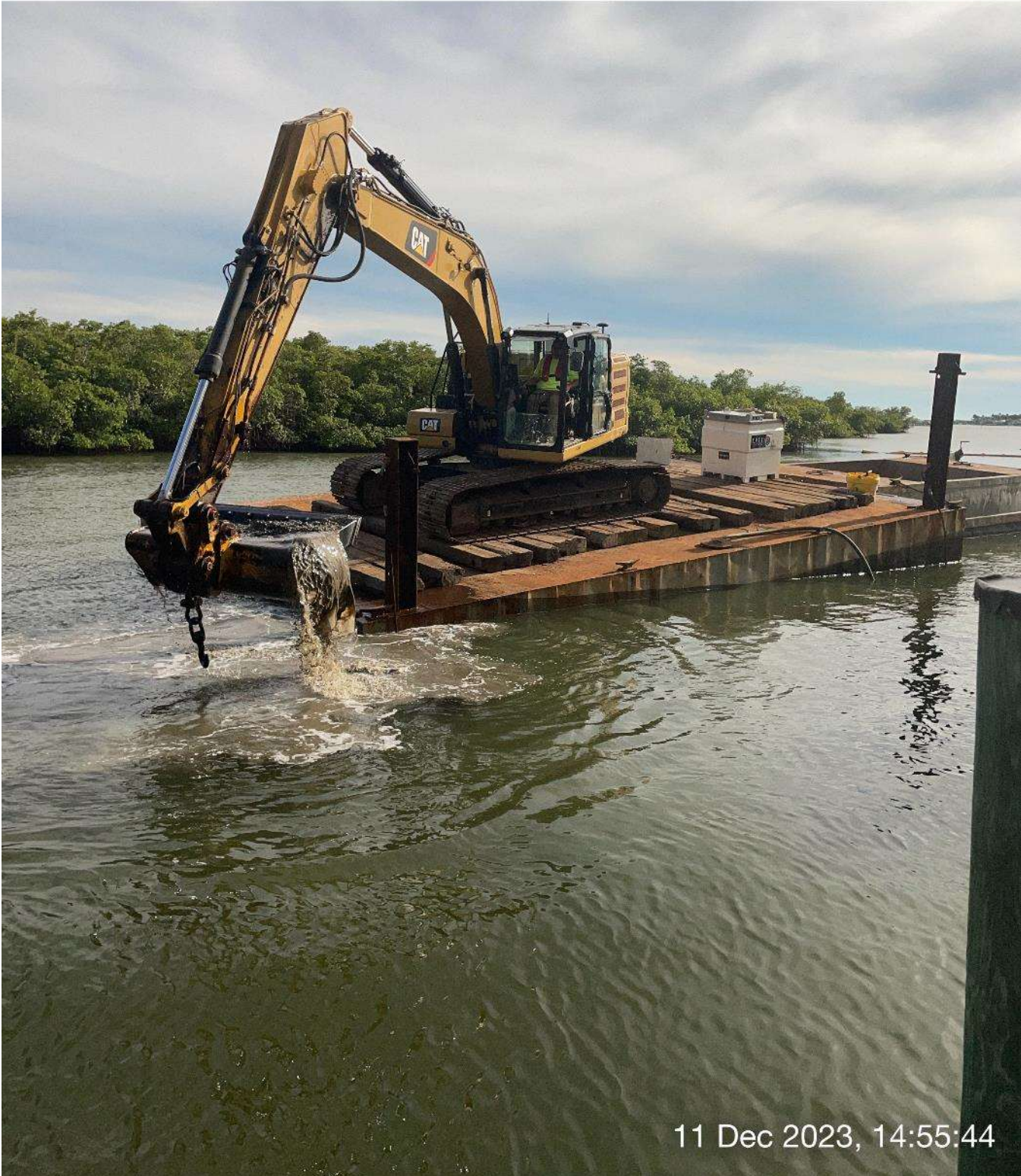
323 excavator removing sediment at station 6+00 in Canal Main B.
