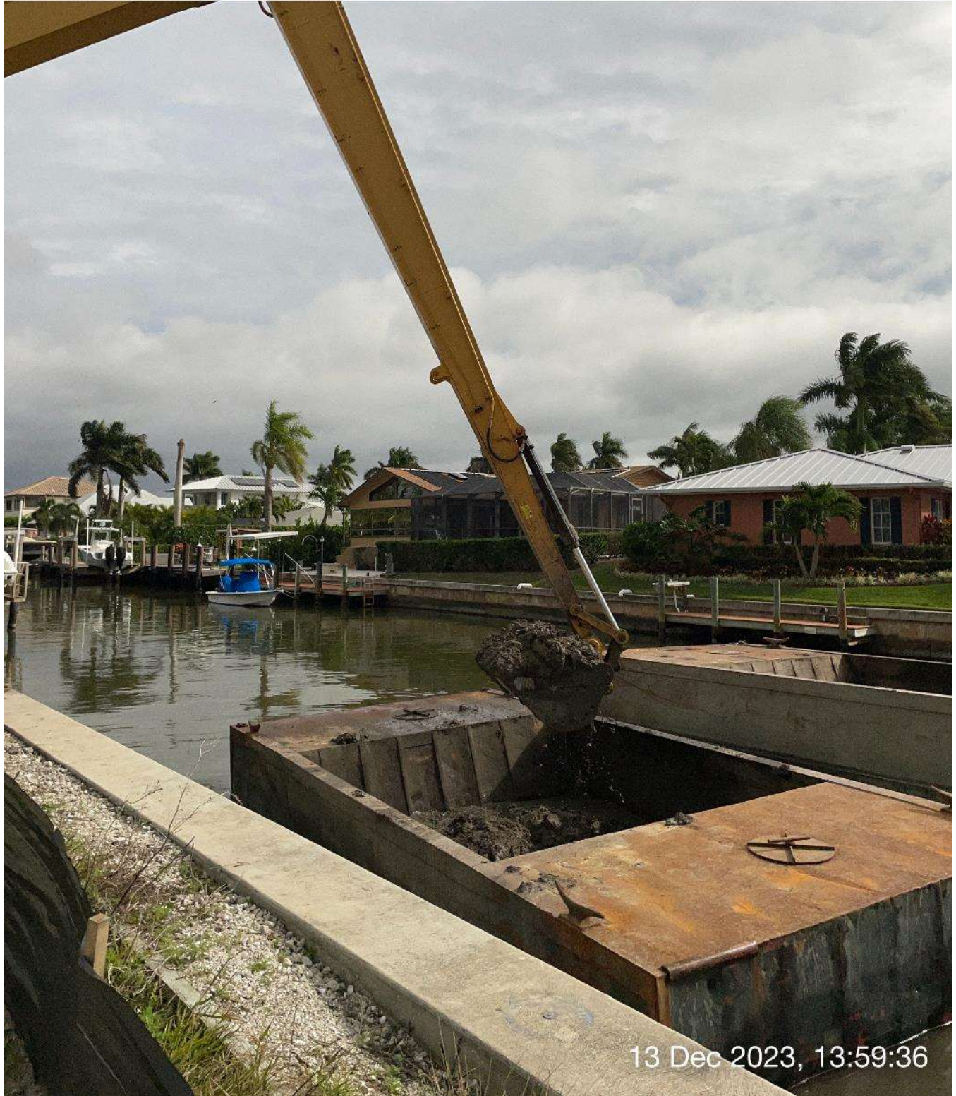
Long reach excavator removing sediment from hopper.
