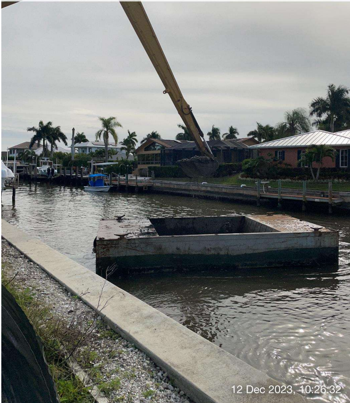
Long reach excavator removing sediment from hopper.
