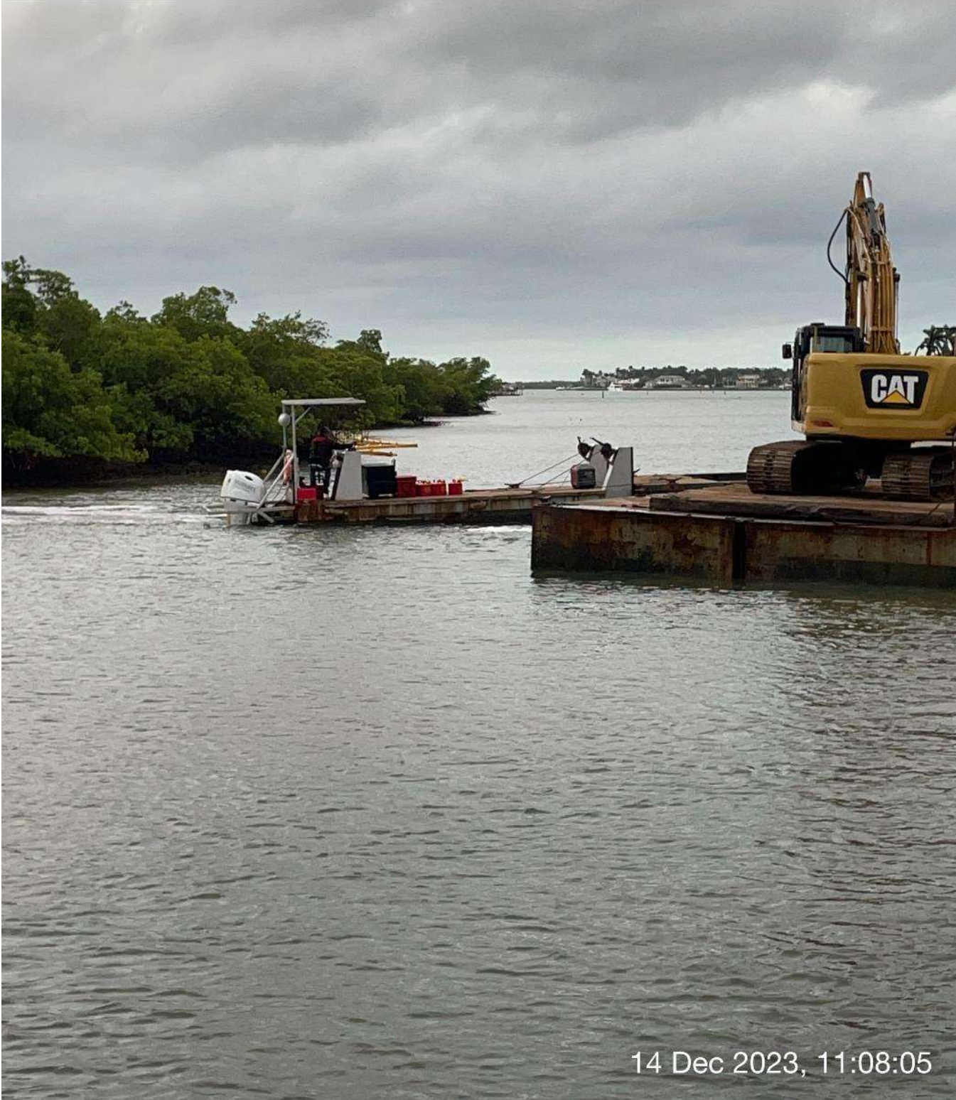
Push boat taking hopper to staging area.
