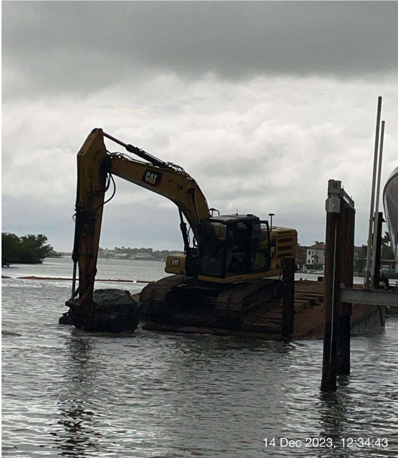
323 excavator removing sediment at station 5+25.
