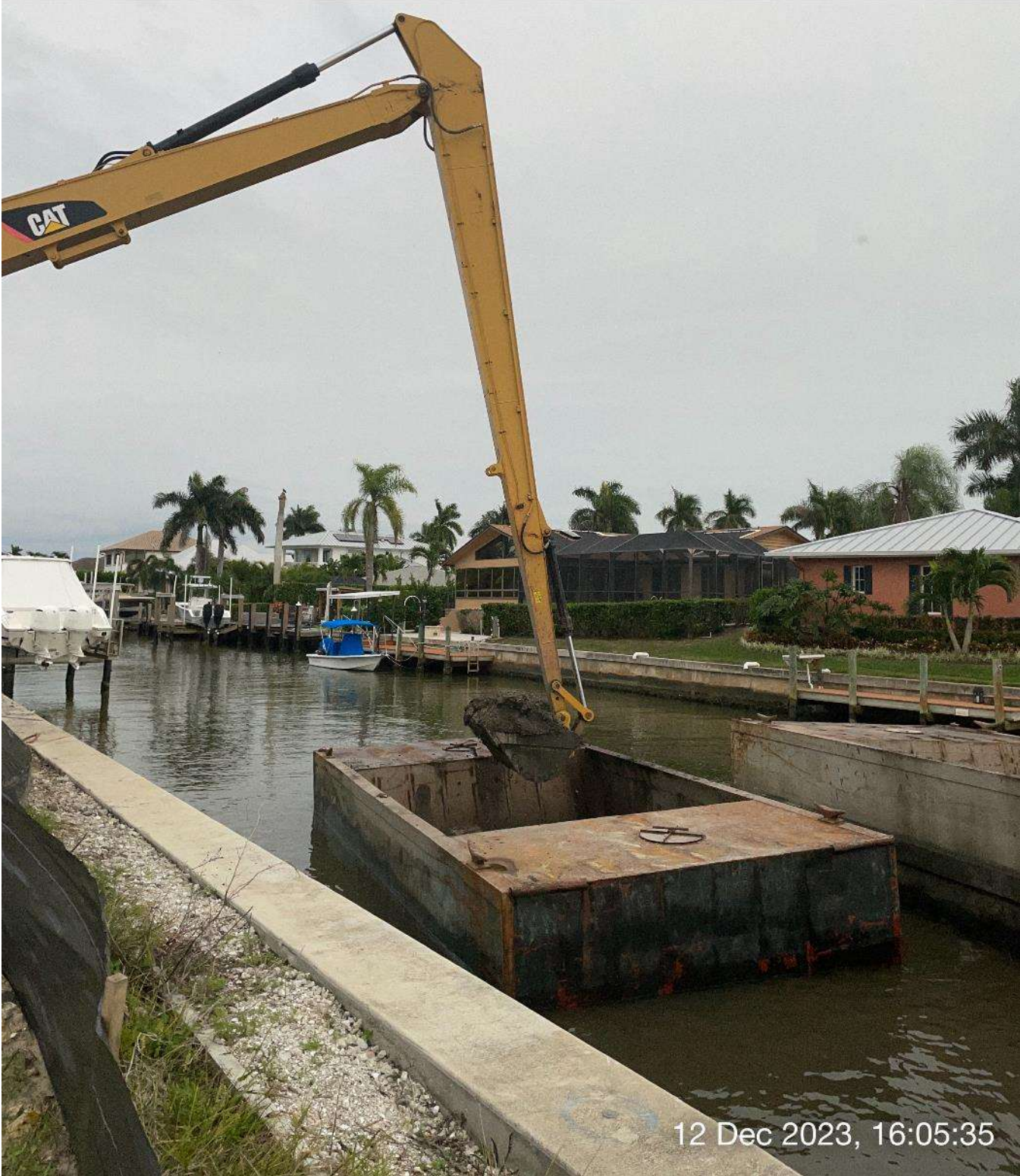
Long reach excavator removing sediment from hopper.
