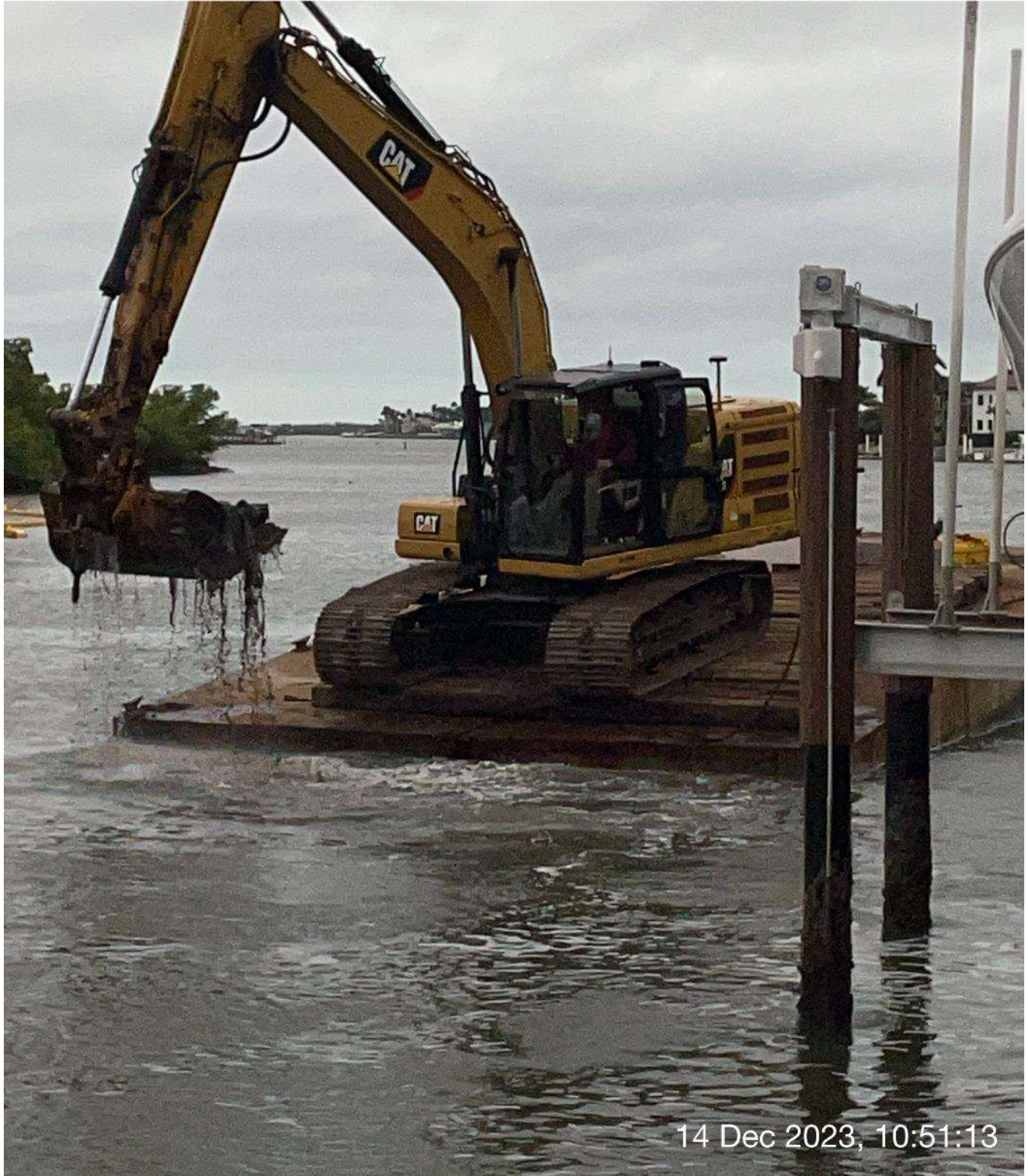
323 excavator removing sediment at station 5+25.
