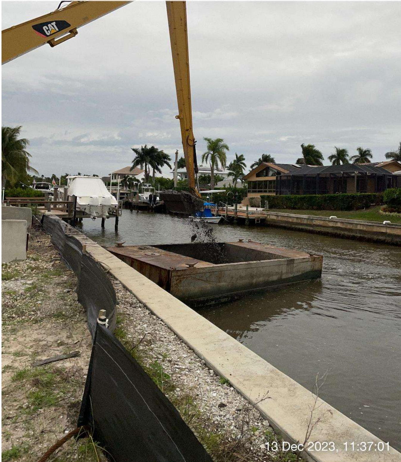
Long reach excavator removing sediment from hopper.
