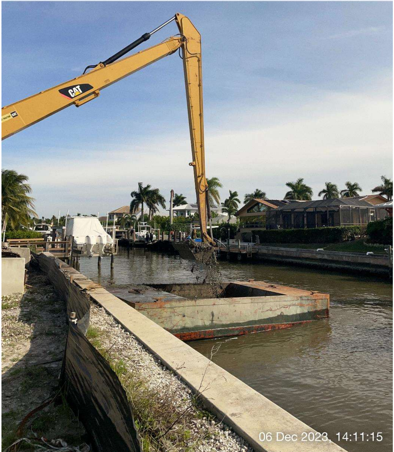
Long reach excavator removing sediment from hopper.
