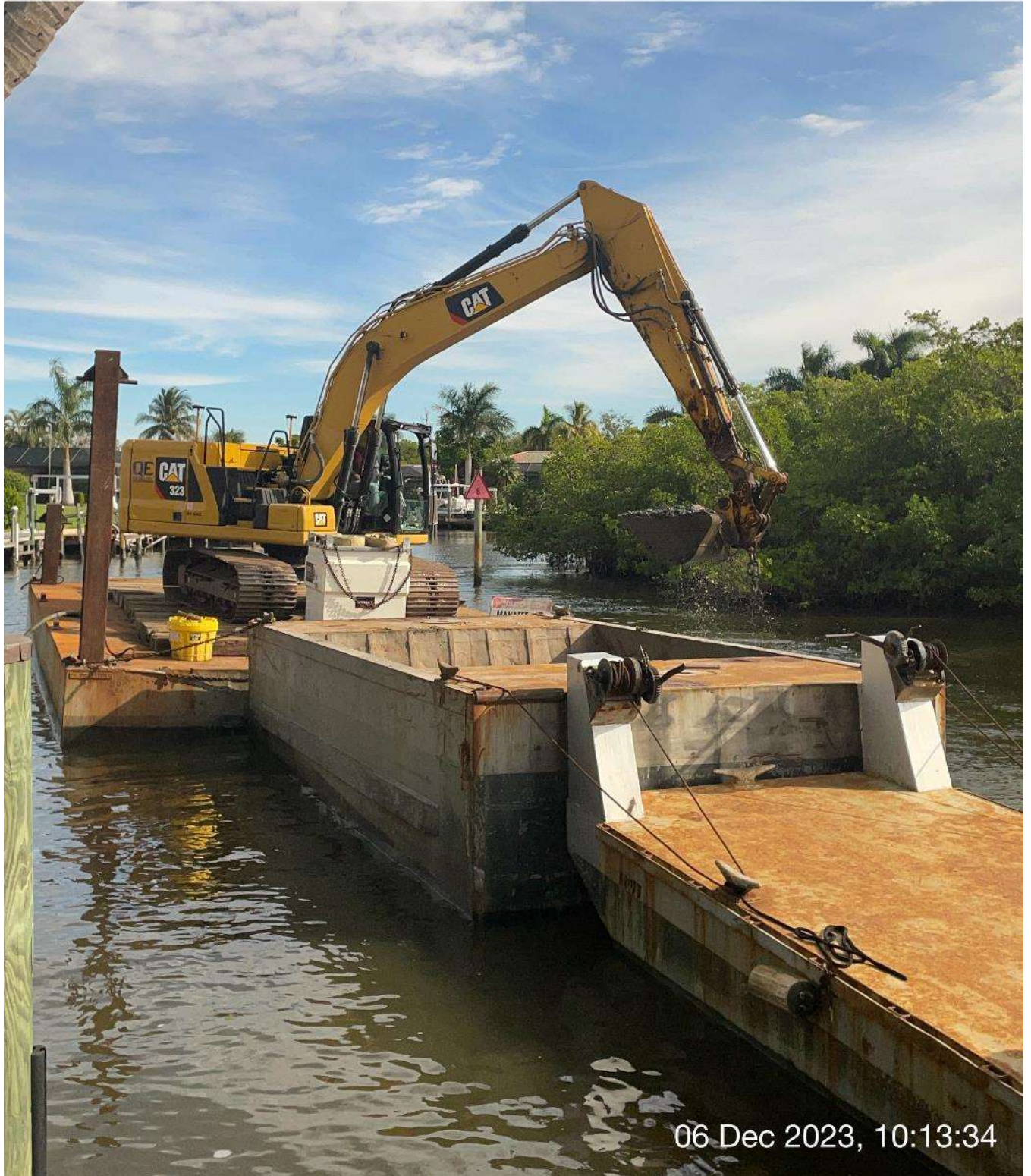
323 excavator removing sediment at station 7+25 in Canal Main B.
