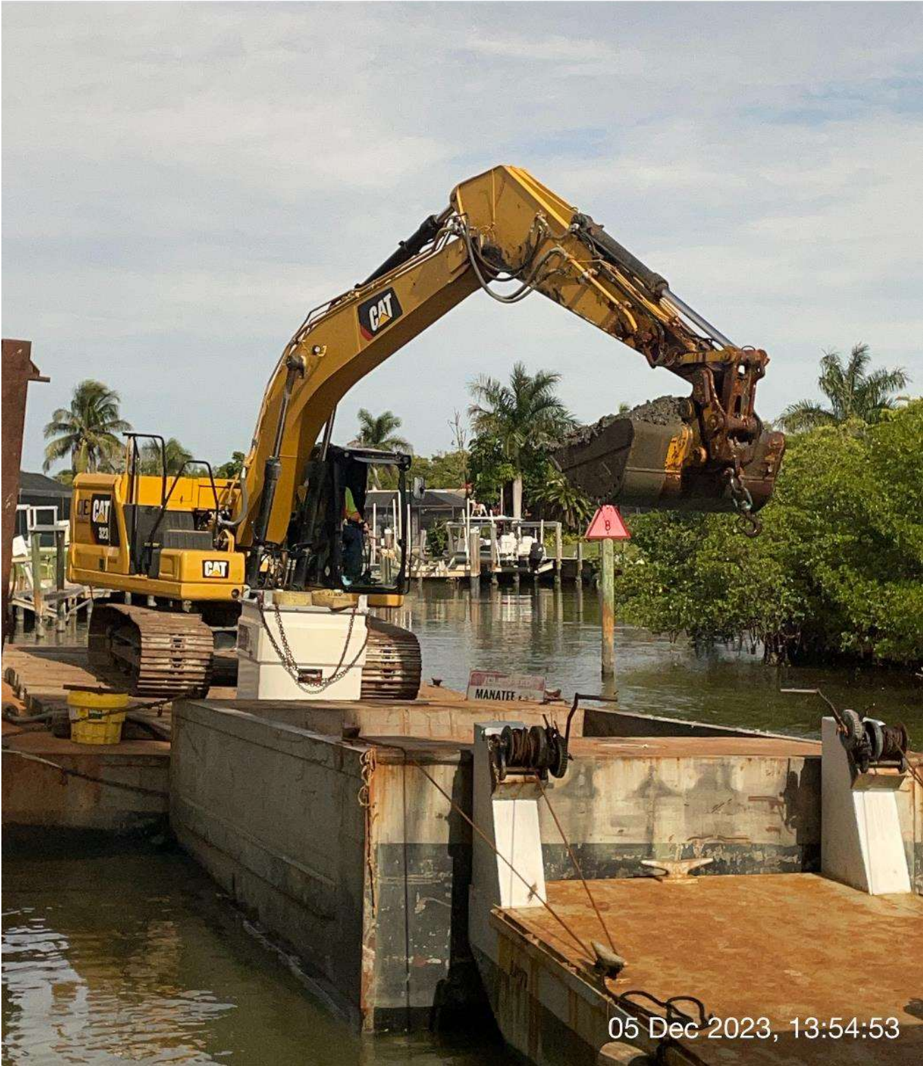
323 excavator removing sediment at station 7+50 in Canal Main B.
