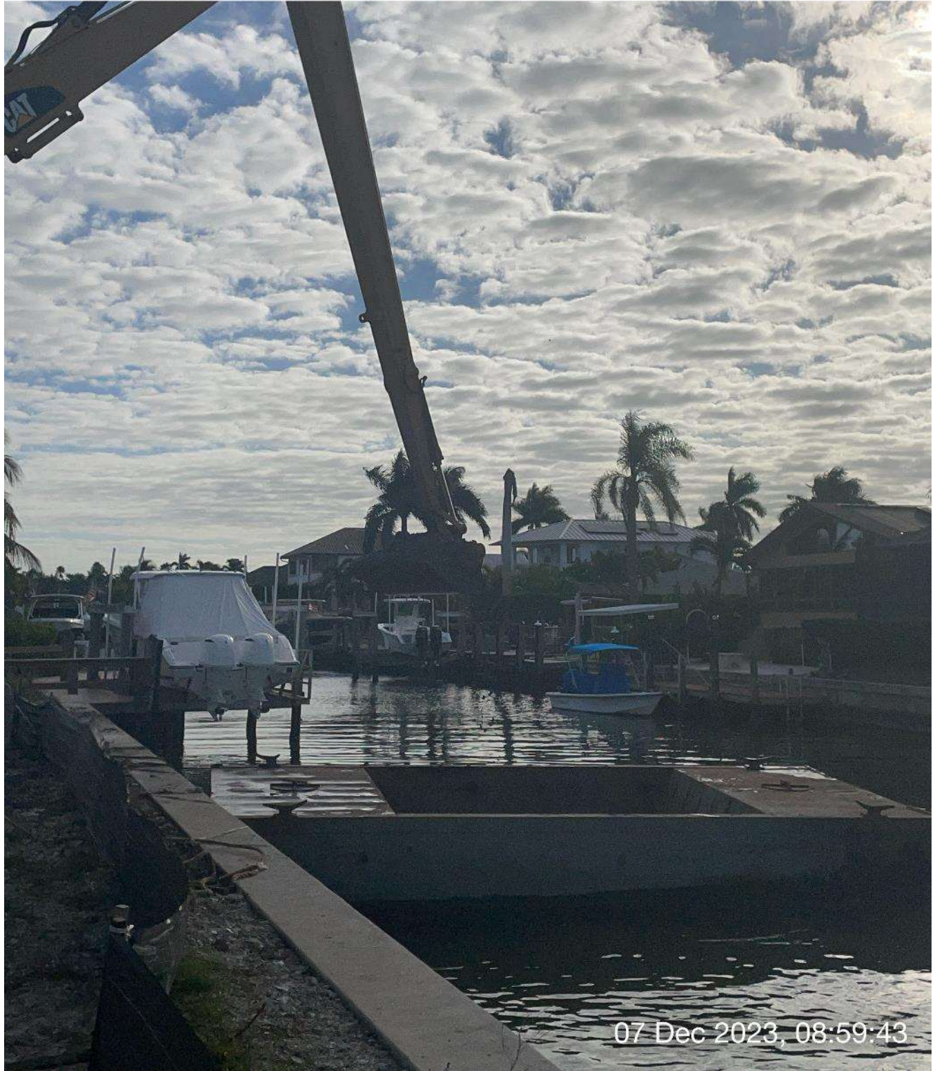
Long reach excavator removing sediment from hopper.
