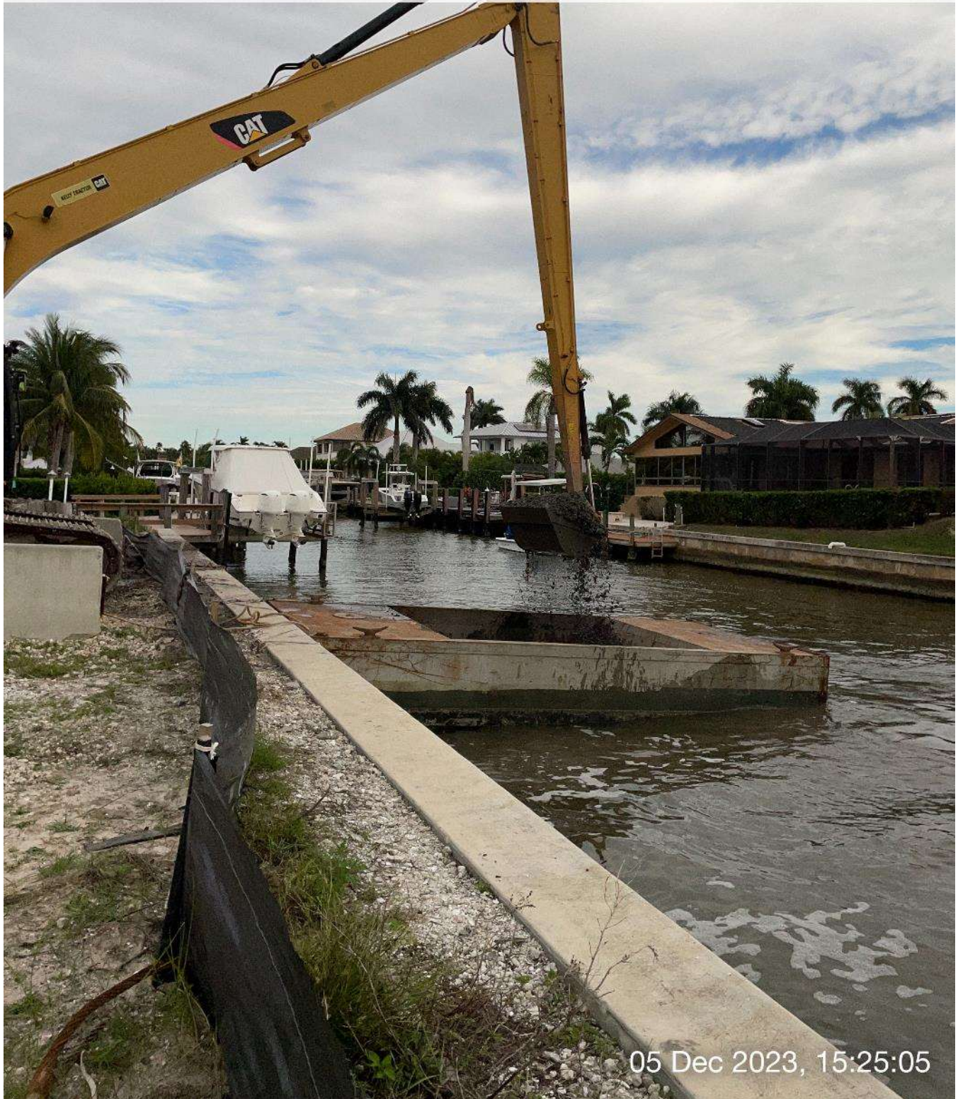
Long reach excavator removing sediment from hopper.
