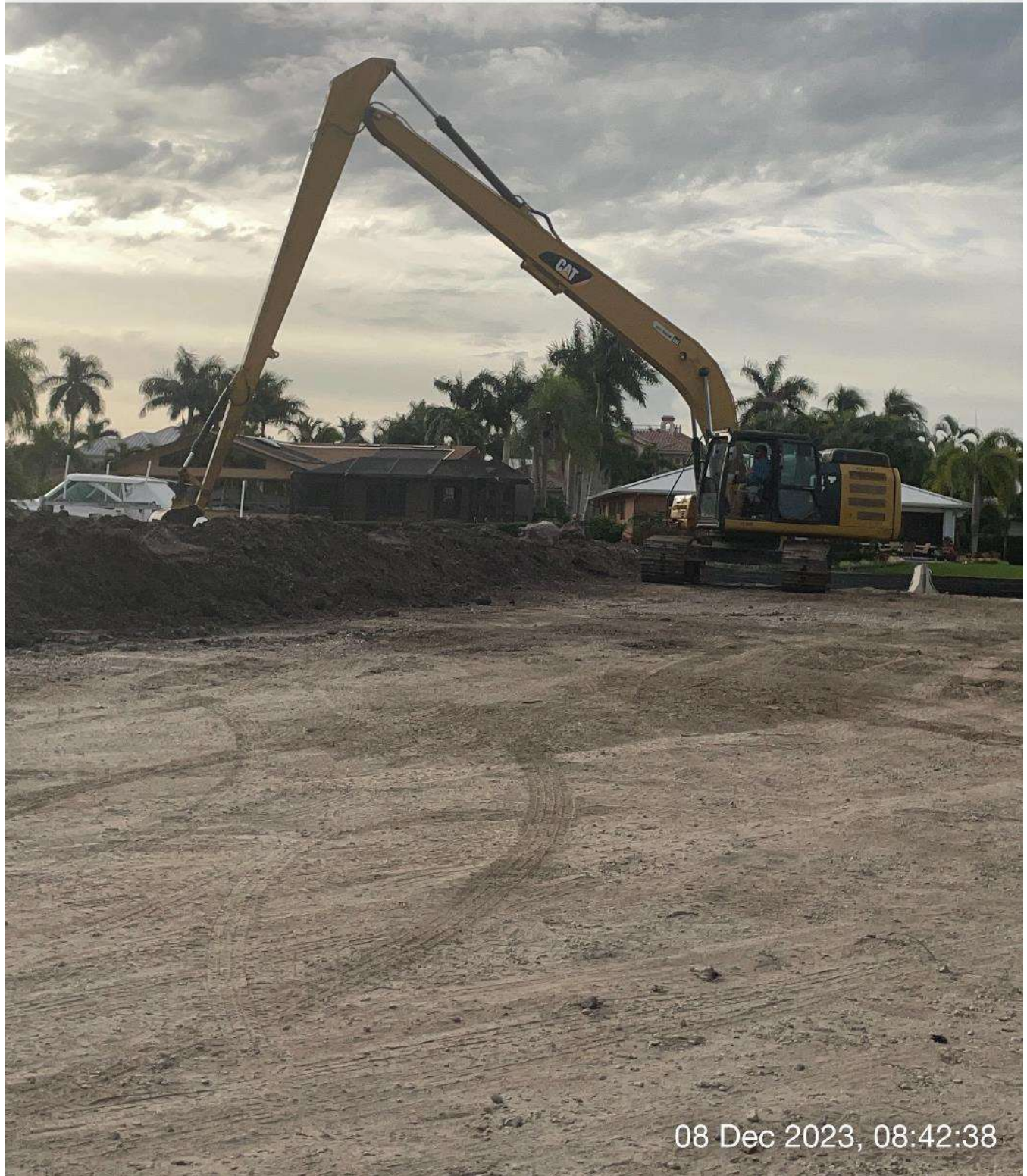
Long reach excavator separating wet and dry material on staging area.
