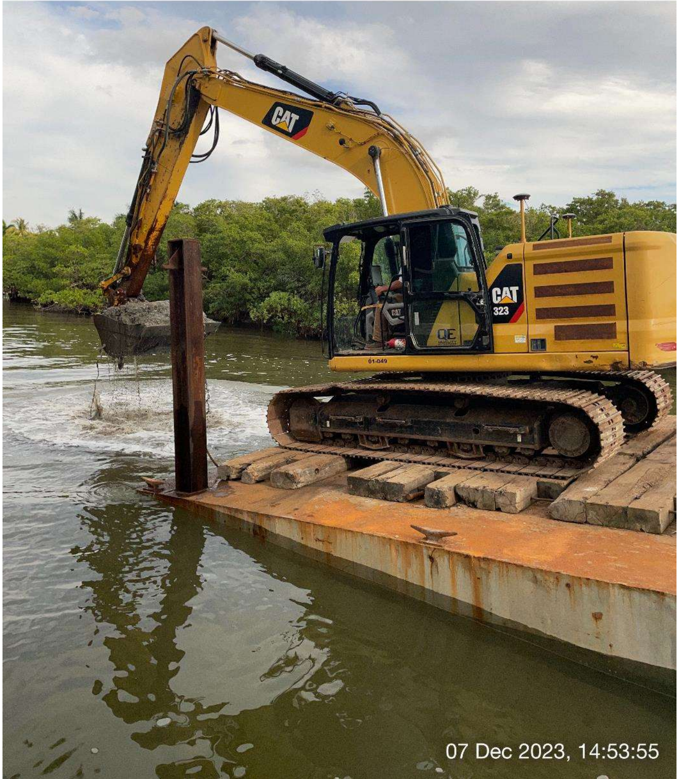
323 excavator removing sediment at station 6+50 in Canal Main B.
