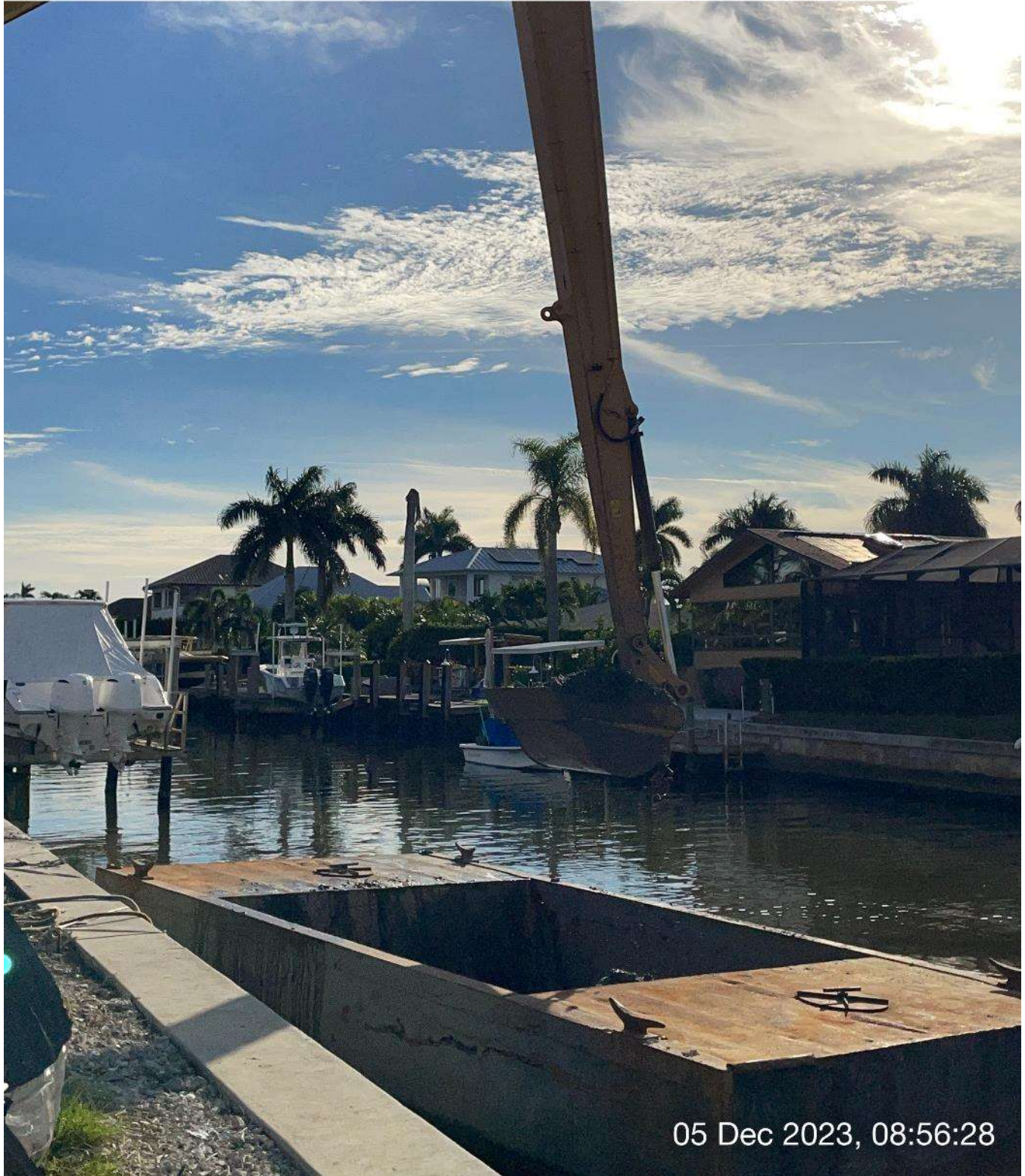
Long reach excavator removing sediment from hopper.
