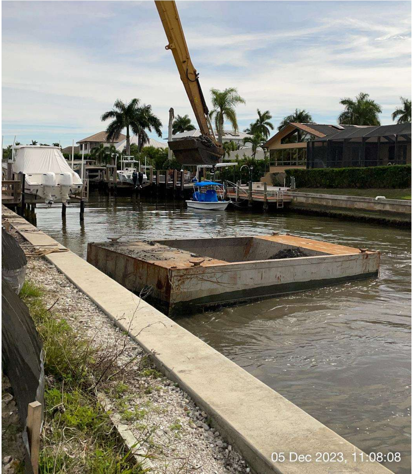
Long reach excavator removing sediment from hopper.
