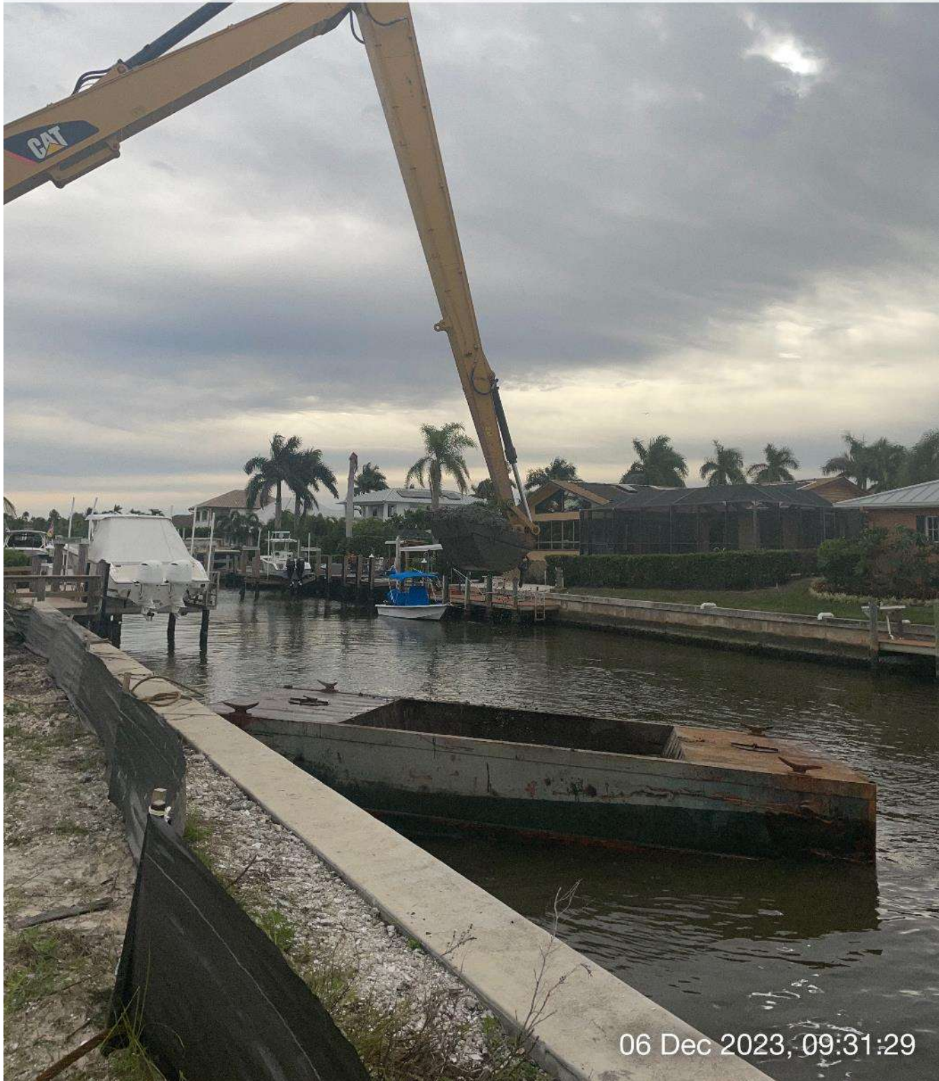
Long reach excavator removing sediment from hopper.
