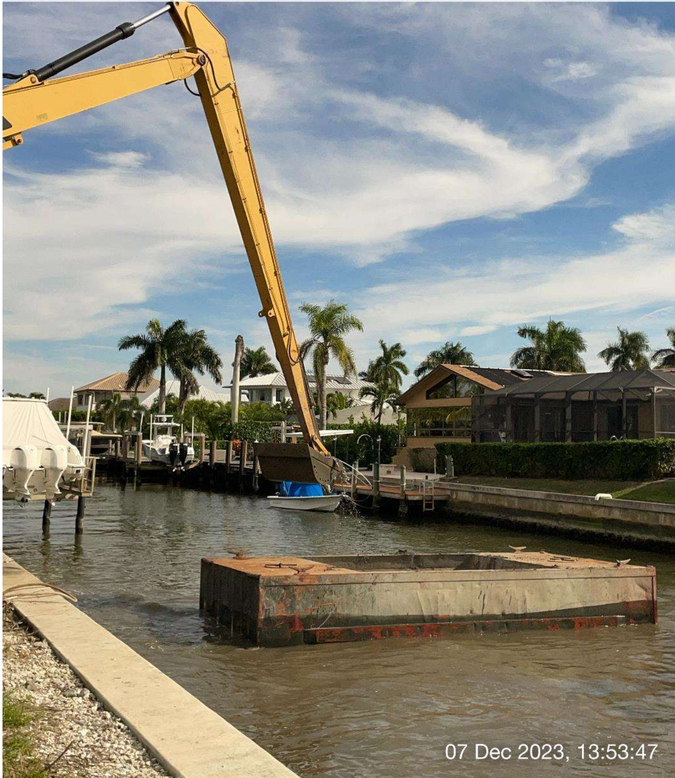
Long reach excavator removing sediment from hopper.
