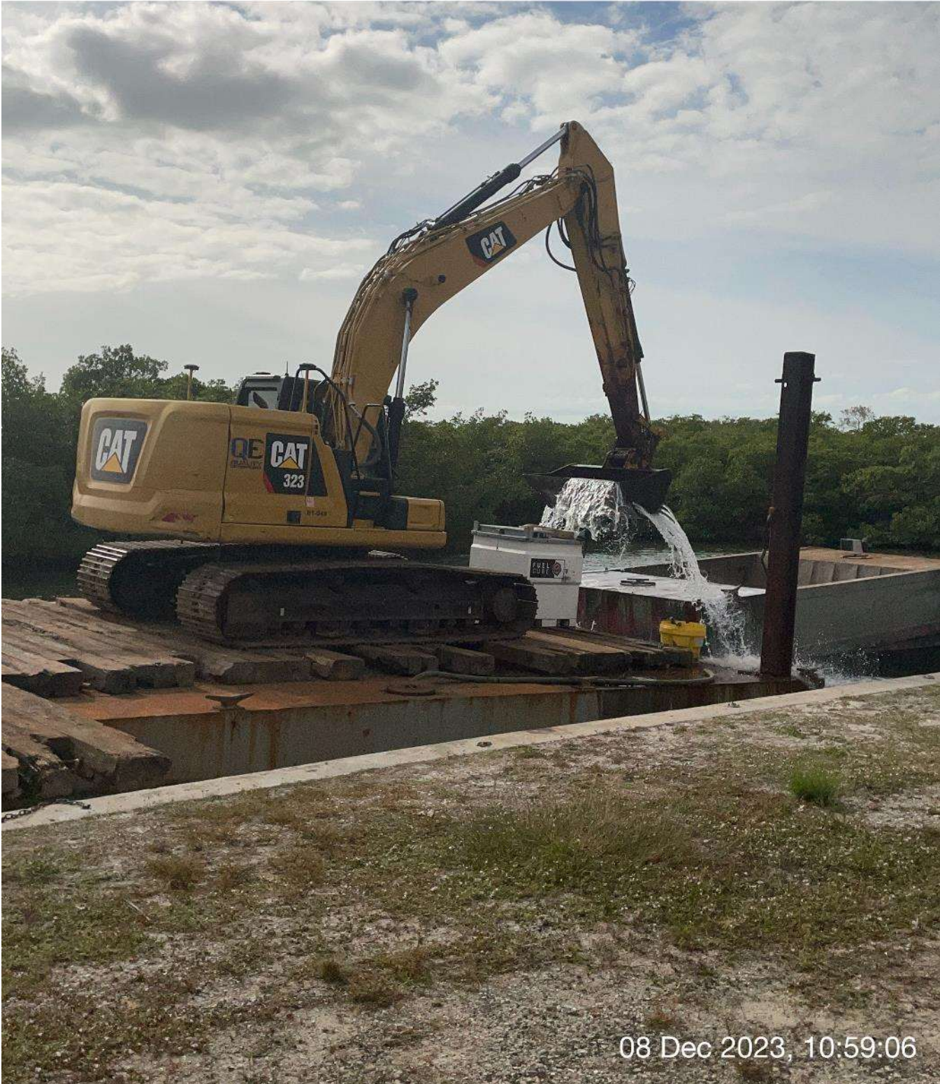
323 excavator rinsing the barge and hopper.
