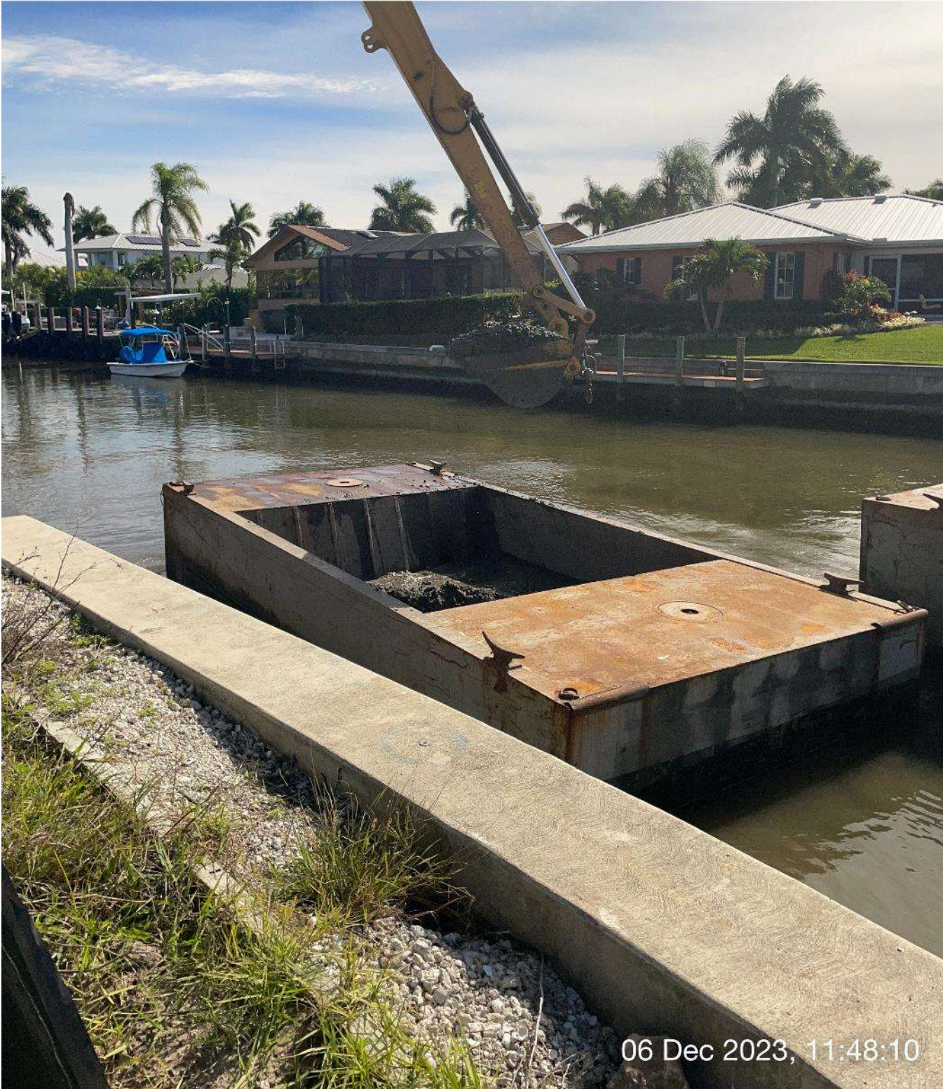
Long reach excavator removing sediment from hopper.
