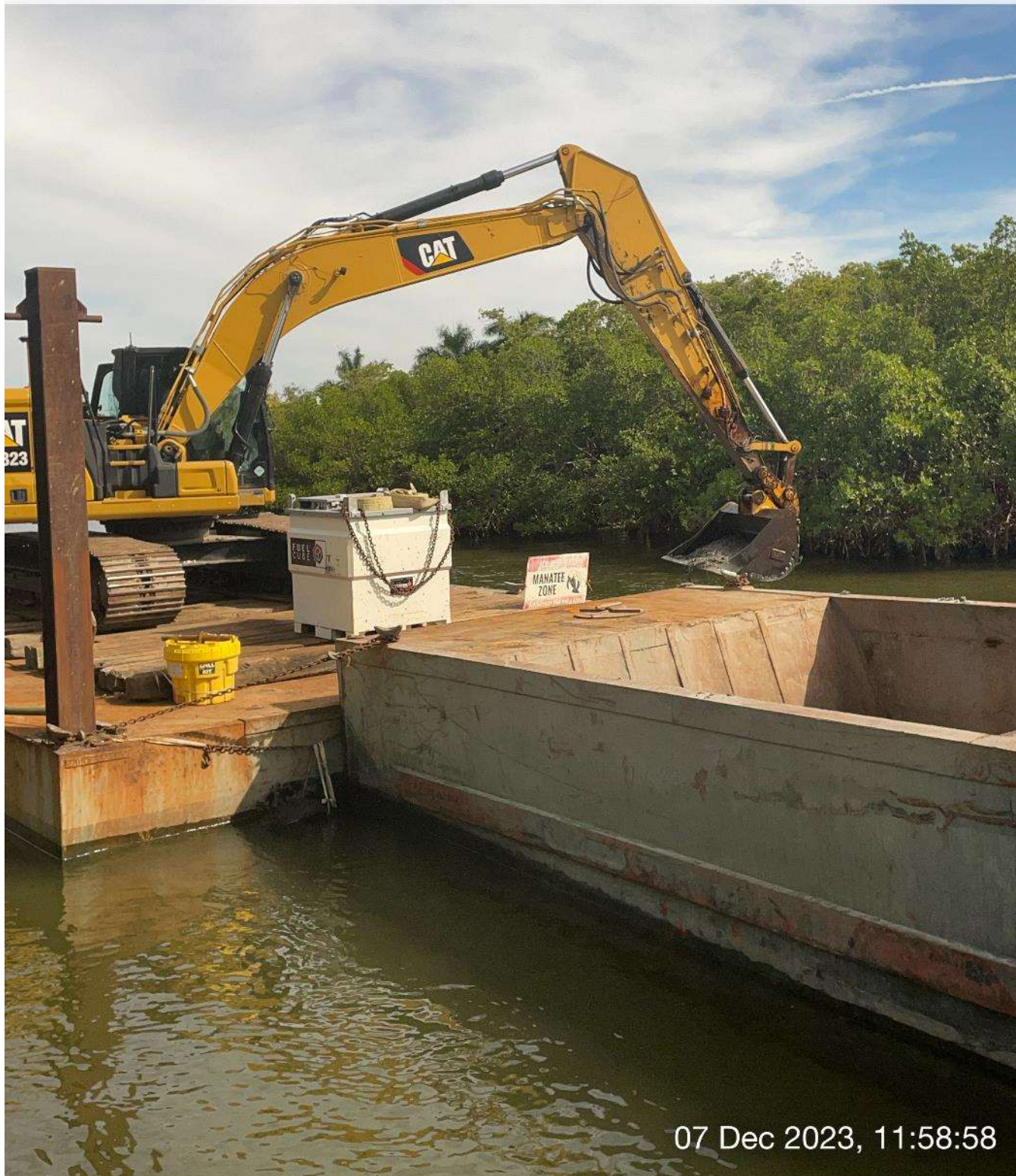
323 excavator removing sediment at station 7+00 in Canal Main B.
