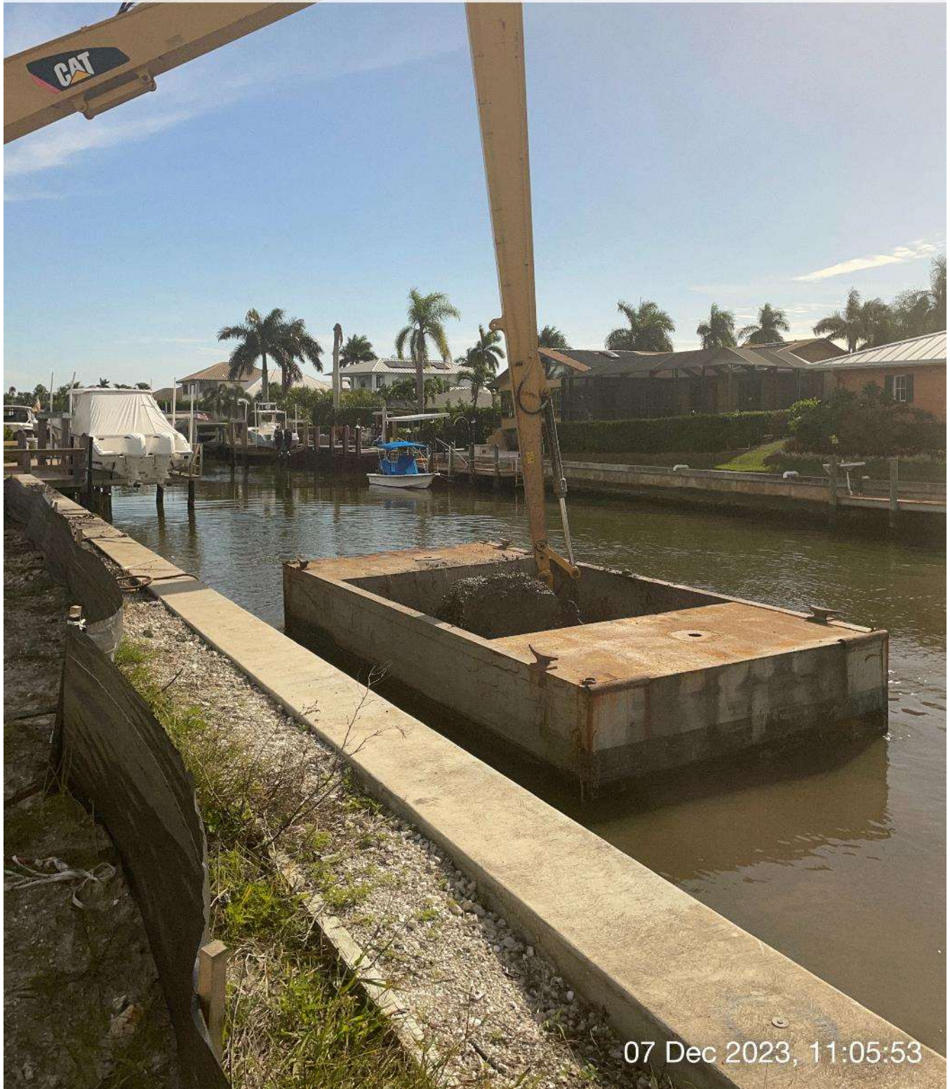
Long reach excavator removing sediment from hopper.
