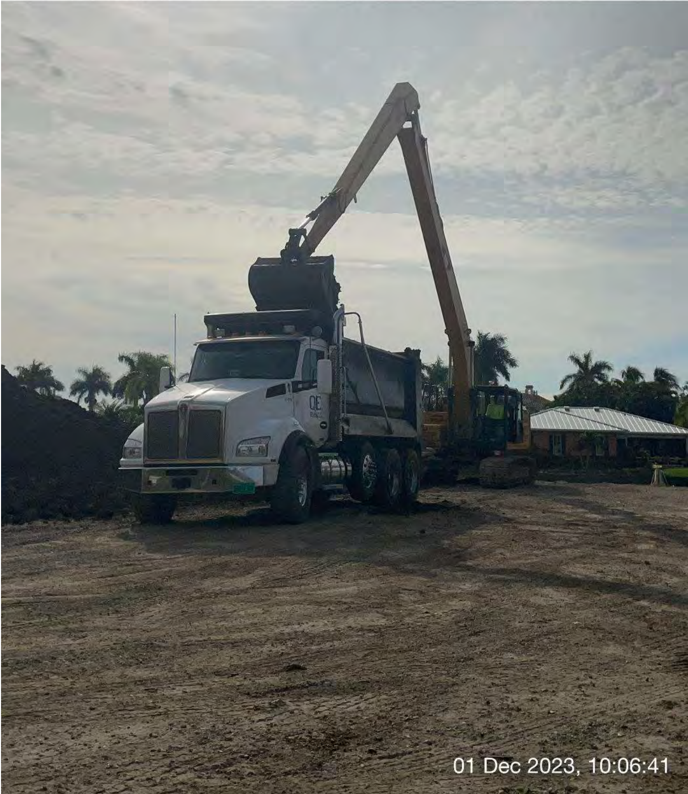
Long reach excavator loading dry sediment into dump truck.
