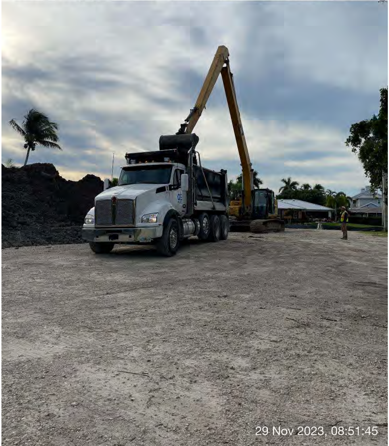
Long reach excavator loading sediment into dump truck.
