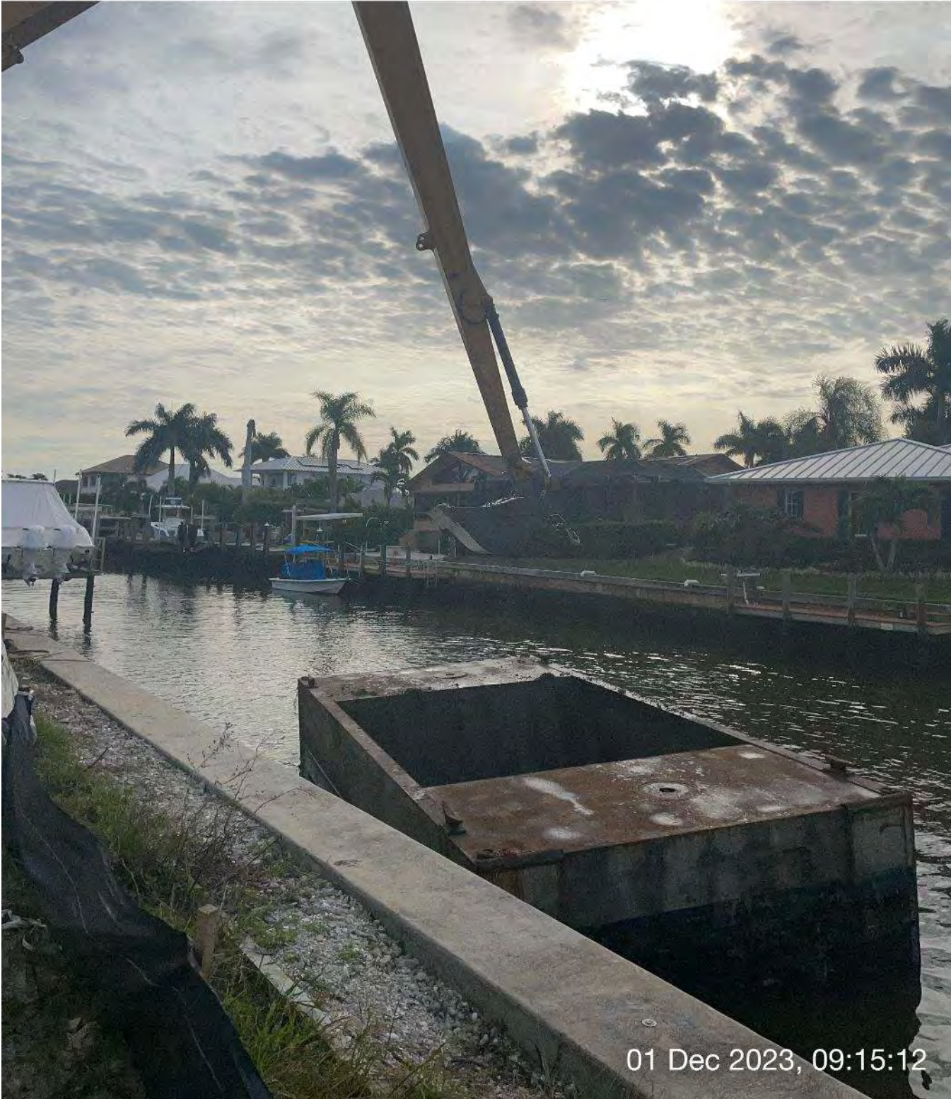
Long reach excavator removing sediment from hopper.
