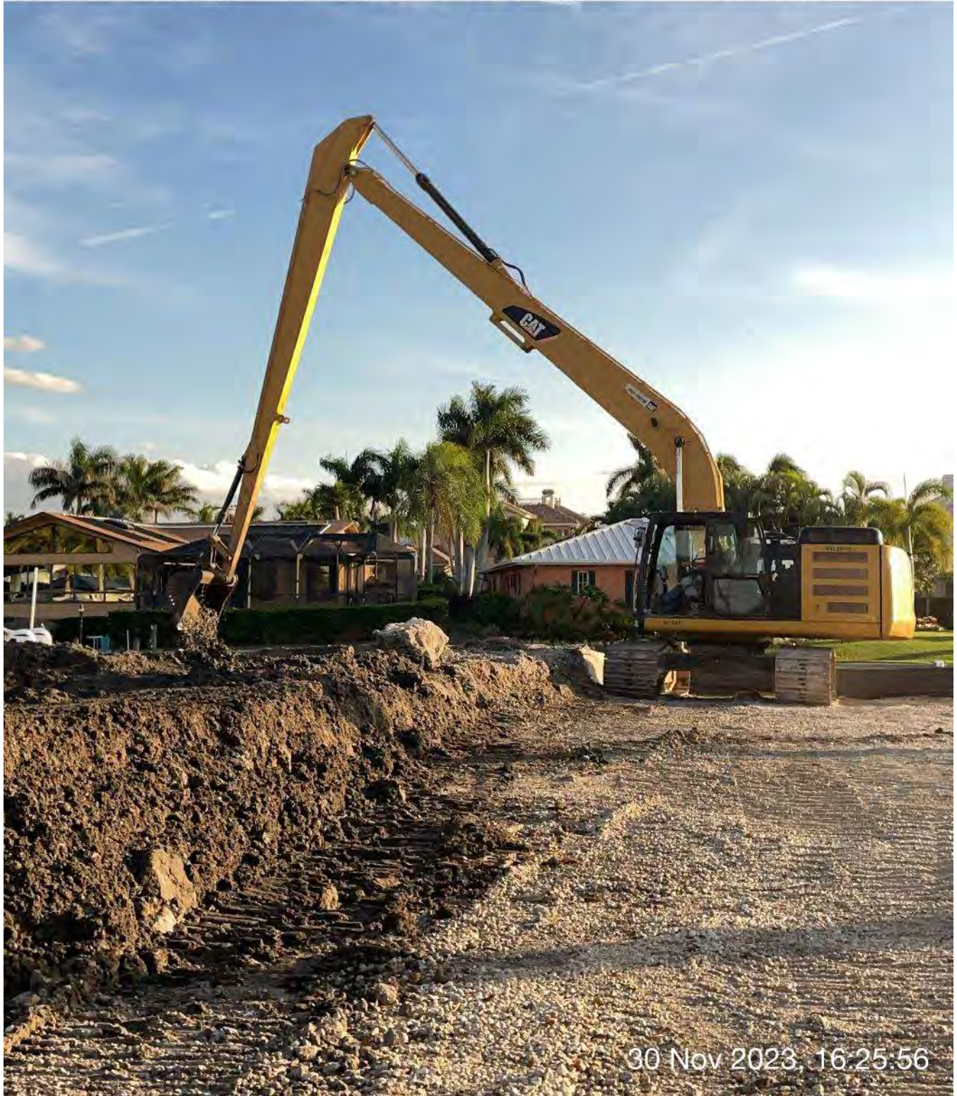
Long reach excavator spreading sediment onto staging area.
