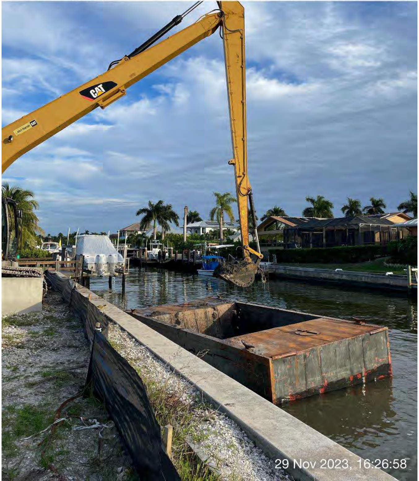
Long reach excavator removing sediment from hopper.
