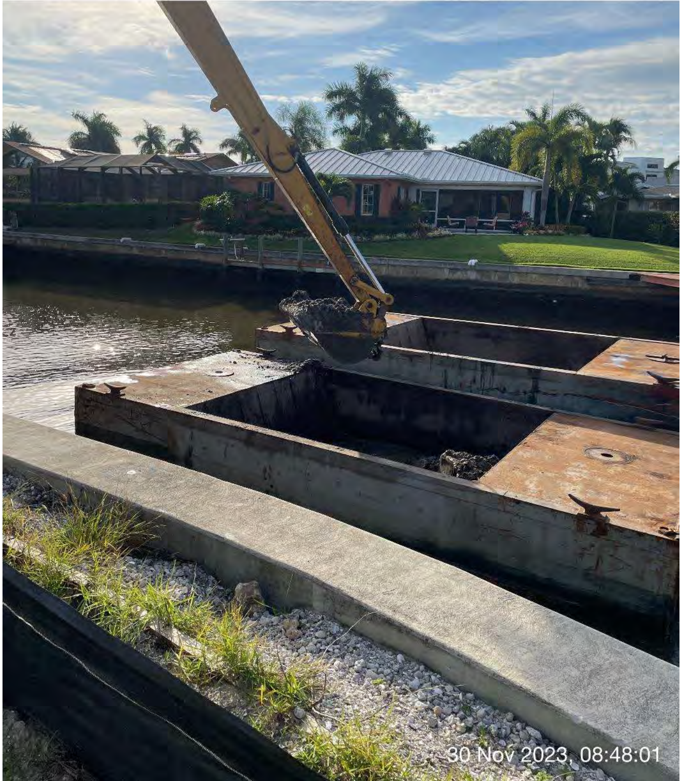
Long reach excavator removing sediment from hopper.
