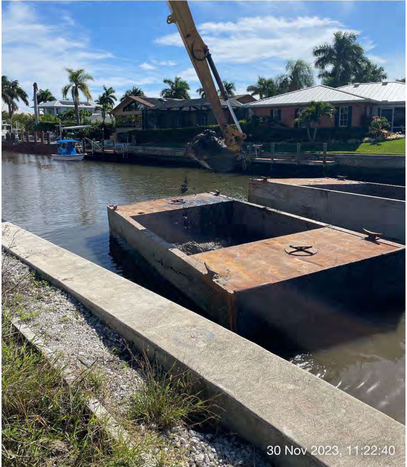
Long reach excavator removing sediment from hopper.
