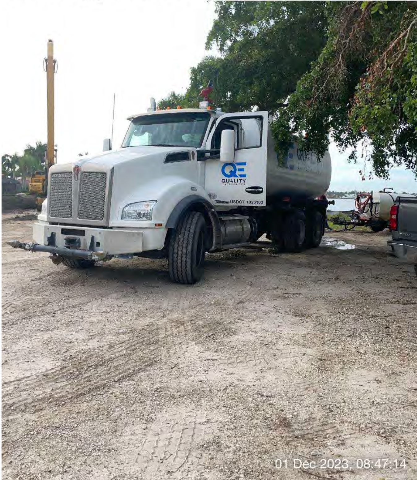
Water truck filling water tank on trailer.
