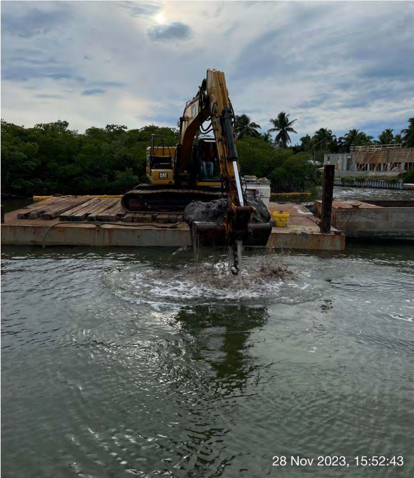
323 excavator removing sediment at station 1+00 in Canal Main B1.
