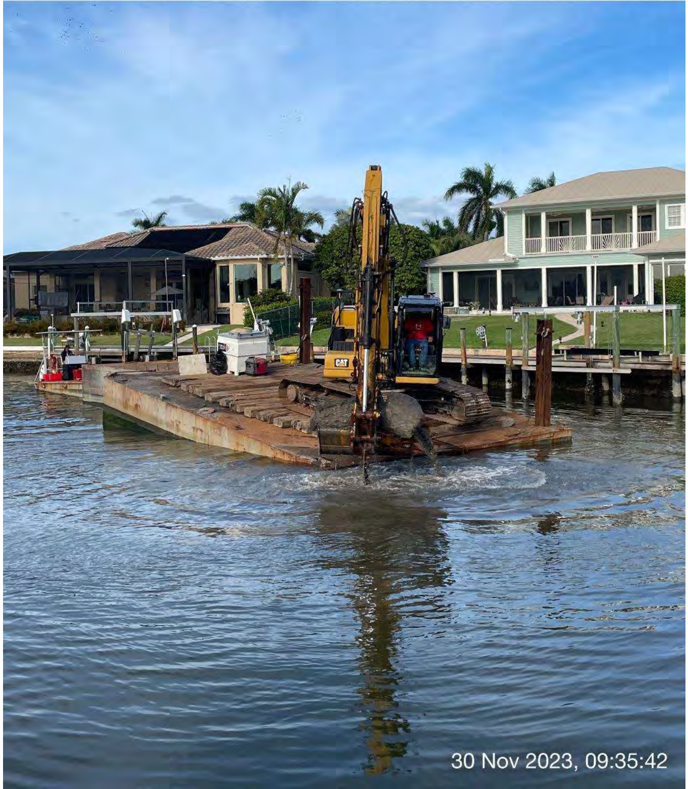
323 excavator removing sediment at station 0+50 in Canal Main B1.
