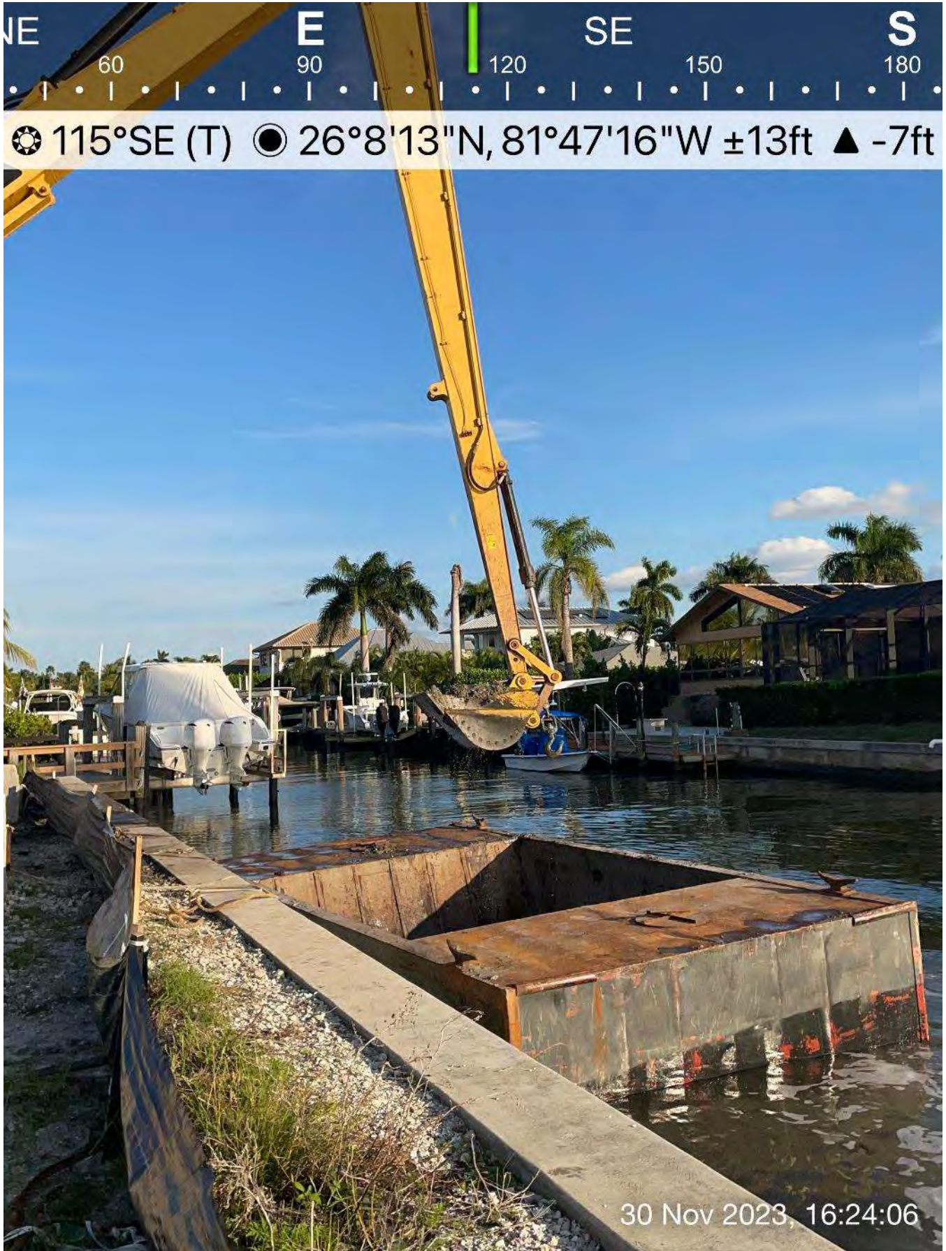
Long reach excavator removing sediment from hopper.
