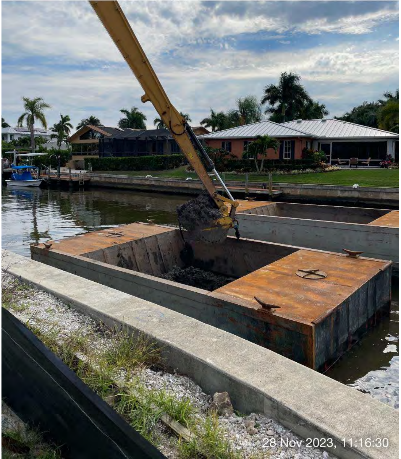
Long reach excavator removing sediment from hopper.
