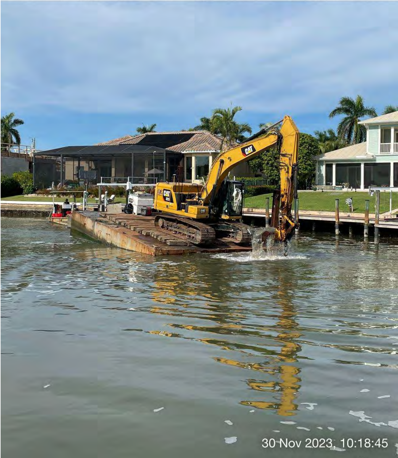
323 excavator removing sediment at station 0+00 in Canal Main B1.
