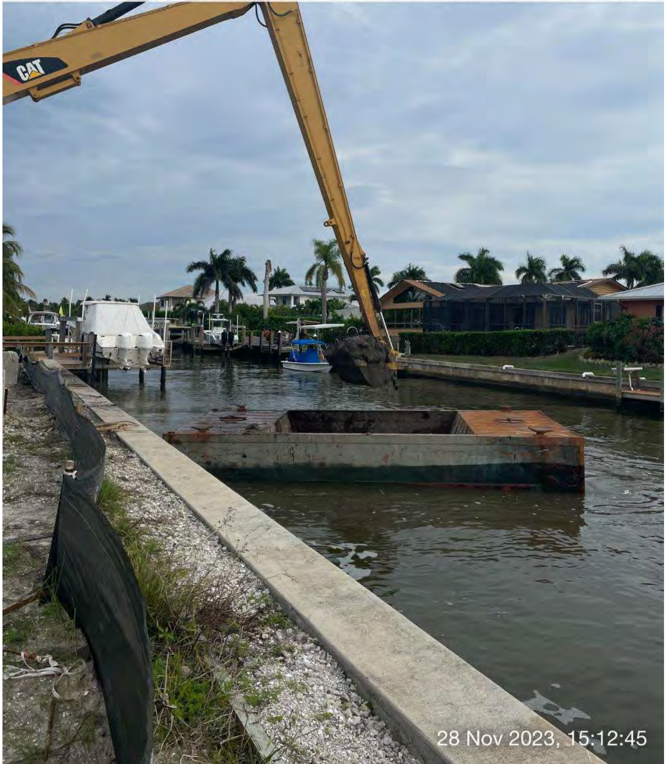
Long reach excavator removing sediment from hopper.
