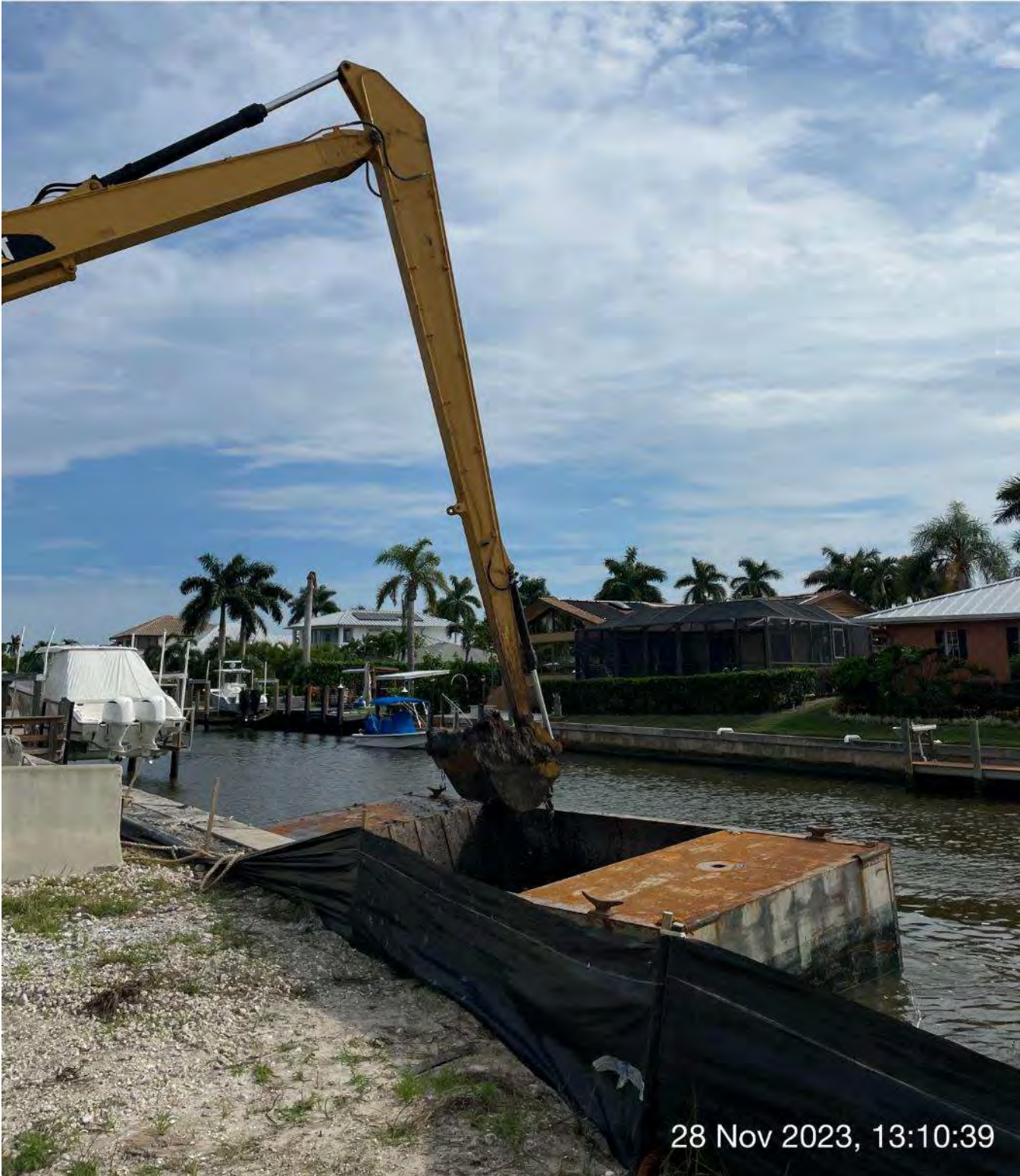
Long reach excavator removing sediment from hopper.
