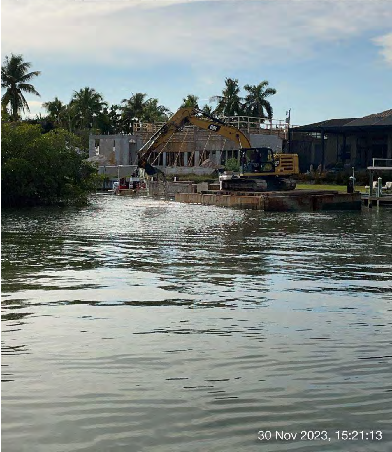
323 excavator removing sediment at station 8+50 in Canal Main B.
