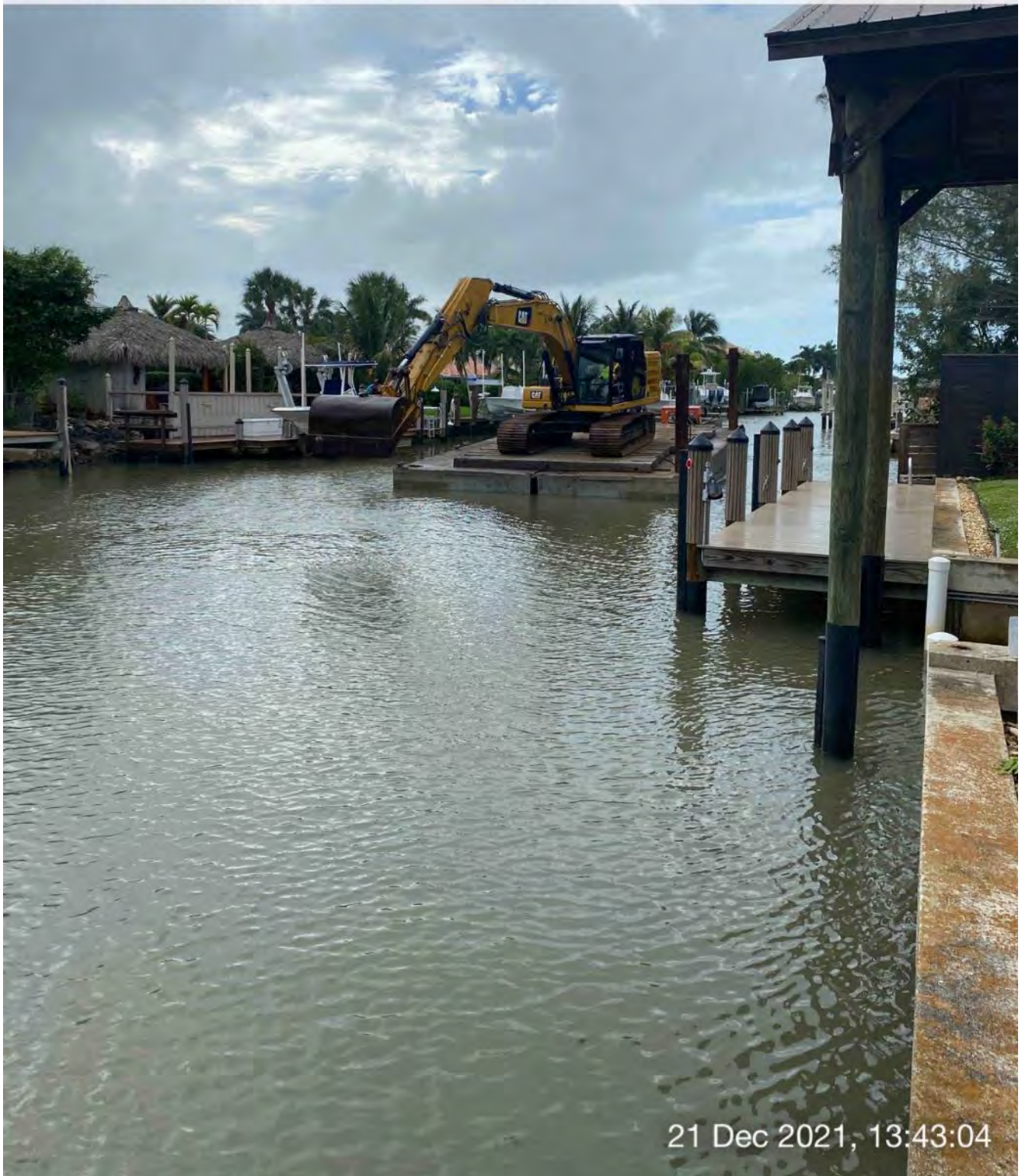
323 excavator checking bottom elevations at station 12+50
