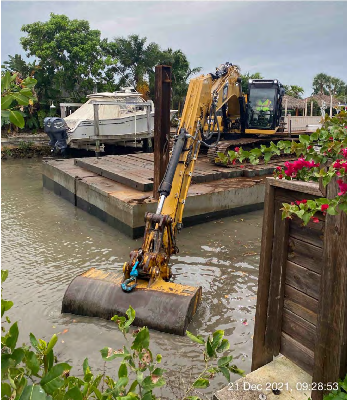
323 excavator removing material and transferring to hopper at station 13+00
