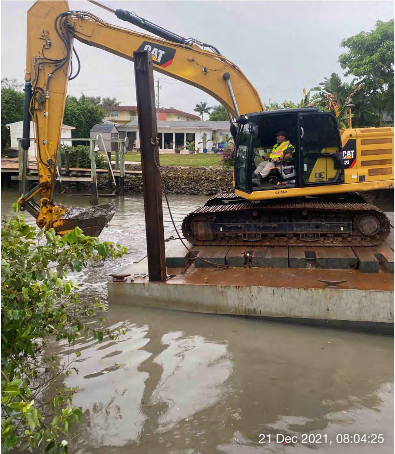
323 excavator removing material at station 13+50
