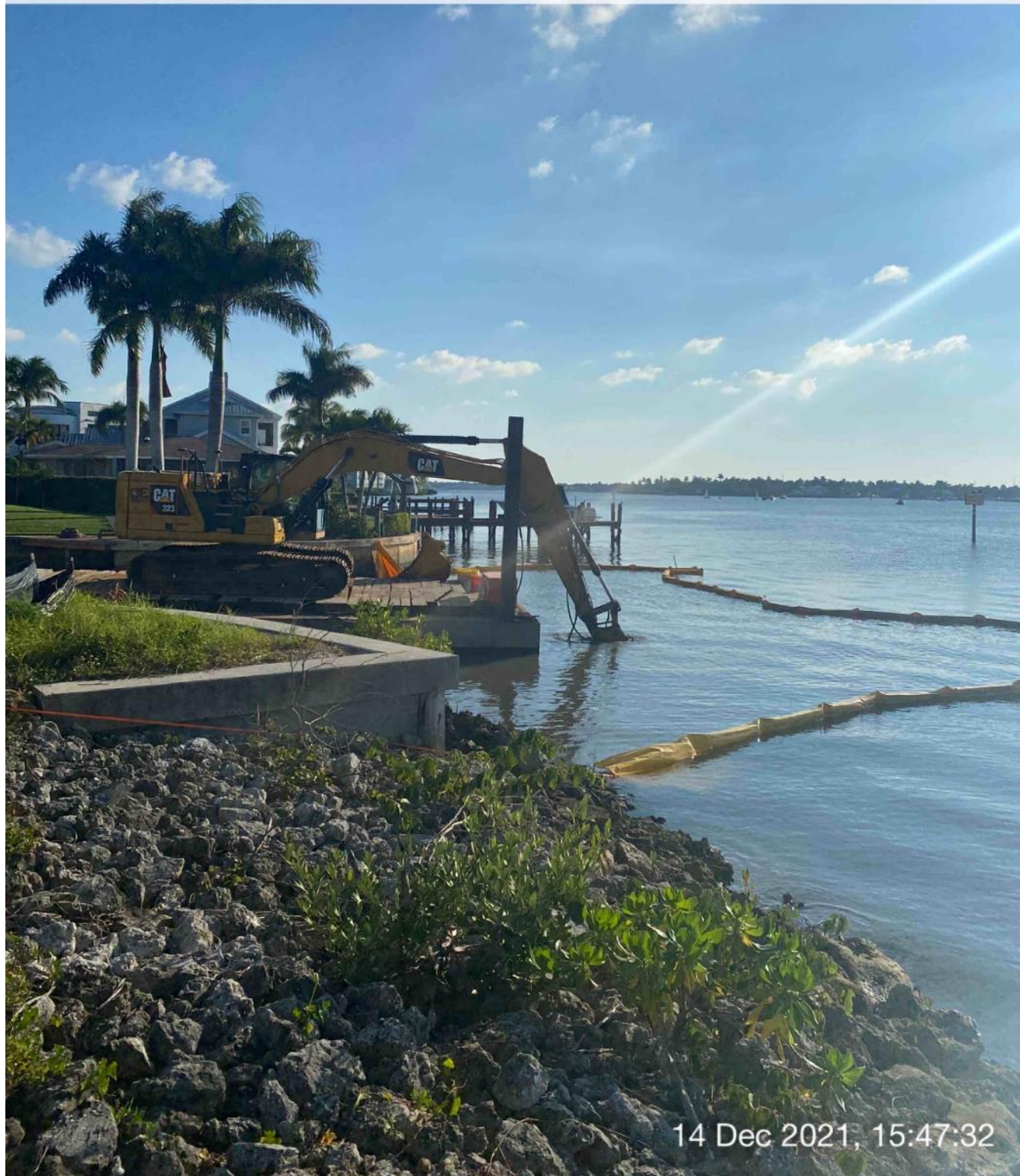
323 excavator grinding rock at station 1+00
