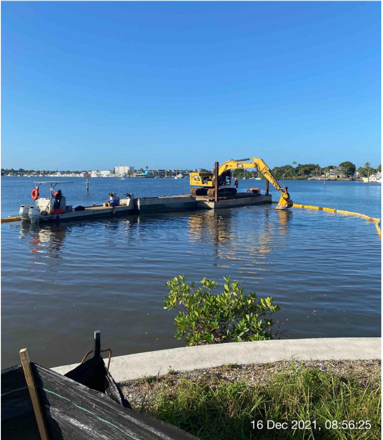
323 excavator removing material from station 0+00
