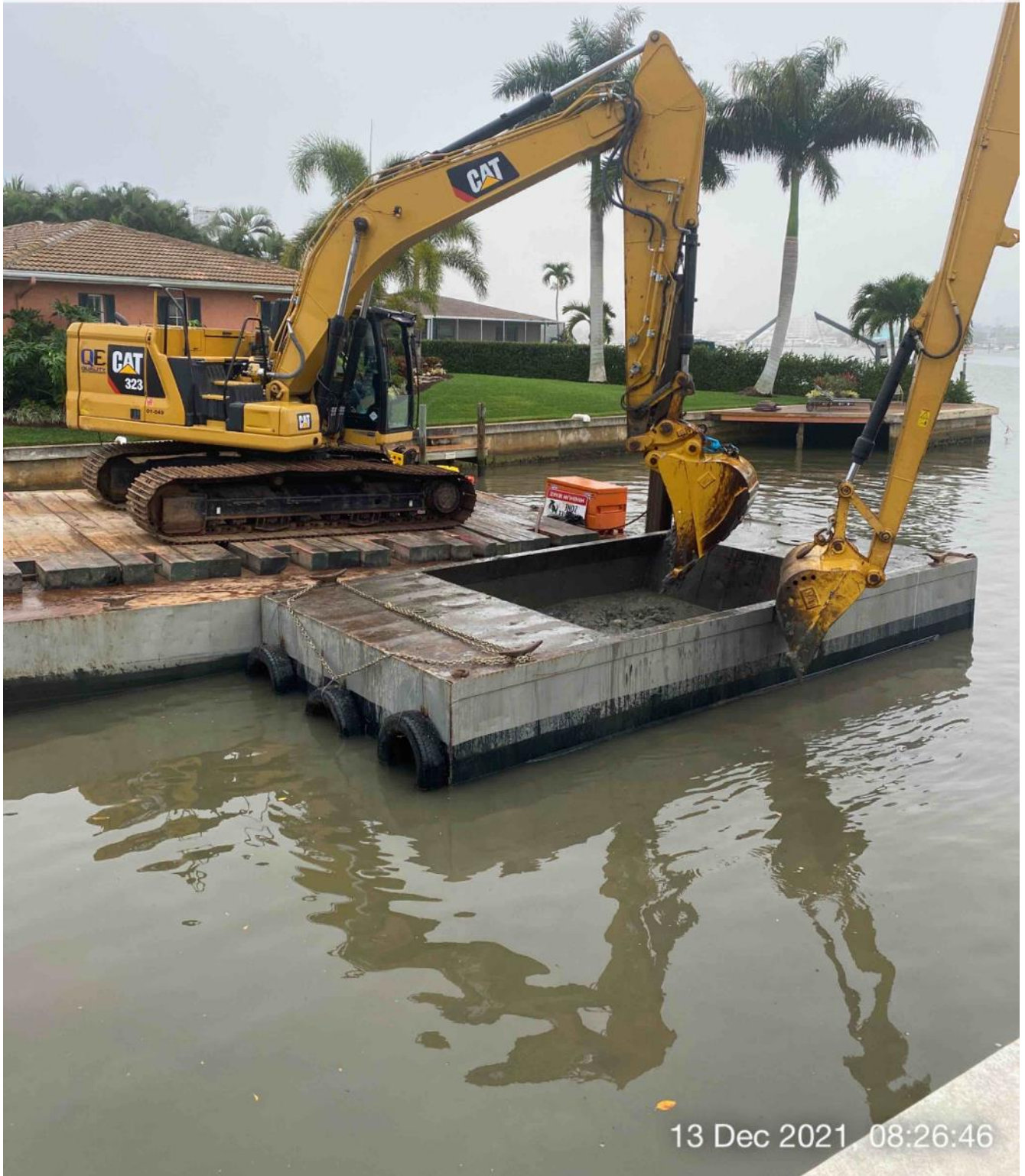
323 excavator removing material from station 1+50 and transferring it to hopper
