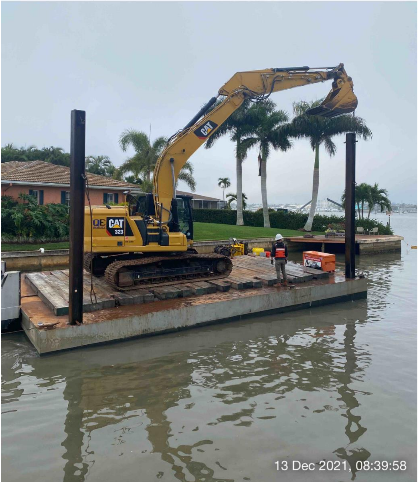
323 excavator lifting spud to allow push boat to move barge from station 4+00 to 3+50
