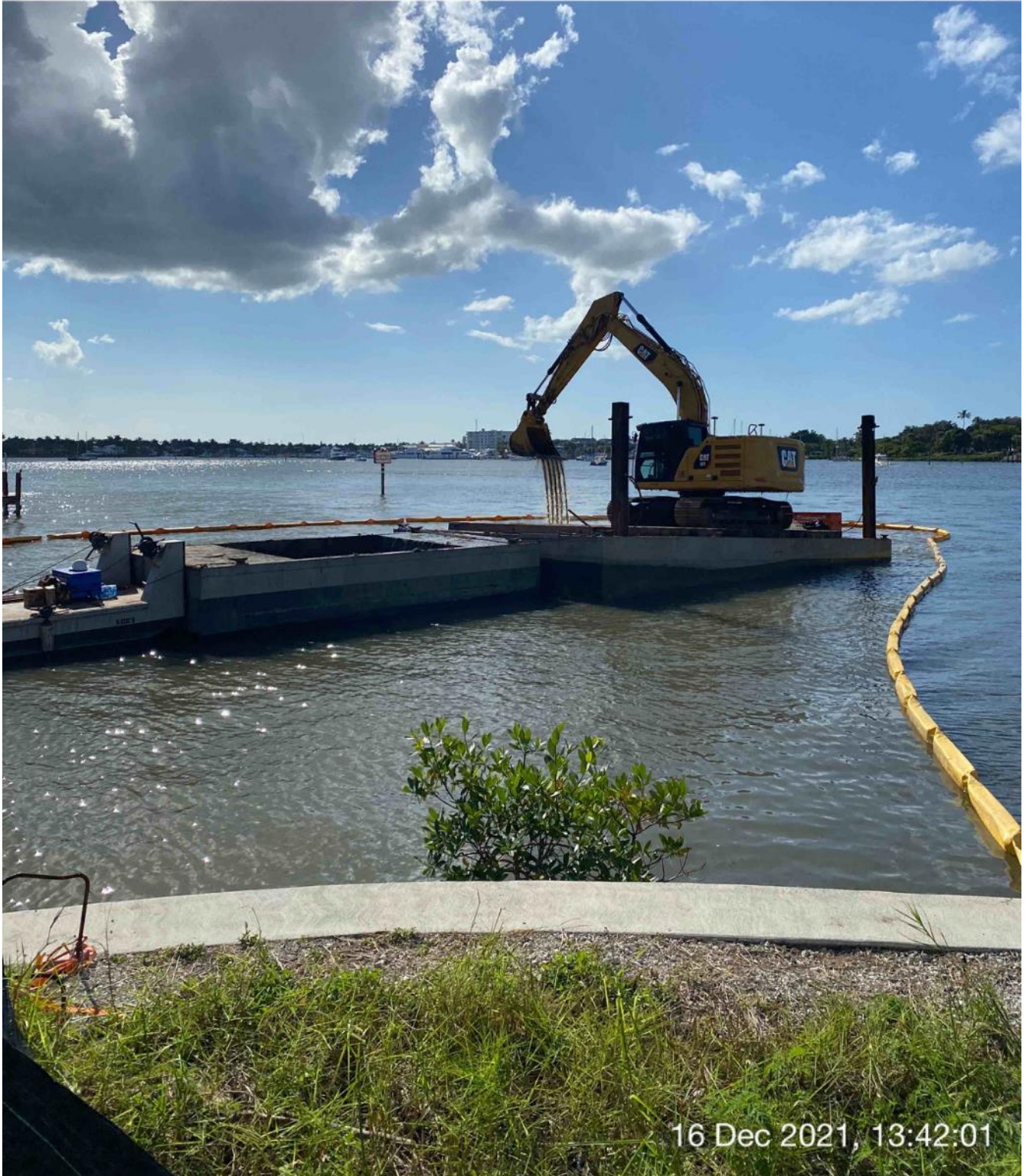
323 excavator removing material from station 0+50 and transferring it to hopper
