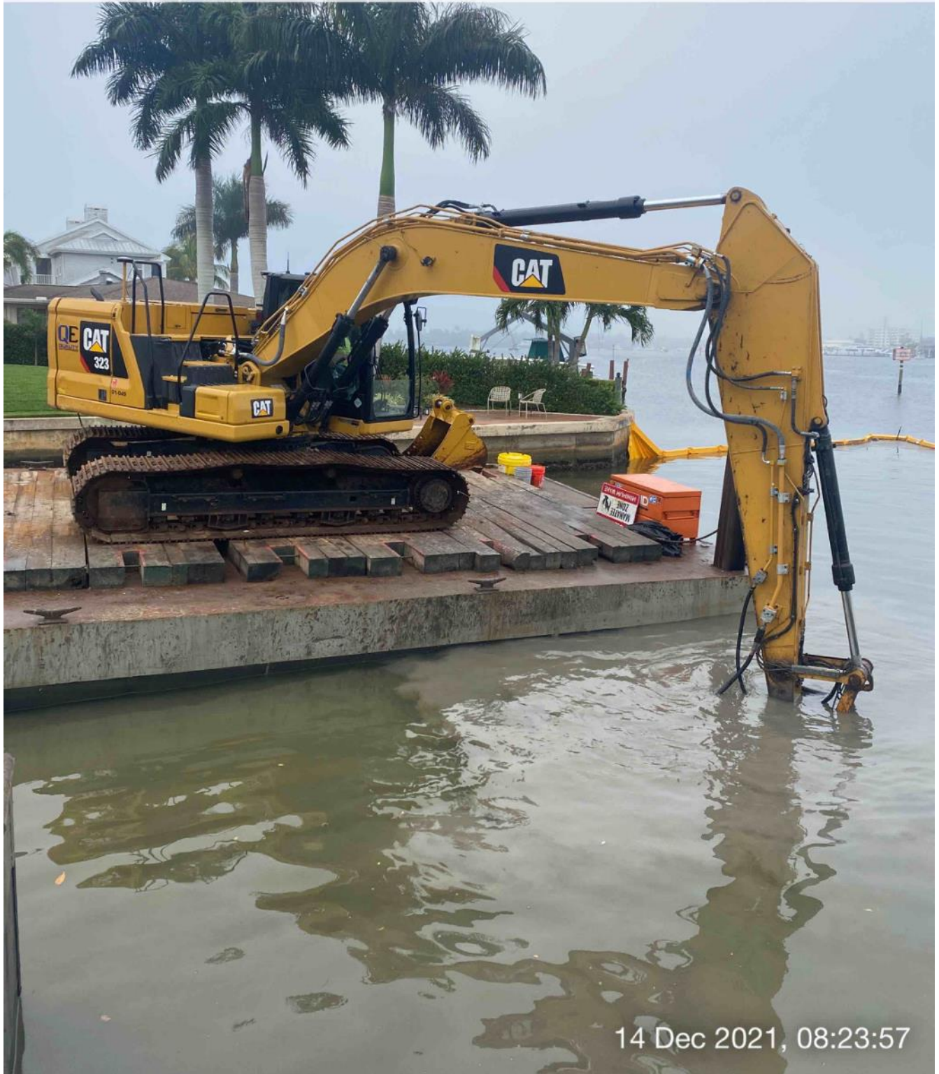
323 excavator grinding rock at station 1+50
