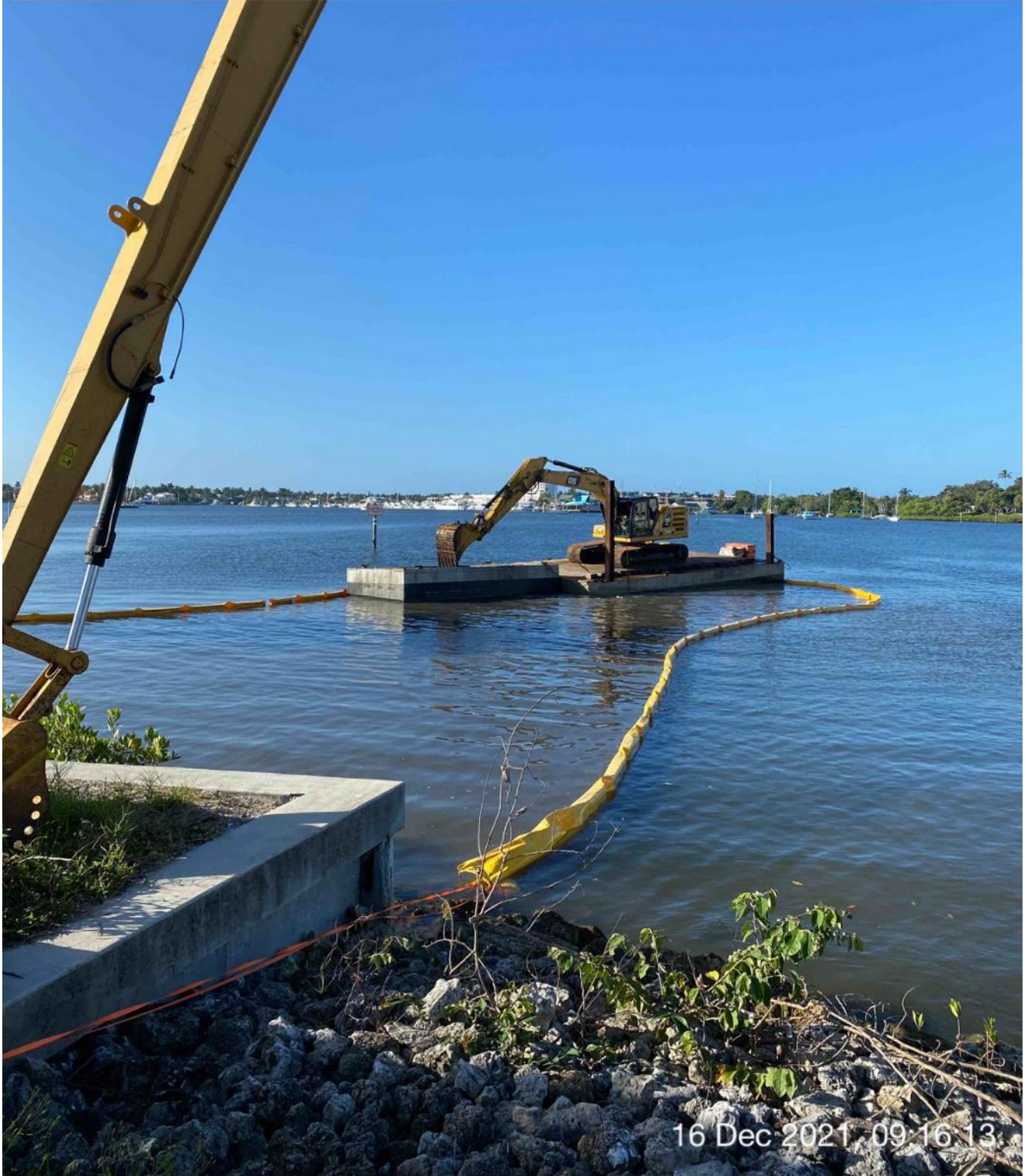
323 excavator removing material from station 0+00 and transferring it to hopper
