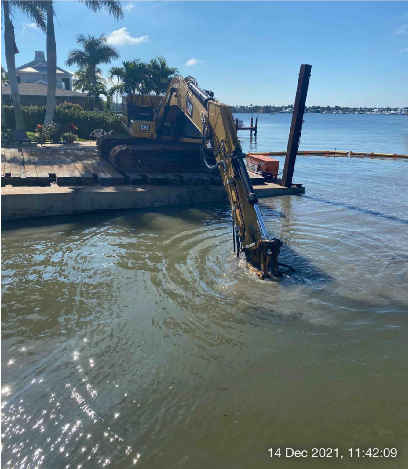
323 excavator grinding rock at station 1+50
