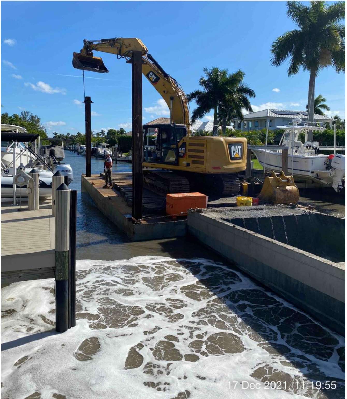
323 excavator lifting spud to allow push boat to move barge from station 3+50 to 3+00
