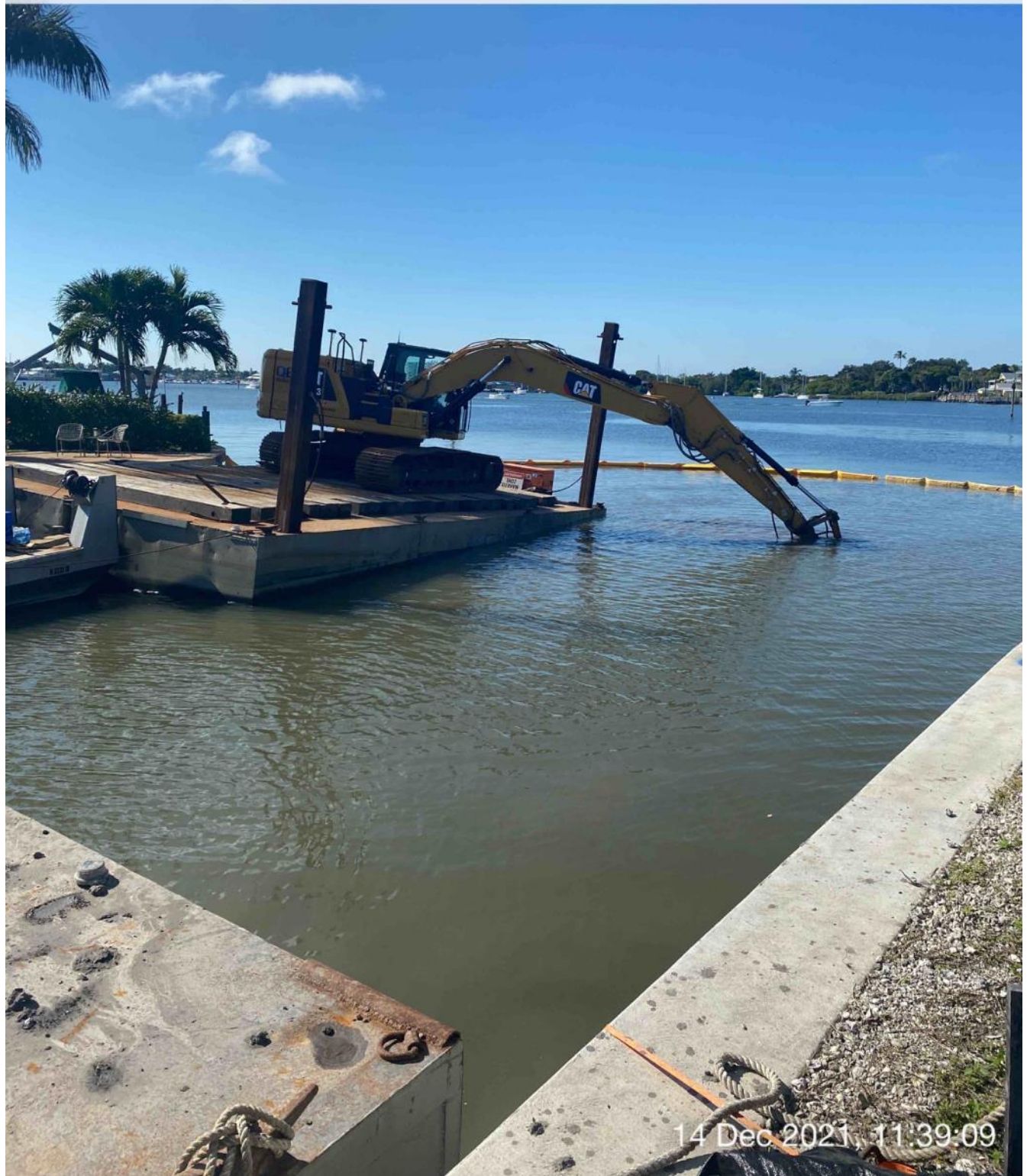
323 excavator grinding rock at station 1+50
