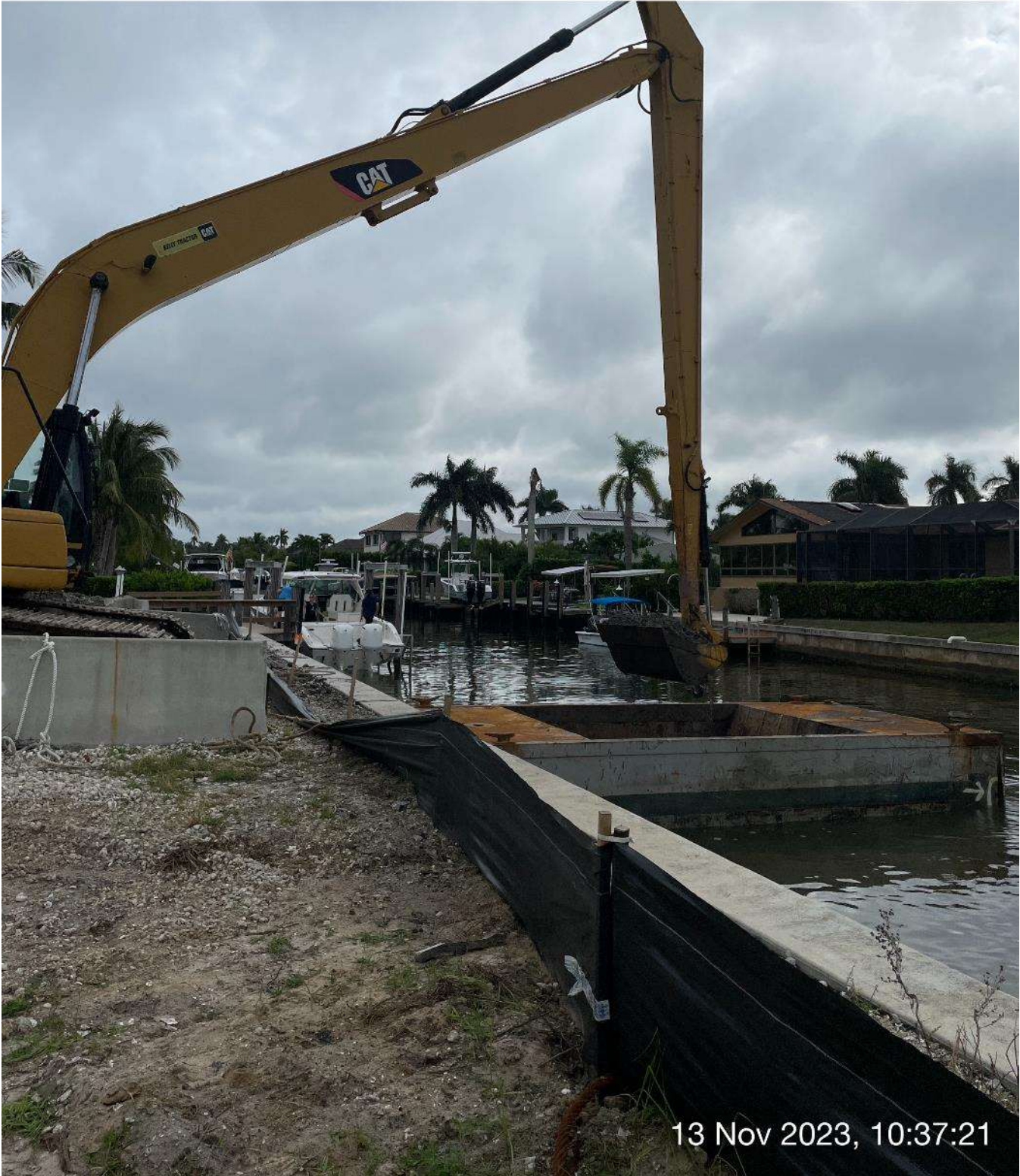
Long reach excavator removing sediment from hopper.
