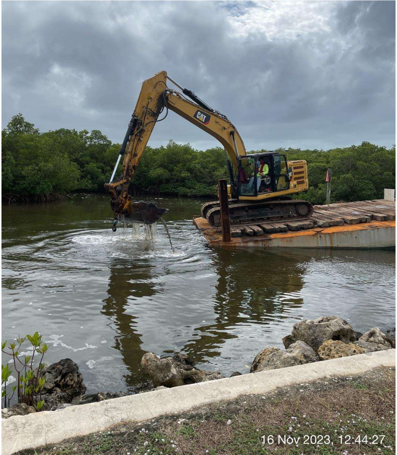
323 excavator removing sediment at station 2+25 in Canal Main B1.
