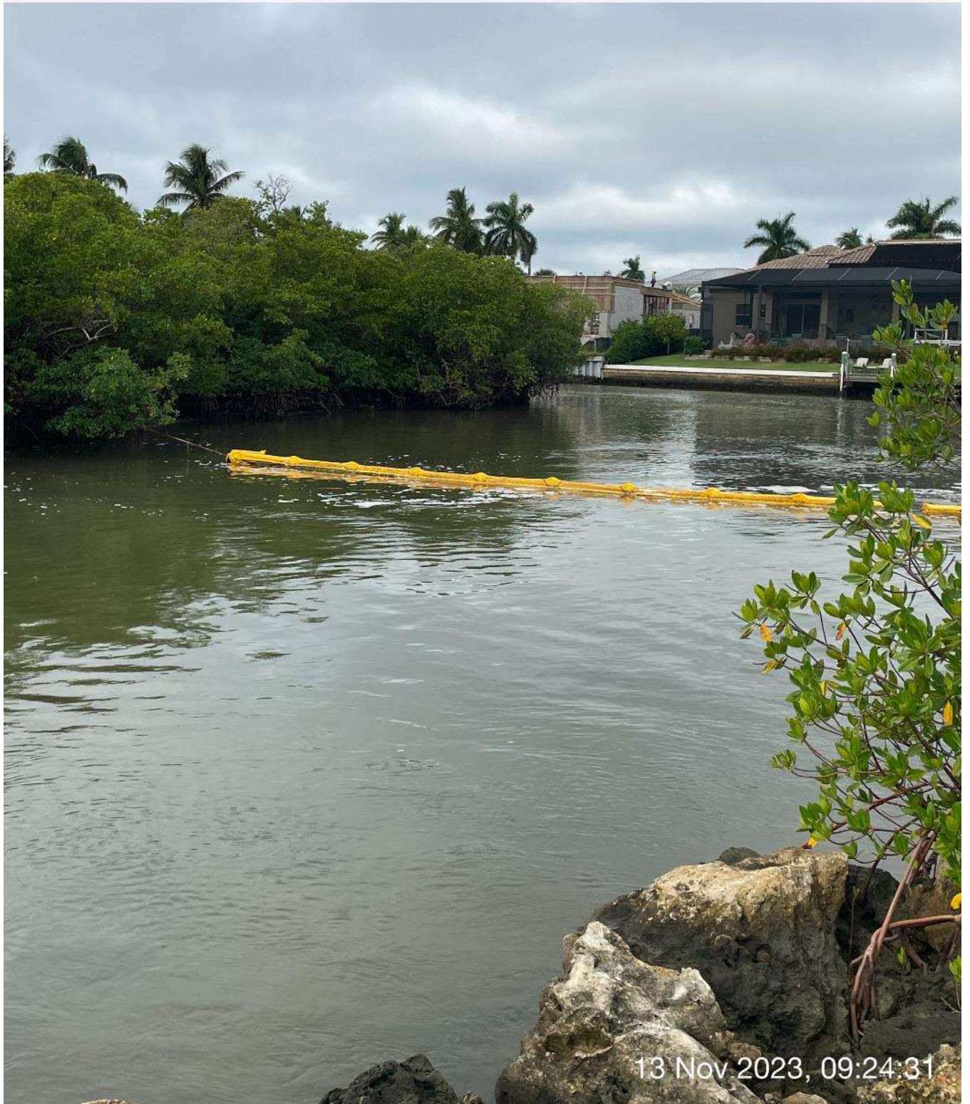
Turbidity curtain in place at station 1+50 in Canal Main B1.
