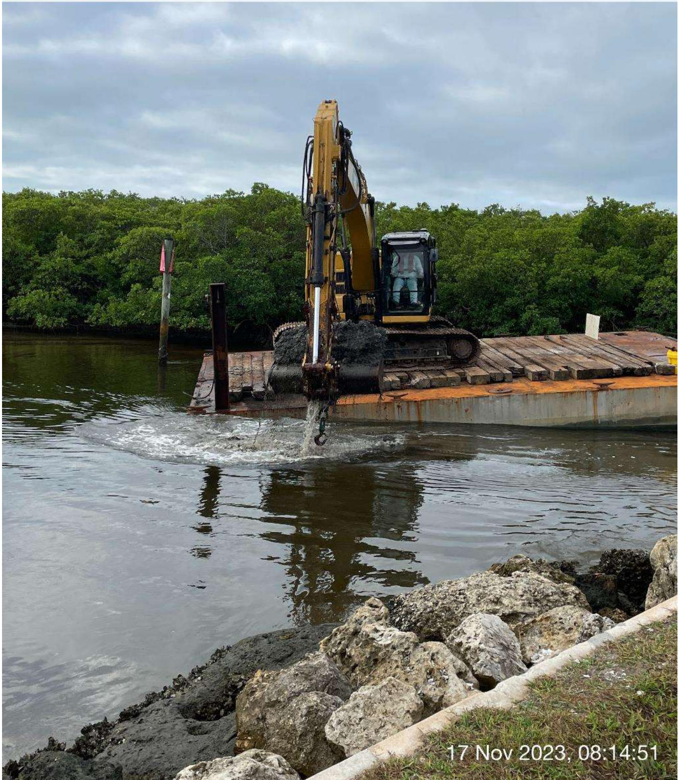
323 excavator removing sediment at station 2+00 in Canal Main B1.
