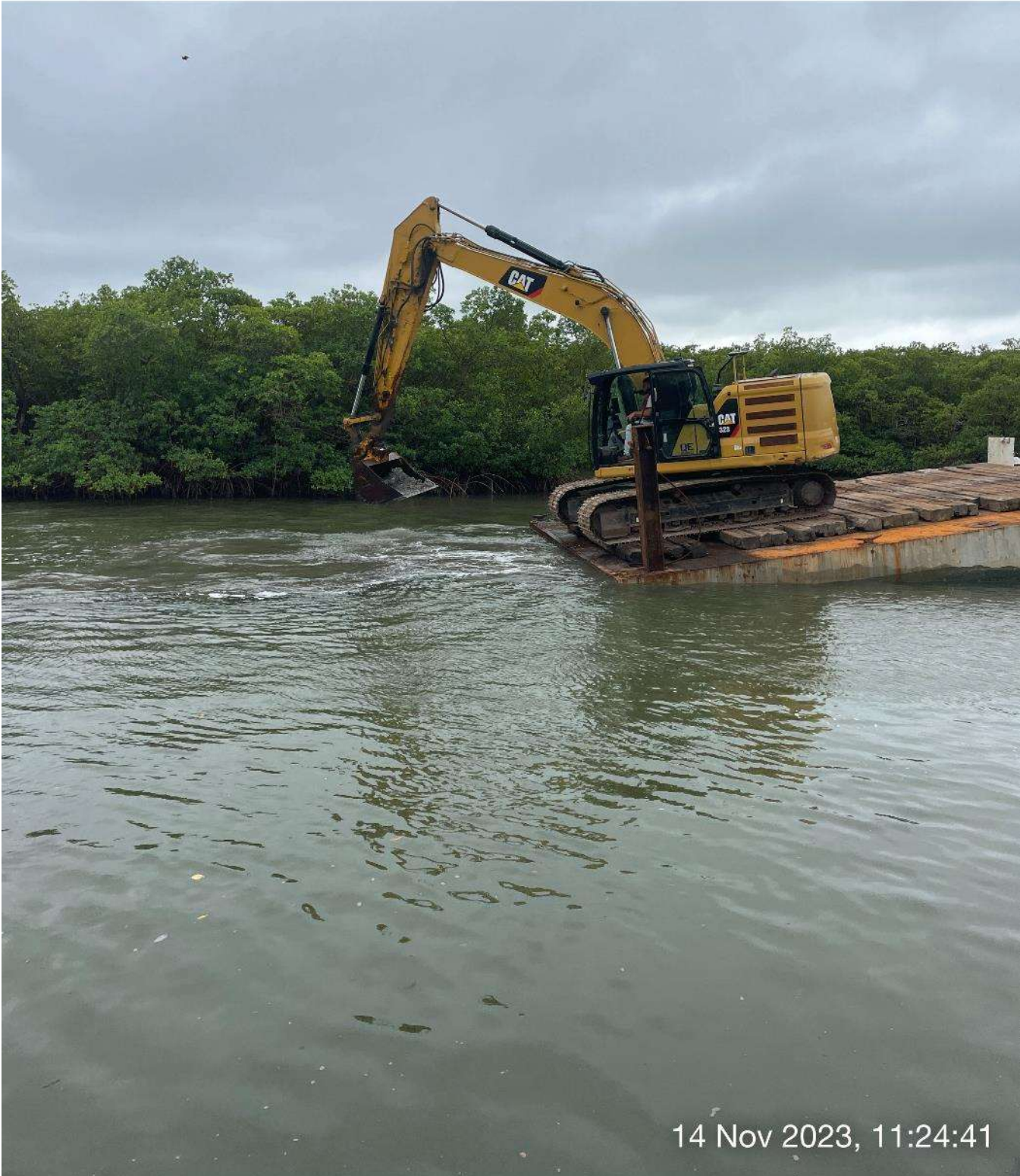
323 excavator removing sediment at station 2+50 in Canal Main B1.
