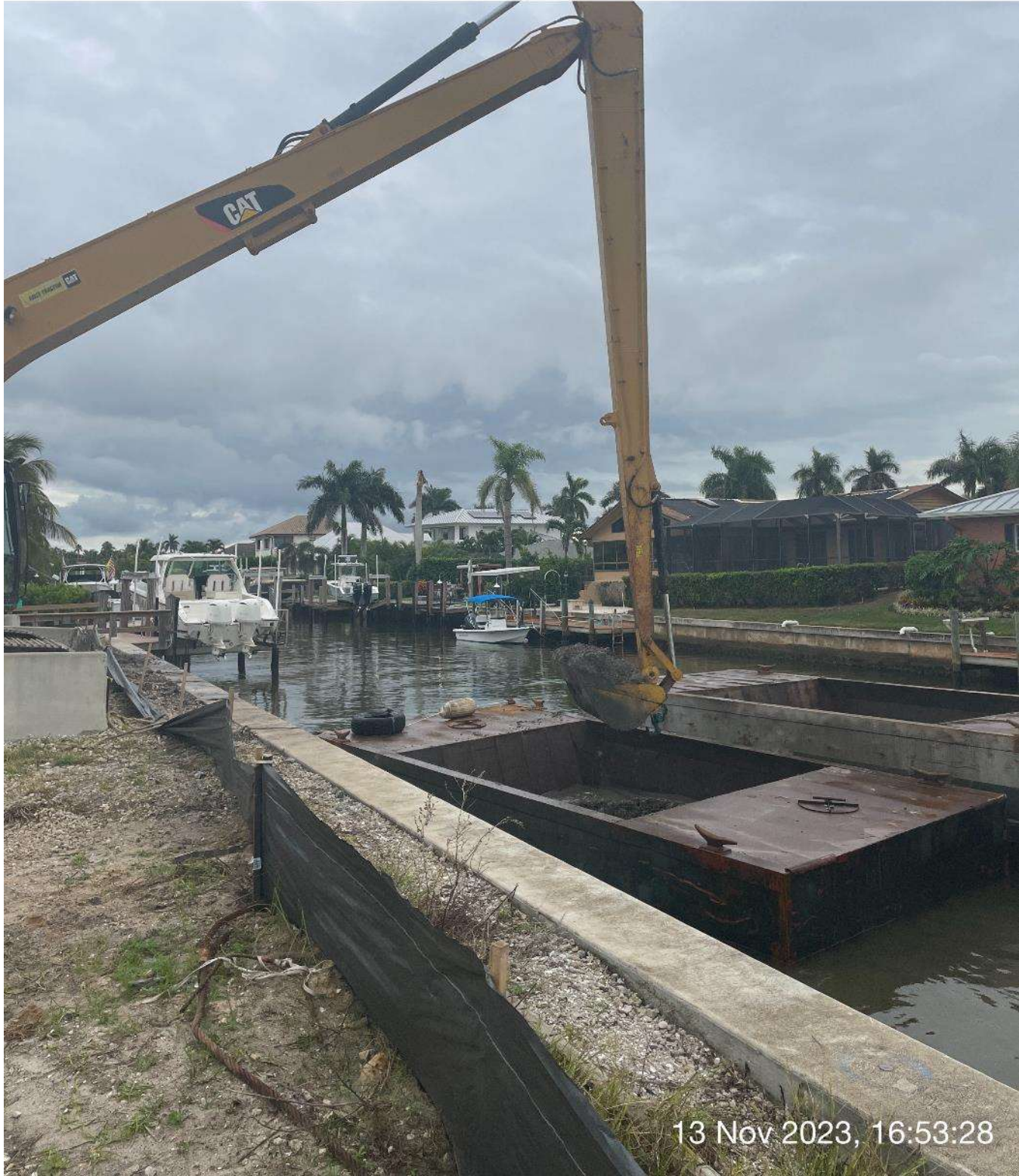
Long reach excavator removing sediment from hopper.
