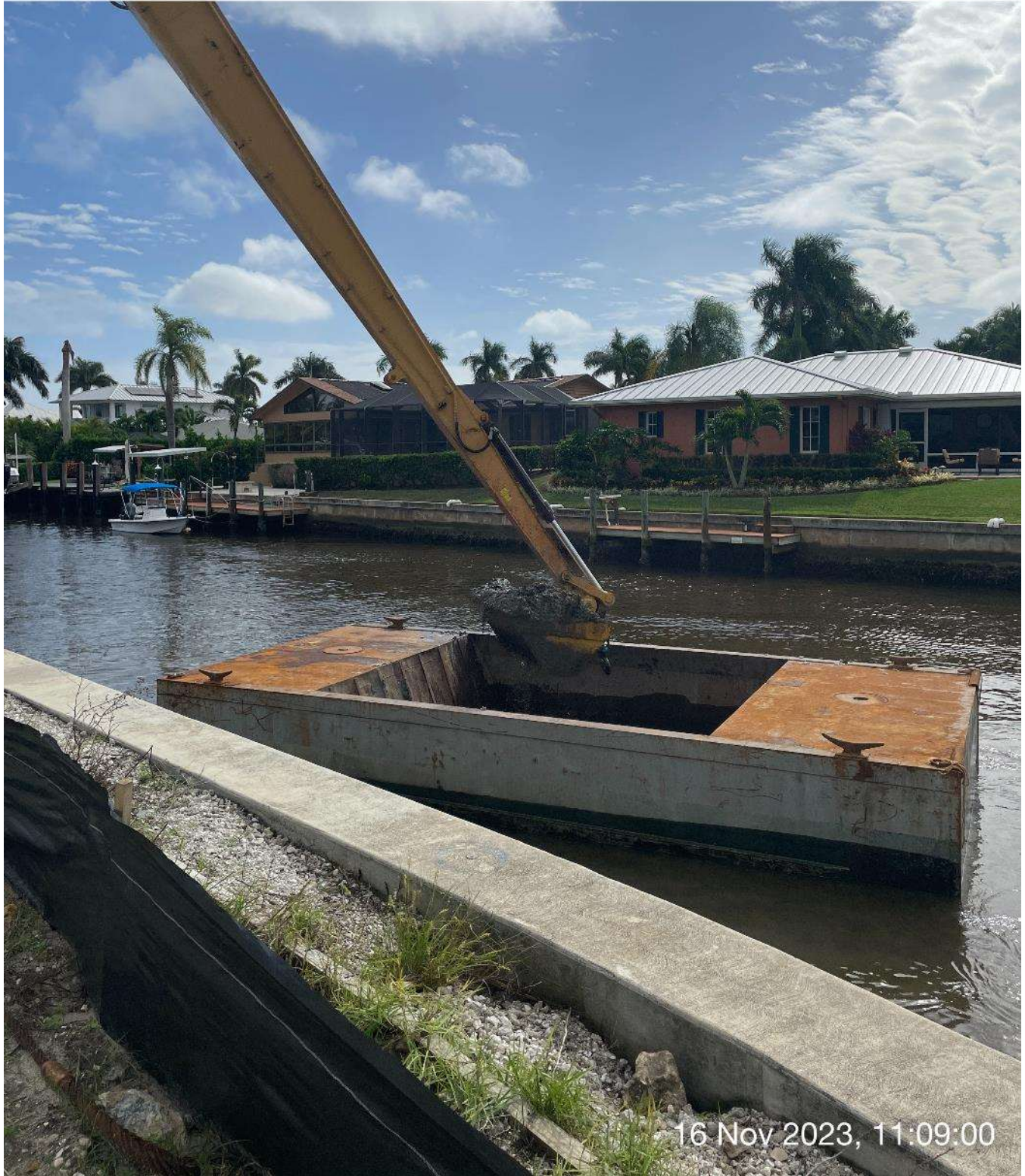
Long reach excavator removing sediment from hopper.
