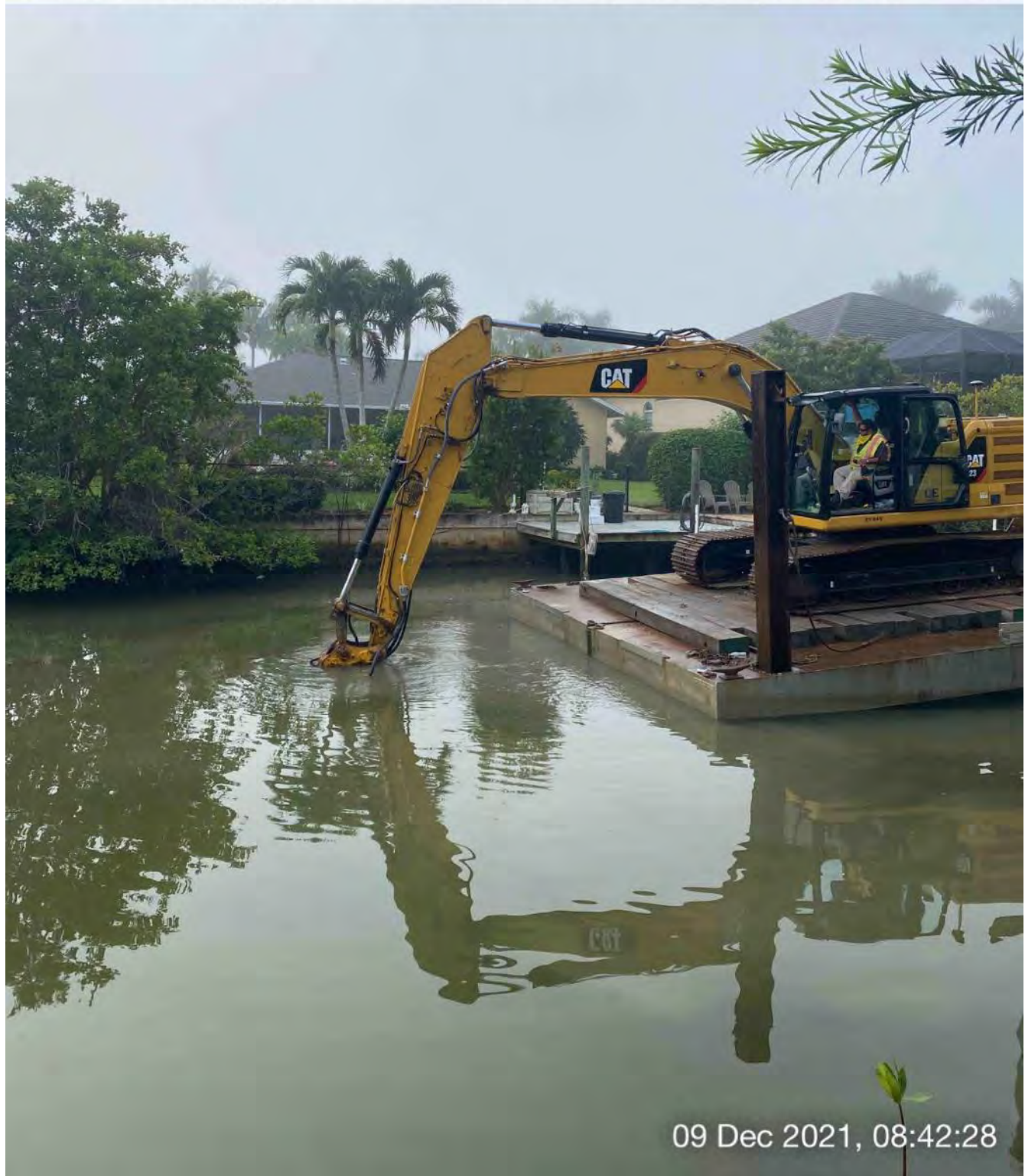
323 excavator grinding rock at station 8+50
