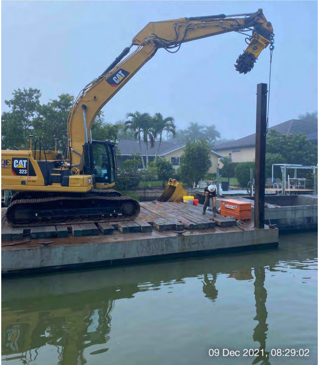
323 excavator lifting spud to allow push boat to move barge from station 8+50 to 8+00
