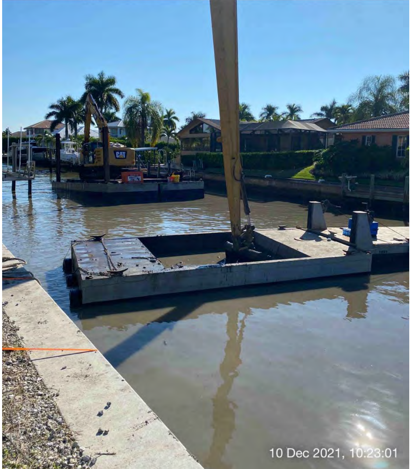
Hopper of material at station 1+50
