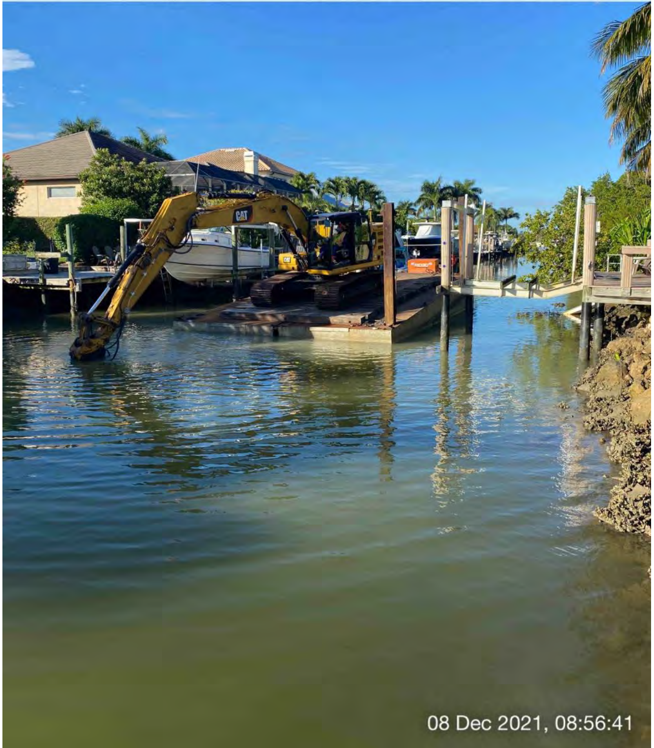
323 excavator grinding rock at station 8+50
