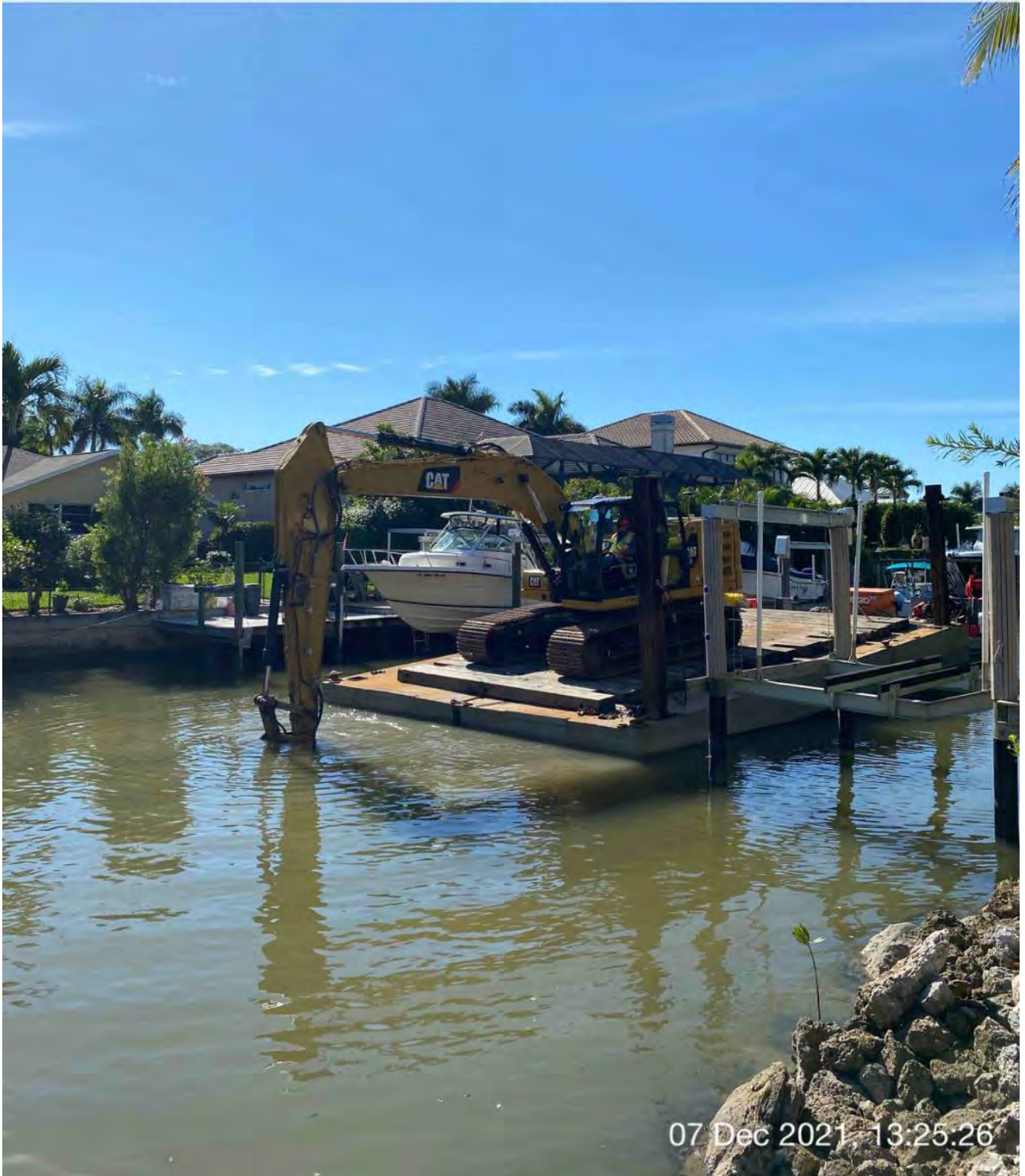
323 excavator grinding rock at station 8+50
