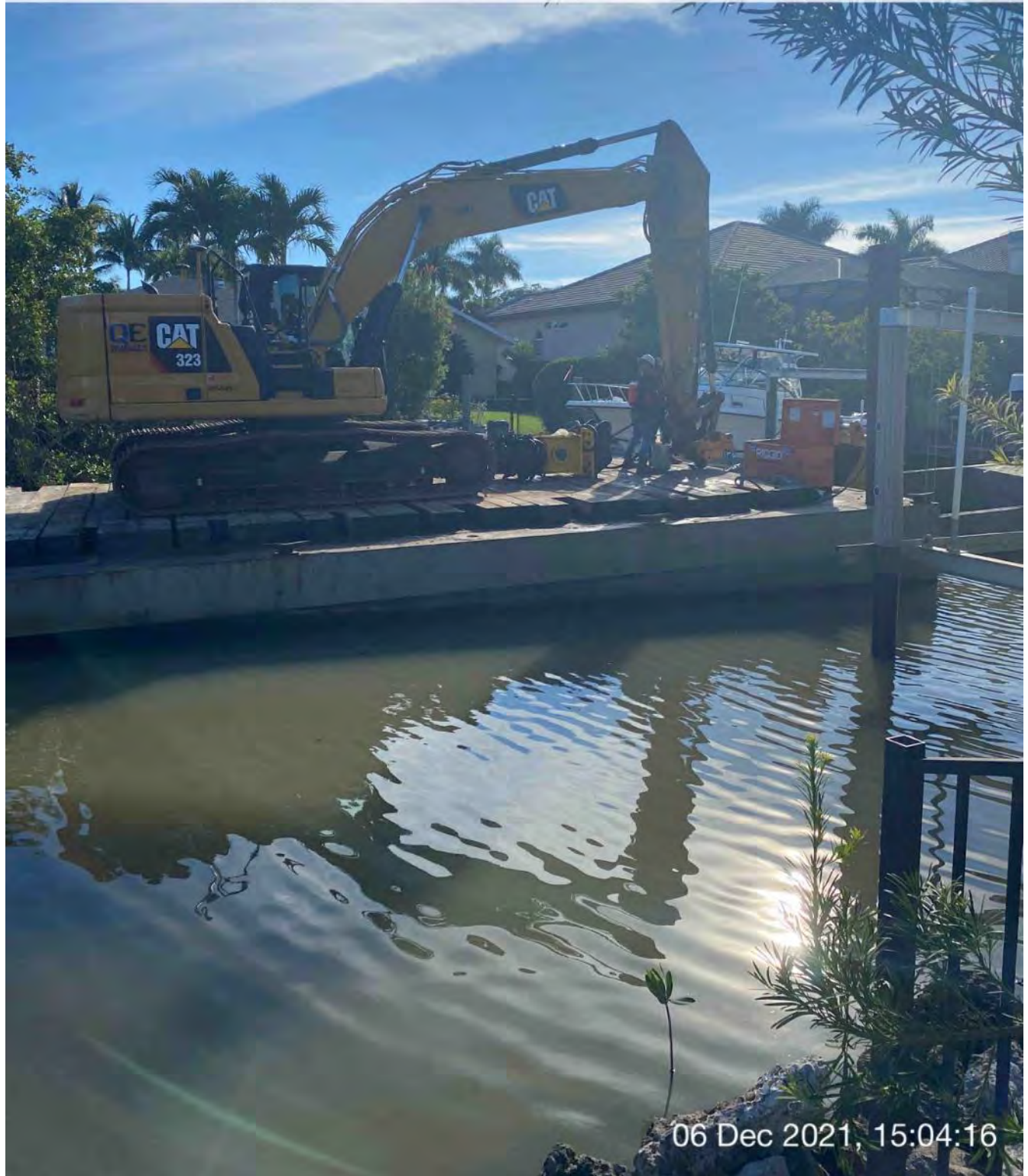
Removing Epiroc grinder attachment
