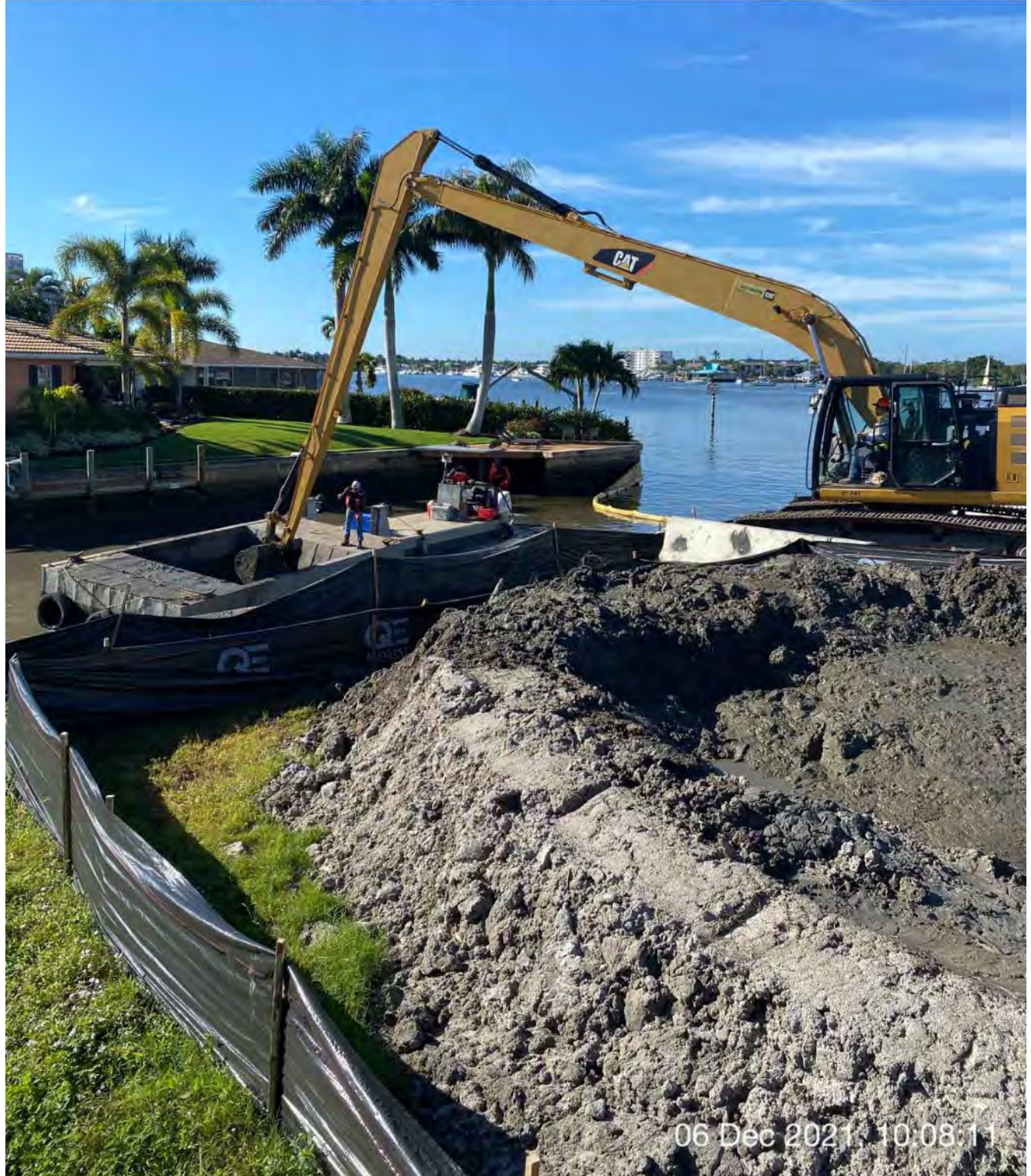
326 excavator transferring material from hopper to dewatering site
