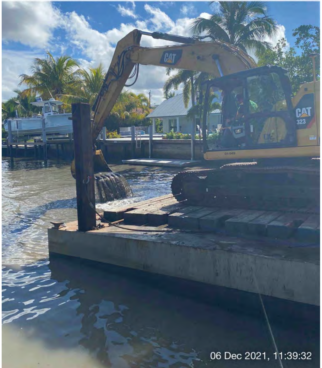
323 excavator removing material from station 9+50
