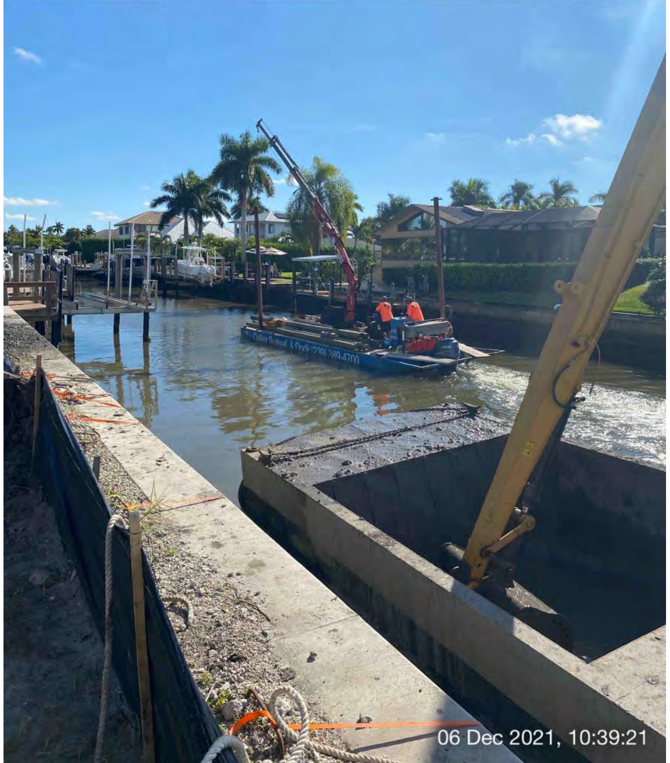
Collier Seawall and dock entering Canal CC-CC
