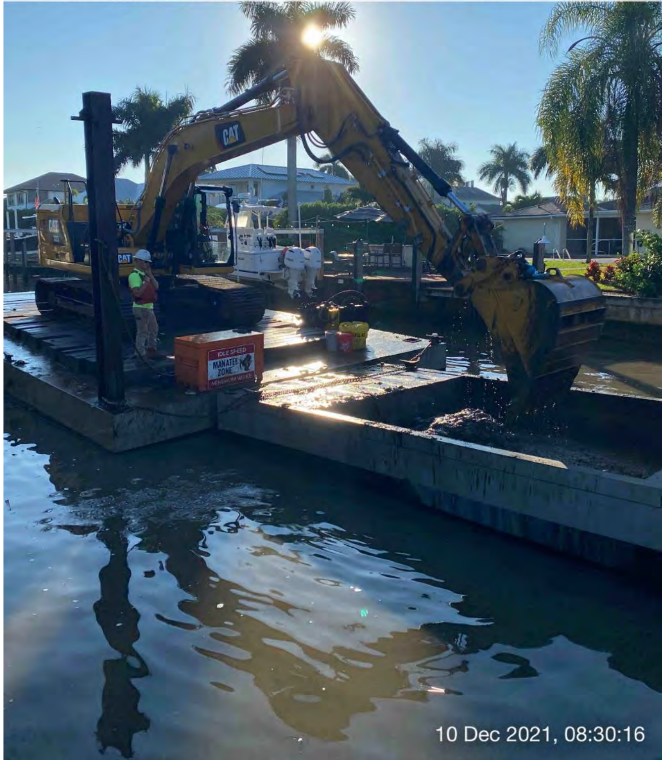
323 excavator removing material from station 4+00 and transferring it to hopper
