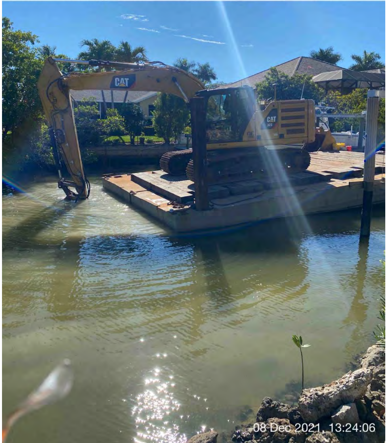
323 excavator grinding rock at station 9+00
