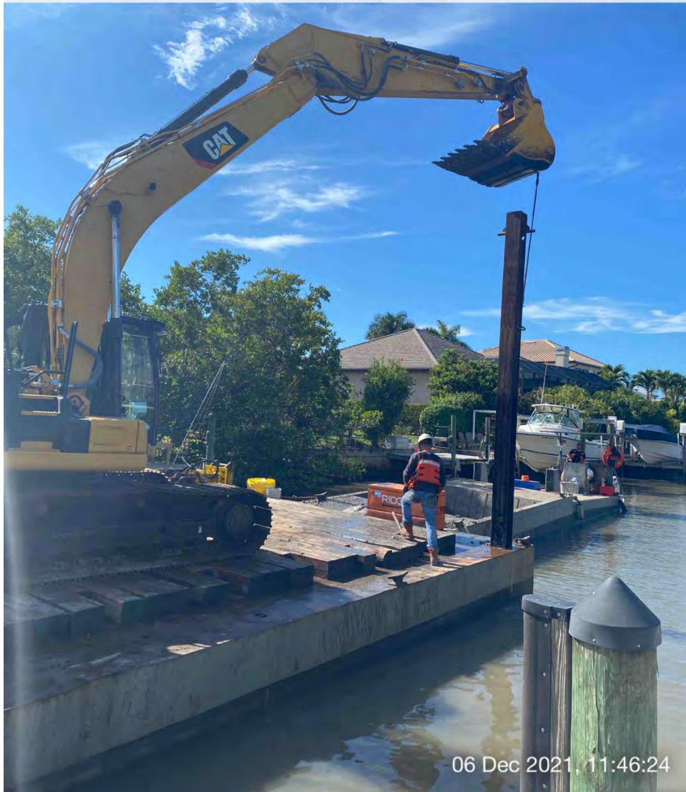
323 excavator lifting spud to allow push boat to move the barge
