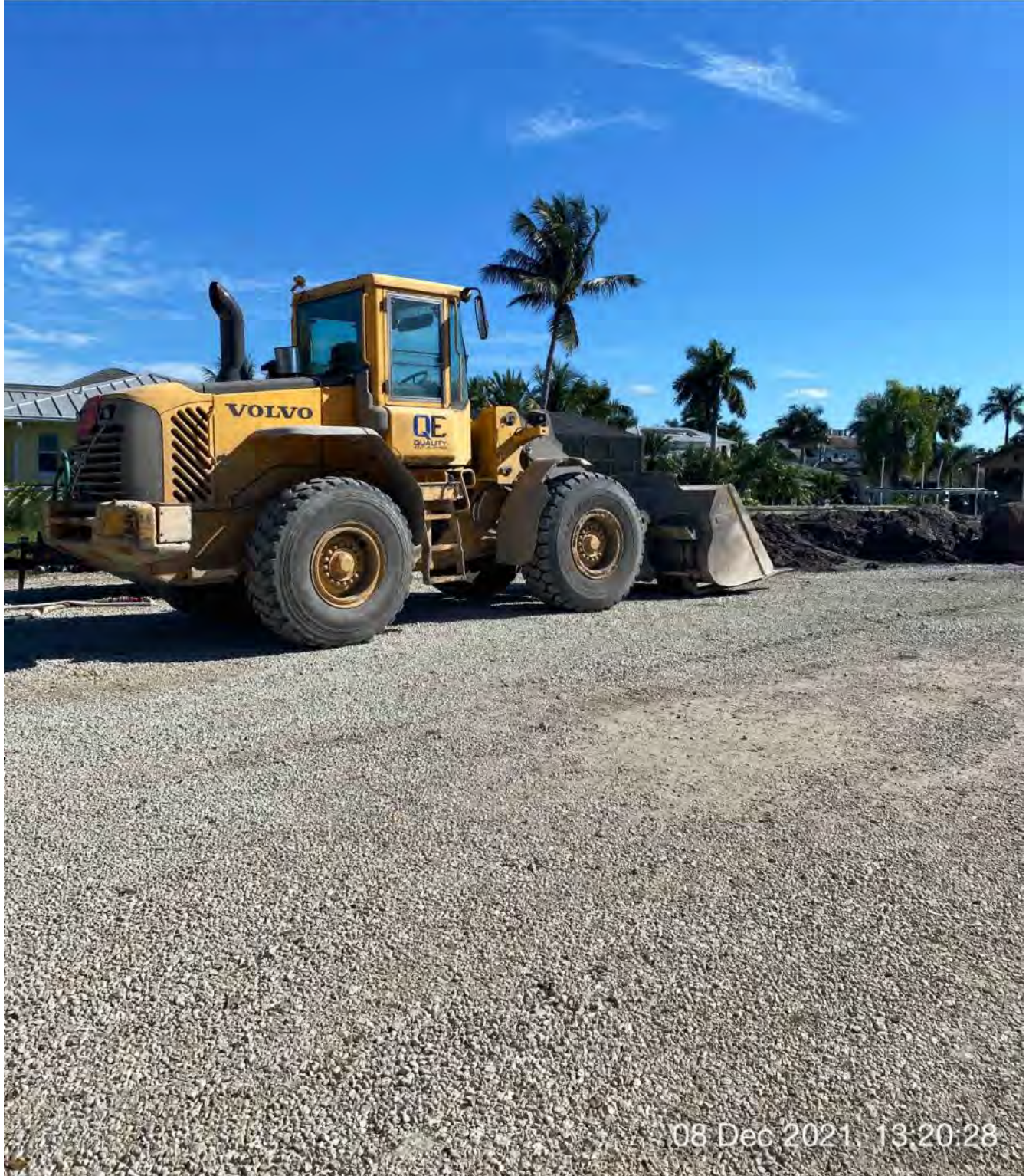
Front end loader at 1300 Curlew Avenue
