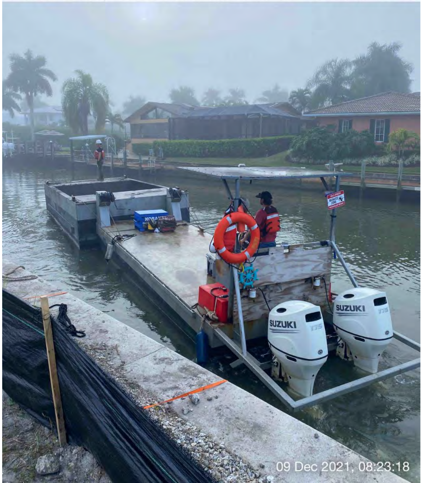
Push boat transporting hopper from station 1+50 to station 8+50
