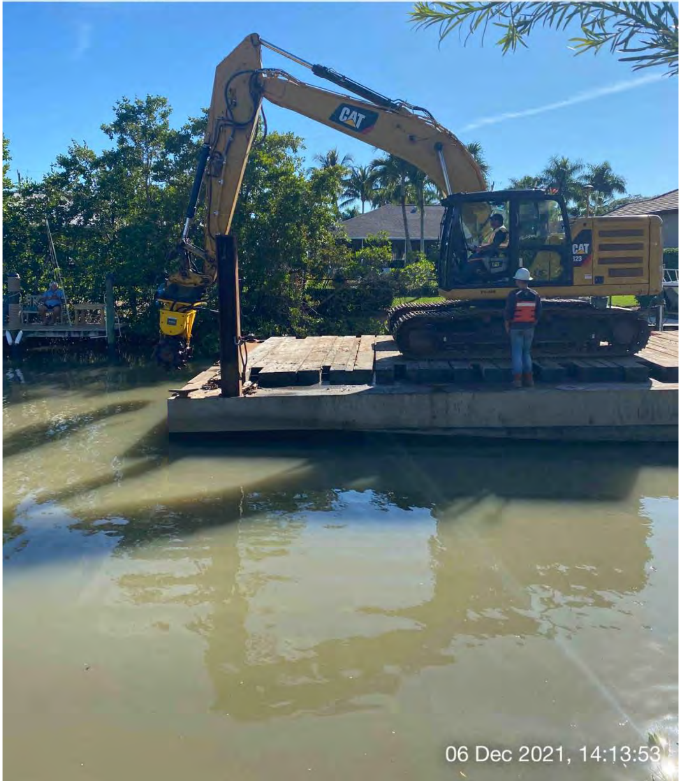
323 excavator with Epiroc grinder attachment
