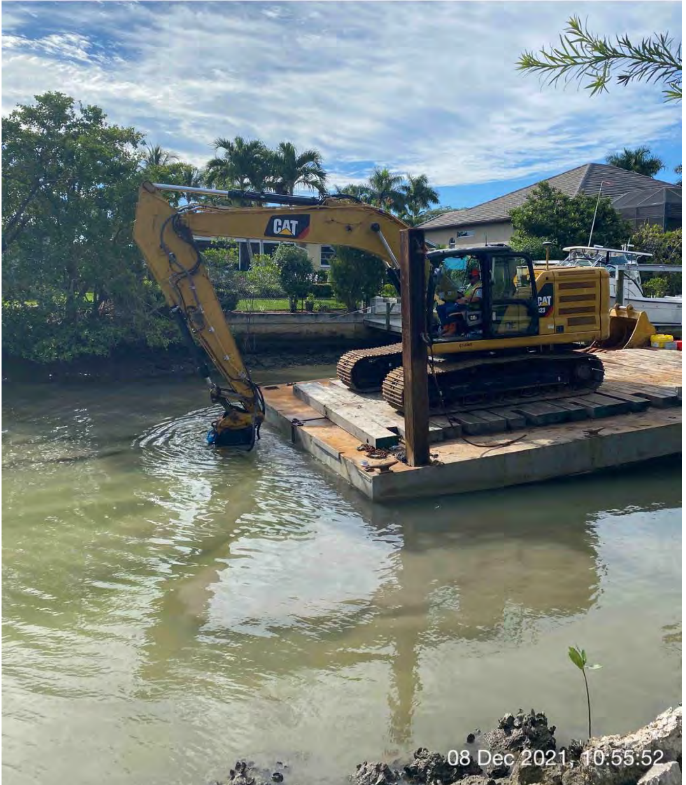
323 excavator grinding rock at station 8+50
