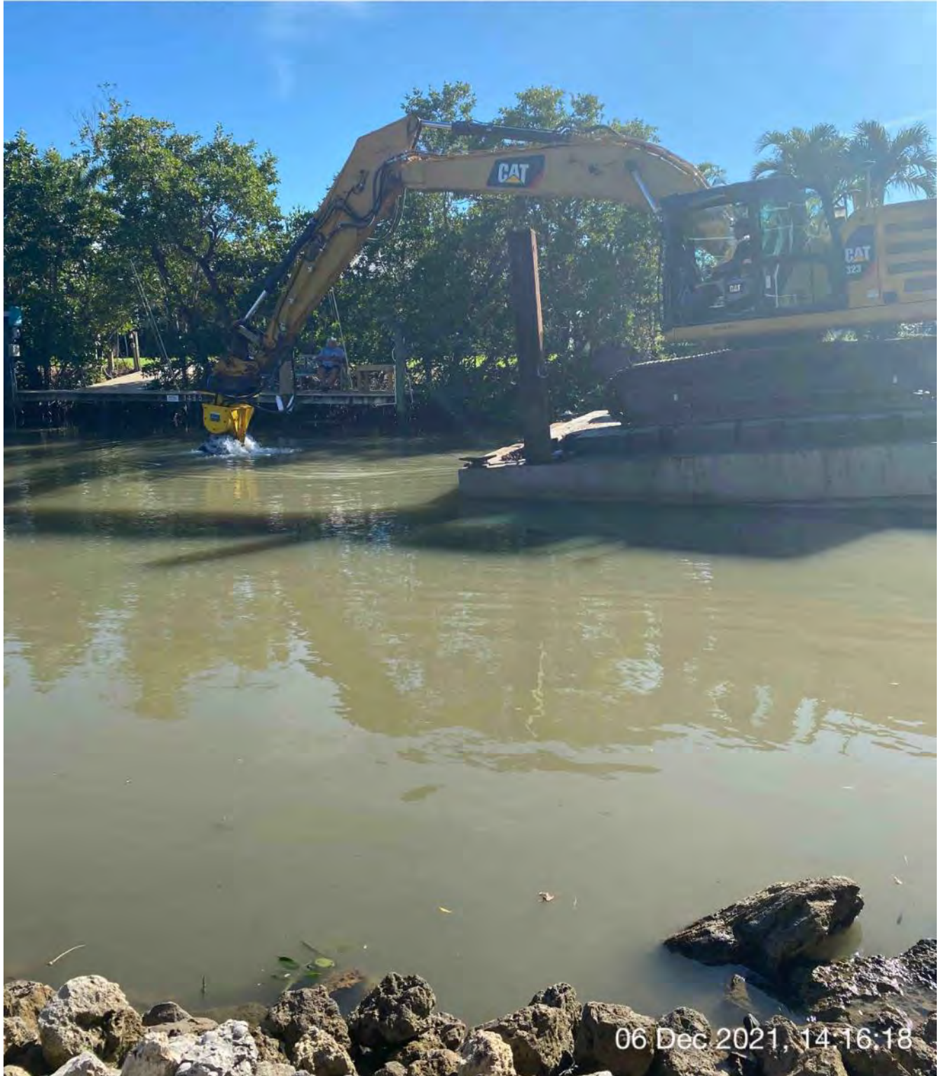
323 excavator with Epiroc grinder attachment grinding rock at station 9+00
