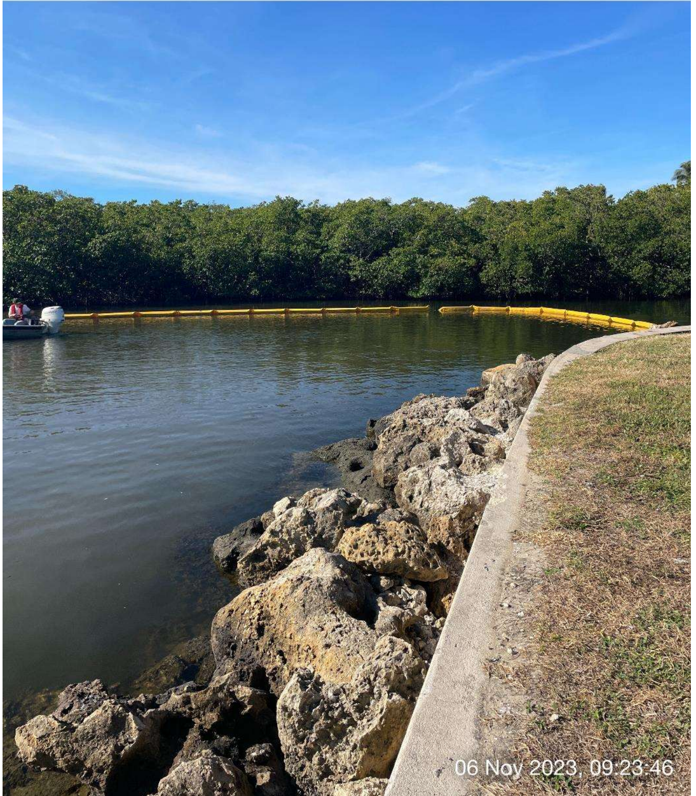
Turbidity curtain in place at station 2+00 in Canal Main B1.
