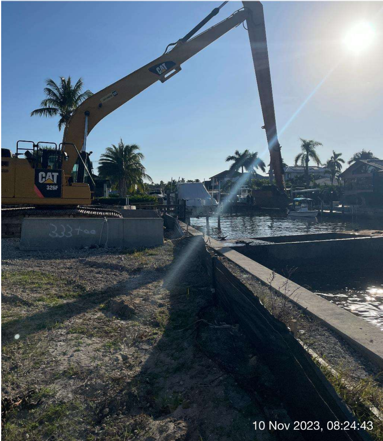
Long reach excavator removing sediment from hopper.
