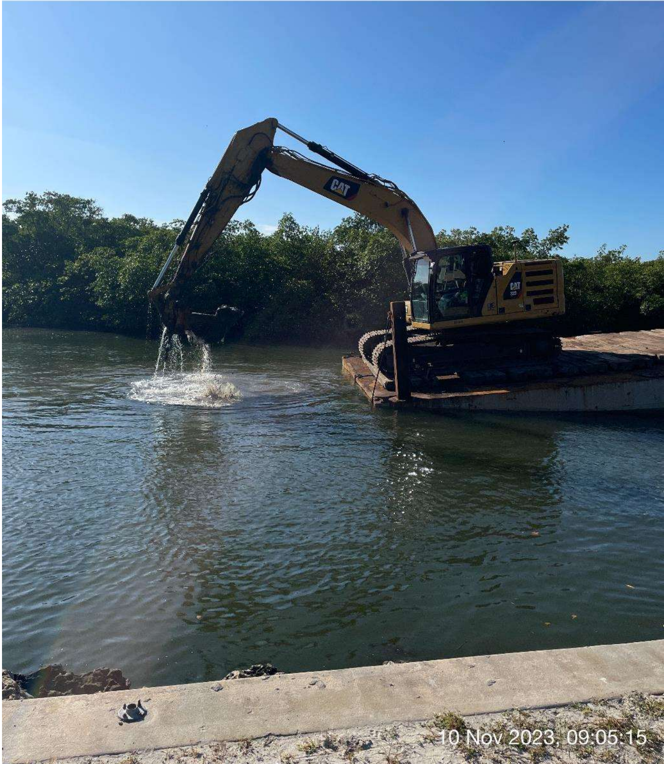
323 excavator removing sediment from station 3+00 in Canal Main B1.
