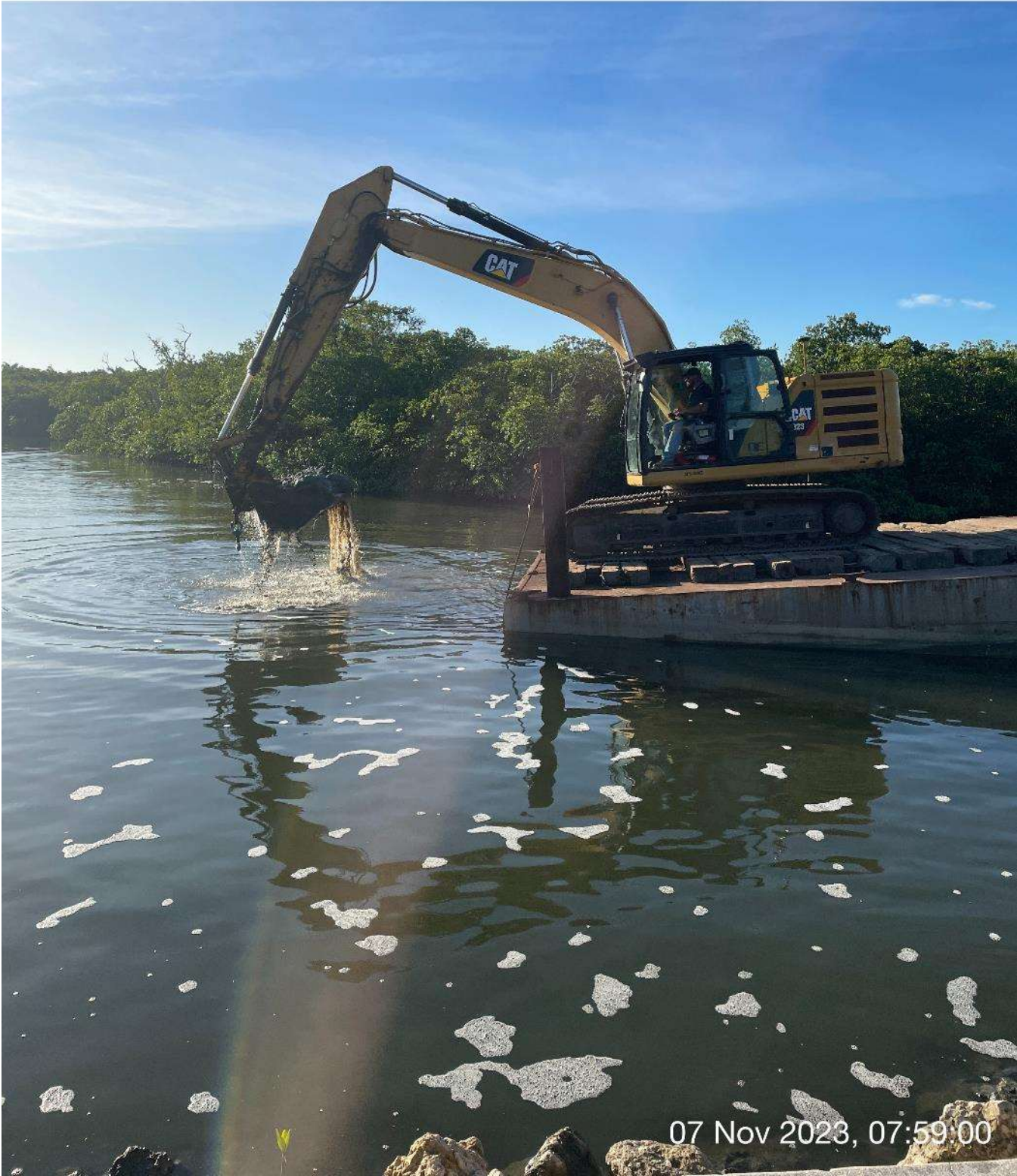
323 excavator removing sediment at station 3+50 in Canal Main B1.
