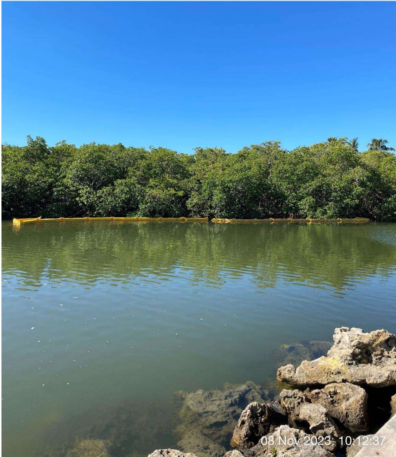
Turbidity curtain open in Canal Main B1.
