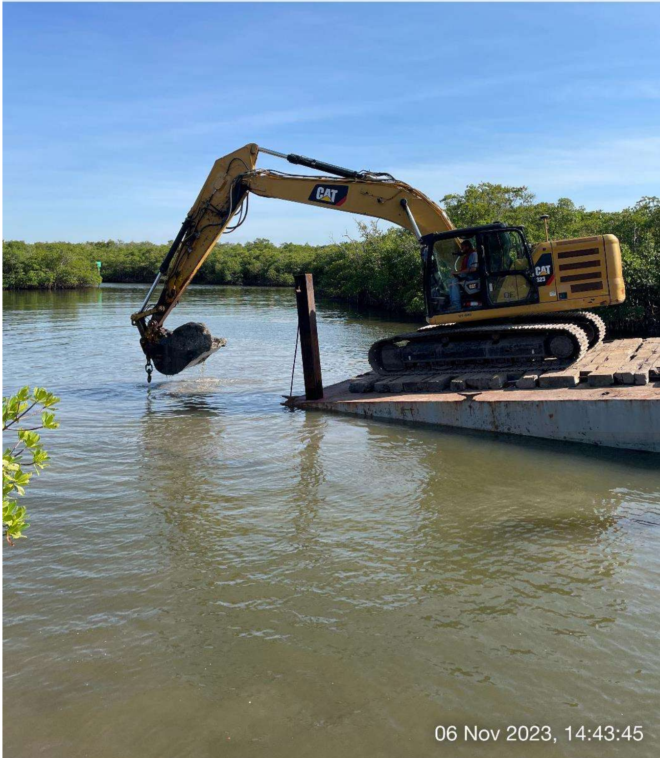
323 excavator removing sediment at station 3+75 in Canal Main B1.
