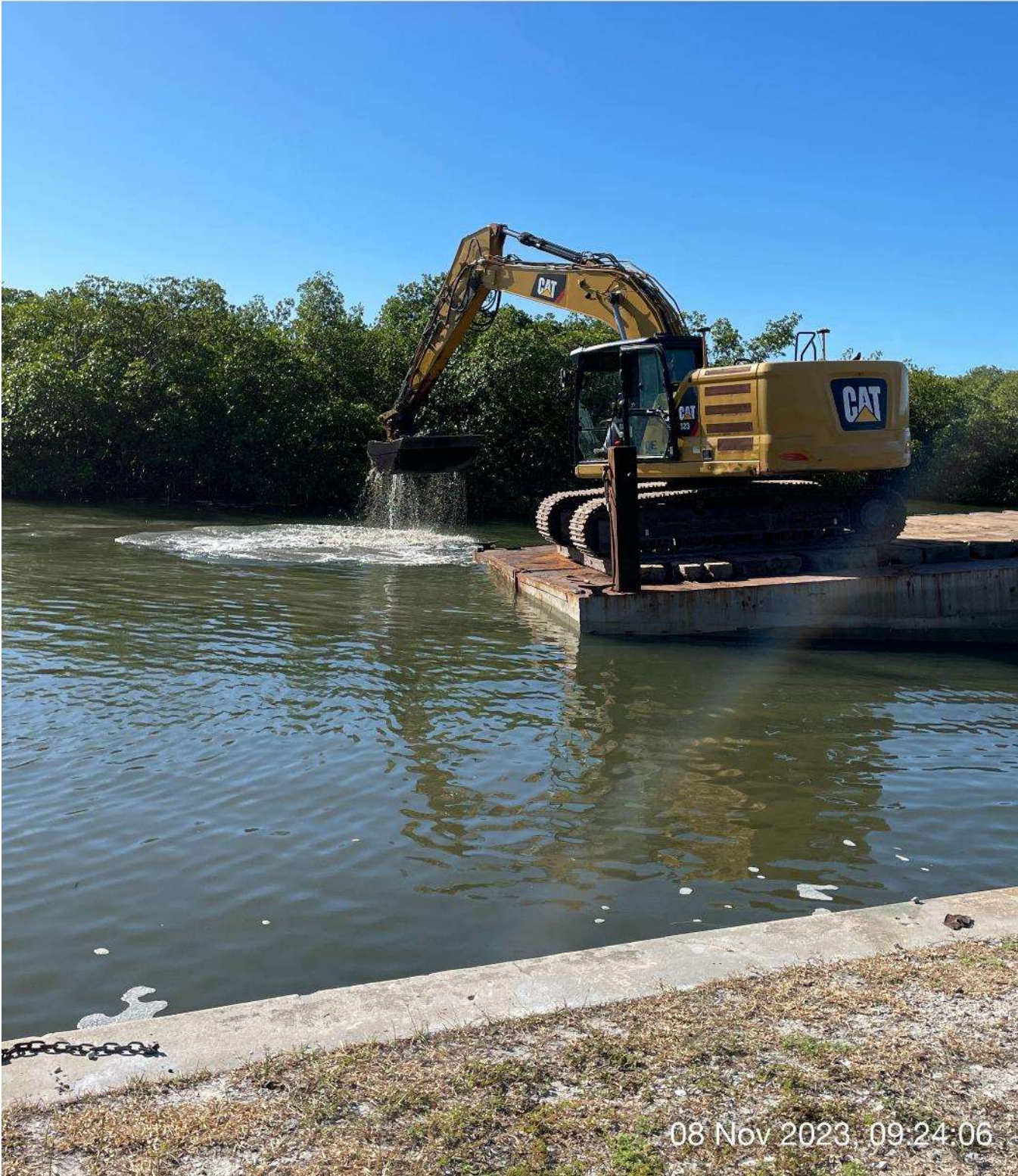
323 excavator removing sediment at station 3+00 in Canal Main B1.
