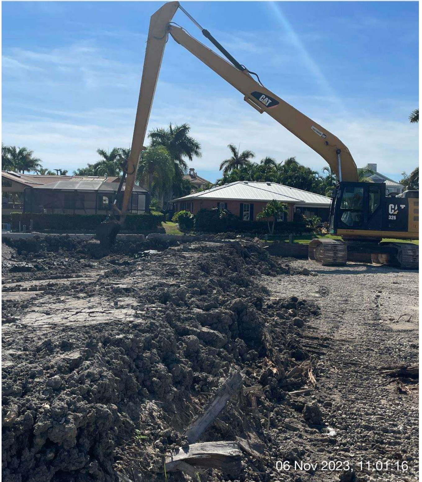
Long reach excavator spreading sediment on staging area.
