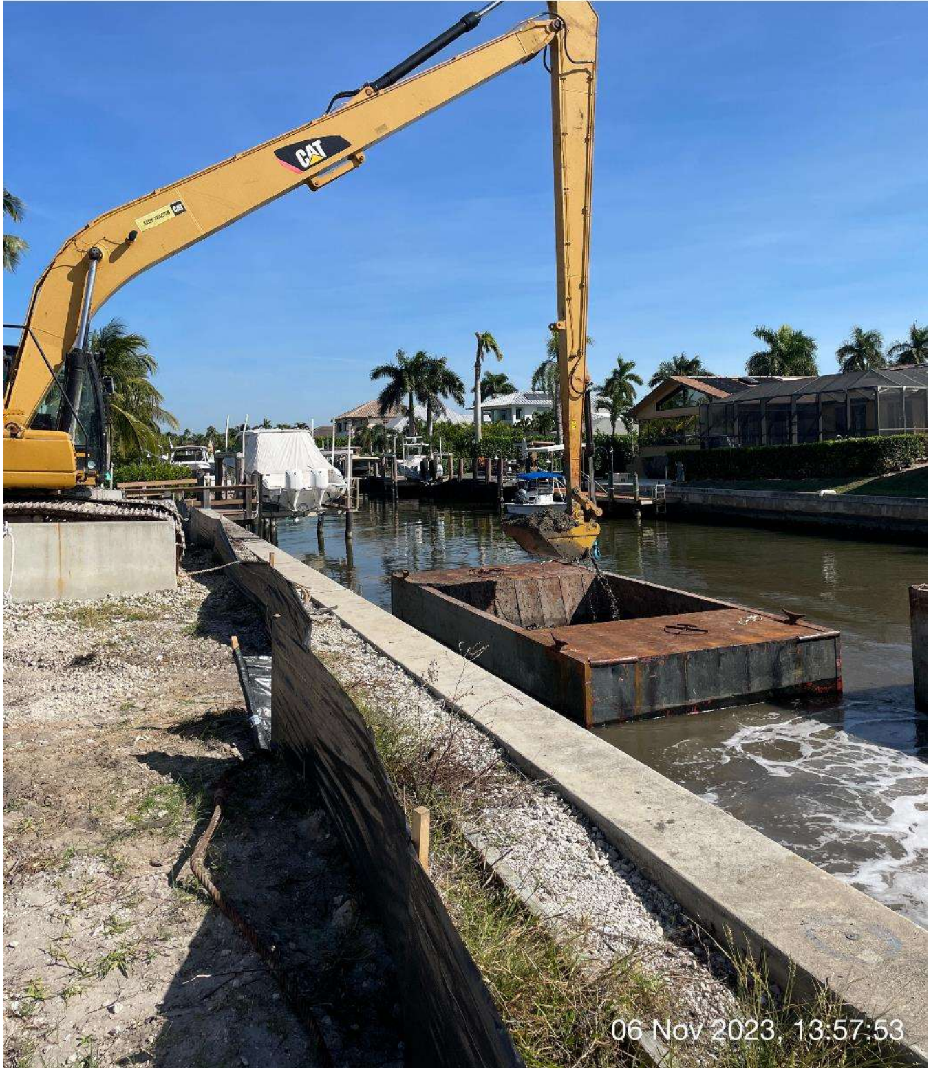
Long reach excavator removing sediment from hopper.
