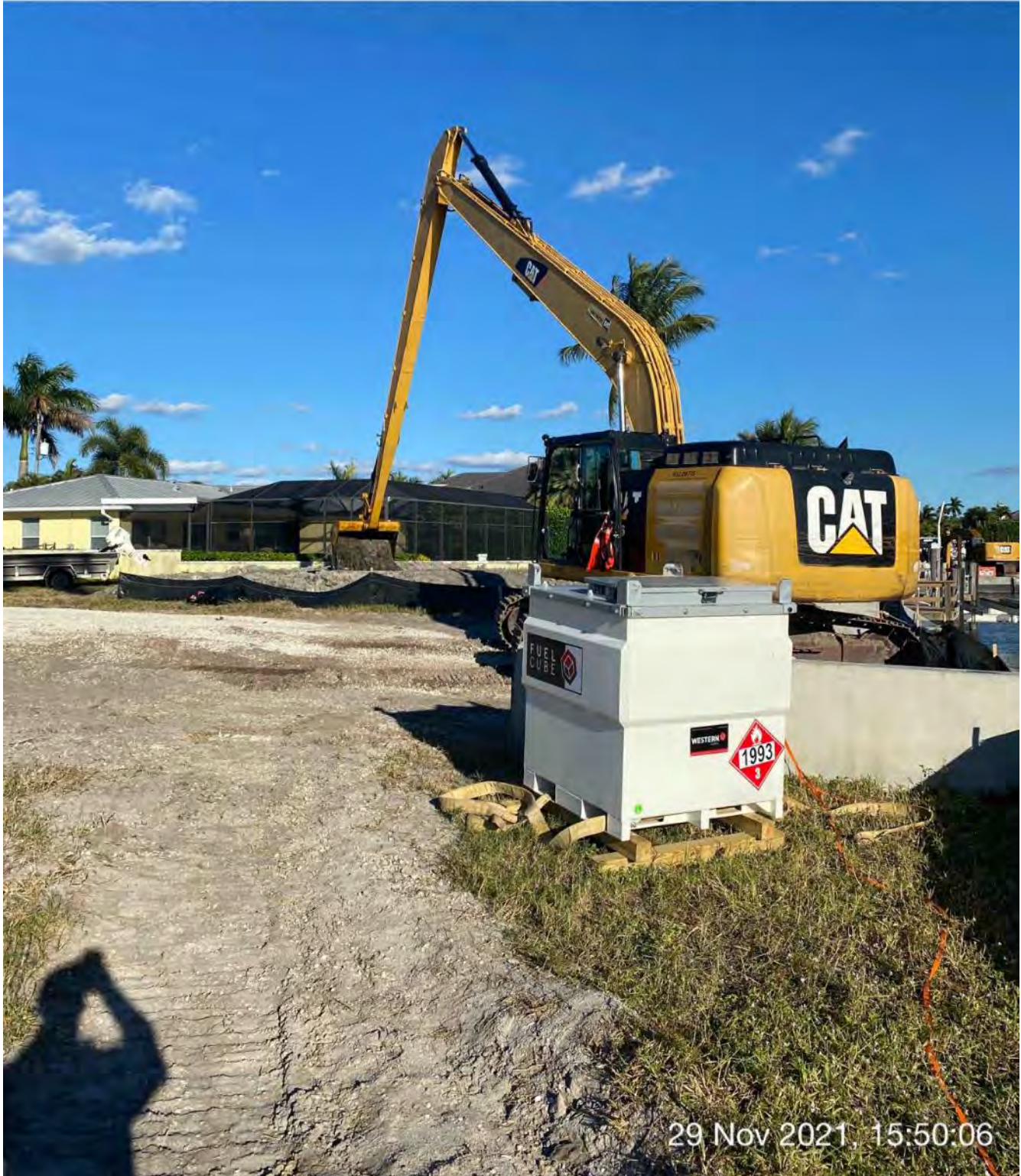
326 excavator transferring sediment from station 2+00 to dewatering site at 1300 Curlew Avenue
