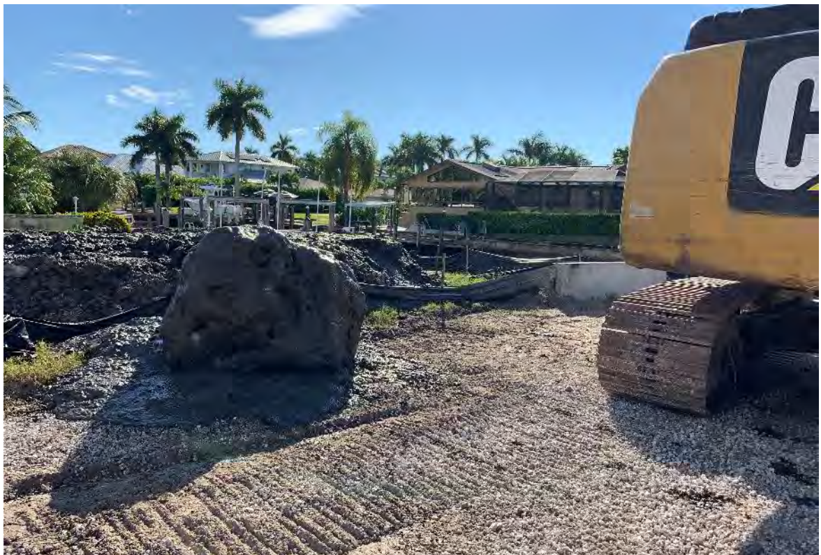
Large rock removed from Canal CC-CC
