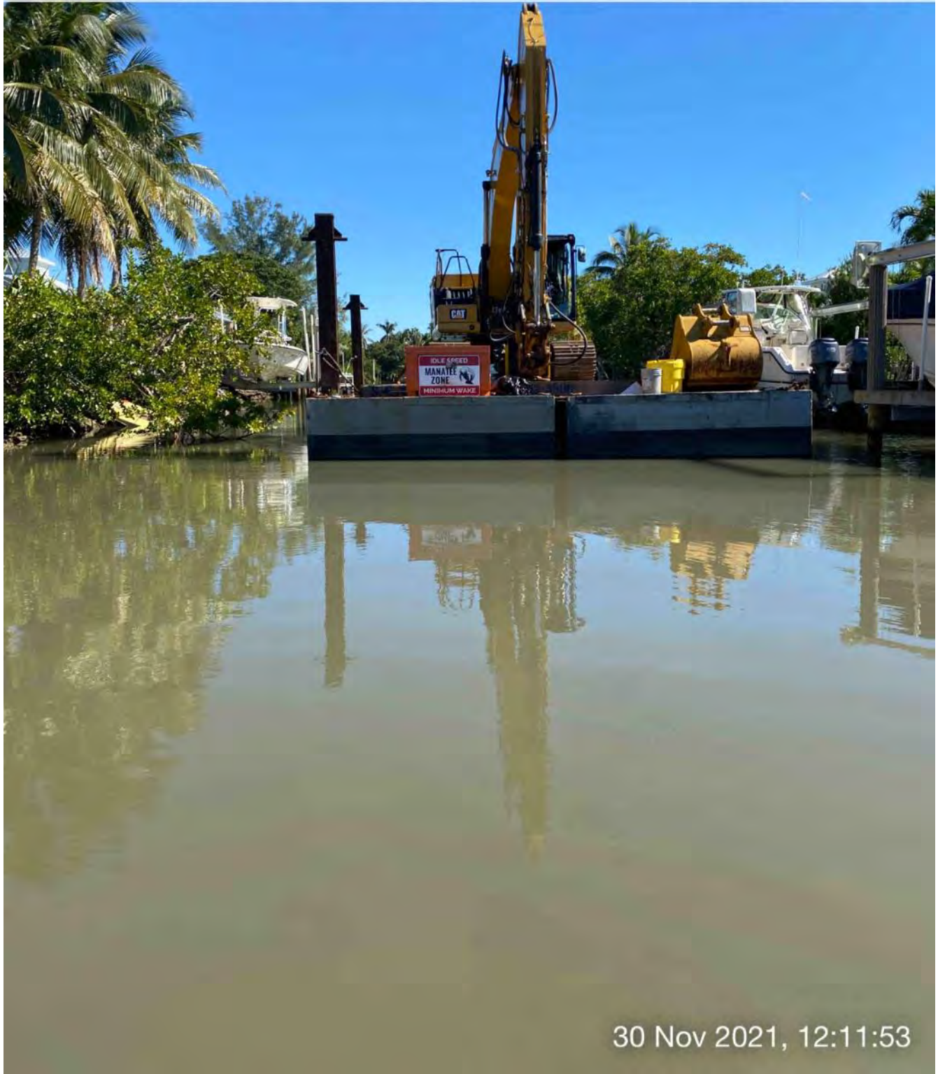
323 excavator sitting on barge at station 7+50
