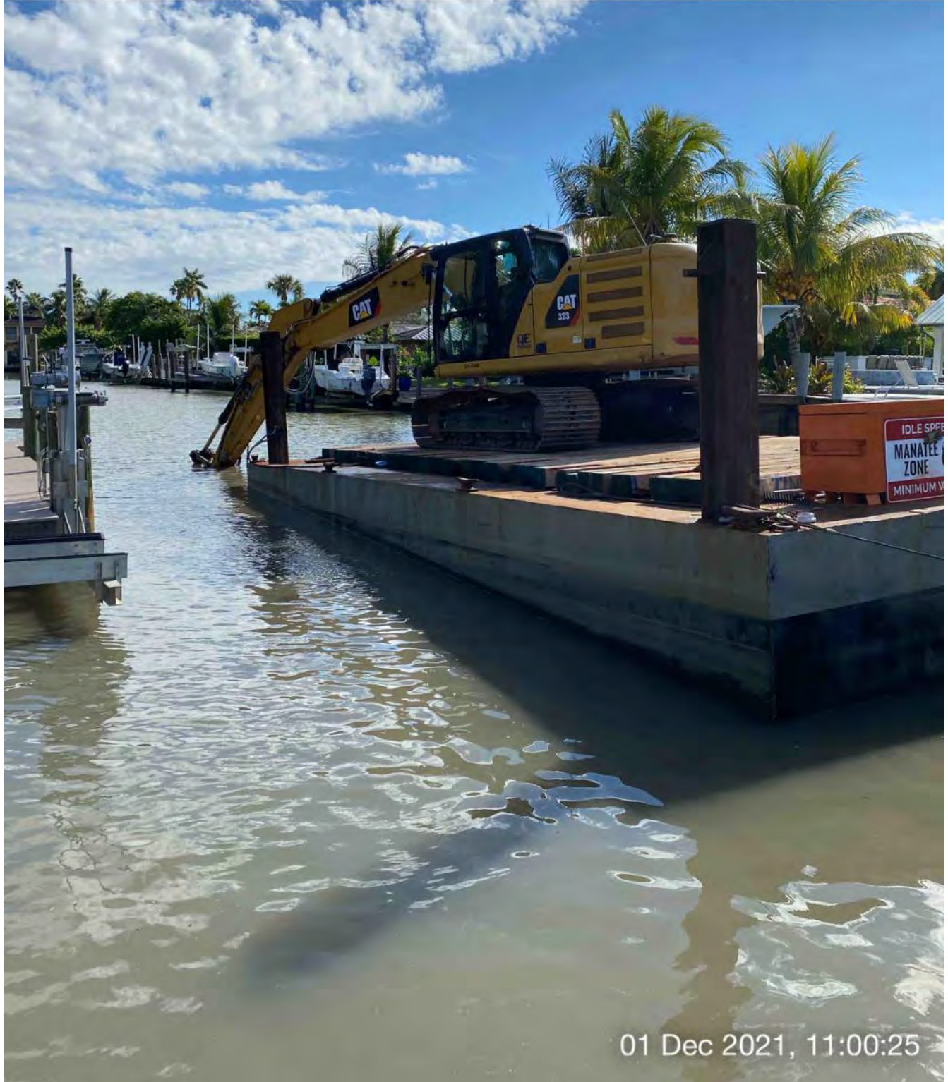
323 excavator grinding rock at station 9+50
