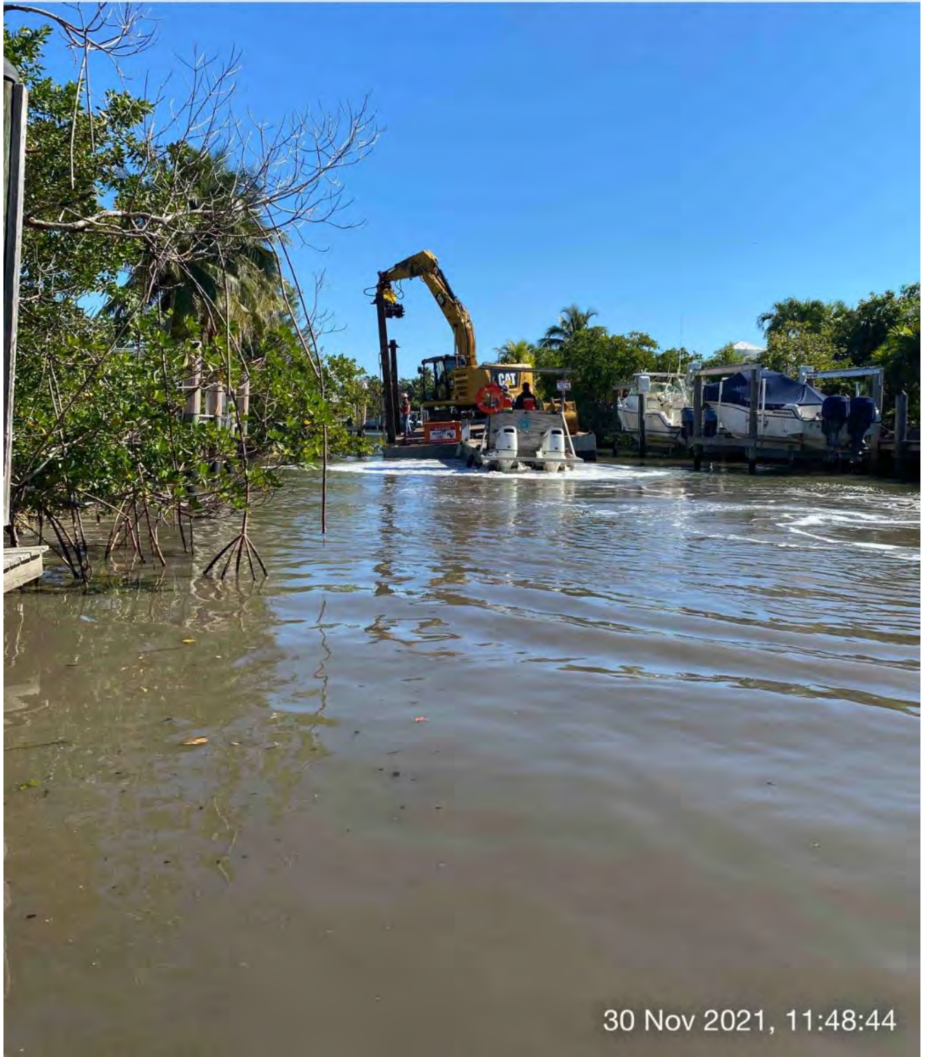
323 excavator lifting spud to allow push boat to position barge for grinding at station 7+00
