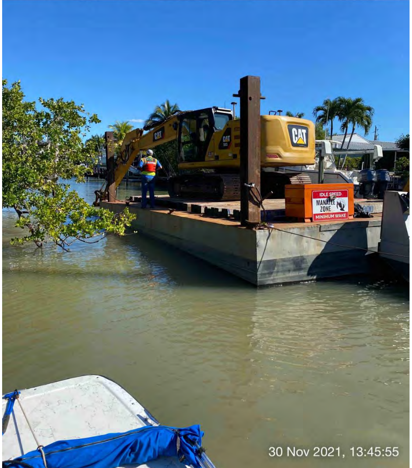
323 excavator grinding rock at station 8+00
