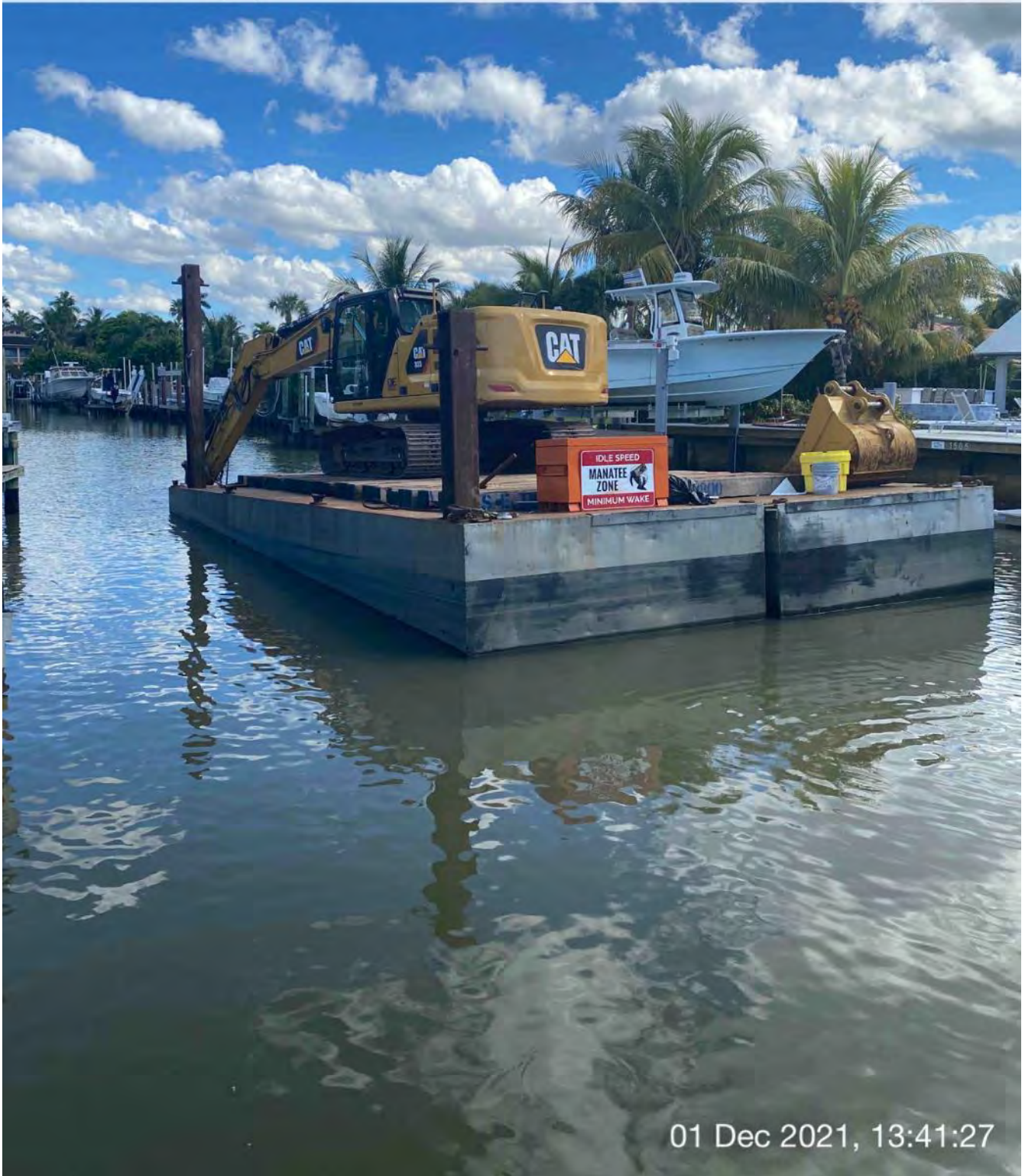
323 excavator grinding rock at station 9+50
