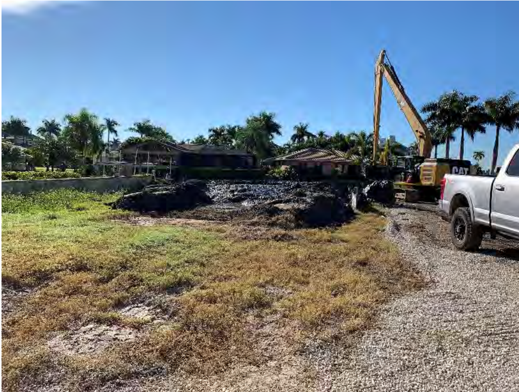
Staging area with removed material drying.
