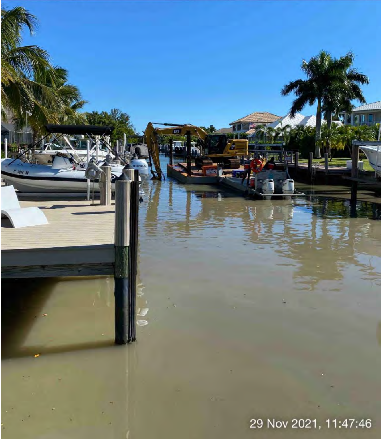
323 excavator grinding rock at station 4+00
