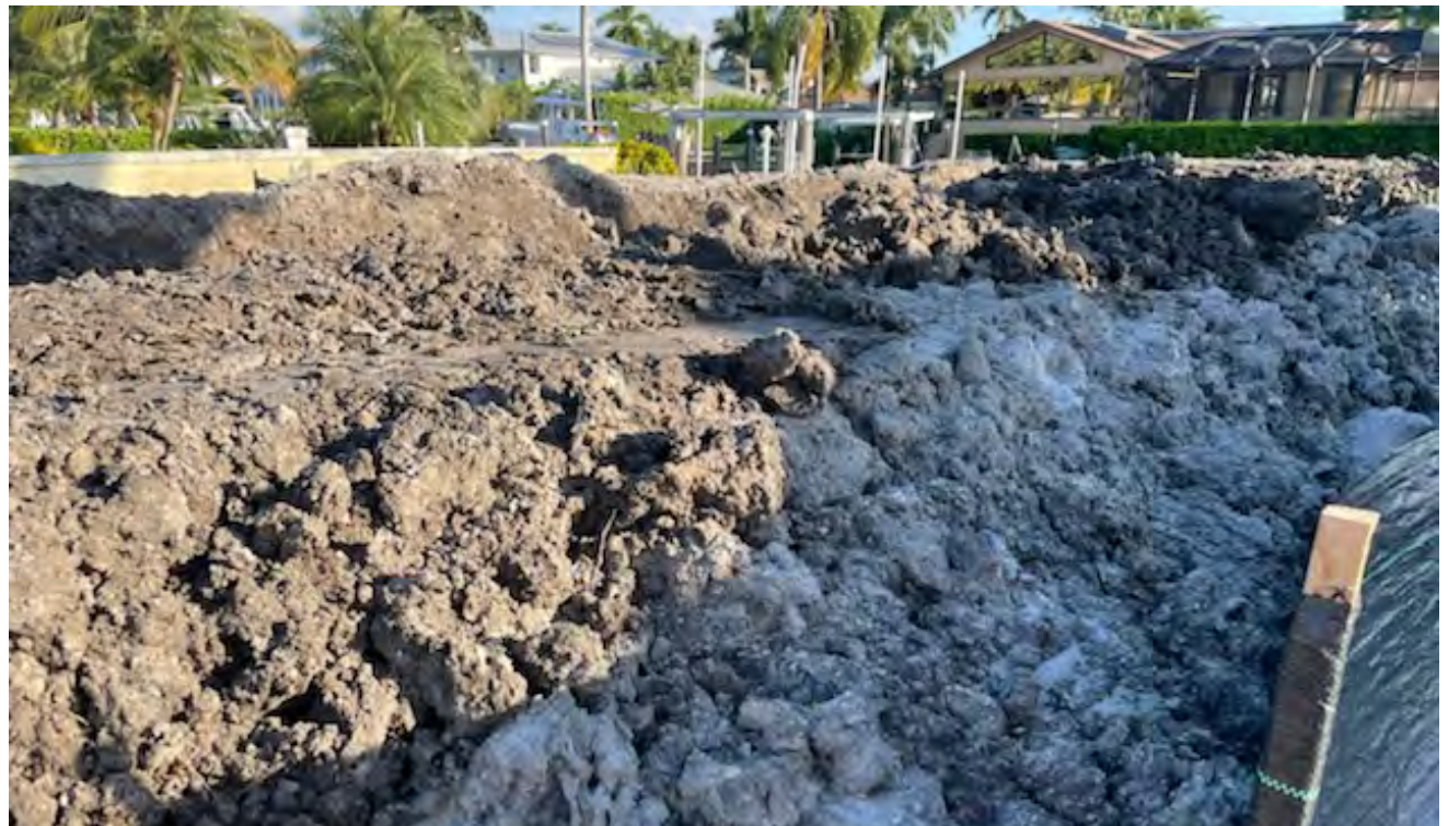
Material from canal drying at dewatering area
