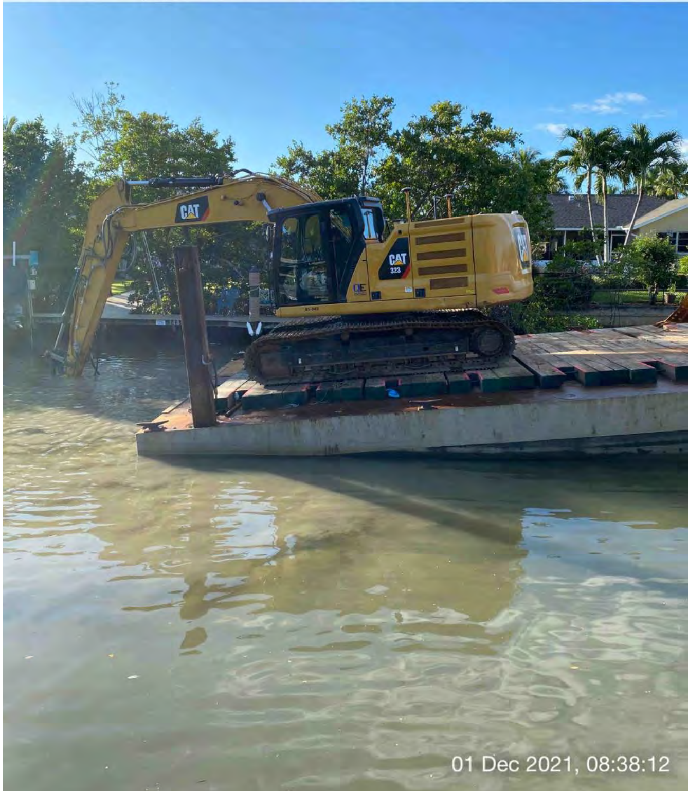
323 excavator grinding rock at station 9+00
