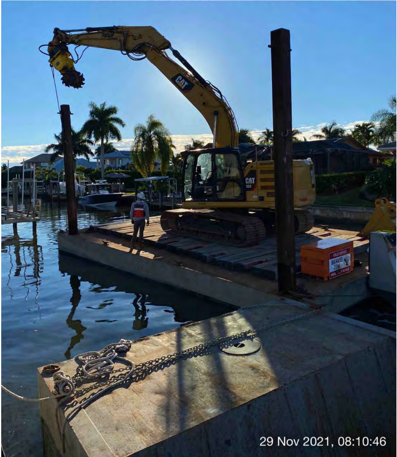
323 excavator lifting spud to allow push boat to position barge for grinding
