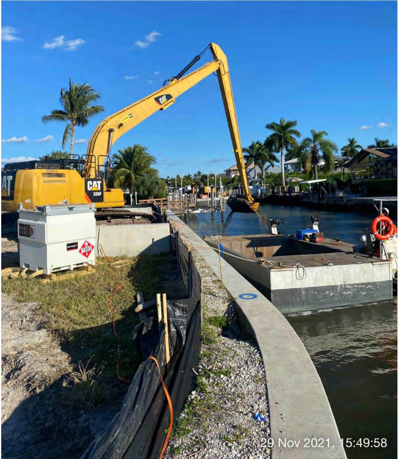
326 excavator removing sediment from station 2+00
