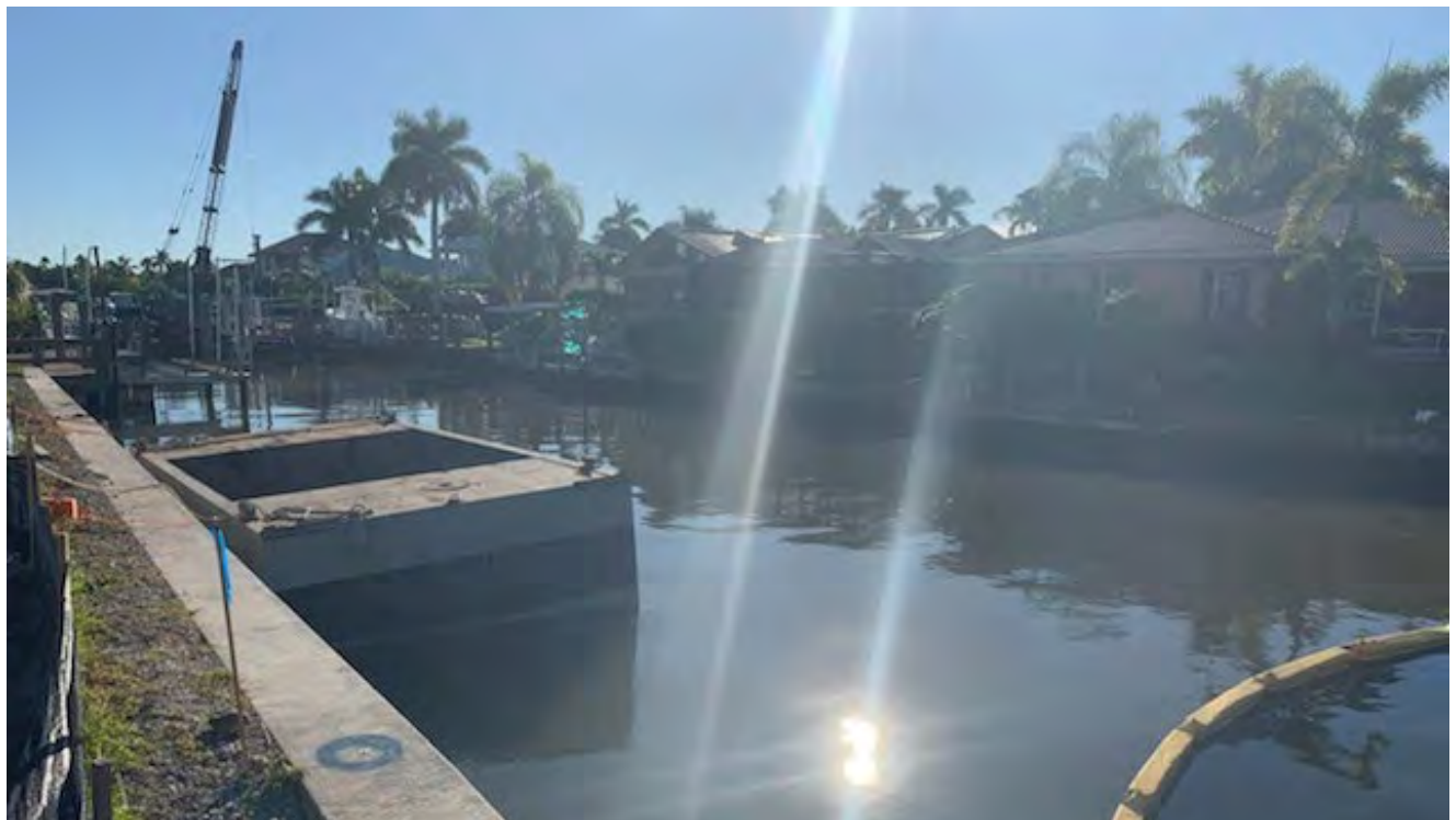
Turbidity curtain across the mouth of Canal CC-CC
