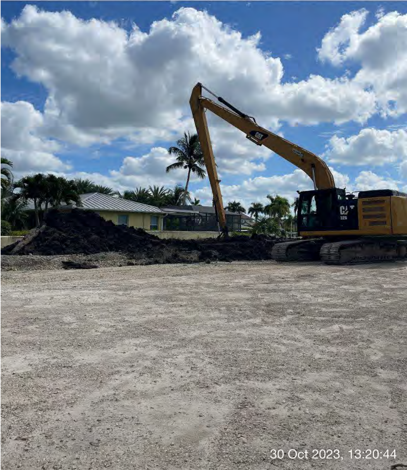
Long reach excavator separating wet and dry material on staging area at 1300 Curlew Avenue.
