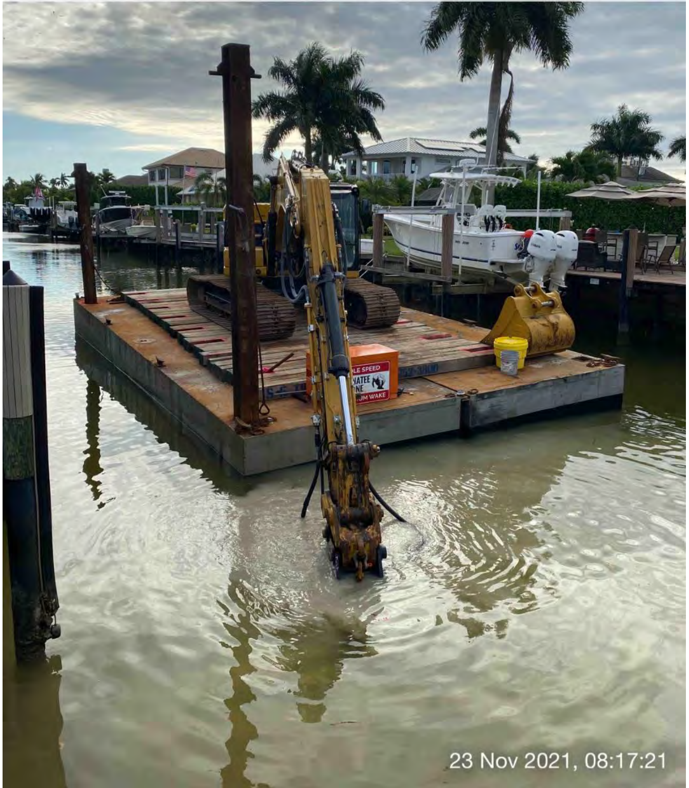
323 excavator grinding rock at station 3+50
