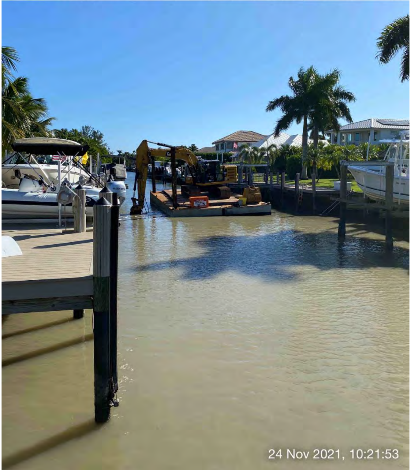
323 excavator grinding rock at station 3+50
