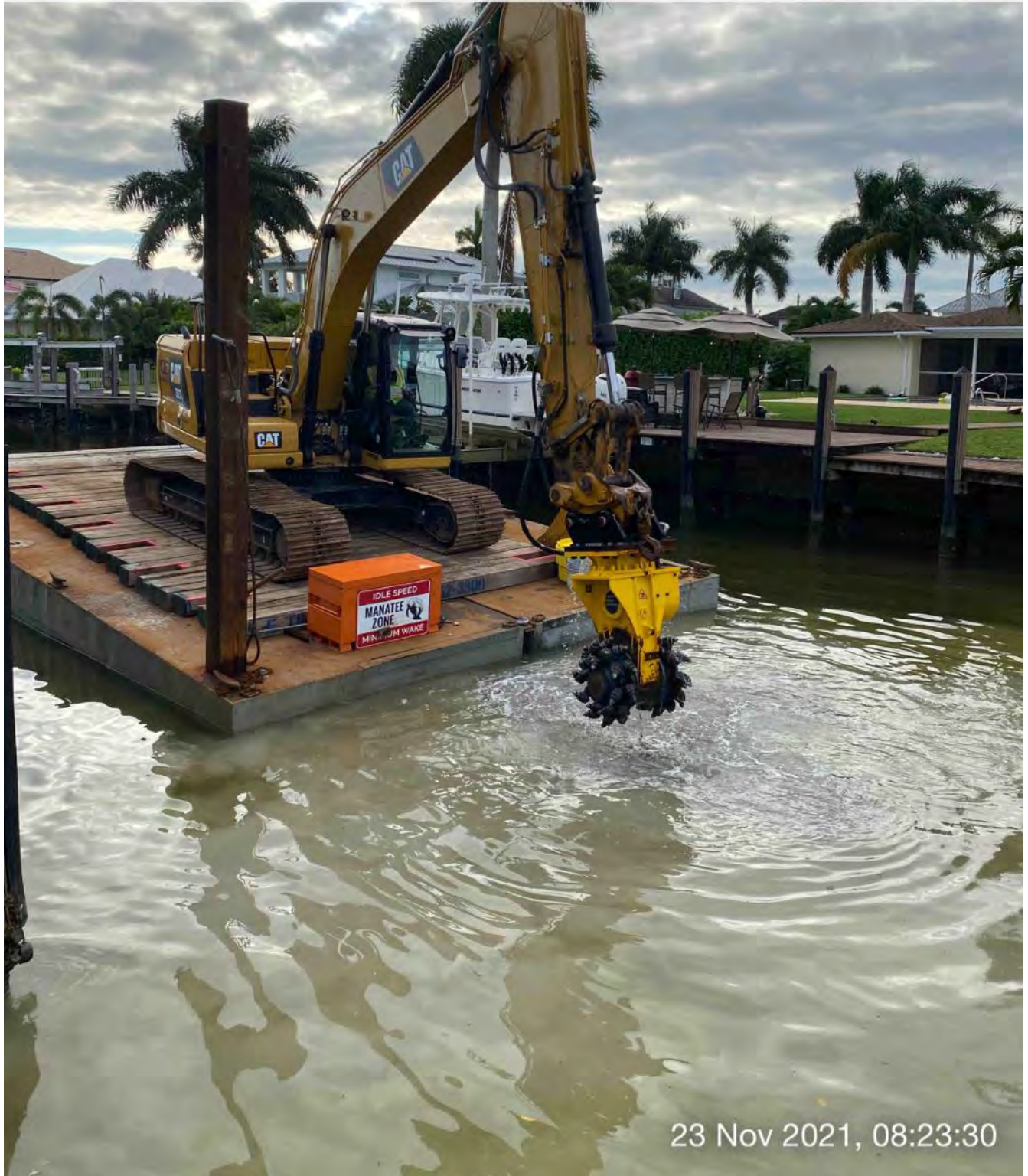
323 excavator grinding rock at station 3+50
