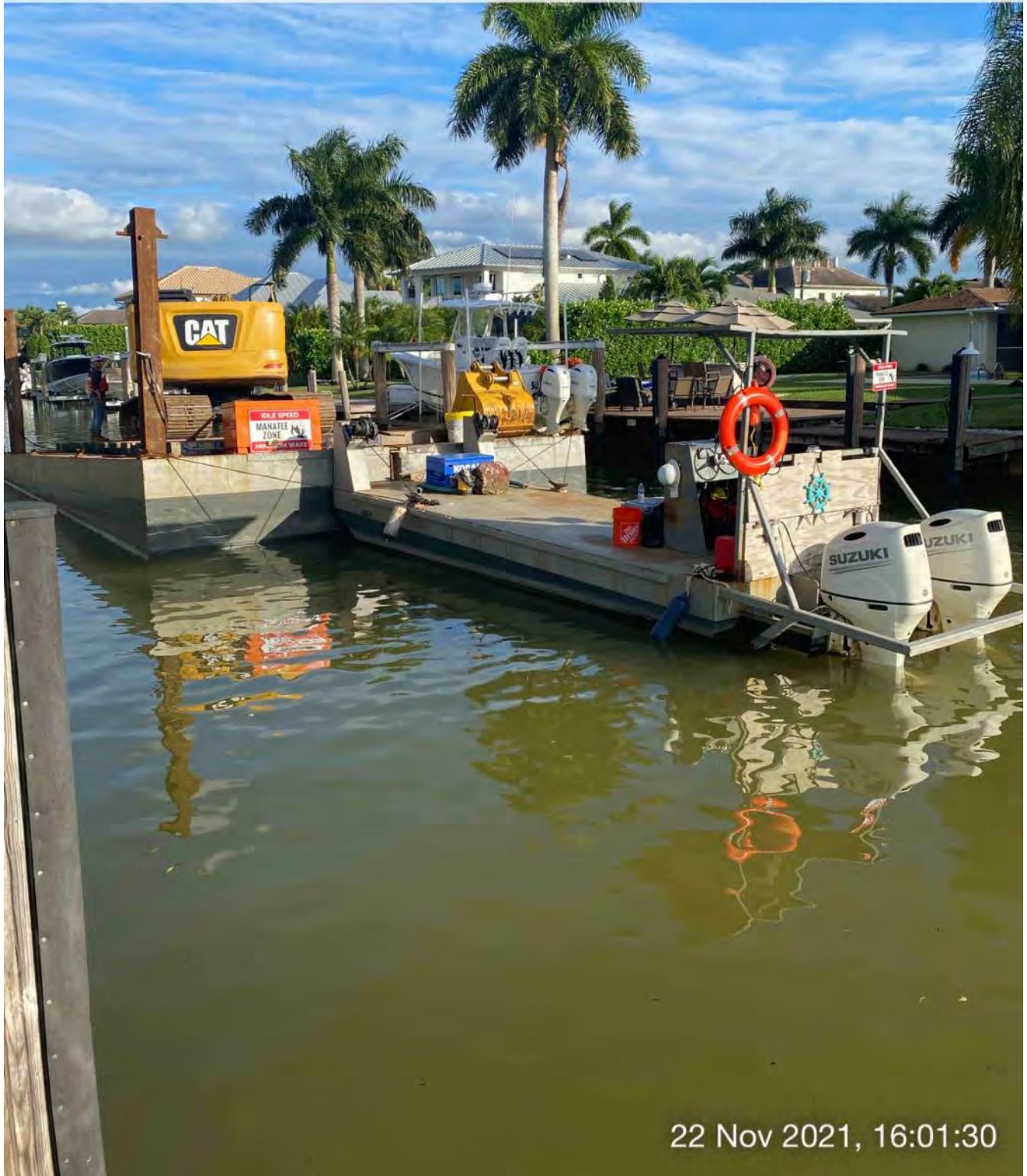
323 excavator grinding rock at station 3+50 with push boat positioning barge
