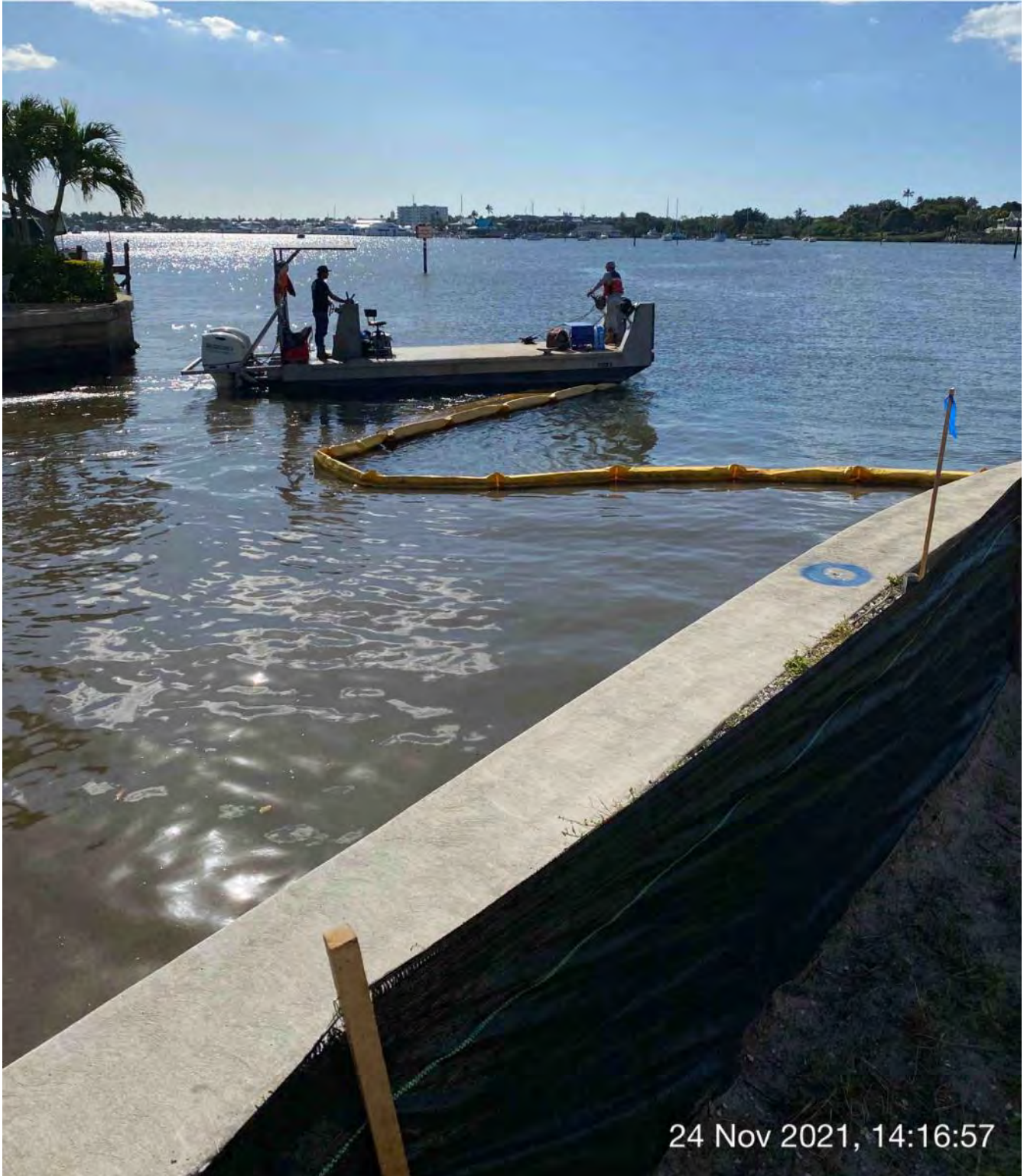
Removing turbidity curtain from across the mouth of Canal CC-CC
