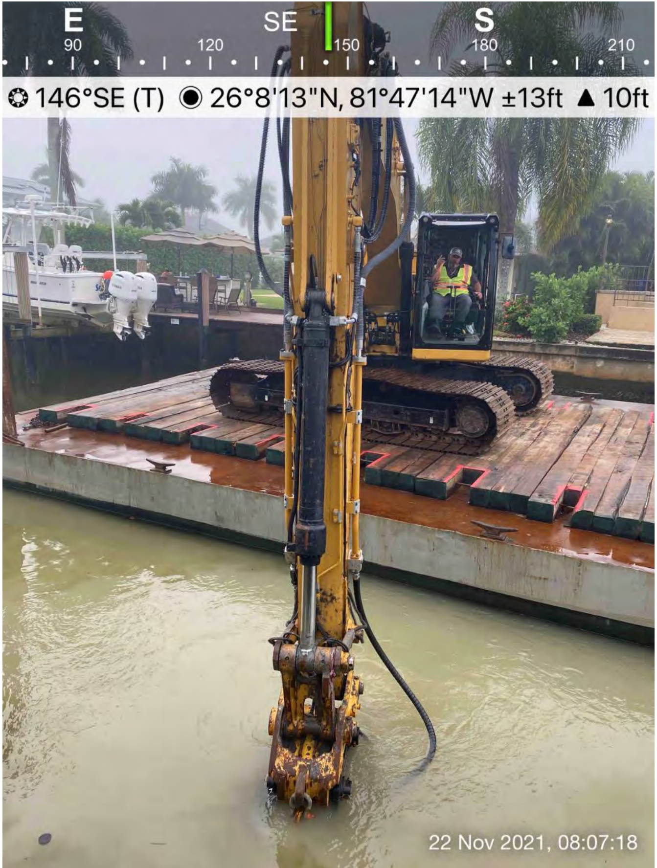
323 excavator grinding rock at station 2+50
