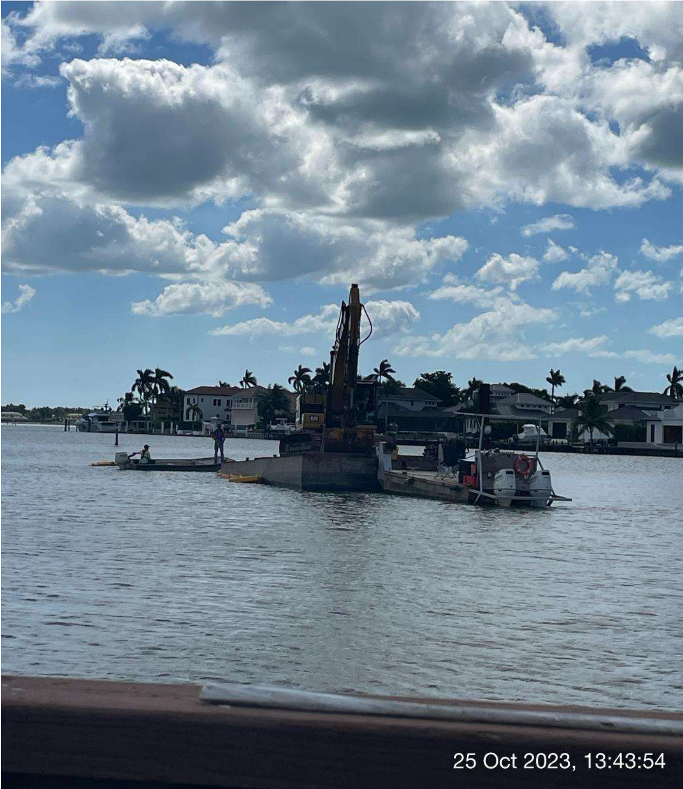
Contractor using magnet to locate missing cutter drum.
