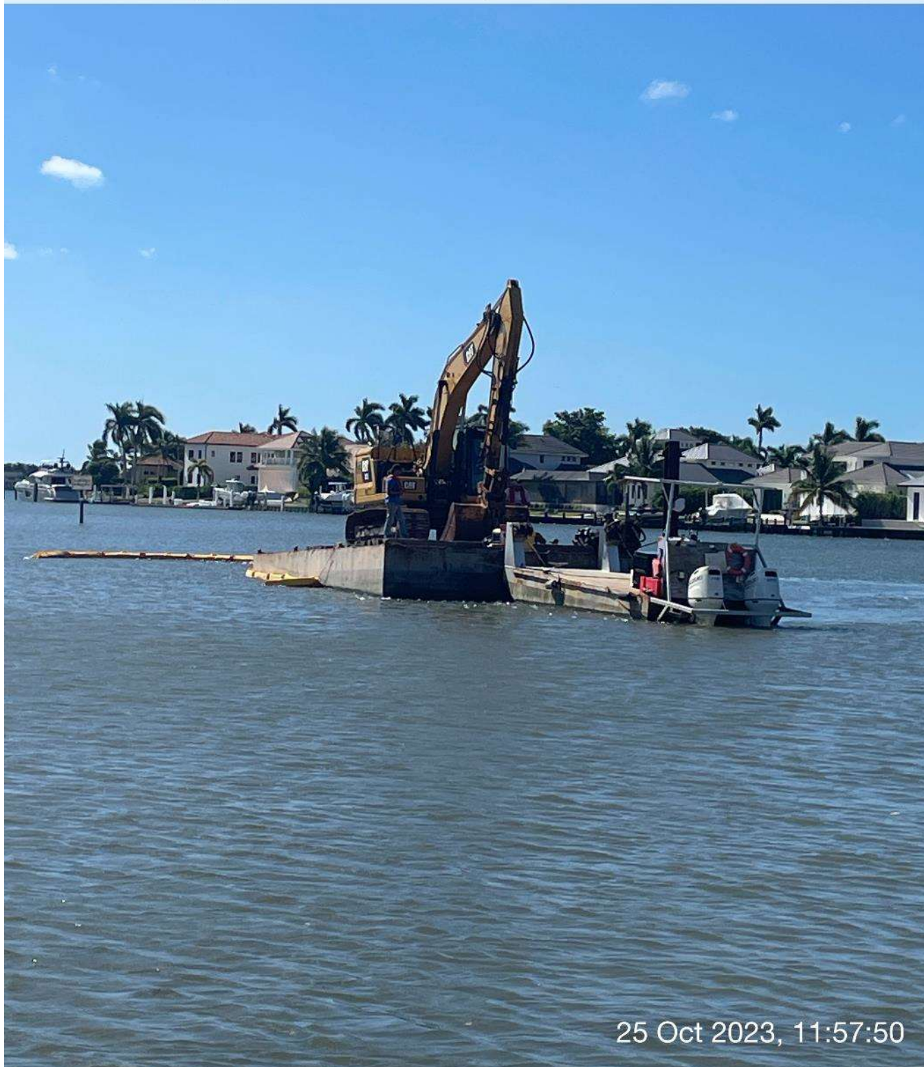
Mechanic arriving on site.
