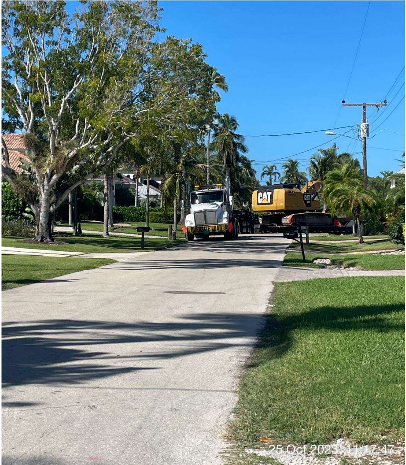
Long reach excavator leaving staging area at 1387 Marlin Drive.
