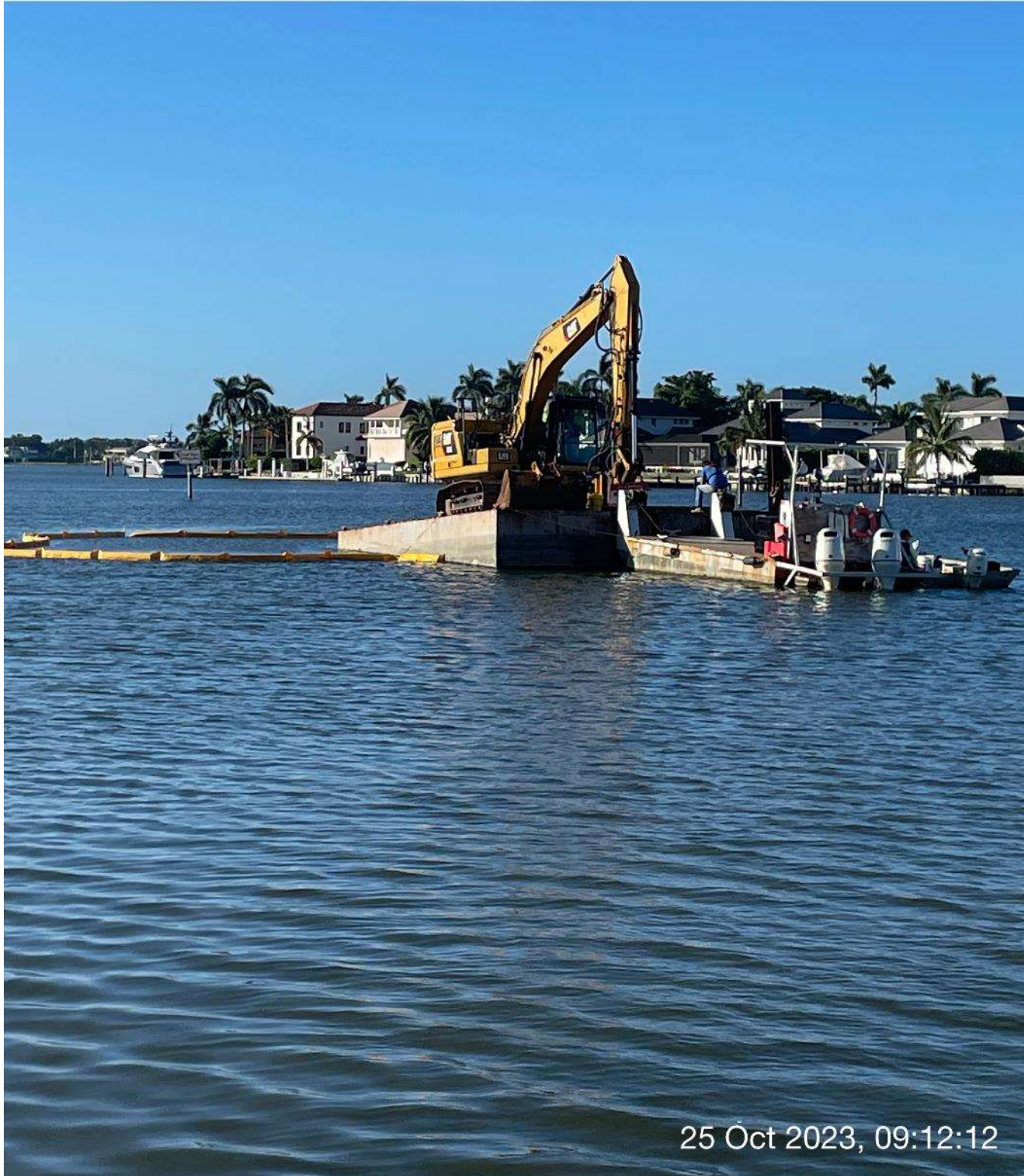
323 excavator switching from Epiroc grinder attachment to bucket attachment.
