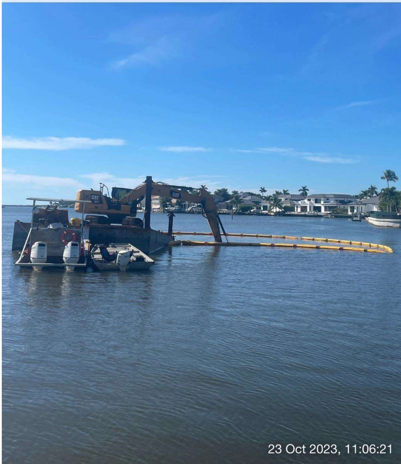
323 excavator grinding rock at station 2+25 in Canal Main B.
