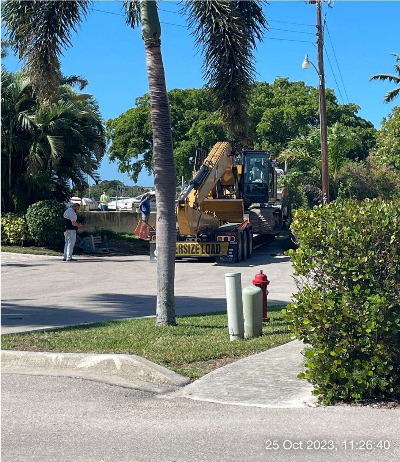
Long reach excavator arriving at staging area at 1300 Curlew Avenue.
