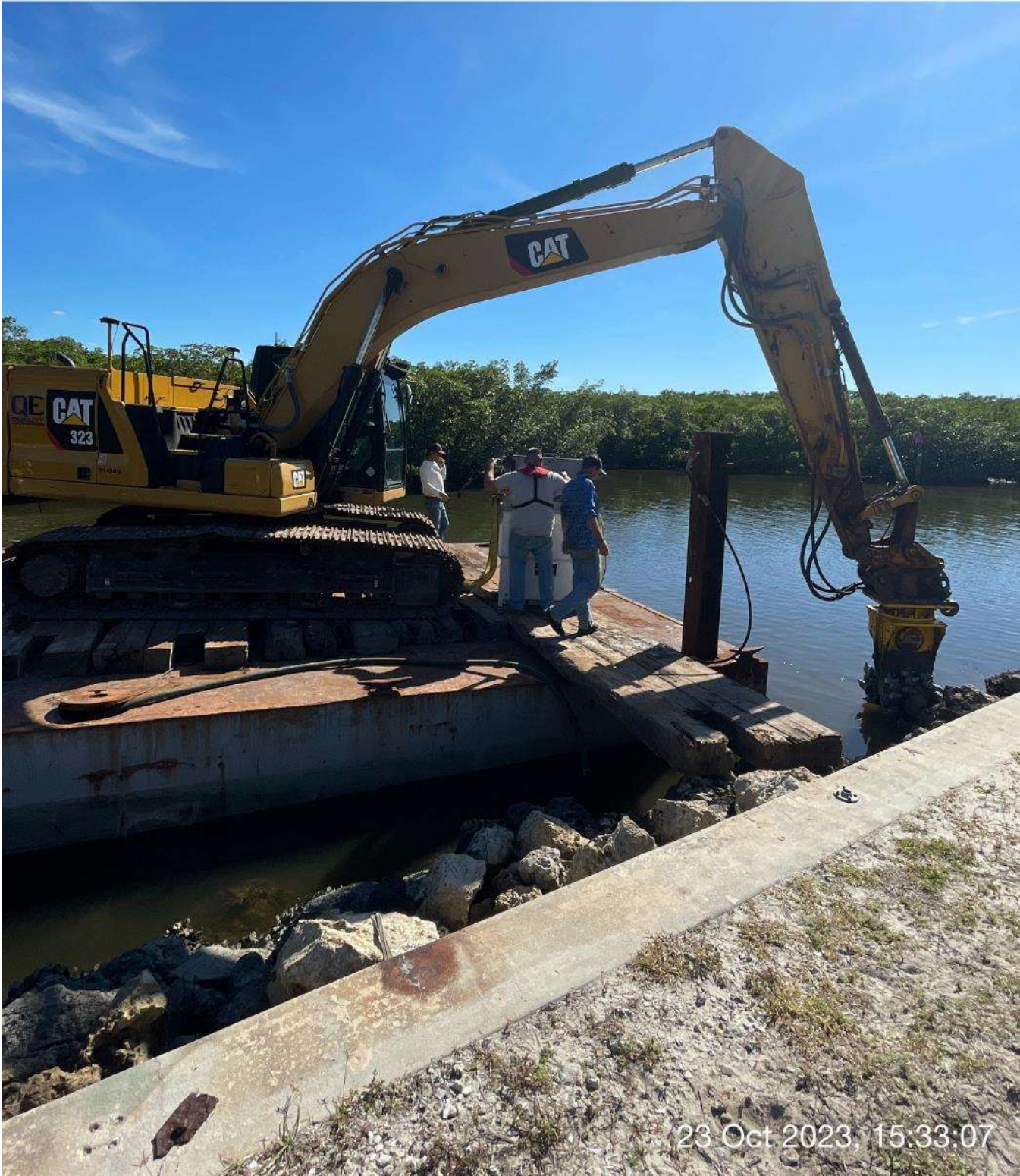
Contractor refueling 323 excavator.
