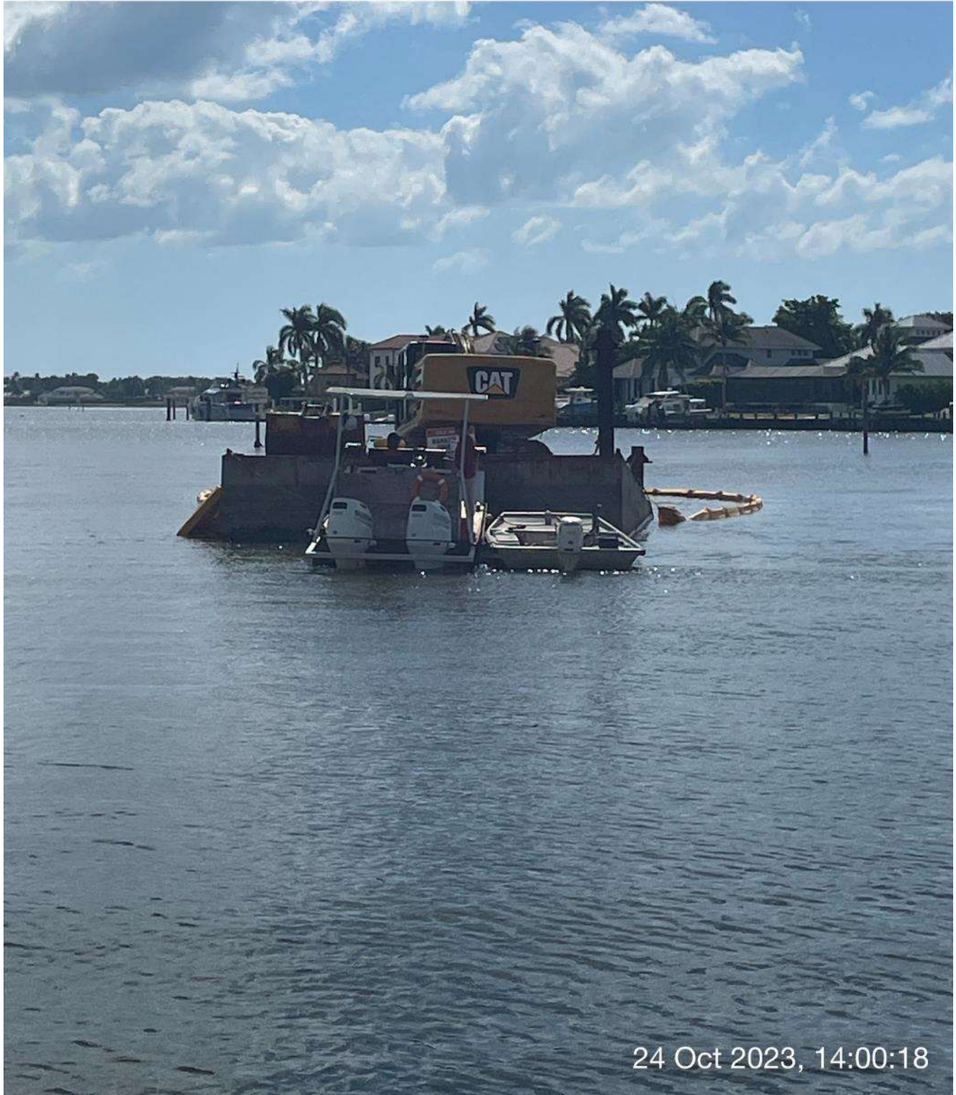
323 excavator grinding rock at station 1+00 in Canal Main B.
