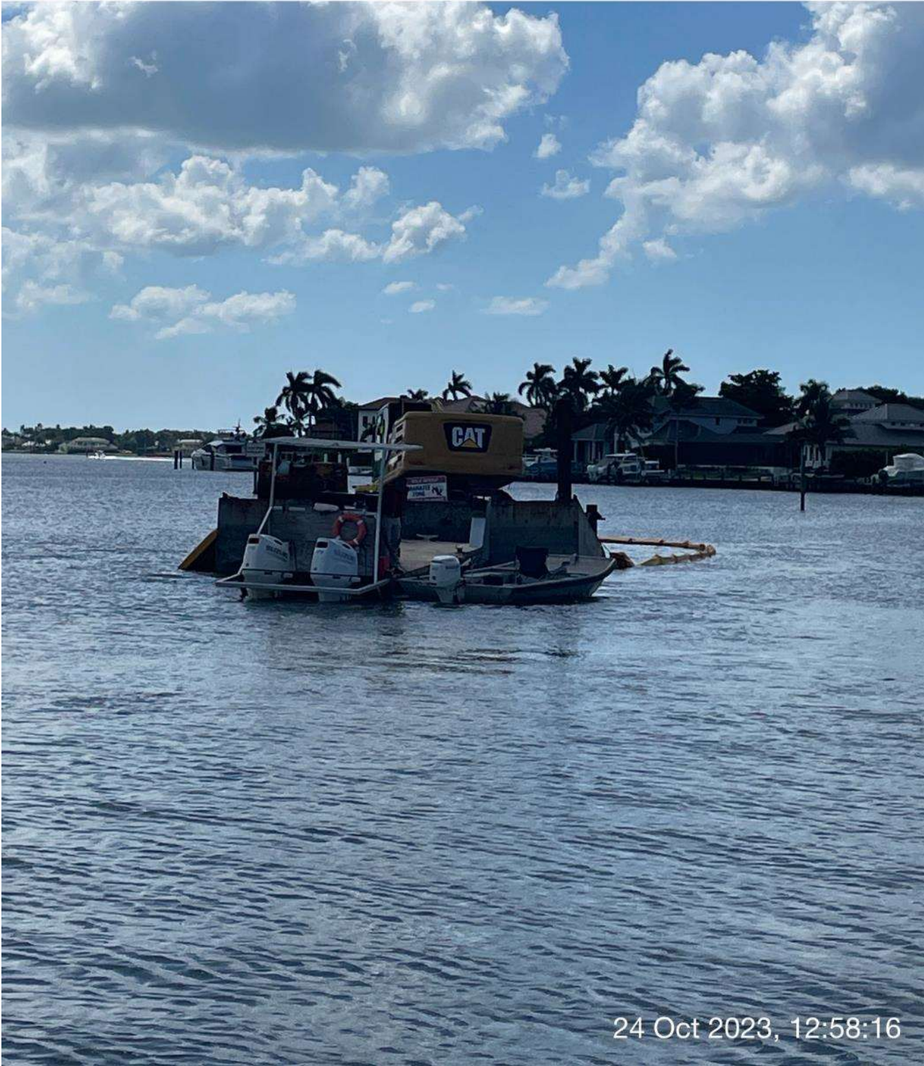
323 excavator grinding rock at station 1+50 in Canal Main B.
