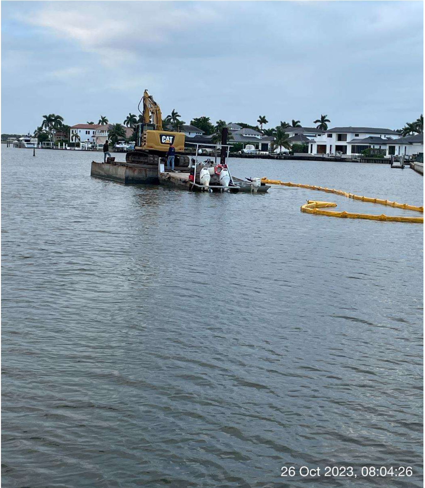
Contractor arriving at station 1+00 in Canal Main B.
