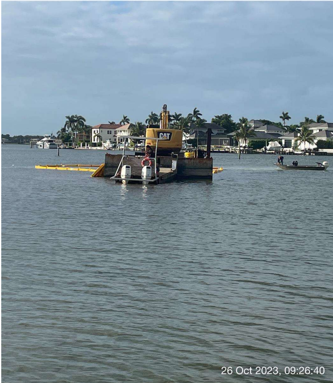
323 excavator digging for missing cutter drum at station 1+00 in Canal Main B.
