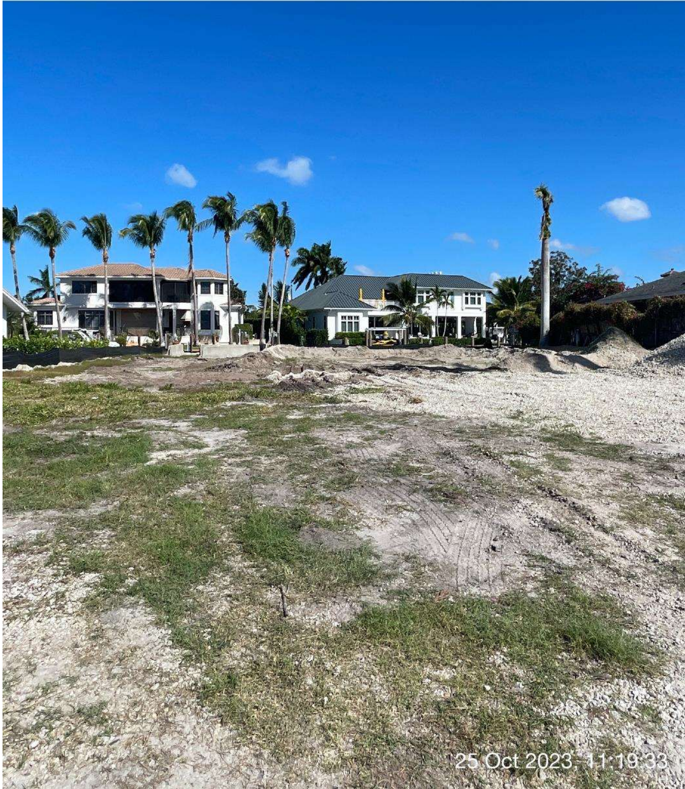
Staging area at 1387 Marlin Drive.
