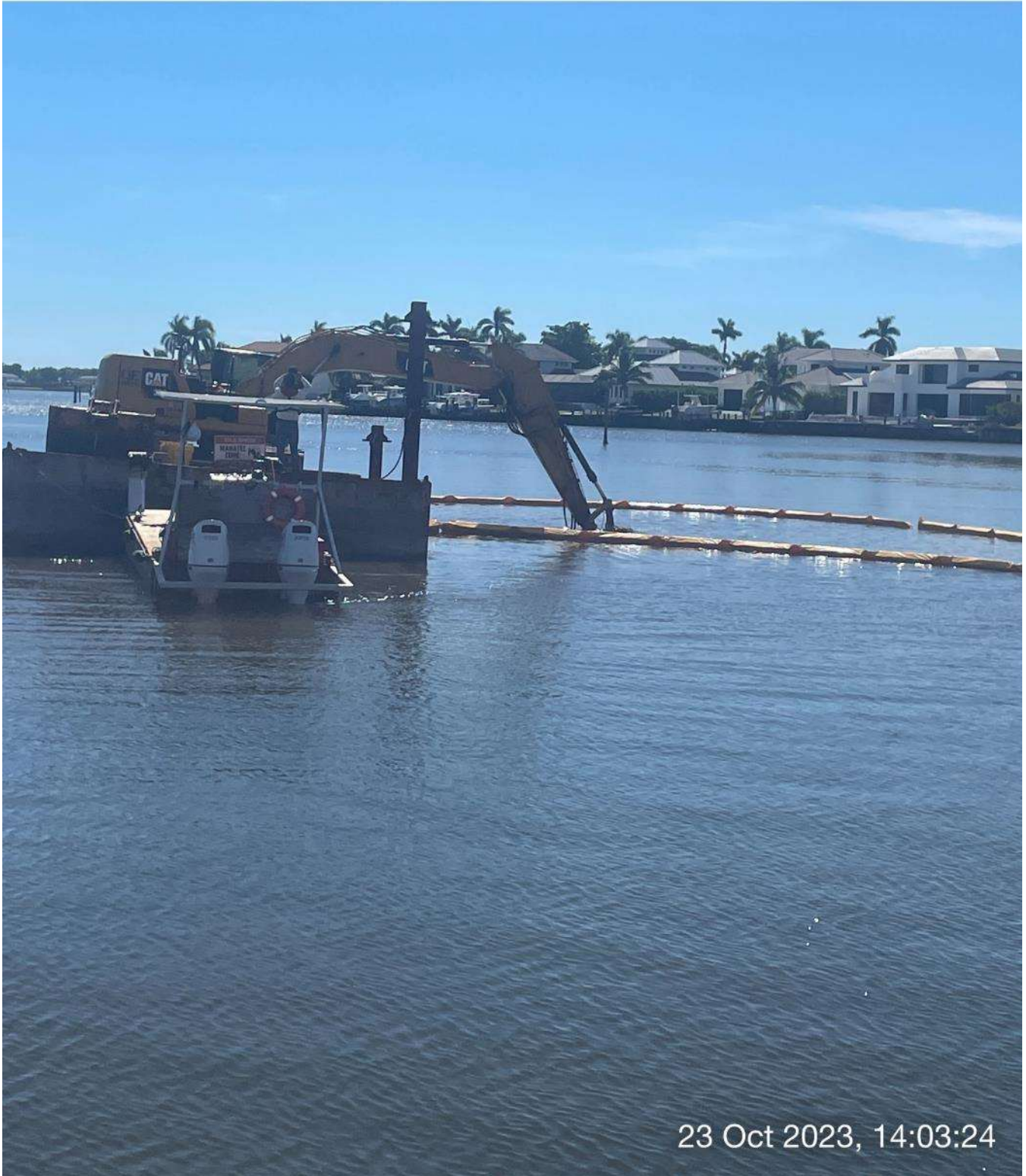
323 excavator grinding rock at station 2+00 in Canal Main B.
