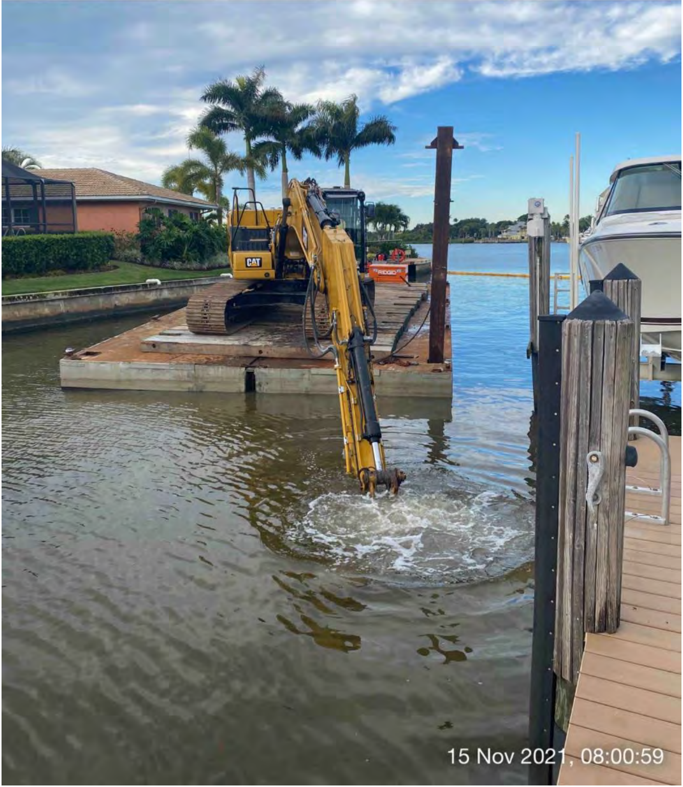
323 excavator removing material from station 2+50
