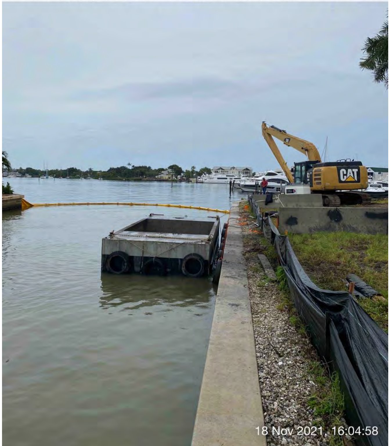
Turbidity curtain, hopper, and 326 excavator
