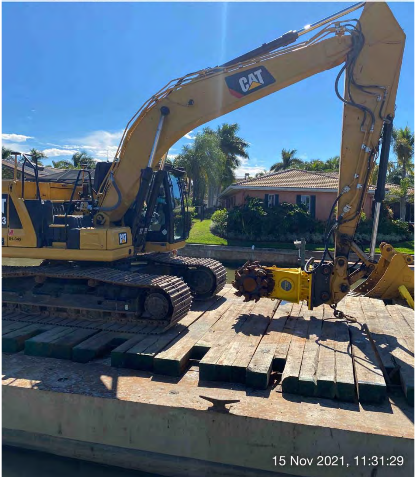
323 excavator with Epiroc grinder on barge at station 2+00
