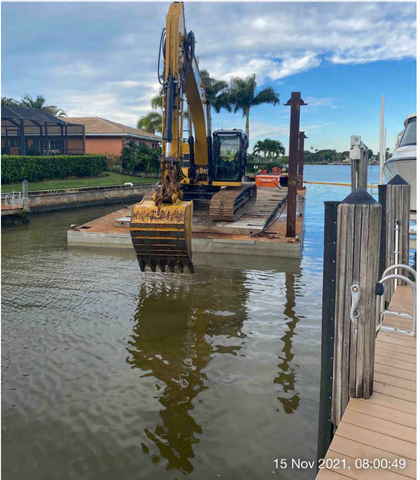
323 excavator removing material from station 2+50
