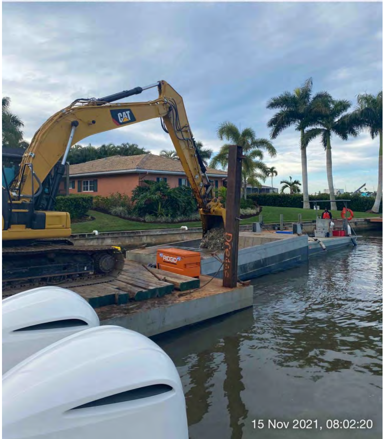
323 excavator transferring material from station 2+50 to hopper
