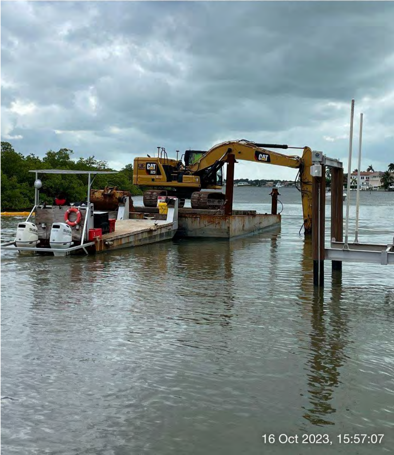
323 excavator grinding rock at station 5+50 in Canal Main B.
