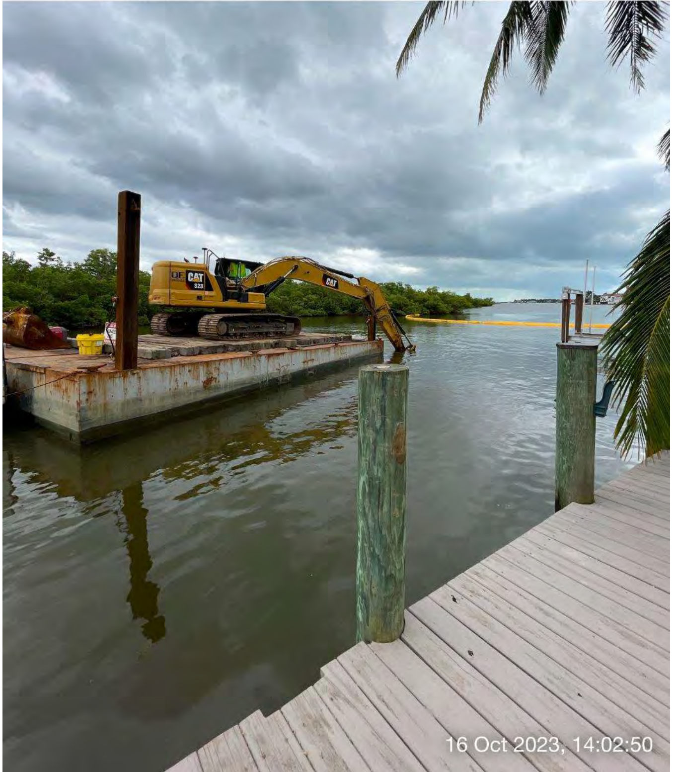
323 excavator grinding rock at station 6+00 in Canal Main B.
