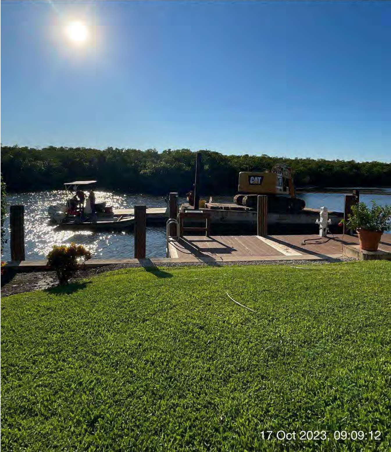
323 excavator grinding rock at station 4+50 in Canal Main B.
