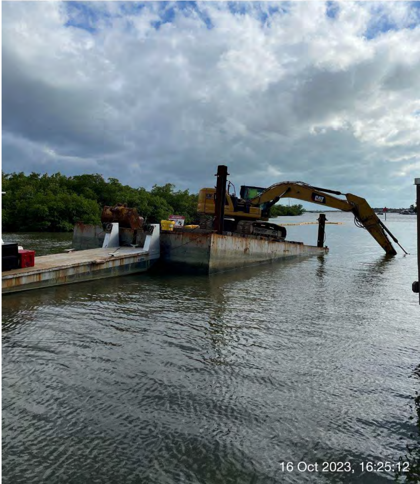
323 excavator grinding rock at station 5+00 in Canal Main B.
