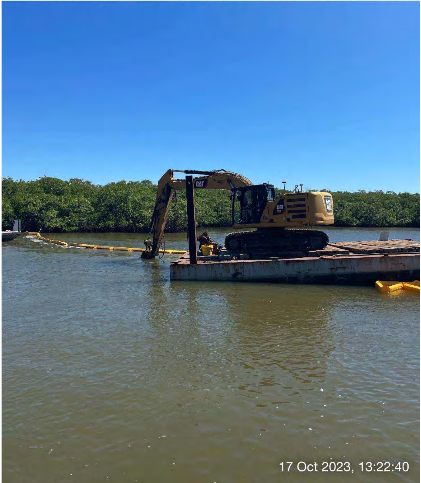
323 excavator grinding rock at station 3+75 in Canal Main B.
