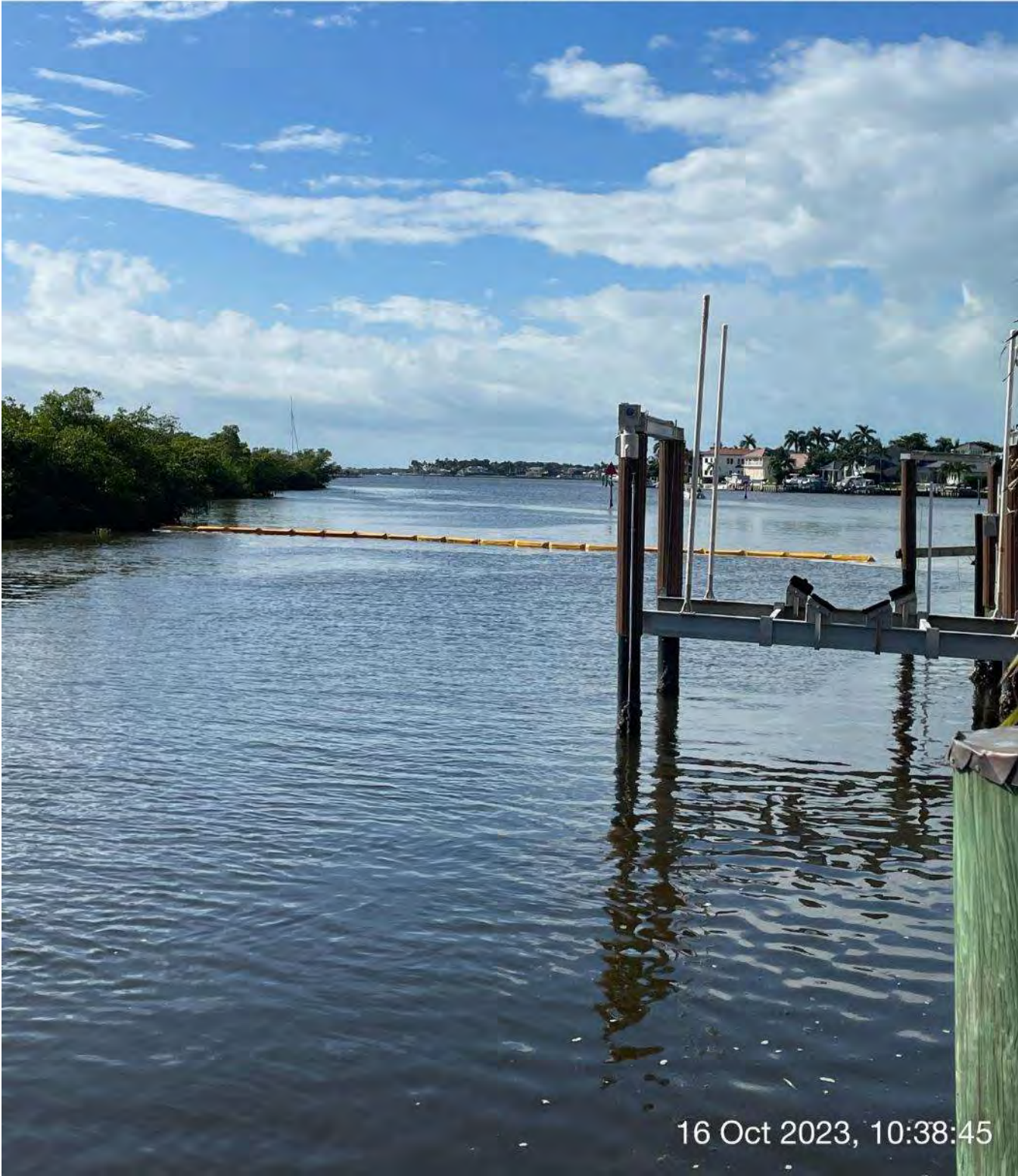
Turbidity curtain in place at station 4+50 in Canal Main B.
