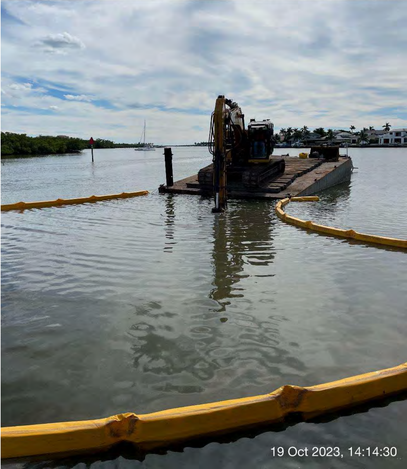
323 excavator grinding rock at station 2+75 in Canal Main B.
