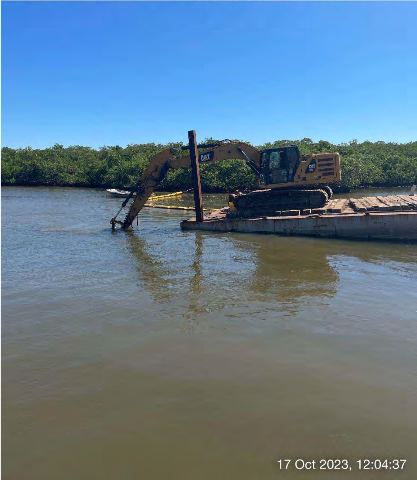
323 excavator grinding rock at station 4+00 in Canal Main B.
