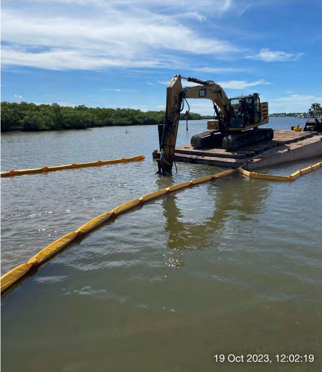
323 excavator grinding rock at station 3+00 in Canal Main B.
