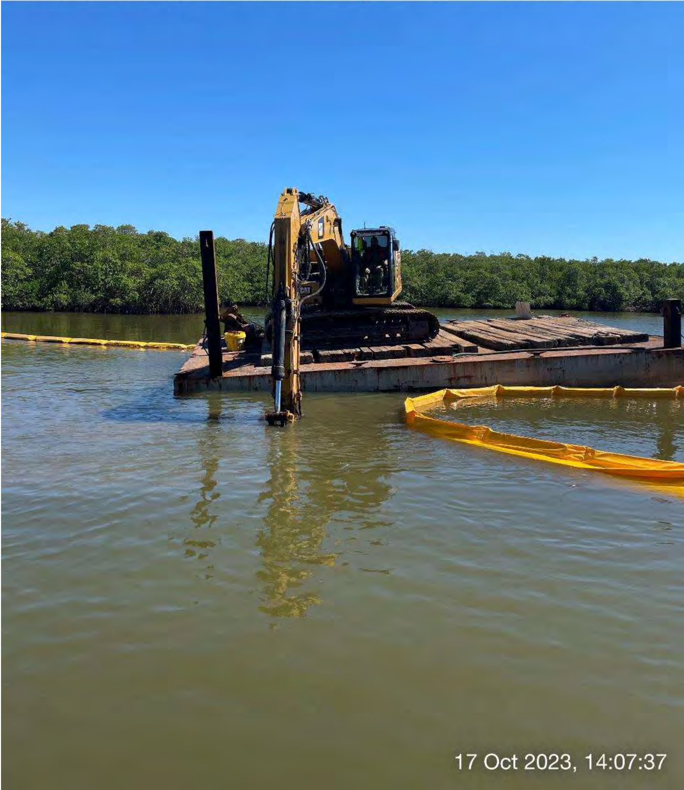
323 excavator grinding rock at station 3+50 in Canal Main B.
