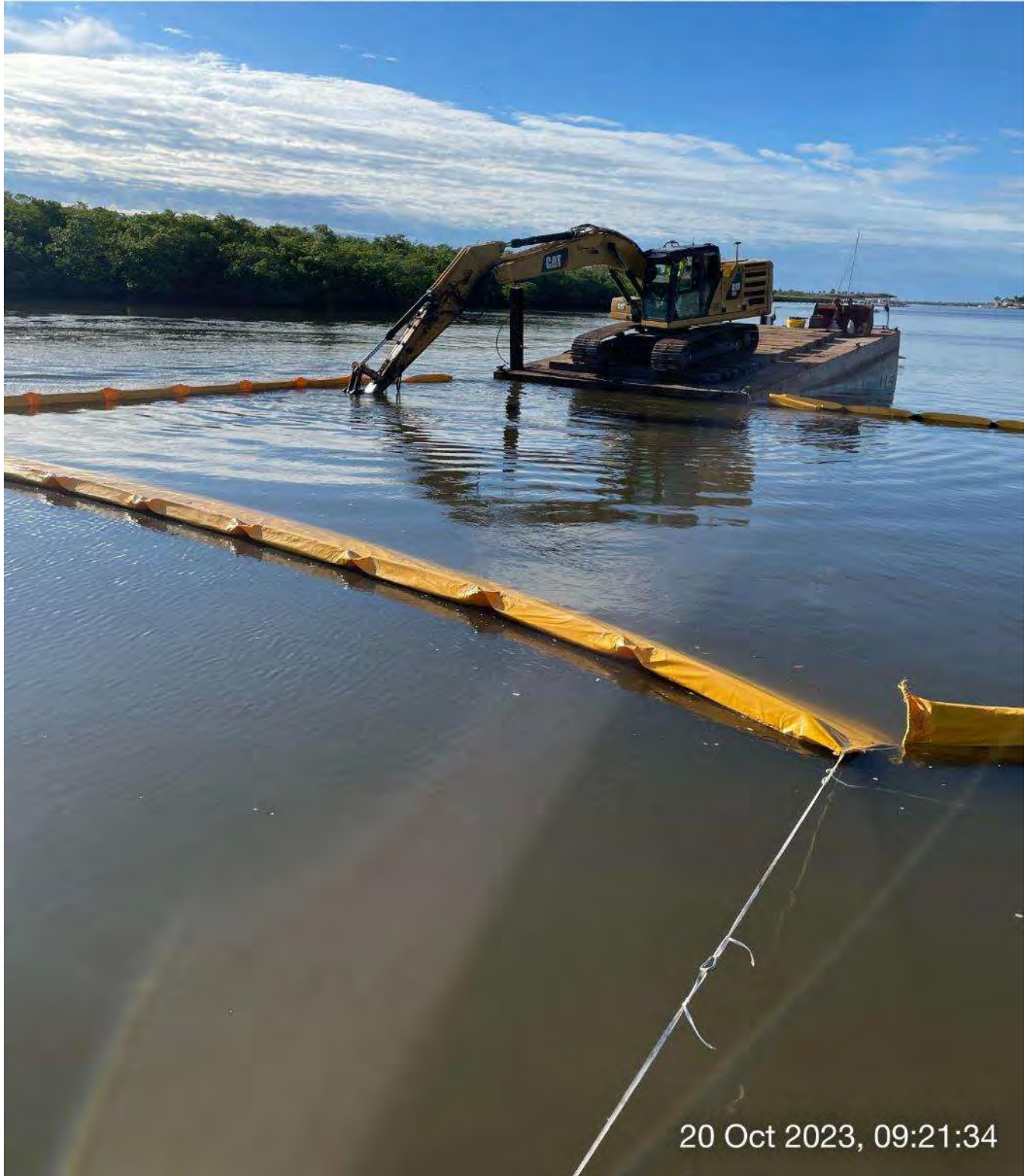
323 excavator grinding rock at station 2+50 in Canal Main B.
