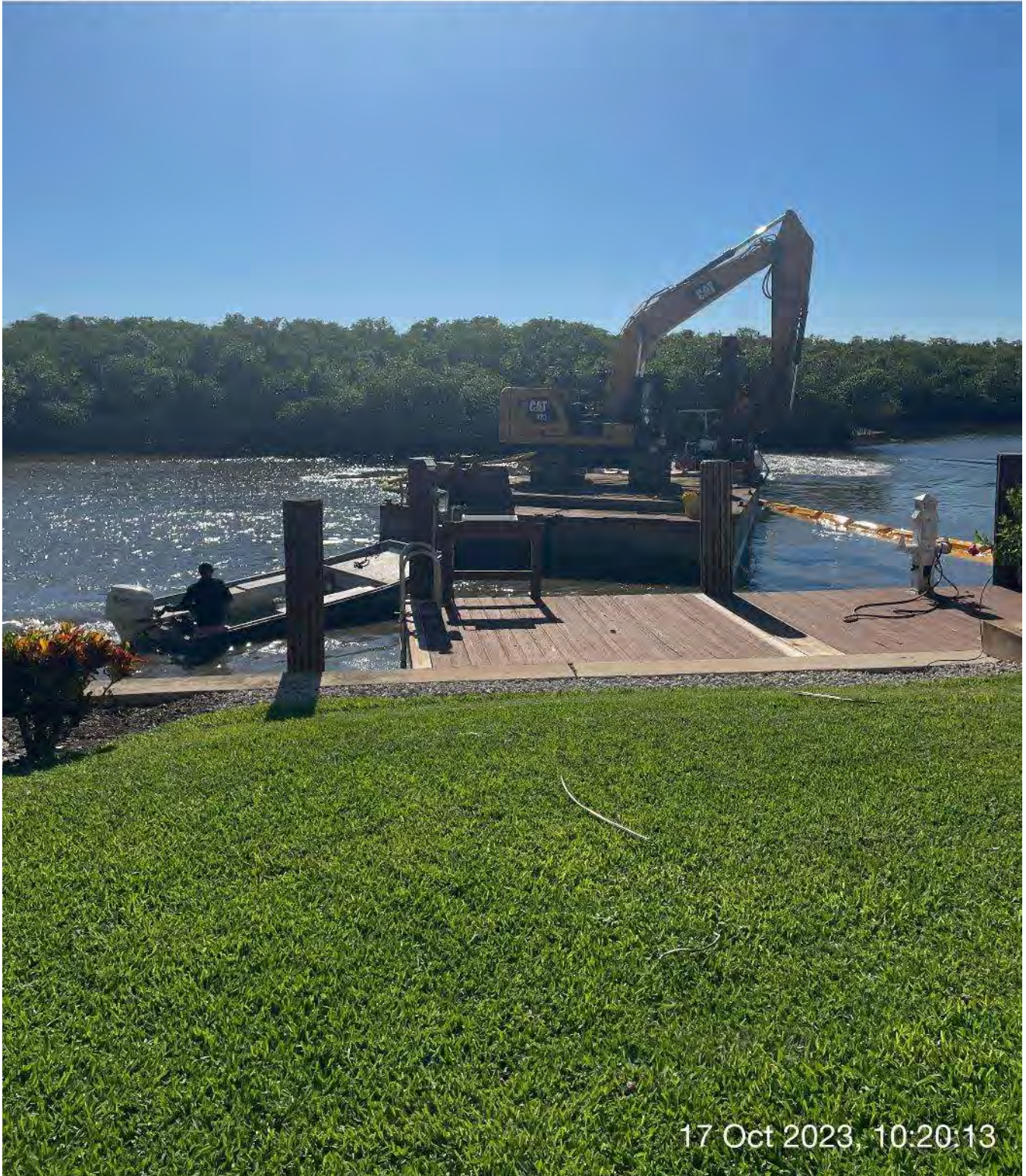
Contractor moving barge and turbidity curtain.
