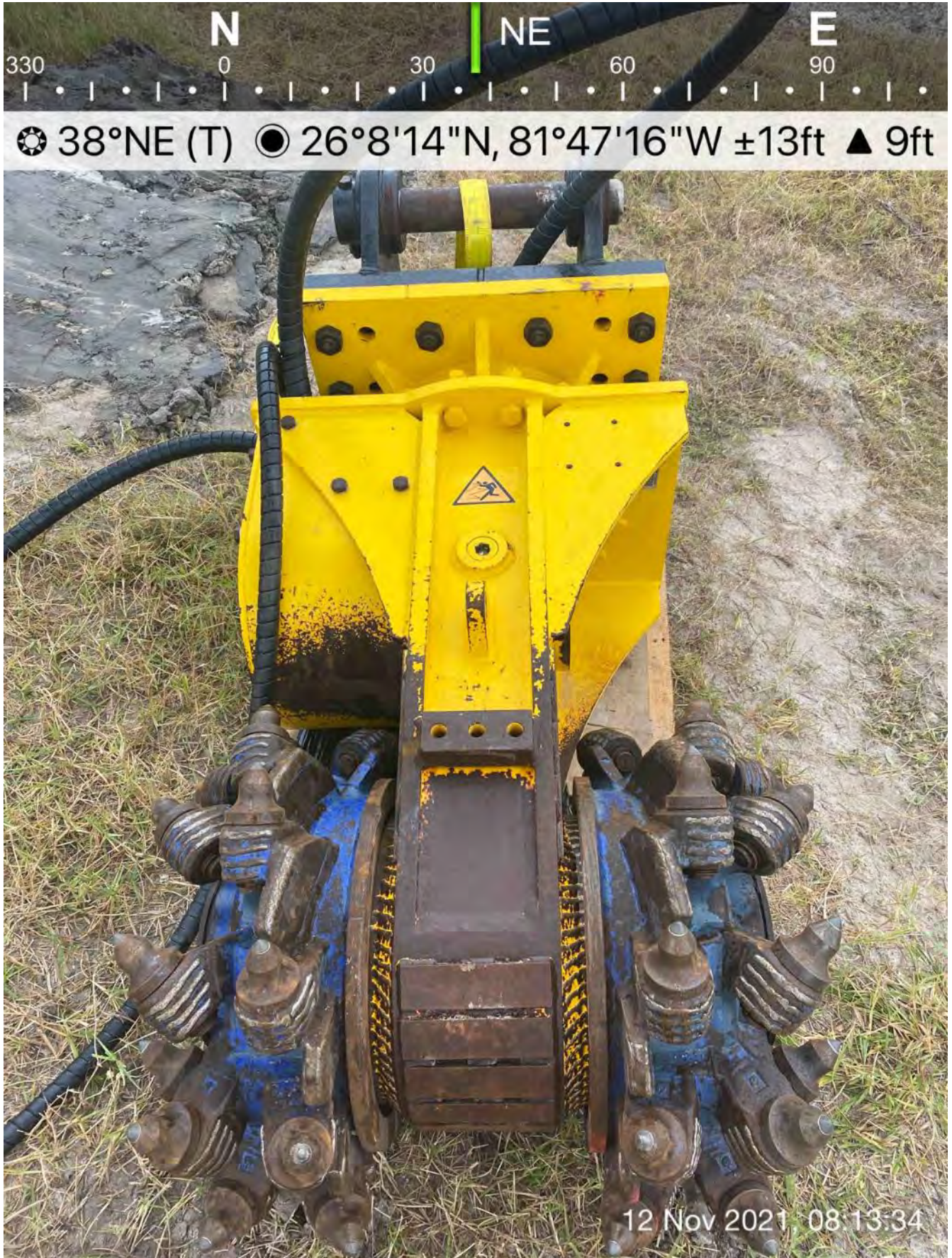
Epiroc grinder on the empty lot at 1300 Curlew Avenue
