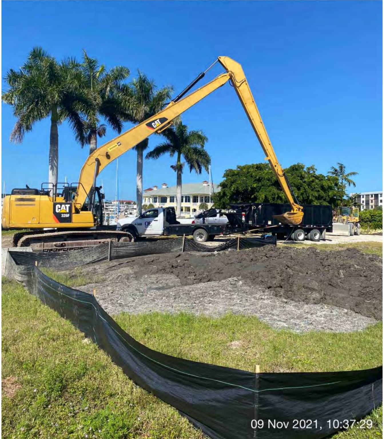
326 excavator towing dump truck
