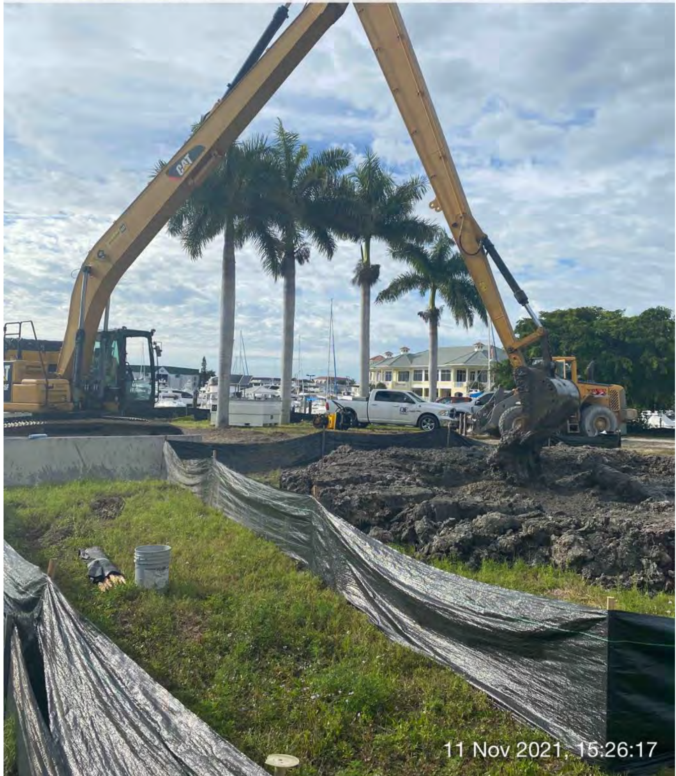
326 excavator transporting rock and sediment from the hopper to the dewatering site at 1300 Curlew Avenue
