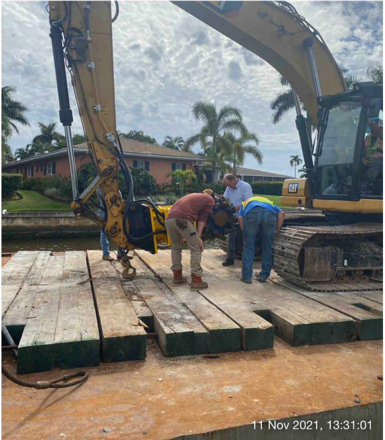
Inspecting Epiroc grinder attached to 323 excavator
