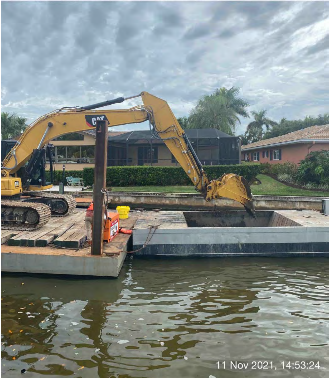
323 excavator transporting rock and sediment from station 3+00 to hopper
