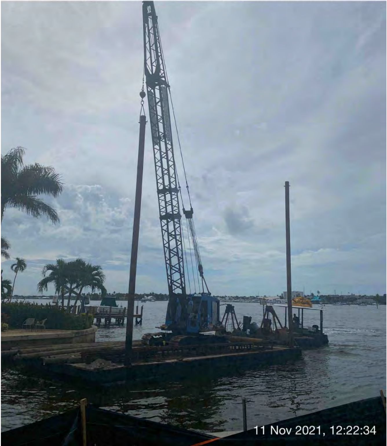
Another contractor's barge, crane, and push boat entering Canal CC-CC
