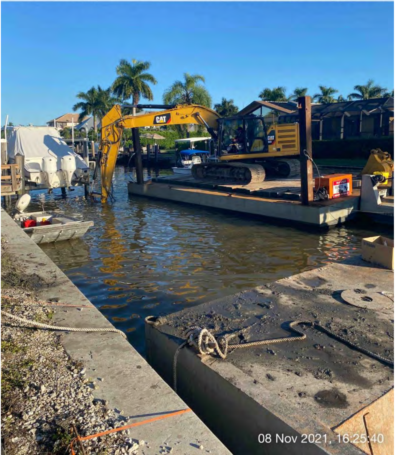
323 excavator grinding rock at station 2+50
