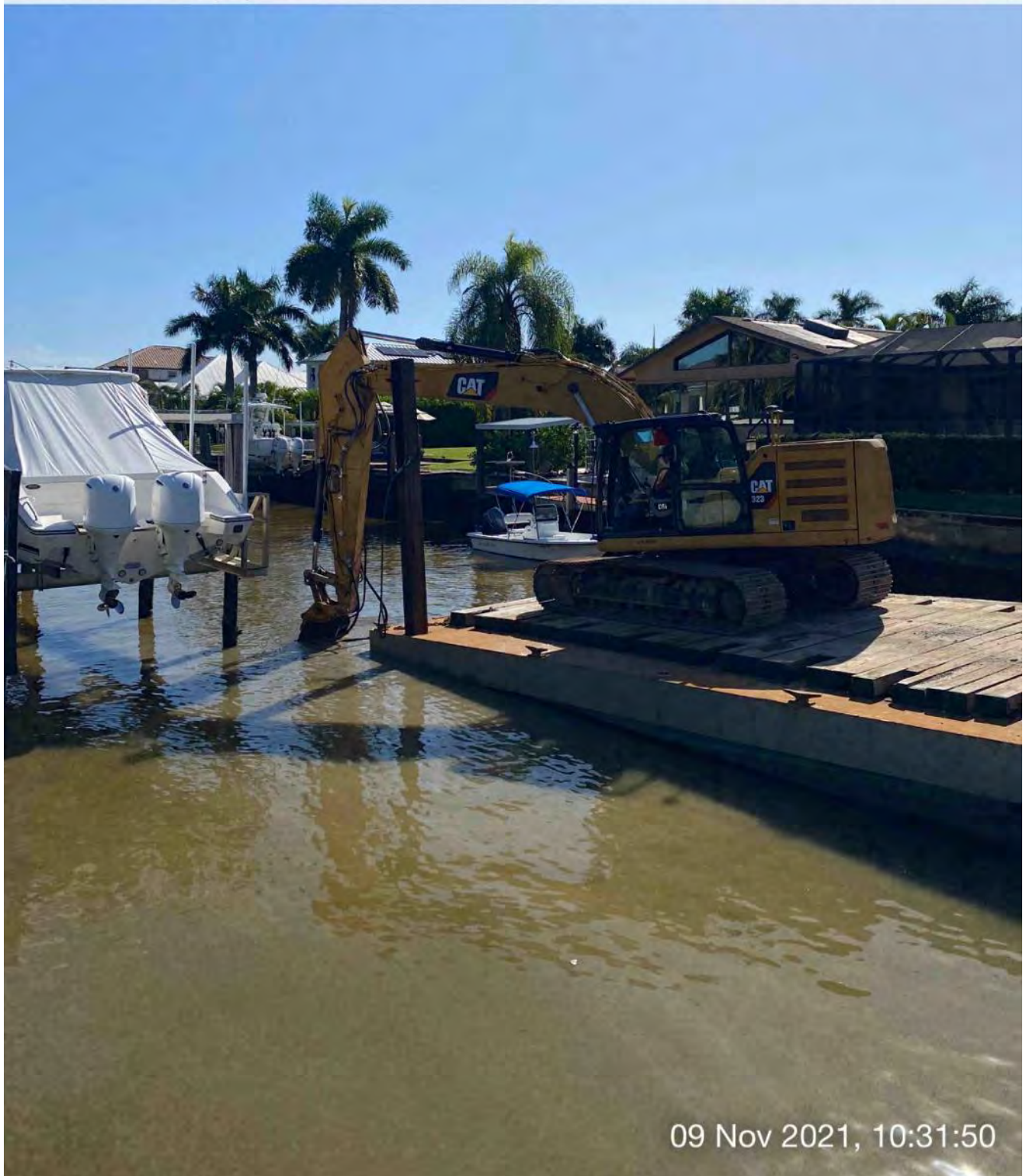
323 excavator grinding rock in Canal CC-CC at station 2+50
