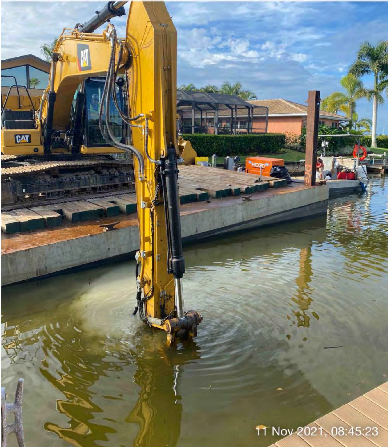
323 excavator grinding rock at station 3+00
