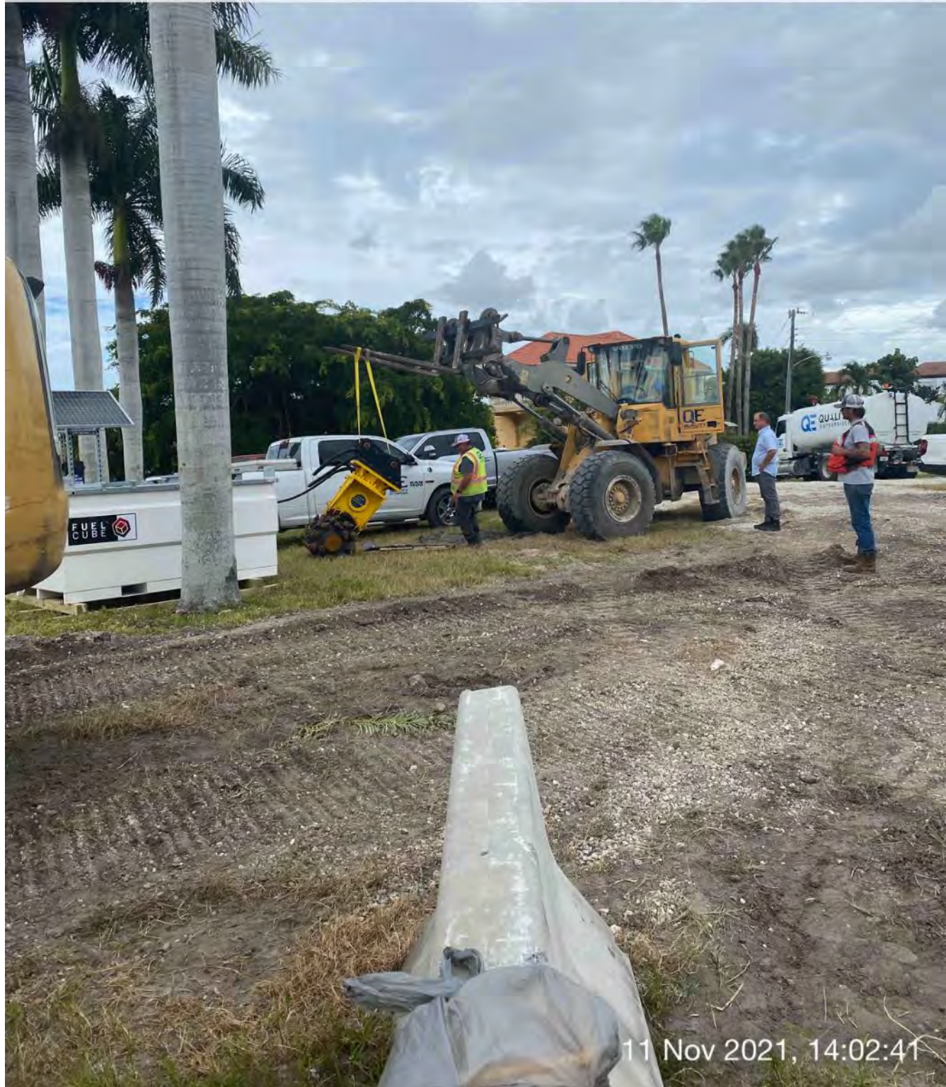
Front end loader transporting Epiroc grinder to the empty lot at 1300 Curlew Avenue
