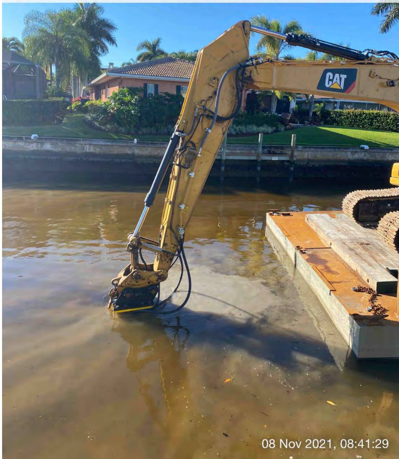
323 excavator grinding rock near station 1+50
