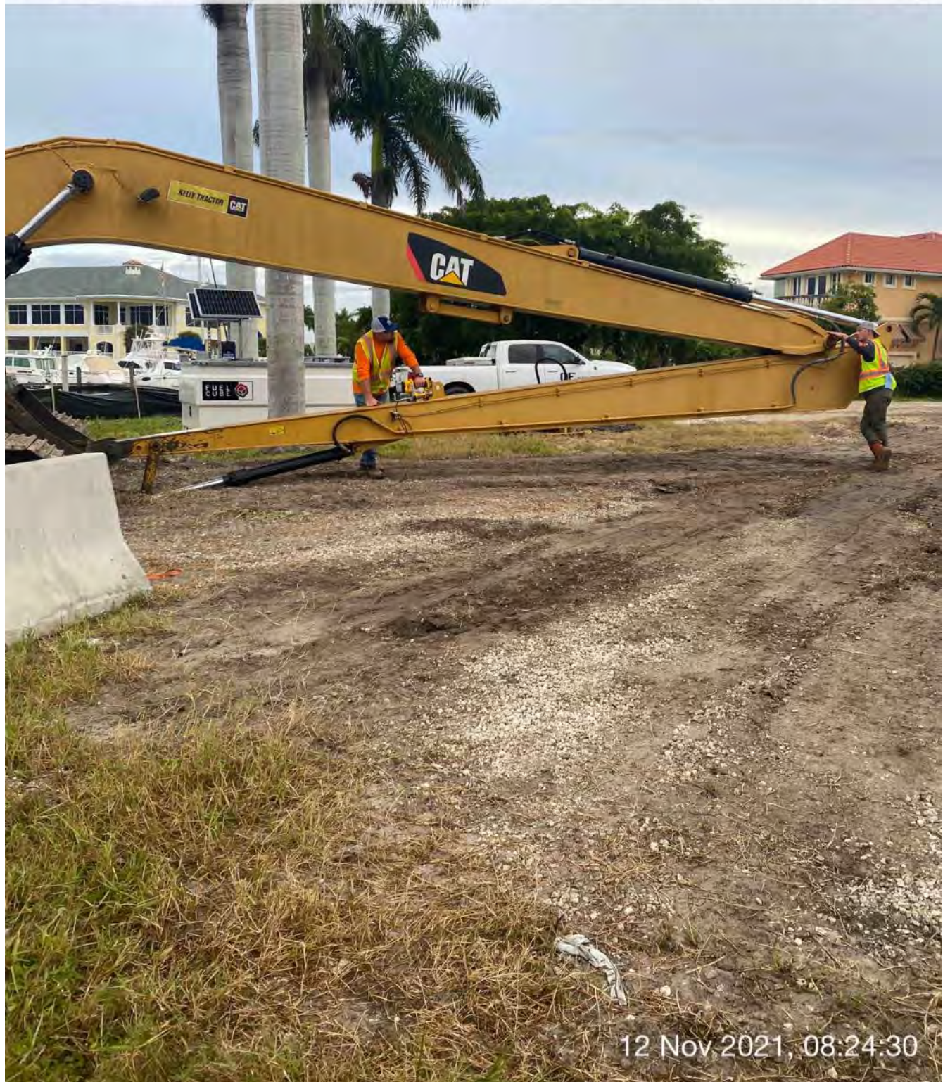
Inspecting, greasing, and cleaning the 326 excavator
