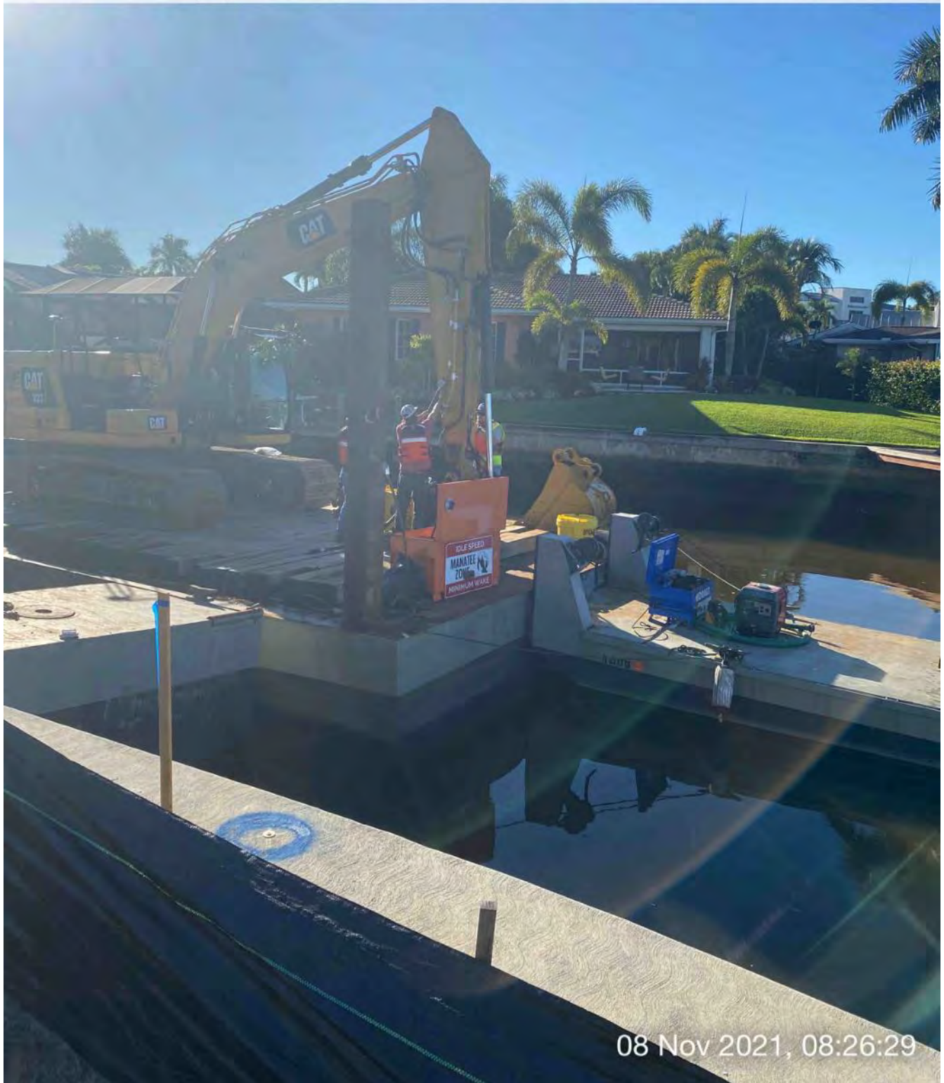
323 excavator on barge attached to push boat
