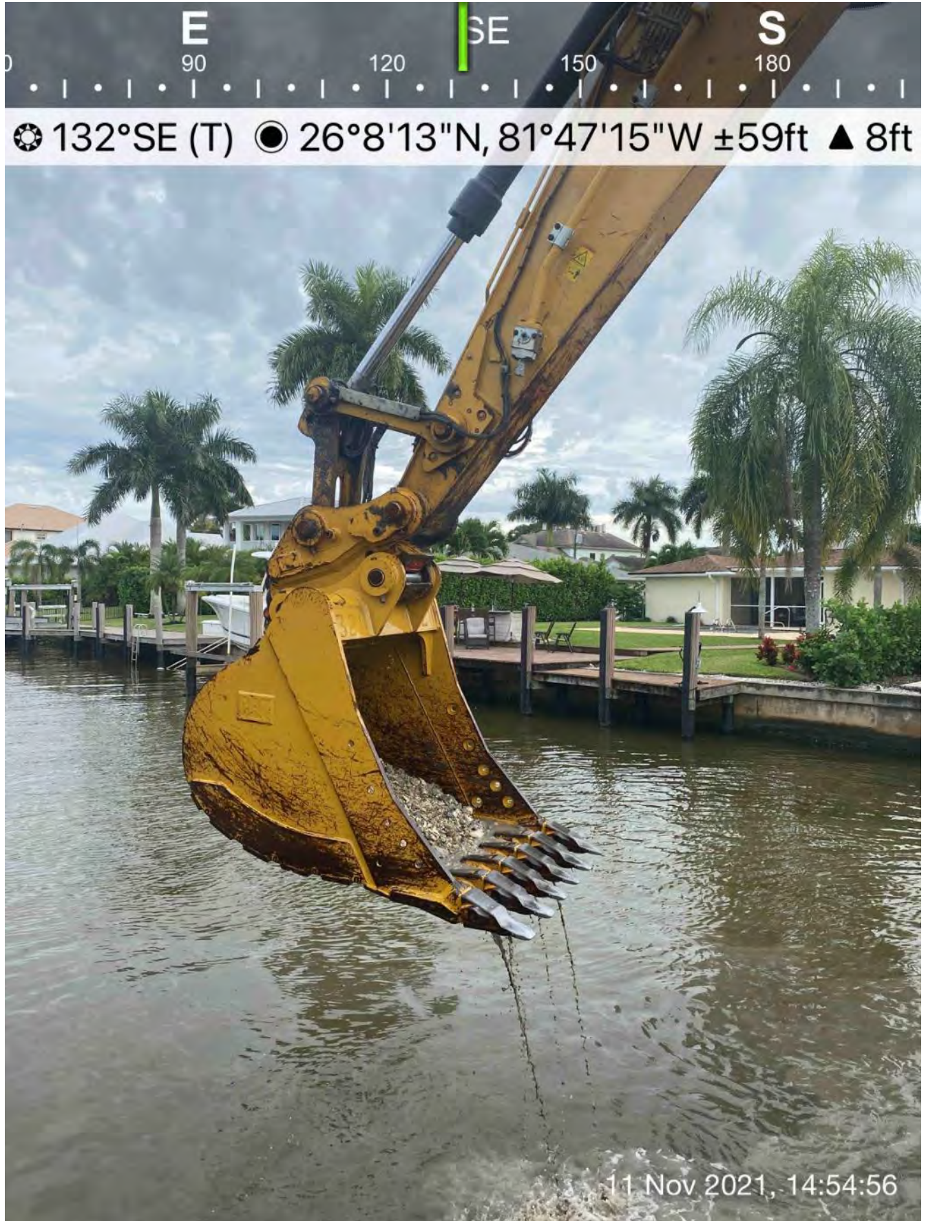
323 excavator transporting rock and sediment from station 3+00 to hopper
