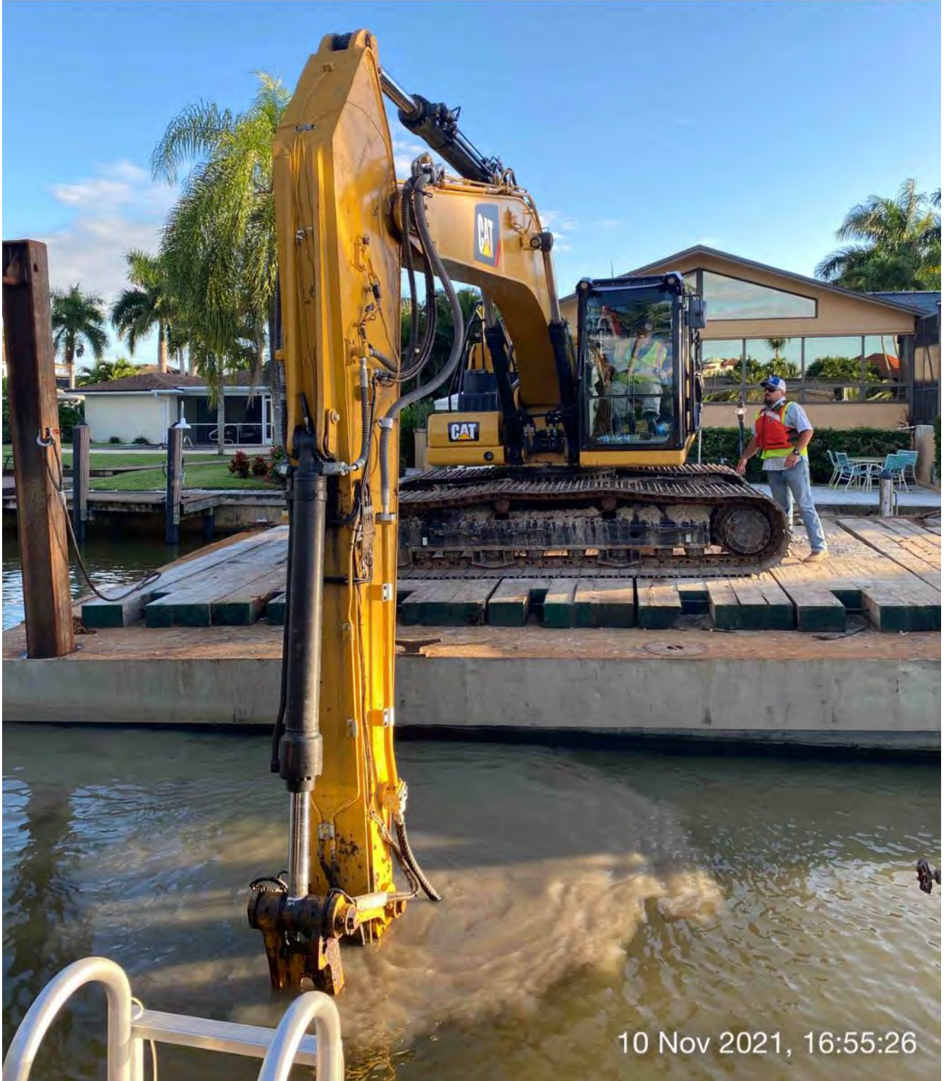
323 excavator grinding rock at station 2+50
