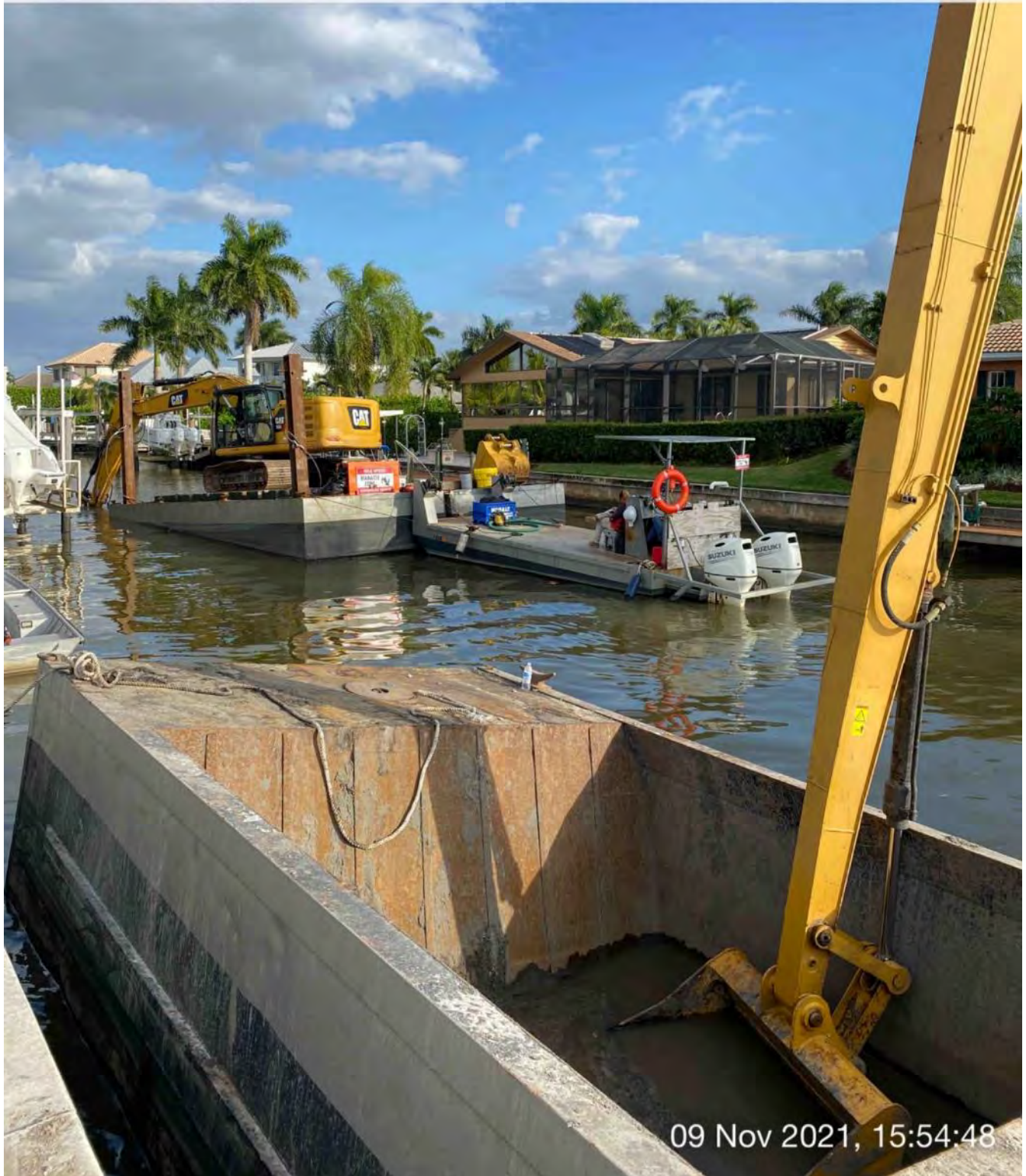
323 excavator grinding rock at station 2+50 and 326 excavator holding barge in place
