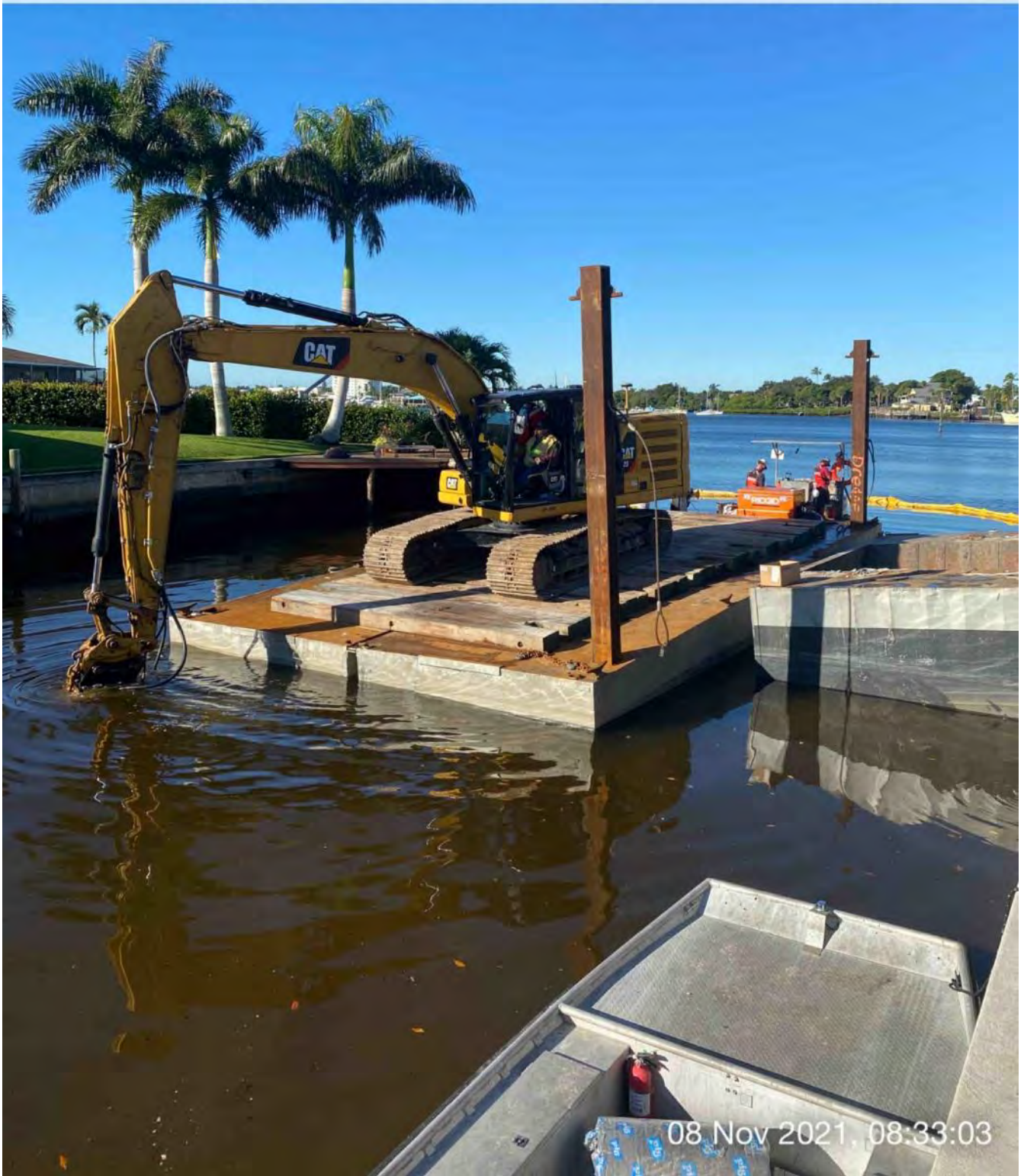
323 excavator on barge grinding rock at station 1+50
