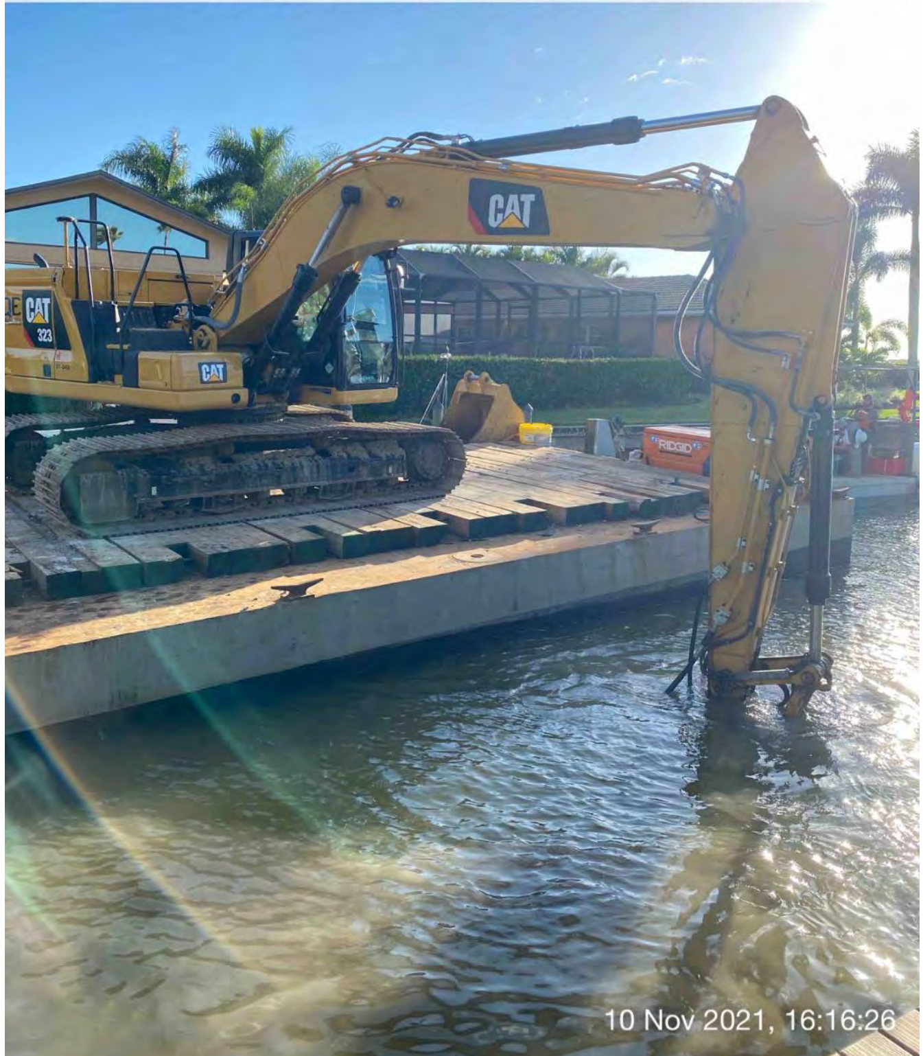
323 excavator grinding rock at station 2+50
