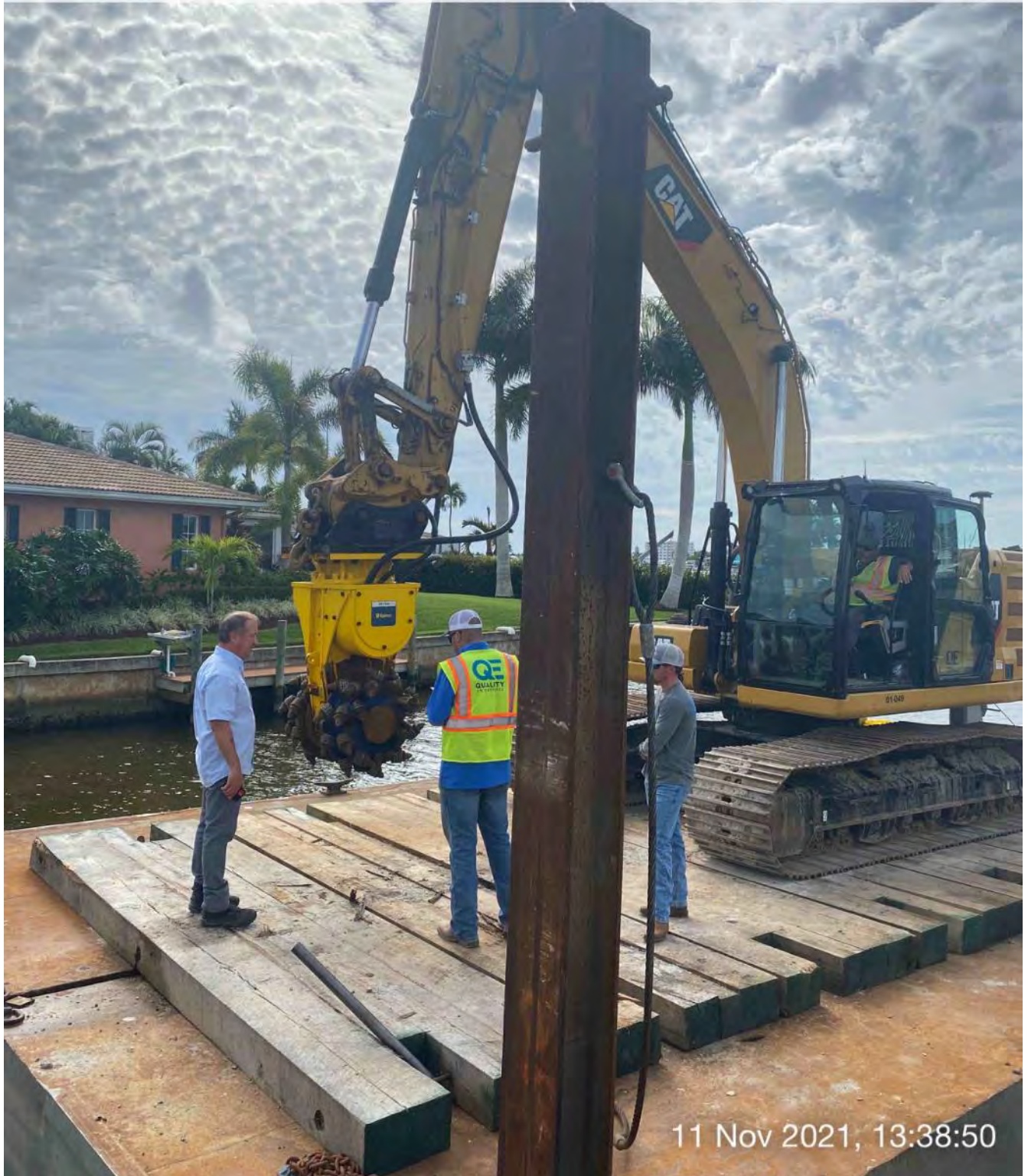
Inspecting Epiroc grinder attached to 323 excavator
