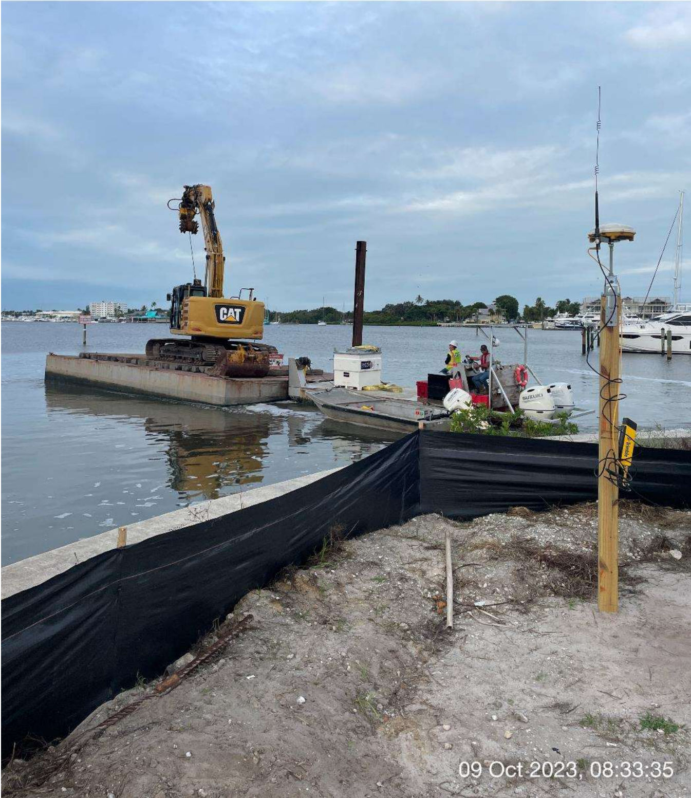
Contractor transporting fuel cube to staging area at 1387 Marlin Drive.
