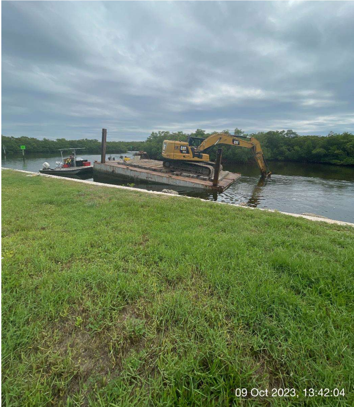
323 excavator grinding rock at station 3+00 in Canal Main B1.
