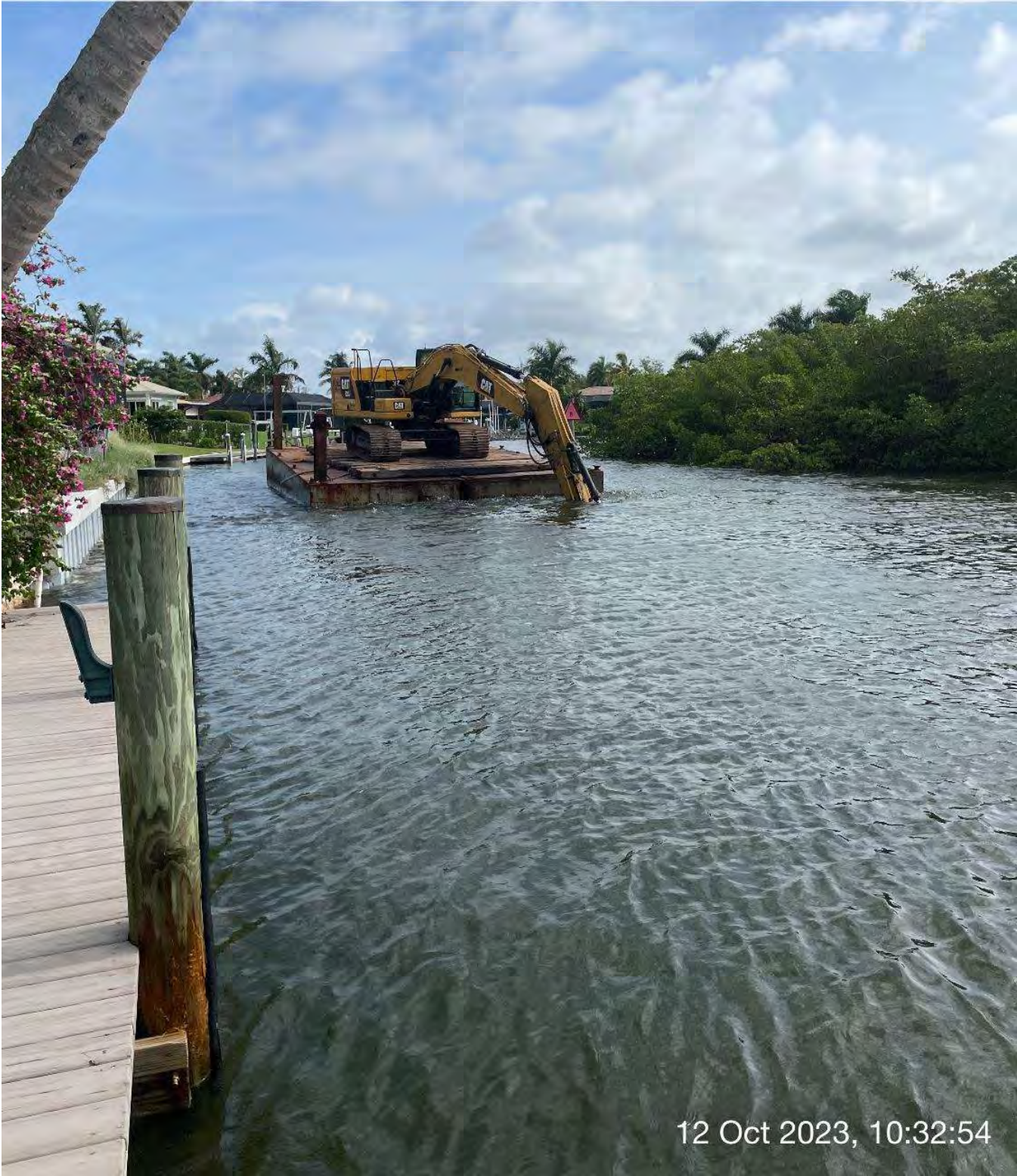
323 excavator grinding rock at station 7+50 in Canal Main B.
