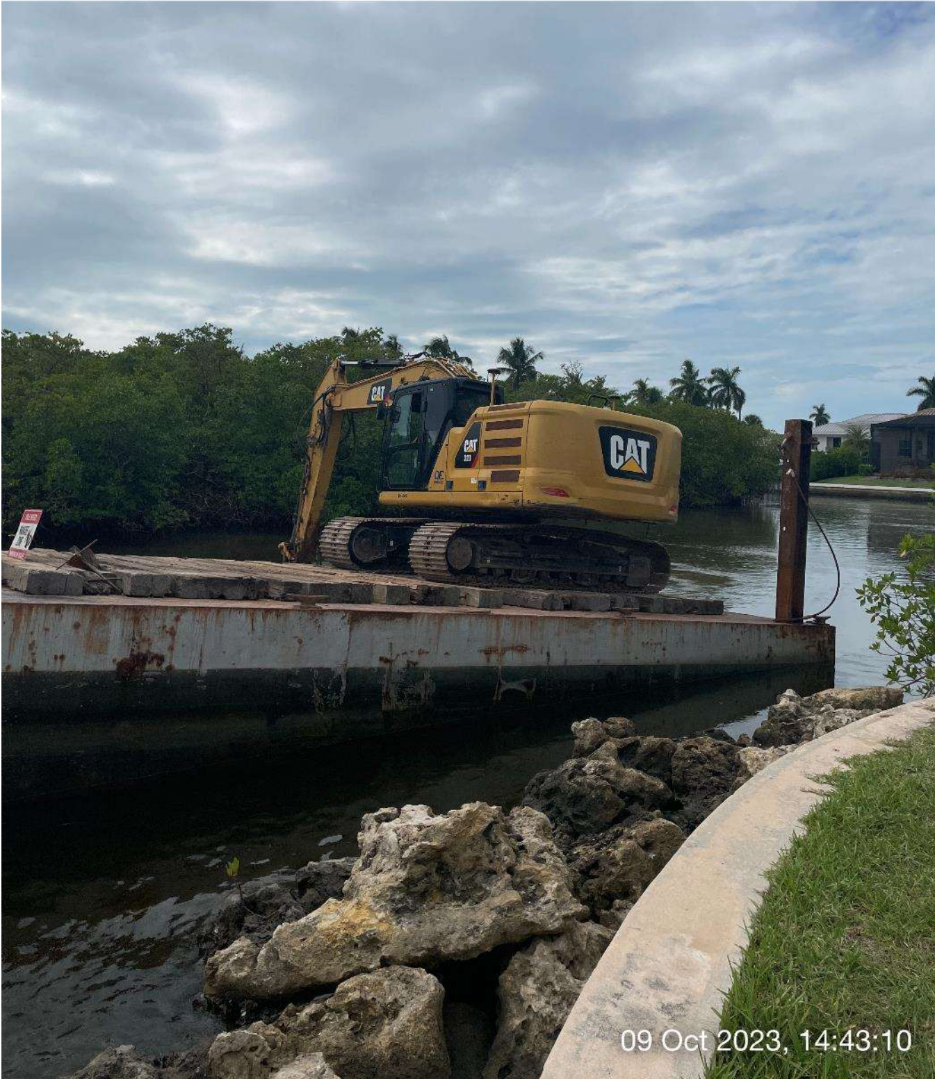
323 excavator grinding rock at station 2+00 in Canal Main B1.
