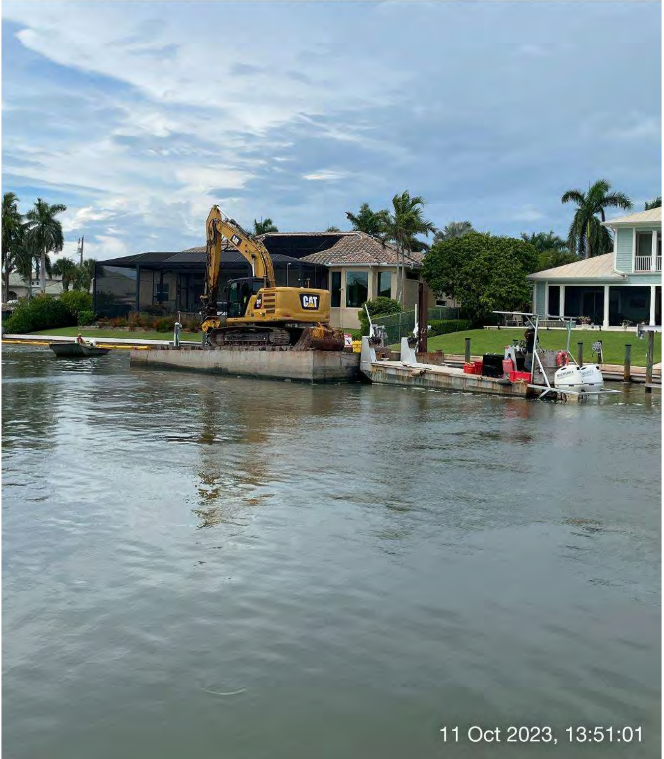
323 excavator grinding rock at station 0+00 in Canal Main B1.
