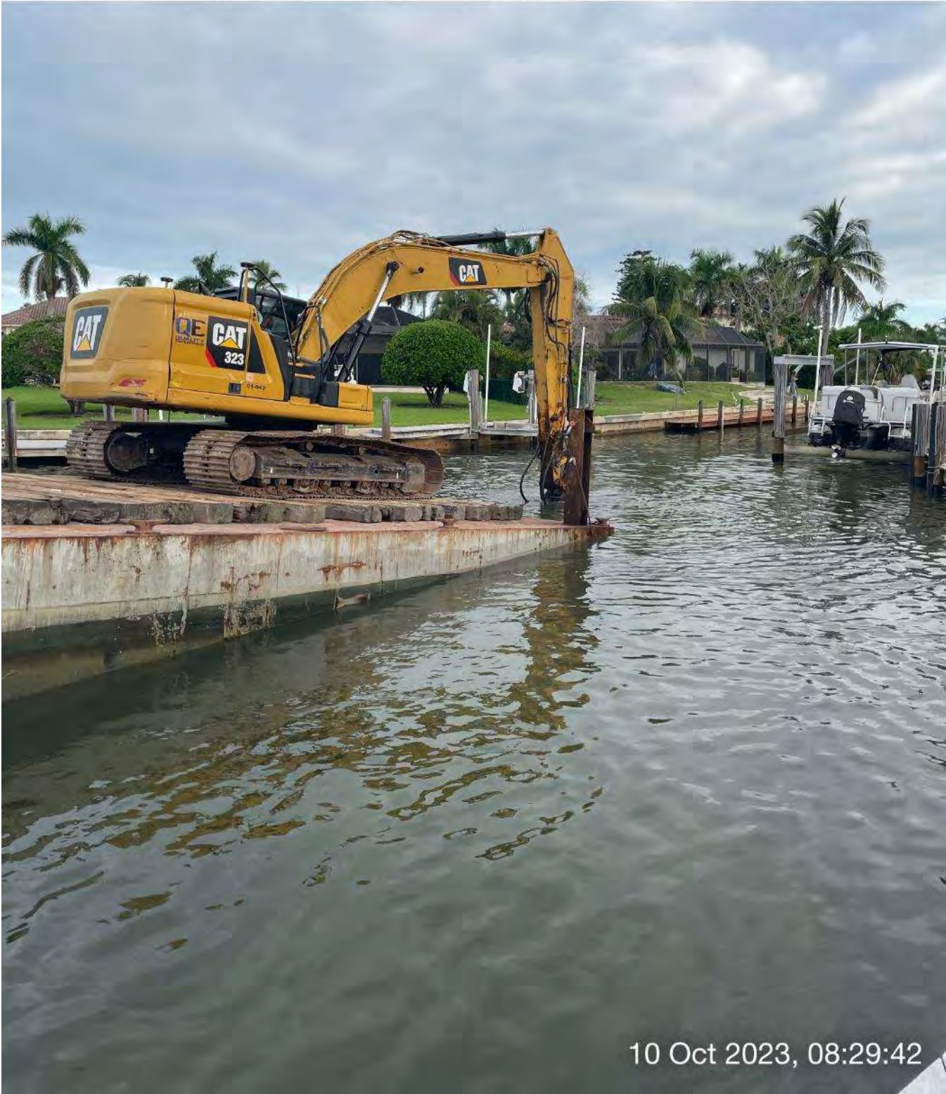
323 excavator grinding rock at station 10+00 in Canal Main B.
