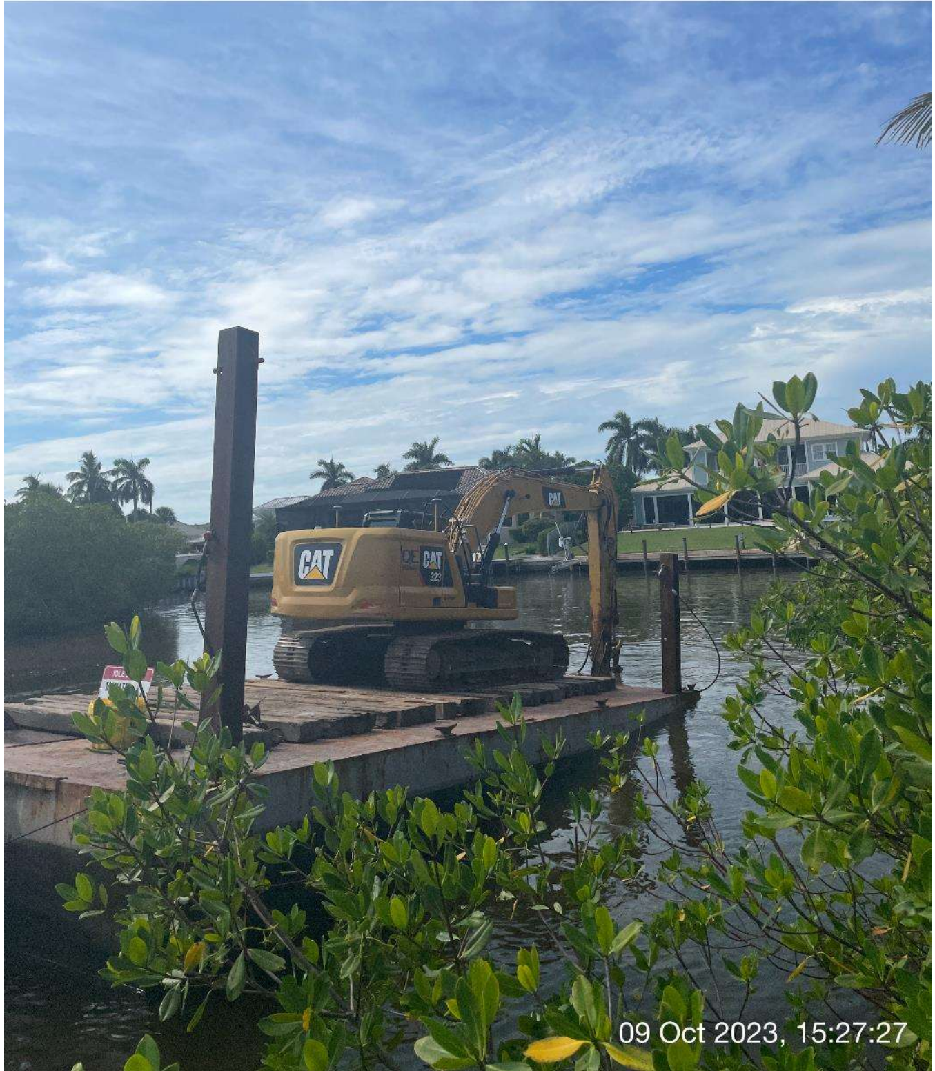
323 excavator grinding rock at station 1+50 in Canal Main B1.
