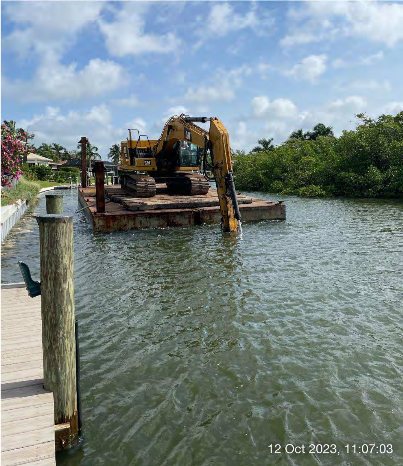
323 excavator grinding rock at station 7+00 in Canal Main B.
