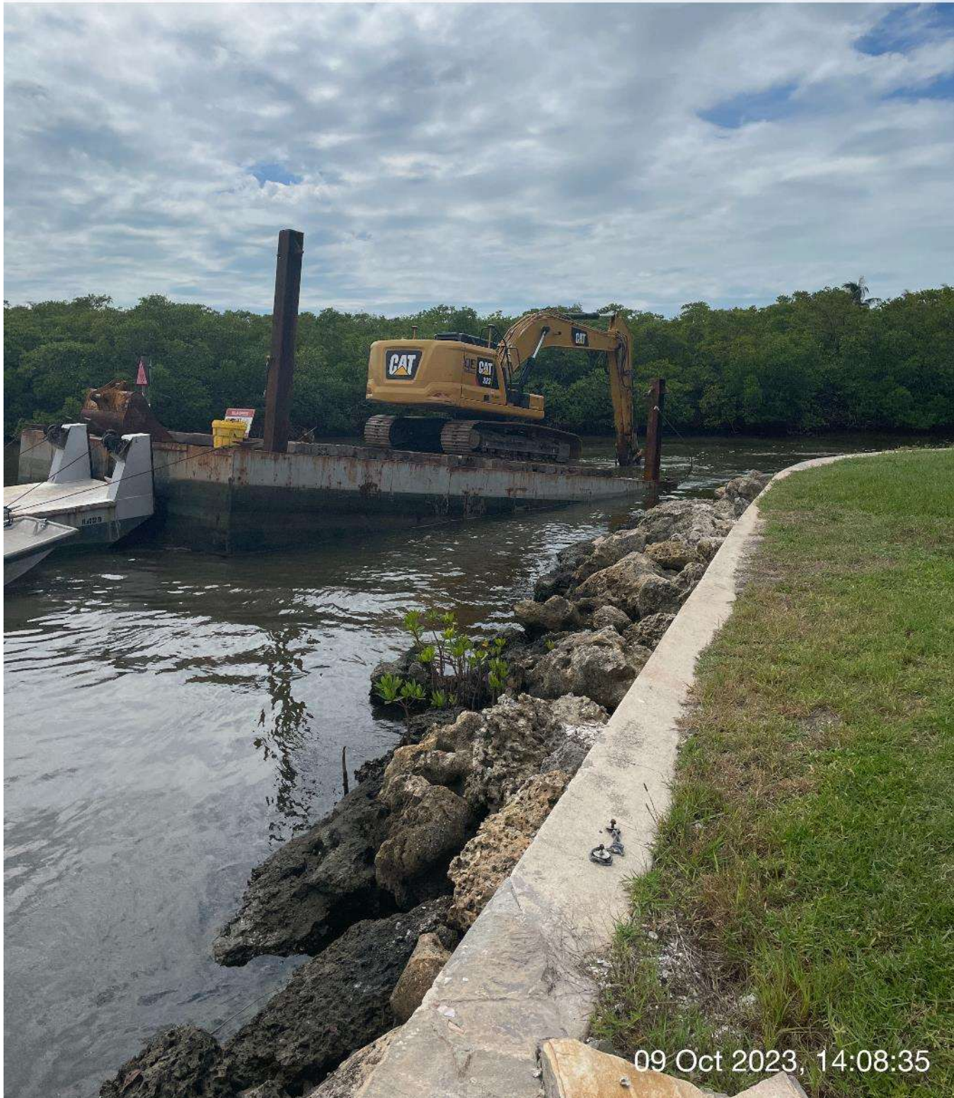
323 excavator grinding rock at station 2+50 in Canal Main B1.
