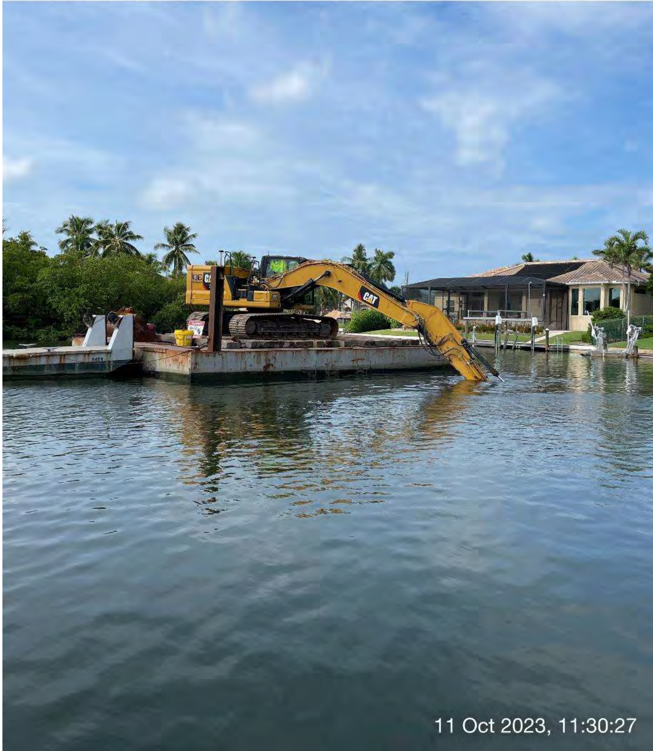
323 excavator grinding rock at station 0+50 in Canal Main B1.
