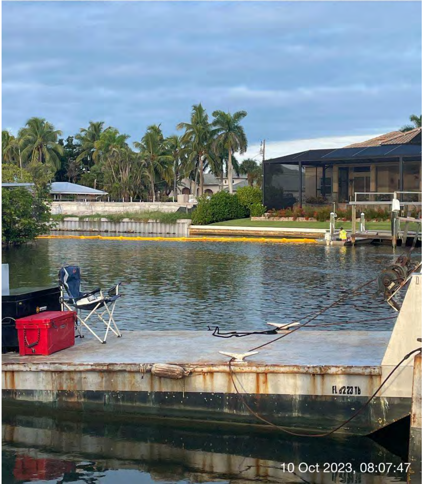
Turbidity curtain in place at station 8+50 in Canal Main B.
