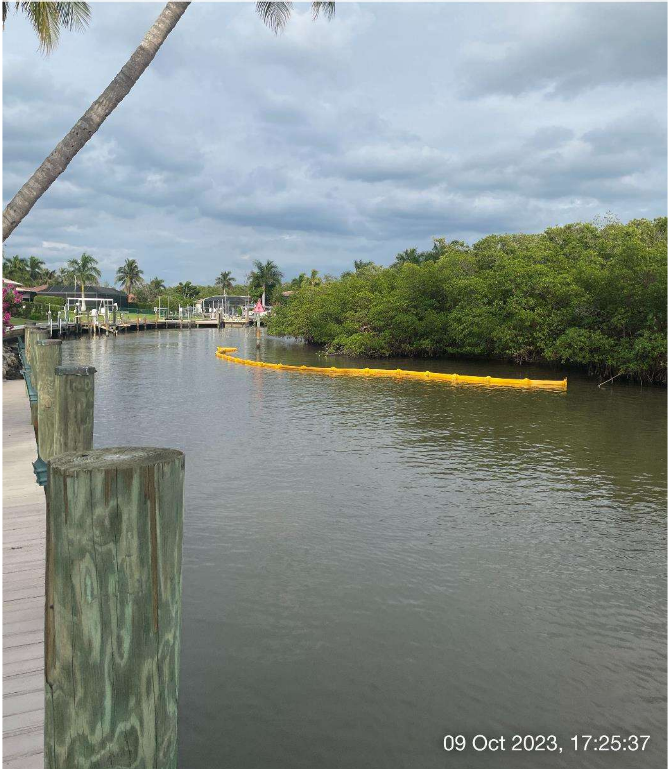
Turbidity curtain open at station 7+00 in Canal Main B.
