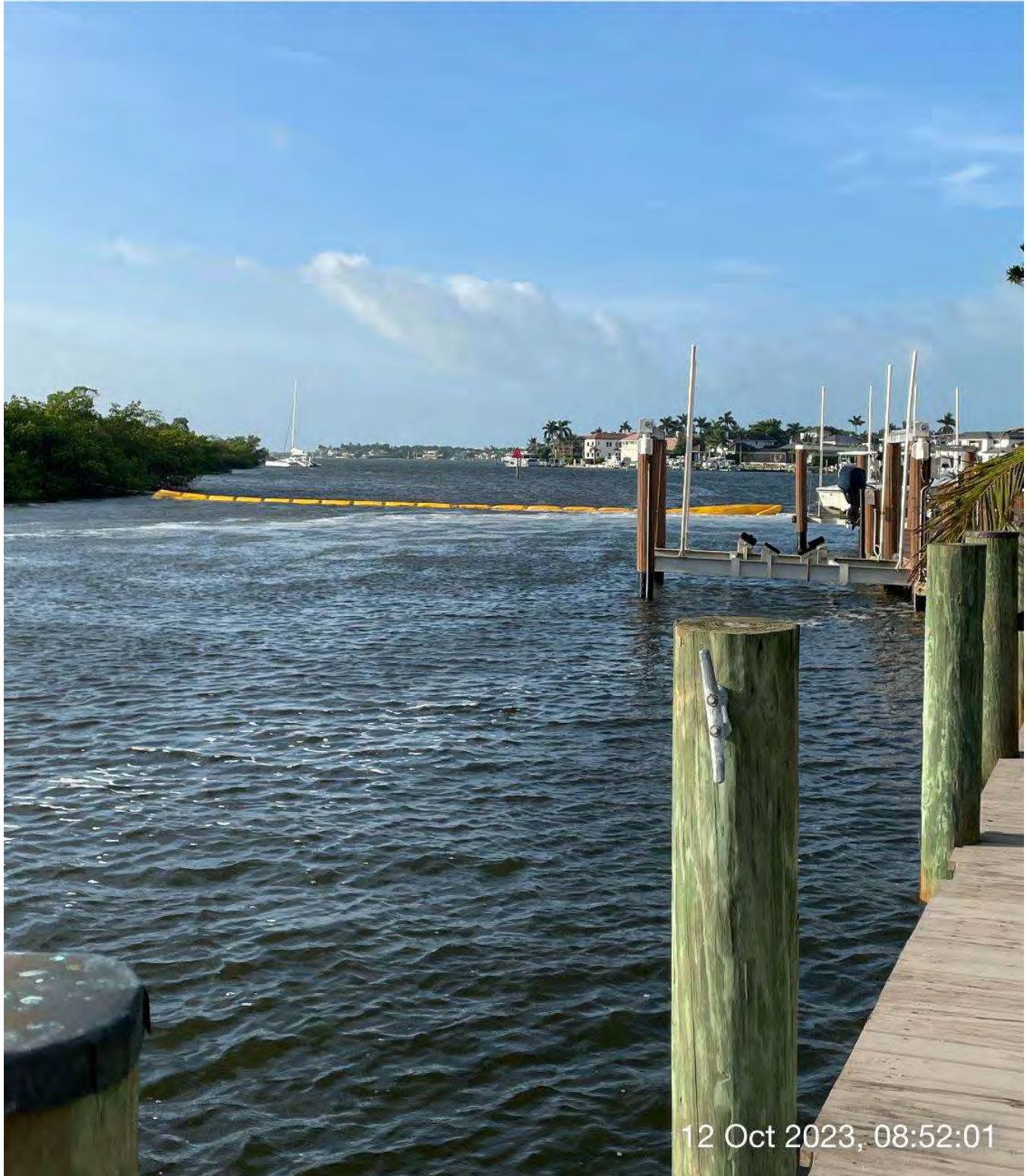
Turbidity curtain in place at station 4+00 in Canal Main B.
