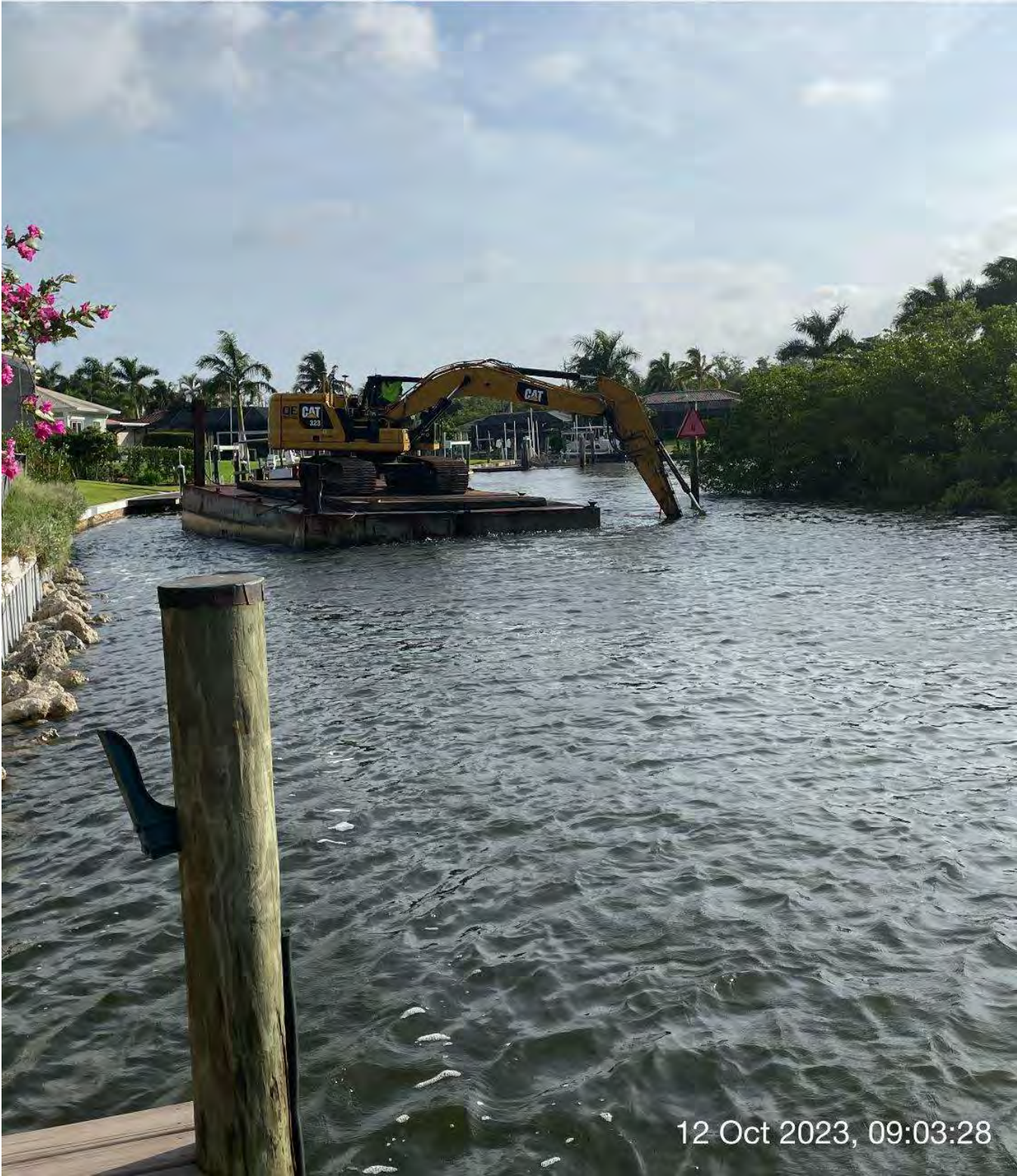
323 excavator grinding rock at station 8+00 in Canal Main B.
