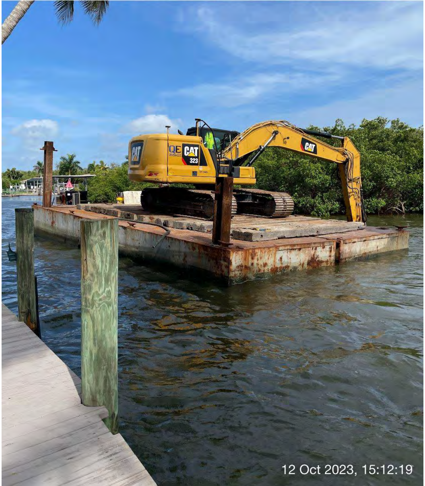
323 excavator grinding rock at station 6+50 in Canal Main B.
