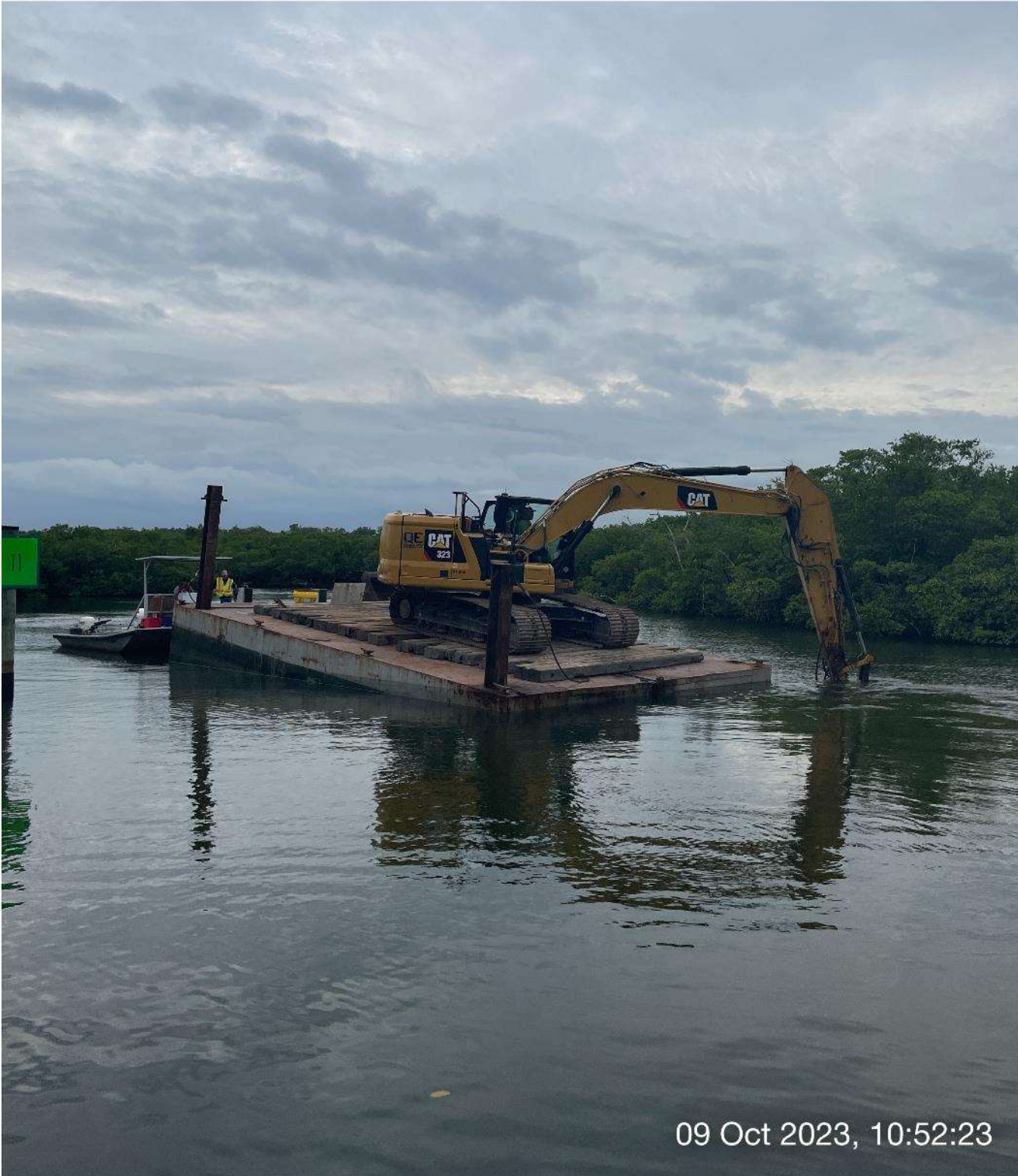
323 excavator grinding rock at station 4+00 in Canal Main B1.
