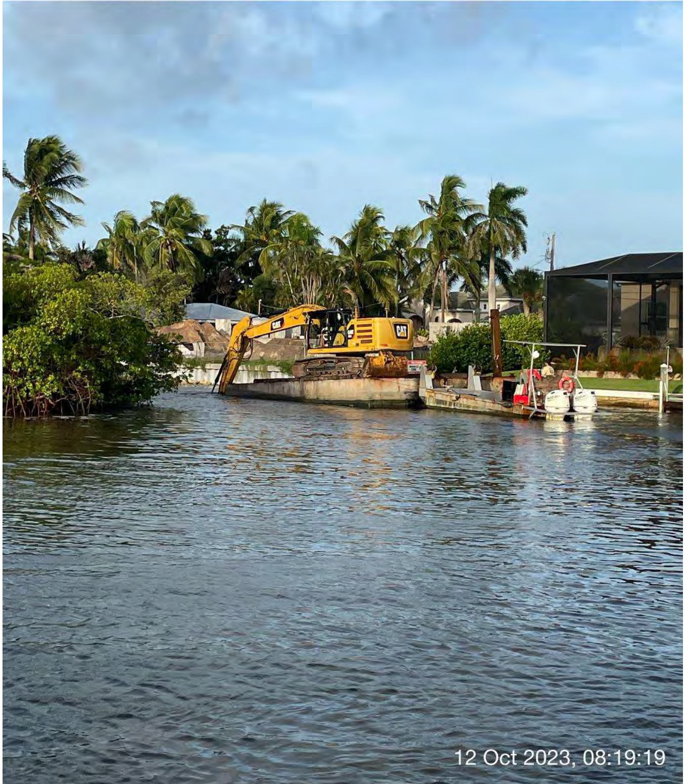
323 excavator grinding rock at station 8+50 in Canal Main B.
