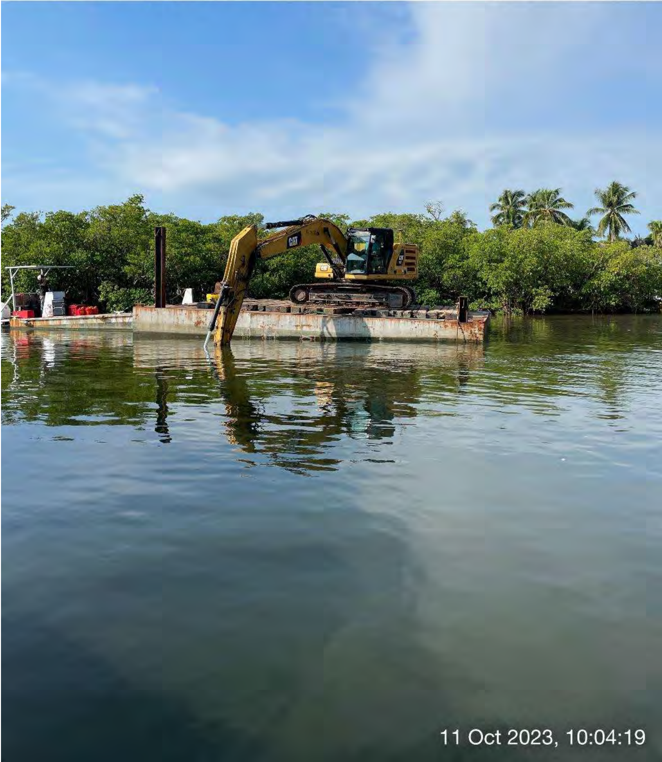
323 excavator grinding rock at station 1+00 in Canal Main B1.
