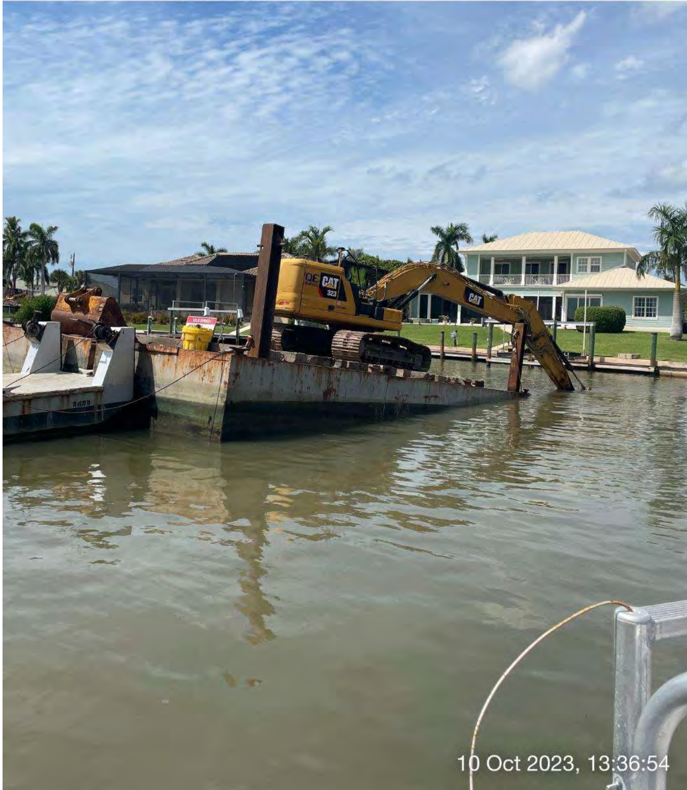
323 excavator grinding rock at station 9+50 in Canal Main B.
