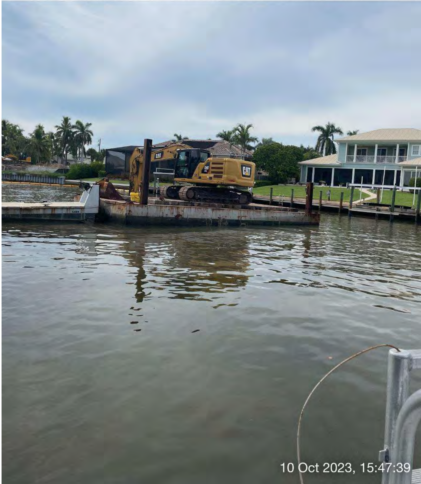
323 excavator grinding rock at station 9+00 in Canal Main B.
