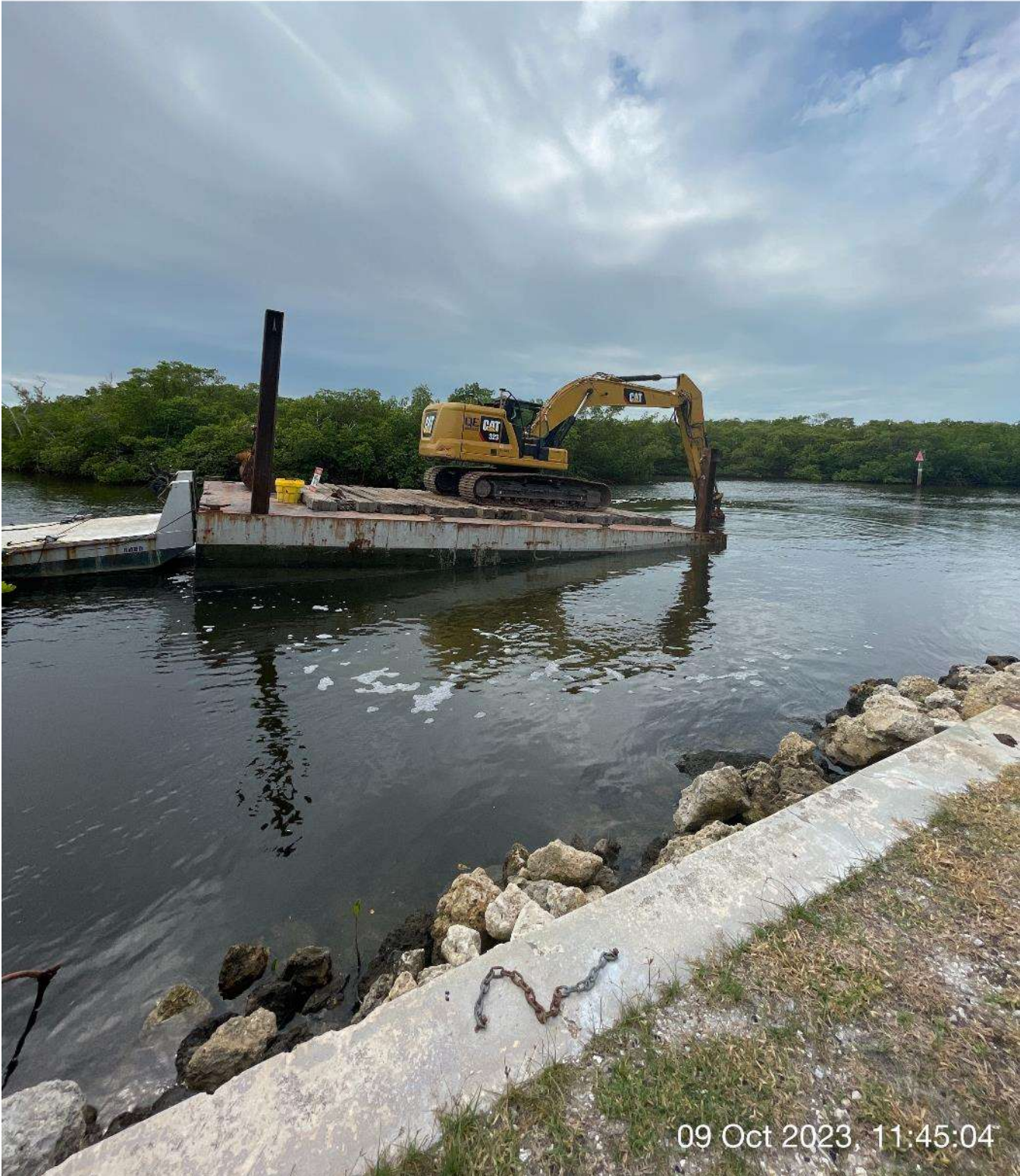
323 excavator grinding rock at station 3+50 in Canal Main B1.
