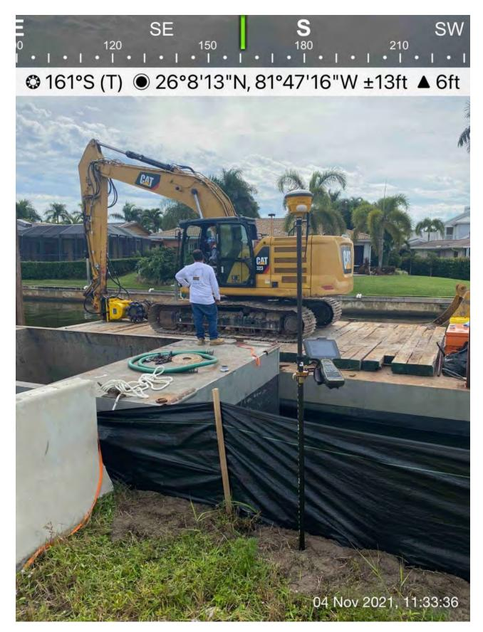
• 326 excavator removing material from Canal CC-CC around station 1+50 and moving sediment to dewatering site on the empty lot at 1300 Curlew Avenue.
