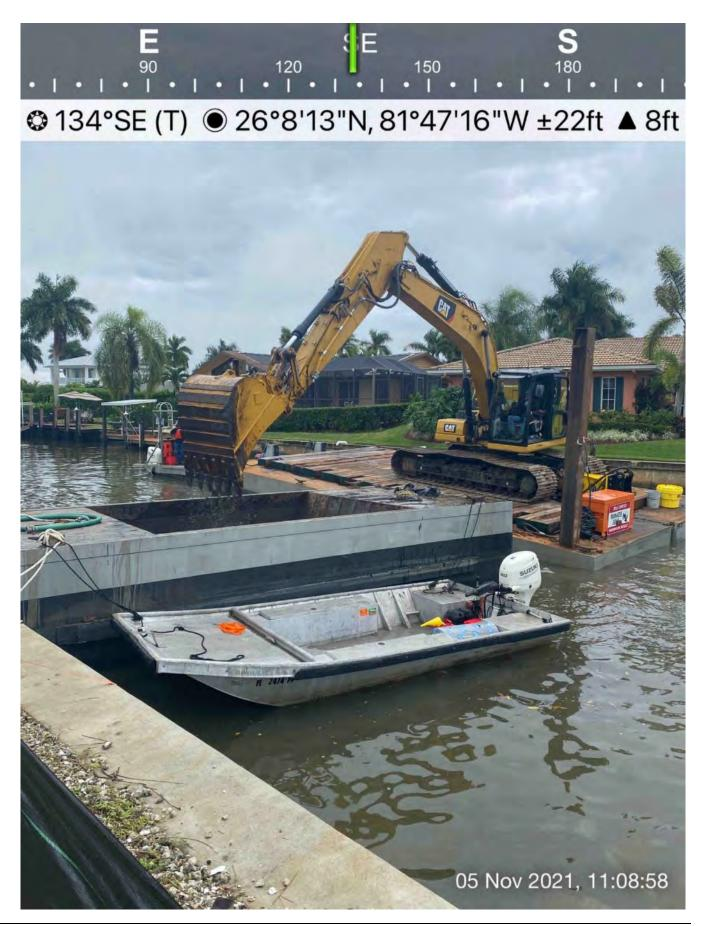
• 323 excavator lifting spud to move barge and 326 excavator holding the turbidity curtain.
