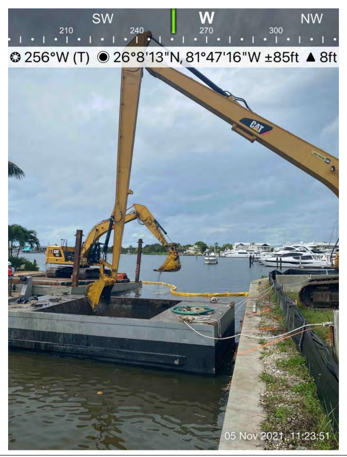
• Support boat holding turbidity curtain out so that 323 excavator can remove material near station 1+00.
