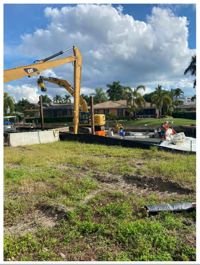
• Push boat moving barge with 323 excavator lifting spud to allow mobility near station 01+50.
