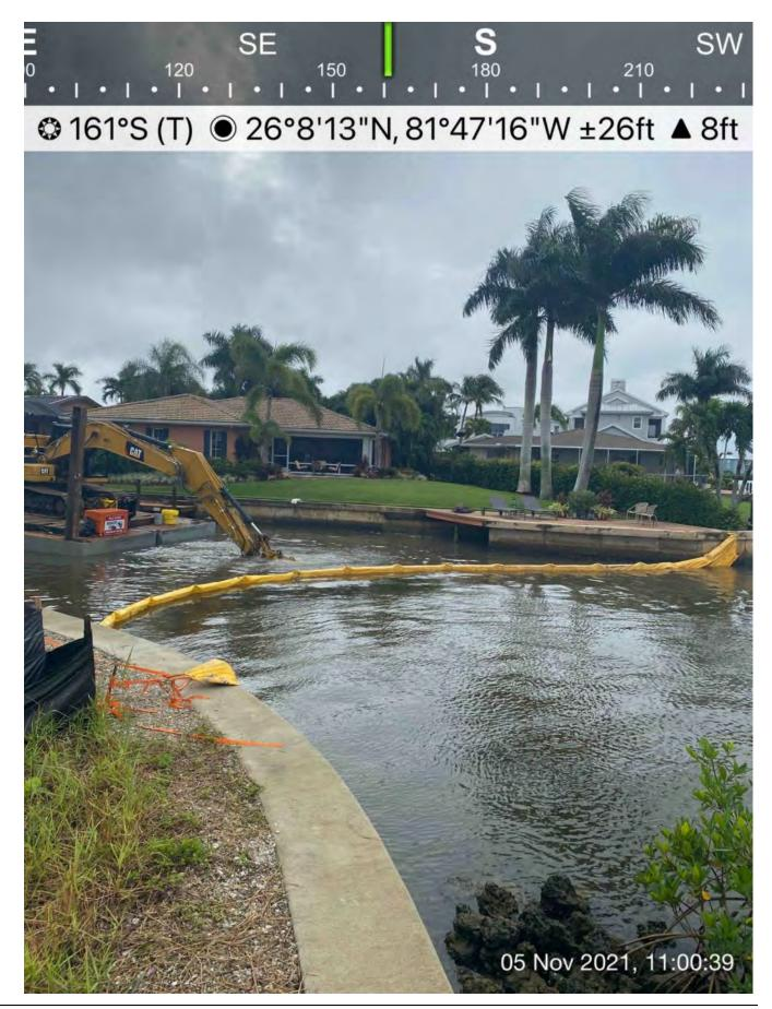
• 323 excavator removing material from station 1+00 and transferring into the hopper.
