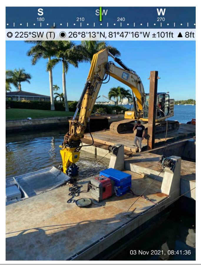
326 excavator removing material and transferring from hopper to dewatering site and 323 excavator grinding rock.
