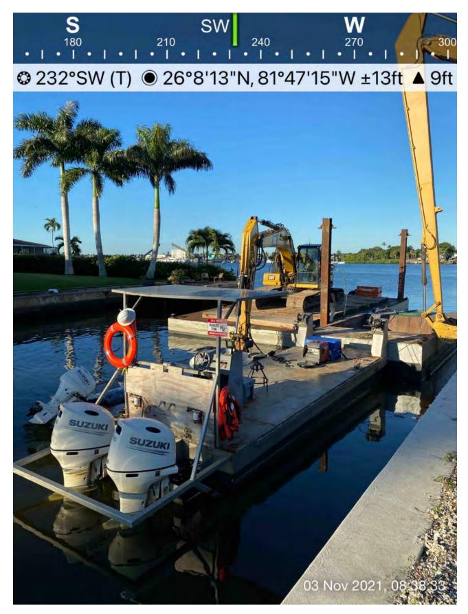
• 323 excavator grinding rock in Canal CC-CC near station 1+50.
