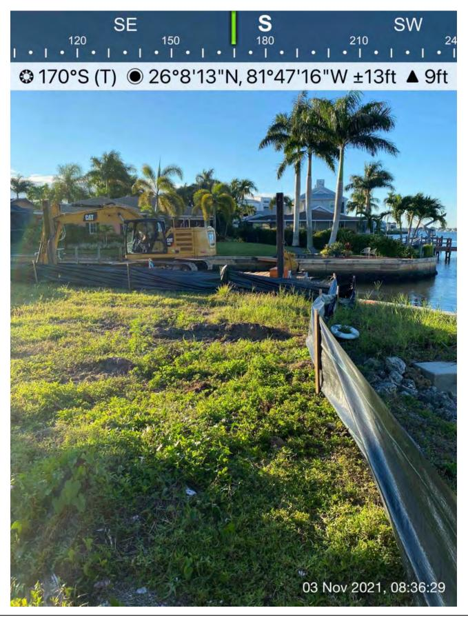
• 323 excavator with Epiroc grinder, push boat, hopper, and support boat in Canal CC-CC near station 1+50.
