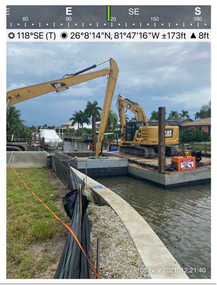
• 326 excavator transferring material from the hopper to the dewatering site on the empty lot at 1300 Curlew Avenue.
