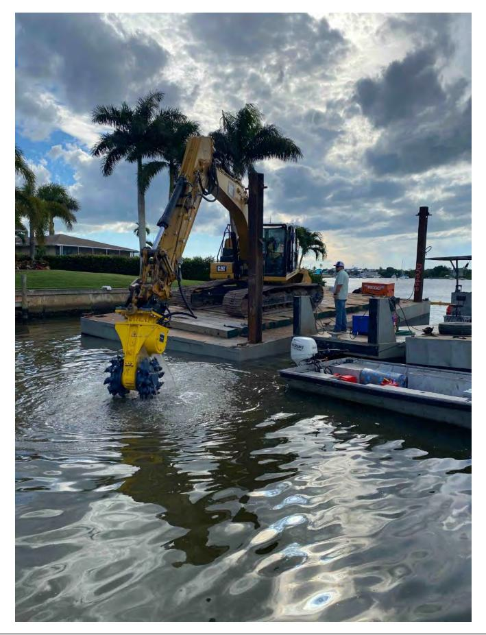
• 323 excavator with Epiroc cutter attachment grinding rock near station 01+50 and 326 excavator holding hopper in place.
