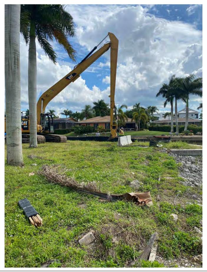
• Push boat mobilizing barge with 323 excavator lifting spud to allow mobility near station 01+50.
