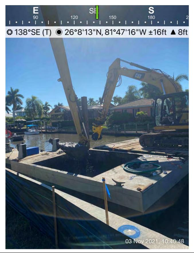
• 323 excavator, barge, push boat, support boat, and hopper as they were staged overnight from 11/2 to 11/3.
