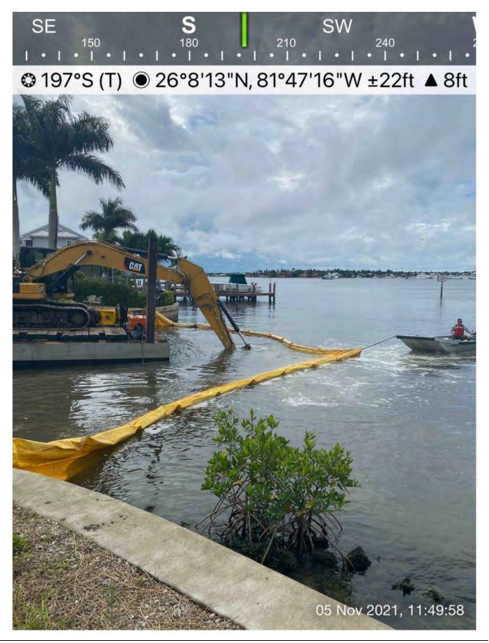
• 326 excavator holding the hopper in place while 323 excavator sits on the barge.
