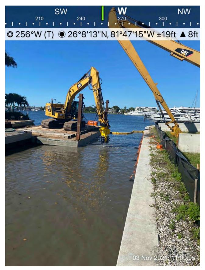
• 323 excavator grinding rock and 326 excavator transferring dredged material from hopper to dewatering site at the empty lot.
