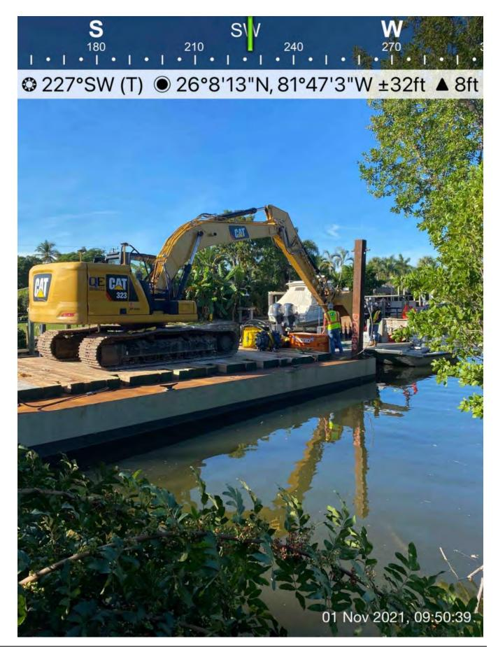
• 326 excavator on barge with Epiroc grinder.
