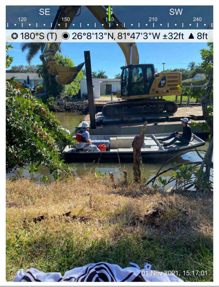
• 326 excavator with a full bucket about to dump sediment into the hopper.
