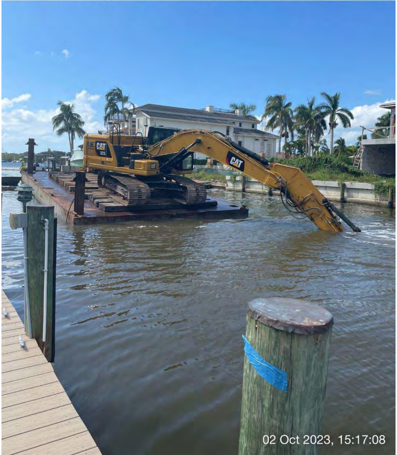
323 excavator removing sediment at station 3+00 in Canal X-X.
