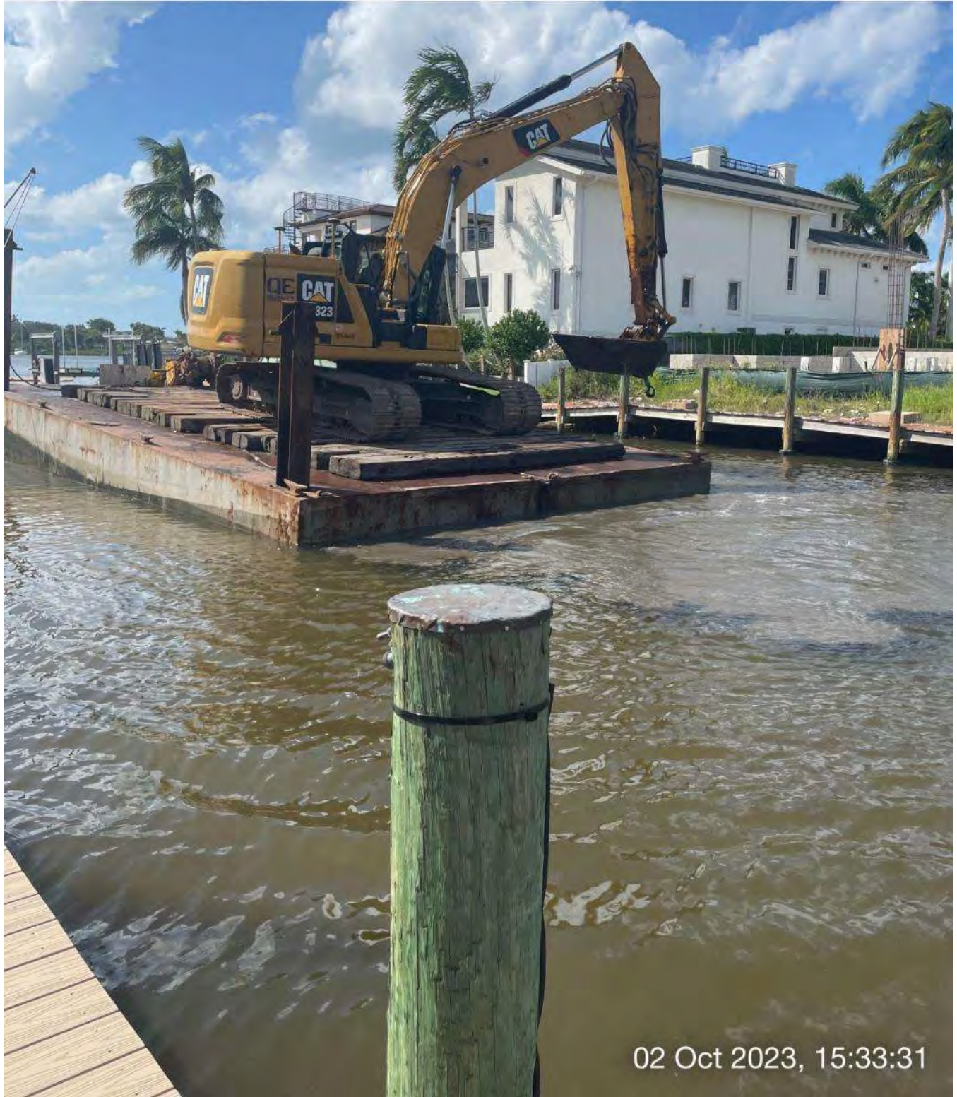
323 excavator removing sediment at station 2+50 in Canal X-X.
