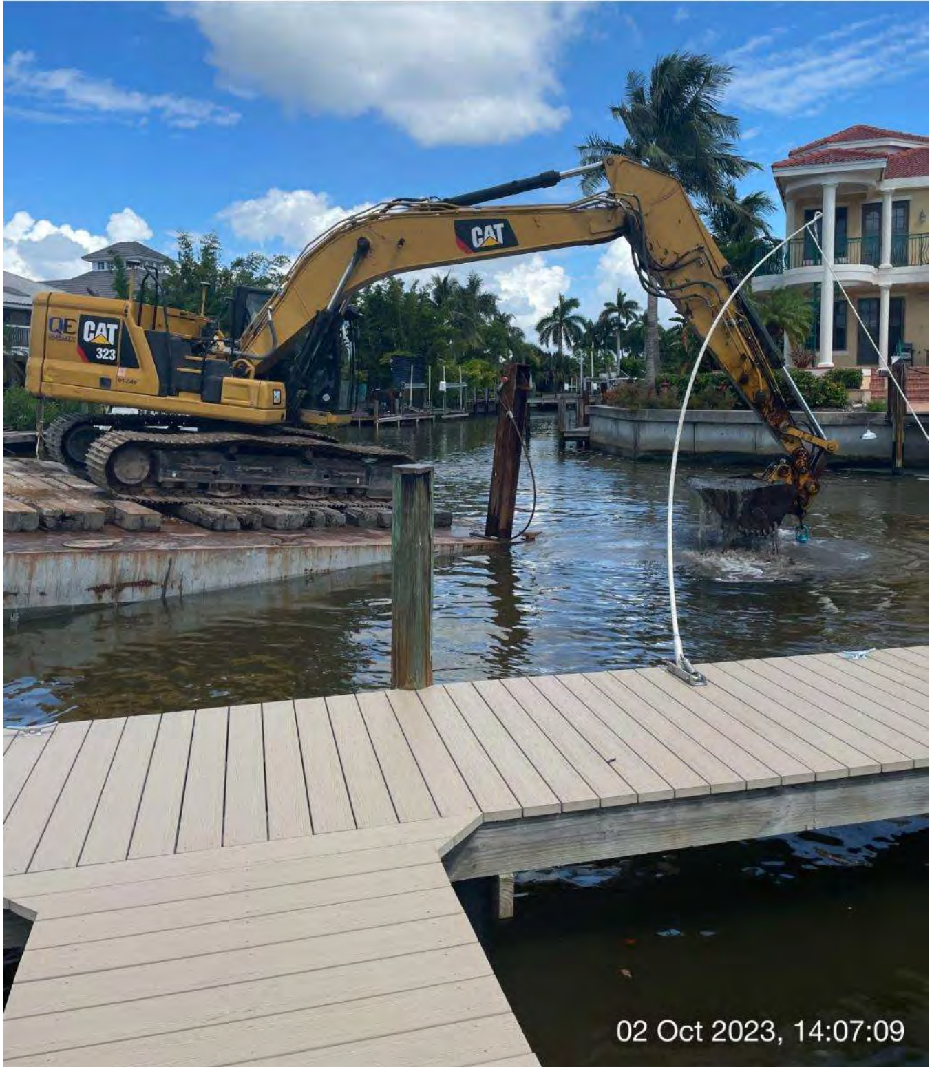
323 excavator removing sediment at station 0+50 in Canal Y-Y.
