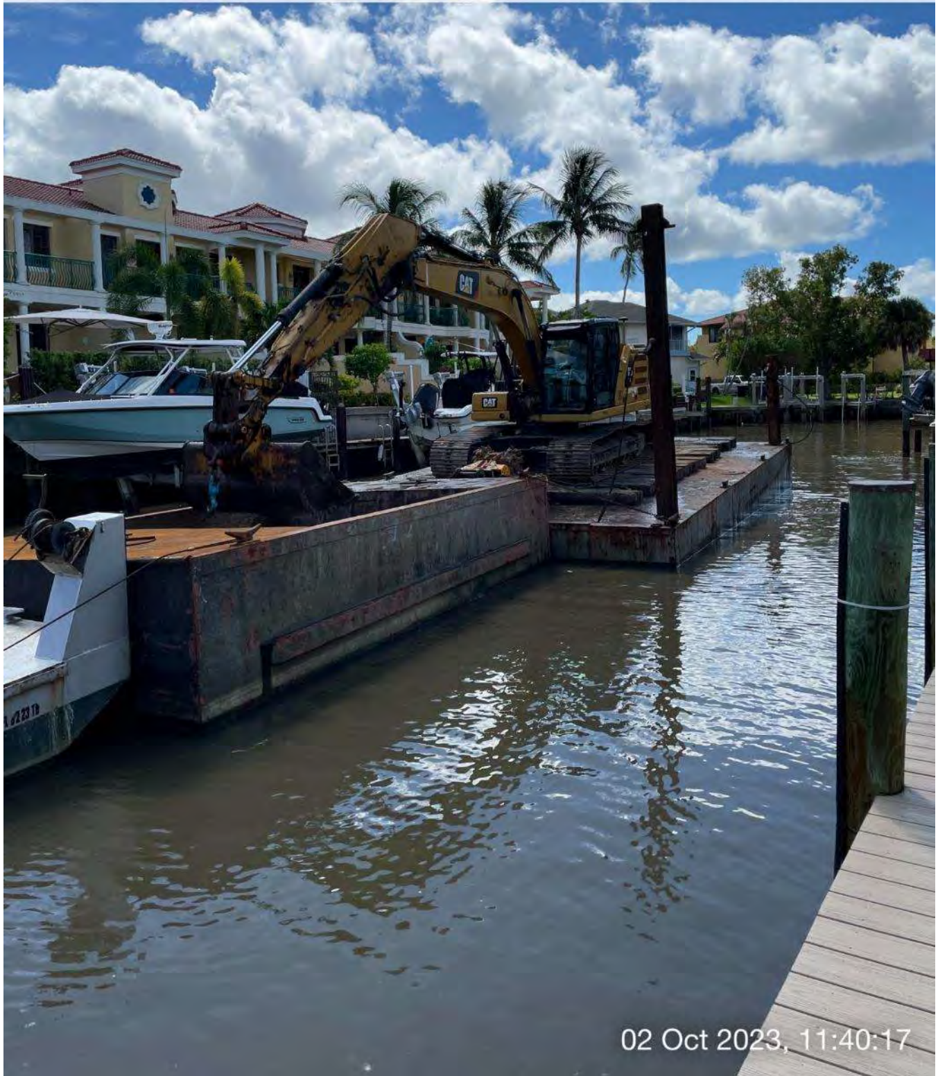
323 excavator removing sediment at station 2+50 in Canal Y-Y.
