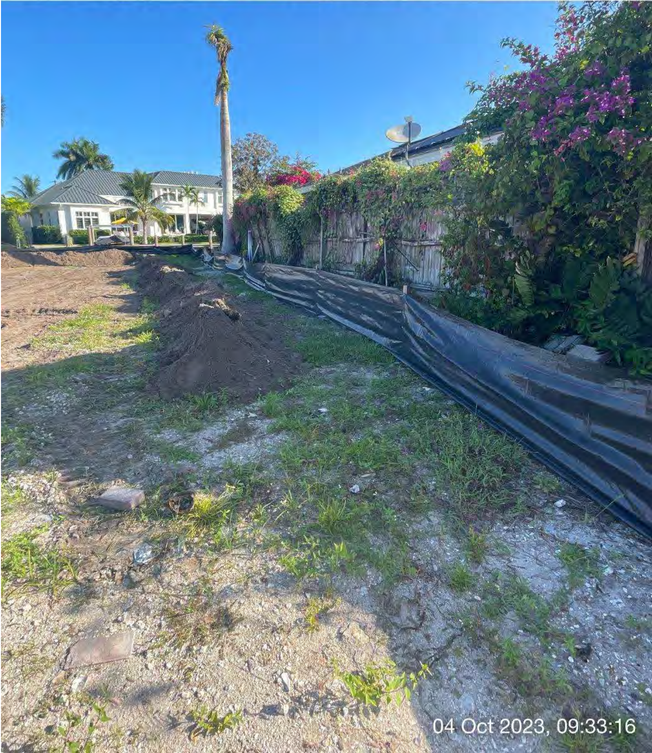
Silt fence at staging area.
