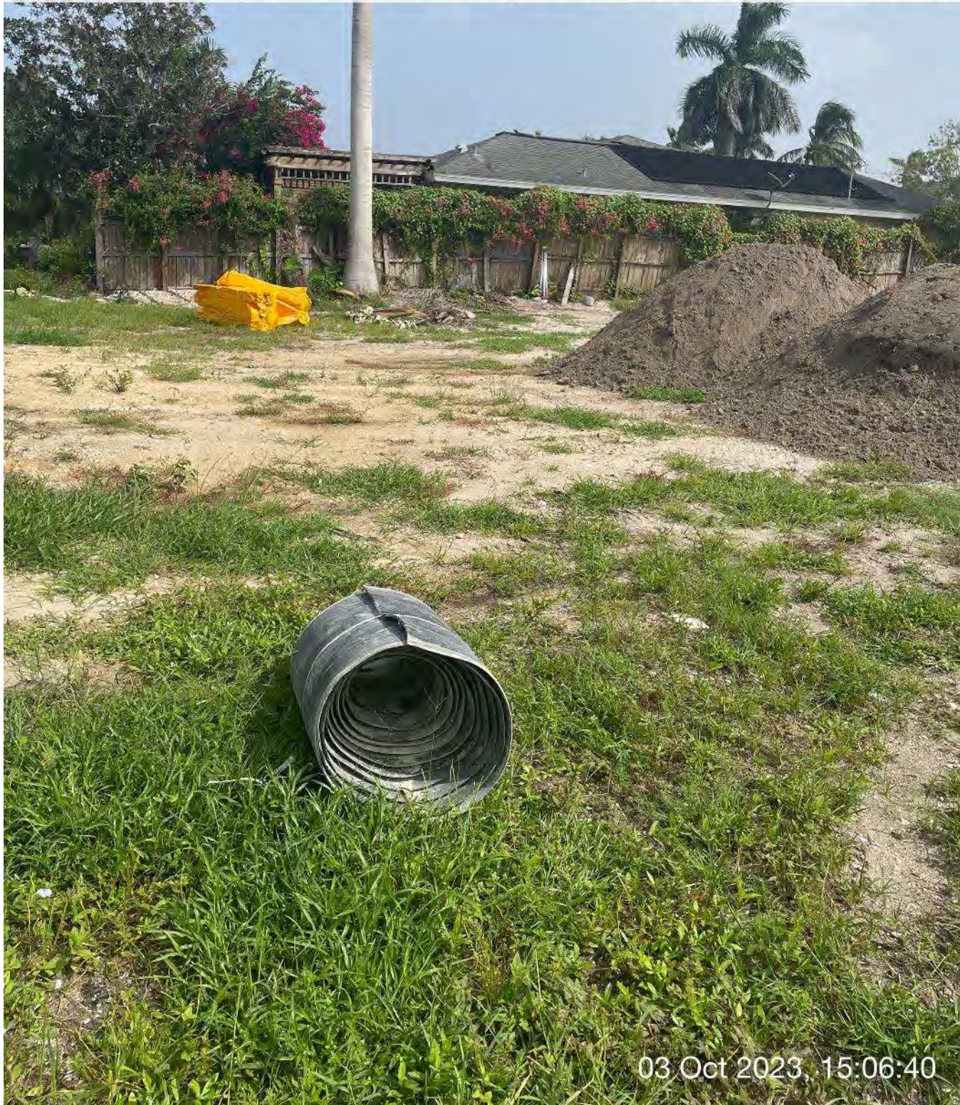
Material for silt fence at staging area at 1387 Marlin Drive.
