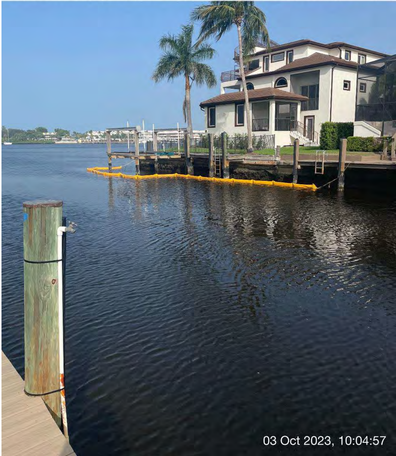
Turbidity curtain at station 1+00 in Canal X-X.
