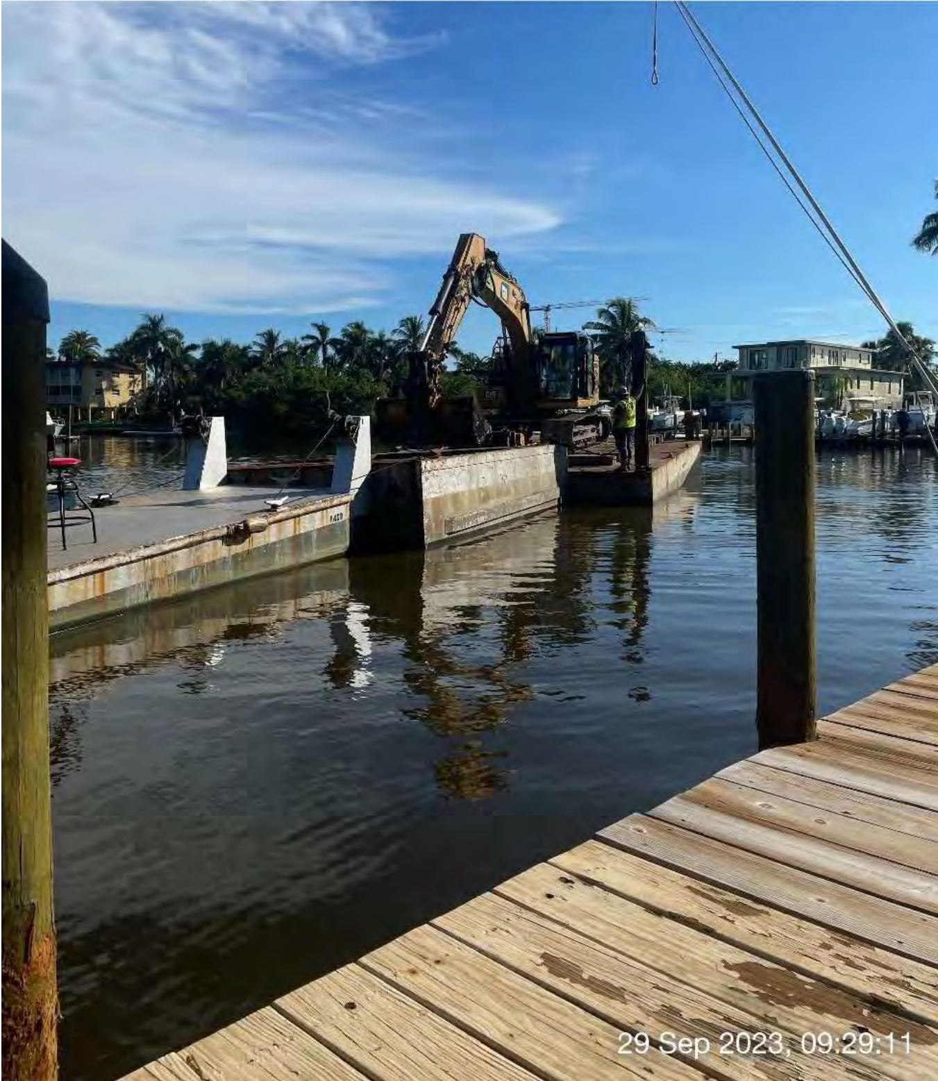
323 excavator removing sediment at station 13+00 in Canal X-X.
