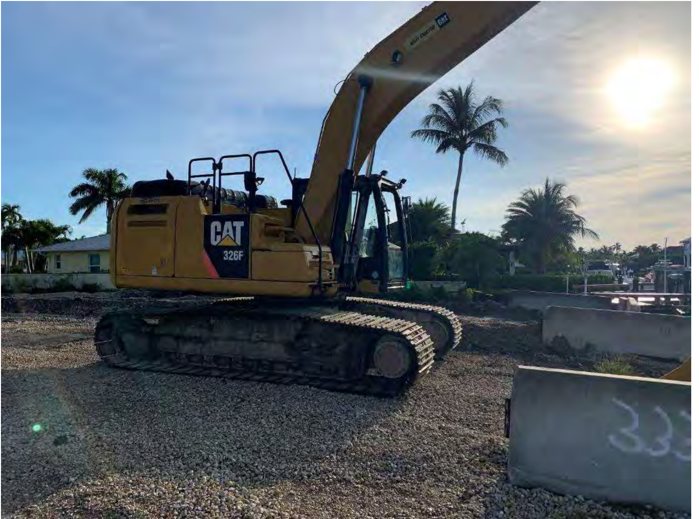
Long reach excavator at staging area.
