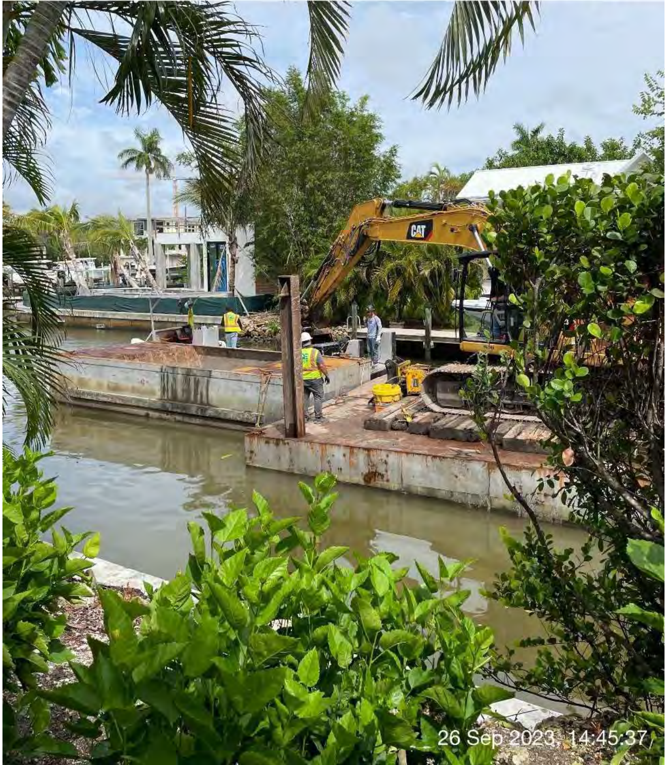
Dredging paused. Getting tools to grease equipment on the excavator.
