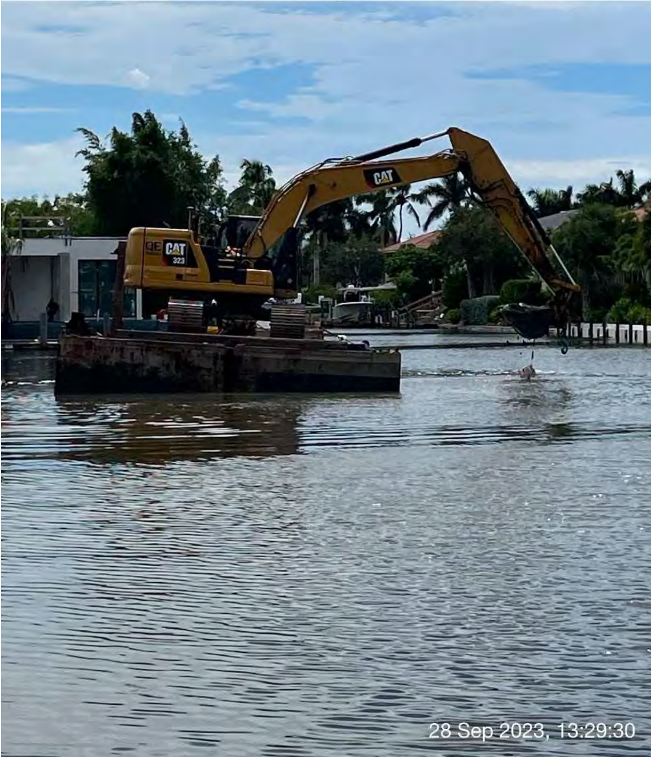
323 excavator removing sediment at station 14+50 in Canal X-X.
