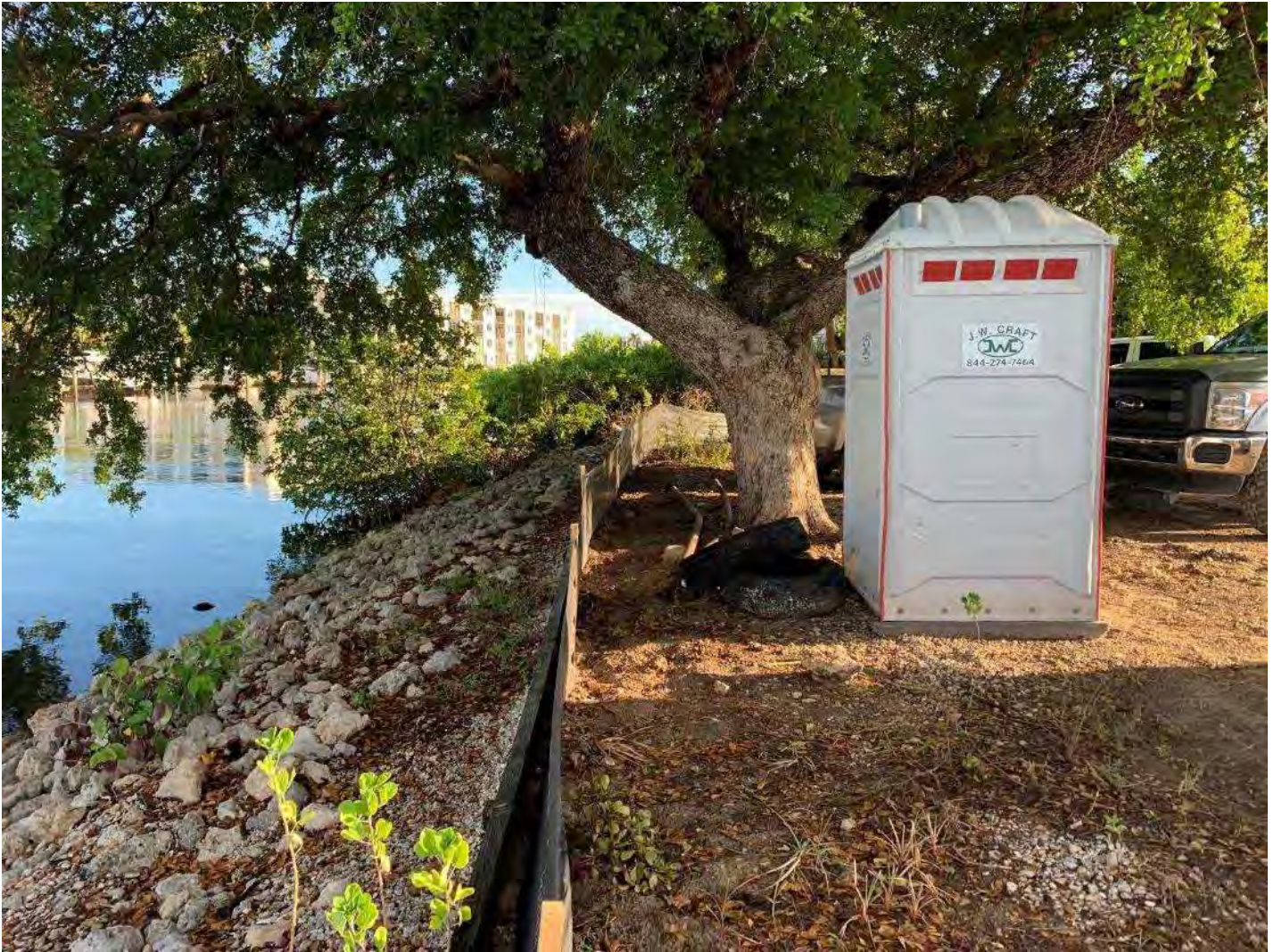
Silt fence in place at staging area.
