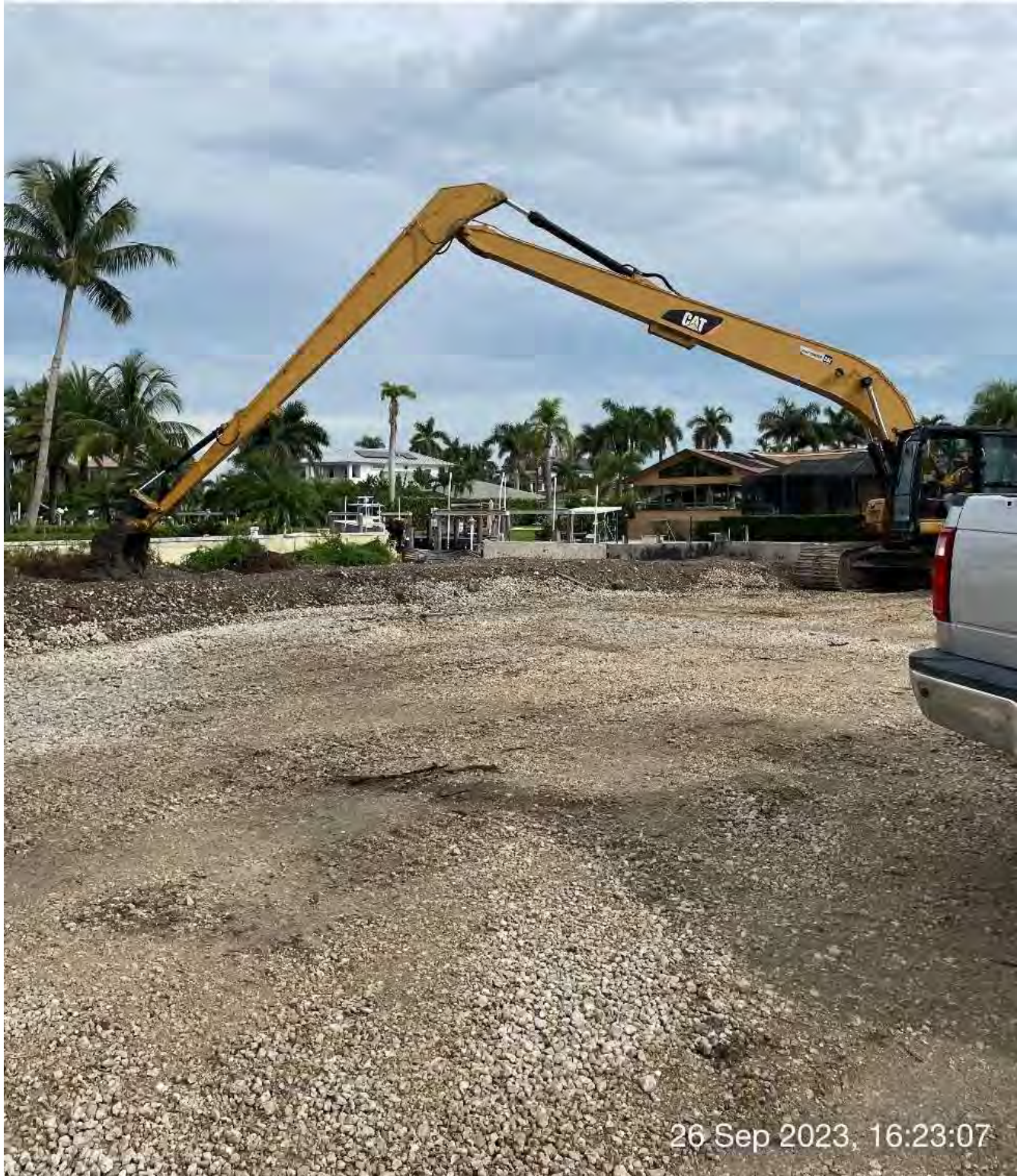
Unloading material from hopper onto the staging area.
