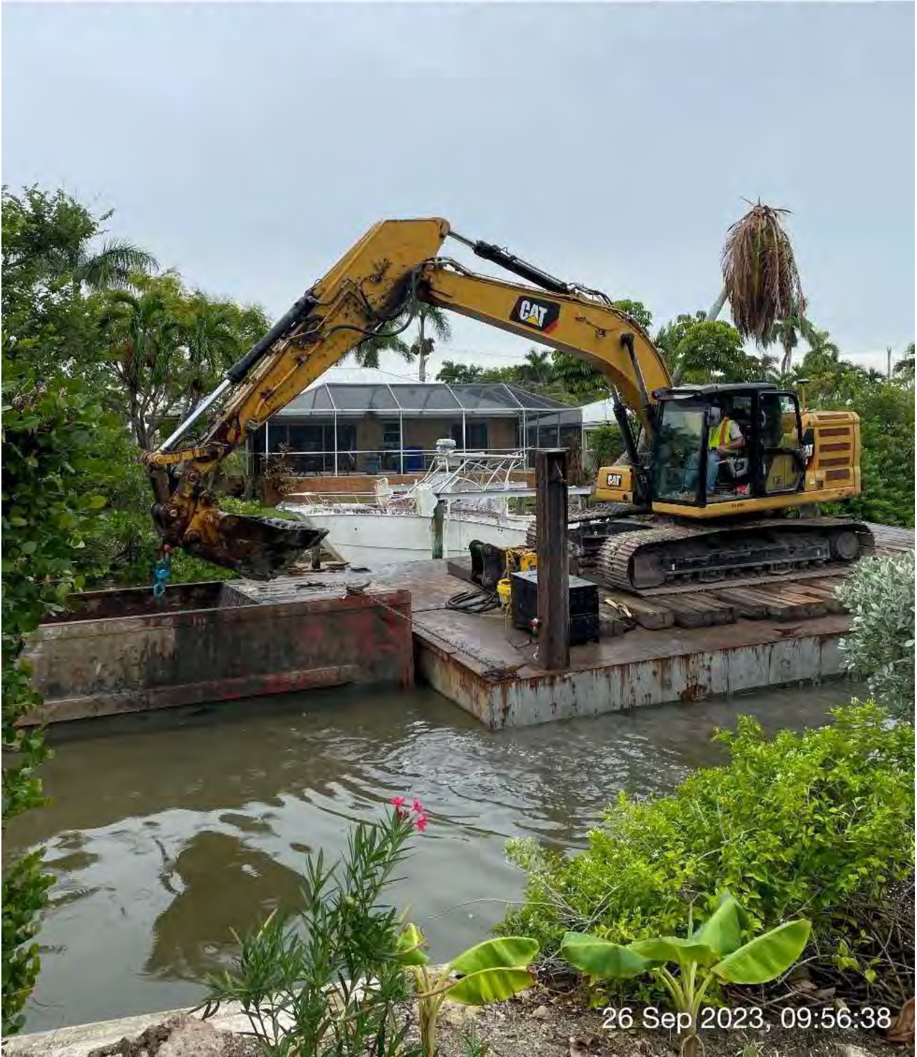
Removing sediment from station 2+50 and placing it in the hopper.
