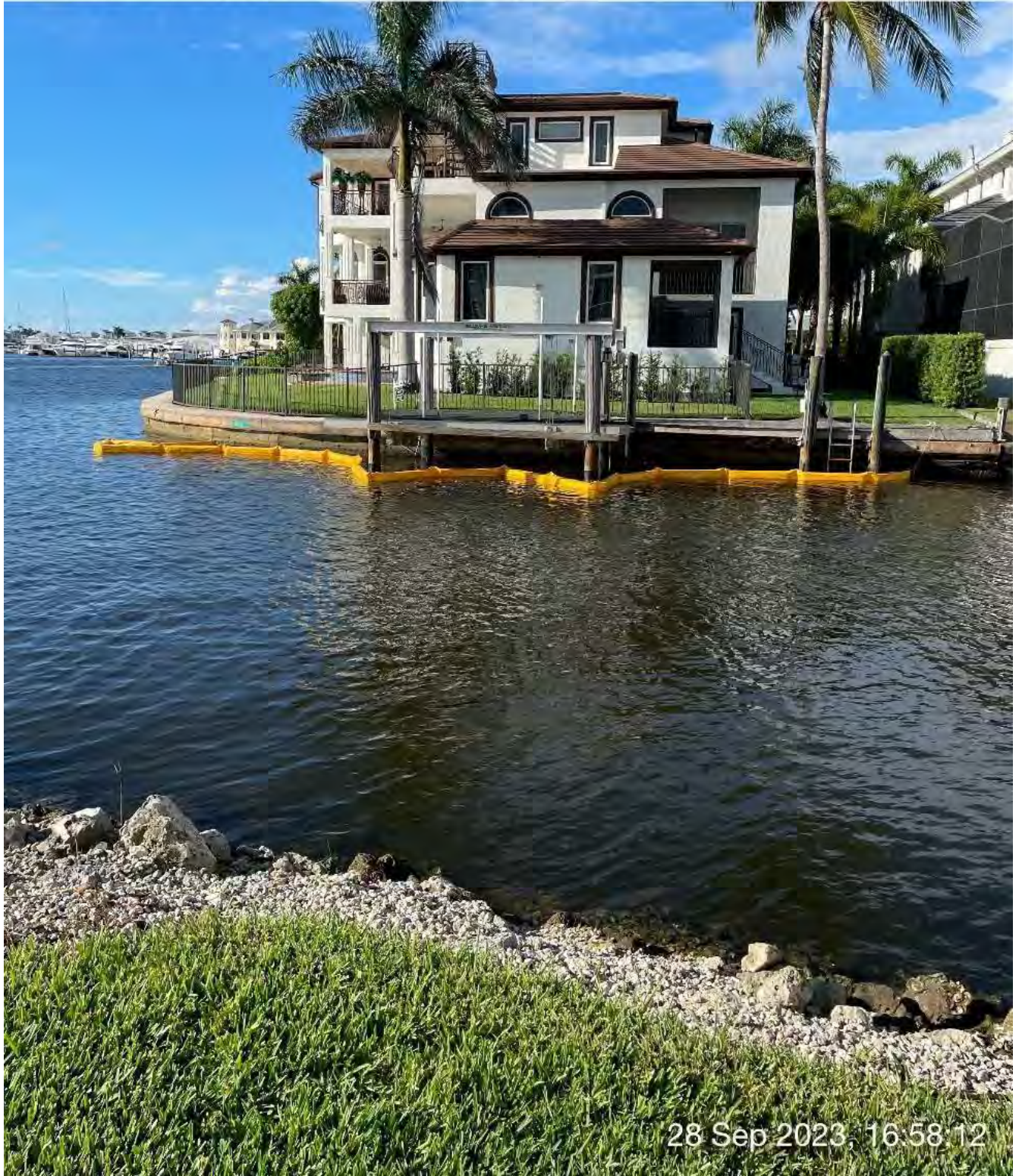
Turbidity curtain open at the end of the day at station 1+00 in Canal X-X.
