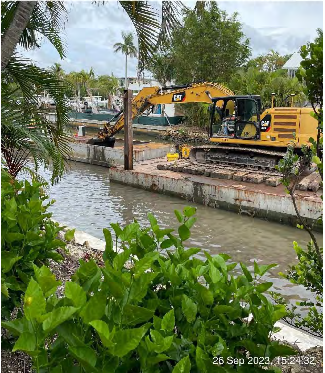
Placing dredge material from station 2+00 into the hopper.
