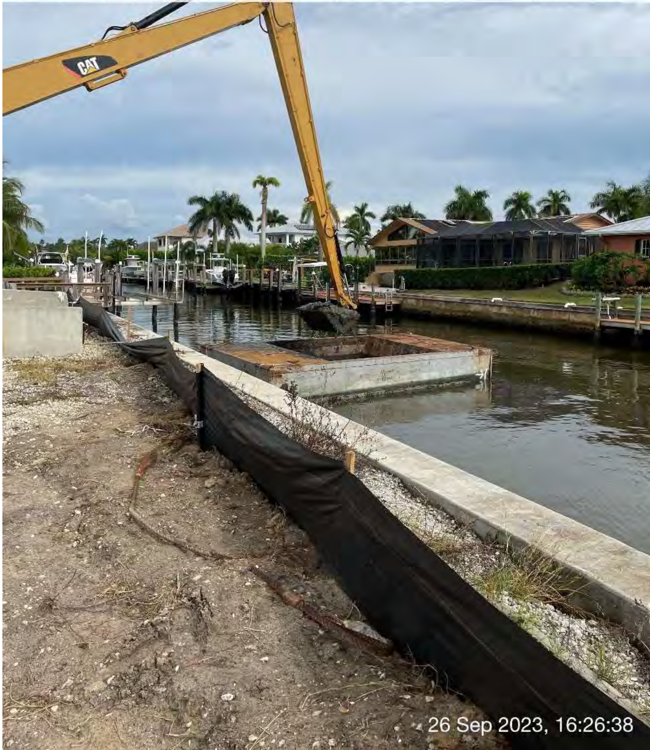
Removing material from the hopper to be placed onto the staging area.
