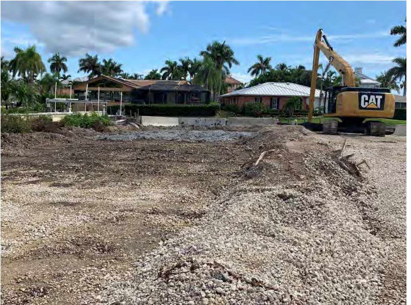
Material from Canal AA-AA being placed onto the staging area.
