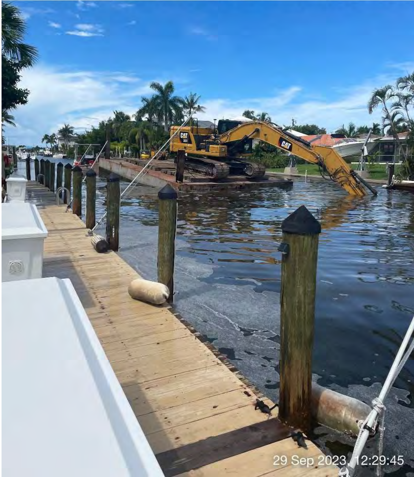
323 excavator removing material at station 10+00 in Canal X-X.
