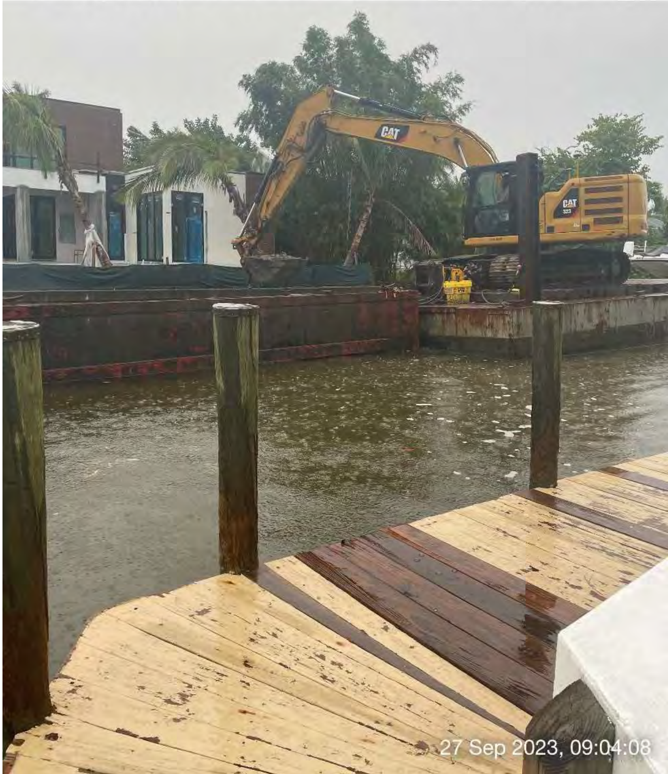
Contractor placing dredge material into hopper from station 1+50 in Canal AA-AA.
