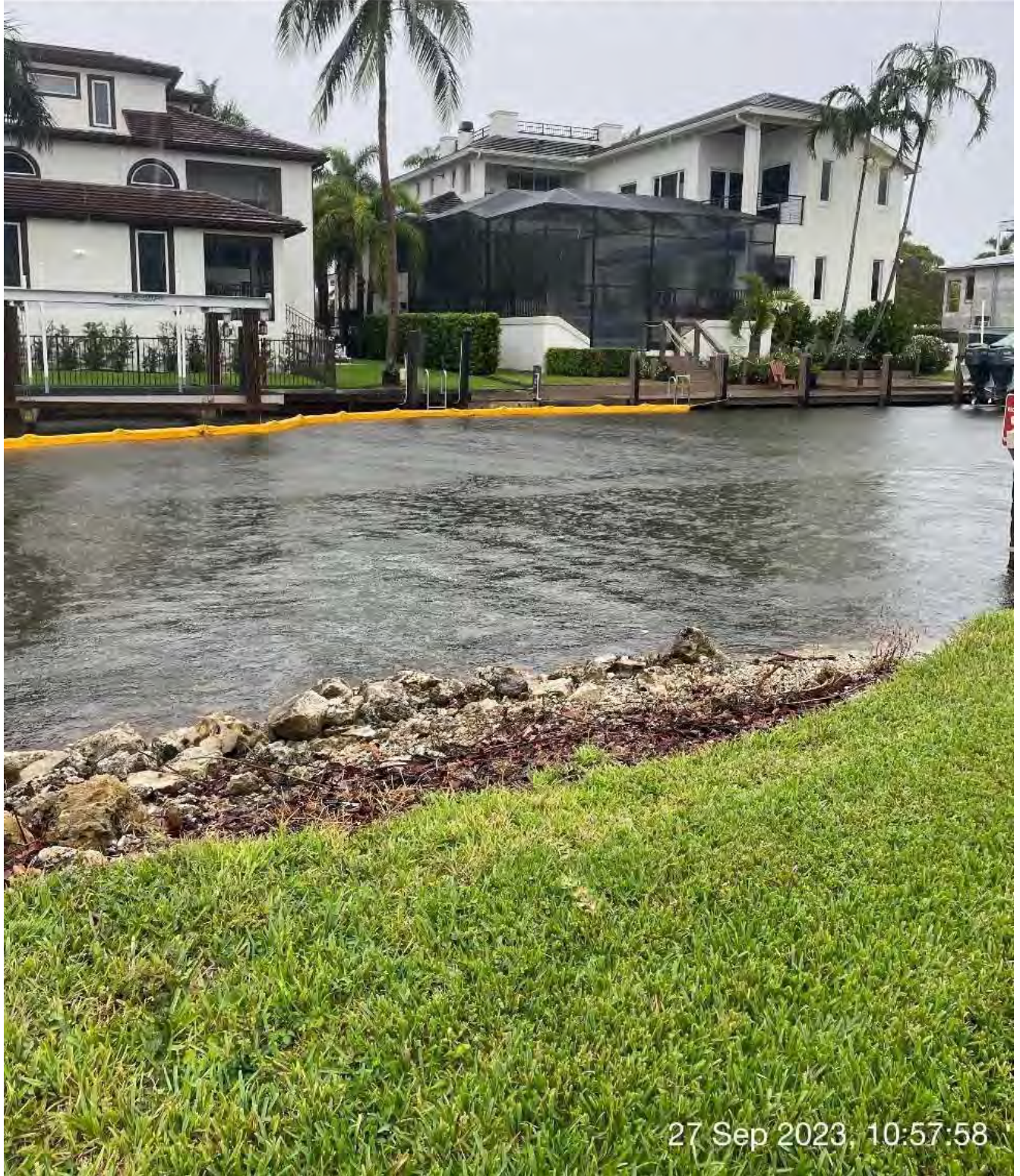
Turbidity curtain open at the end of the day in Canal X-X.
