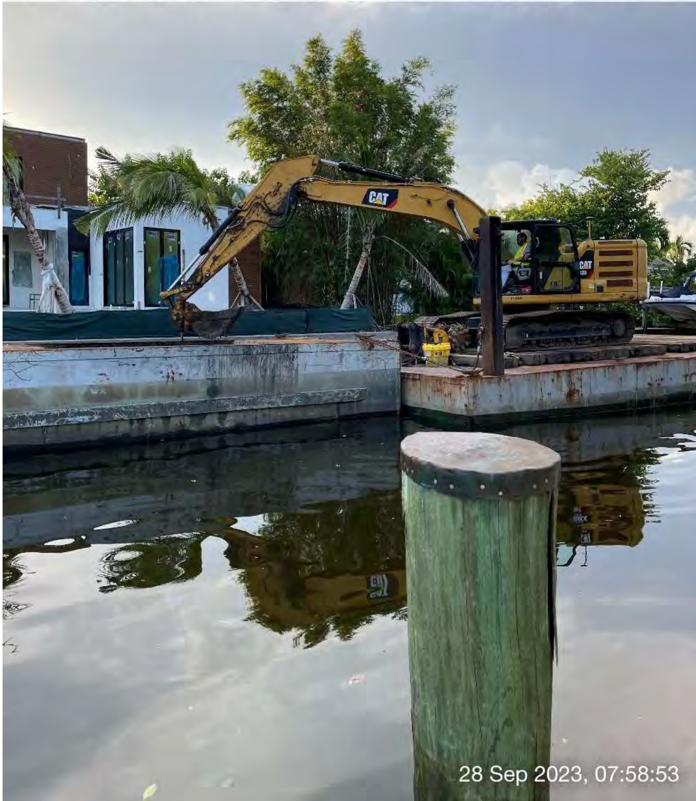
323 excavator removing sediment from station 1+00 in Canal AA-AA.
