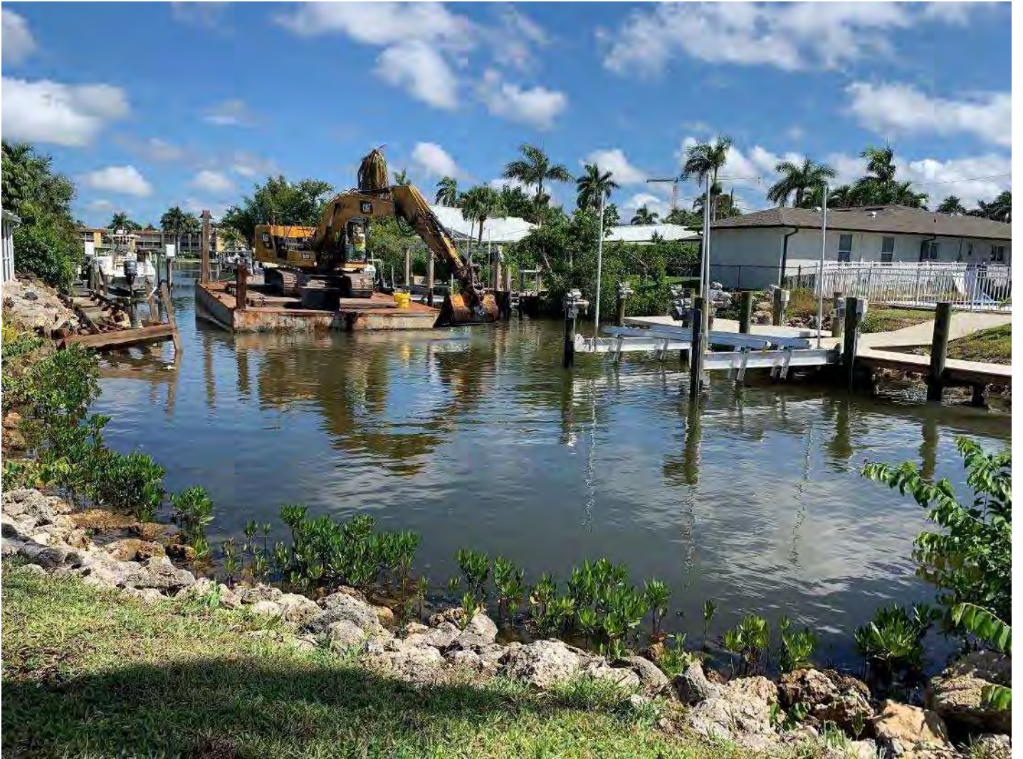
Contractor removing sediment at station 4+00 in Canal AA-AA.
