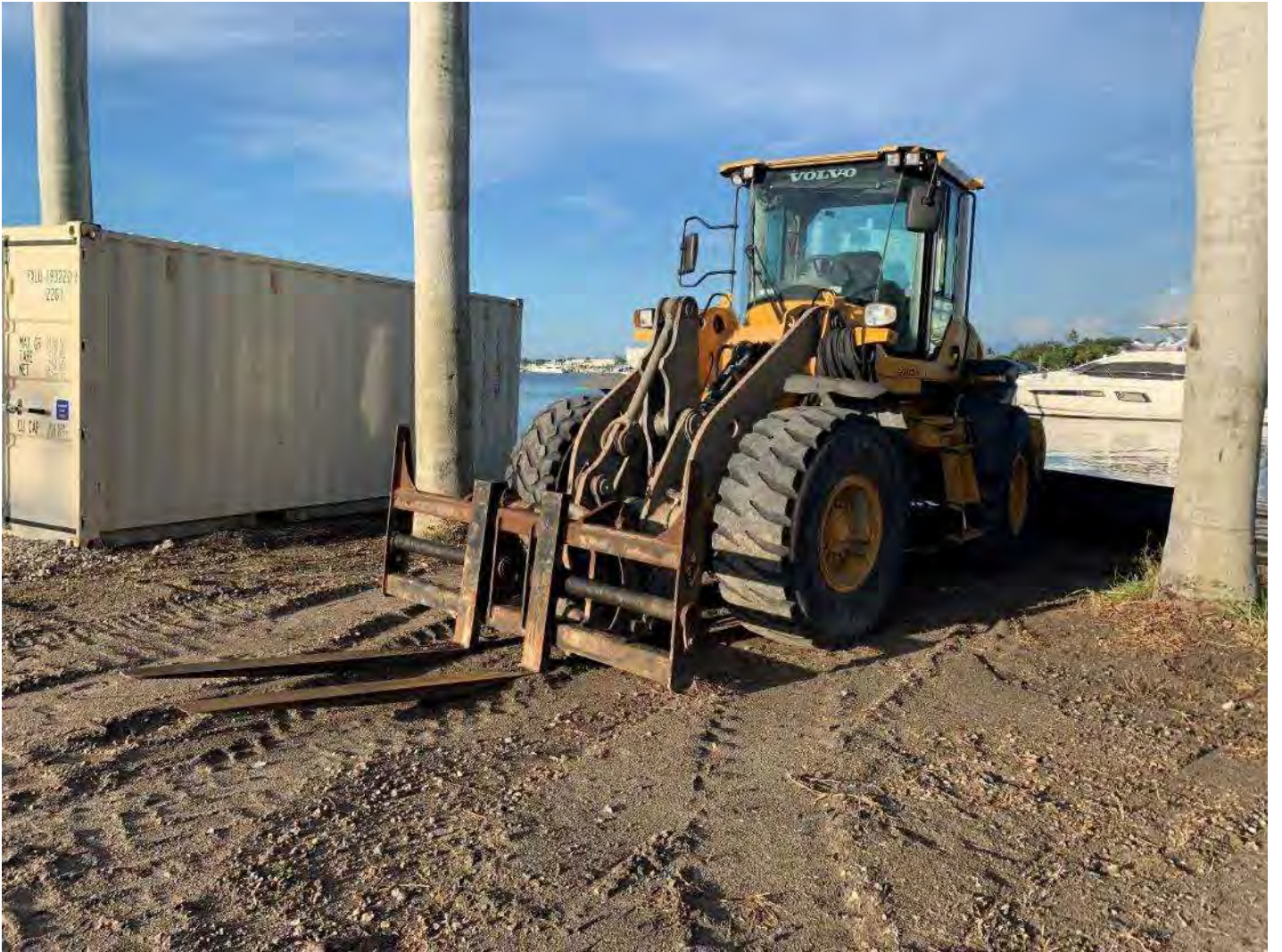
Front end loader at staging area.
