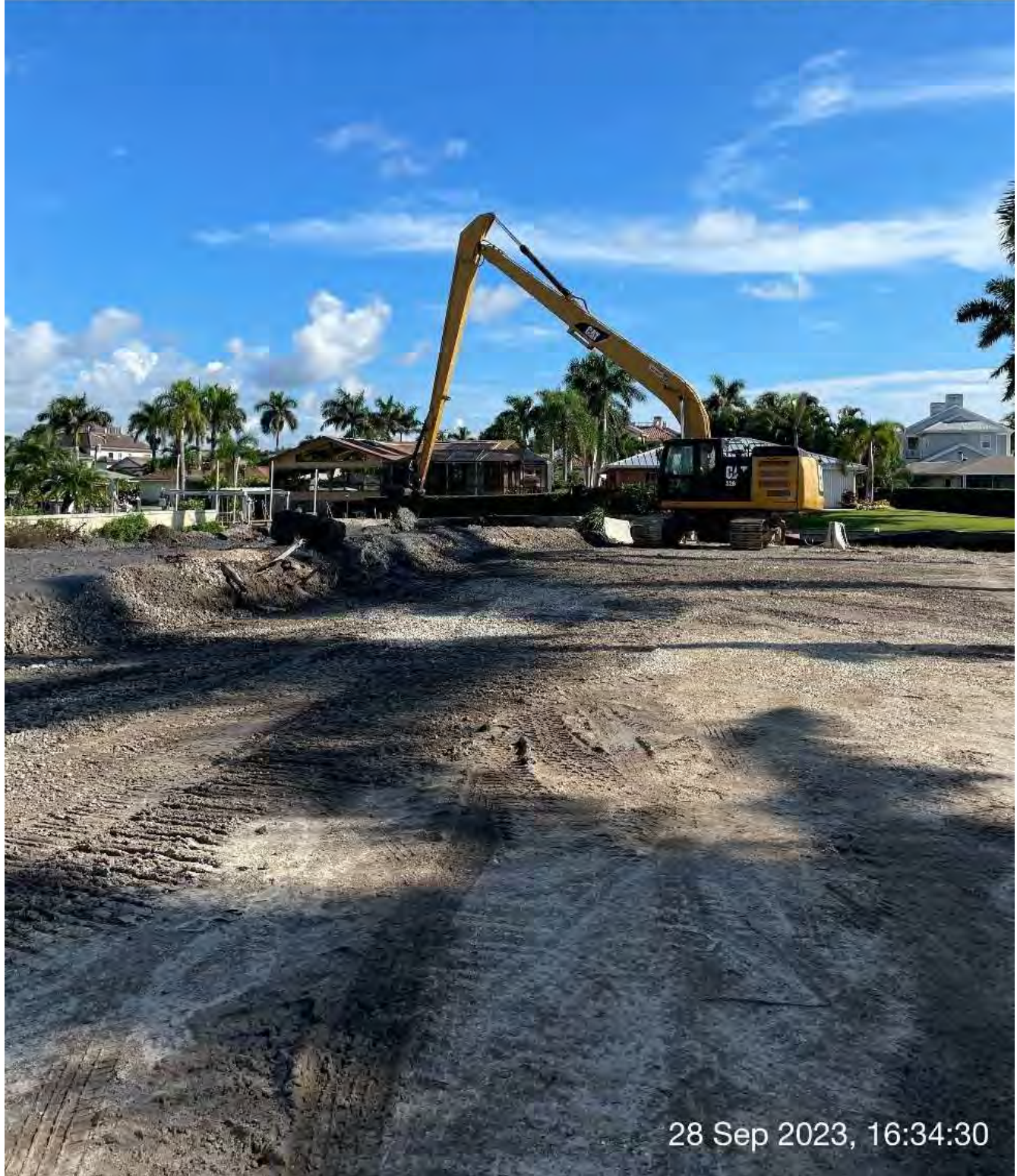
Long reach 326 excavator unloading material from 4 th hopper of the day.
