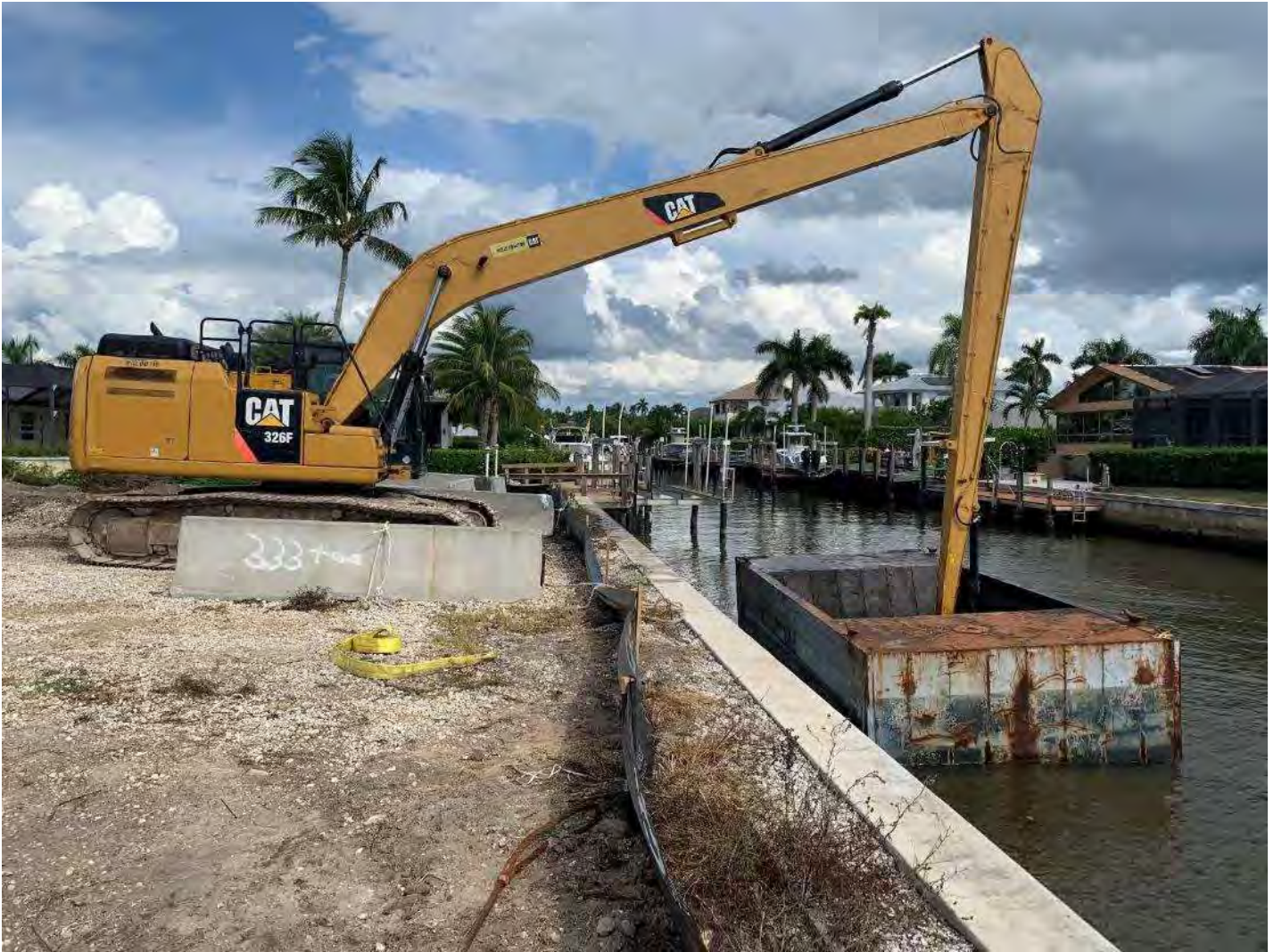
Unloading dredged material from hopper onto staging area.
