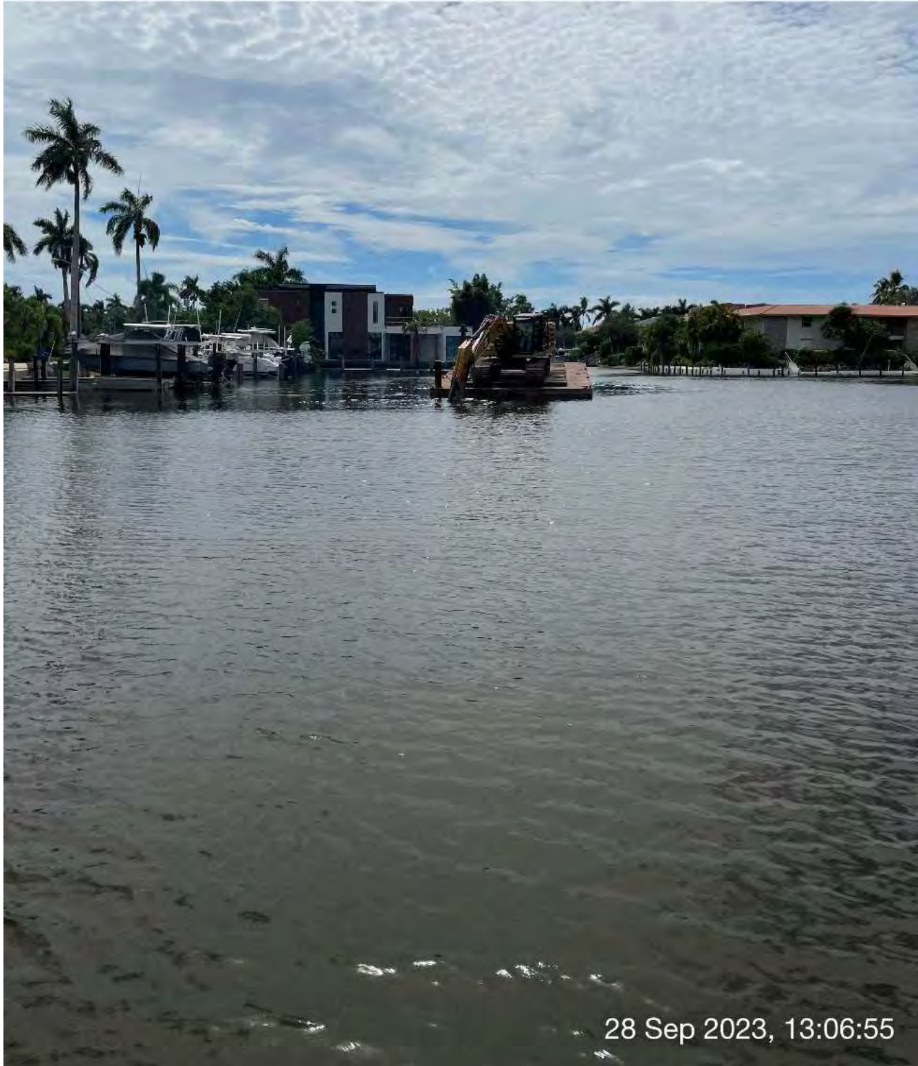
323 excavator removing sediment at station 15+00 in Canal X-X.
