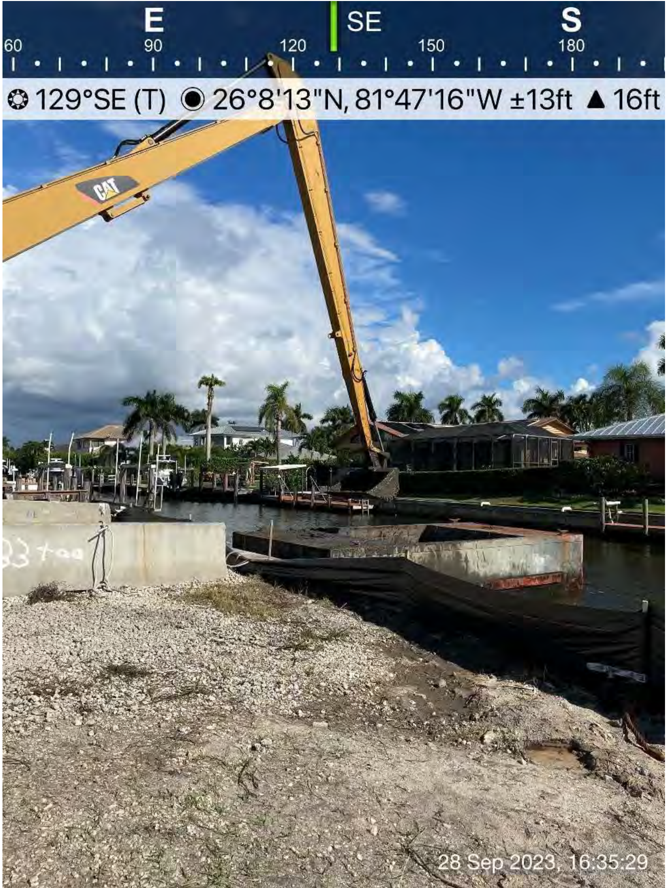
Long reach 326 excavator unloading material from 4 th hopper of the day.
