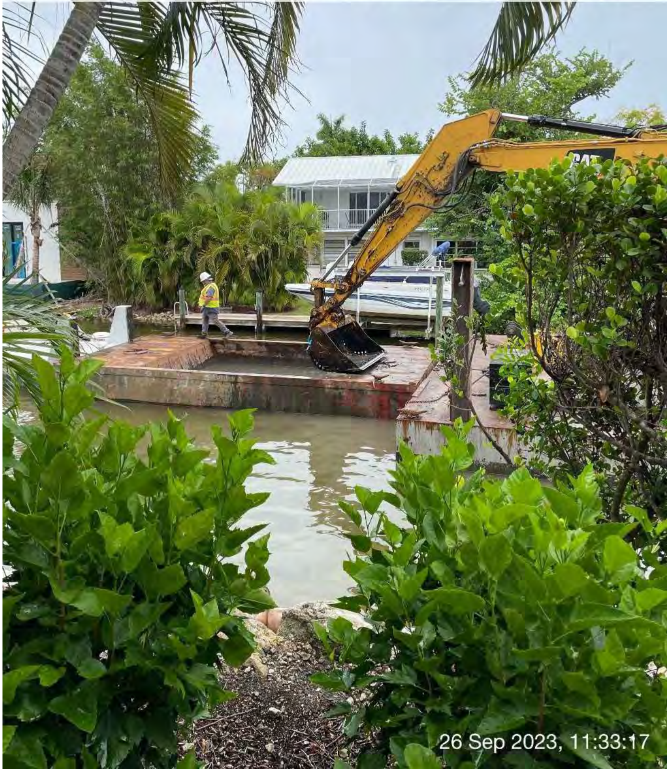
Preparing to move full hopper to the staging area.
