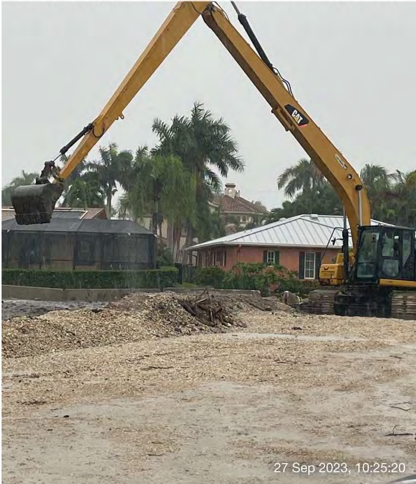
Contractor unloading material from hopper onto staging area.
