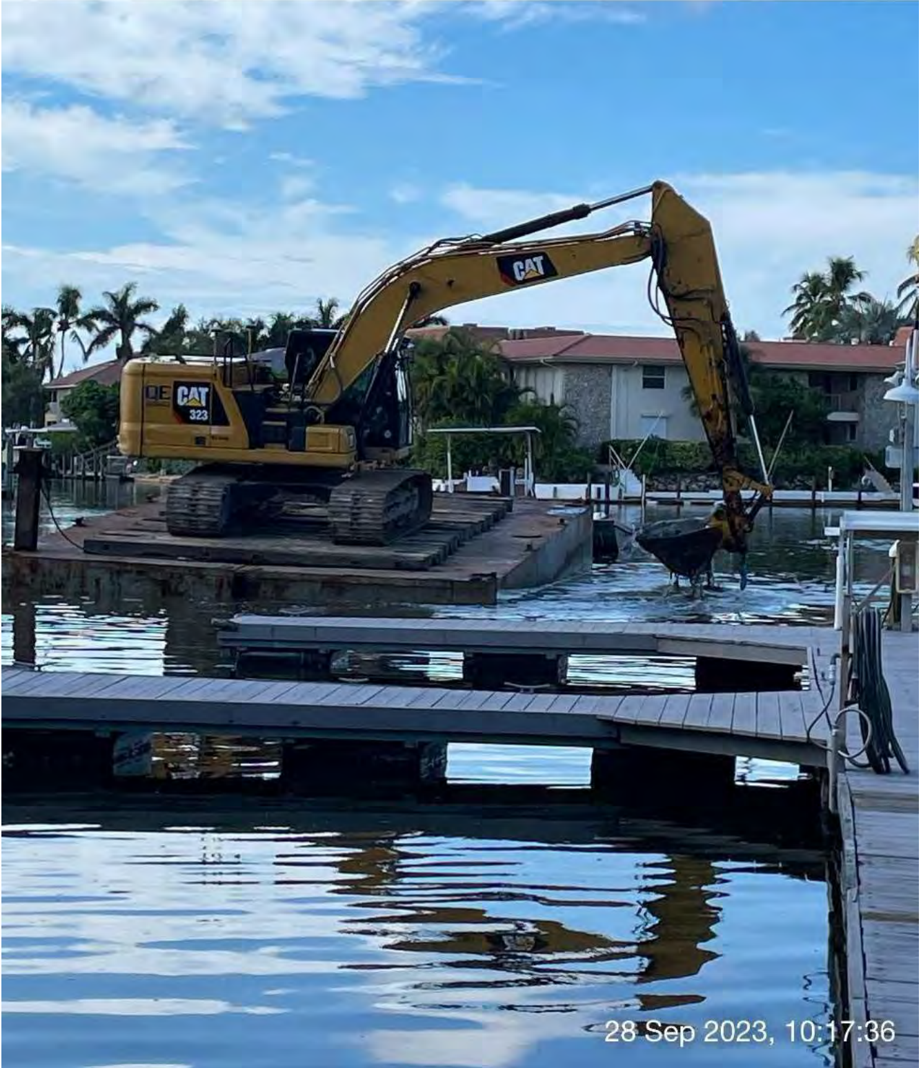
323 excavator removing sediment at station 16+00 in Canal X-X.
