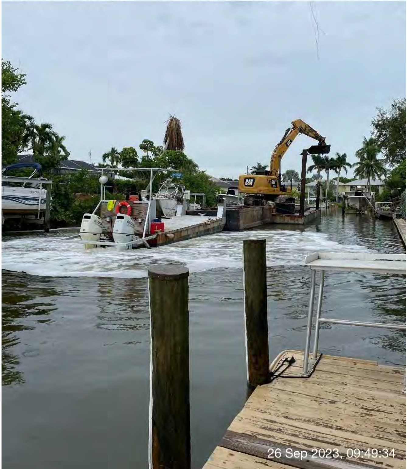
Push boat readjusting dredge position to station 2+50.
