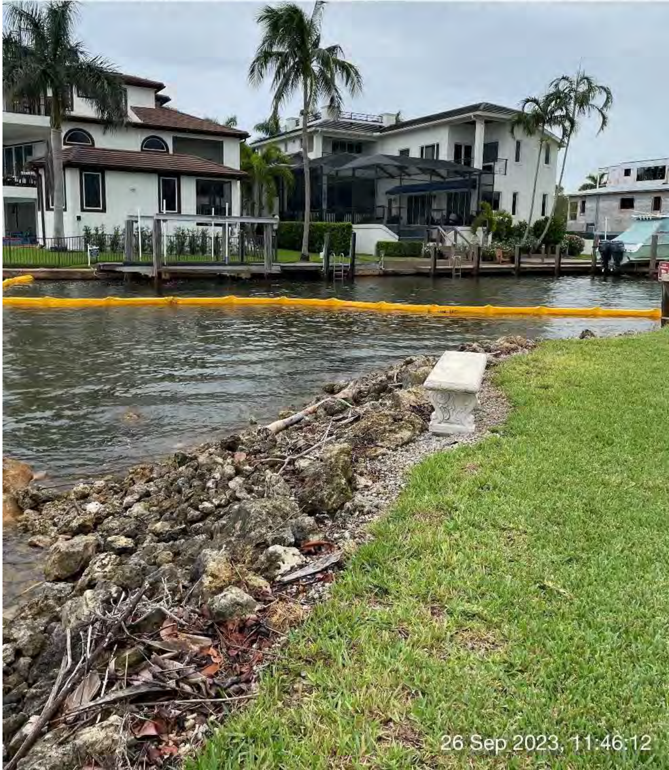
Closing turbidity curtain across Canal X-X at station 1+00.
