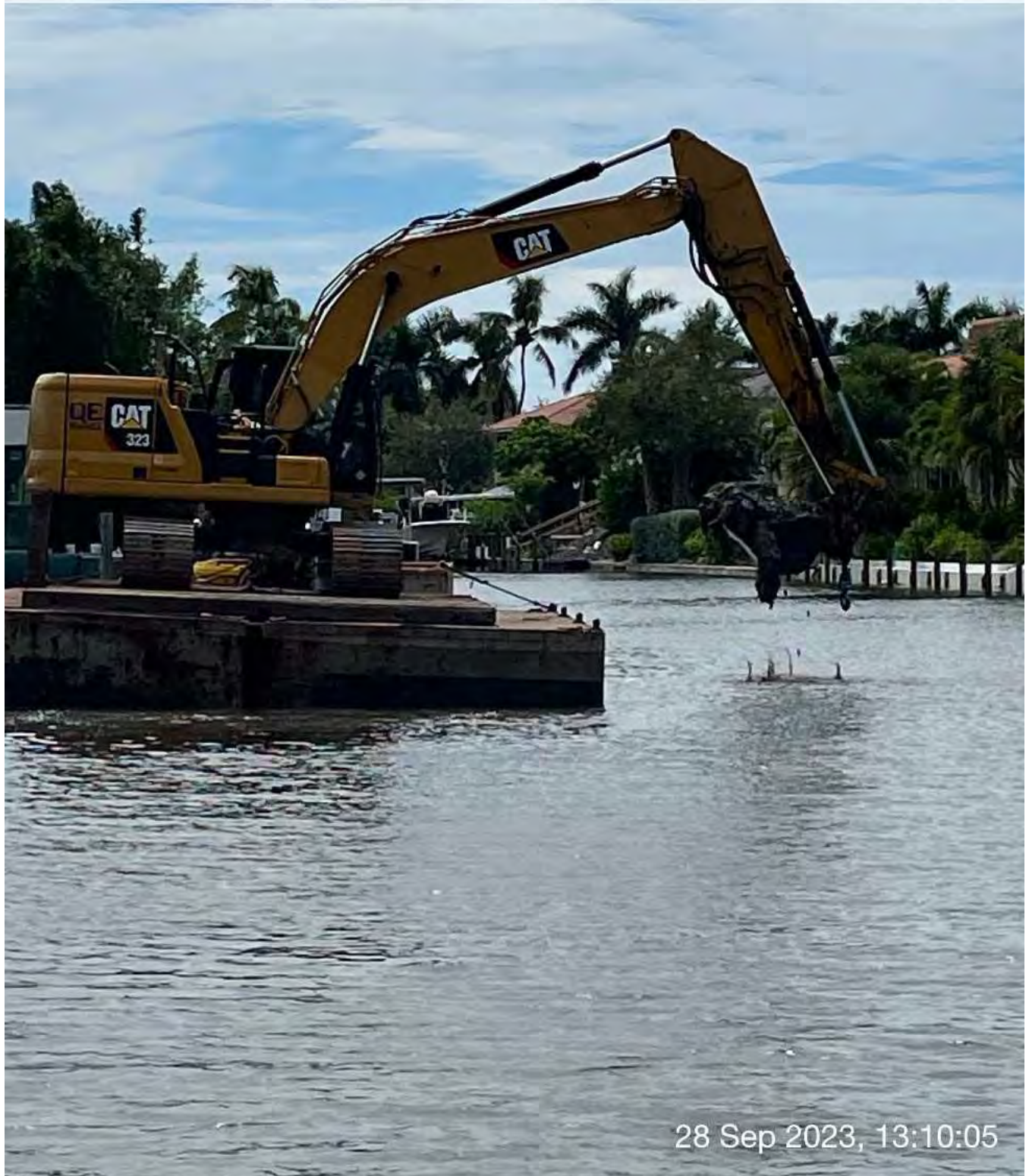
323 excavator removing sediment and large debris at station 15+00 in Canal X-X.
