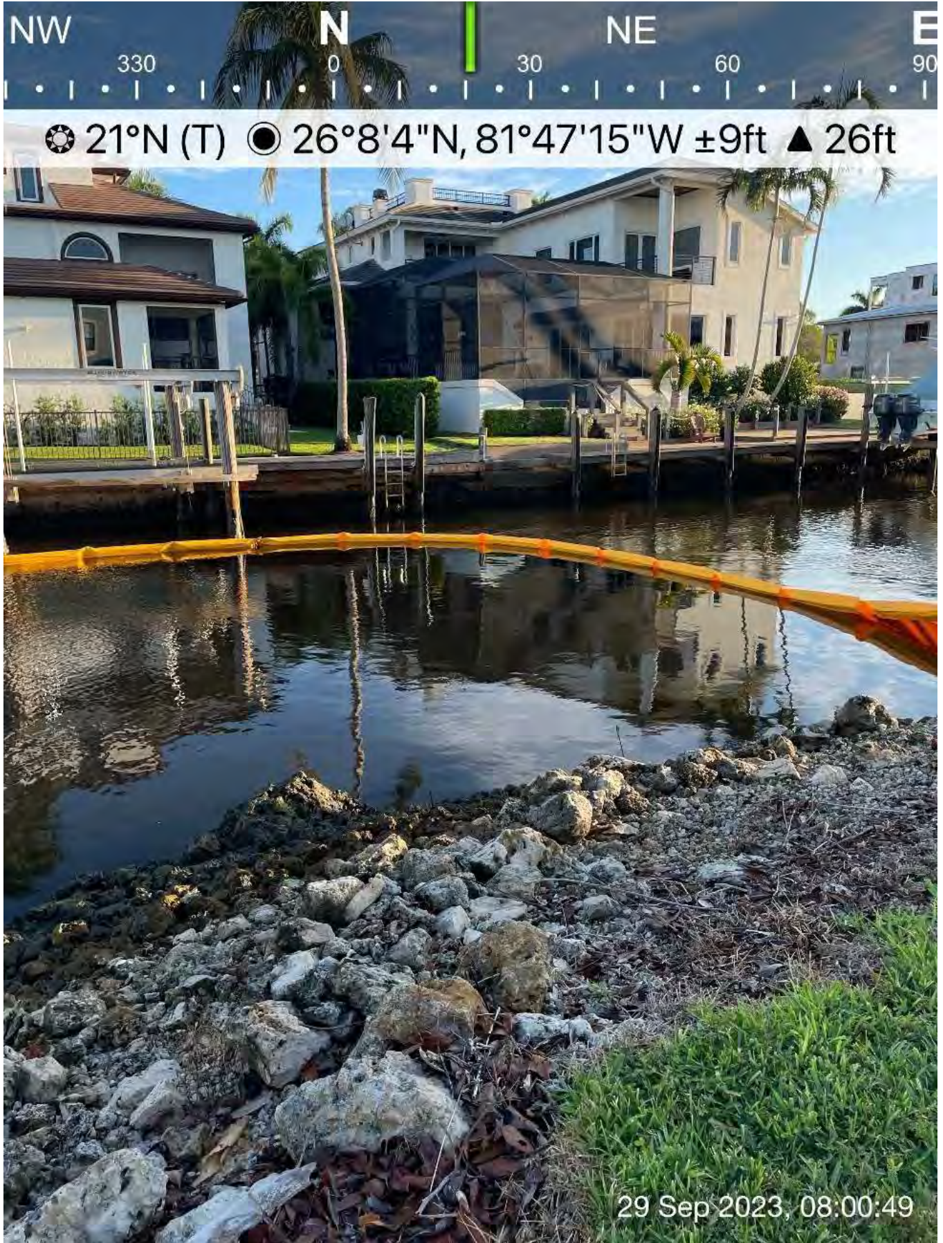
Turbidity curtain in place at station 1+00 in Canal X-X.
