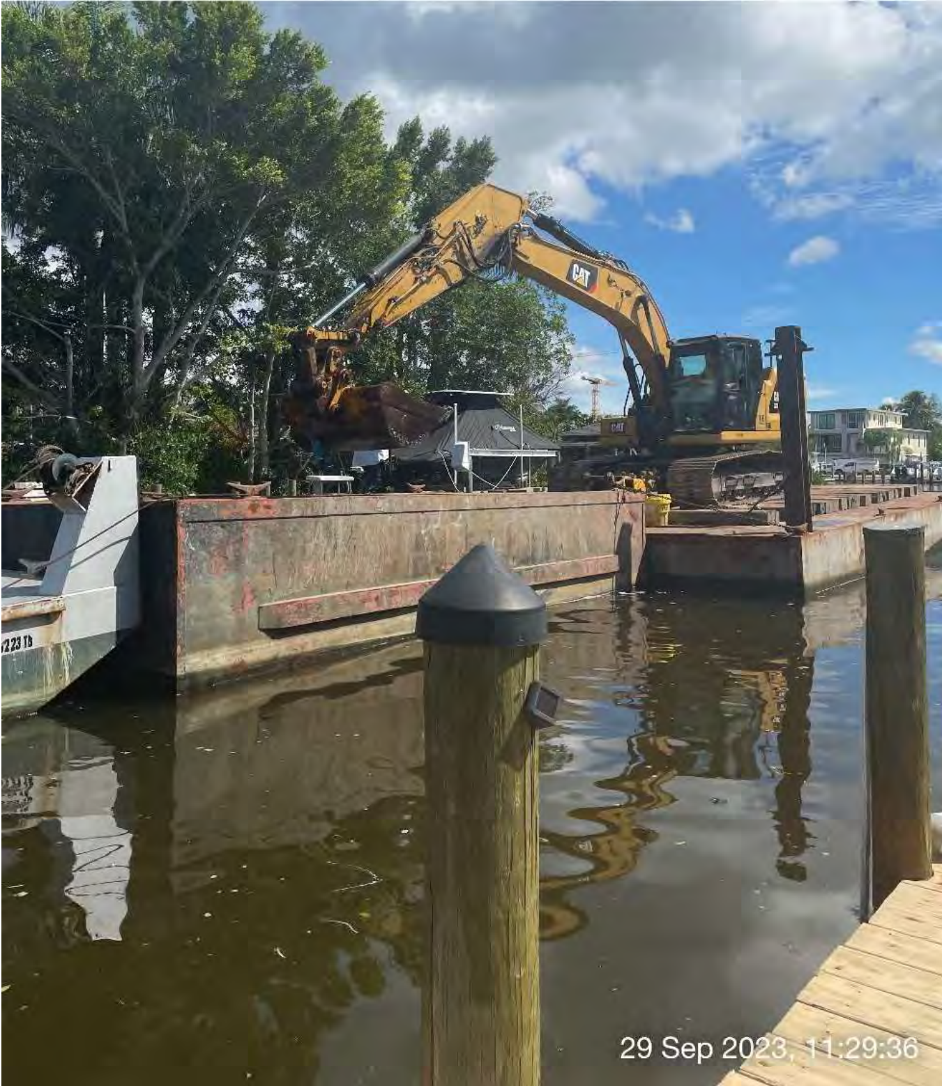
323 excavator removing sediment at station 11+50 in Canal X-X.
