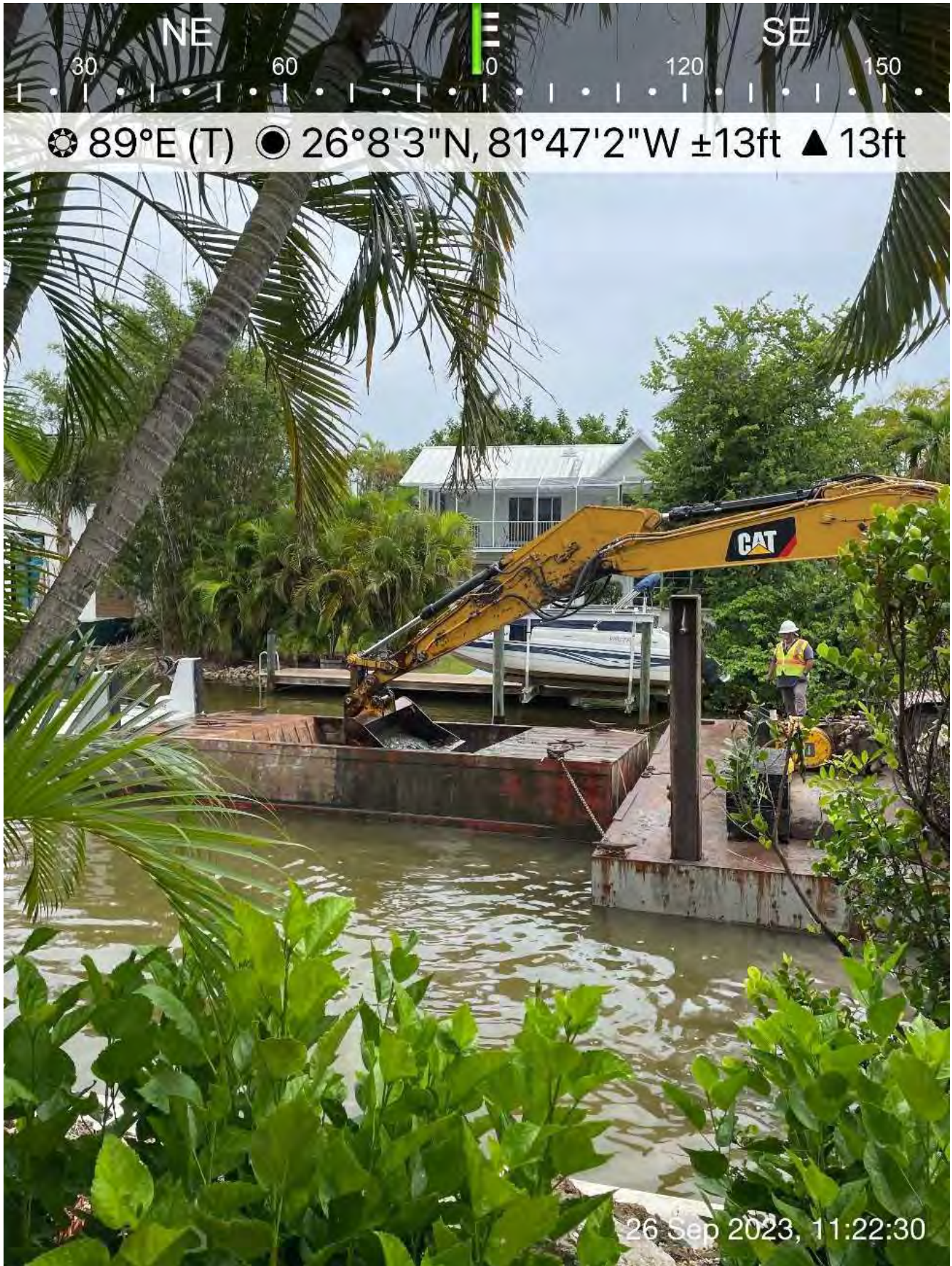
Placing sediment from station 2+50 into the hopper.
