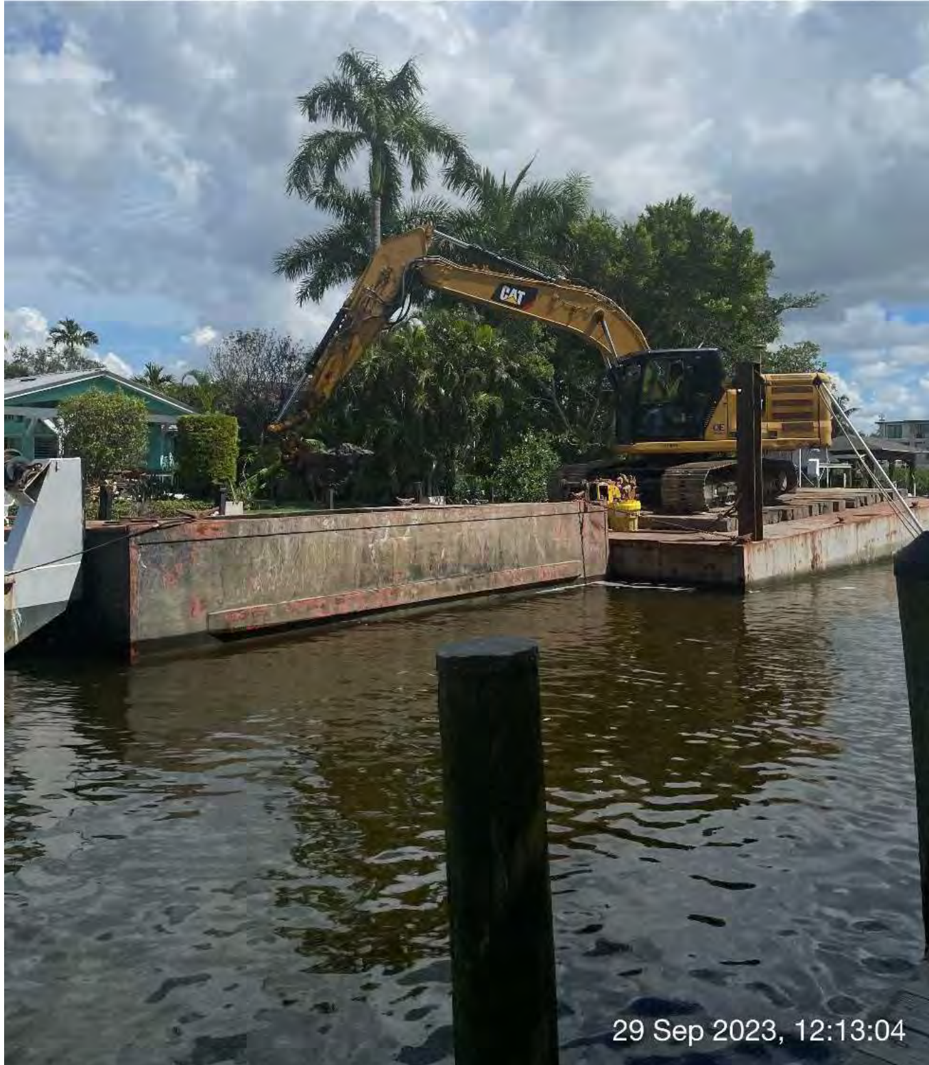
323 excavator removing material at station 10+50 in Canal X-X.
