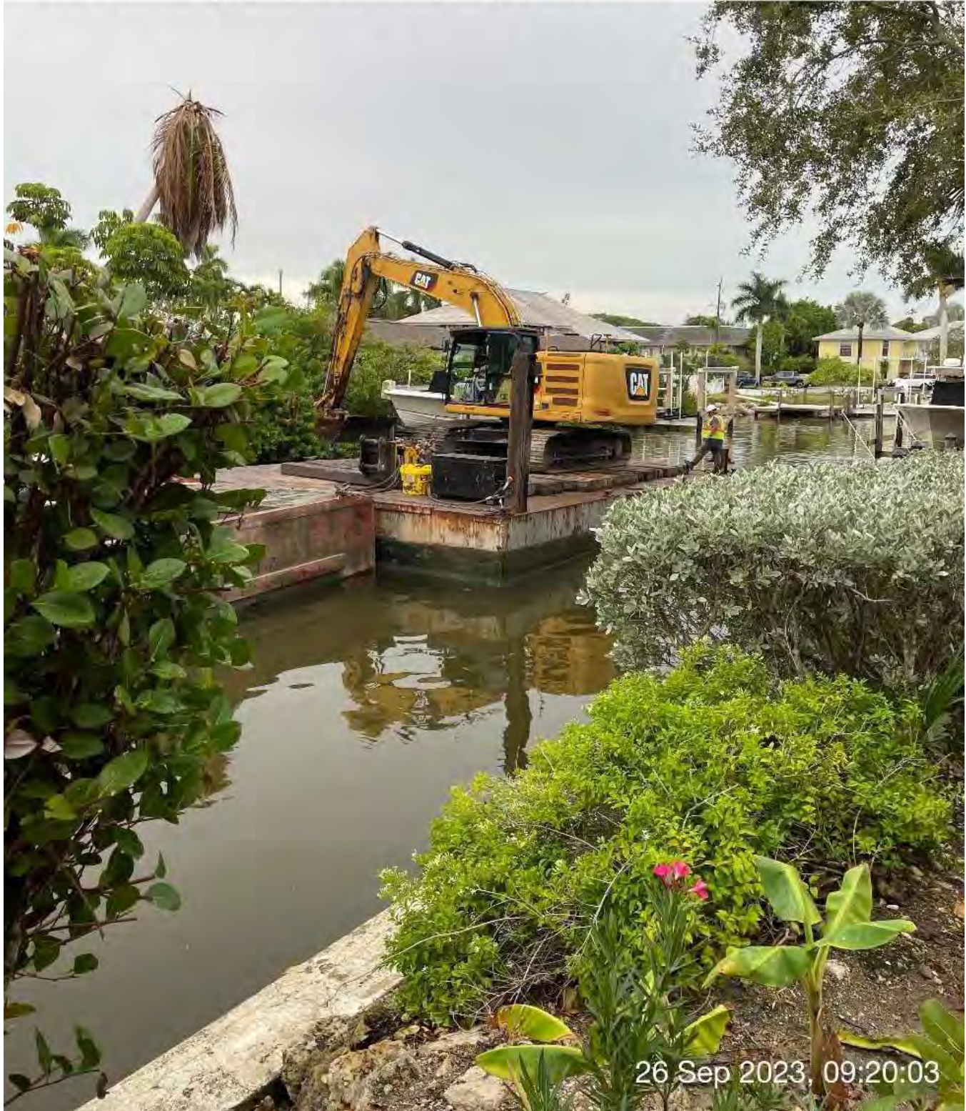
Removal of sediment from Canal AA-AA at station 3+00.
