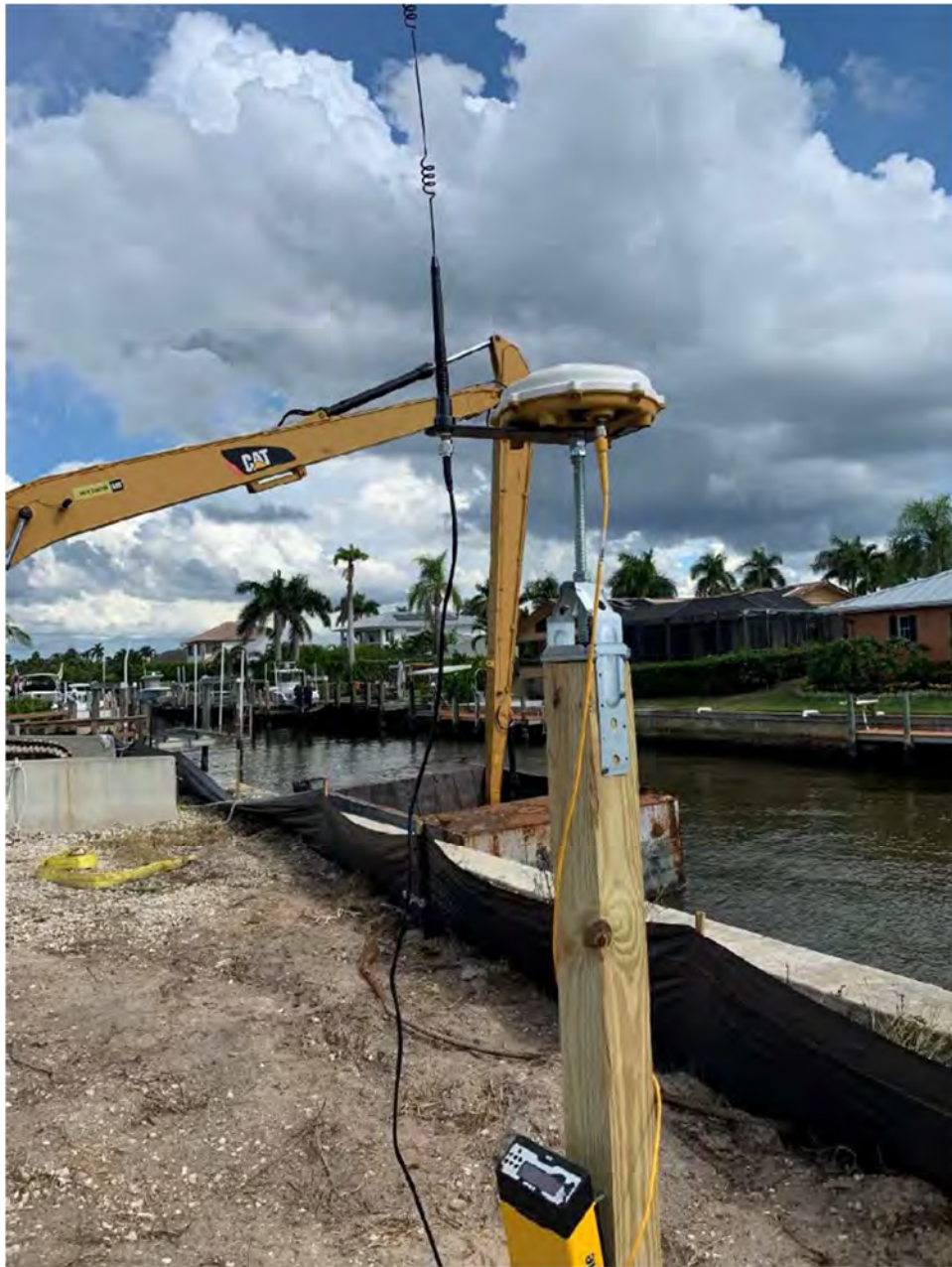
GPS base station at staging area.
