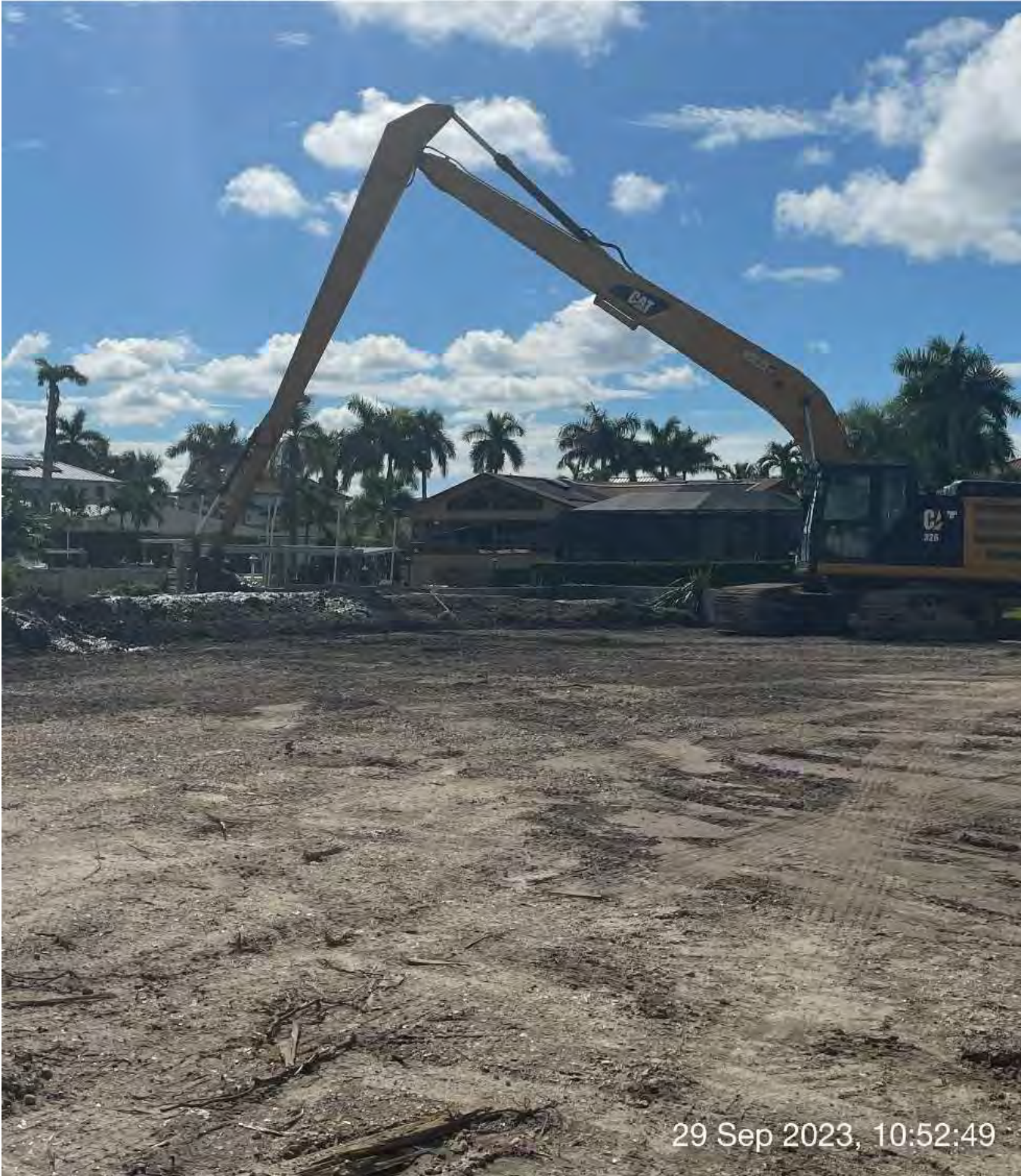
326 excavator unloading material from hopper and spreading it on the staging area.
