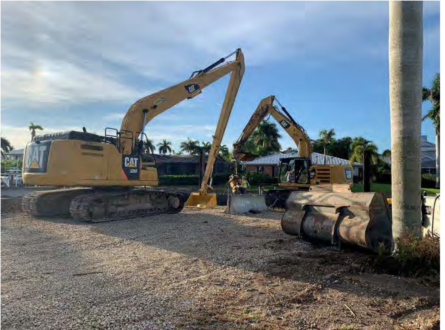
Contractor loading Epiroc grinder onto the barge.
