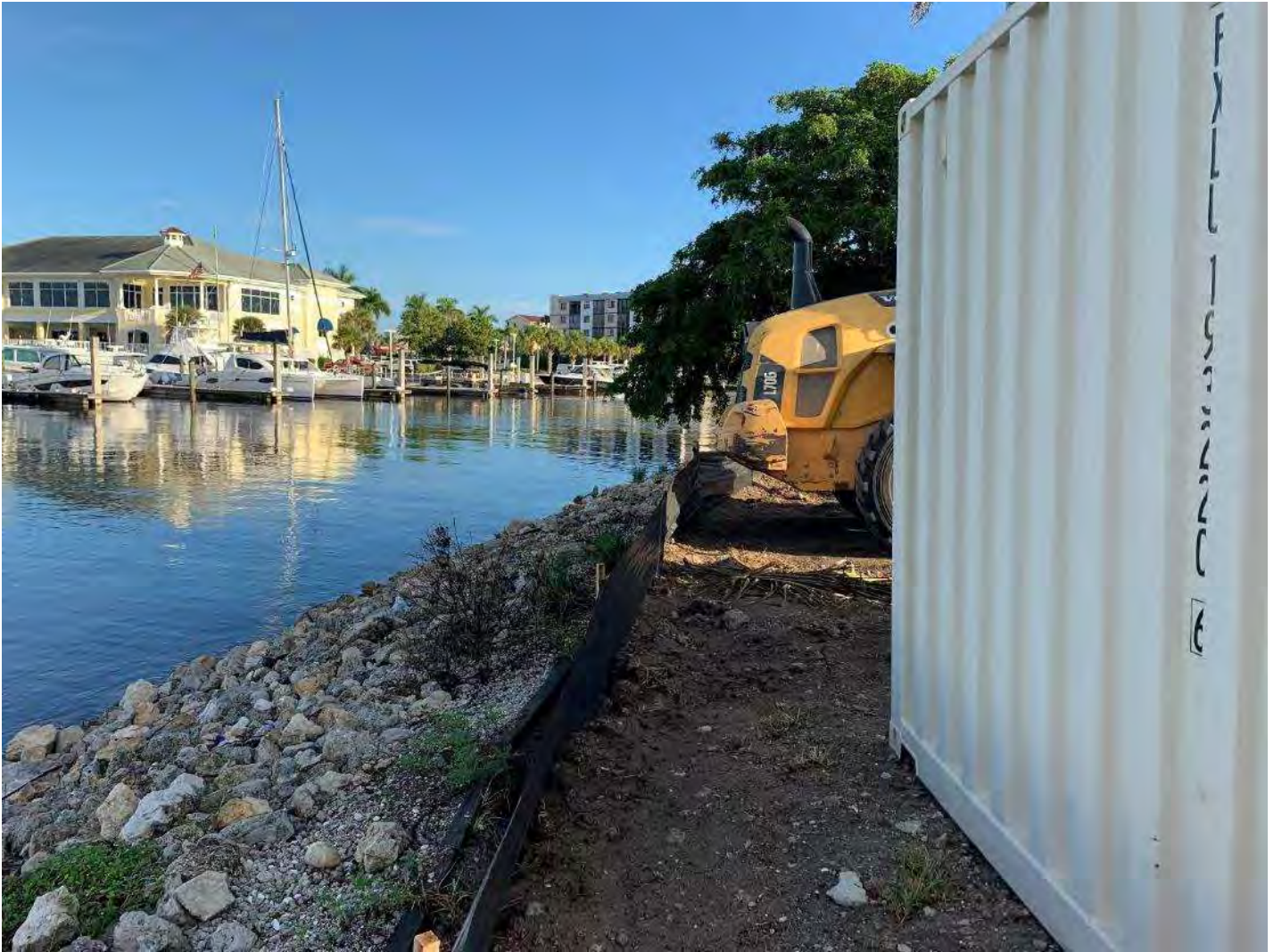
Silt fence in place behind Conex box.
