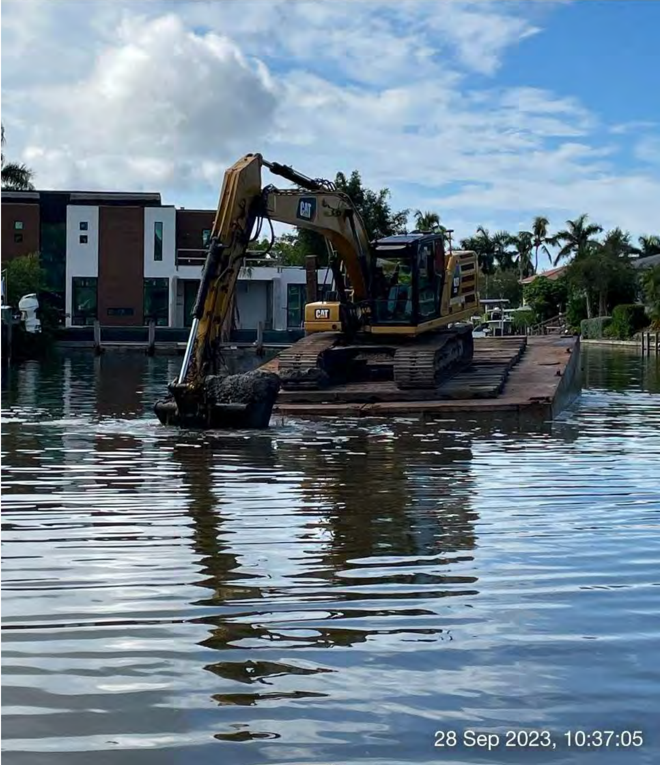
323 excavator removing sediment at station 15+50 in Canal X-X.
