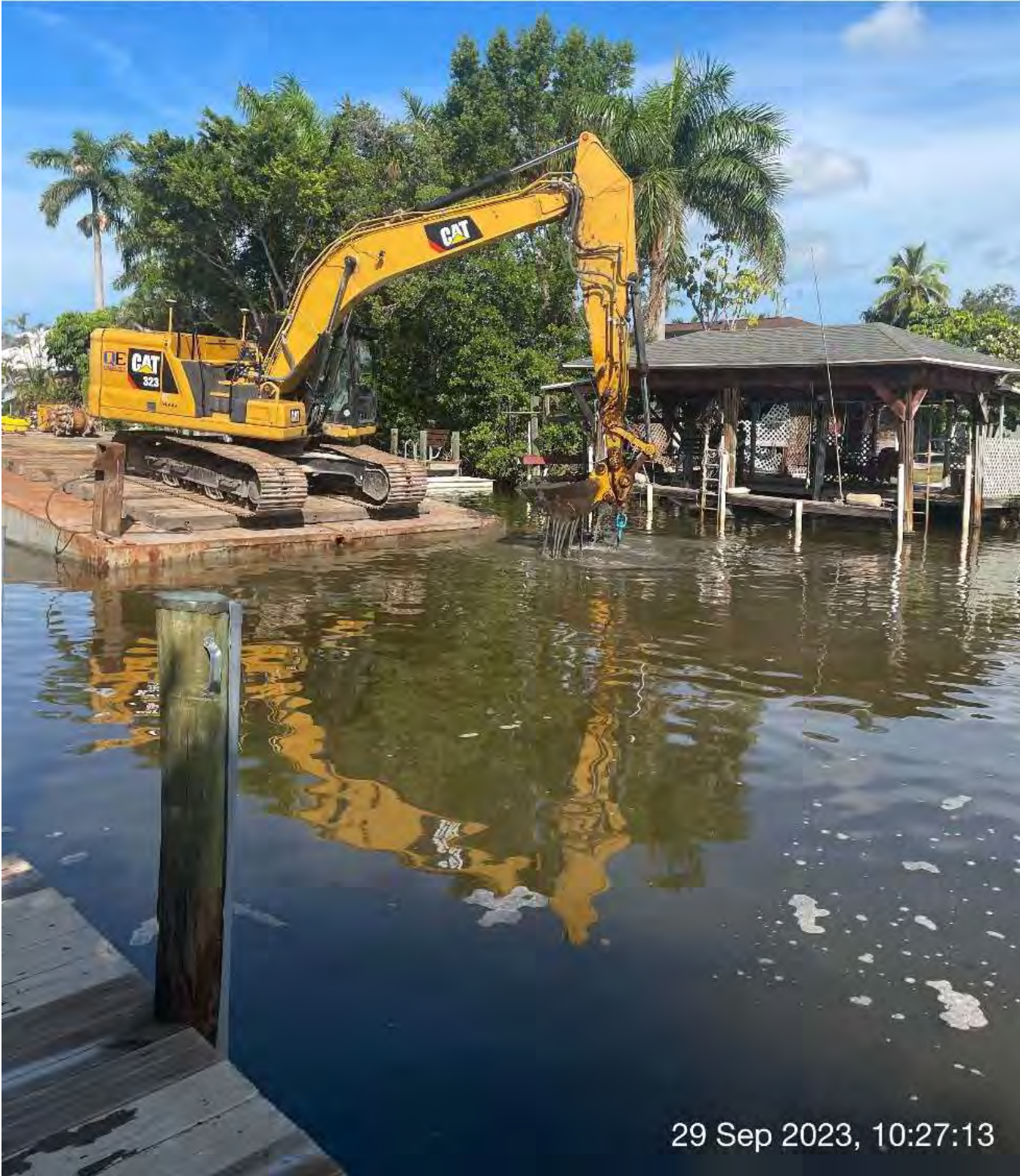
323 excavator removing sediment at station 12+00 in Canal X-X.
