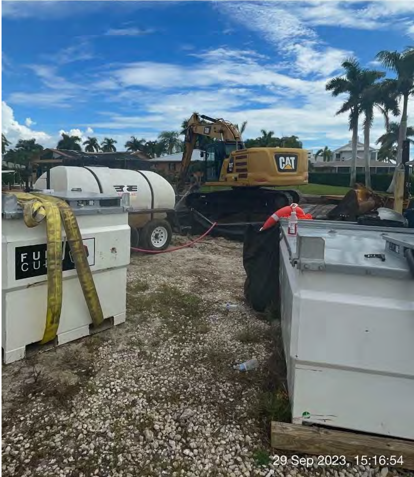
Contractor spraying off equipment with water from the water tank.
