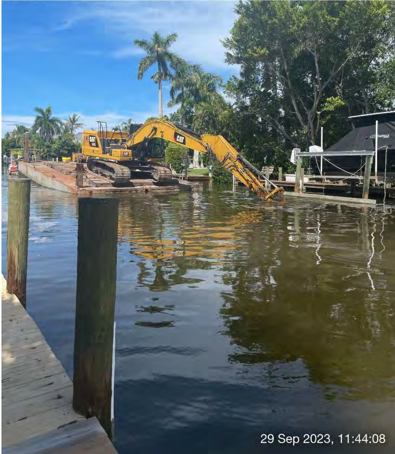
323 excavator removing sediment at station 11+00 in Canal X-X.
