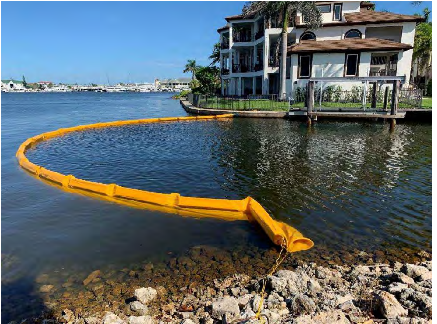
Turbidity curtain in place at mouth of Canal X-X (station 1+00).
