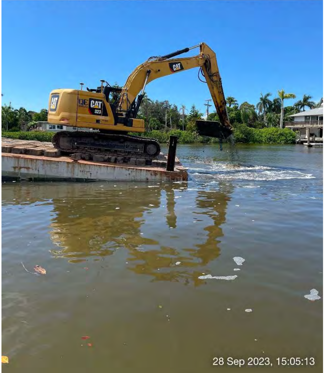
323 excavator removing sediment at station 14+00 in Canal X-X.
