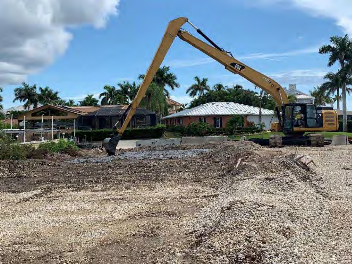
Material from Canal AA-AA being placed into the staging area.
