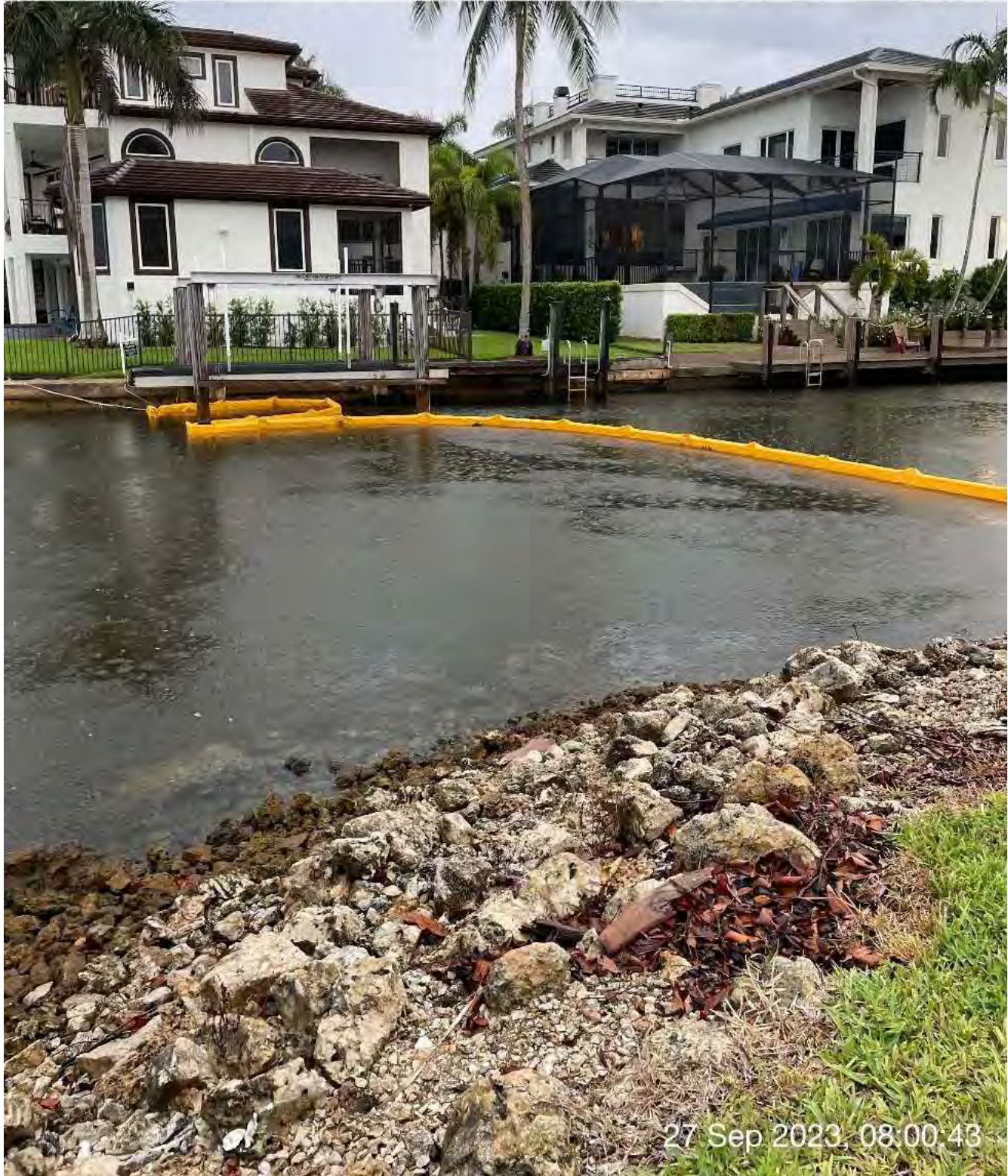
Turbidity curtain in place at station 1+00 in Canal X-X.
