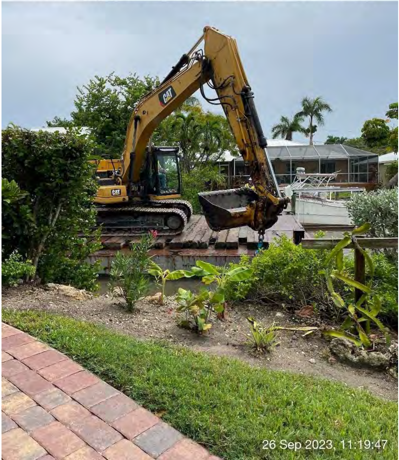
Removing sediment from station 2+50.
