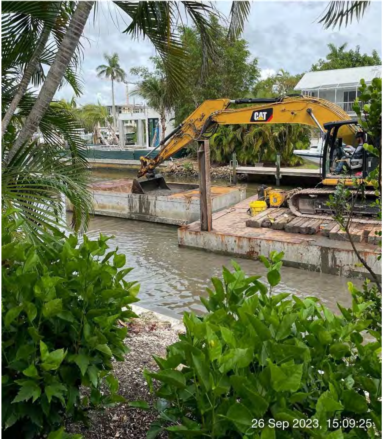
Dredging resumed at station 2+00 in Canal AA-AA.
