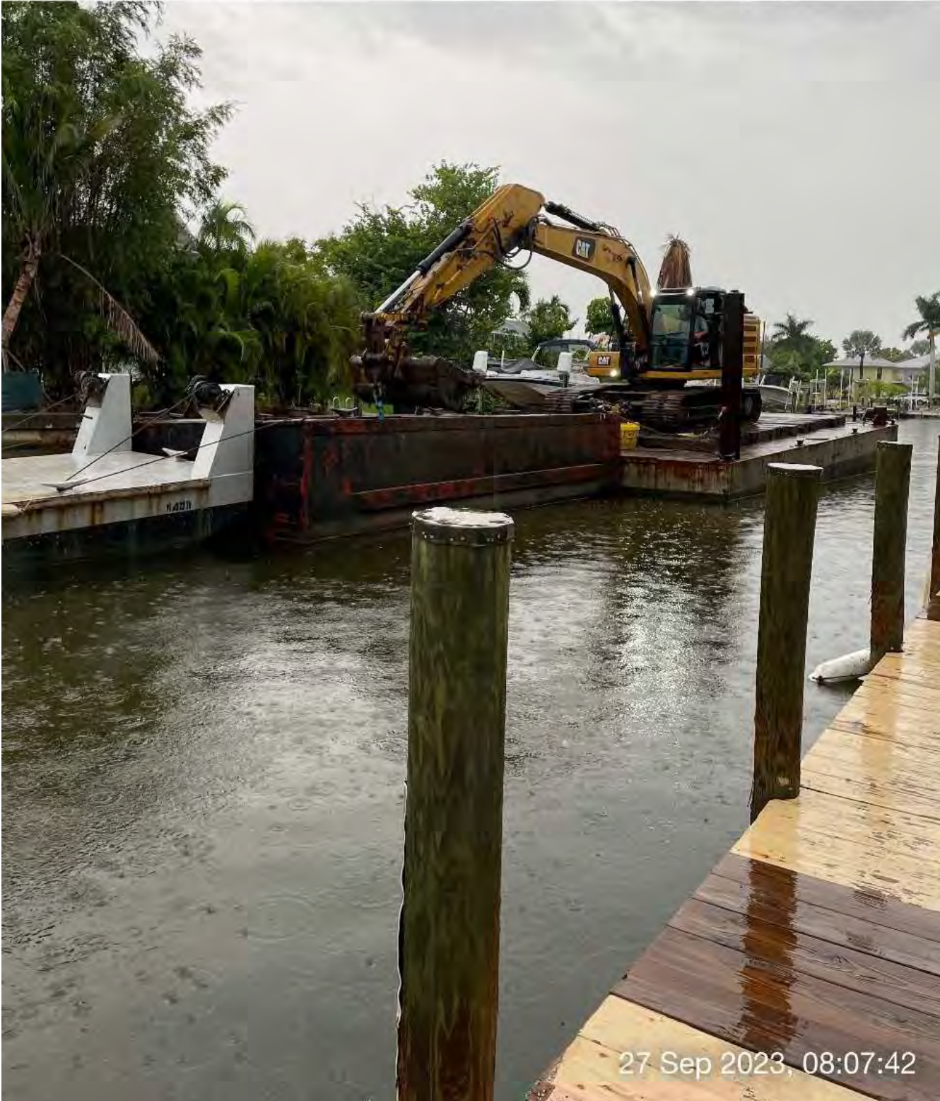
Contractor placing dredge material into hopper at station 2+00 in Canal AA-AA.
