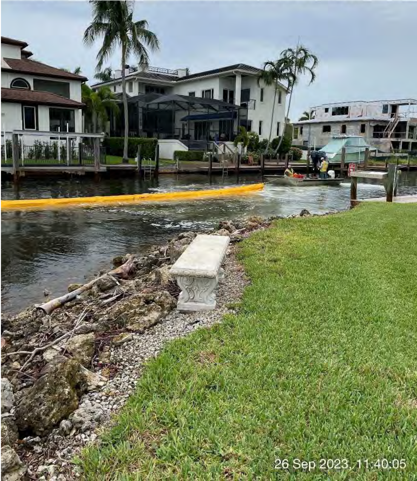
Opening the turbidity curtain allowing hopper to exit Canal X-X.
