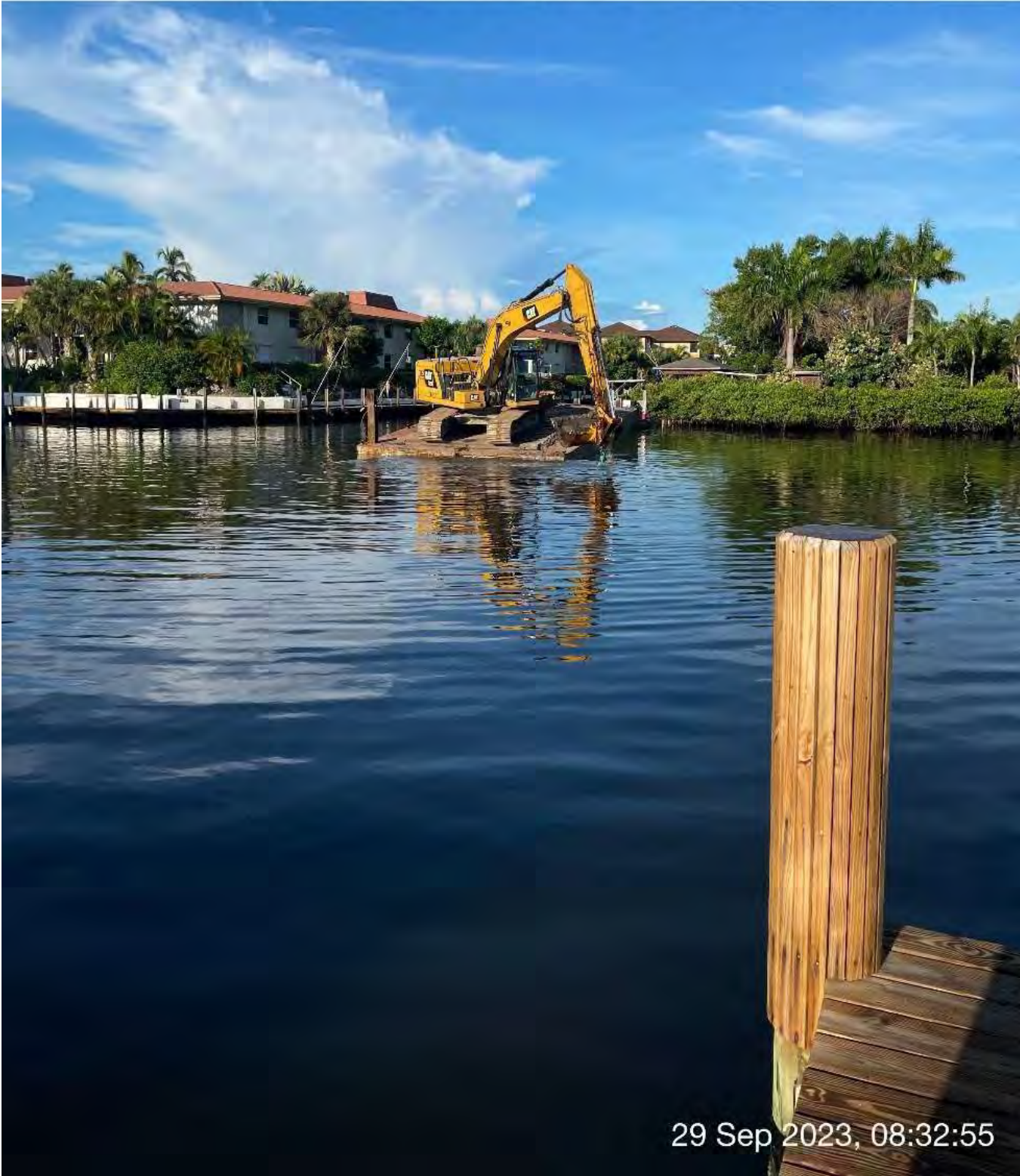
323 excavator removing sediment at station 13+50 in Canal X-X.
