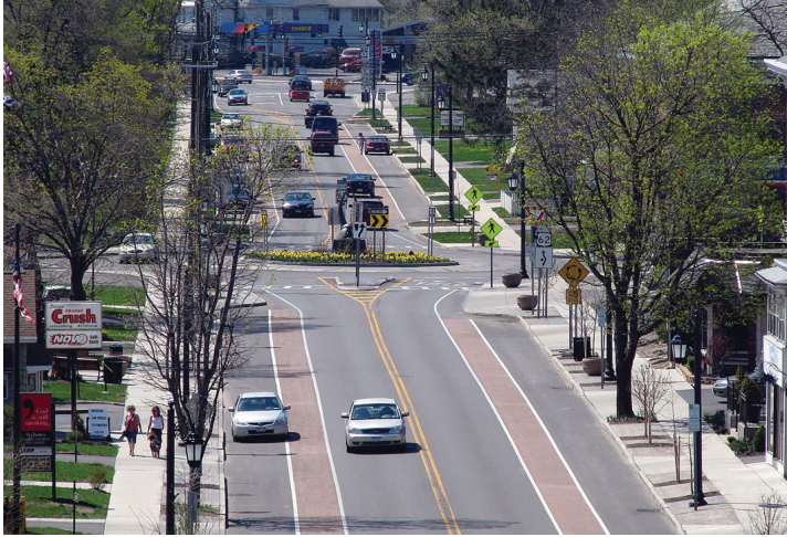
In Hamburg, N.Y., a series of roundabouts on Route 62 helps calm traffic and create a sense of place.
