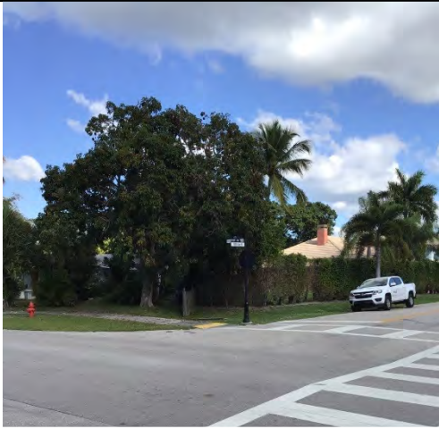
1. Lake 19: Stormwater Inlets capturing runoff from 10 th St N
