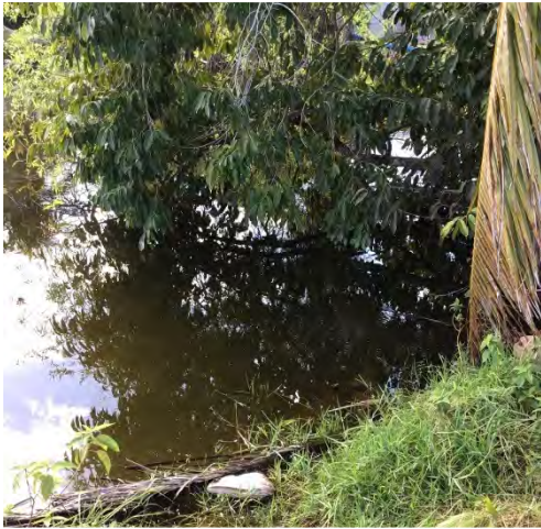
9. Lake 19: 24" reinforced concrete pipe discharging into Lake 19.
