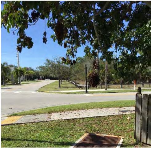
3. Lake 19: Stormwater Inlet capturing runoff from 10 th St N and 14 th Ave N. 30" reinforced concrete pipe discharging into Lake 19
