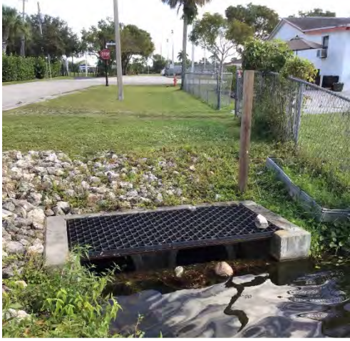
13. Lake 19: Stormwater grate outfall with weir with 2 - 30" reinforced concrete pipe discharging from Lake 19.
