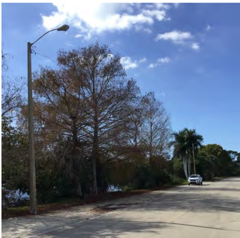
11. Lake 19: Light poles with overhead and underground utilities. Proposed staging area for dewatering activities
