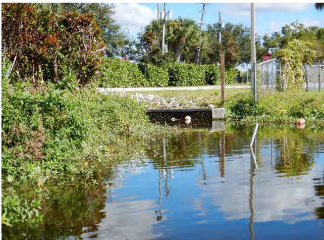
5. Lake 19: Outfall on northeast corner of lake
