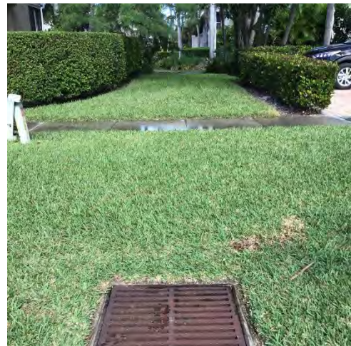
22. Lake 31: Stormwater inlet along 8 th Ave S that captures runoff from road and conveys the discharge from Lakes 11 and 31 to cove pump station.
