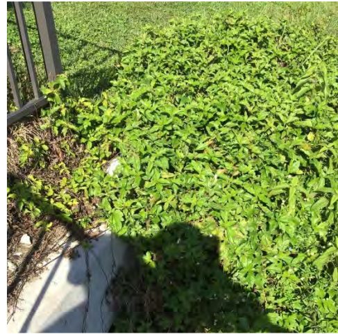
Lake 11: Stormwater inlet along W Lake Dr with 24" PVC pipe running between two residents along Lake 11 with concrete headwall
