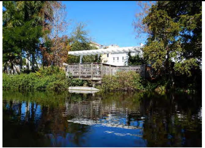
8. Lake 11: View of observation deck with headwall and culvert below
