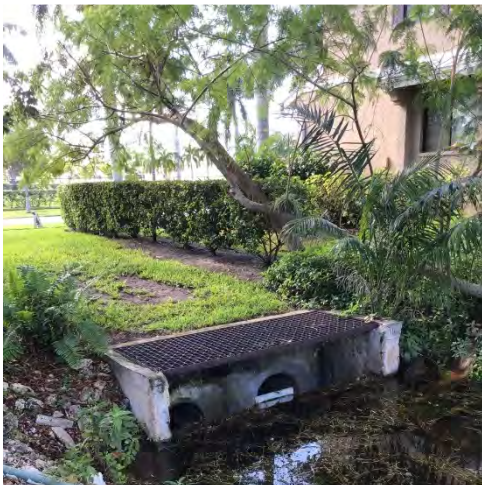
21. Lake 31: Lake 31 and main discharge structure from Lakes 11 and 31.
