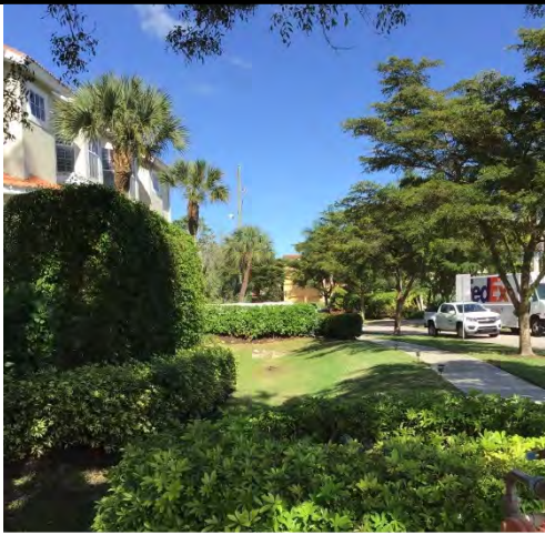
1. Lake 11: Stormwater inlets and grassed dry retention swales for private condos
