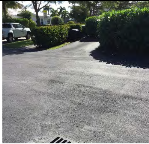
2. Lake 11: Stormwater inlets and grassed dry retention swales for private condos
