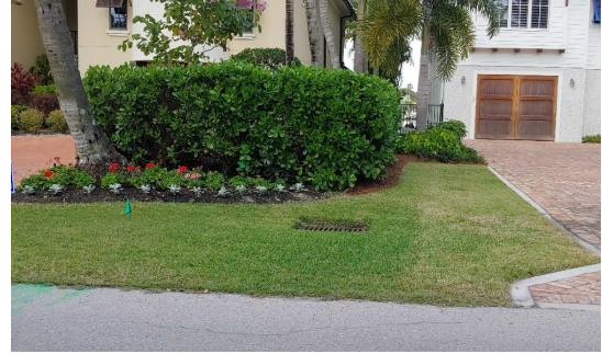
Figure 12. Catch Basin with No Swale
