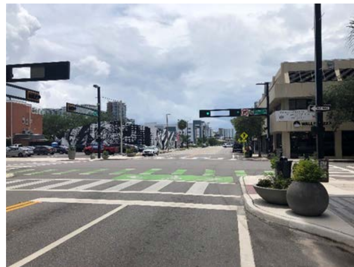
City of Tampa Bike and Pedestrian Crossing
