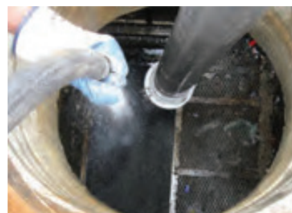
Hinged screens allow for full vacuum access to inner basket and lower sediment chambers.
