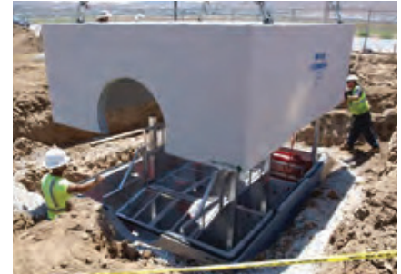
Minimal excavation required
