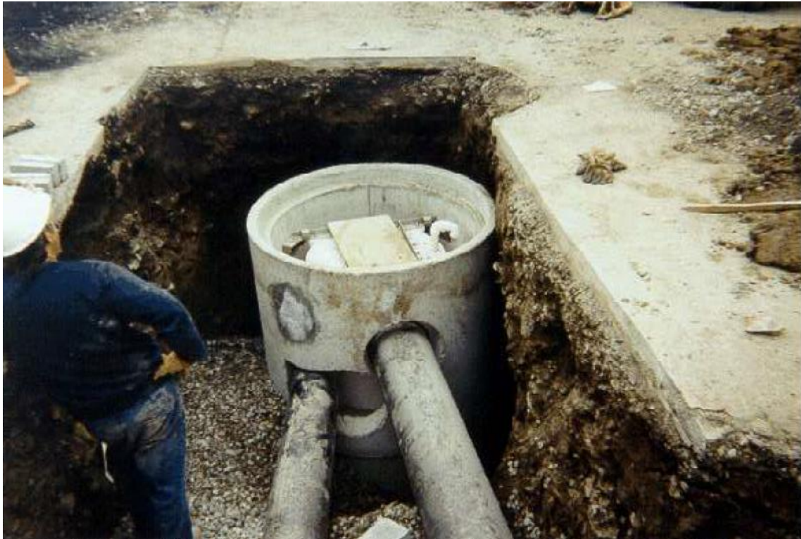
Figure 3: Photo of Downstream Defender installation
