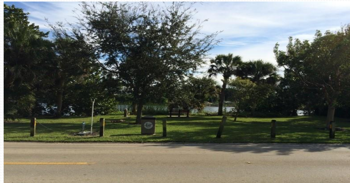
Alligator Lake Generator Site
