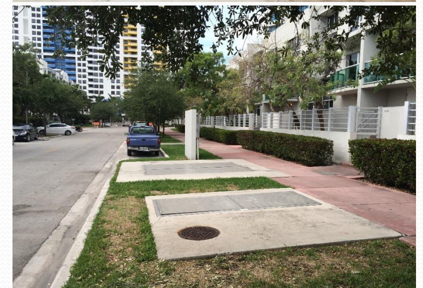
Typical Underground Pump Stations with Elevated Control Panel
