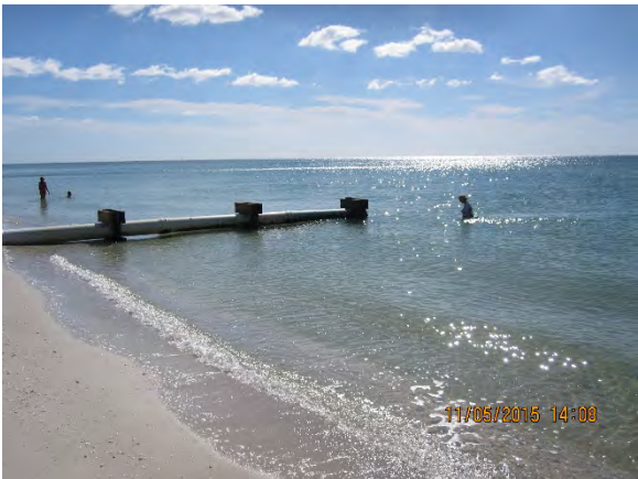
Figure 24 – Outfall #5 Looking Southwest
