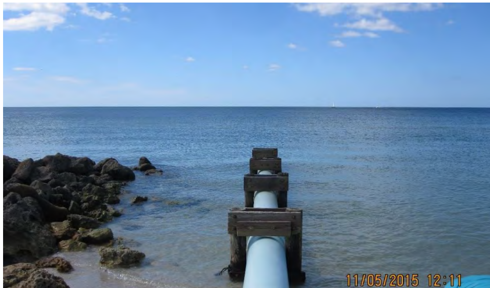
Figure 2-1. Typical Beach Outfall (Outfall 3 Shown)
