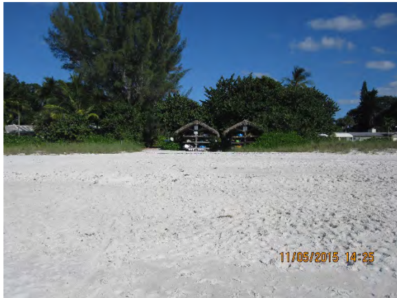
Figure 40 – Outfall #7 Looking East
