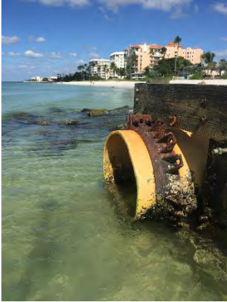
Figure 12 – Outfall #2 Looking North
