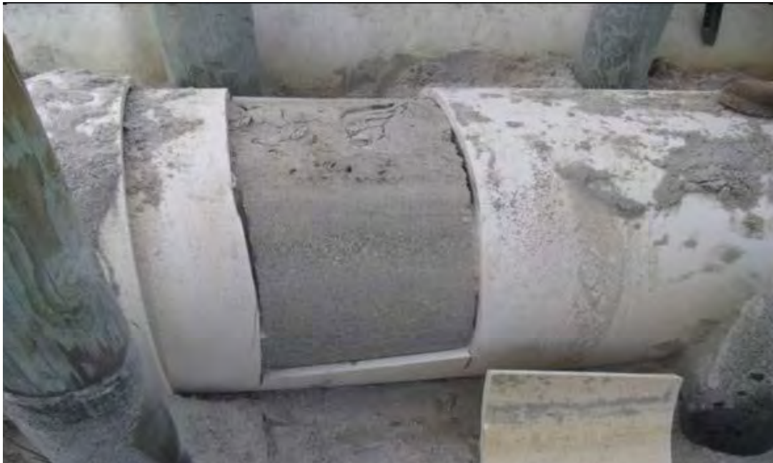
Figure 1-4. Typical Clearing of Outfall Blockages (Outfall 6)
