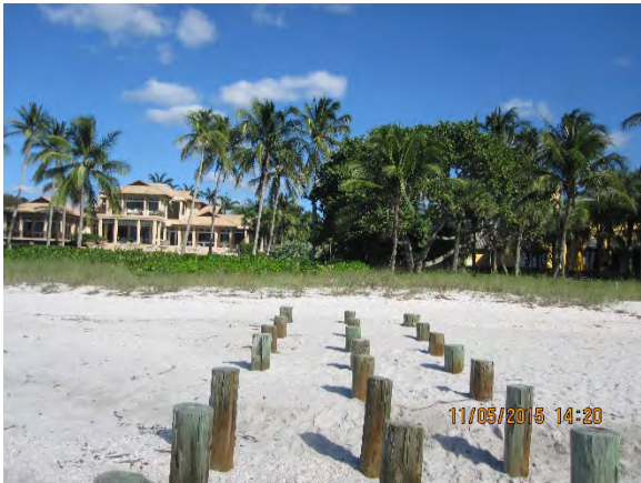
Figure 32 – Outfall #6 Looking East
