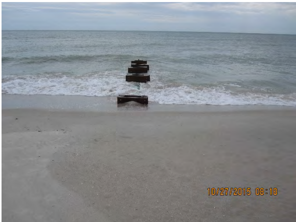
Figure 49 – Outfall #9 Looking West
