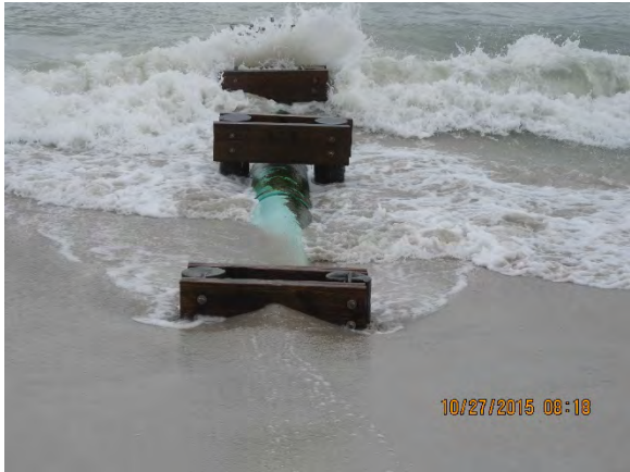
Figure 50 – Outfall #9 Looking West
