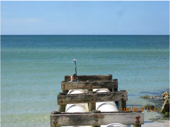
Figure 8 – Outfall #2 Looking West
