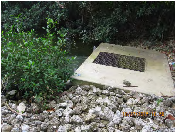
Figure 30 – Outfall #8 Looking North
