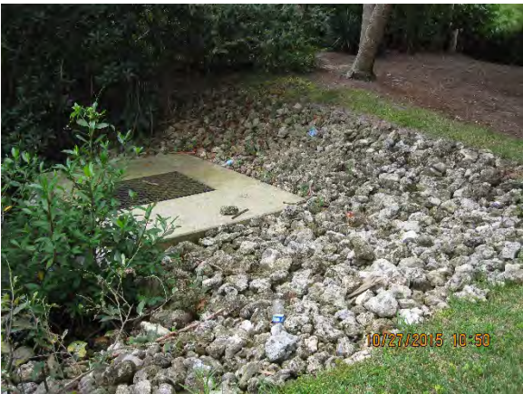
Figure 29 – Outfall #8 Looking West
