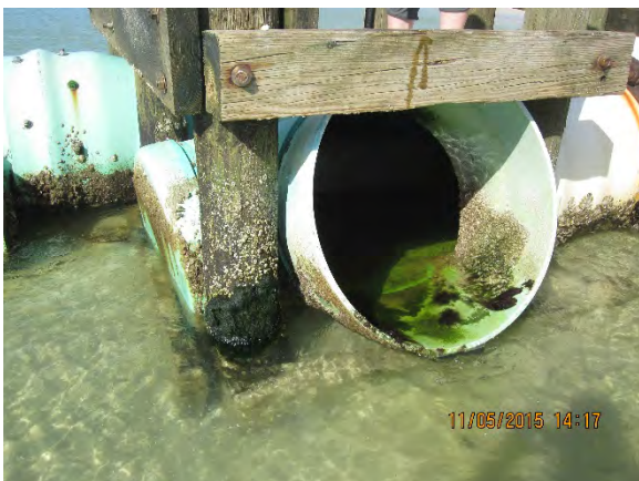
Figure 37 – Outfall #6 South-side of South-pipe
