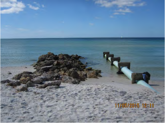
Figure 14 – Outfall #3 Looking West
