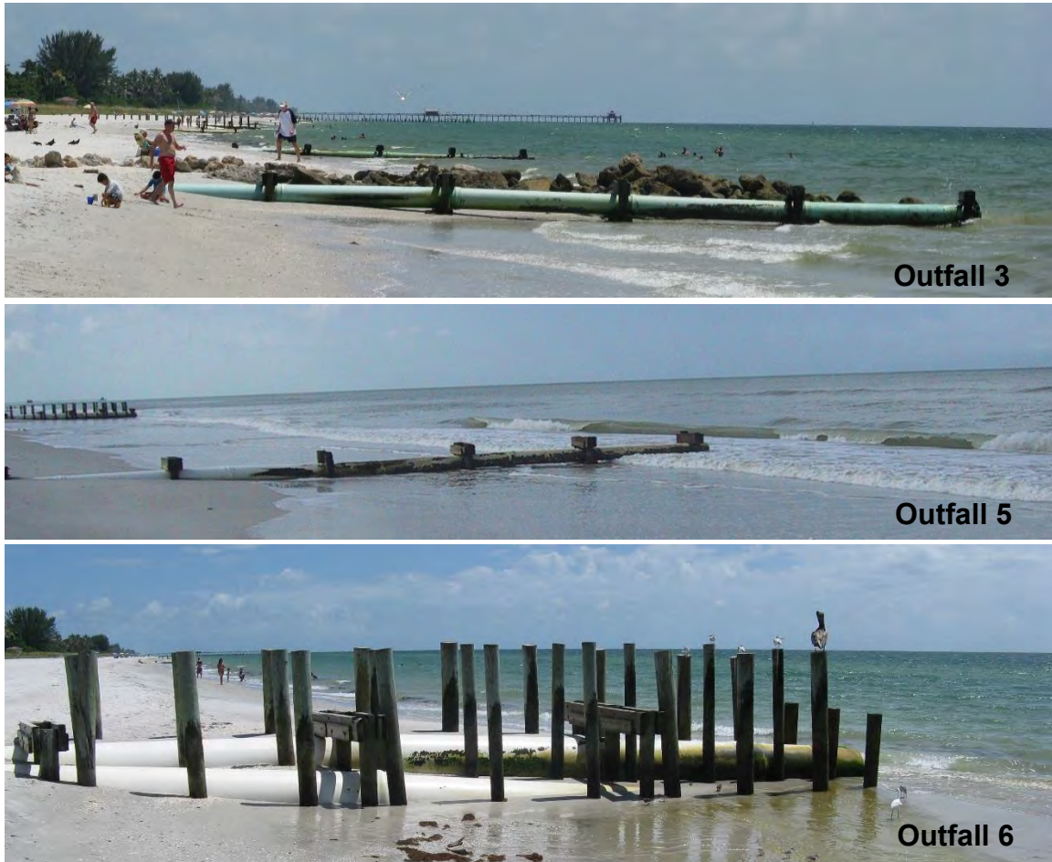
Figure 1-7. Typical pipes and wooden pile mountings on the beach
