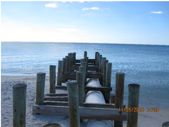
Figure 33 – Outfall #6 Looking West
