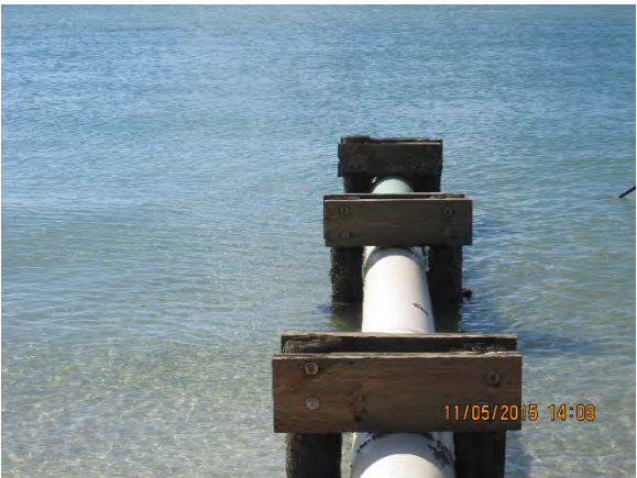
Figure 23 – Outfall #5 Looking West
