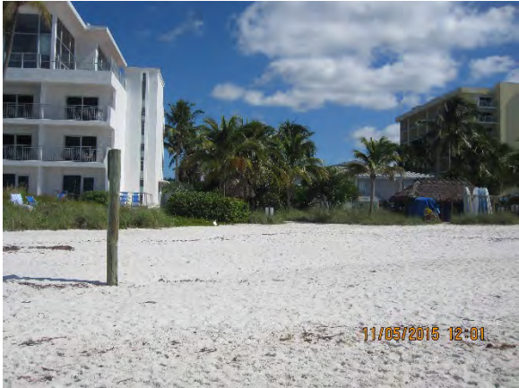
Figure 7 – Outfall #2 Looking East
