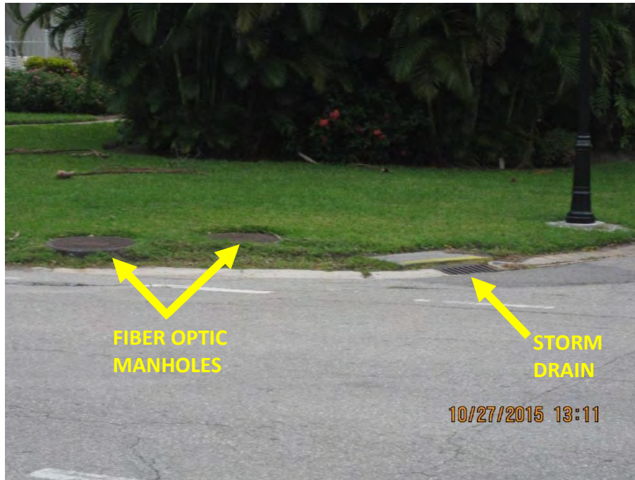
Figure 3-7. Typical Intersection with Utilities – Storm Drain with Adjacent Fiber Optic Cable Manholes
