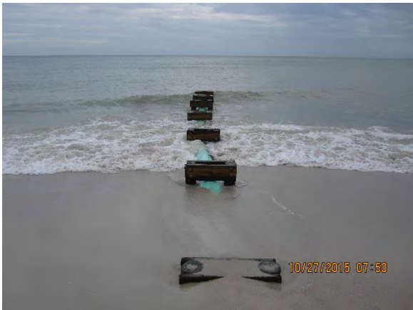
Figure 54 – Outfall #10 Looking West
