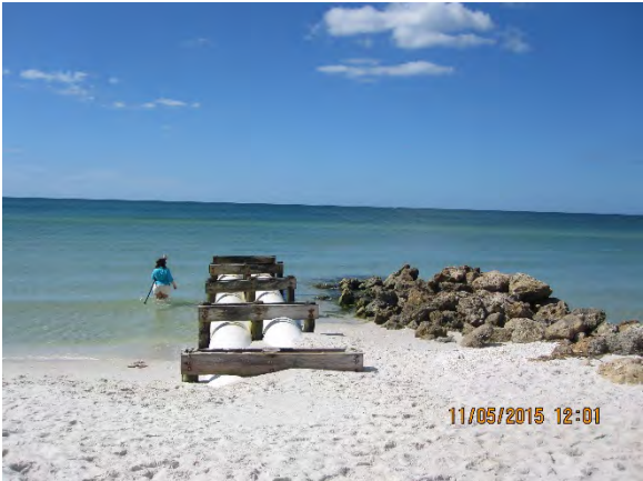
Figure 9 – Outfall #2 Looking West
