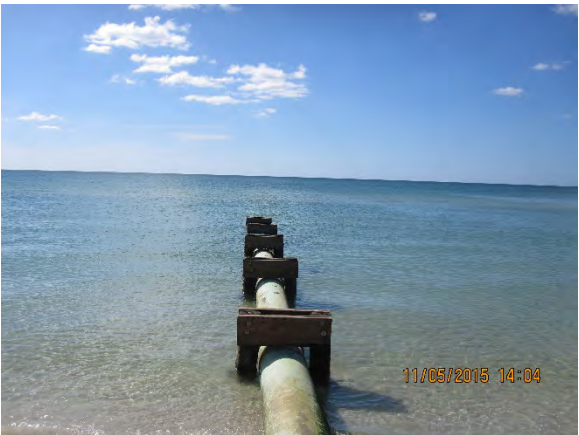
Figure 18 – Outfall #4 Looking West
