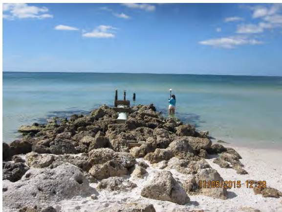
Figure 3 – Outfall #1 Looking West
