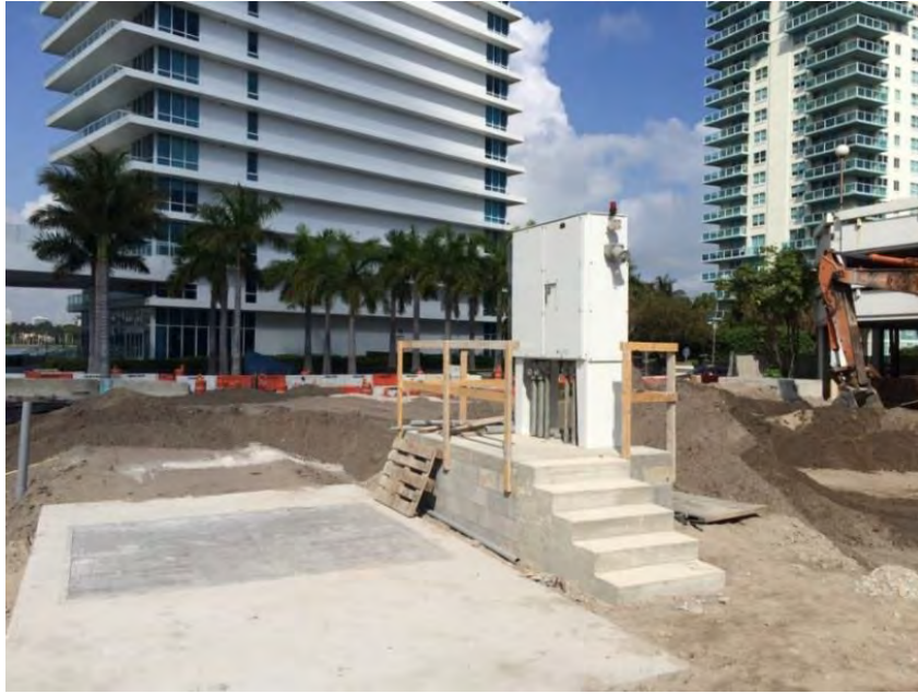
Figure 3-16. Electrical Components Installed on Raised Access Platforms
