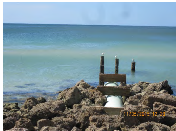
Figure 2 – Outfall #1 Looking West
