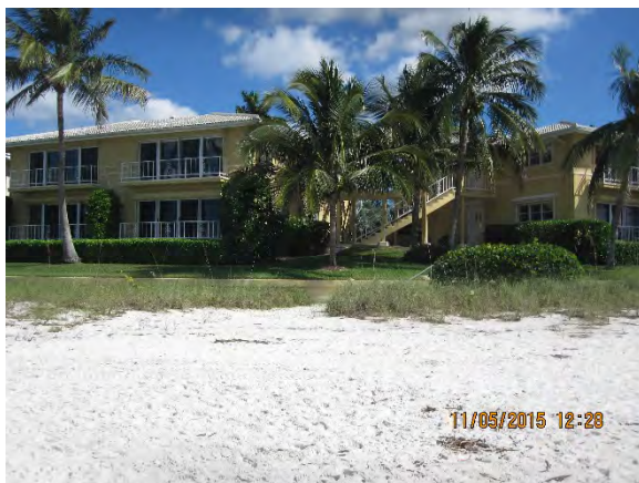
Figure 1 – Outfall #1 Looking East
