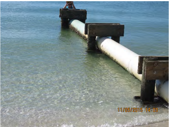
Figure 27 – Outfall #5 Looking Northwest
