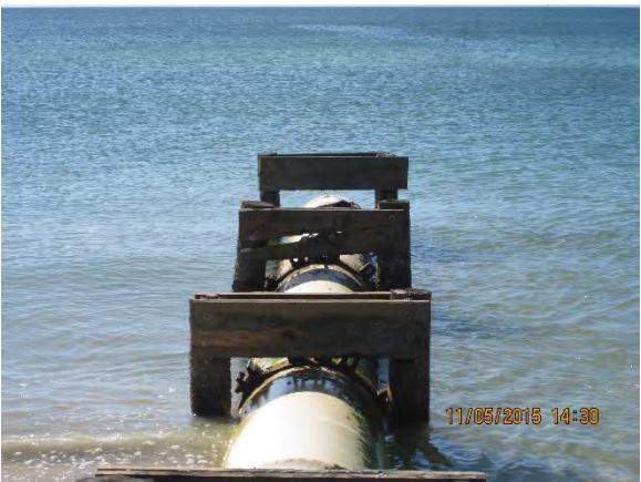
Figure 45 – Outfall #8 Looking West
