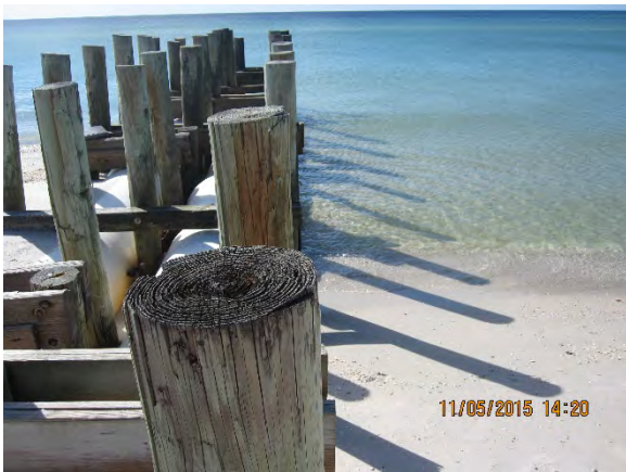
Figure 35 – Outfall #6 Looking West, North Side
