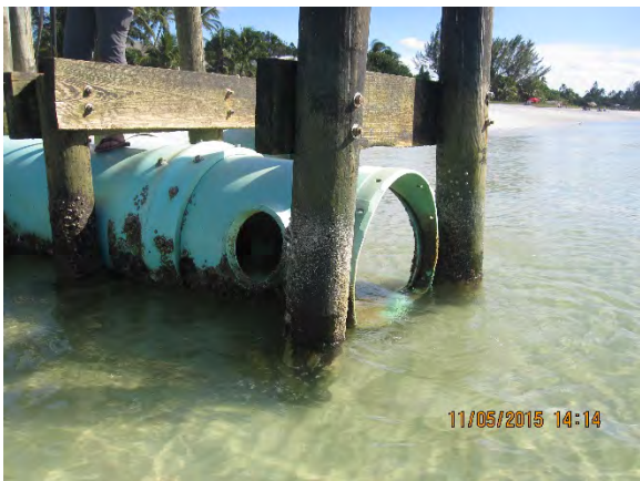
Figure 36 – Outfall #6 North-side of North-pipe
