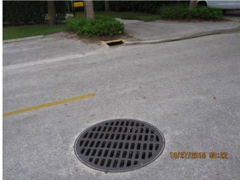
Figure 3-3. Typical Storm Sewer Manhole in Foreground with Curb Inlet in Background
