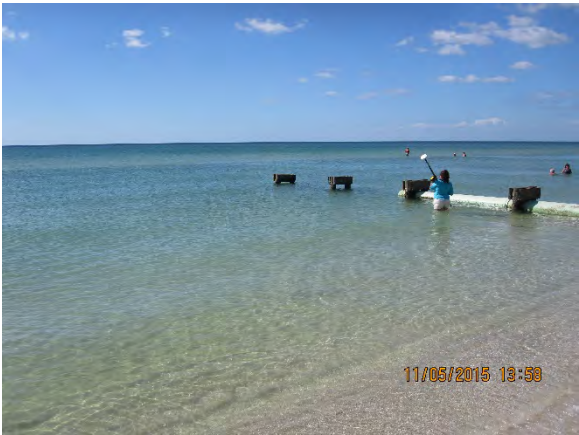
Figure 19 – Outfall #4 Looking Northwest
