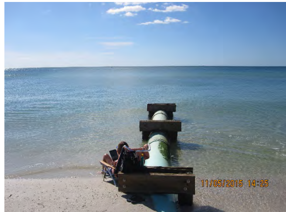
Figure 41 – Outfall #7 Looking West
