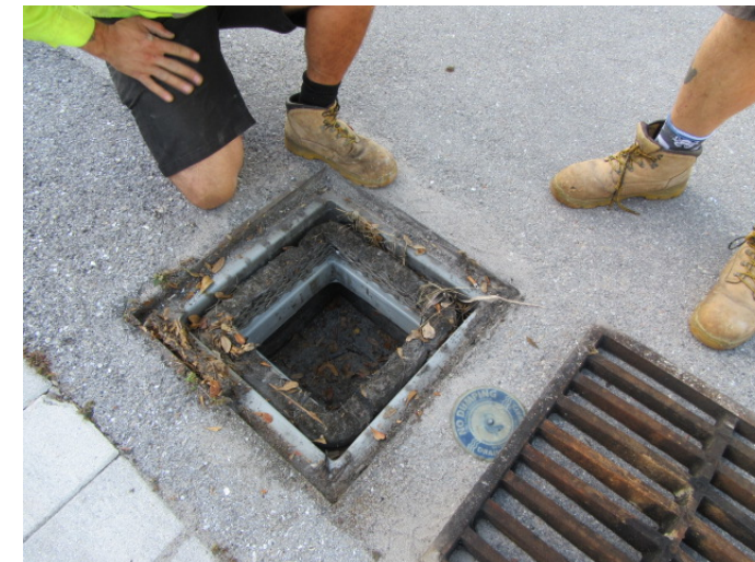
Source: Andy Holland, City of Naples Inlet Baskets Installed Near Lake Manor (6 th Ave Near 10 th St N)
