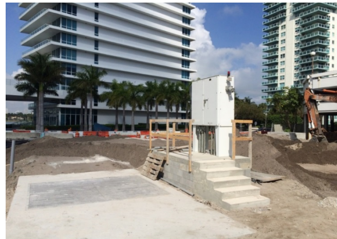
Typical Underground Pump Stations with Elevated Control Panel
