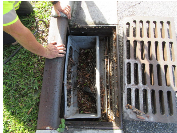
Source: Andy Holland, City of Naples Inlet Baskets Installed Near Lake Manor (6 th Ave Near 10 th St N)
