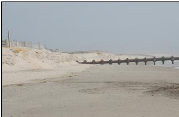
Photograph 1: Elevated outfall discharge in Avalon NY - in April 2011 - weather moderate storms and does not interrupt alongshore transport like a groin.
