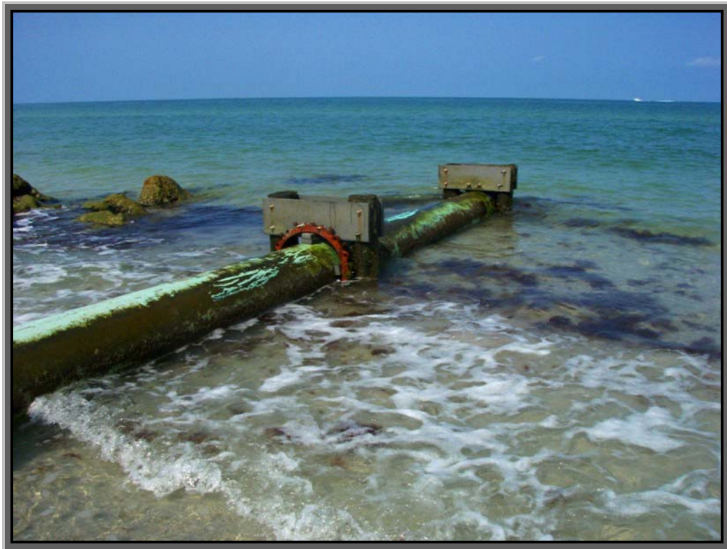
Figure 1 ~ Single 18-inch culvert- Outfall #3
