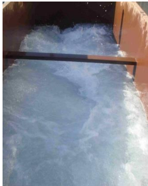
Inside View of Hopper Agitator
