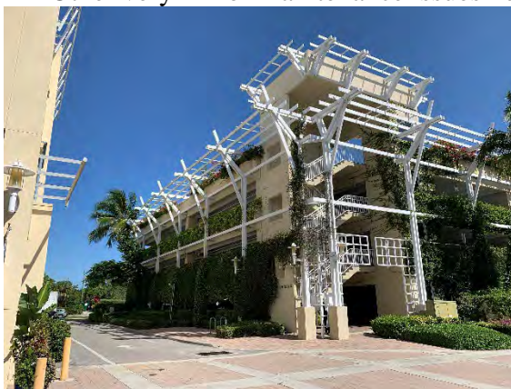
Photograph 1: Corner of Building
