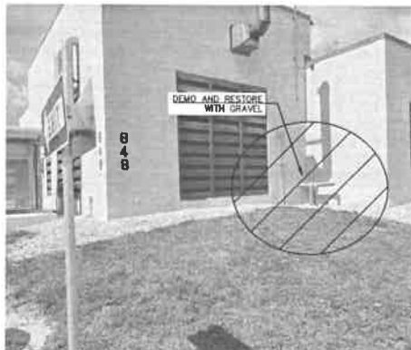
EX. DIESEL WELL GEN #1
