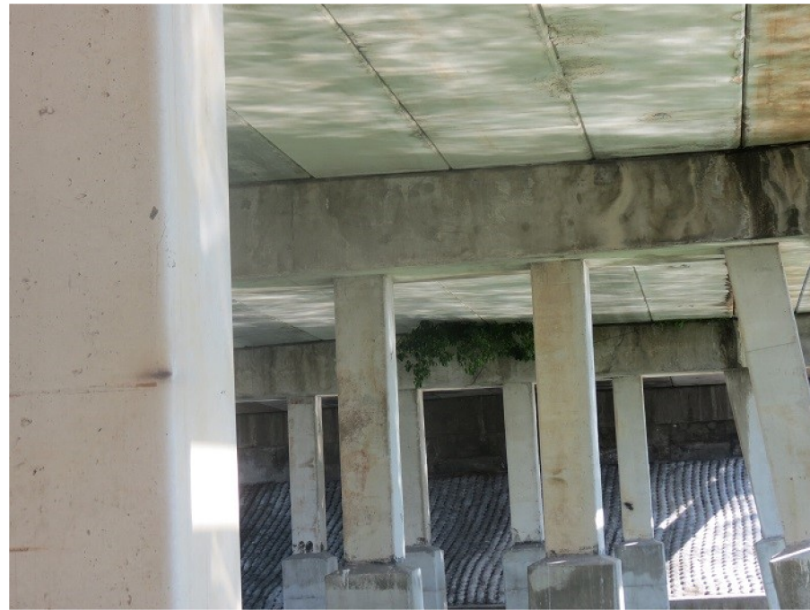
PHOTO 1 - VEGETATION AT BENT 4
