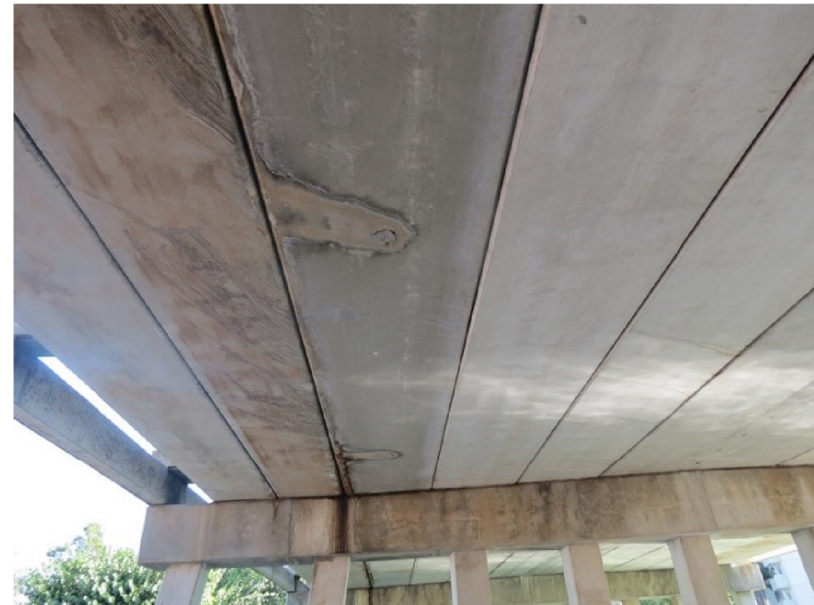
PHOTOS 14 - LOOSE PATCH FOR OLD PICK POINTS
