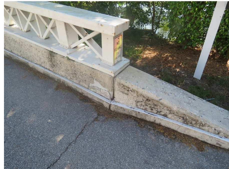
PHOTO 4 - EXISTING STUCCO FINISH ON BARRIERS
