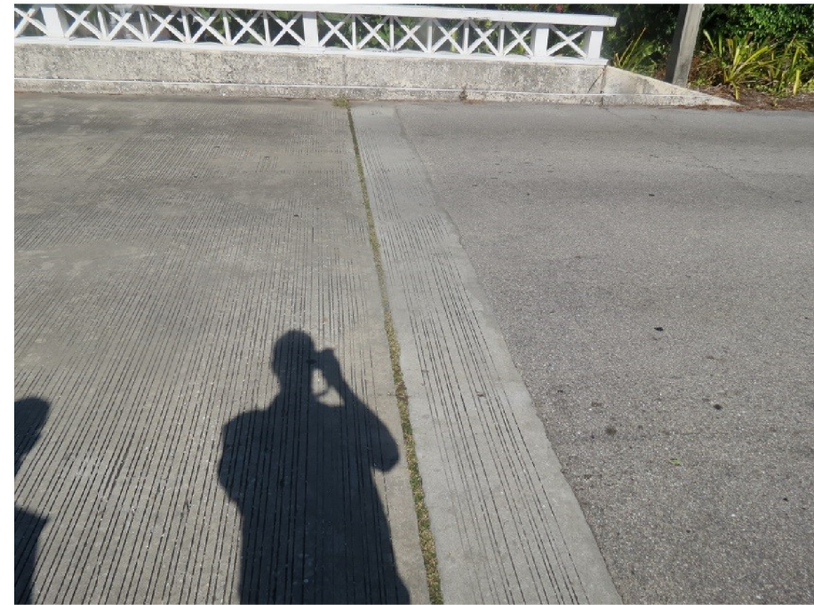
PHOTO 2 - EXPANSION JOINT AT END BENT 2
