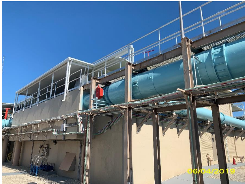
Existing interconnecting walkway/pipe support for Accelerator No. 3
