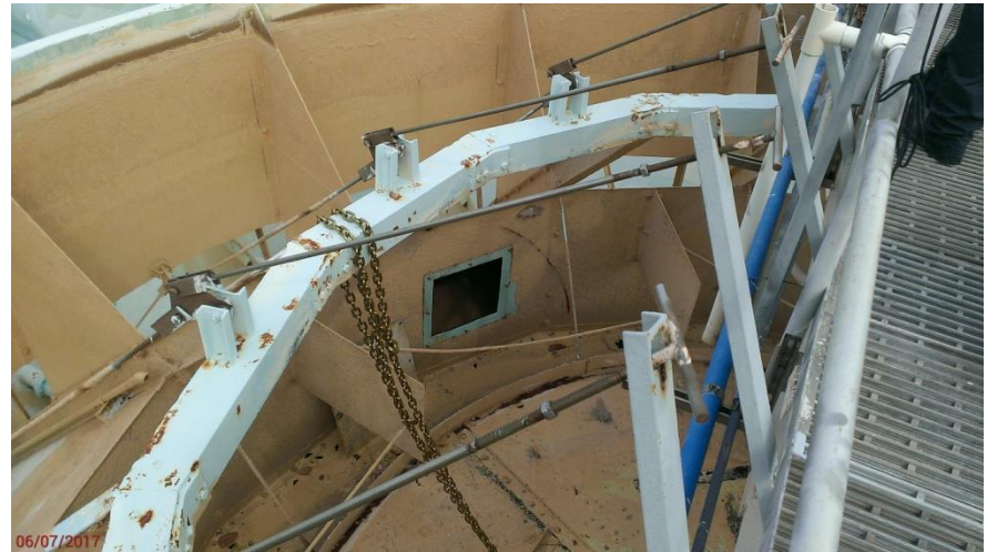
Support structure; impellor/rotor assembly below
