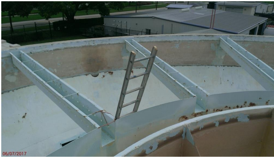
Radial launder with collection launder in foreground
