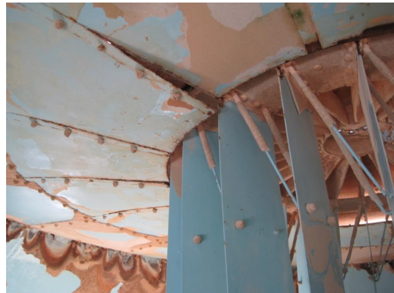
Deck plate assembly with impellor/rotor assembly
