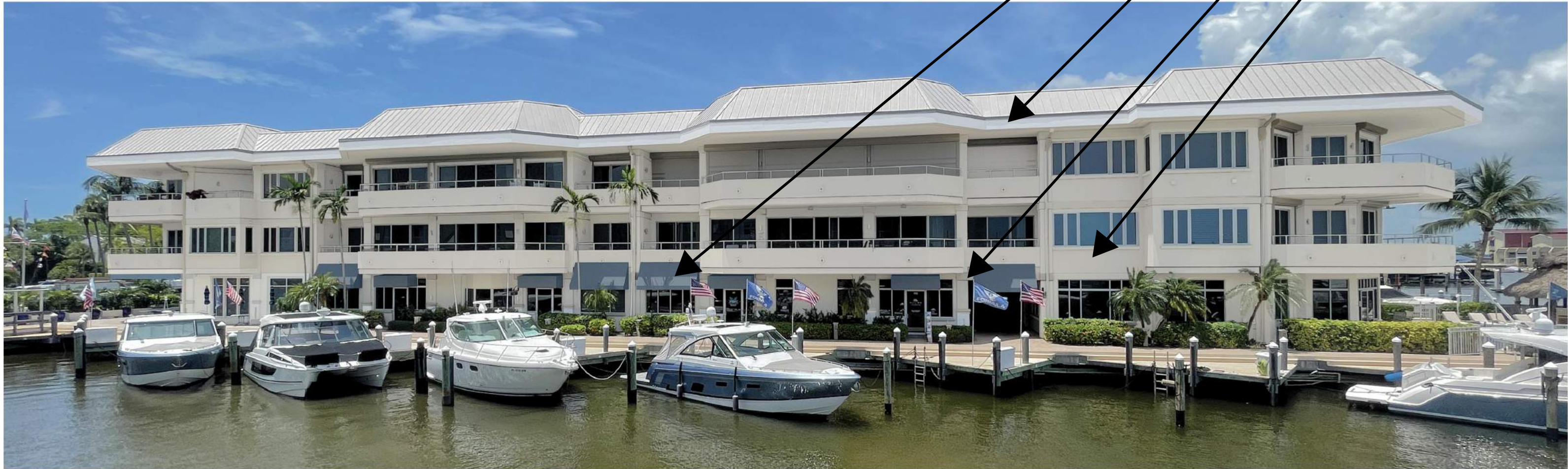
SOUTH FACADE - AFTER
