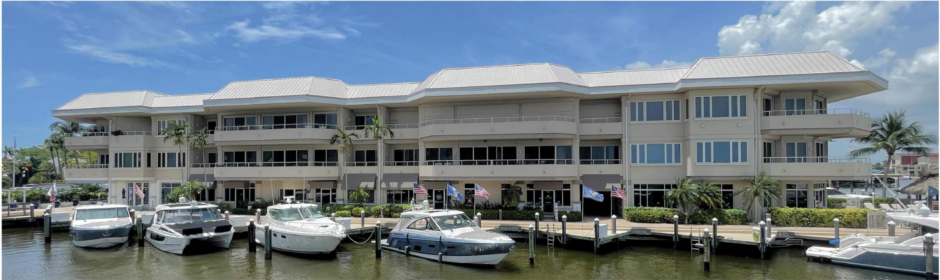
SOUTH FACADE - BEFORE
