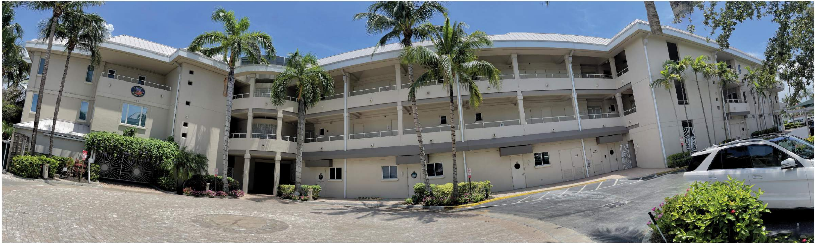
NORTH FACADE - BEFORE
