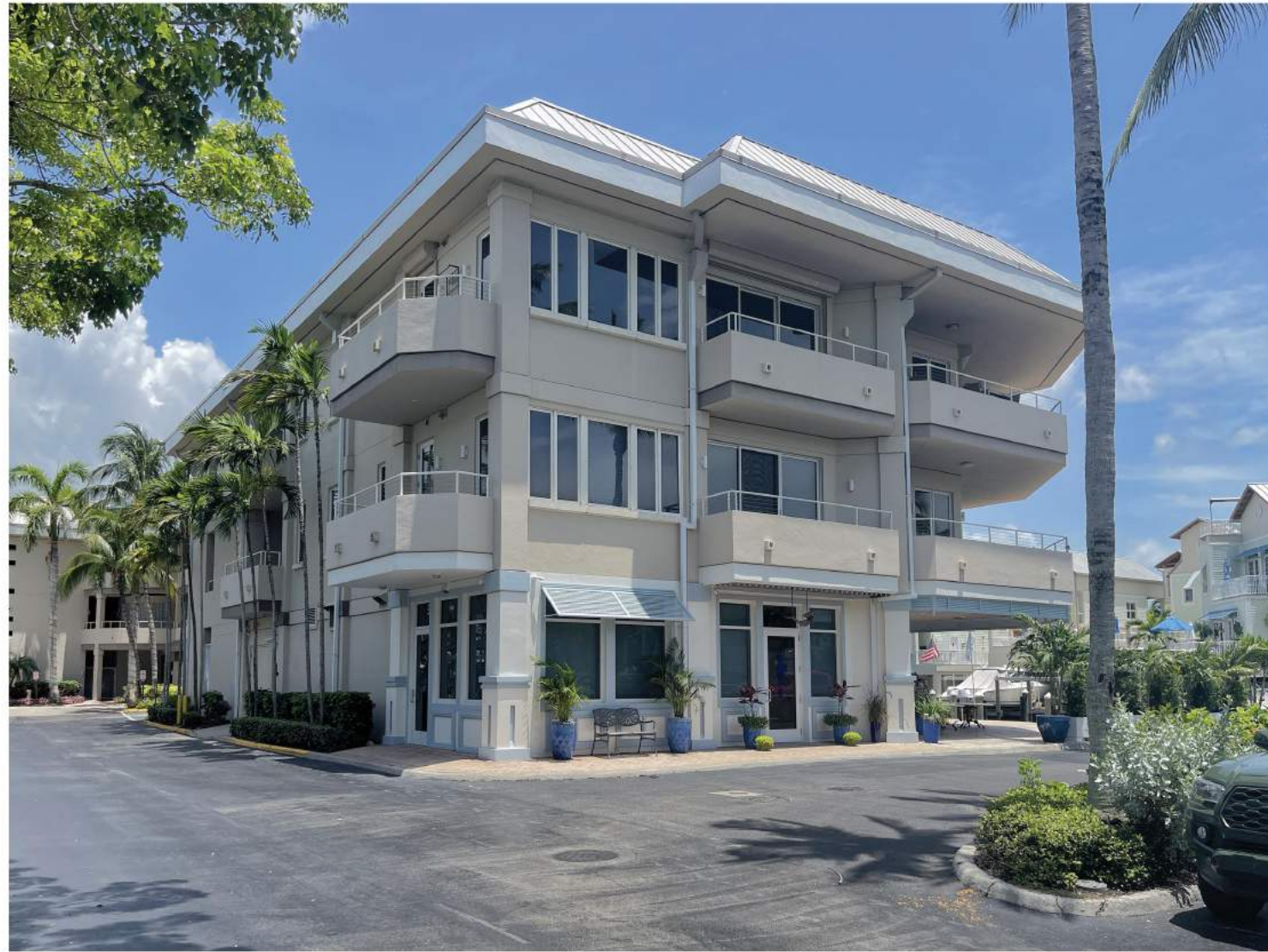
WEST FACADE - BEFORE
