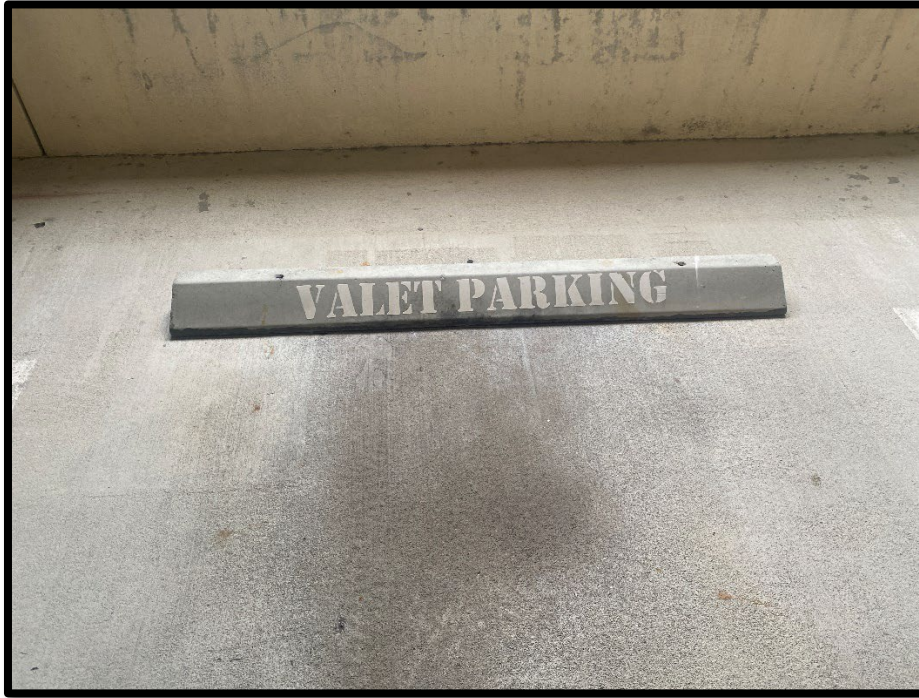
Figure 4: Designated valet parking spaces may be marked on the curb stops in the garage, as applicable.
