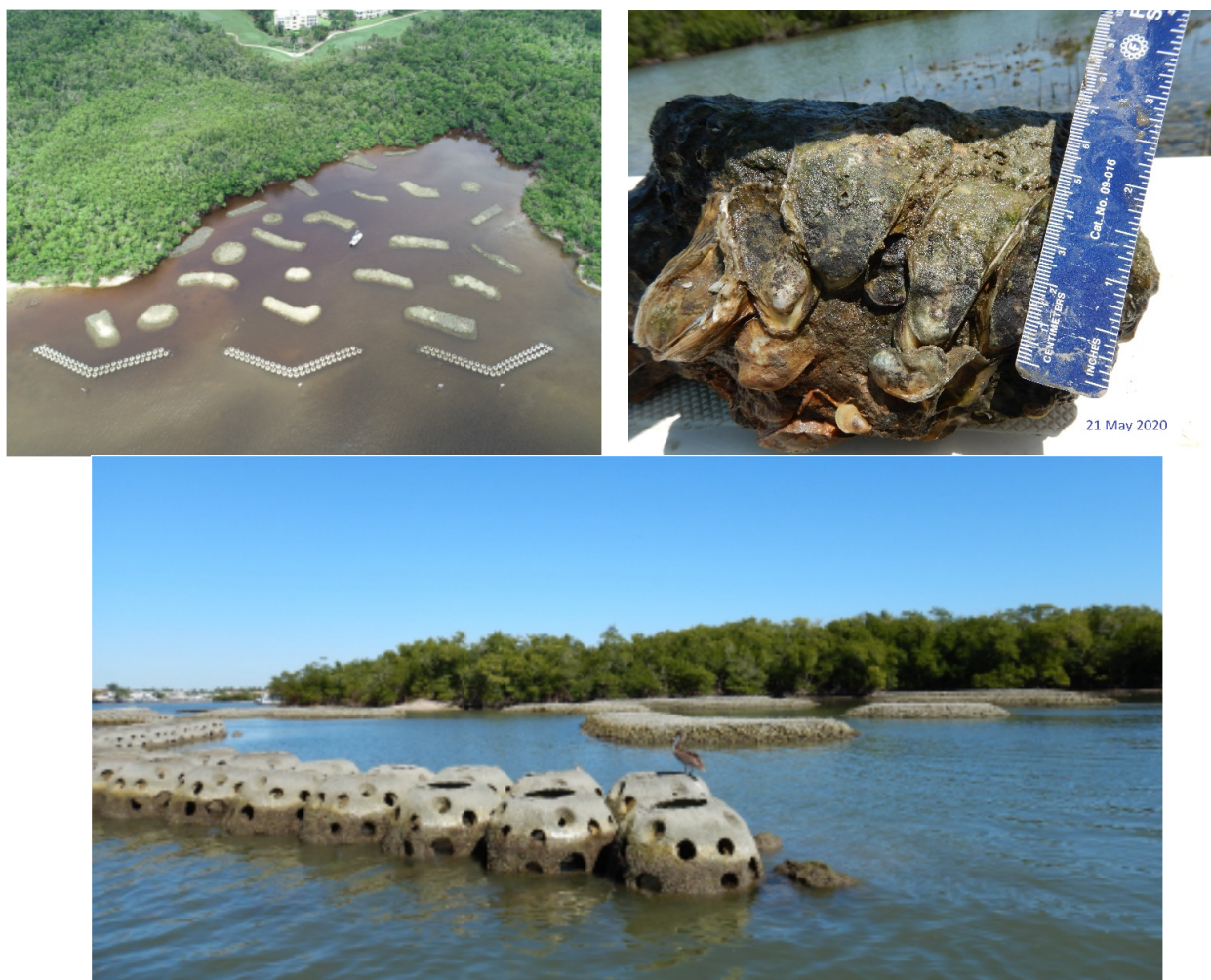
Figure 6. (Left-Top) Aerial view of the restoration site in Naples Bay, FL, USA that includes three chevron-shaped reefs constructed of Reef Balls™ (bottom of photograph), reefs constructed of loose, fossilized shell surrounded by a perimeter of large limestone rocks (closest to the Reef Ball™ structures), and reefs constructed of loose, fossilized shell with no rock perimeter (closest to mangrove shoreline). (Right-Top) Oyster recruitment on limestone rock after 12 months. (Bottom) Profile view of Reef Balls™ and limestone/loose shell reefs.
