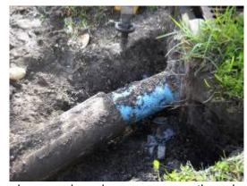
75% less expensive than replacing underground pipe. Lining is a non-invasive process, as there is minimal disruption to pavement, landscape and traffic. Cured in place pipe lining creates a new inner load-bearing pipe, which is independent of the old host pipe, and remains fully functional in the eventuality of the old pipe deteriorating completely. The lining can be applied in any material and shape pipe.
