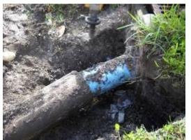
new inner load-bearing pipe, which is independent of the old host pipe, and remains fully functional in the eventuality of the old pipe deteriorating completely. The lining can be applied in any material and shape pipe. This CIP programs \$200,000 in each of the next 4-years to line deteriorated pipe throughout the City.
